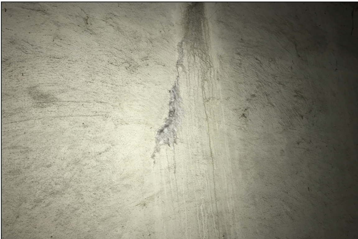
abutment at Bent 2 between girders 2 and 3, crack with efflorescence.
