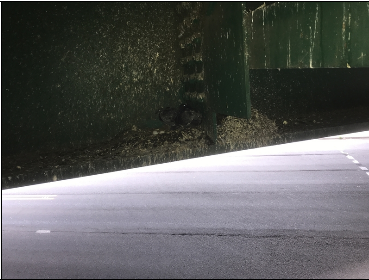
Bird feces on girder ends and at stiffeners
