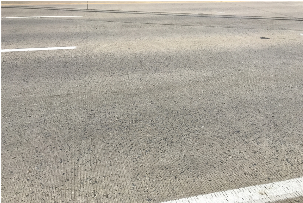
deck has large transverse cracks up to .040"
