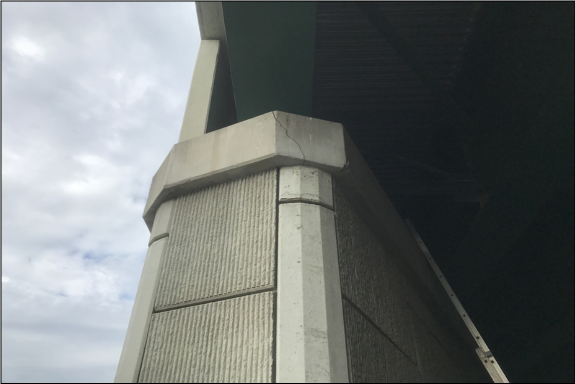
Crack in MSE wall at south west end
