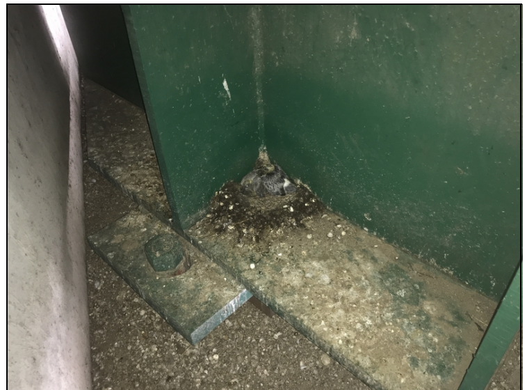
Bent 2 Girder 5, nest on bottom flange.
