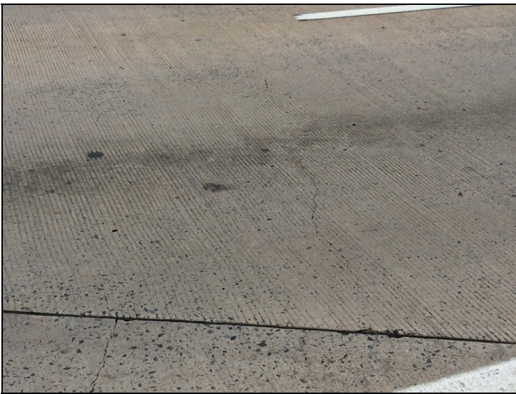
Deck at Bent 1cracks up to 0.040"
