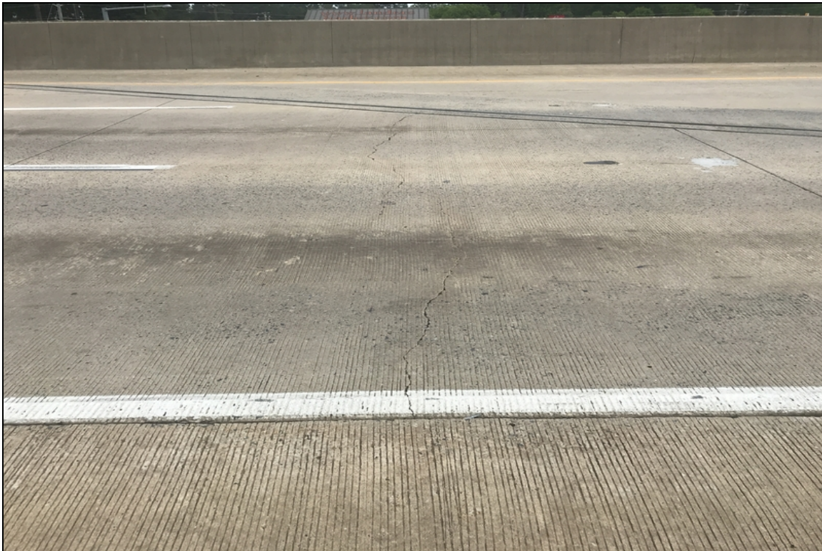
approach slabs have large tranverse and longitudinal cracks
