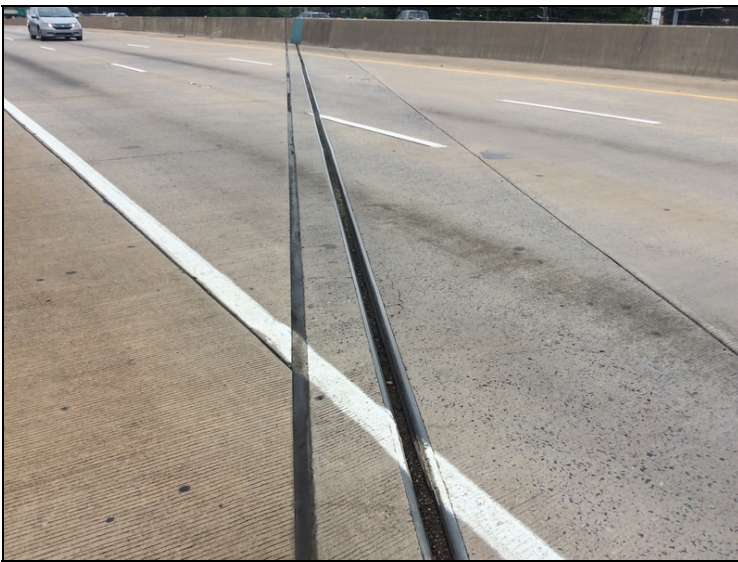
Bent 1 joint seal half full of debris
