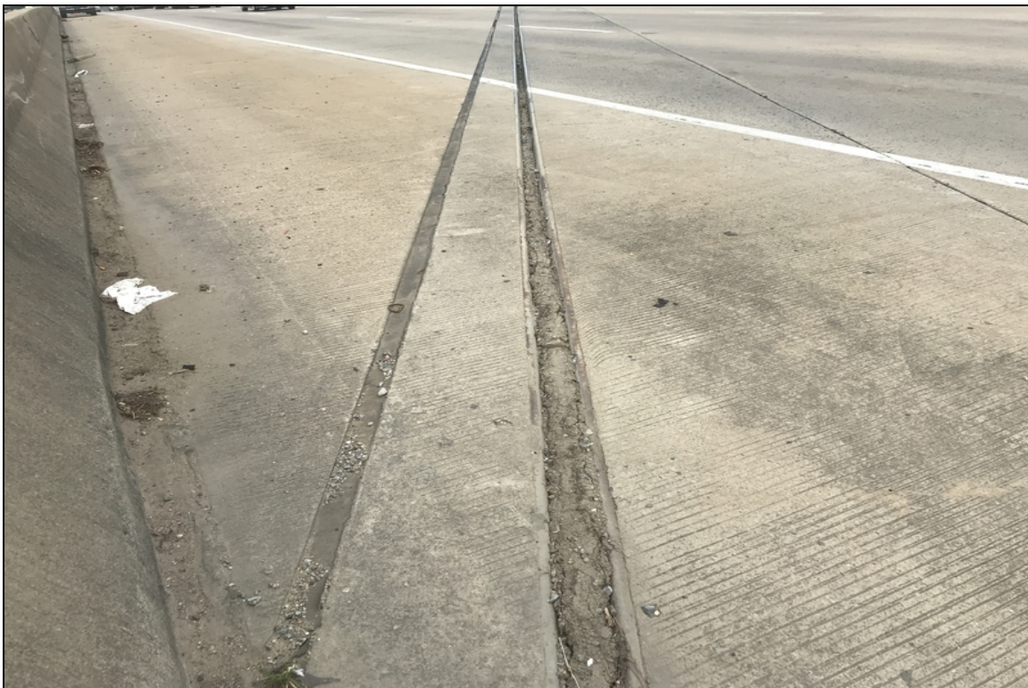
Joint at bent 1 is full of debris
