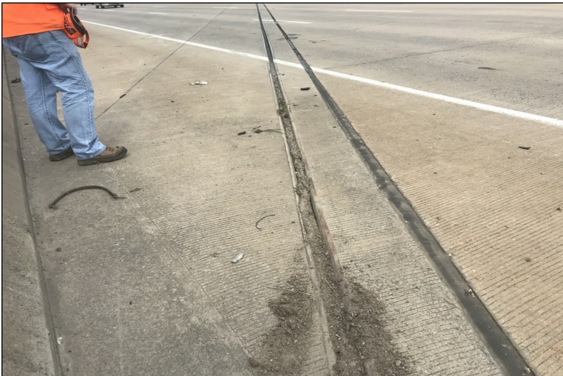
Joint at bent 2 are full of debris
