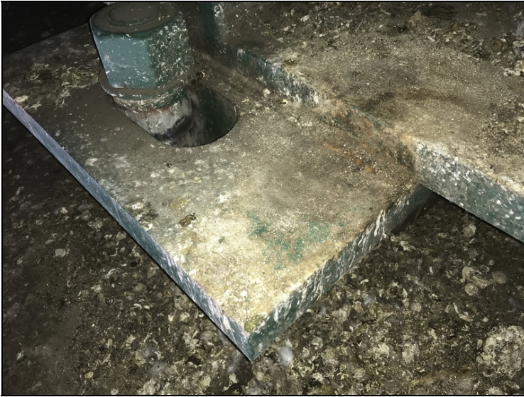
droppings around sole plate causing rust to form
