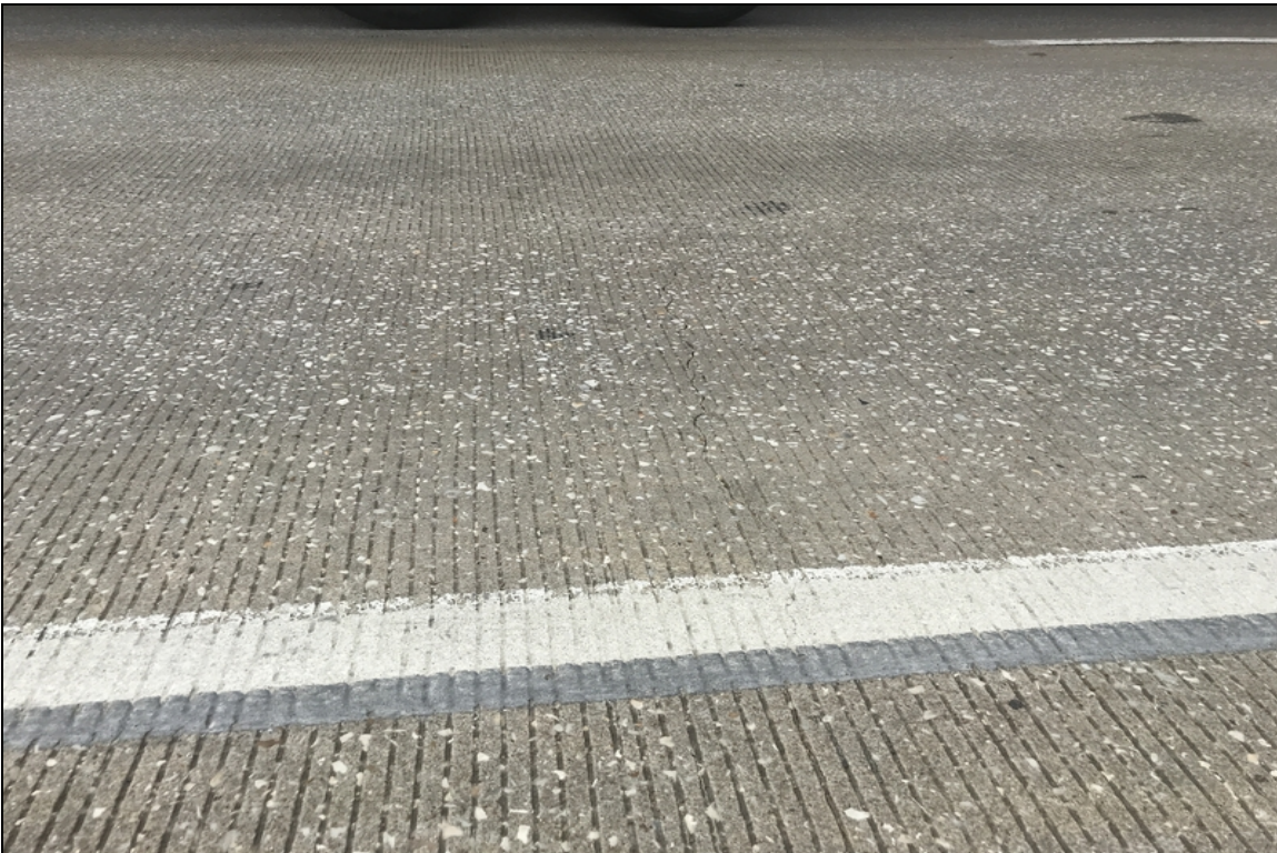
Deck has large transverse cracks up to .040"
