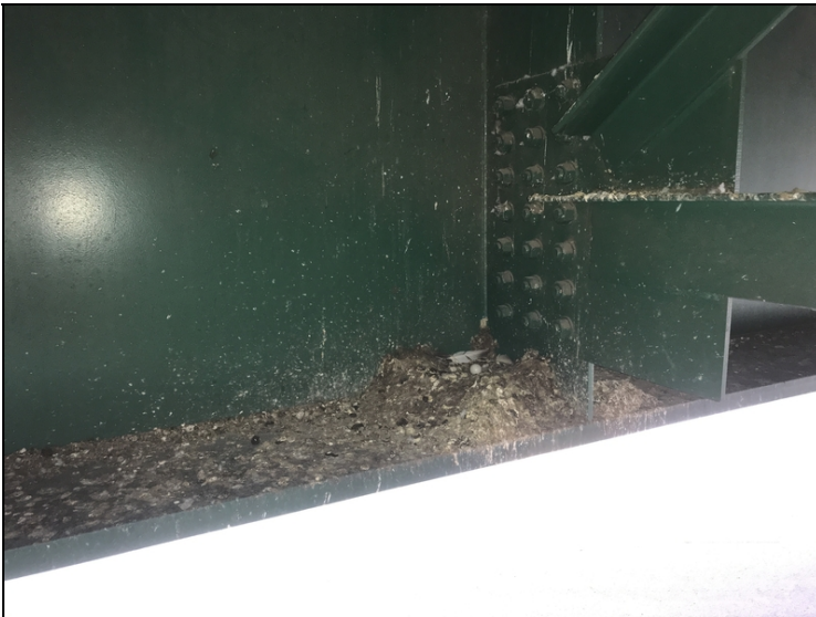
Large deposits of bird feces at beam ends
