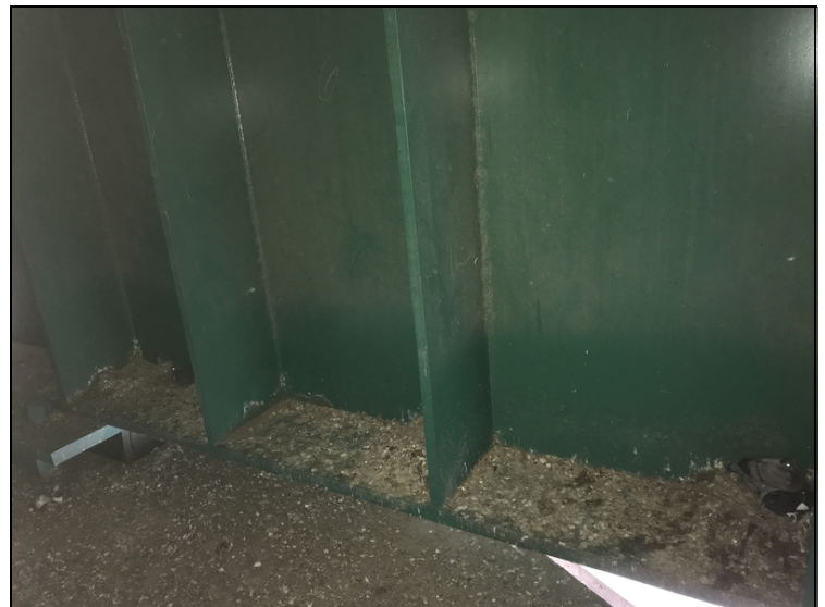
Bent 2 girder 6, bird nests on bottom flange, typical.
