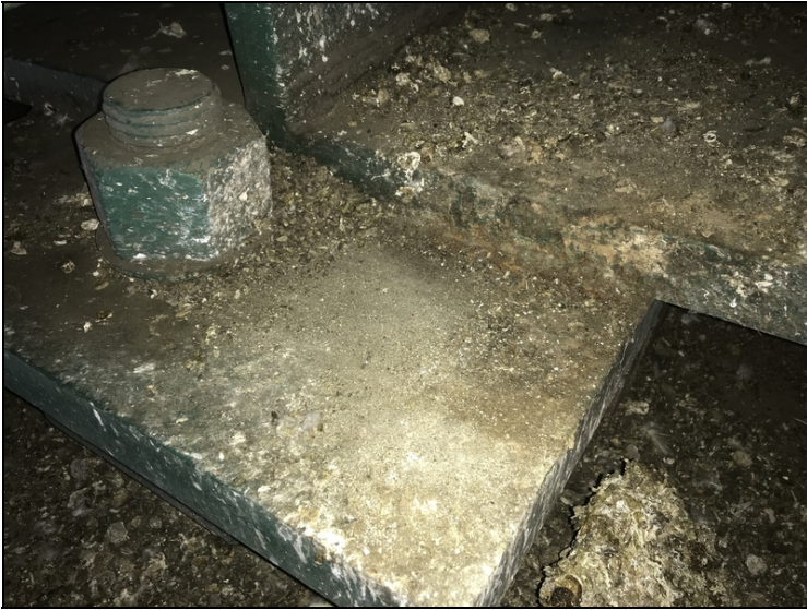
Bent 2 bearing 2 has piles of bird feces around sole plate
