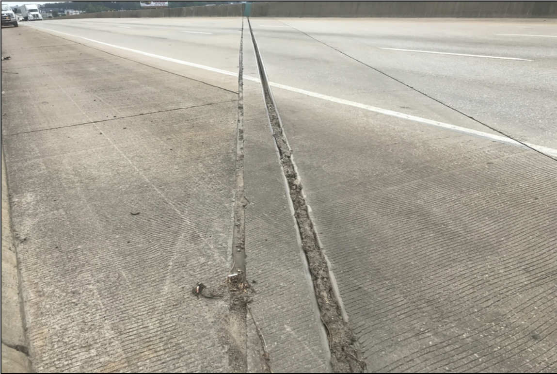
Joint at bent 2 has debris impactation on shoulder
