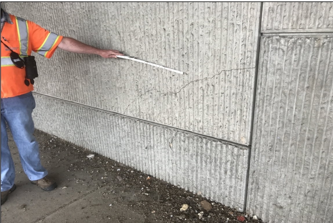
Cracks in MSE wall at bent 1 between girder 4 and 5 traffic impact
