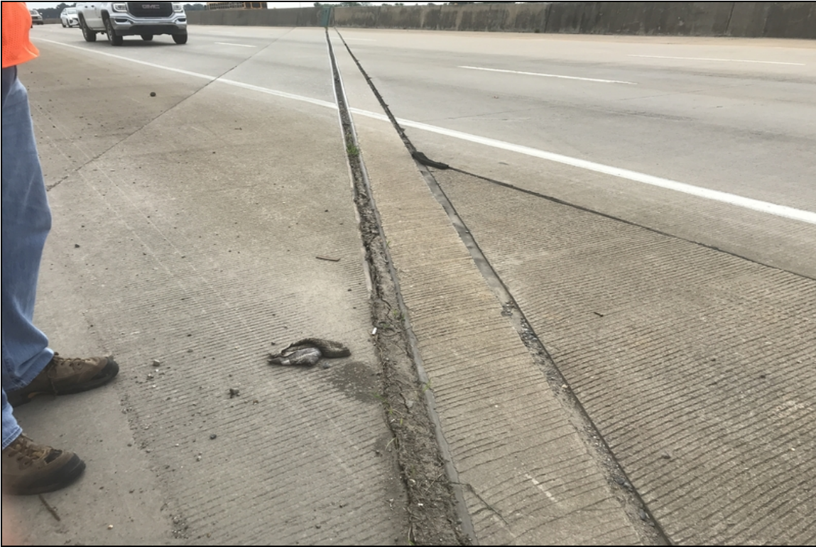
Joint at bent 1 has debris impactation on shoulder and 10' of torn and leaking joint in right hand lane
