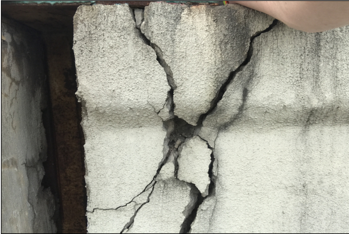
North side at bent 2 parapet wall has large cracks and spalls from traffic impact
