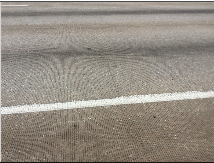
Cracks in deck up to 0.040"
