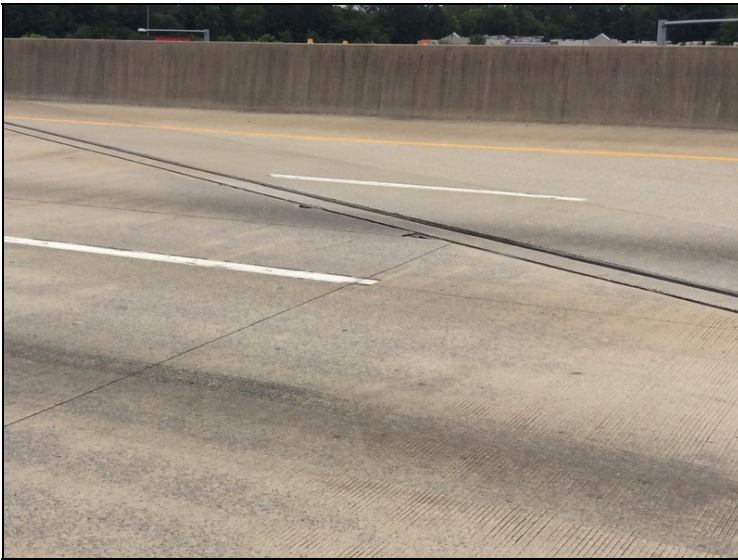
Small spalls in approach slab at bent 2
