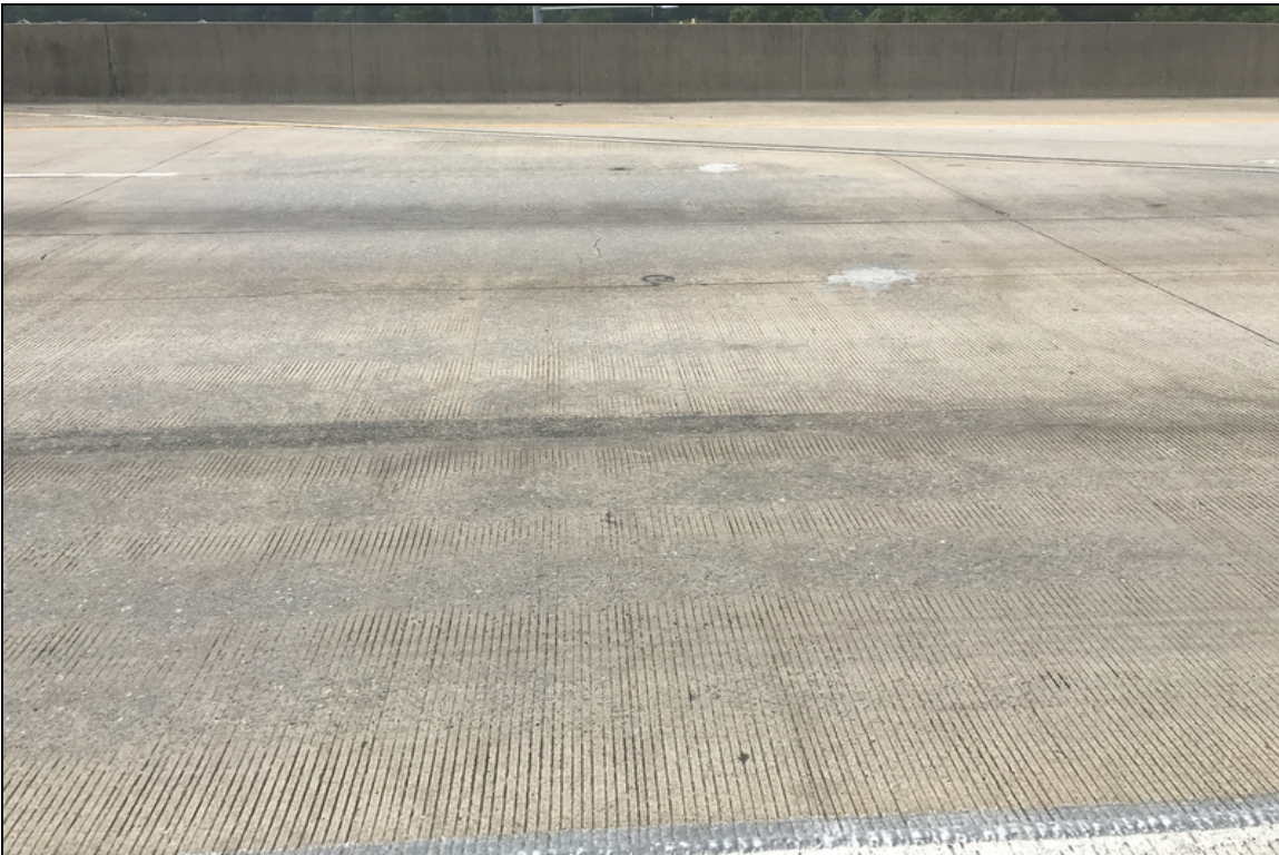
Large Transverse cracks up to .040" in the approach slabs
