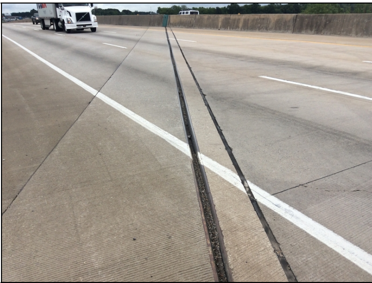
Joints are half full of debris
