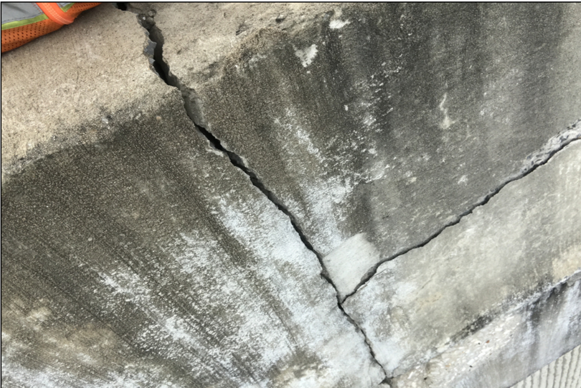
Large delamination in the parapet wall on the north side at bent 1
