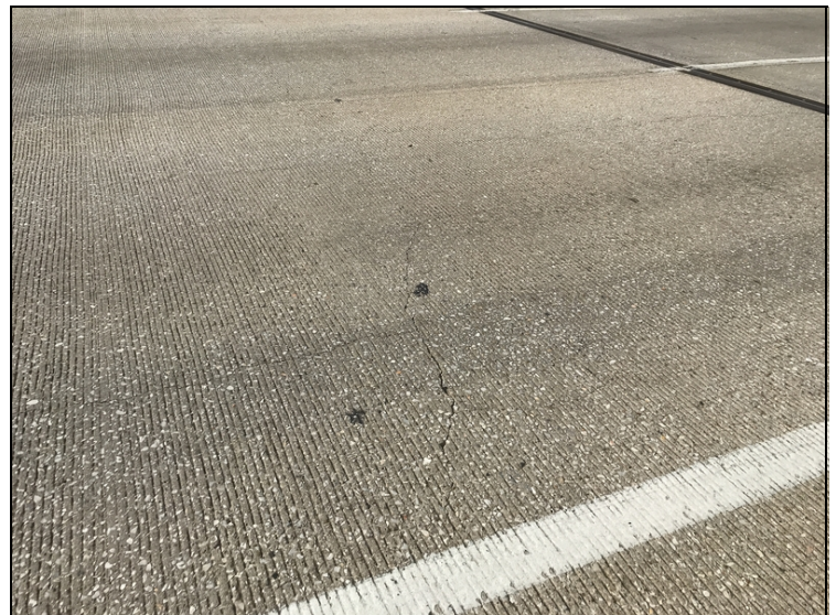
Span 1, large transverse crack.
