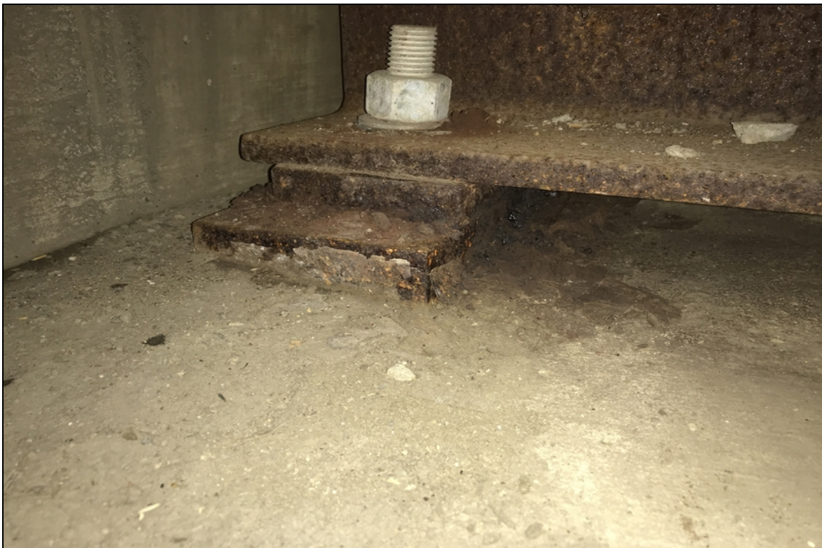
Bent 1 bearing 4, corrosion.
