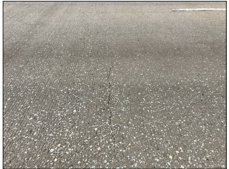
Span 5, large transverse crack.
