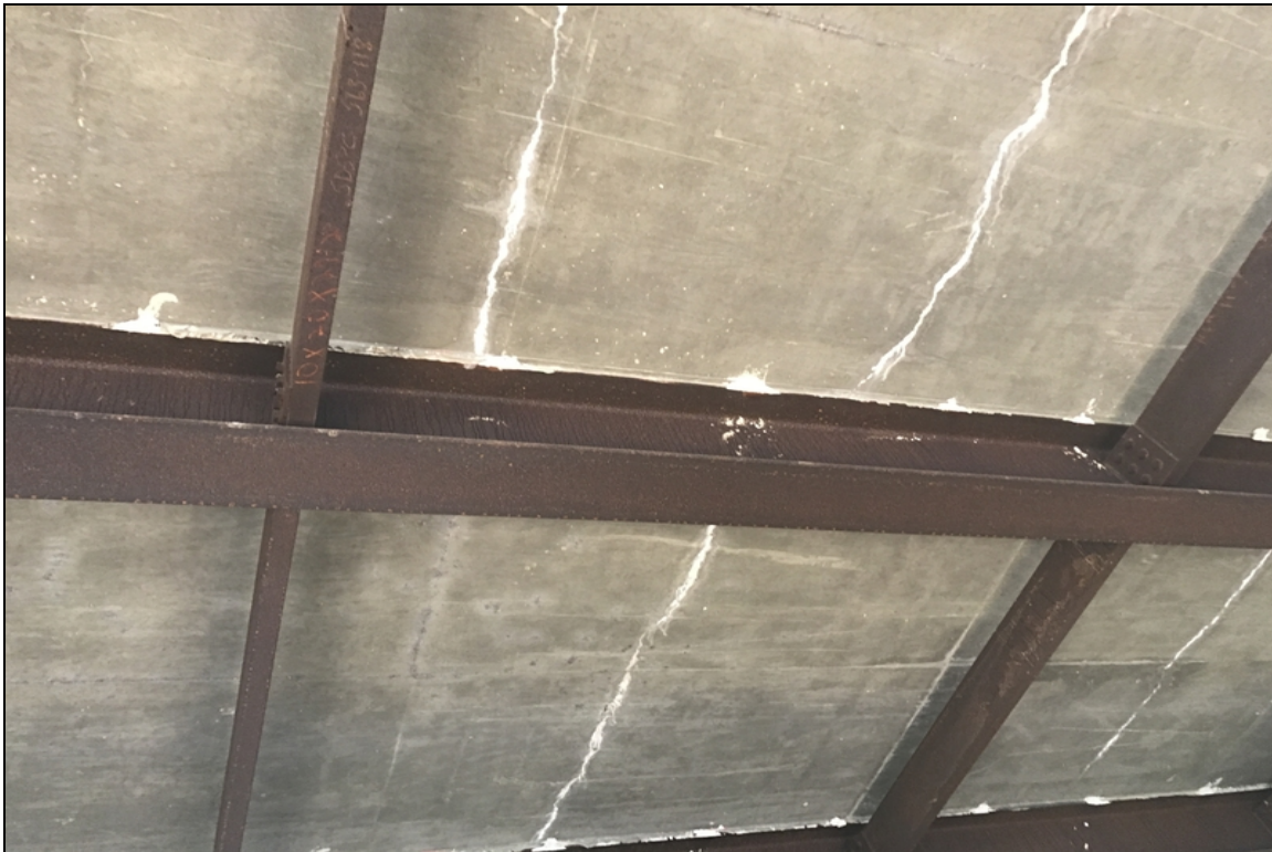
Span 4, cracks with efflorescence, typical.
