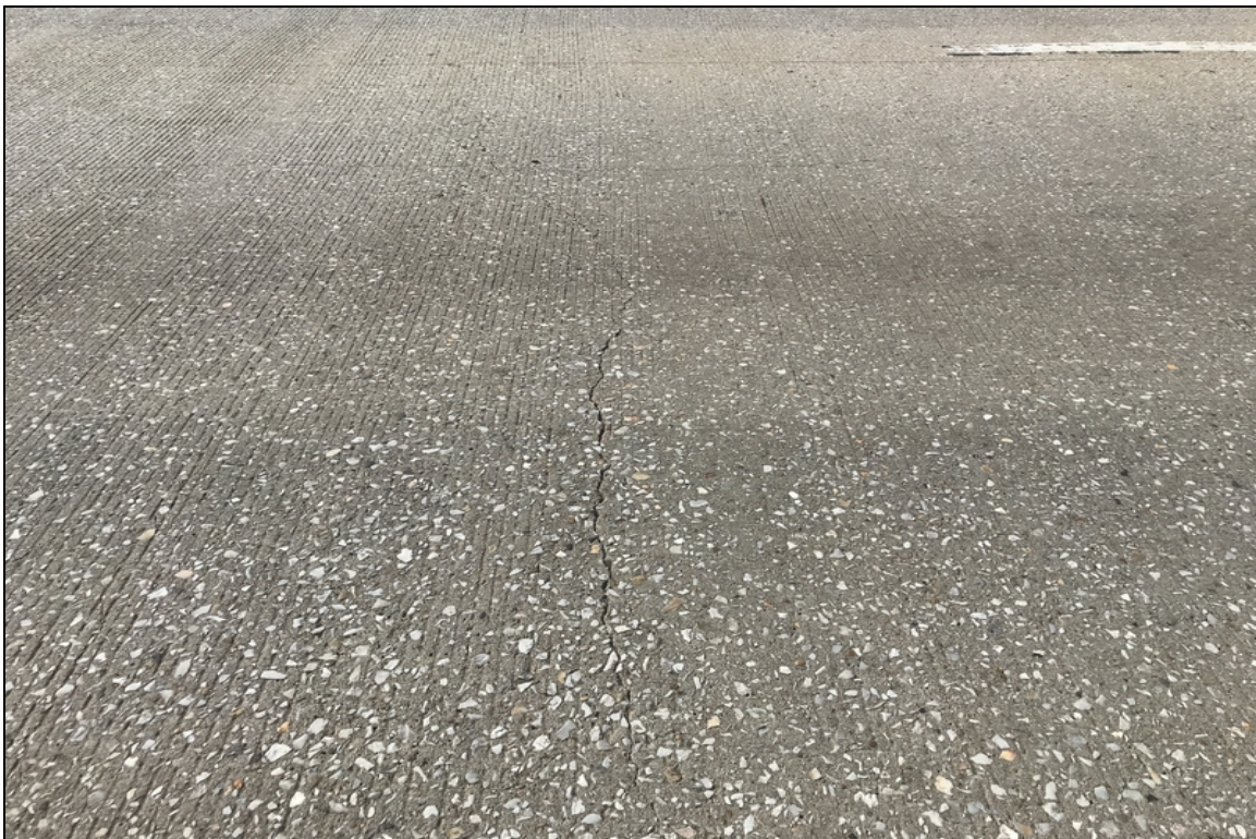
Span 5, large transverse crack.
