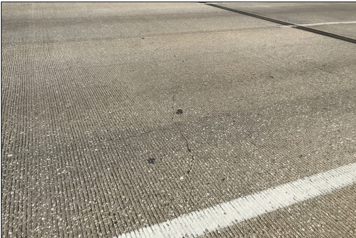
Span 1, large transverse crack.
