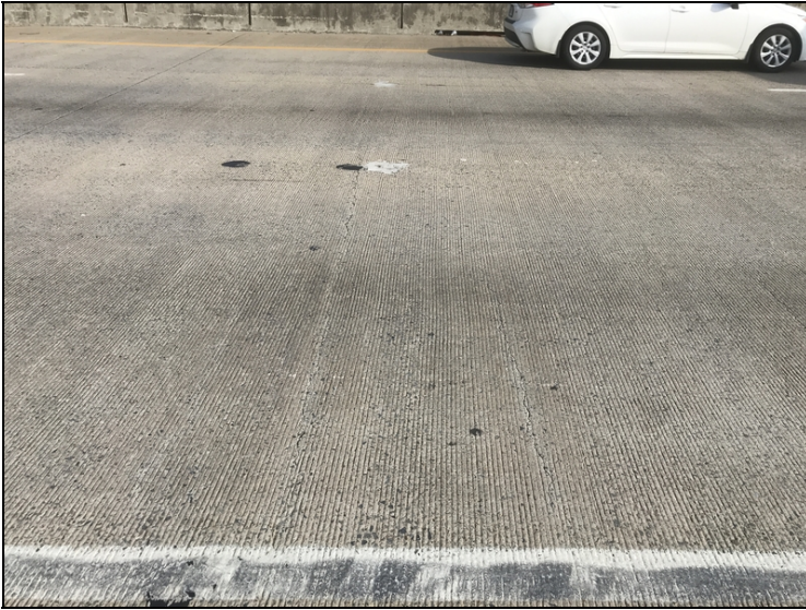
Span 2, large transverse cracks.
