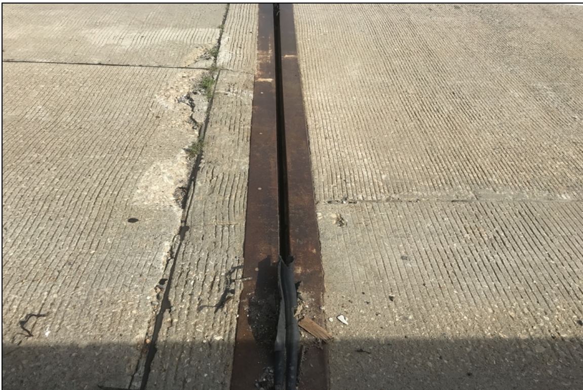
Bent 1 right side, missing joint seal.
