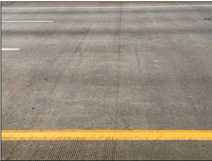
Span 5 unsealed cracks up to 1/8"
