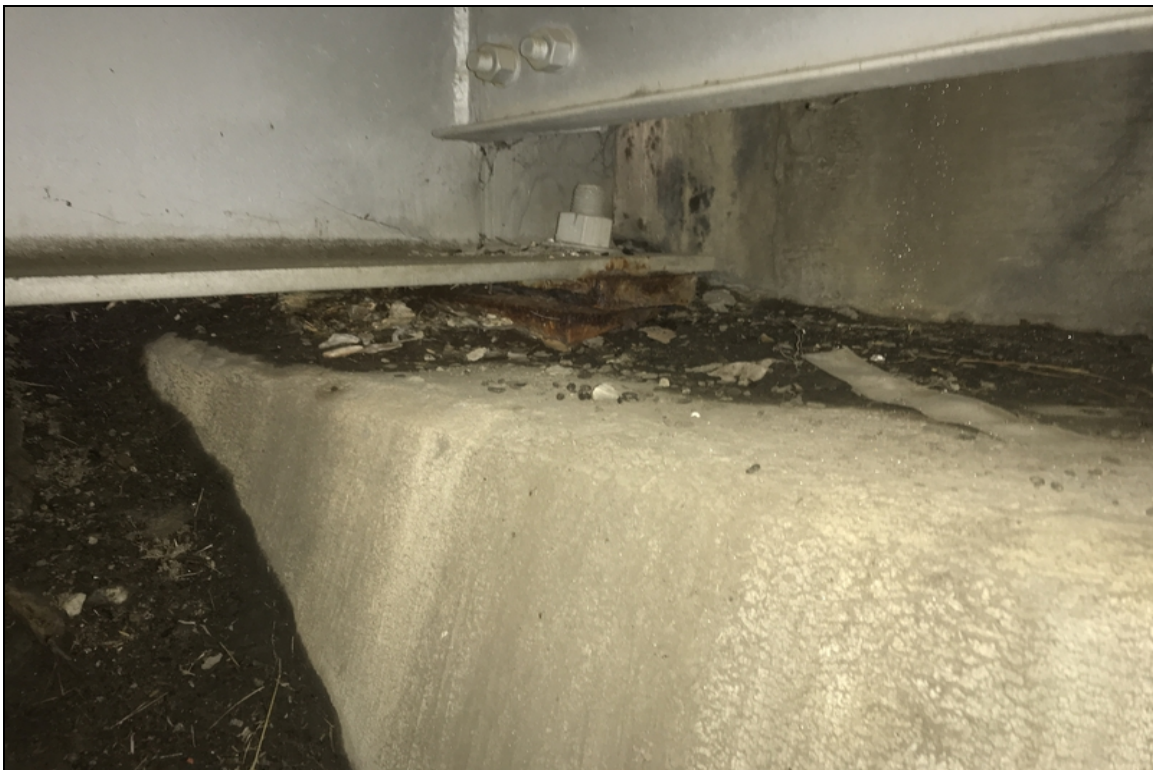
Bent 6 bearing 1, debris around bearing.
