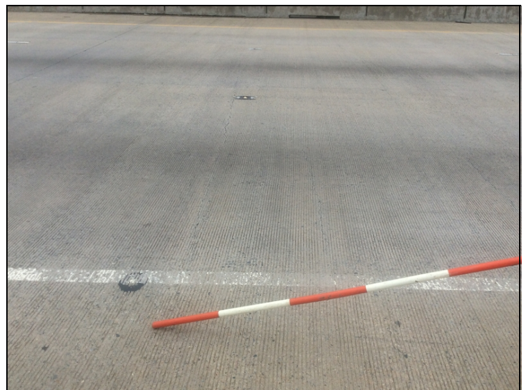
Span 2 large unsealed cracks up to 1/8" on 3 to 4 foot spacing. Common all spans.
