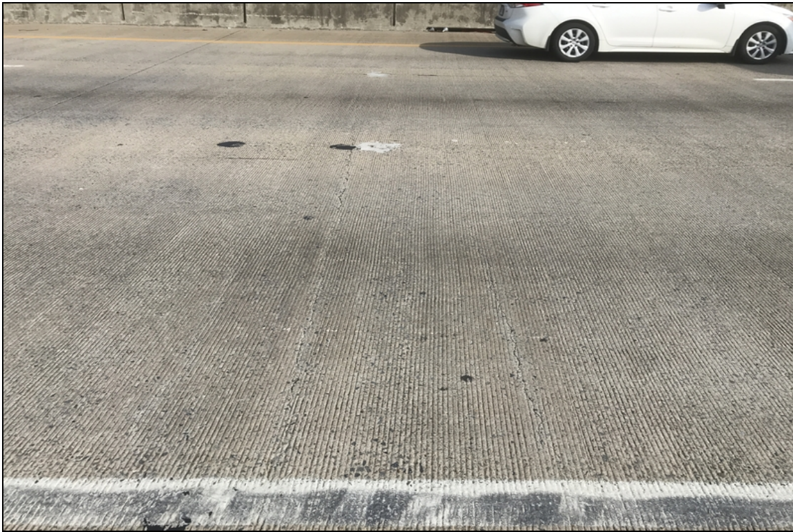
Span 2, large transverse cracks.
