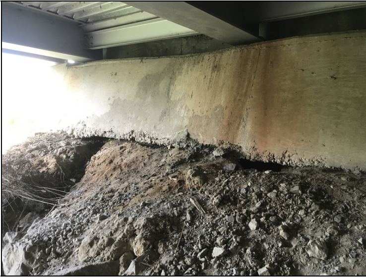
Bent 1, erosion under the abutment exposing pile between beams 7 and 8.
