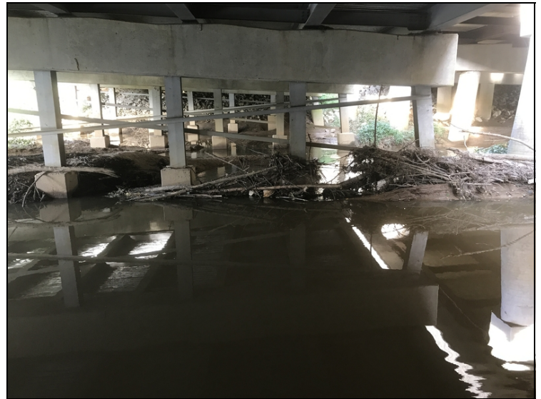
Bent 4, debris buildup around piling.
