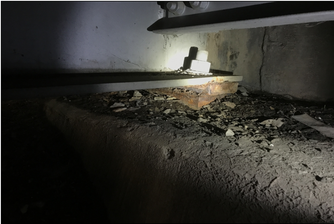
Bent 6 bearing 1, corrosion.
