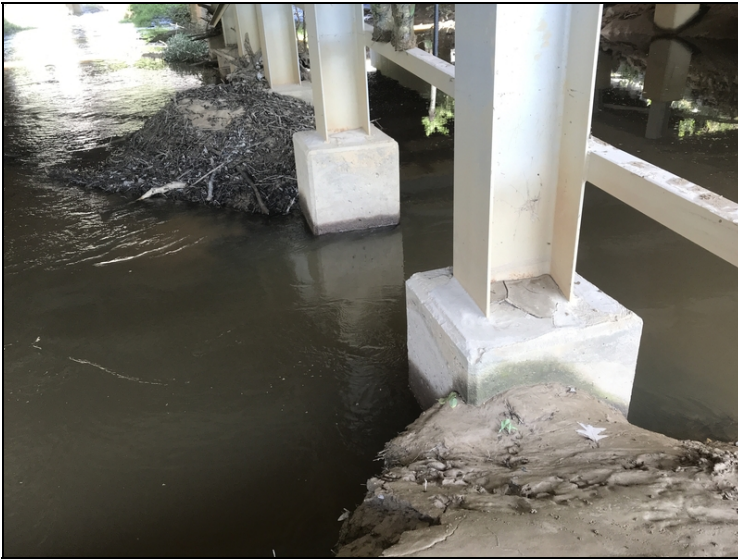
Bent 4 Pile at top of encasement has dirt and silt causing rust to form.
