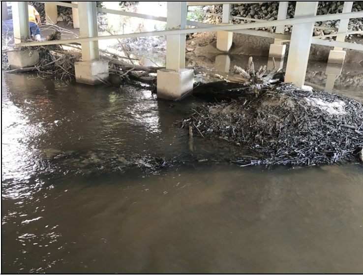
Bent 4 logs and debris restricting water flow
