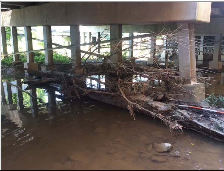
Bent 4: large trees laying against piling
