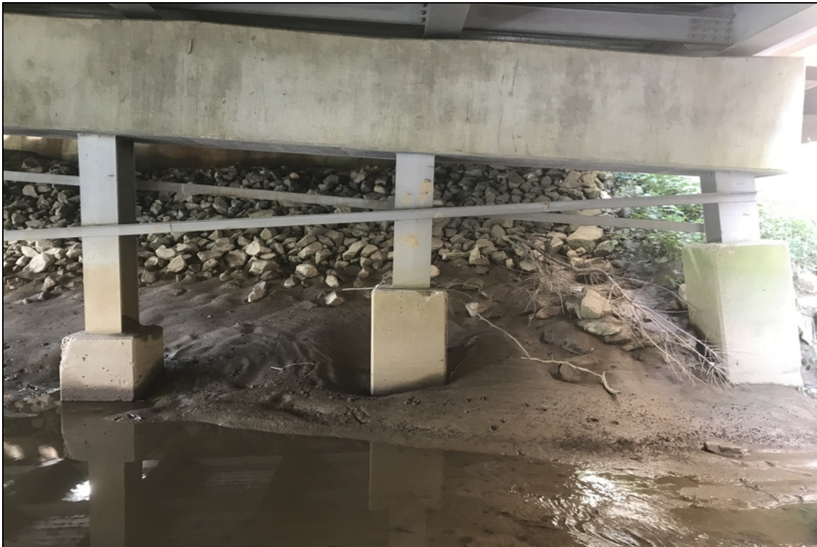
Bent 2, piles 1-3, spalls on concrete encasement.
