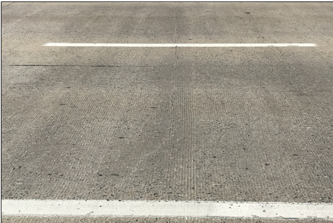
Span 4, large transverse crack.
