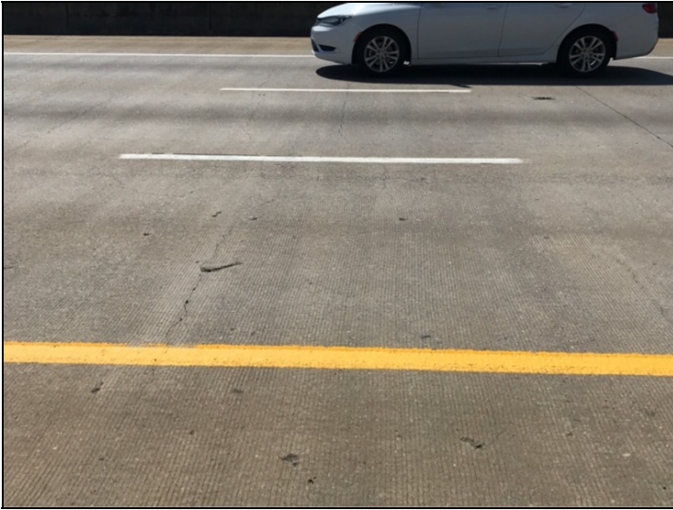
Span 4 unsealed cracks up to 1/8"
