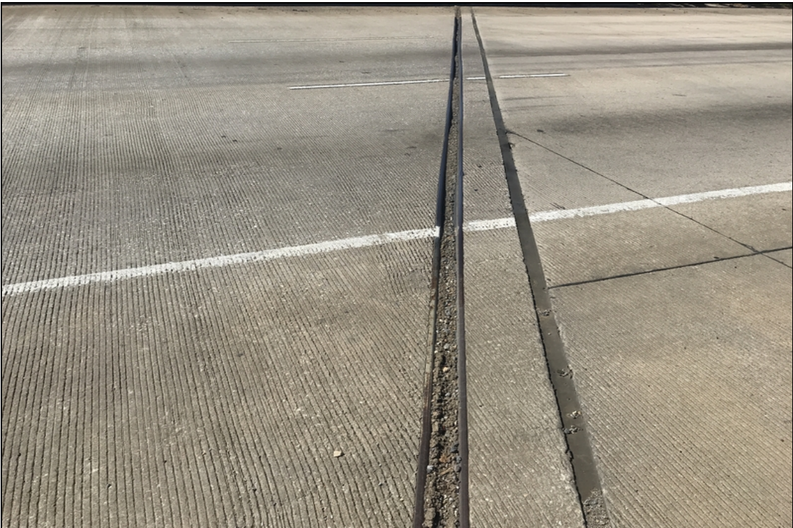
Bt. 1, joint full of debris.
