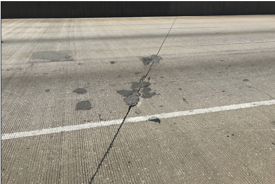
Spalls filled with asphalt over Bt. 3.
