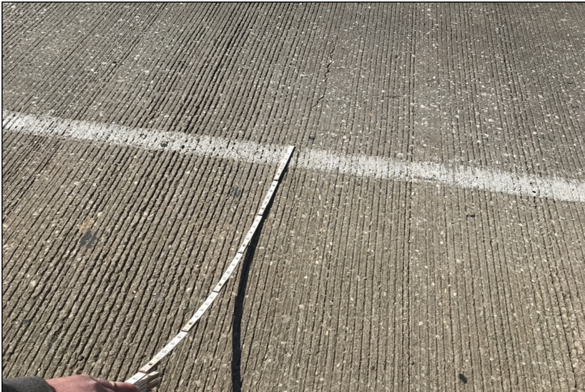
Deck cracking up to 0.030".
