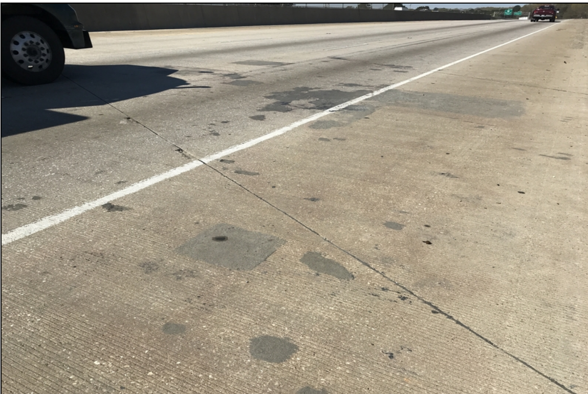
Span 3, spalls patched with epoxy & asphalt.
