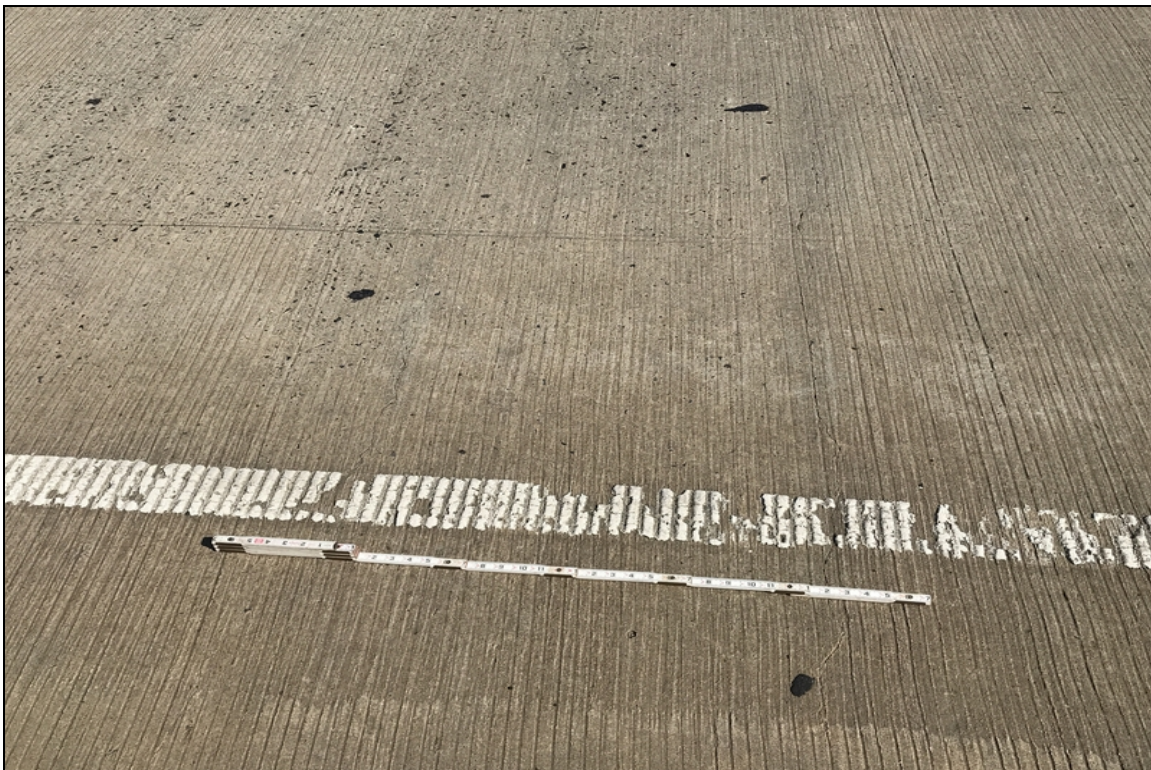
Deck cracking up to 0.020".
