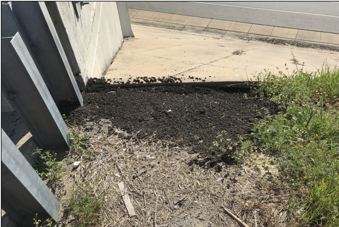
Asphalt has been place to repair erosion under slope pavement at Bt. 1.
