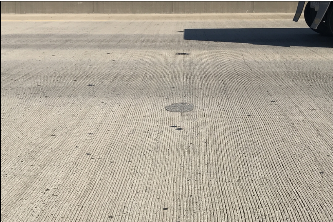
Spall filled with asphalt.
