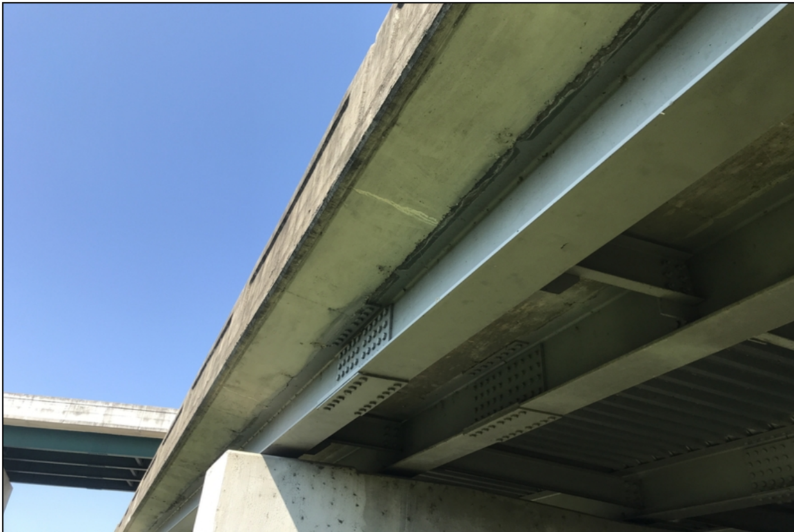
Crack with efflorescence on overhang
