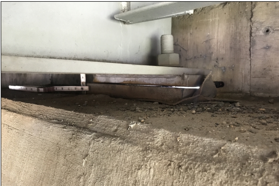
Bent 6 bearing 6 bearing is floating, causing the sole and masonry plates to collide against each other.
