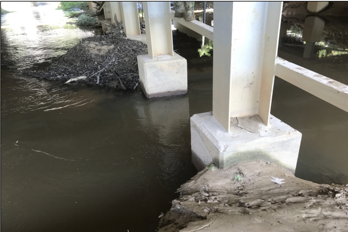
Bent 4 Pile at top of encasement has dirt and silt causing rust to form.
