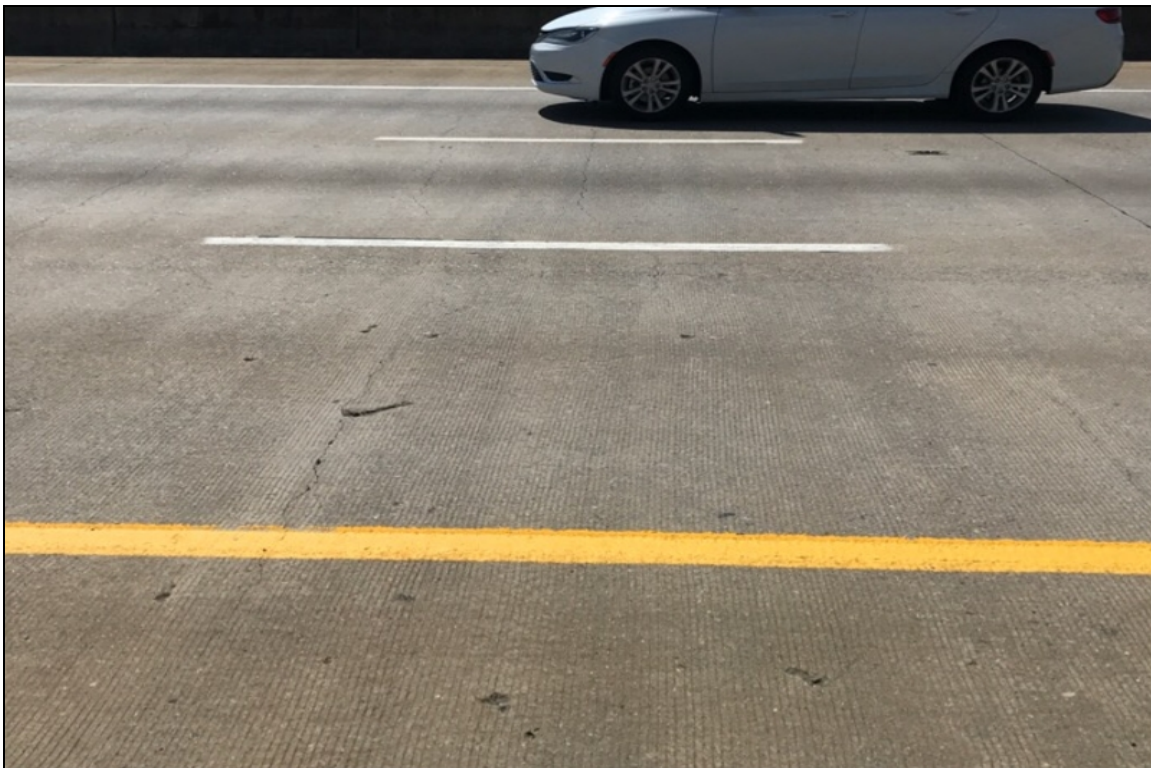
Span 4 unsealed cracks up to 1/8"
