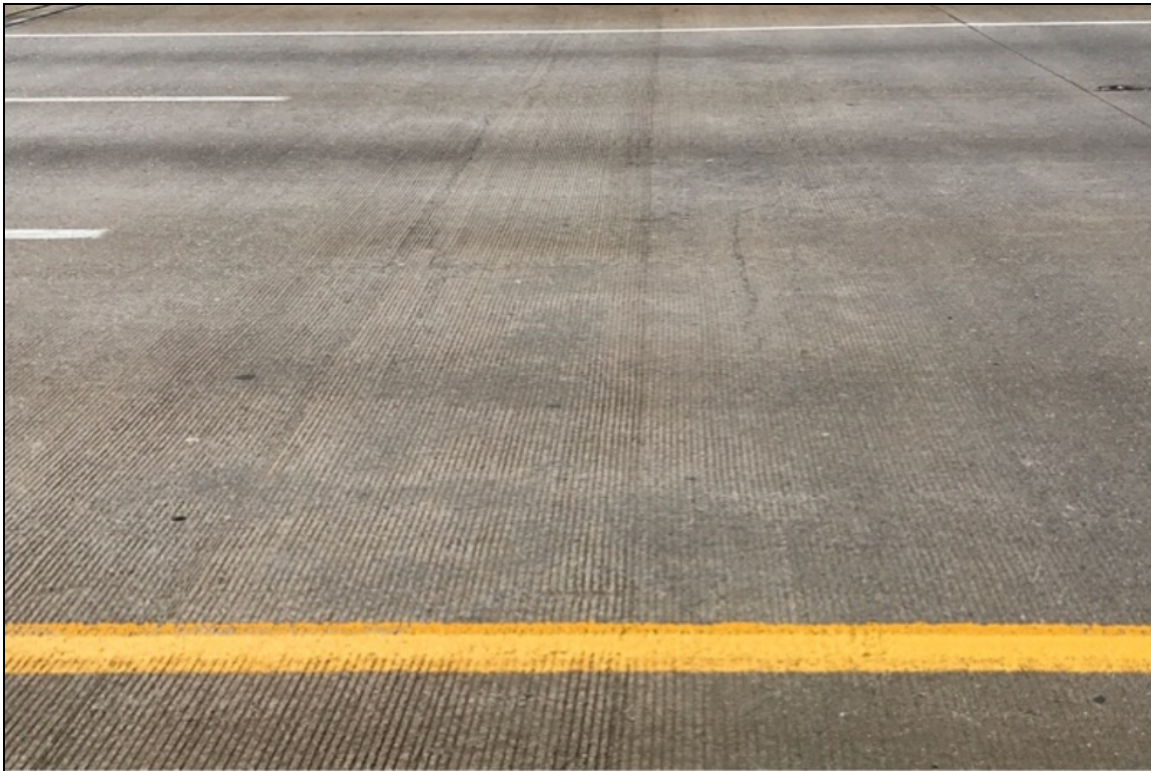
Span 5 unsealed cracks up to 1/8"
