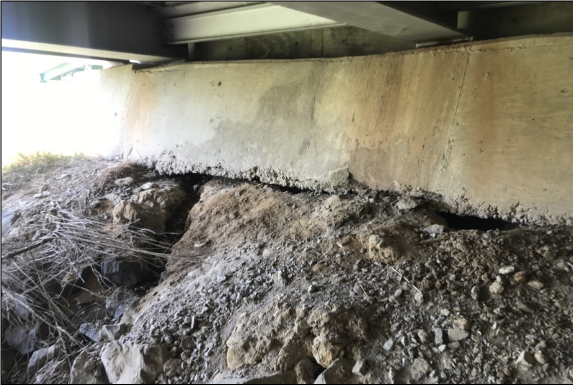
Bent 1, between girders 7 & 8: material is being eroded from under the beam seat exposing piling.
