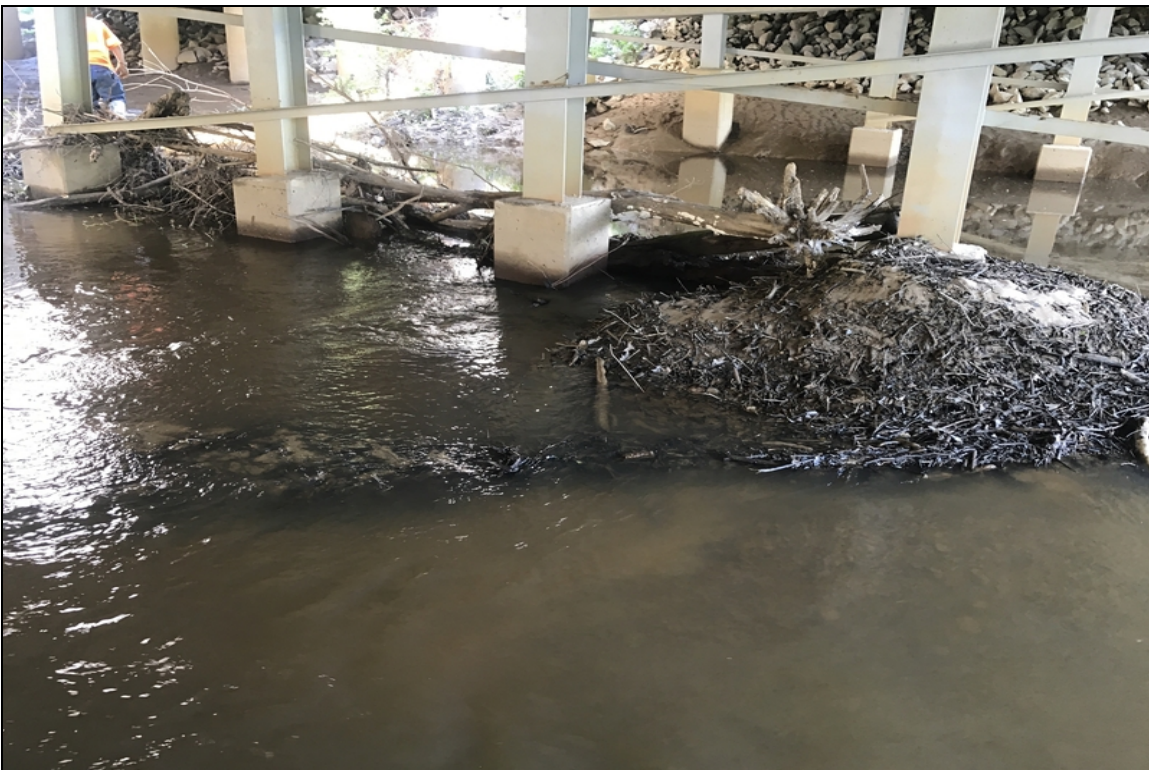
Bent 4 logs and debris restricting water flow
