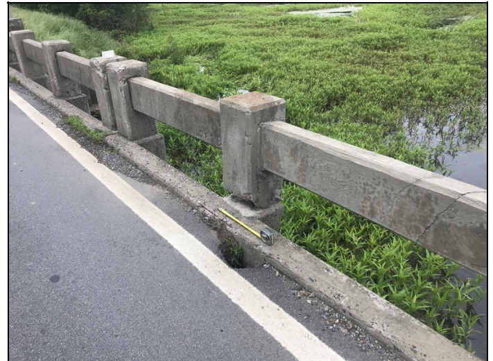
Right bridge rail in spans 3&4 have broken post.
