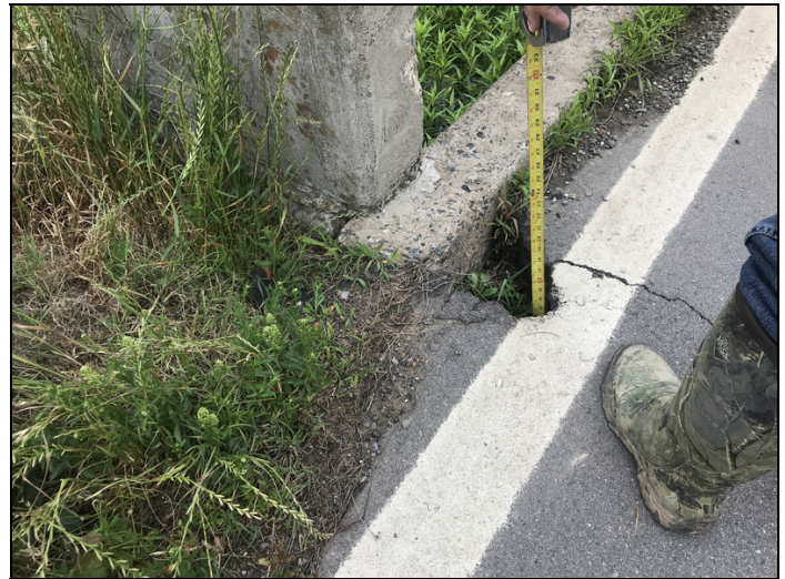
Erosion is causing a void under on the right side of approach roadway at south end of bridge.
