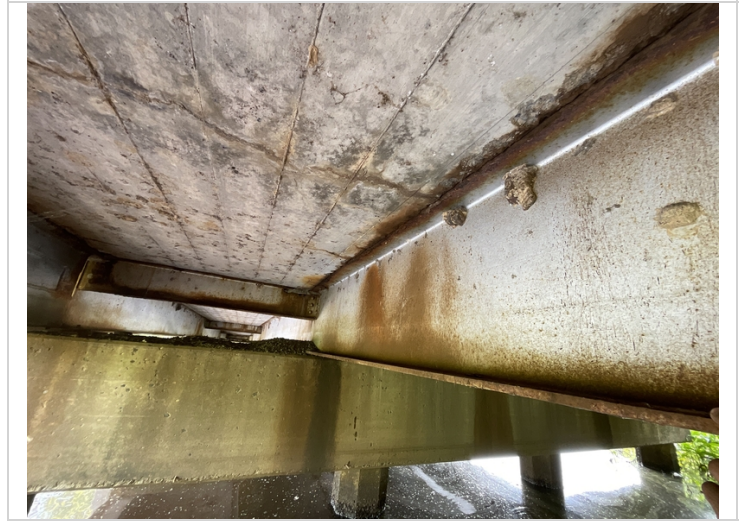
Deck over bent 2 beam 1,2,3,4 and 5 moving up to 1/4" due to not being composite to superstructure.
