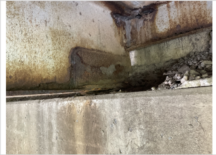
Bent 5 beam 3 has a 1"x1" hole in the haunch area
