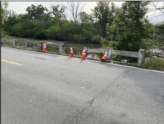
Left bridge rail in span in span 4 has been damaged from traffic impact. 6' of rail is missing. 5 post are damaged.
