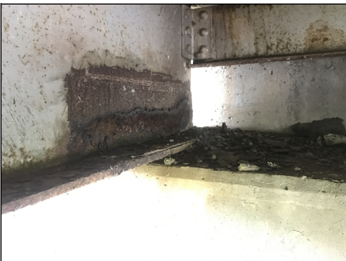
Span 1 @ bent 1: bottom flange with measurable section loss.
