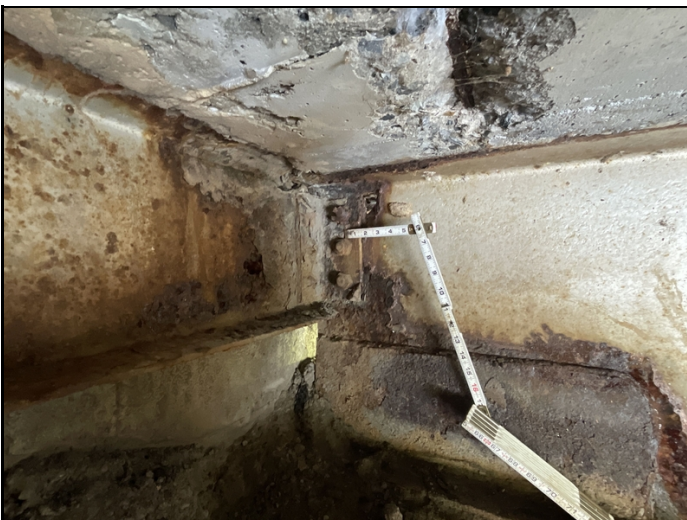
Bent 5 beam 3 has a 1"x1" hole in the haunch area
