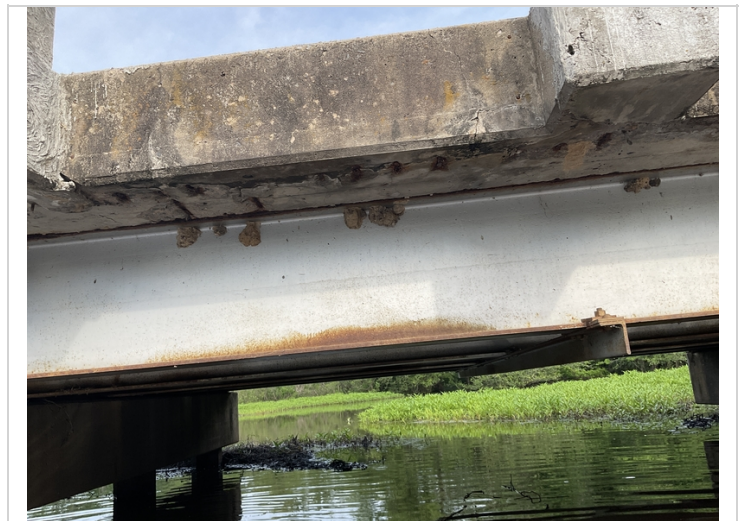
Exposed rebar on left side of span 2
