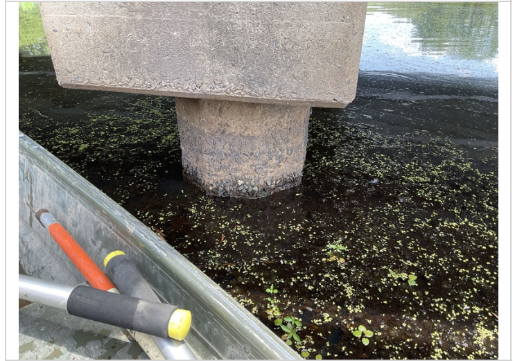
Abrasion at columns
