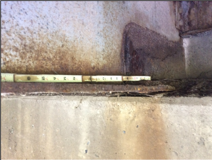
Bent 5, span 4, girder 1: beam end with measurable section loss.
