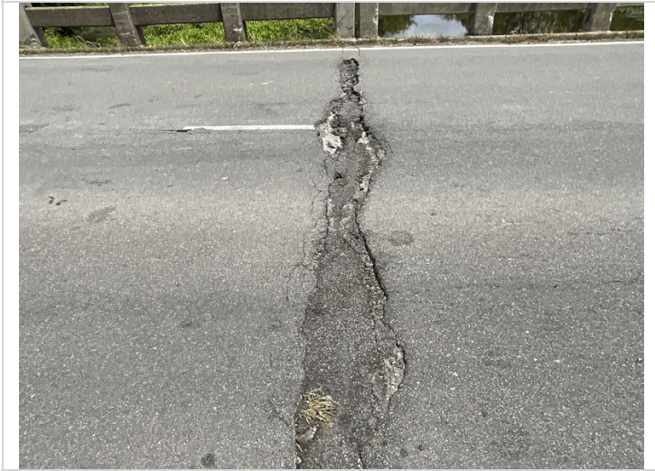
large potholes in the wearing surface over bent 2
