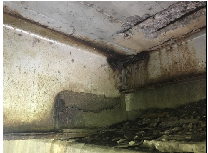
bent 5 beam 3 has a 1" hole in haunch area
