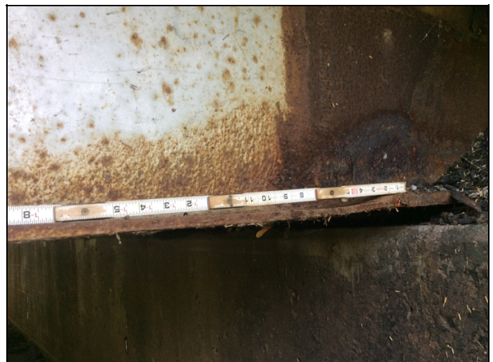
bent 5 beam 3 has a 1" hole in haunch area
