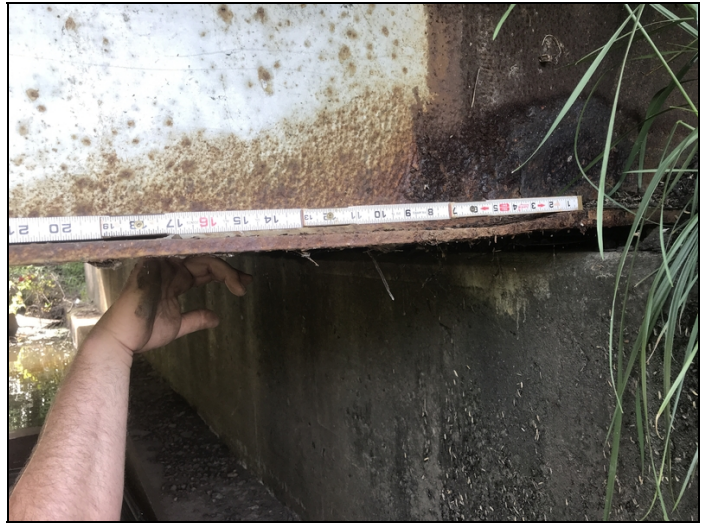
Bent 5, span 4, girder 5: 1/4" section loss to the bottom flange 25" out from backwall. Full flange thickness is 1/2".
