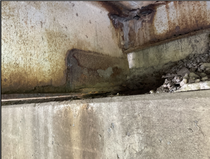
Bent 5 beam 3 has a 1"x1" hole in the haunch area
