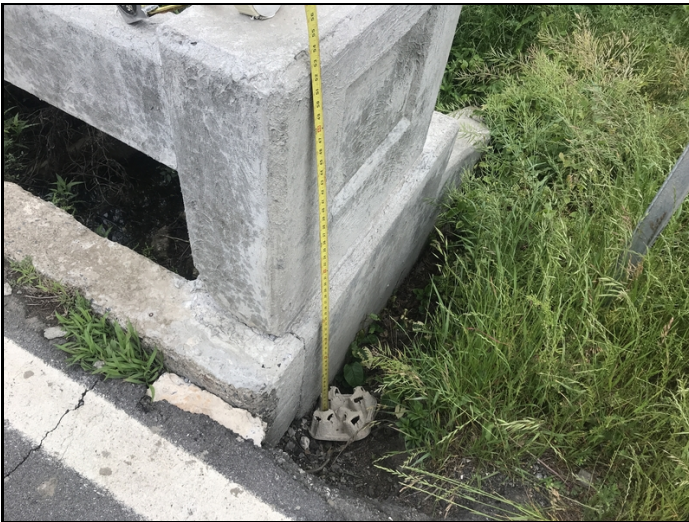
Erosion at north end of bridge at right wing wall
