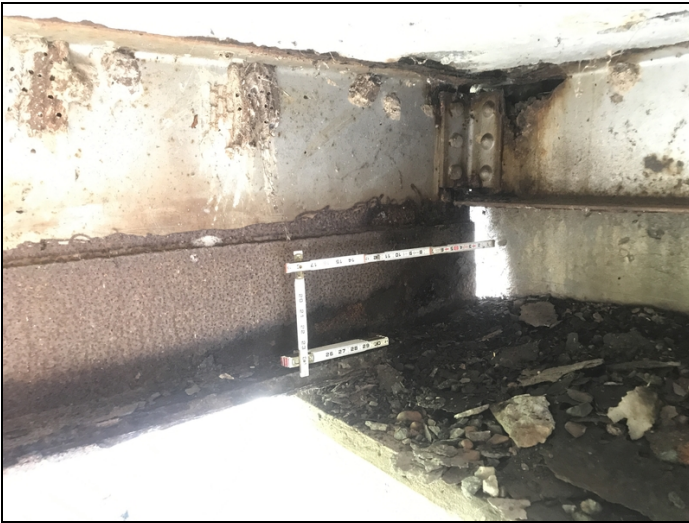
Bent 5, span 4, girder 1: beam end with measurable section loss.
