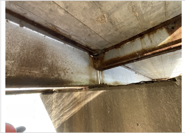
Bent 2 beam 2 3"x2" hole at top web and laminated rust at lower web and flange
