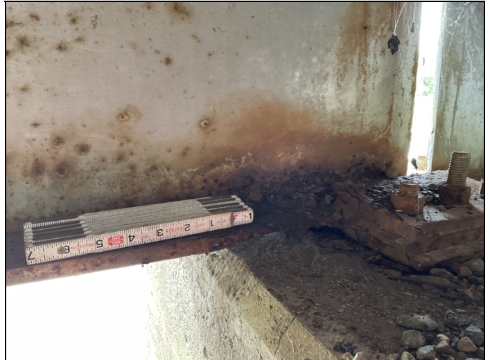
Bent 3 span 2 beam 1 has section loss on the right bottom flange is down to a knives edge
