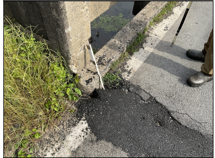
Erosion has caused a void in the right side of approach roadway at south end of bridge
