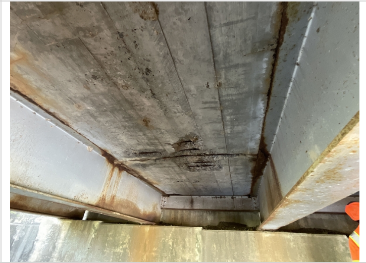
Large spalls with rebar in the soffit Span 1 between beam 3 and 4 large spall with rebar
