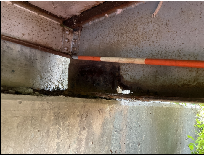
Bent 1 beam 1 has a 3"x6" hole and the lower web is a knife edge
