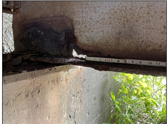
Bent 1 beam 1 has a 3" hole in bottom of web. Bottom flange on right side is down to a knives edge.
