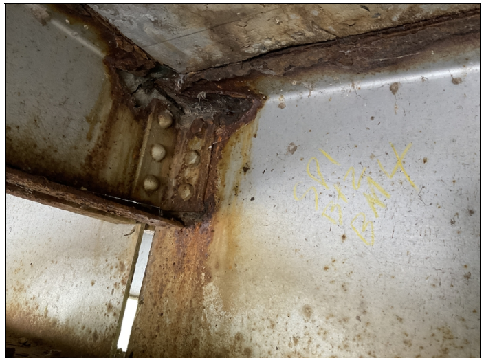
Bent 2 span 1 beam 4 has a one 1" hole in the upper web.
