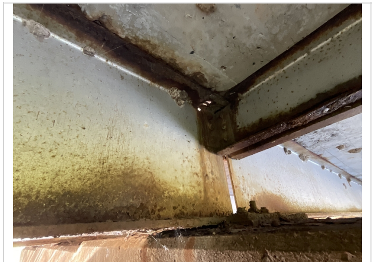
Bent 2 beam 4 1" hole at upper web laminated rust at lower web and flange
