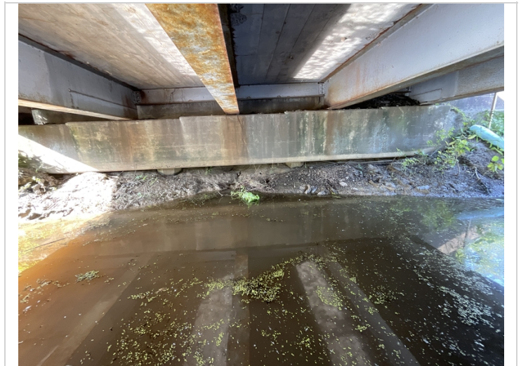
Bent 5 erosion
