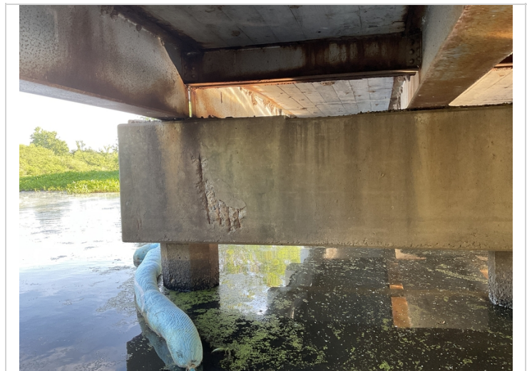
Bent 4 ahead right spall with rebar
