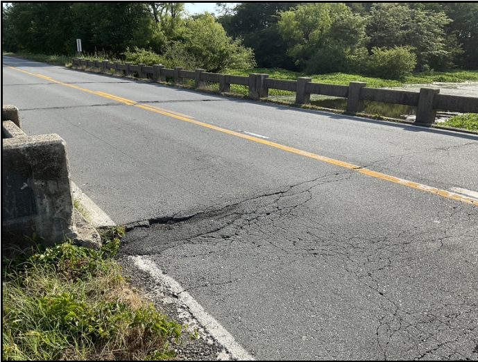
Pothole at bent 5
