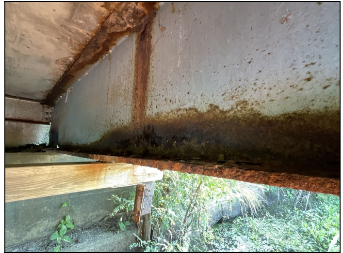
Bent 1 beam 1 has 8' corrosion
