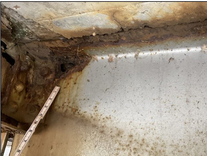
Bent 2 span 1 beam 2 has a 1" x 2" hole in the upper web. Top flange is down to a knives edge.
