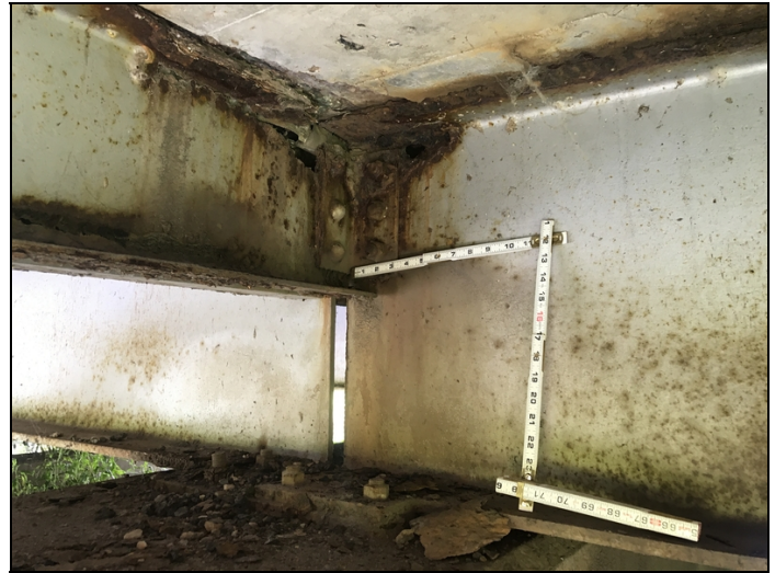
Span 1, bent 2, beam 2: hole in the upper web due to severe section loss to the web and the top flange.
