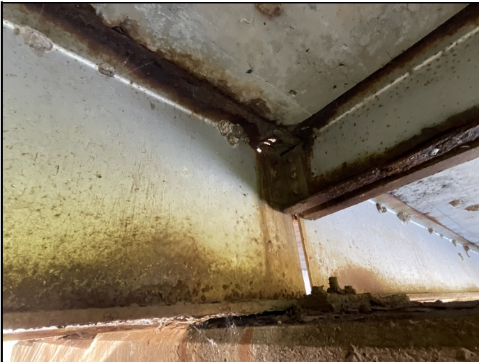
Bent 2 beam 4 1" hole at upper web laminated rust at lower web and flange
