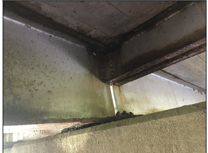
Span 2 girder 2 1" hole in upper web
