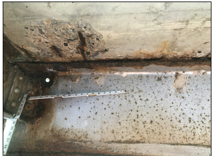
Span 4, bent 4, beam 1: hole in the upper web and the top flange has section loss to a knives edge.
