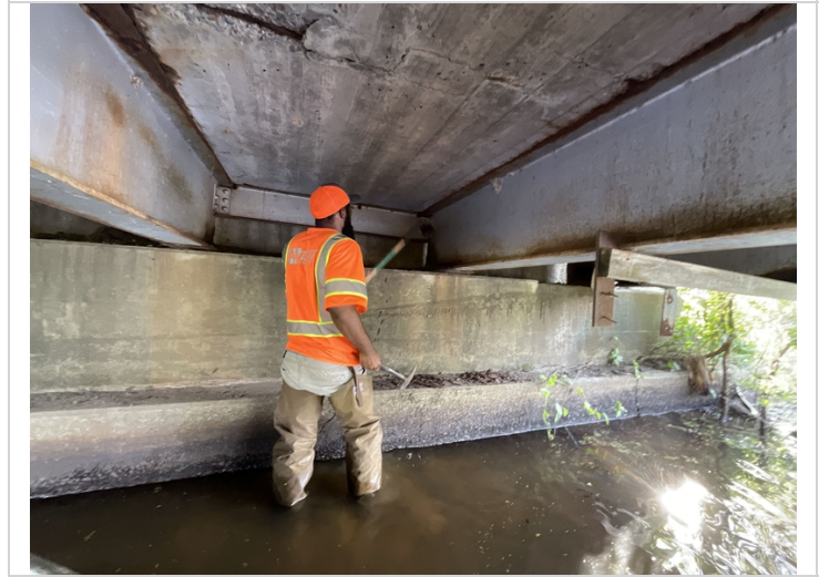
Bent 1 beam ends have deep pitting and laminated rust
