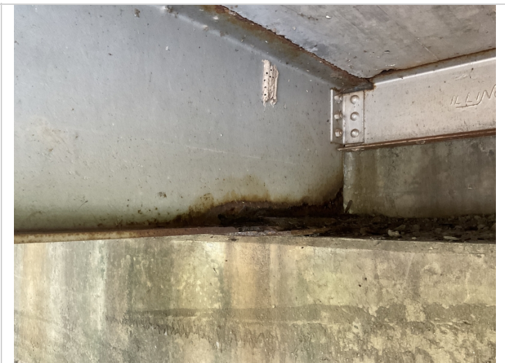
Bent 1 beam 2 has up to 1/8" pitting to the lower web
