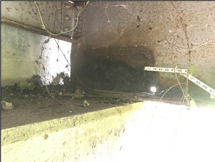
Span 1, bent 1, beam 1: a 1 inch hole in the lower web adjacent to a previous section loss repair. The repair and bottom flange have section loss to them.
