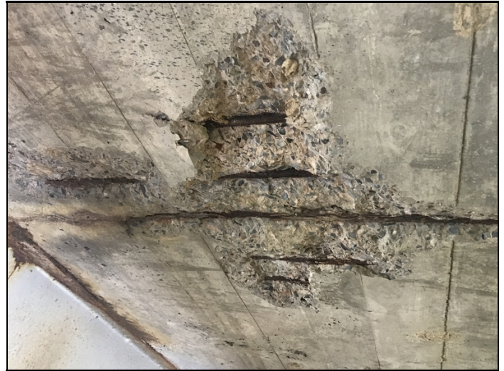
Span 1 large spall with exposed rebar
