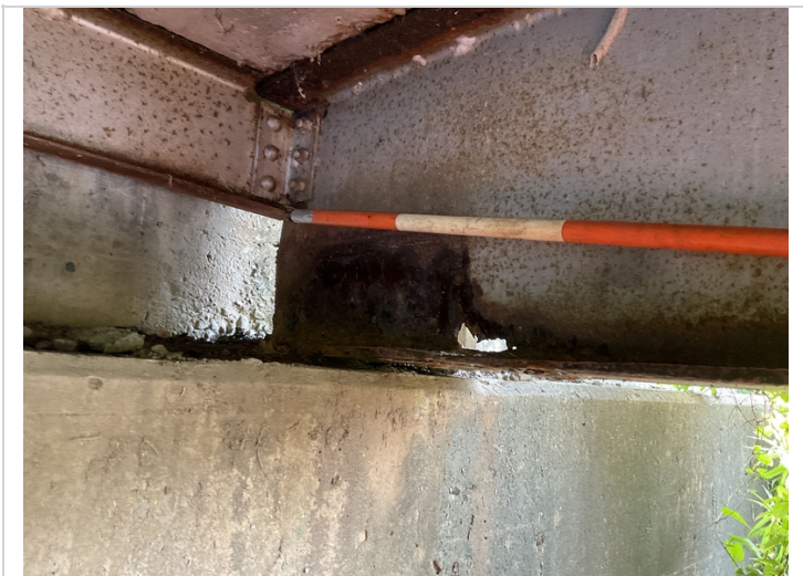
Bent 1 beam 1 has a 3"x6" hole and the lower web is a knife edge
