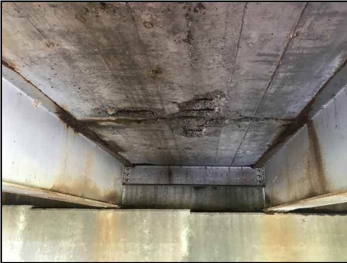
Span 1 soffit between girders 3 & 4: large spall with exposed rebar
