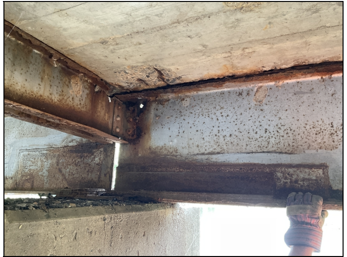
Bent 4, span 4, girder 1: upper web has a 1 inch hole and the upper flange has lost section to a knives edge
