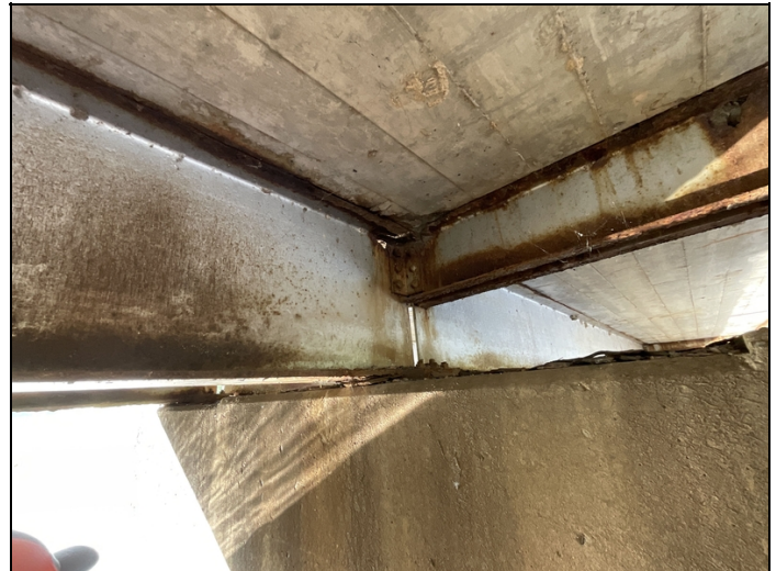
Bent 2 beam 2 3"x2" hole at top web and laminated rust at lower web and flange
