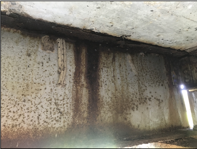
Span 1, bent 2, girder 1: top flange with section loss to a knife edge for approximately 2 foot in length.
