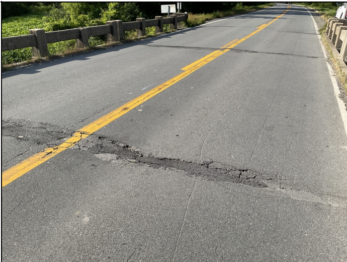
patched areas over joints have spalls
