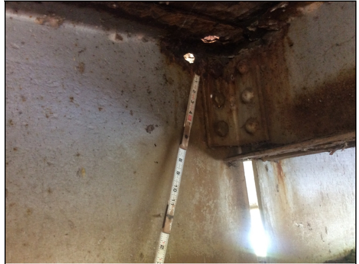
Bent 1 beam 1 has 8' corrosion
