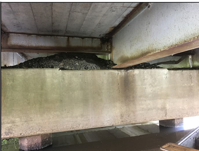
Bent 3: large amount of asphalt debris atop of cap and bottom flanges between girders 3&4. Similar condition at bent 4
