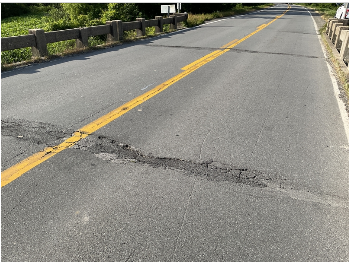
patched areas over joints have spalls
