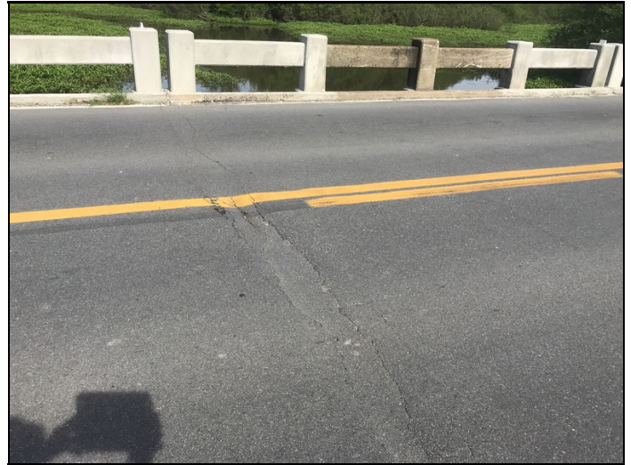
Bent 4: asphalt material is falling through joint leaving a bump in the roadway surface
