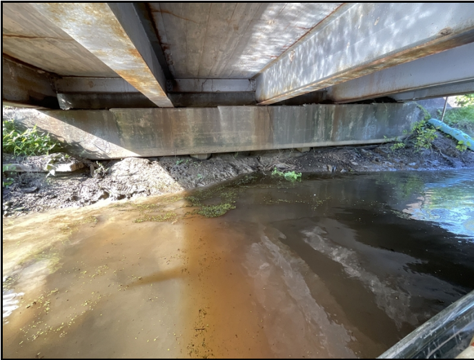
Erosion at bent 5 exposing 3 piles
