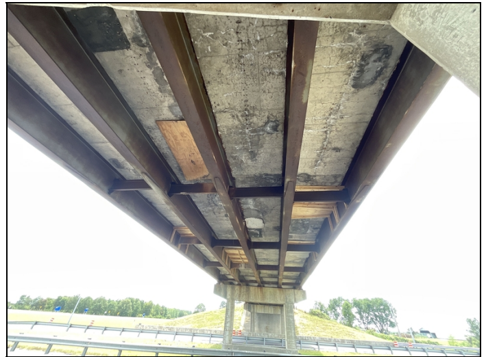
Span 4 repair forms still in place
