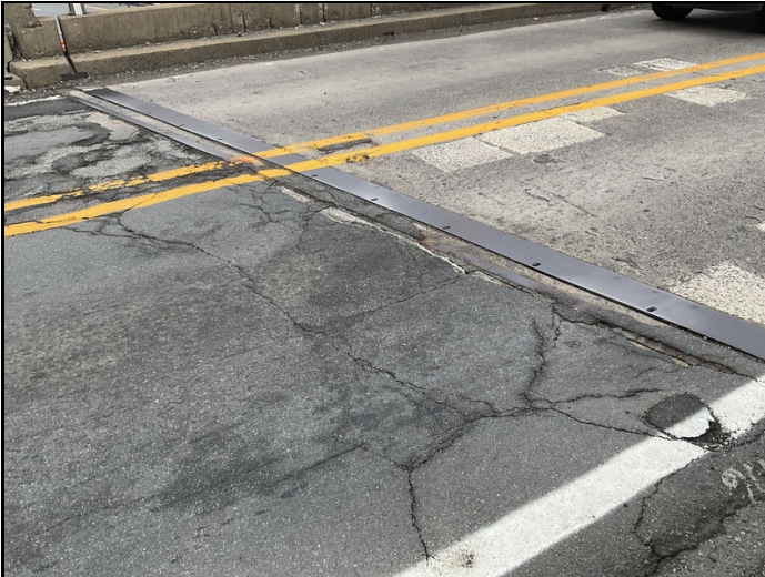
Spalls in the approach roadway bent 1
