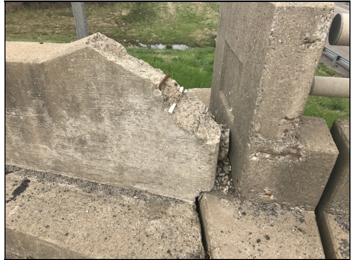
Left approach rail at bent 1 has a large spall.
