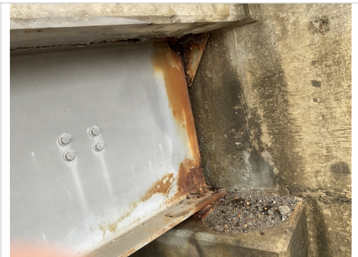
Beam 1 bent 1 corrosion at the bearing and haunches
