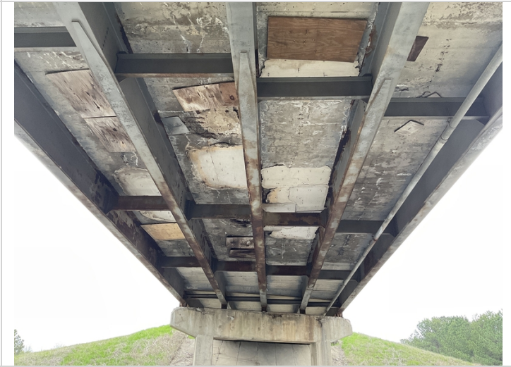
Span 3 soffit has large patches spalls and spalls with rebar
