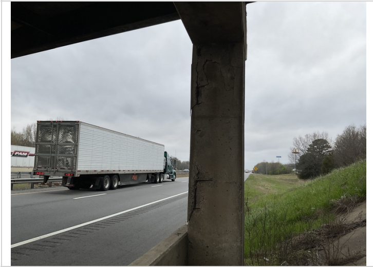
Column 1 at bent 4 has large spall delams and exposed rebar
