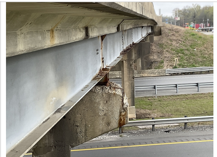
Span 3 beam 1 corrosion
