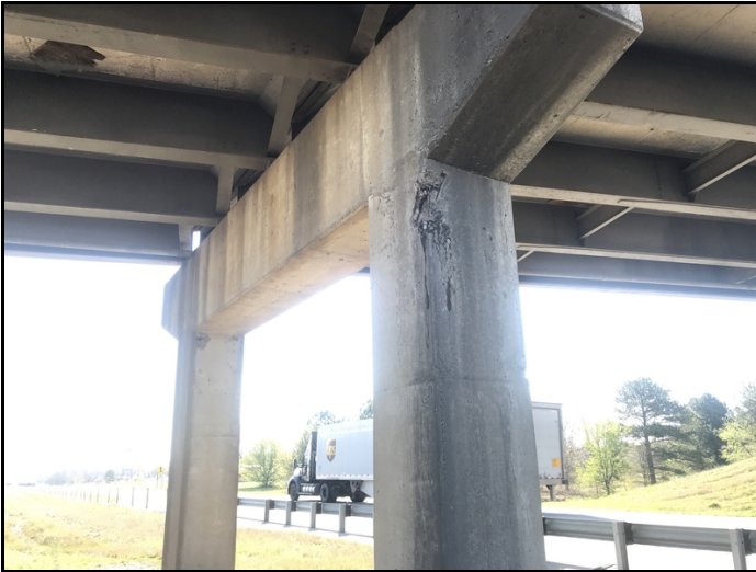
Bent 3, column 1: large spall with exposed rebar.
