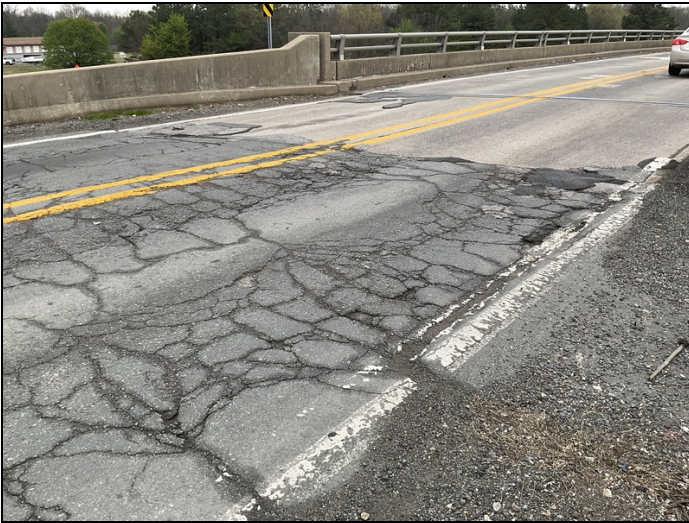
potholes in the Approach wearing surface at north end
