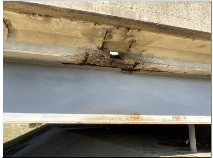
Span 4 right side spall with exposed rebar
