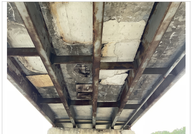
Span 3 paint has failed and corrosion has begun
