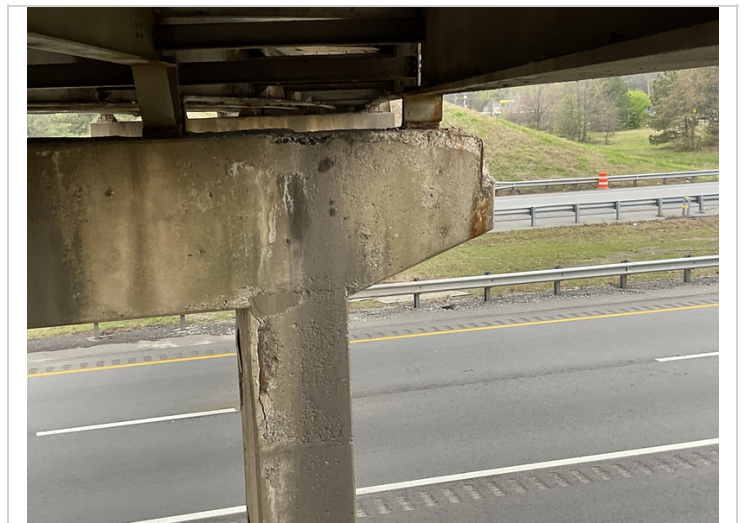
Bent 4 backside spall exposing hoop bars
