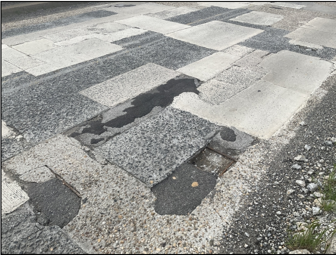
Span 3 large spalls with exposed rebar.
