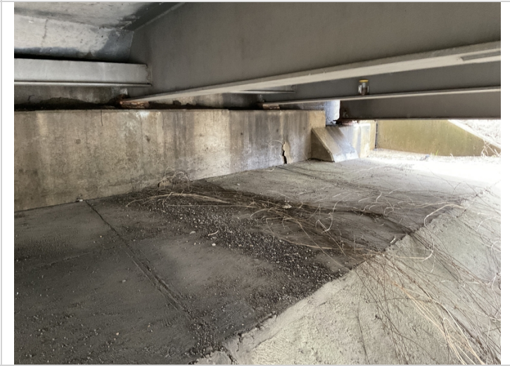
Delamination bent 1
