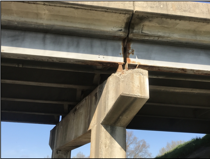
Bent 4: right end of cap with a large spall that is adjacent to girder 5 bearing.
