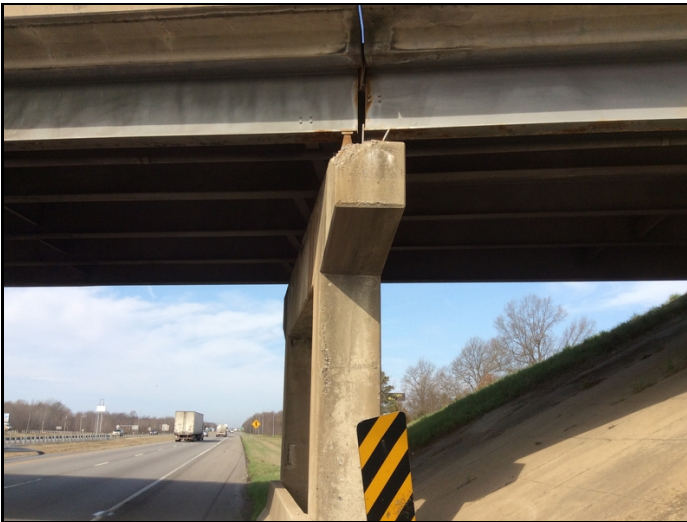
The right end of the cap of bent 4 has a large spall.
