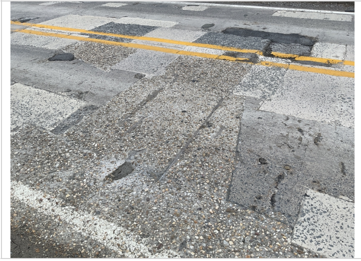
Exposed rebar in the deck span 2. deck has large patches spalls with asphalt and exposed rebar in all spans
