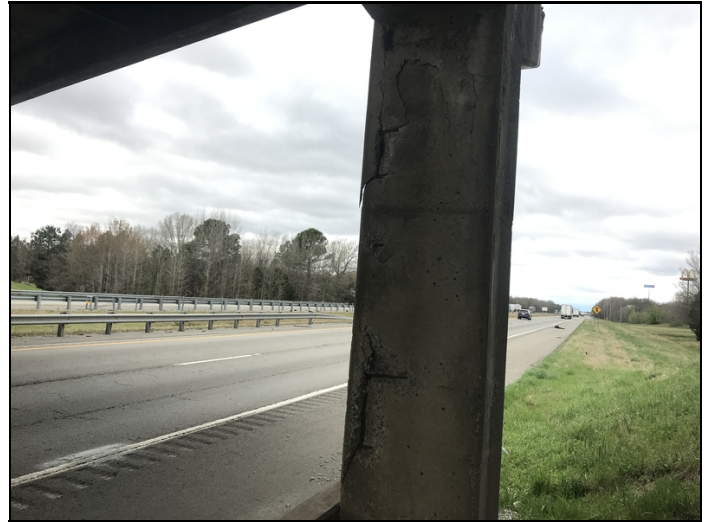
Bent 4 column 1 large spalls with exposed rebar
