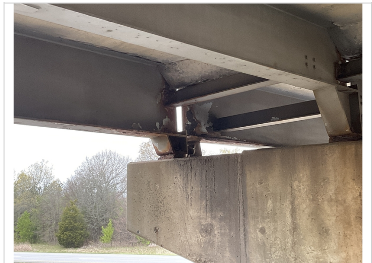
Bent 2 beam 1 corrosion with deep pitting up to 1/8"
