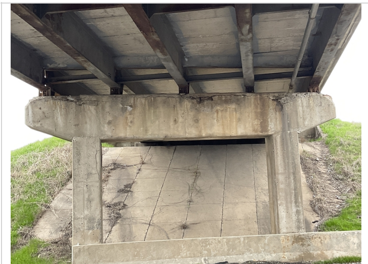
Bent 4 cap has large horizontal cracks spalls and rebar exposed
