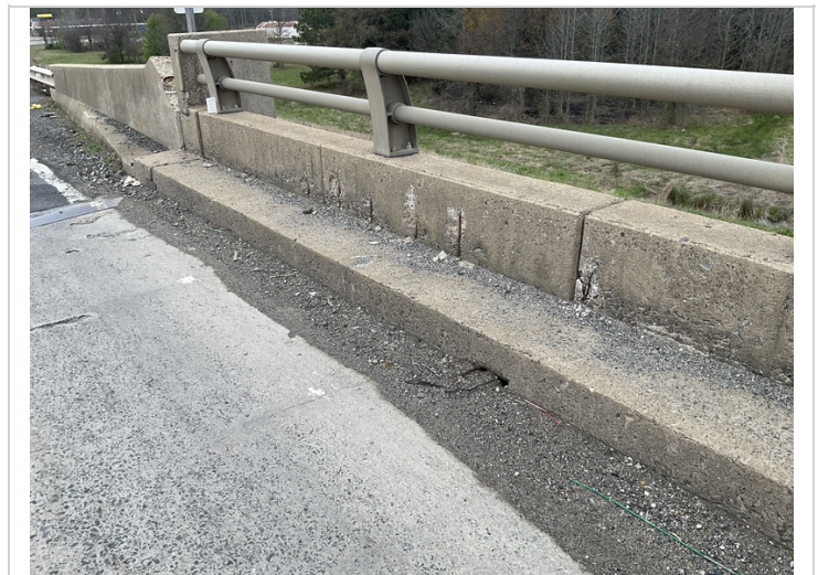
Exposed rebar in the concrete bridge rail left side span 1
