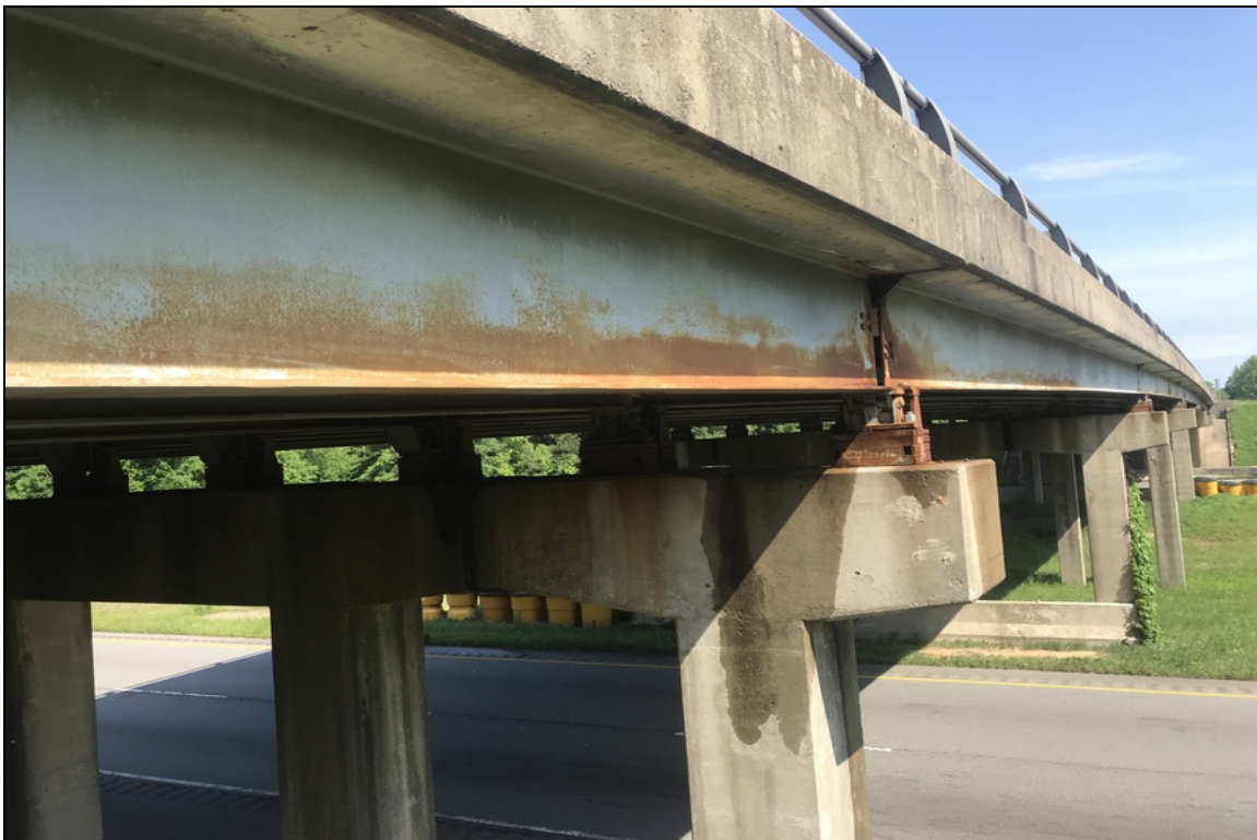
Span 1, girder 8: the lower web and bottom flange with active corrosion mean the beam end
