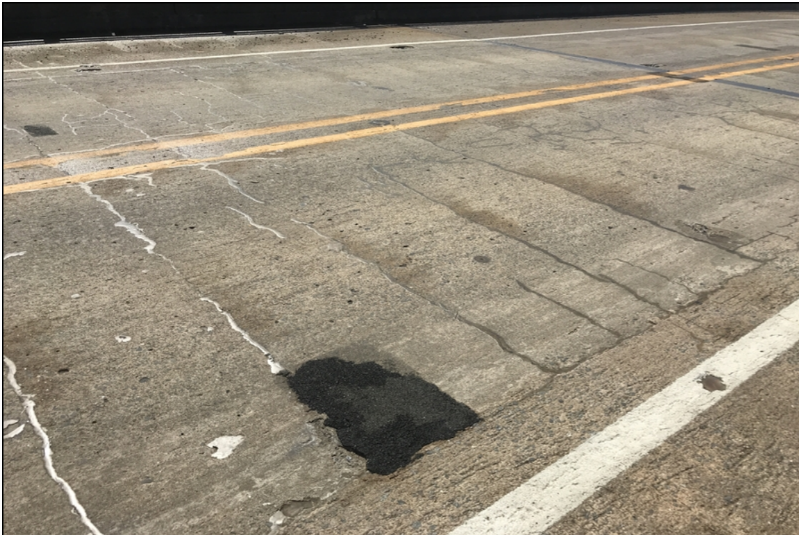
Numerous transverse cracks are sealed
