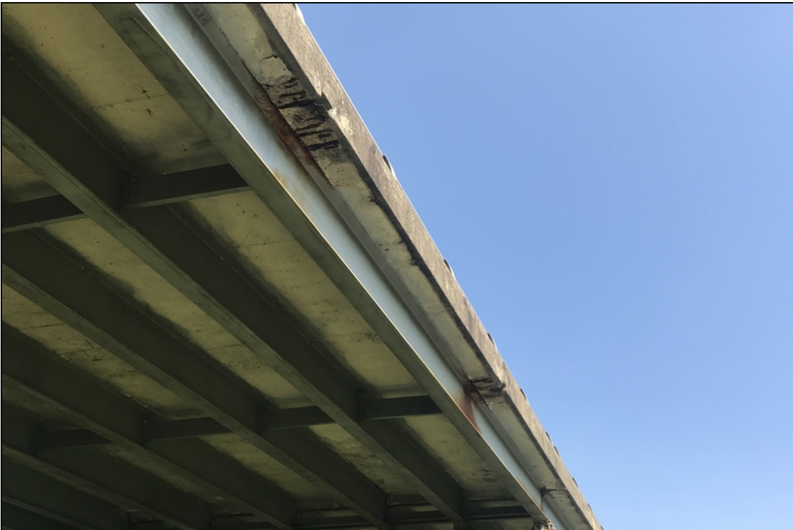
Span 3: right side the soffit has a few spalls with exposed rebar
