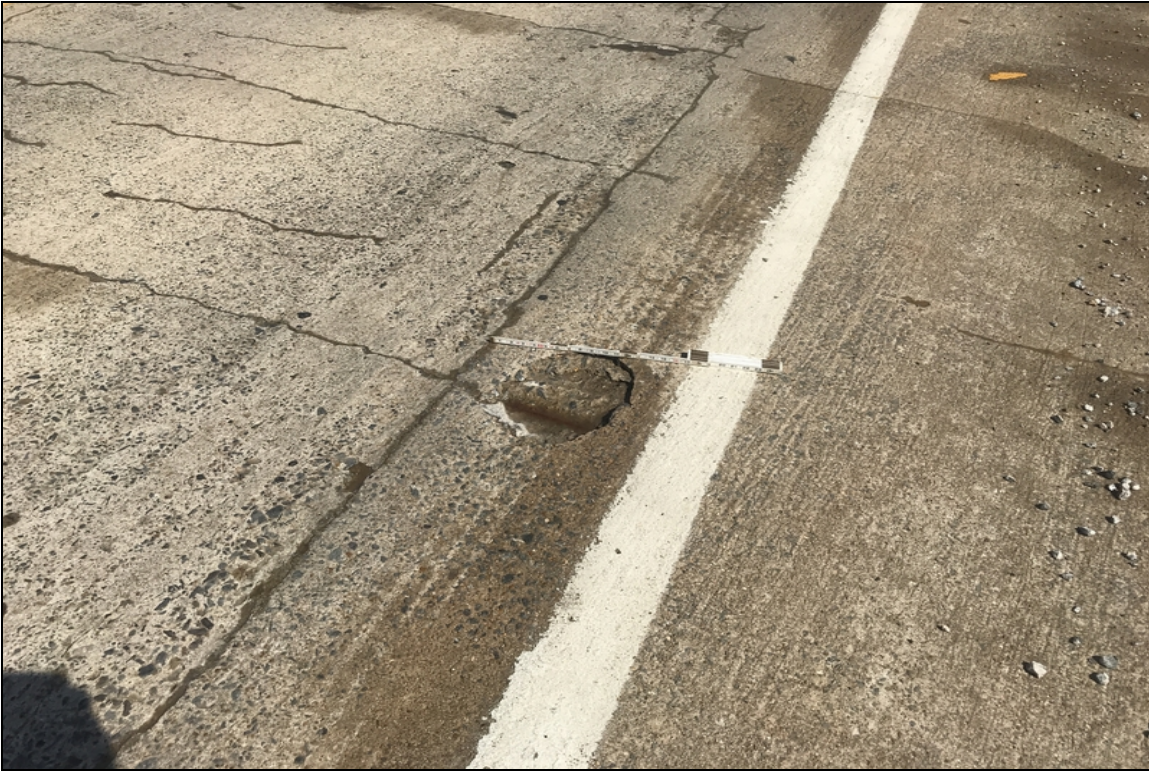
Span 6 with an open spall in northbound lane
