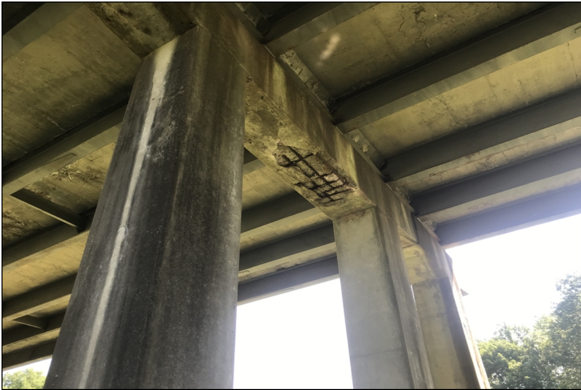
Bent 3, between columns 2 & 3: large spall with exposed rebar
