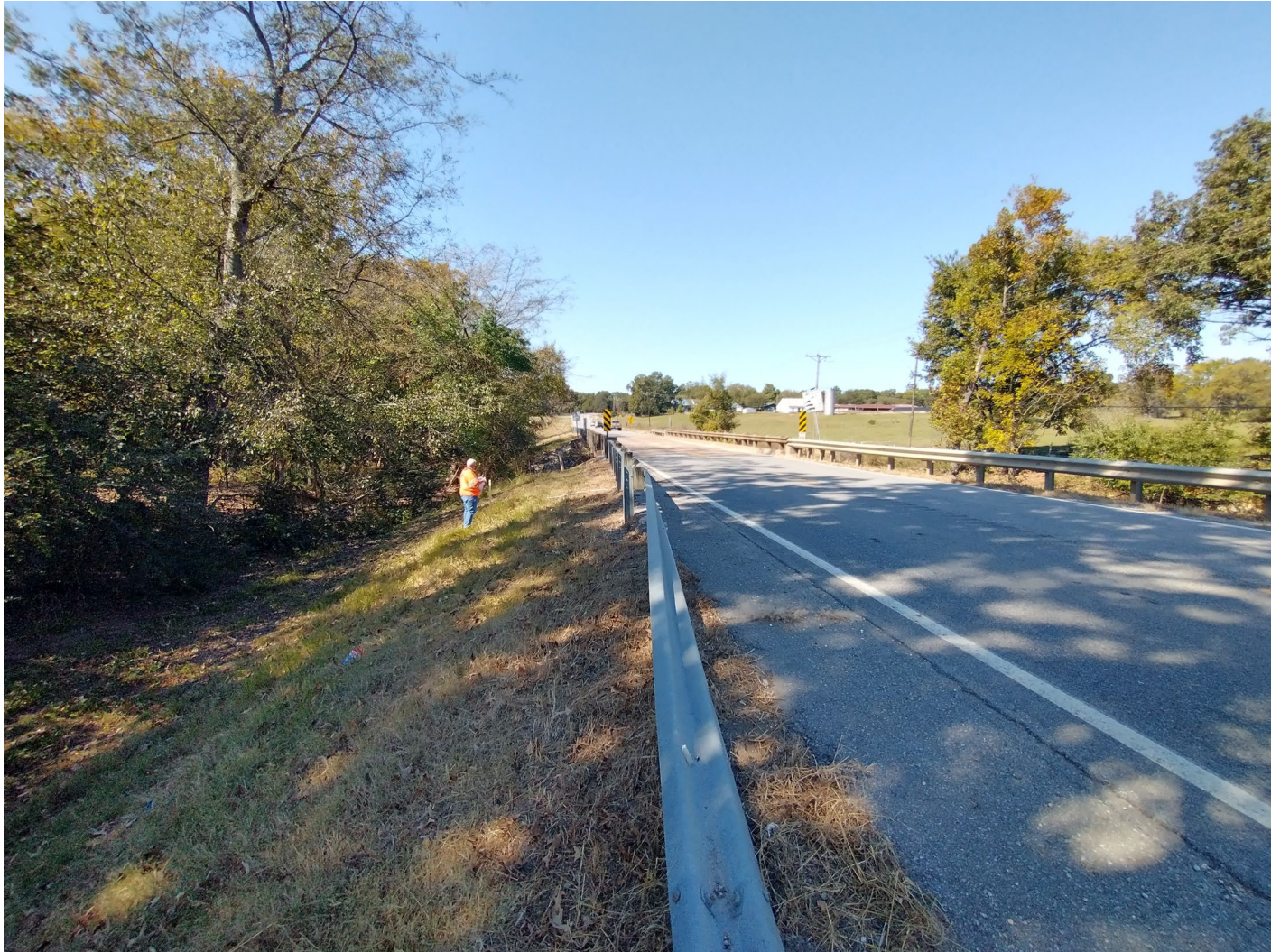
Looking west at the east end of the existing bridge (November 2024)
