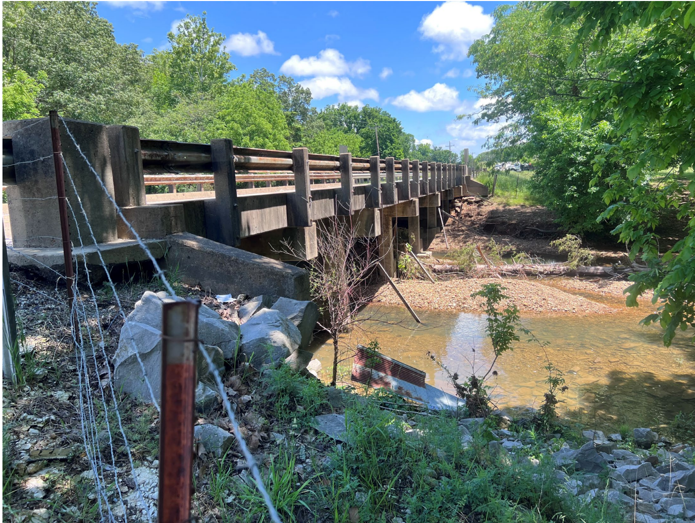
South side of existing bridge, looking east (May 2025)
