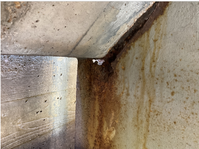
Hole to web below paving haunch to girder 4 @ abutment 2.
