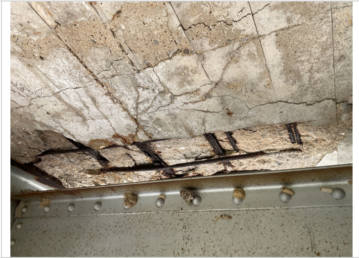
Spalls with rebar exposed, some with 100% s/l & loss of bonding area to concrete to soffit @ Span 4.
