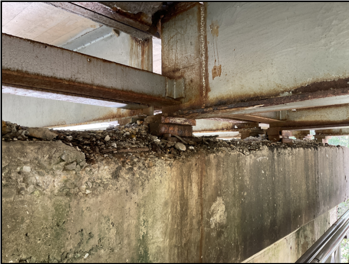
Debris on cap @ Bent 1.
