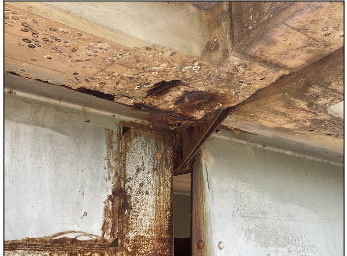
Large spalls with rebar exposed to Left & Right overhangs at Spans 2, 4, 5, & 6. Span 2, rt overhang.
