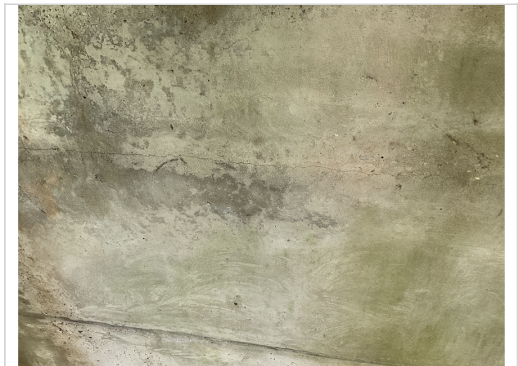
Horizontal cracking to Concrete Pier Wall @ Bent 1.
