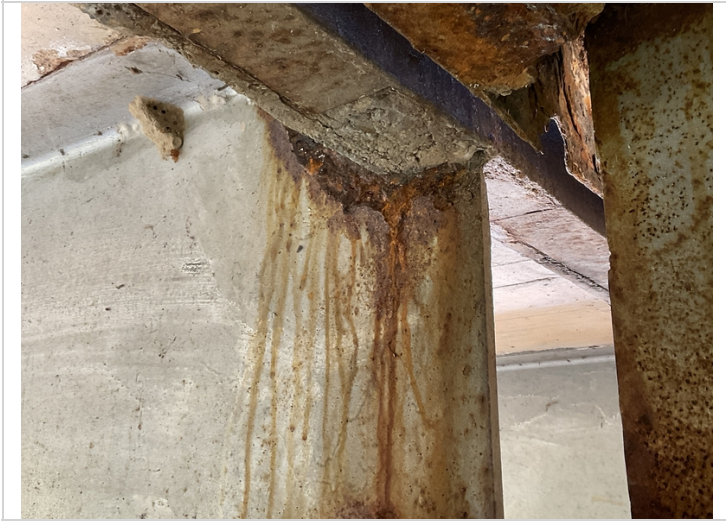
Rust with section loss to web @ girders 1 - 5 @ beginning of span 2.
