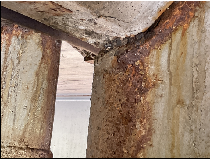
Rust with s/l to web below haunch @ Girder 3 @ end of Span 4.
