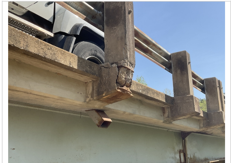
7th post of the right side of span 4 is damaged and has rebar exposed.
