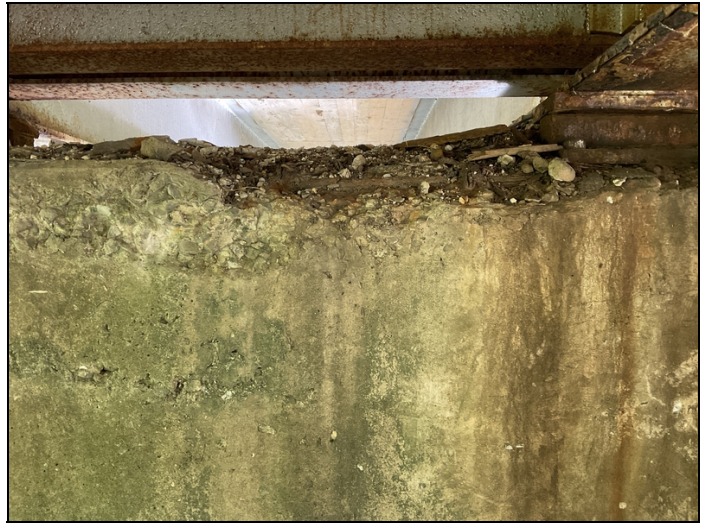
Heavy spalling with rebar exposed, delaminating & cracking to Caps & Columns at Bents 1-5. Bent 1.
