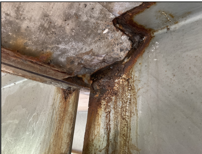
Rust with s/l & holes in web below haunch above repaired area @ Girder 3 @ end of Span 2.
