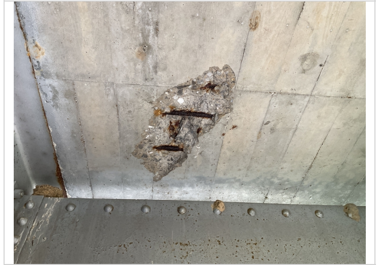
Deep spall with rebar exposed to soffit between girders 1 & 2.
