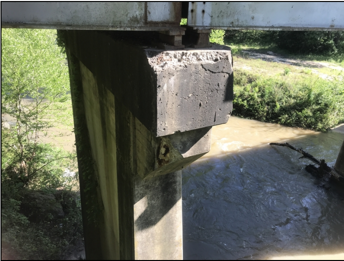
Heavy spalling with rebar exposed, delaminating & cracking to Caps & Columns at Bents 1-5.
