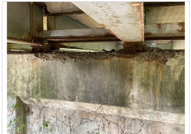
Large spall to ahead side of cap @ bent 1.
