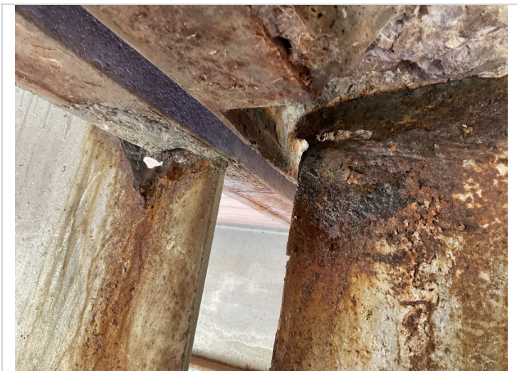
Girder 3 @ end of span 2 & girder 3 @ beginning of span 3 has holes to web below paving haunch.
