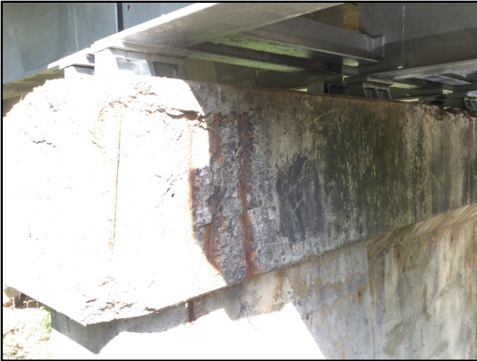
Spalls with rebar exposed to Right end of cap @ Bent 1.
