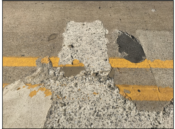
Span 5 - Spall with 1' rebar exposed to deck.
