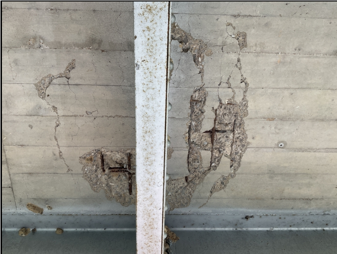
Deep spalls with rebar exposed to soffit at Spans 3, 4 & 5 Span 3, between girders 4 & 5.
