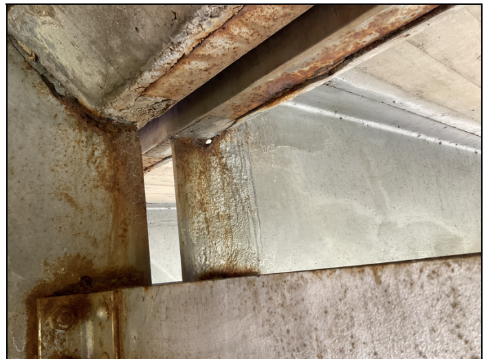
Rust with s/l & hole in web below haunch @ Girder 4 @ end of Span 2.
