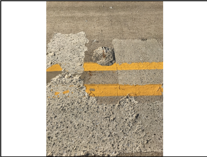
Span 5 - Spall with 1' rebar exposed to deck.
