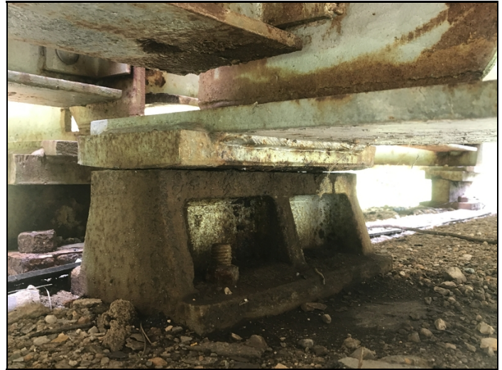
Bent 4 - Fixed Bearing 2 on ahd. Side is non-bearing until loaded.
