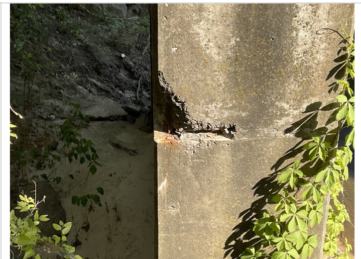
Deep Spall with rebar exposed with section loss to Column 2 @ Bent 1
