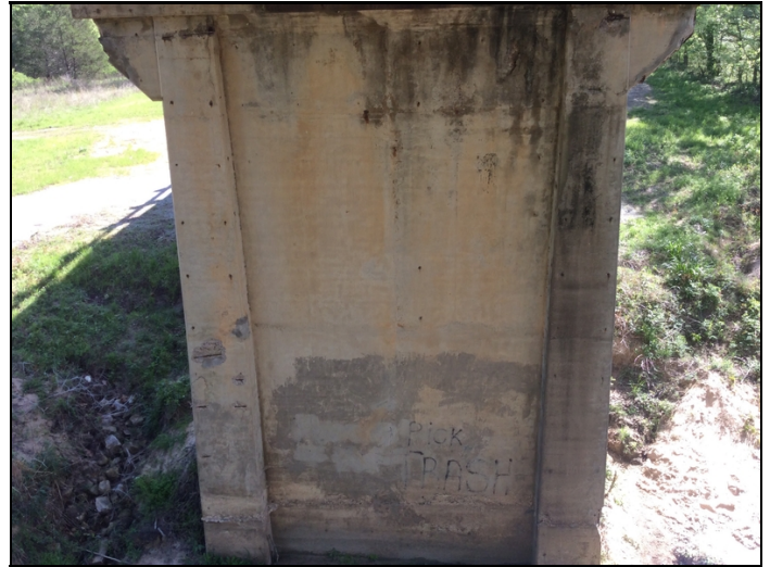
Spalls with rebar exposed to Columns 1 & 2 @ Bent 3.
