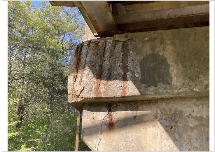
Large spall with rebar exposed to rt ahead side of cap @ bent 1.
