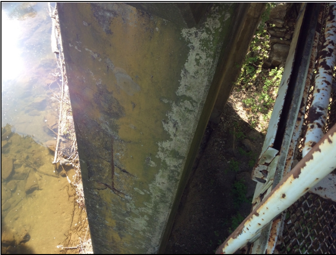
Spalls with rebar exposed to Left Column @ Bent 1.
