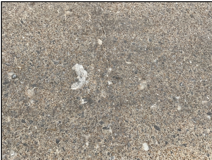
Unsealed cracks to Deck.
