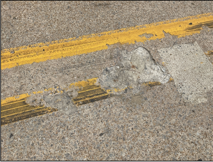
Span 5 - Spall with 1' rebar exposed to deck.
