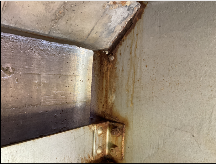
Rust with s/l & hole in web below haunch @ Girder 4 @ Abutment 2.
