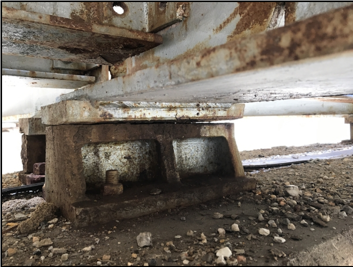
Bent 4 - Fixed Bearing 2 on ahead side is non-bearing until loaded.
