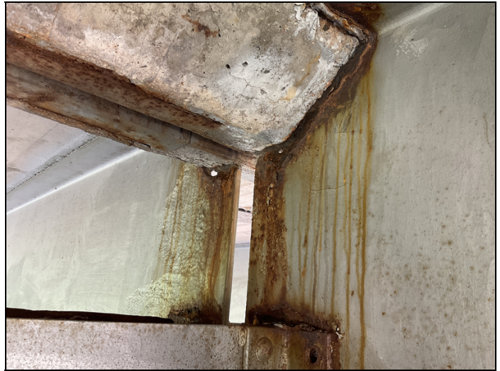
Rust with s/l & holes in webs below haunch @ Girder 3 @ end of Span 4 & beginning of Span 5.
