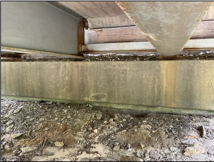
Debris on cap @ Bents 1 - 5 & Abutment 2. Abutment 2.
