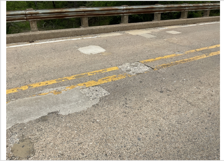
Typical spalls & patched areas to deck @ all spans
