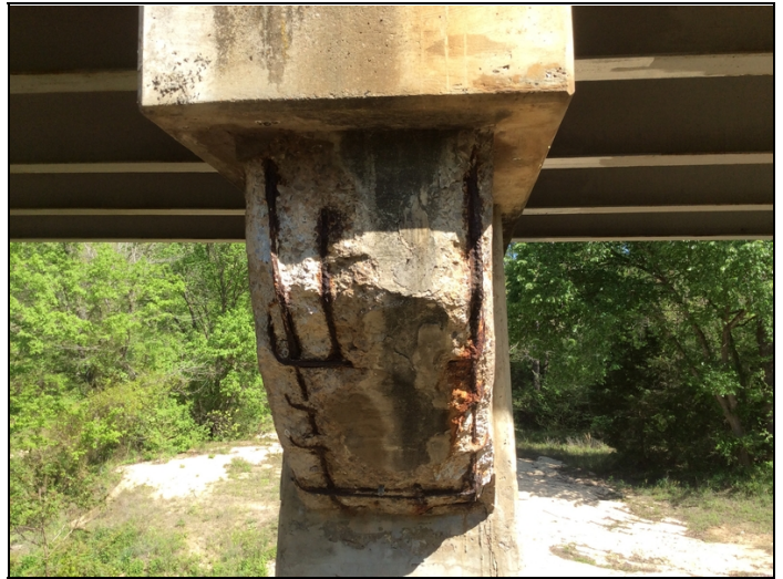
Spalls with rebar exposed to cap support haunch @ Bent 3 Right. Some with 100% section loss.
