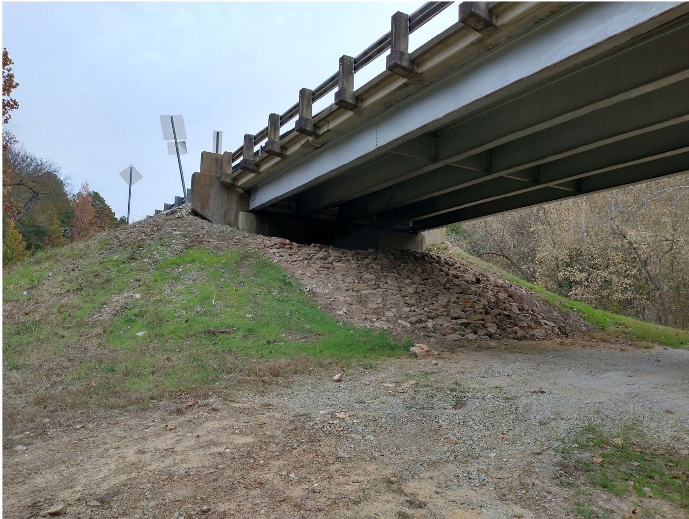
East End of Existing Bridge (March 2022)
