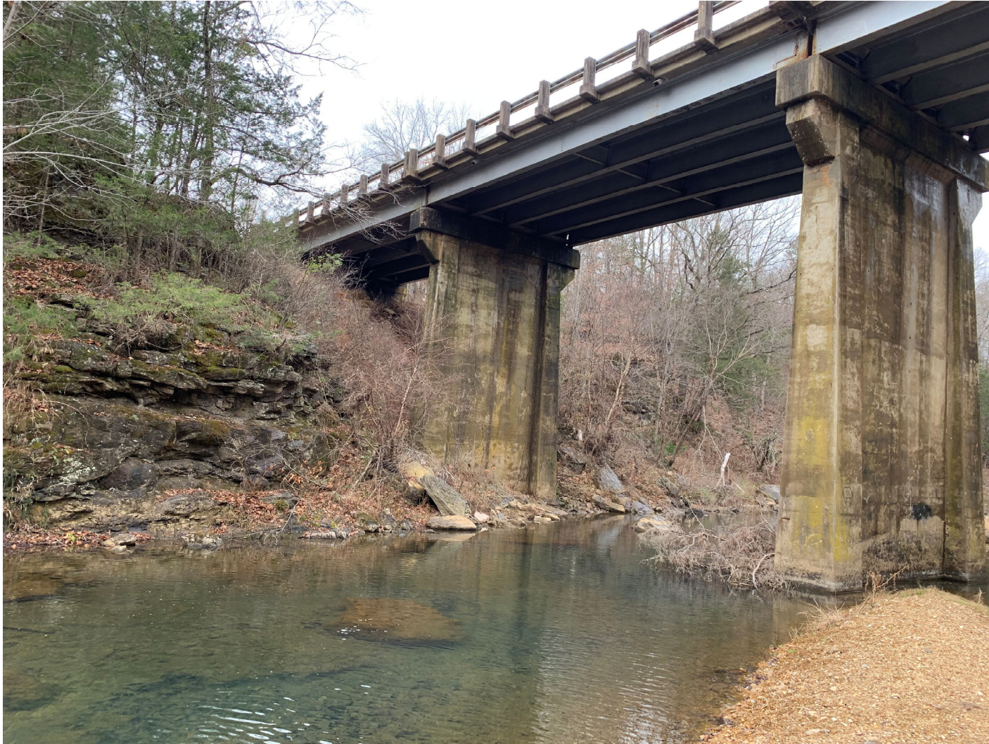
Rock Exposed at the Southwest End of Existing Bridge (March 2022)
