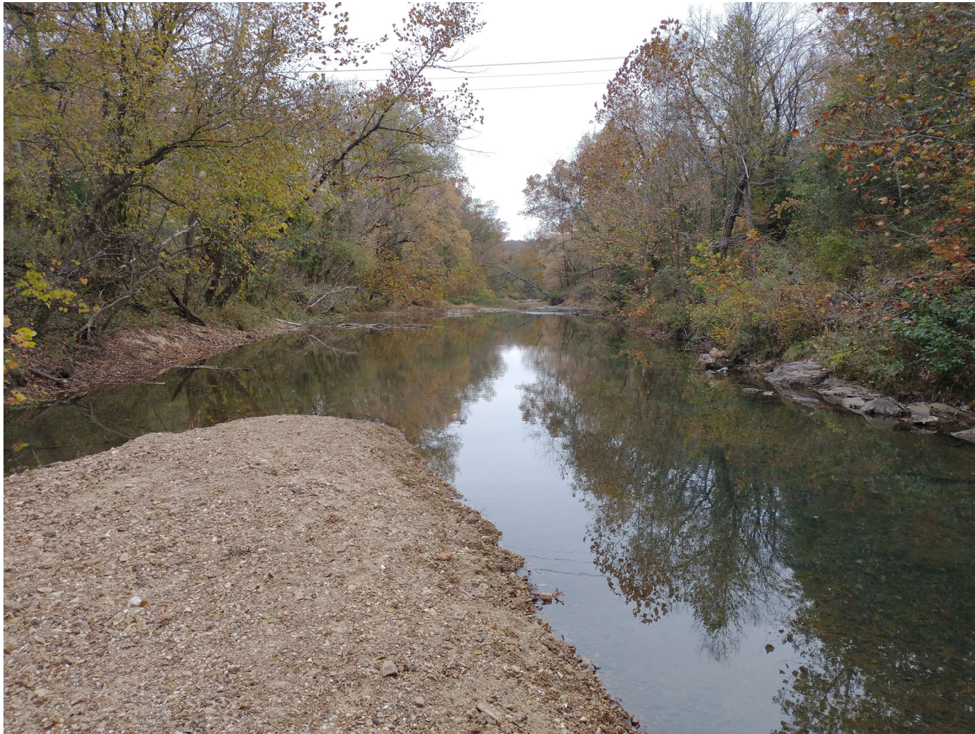
Looking South of the Bridge Downstream (March 2022)
