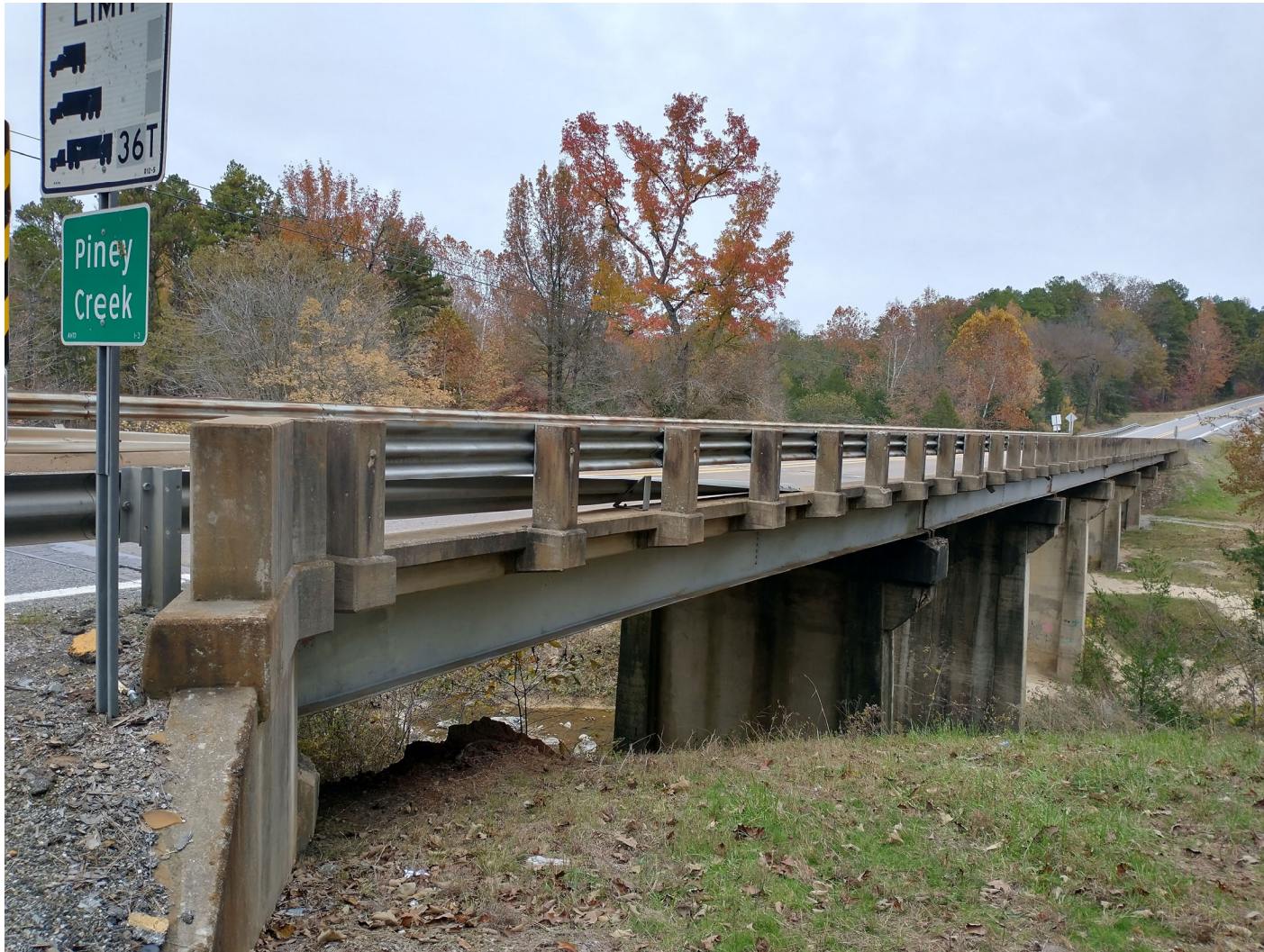
Overall View of Existing Bridge - Looking East (March 2022)
