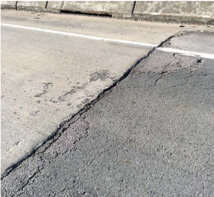
PHOTO 1 Description Roadway settlement @ Abutment 1.
