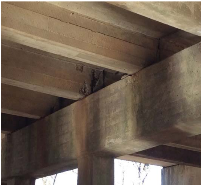
PHOTO 1 Description Full height vertical cracks to Girders 2, 3 & 4 @ beginning of Span 4.
