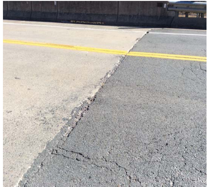
PHOTO 2 Description Roadway settlement @ Abutment 2.
