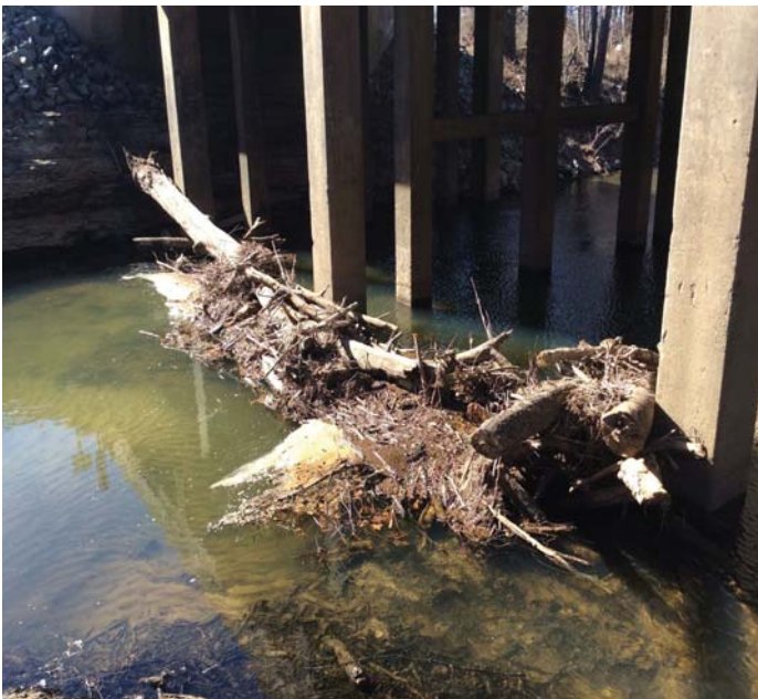
PHOTO 1 Description Drift @ Spans 6 & 7 restricting flow, creating scour at Spans 4, 5 & 6.
