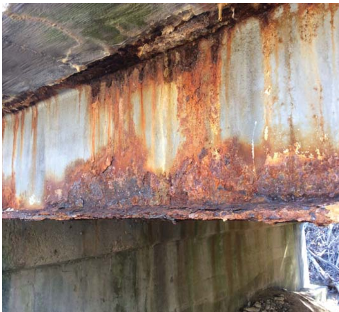
PHOTO 3 Description Bottom flange of Girder 1 at Span 1.
