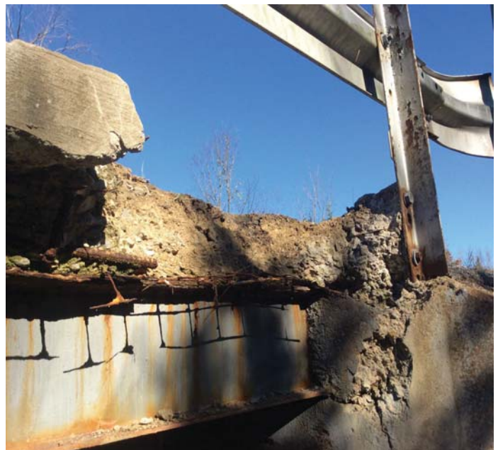
PHOTO 2 Description Deck at Abutment 2 Spalled with 1.5' x 3.5' hole in Deck at Right edge.
