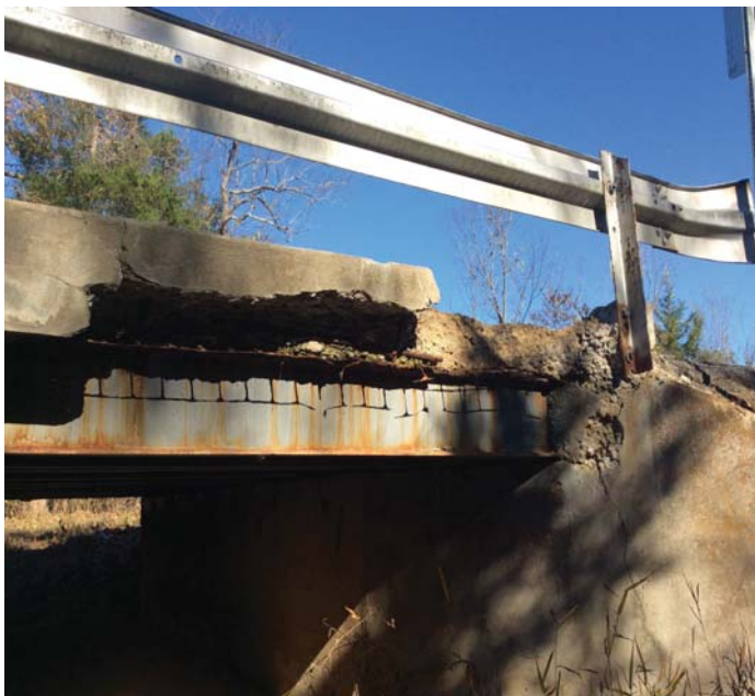
PHOTO 1 Description Deck at Abutment 2 Spalled with 1.5' x 3.5' hole in Deck at Right edge.
