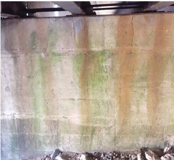
PHOTO 1 Description Moderate vertical cracks to Bent 1.
