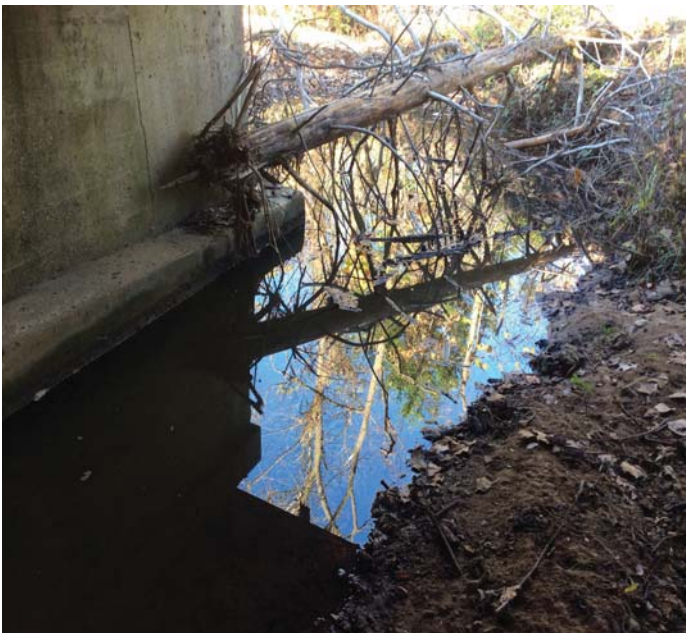
PHOTO 1 Description Scour @ Left end of Bent 1.
