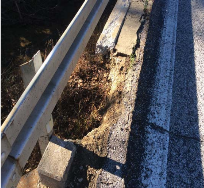
PHOTO 3 Description Deck at Abutment 2 Spalled with 1.5' x 3.5' hole in Deck at Right edge.
