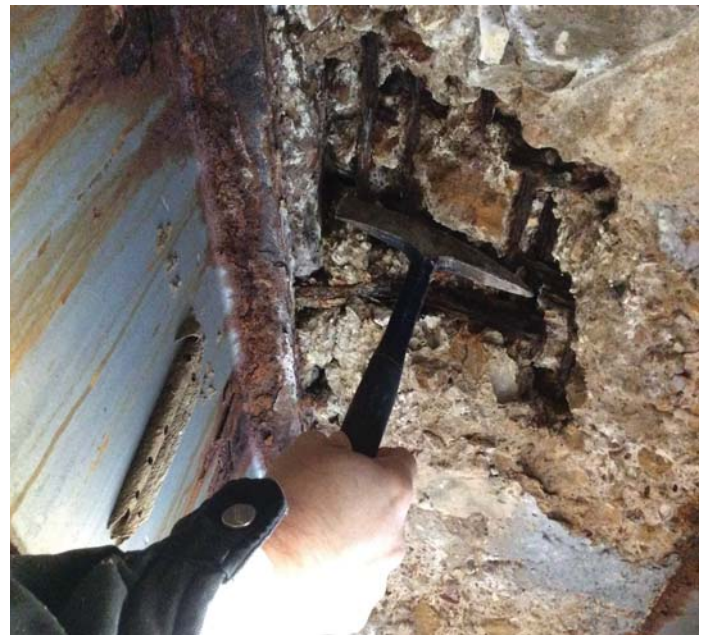
PHOTO 2 Description Deck between Girders 2 & 3 at Span 1 has deep spall with exposed rebar with 100% section loss.
