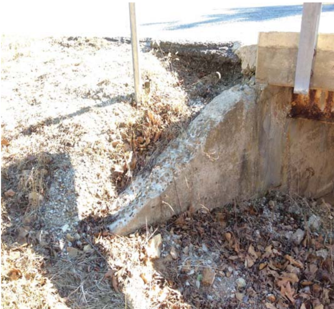
PHOTO 1 Description Erosion to slope behind Left Wing at Abutment 2 beginning to undermine roadway.
