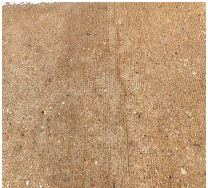
PHOTO 2 Description Transverse cracking to deck @ Span 2. Left lane.
