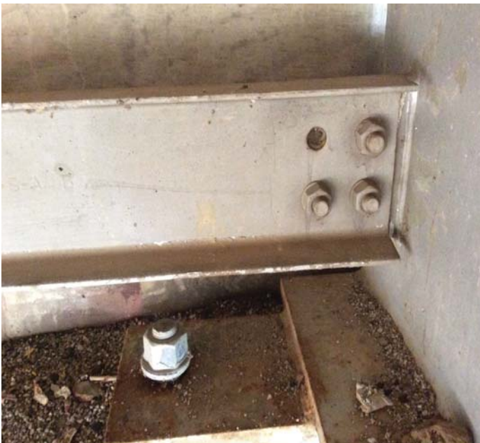
PHOTO 1 Description Diaphragm @ Right side of Girder 3 @ Abutment 1 has 1 bolt missing.
