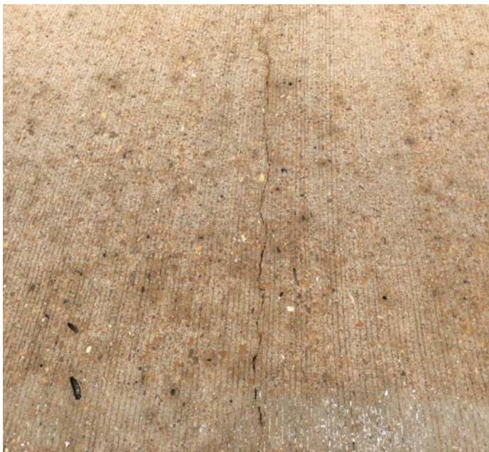
PHOTO 1 Description Transverse cracking to deck @ Span 3. Right lane.
