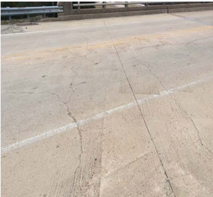
PHOTO 1 Description Unsealed cracks to approach slabs @ Abutment 1 & 2.
