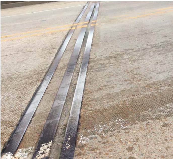
PHOTO 1 Description 18' of Joint seal has separated & leak @ Abutment 1 & 2.
