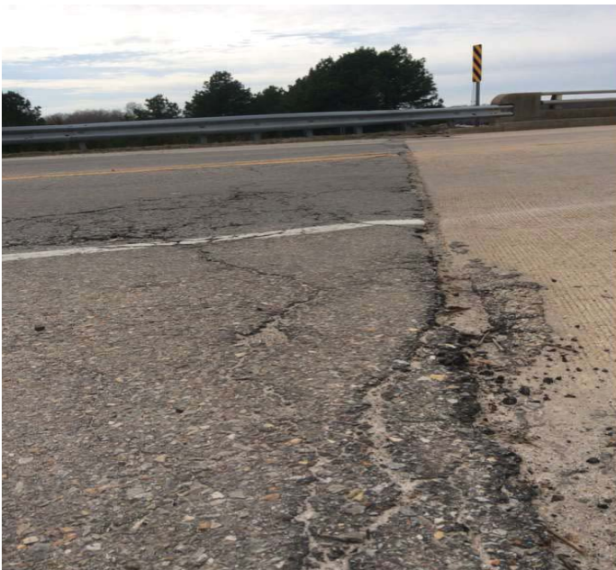
PHOTO 1 Description Visible settlement & potholes to Roadway @ Abutment 1.
