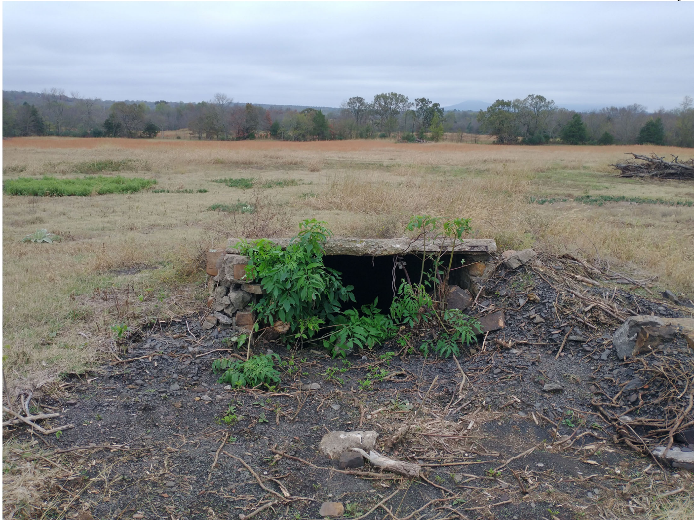
Looking south at abandoned coal shaft entry (November 2024)
