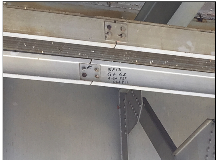
Span 13, Ahead of Pier 12, Walkway: Repaired bolt.
