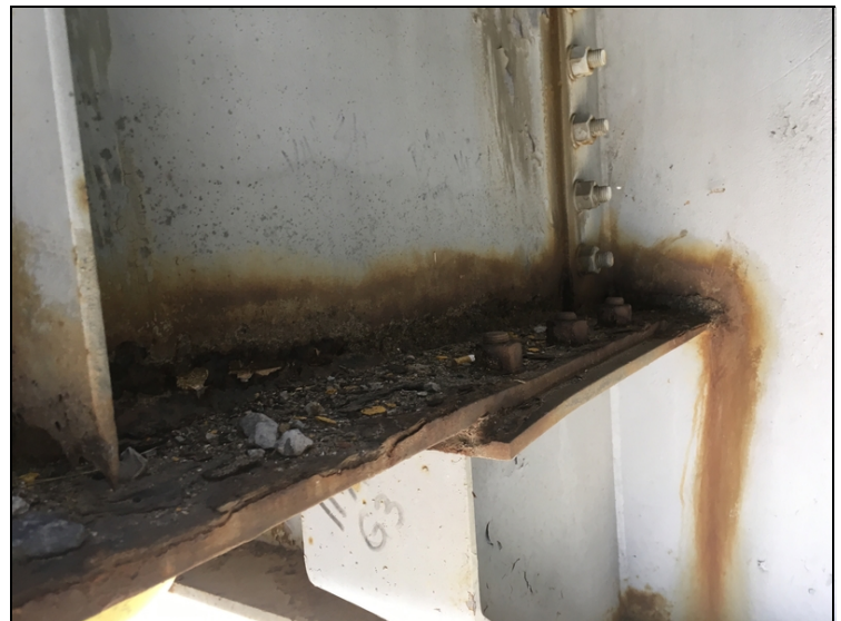
Joint 11 (Girder 3) floor-beam has active corrosion and holes rusted through the web. The bottom flange has approximately 1/8" section loss.
