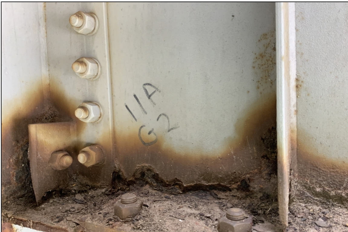
Span 11 Girder 2 Floor beam connection advanced section loss
