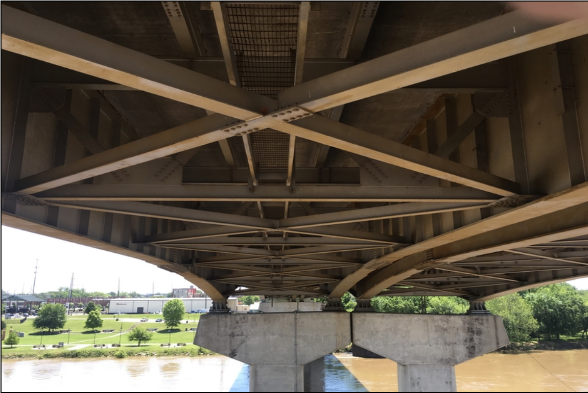
Span 11 and 12 cross frame typical.
