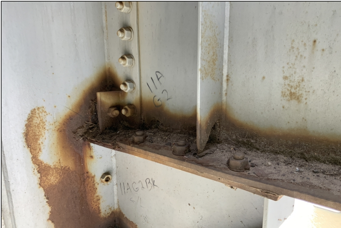
Span 11 2 Second floor beam active corrosion
