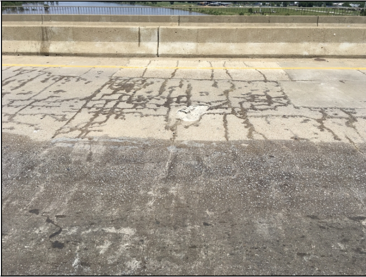
Span 10 (Eastbound - Inside lane) has a deep spall with exposed reinforcing steel in the wheel path.
