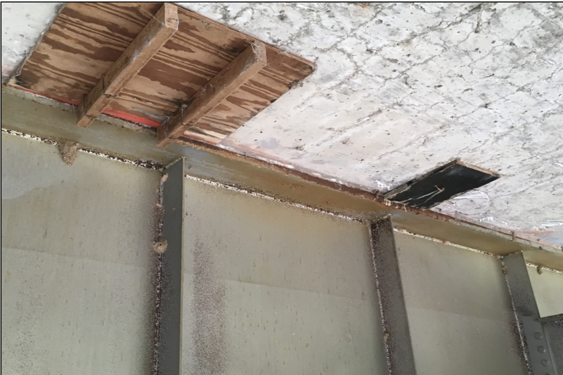
Span 3 & 4 (Girder 1) top flange has active corrosion from the leaching through the deck.
