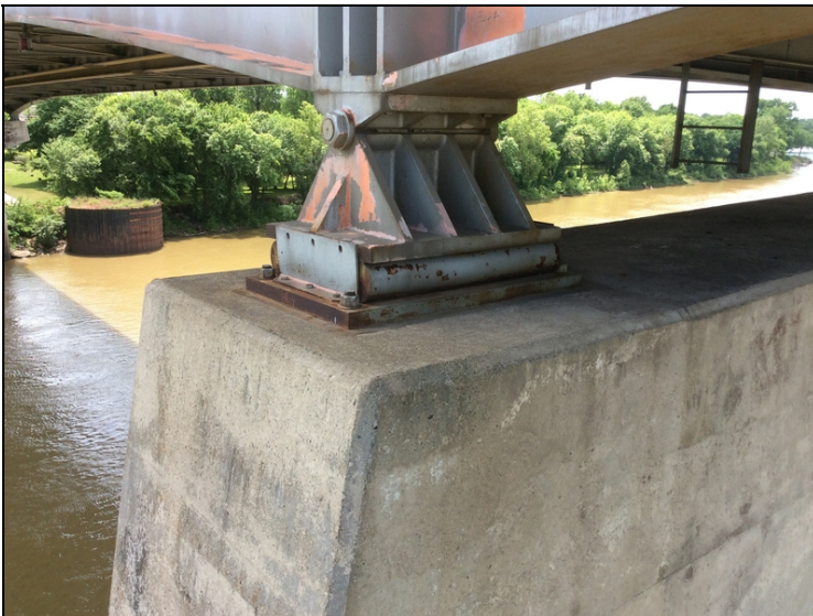
Pier 12 girder 1 bearing. Typical condition of all bearings.
