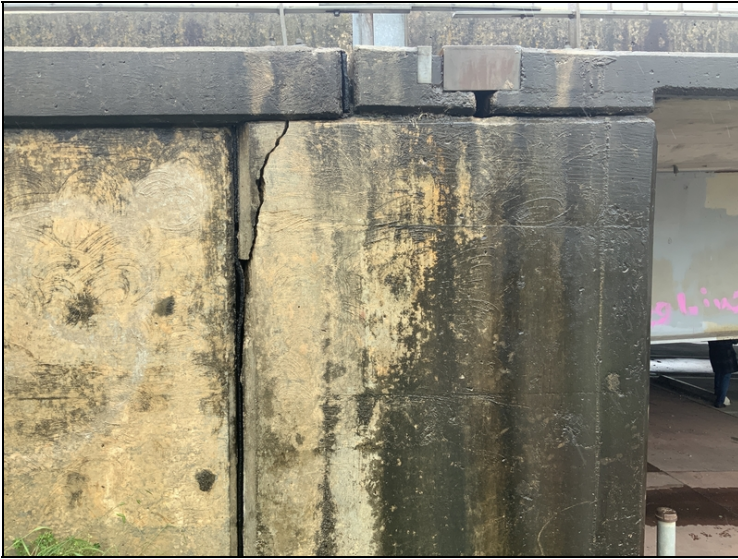
Abutment 2 left wing wall cracking.
