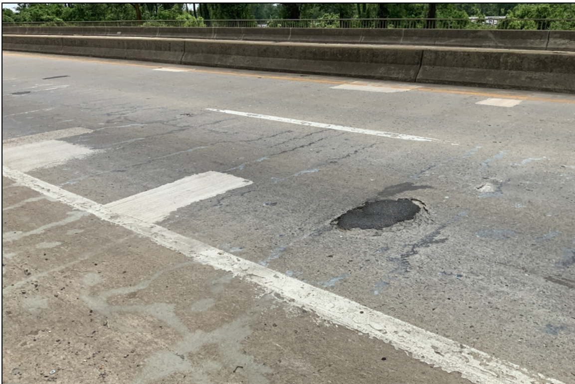
Span 2 Left LRge potholes forming
