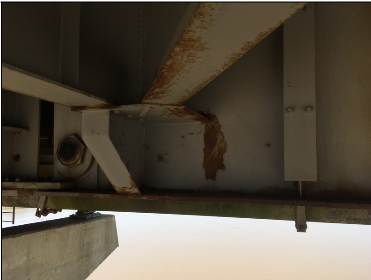
Joint 11 (Girder 2) has active corrosion with light flaking rust to the bottom flange and floor-beam connections.
