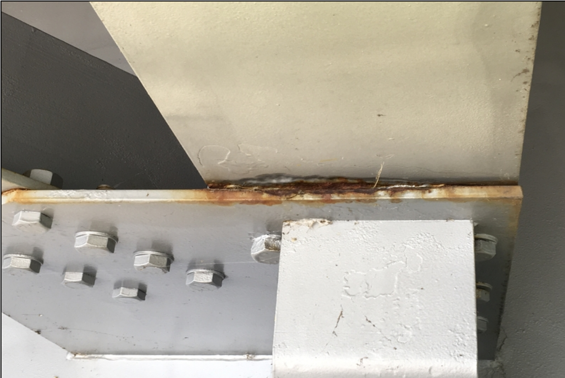
Span 8 (3rd Floor-beam ADH of bent 7) has old section loss scars that has been painted over by maintenance forces with additional corrosion and section loss to the bottom flange of the floor-beam (approximately 1/8" section loss total)
