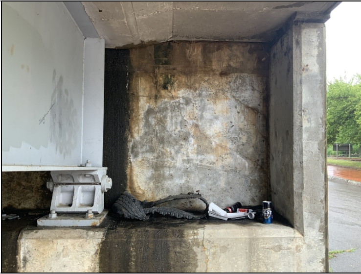
Abutment 2 diagonal cracking in wing wall juncture.
