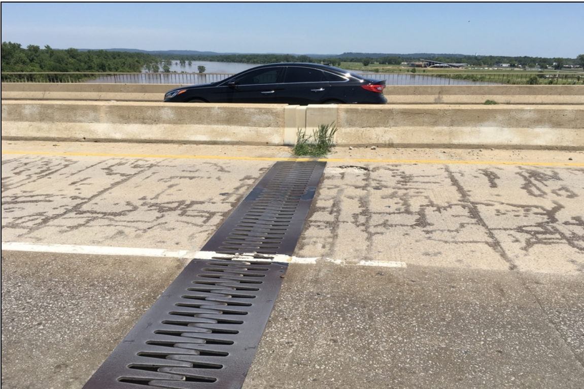
Joint 11 (Eastbound - Inside lane) adjacent to the assembly joint there is a deep spall with exposed reinforcing steel that is in the wheel path on the driving surface.
