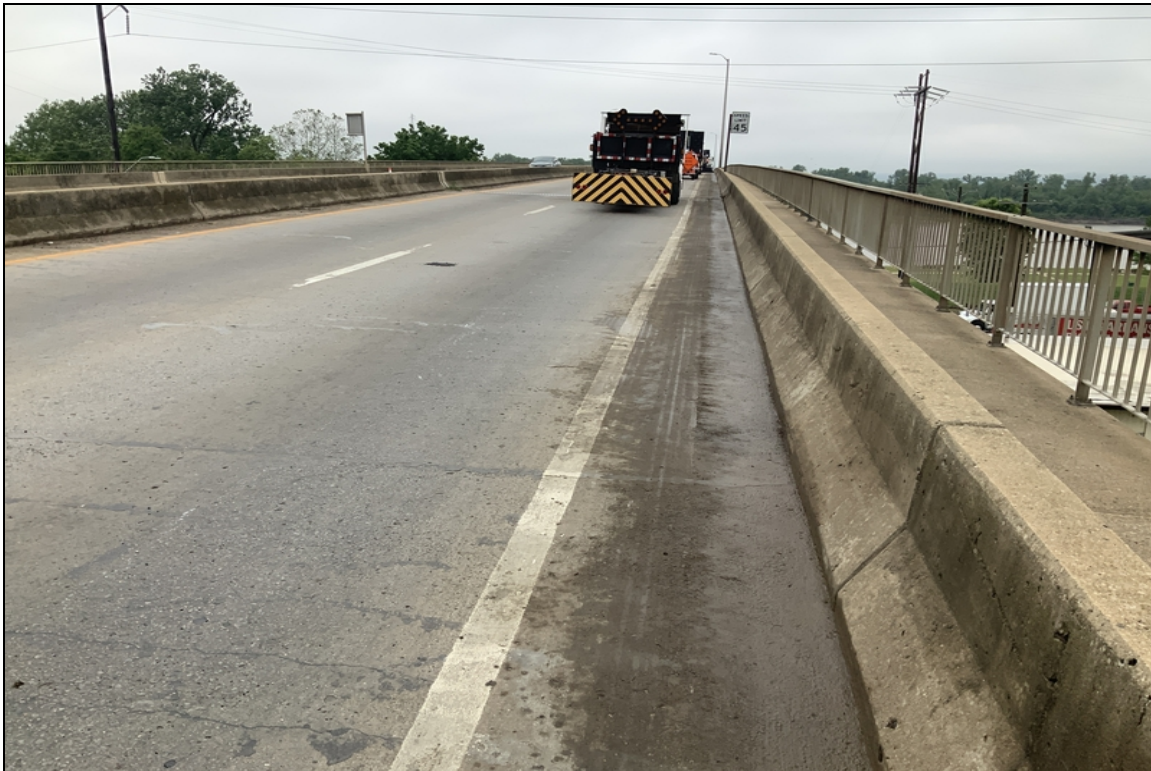
Typical deck with Maintenance forces cleaning gutters and deck drains patching spalls.
