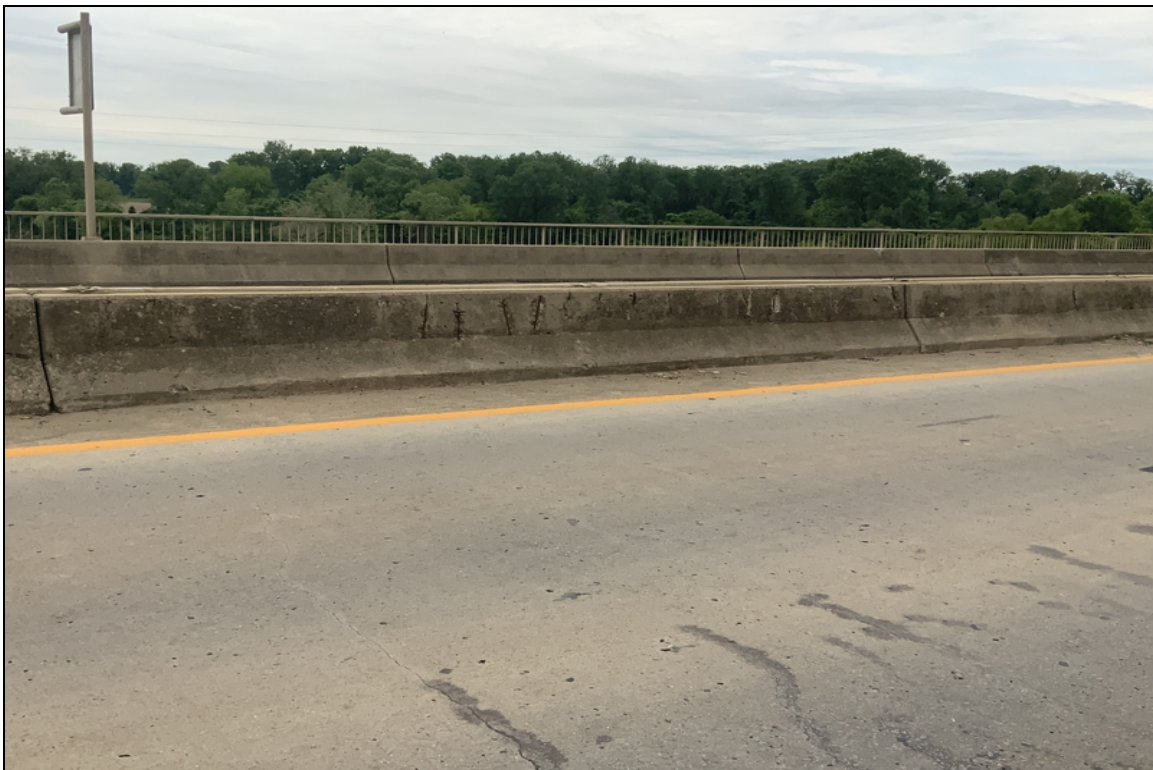
Spalling in parapet walls typical throughout structure.
