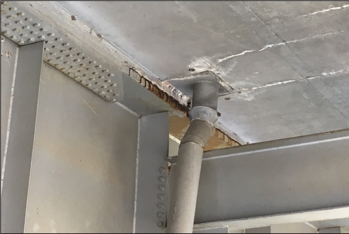
Span 11 (Girder 1) has active corrosion to the top flange (typical at all the drain locations).
