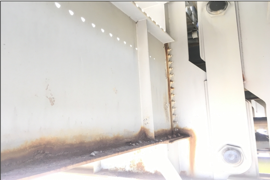
Joint 11A floor-beam bottom flange between girders 3 & 4 has active corrosion along the web and bottom flange with section loss (Typical throughout this floor-beam).
