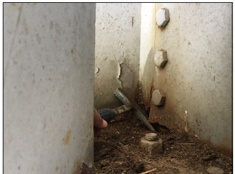
Joint 11 (Girder 3) floor-beam has approximately 1/2" pack rust to the web girder juncture along with a 4" hole that has rusted through the web at this location.
