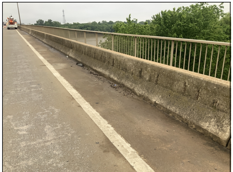
Span 7 Eastbound spalling with exposed reinforcing steel parapet wall.
