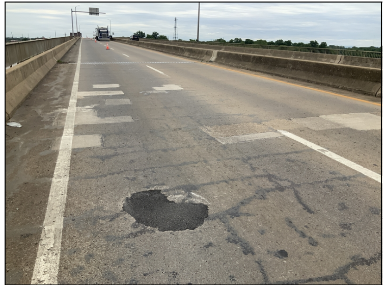
Bent 7 westbound spall with asphalt repair.
