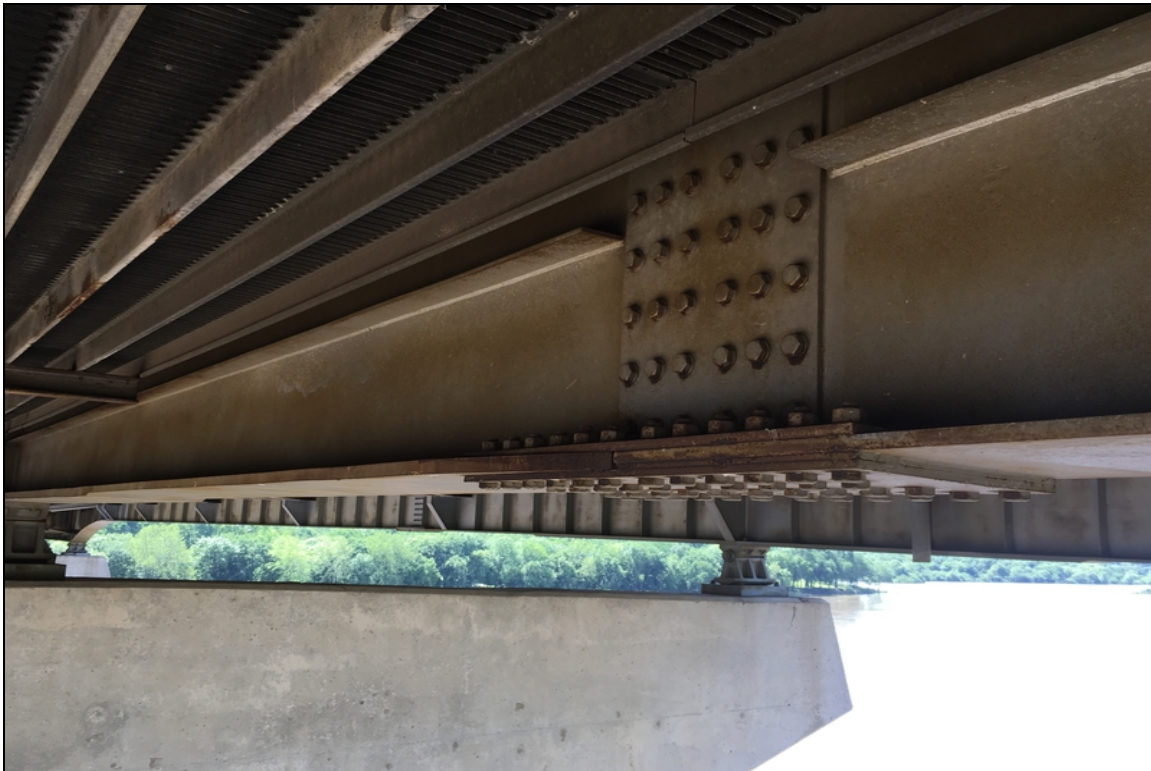
Span 9 (Girder 3 &ndash; 2nd splice plate &ndash; AHD of Bent 9) has active corrosion (Typical with all the splice plate connections throughout the structure).
