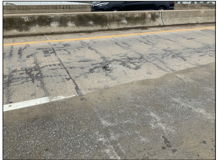
Span 8 eastbound spall. 2' CS-3
