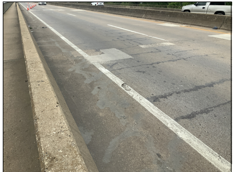
Span 5 west bound spall/delaminated 4' area .
