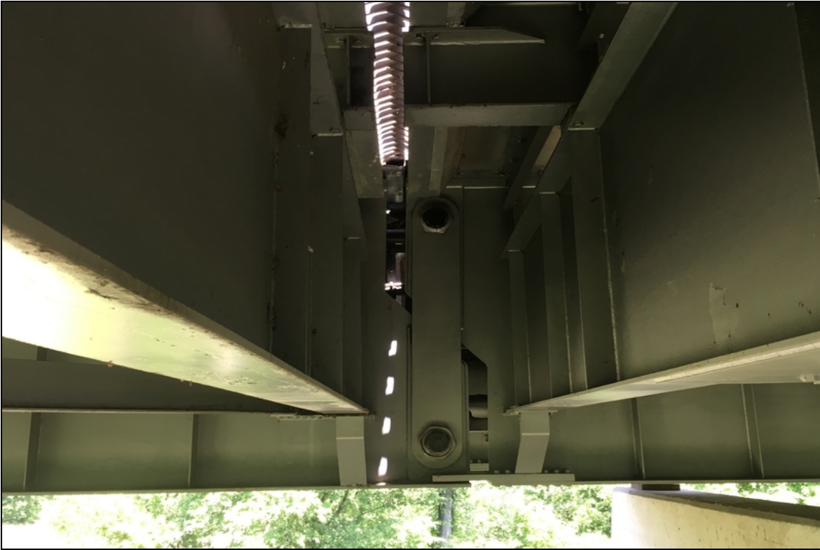
The hangers and parts of the girders adjacent to Bent #4 have been painted (no apparent visible rust at this inspection).
