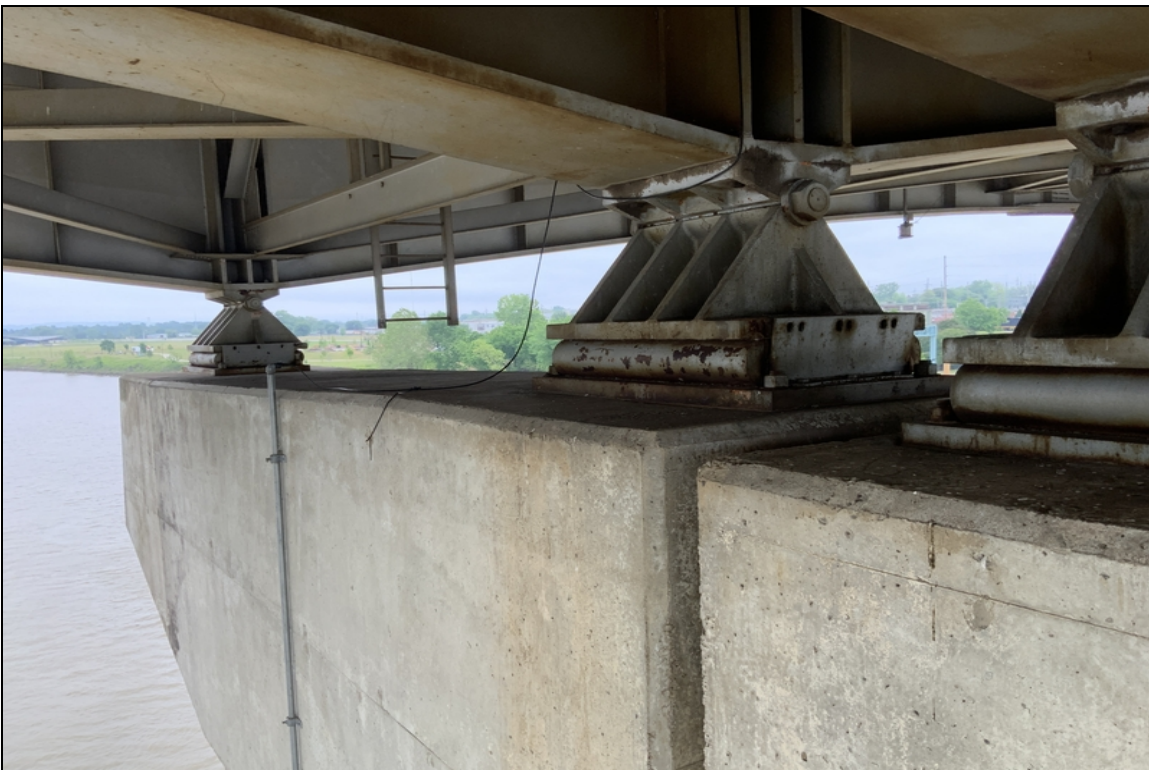
Bent 12 Active corrosion in bearings
