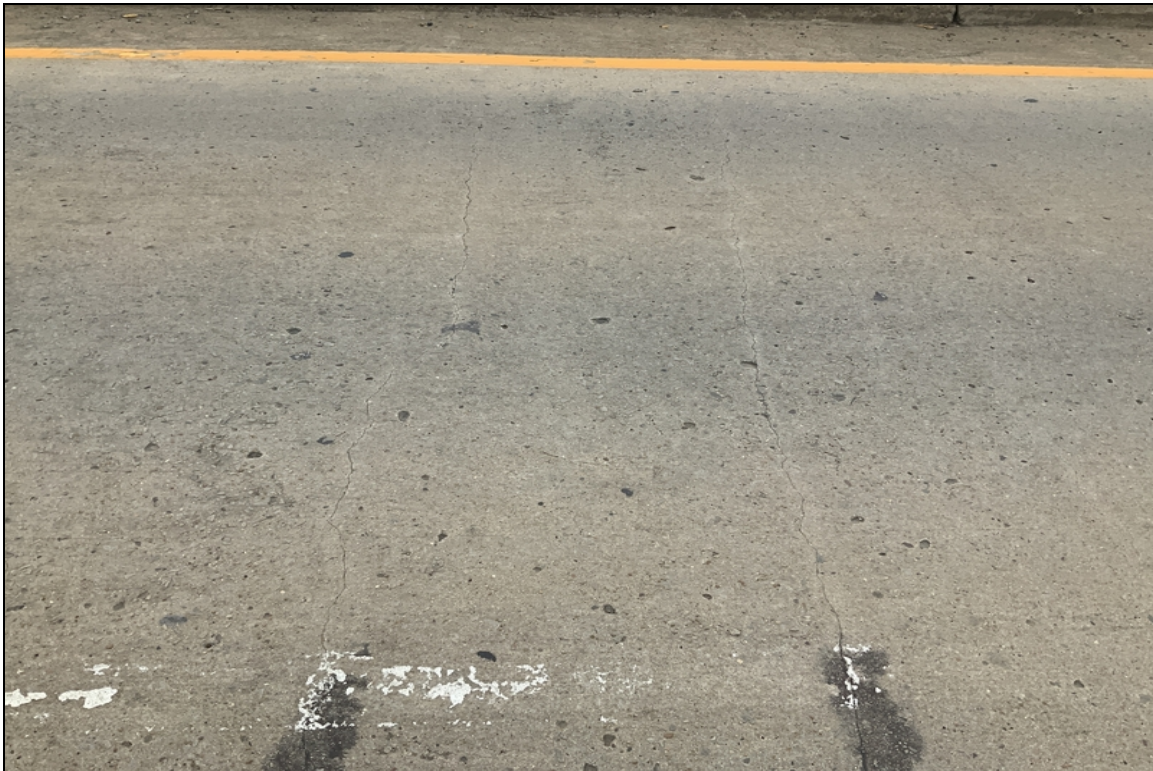
West bound outside lane sealable deck cracking.
