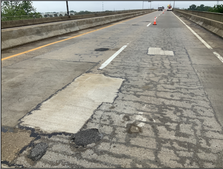
Span 6 eastbound 30' CS-3 spalls with asphalt repairs.
