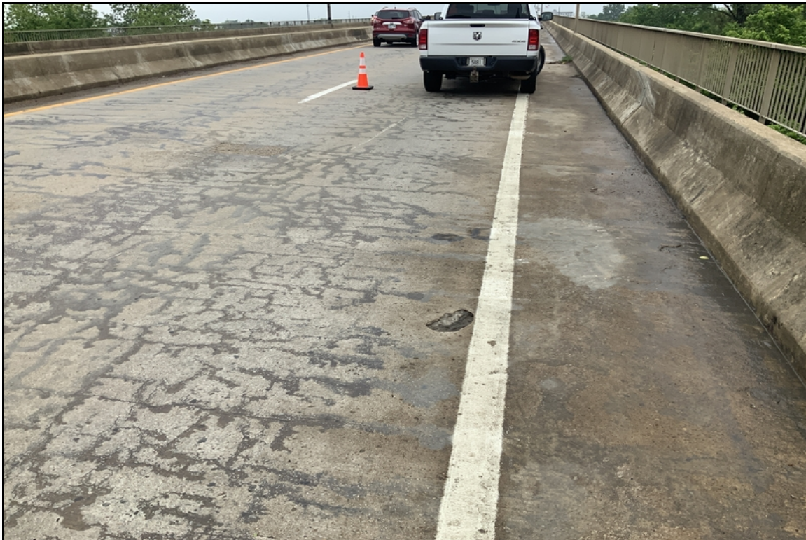
Span 5 eastbound 1' spall. CS-3
