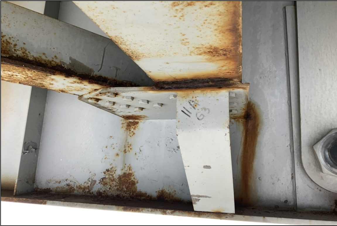
Span 11 Girder 3 Floor beam active corrosion.
