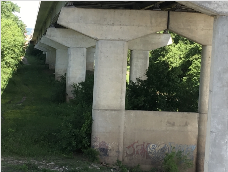
Pier 1-7: Vegetation growing on columns. Typical.
