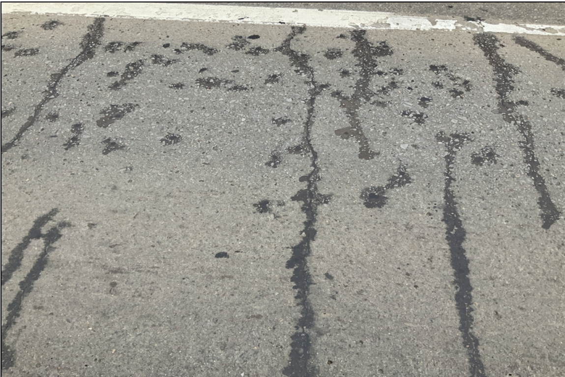
Sealed cracking that has failed this is typical throughout structure.
