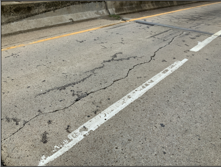
Bent 1 enact bound approach slab large longitudinal crack.21' CS-3
