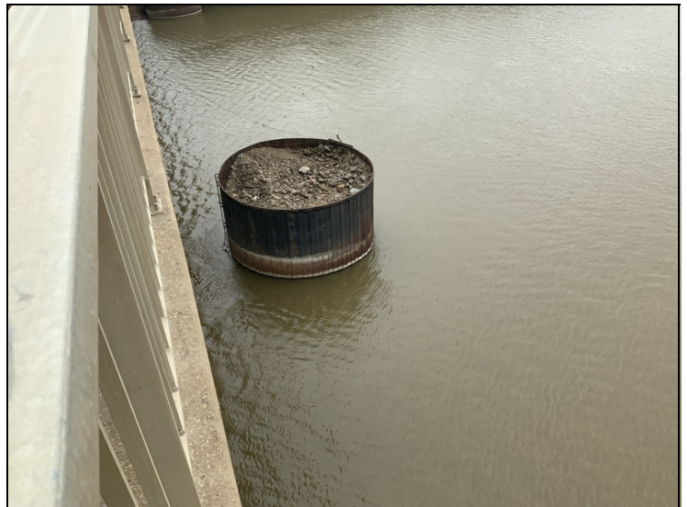
Bent 12 Upstream pier protector missing fill material.
