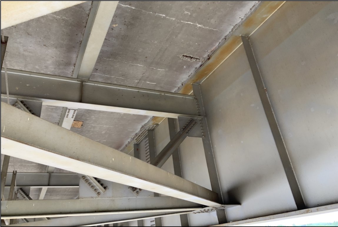
Span 12 Spalling in the undersurface
