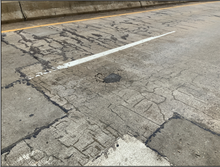
Span 1 eastbound 2x2 spall that has failed with asphalt patch.
