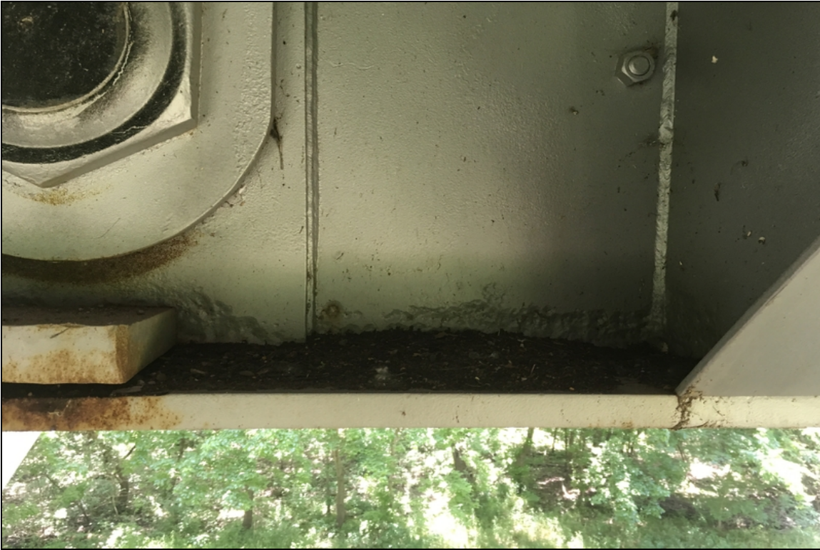
Bent 4 (Girder 2) has old section loss scars that are still present (maintenance forces have cleaned and painted this area).
