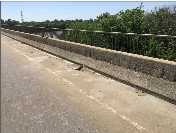
Span 5, Eastbound: Spalling in concrete portions of bridge railing.
