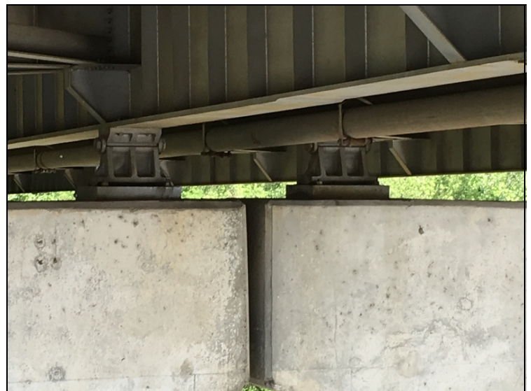
Bearings: Typical corrosion.
