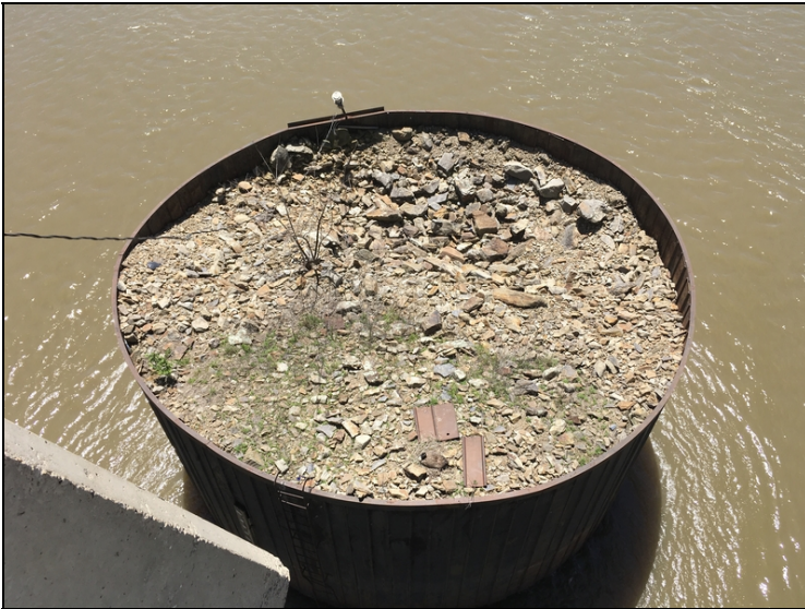
Pier 12, Upstream: Rock fill missing from the cell. Access ladder damaged near the waterline.
