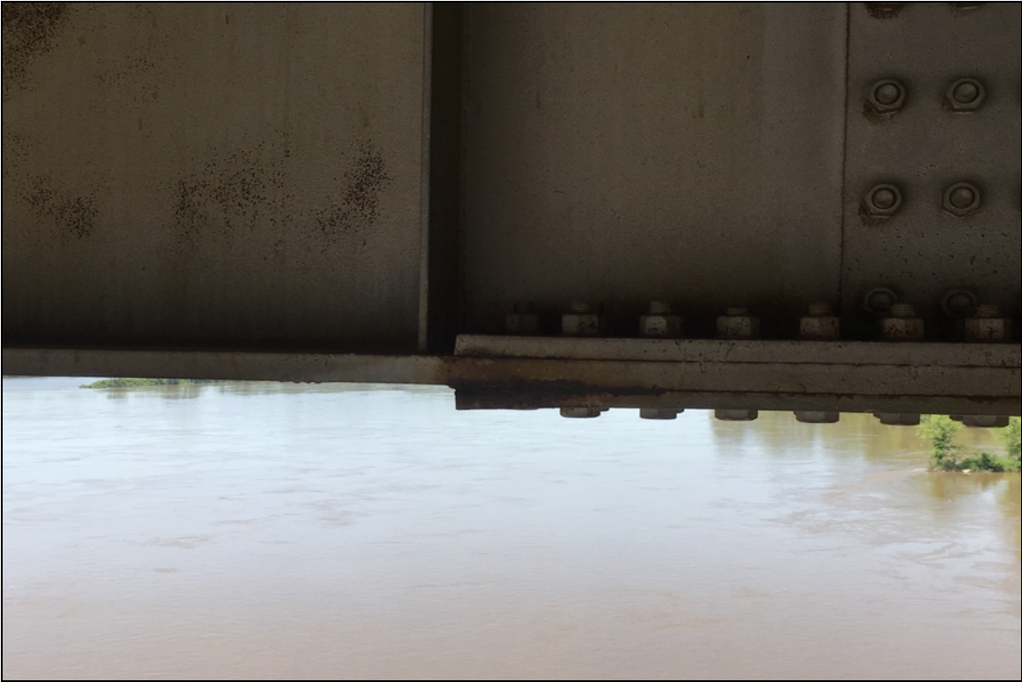
Span 10 (Girder 4 &ndash; AHD of Bent 10) has approximately \frac{1}{4} " pack rust with out-of-plane bending to the 1st splice plate.
