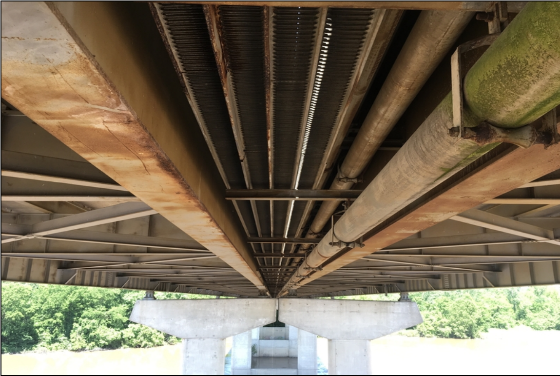
Span 10 (Girders 3 & 4) paint system is failing with light rust showing (typical throughout the structure).
