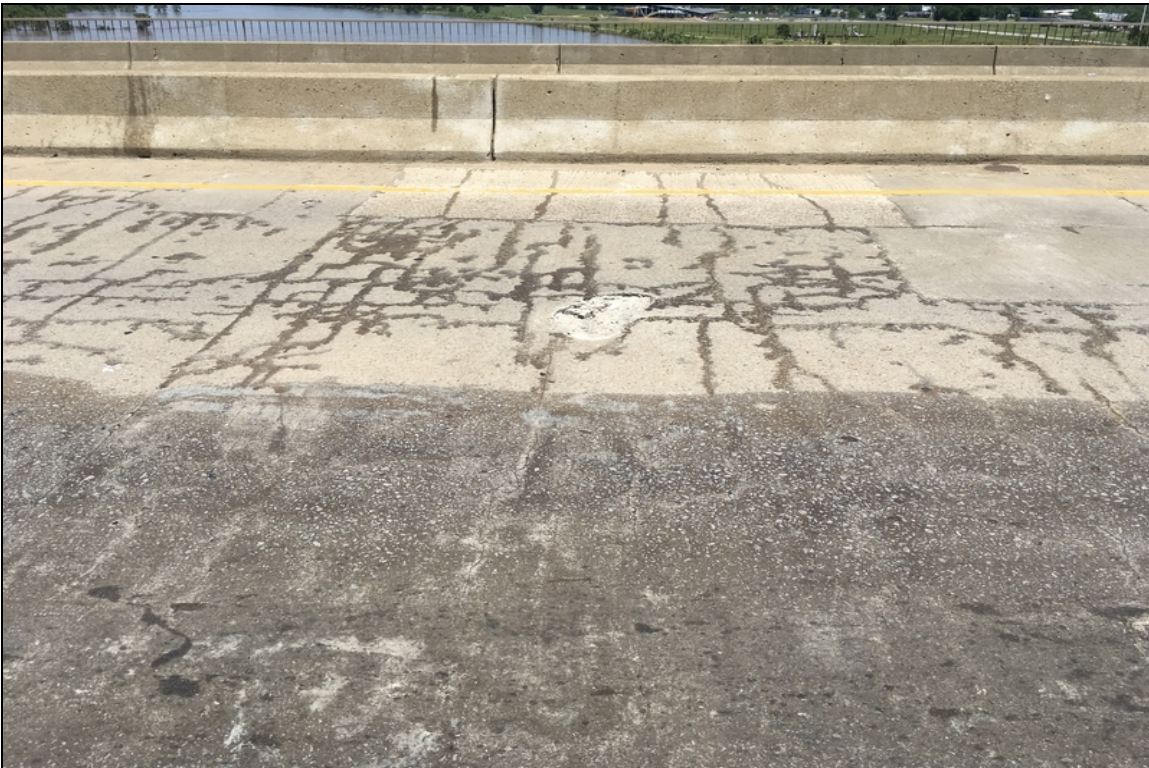
Span 10 (Eastbound - Inside lane) has a deep spall with exposed reinforcing steel in the wheel path.
