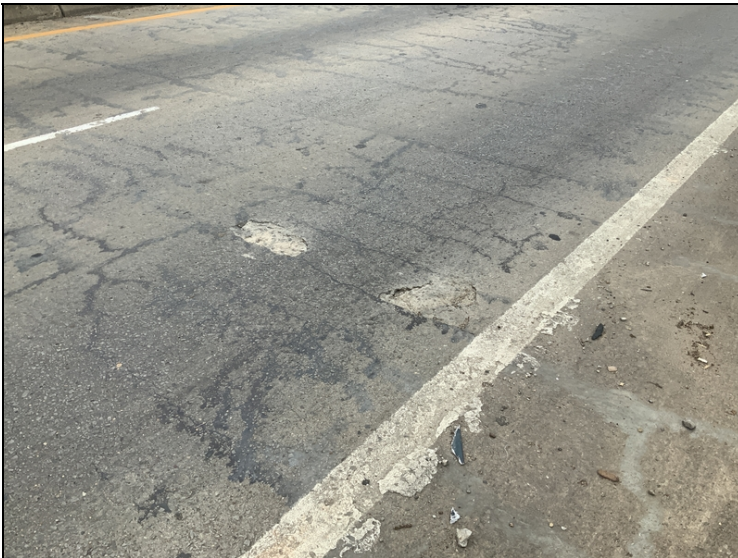
East Abutment 4' CS-3 spalling.
