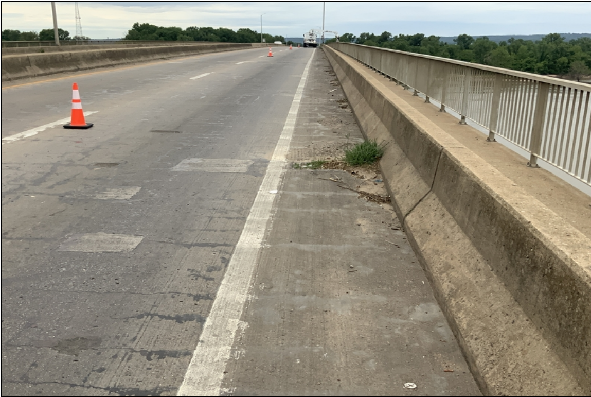
Deck drains full of dirt and debris this is typical with all joints.
