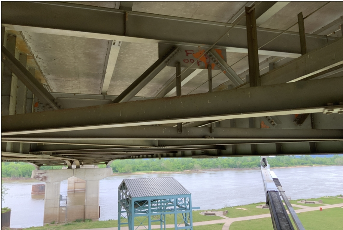
Span 13 Flaking paint
