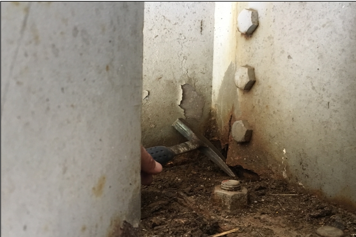
Joint 11 (Girder 3) floor-beam has approximately 1/2" pack rust to the web girder juncture along with a 4" hole that has rusted through the web at this location.
