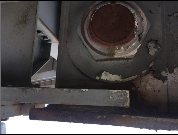
Joint 11 (Girder 3 wind-lock) has approximately 1" of pack rust accumulation between the bottom flange of girder 3 at the wind-lock. Appears pin is froze up at this location.
