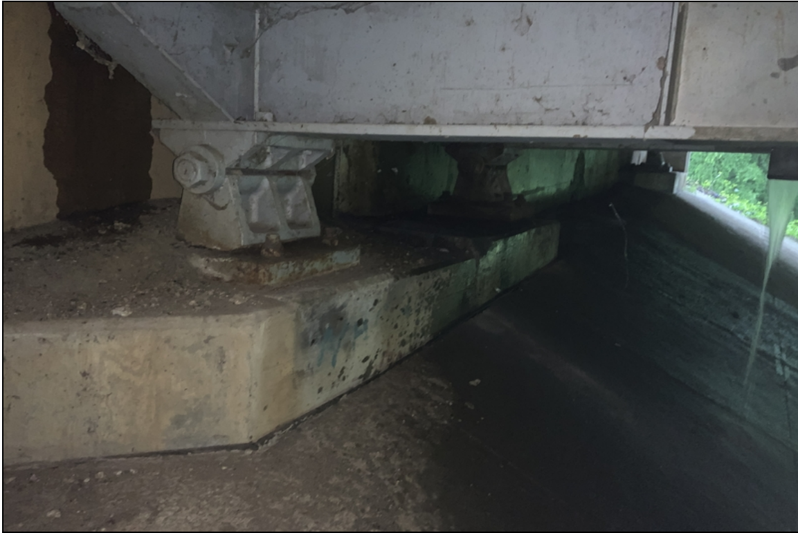
Abutment 1 girders 3 and 4 active corrosion with flaking rust.
