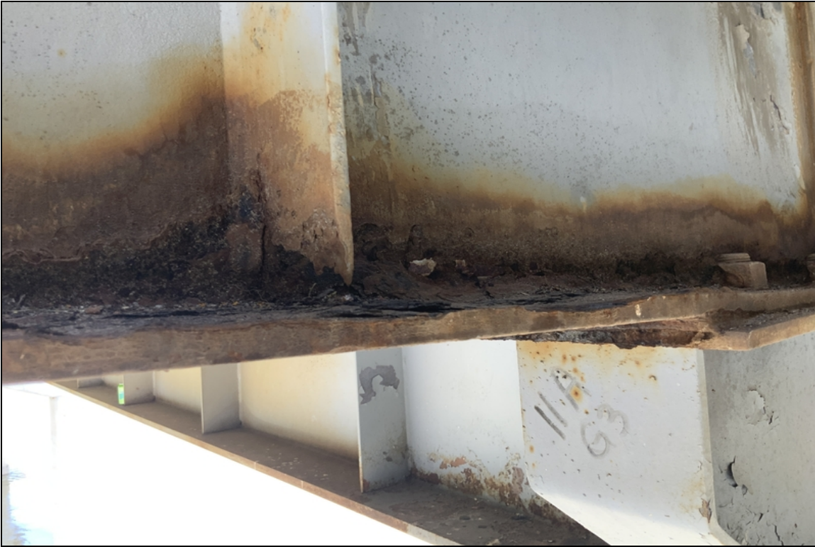
Span 11, Girder 3, Floor Beam Web, At Pin & Hanger: Holes rusted through.
