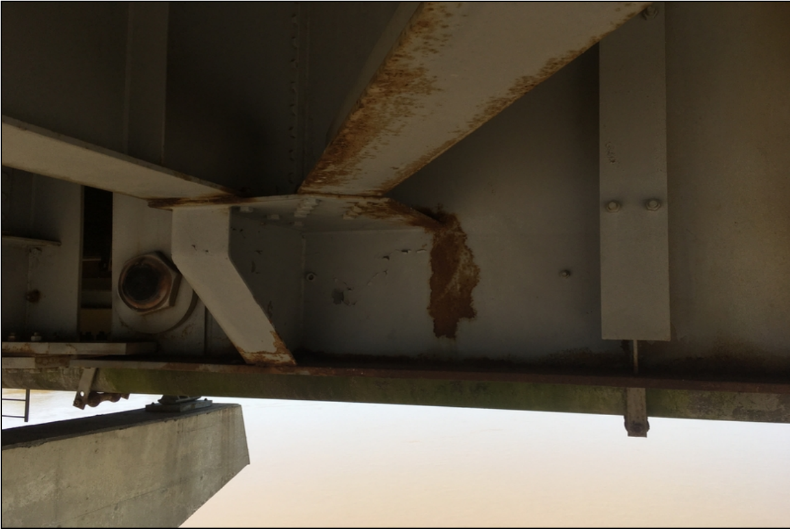
Joint 11 (Girder 2) has active corrosion with light flaking rust to the bottom flange and floor-beam connections.
