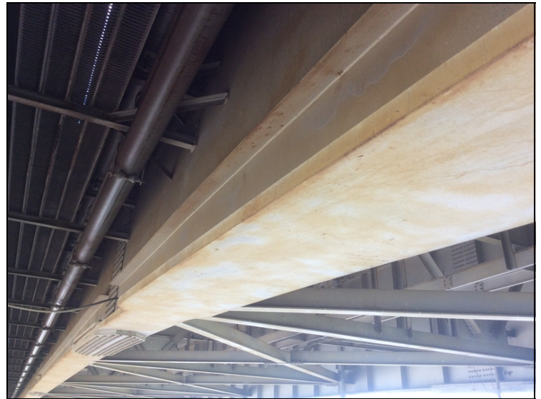
Span 13 Girder 2 typical paint condition.
