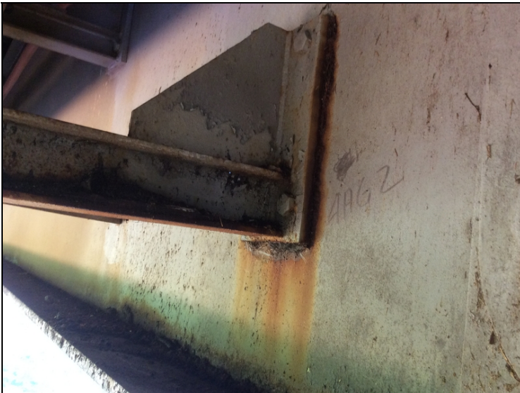
At G2 pack rust at the cantilevered inspection platform to girder connection.
