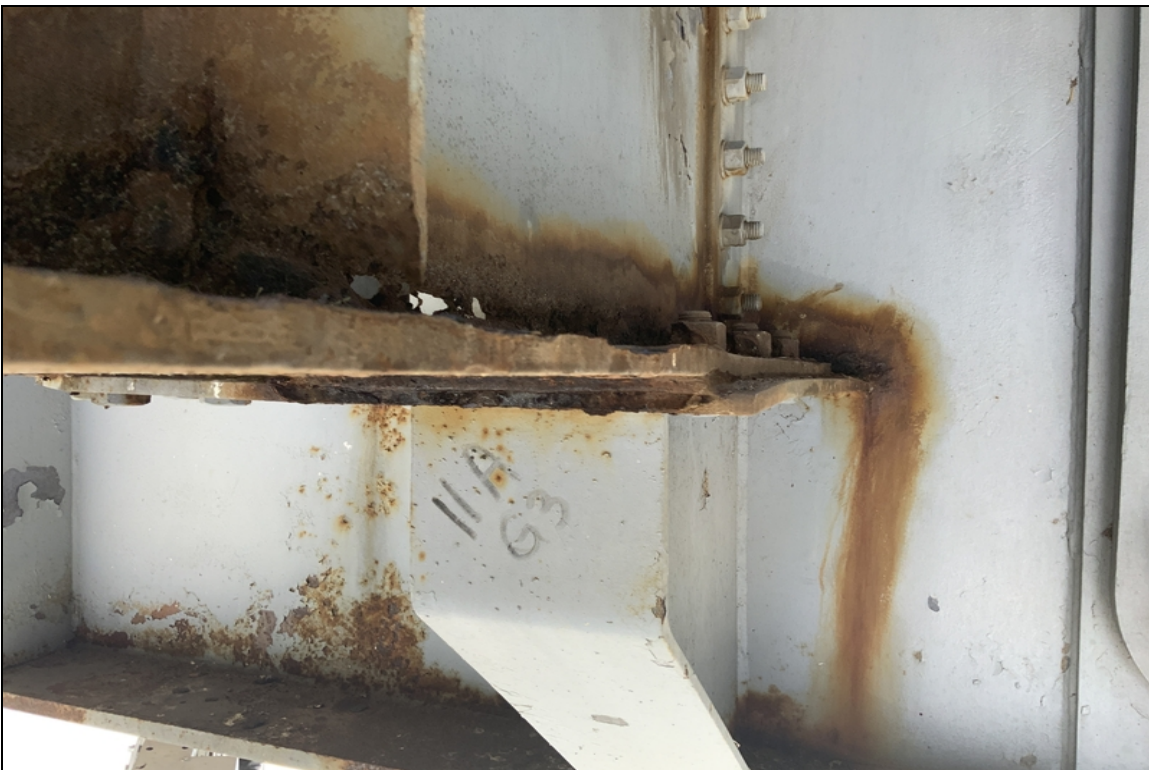
Span 11, Girder 3, Floor Beam Flange: Up to 5/16" section loss.
