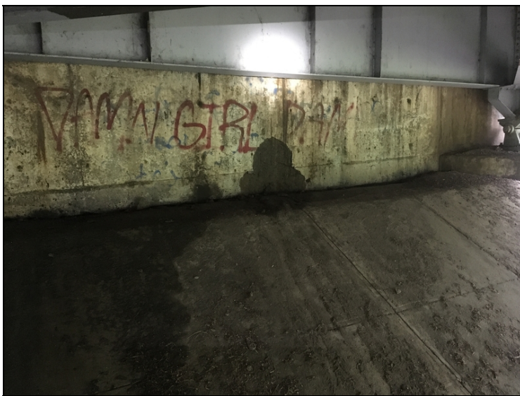
Abutment : Spalling in the back wall with minor vertical cracking.
