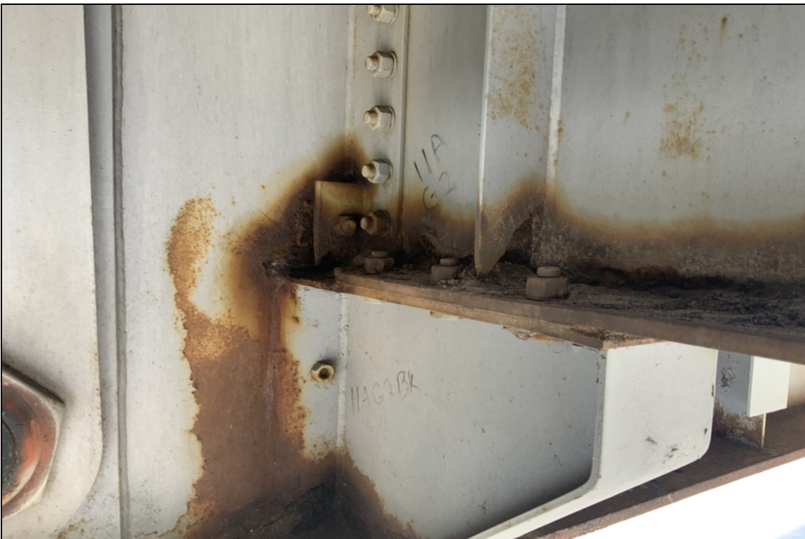
Span 11 Girder 2 1/4" section loss to web, bottom flange
