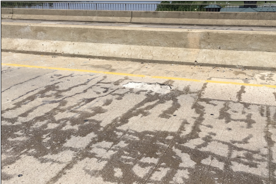
Span 12 (Eastbound-inside lane) has a deep spall with exposed reinforcing steel that is in the wheel path on the driving surface.
