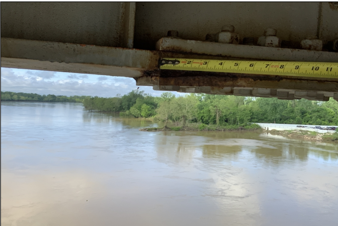
Splice plate corrosion with pack rust
