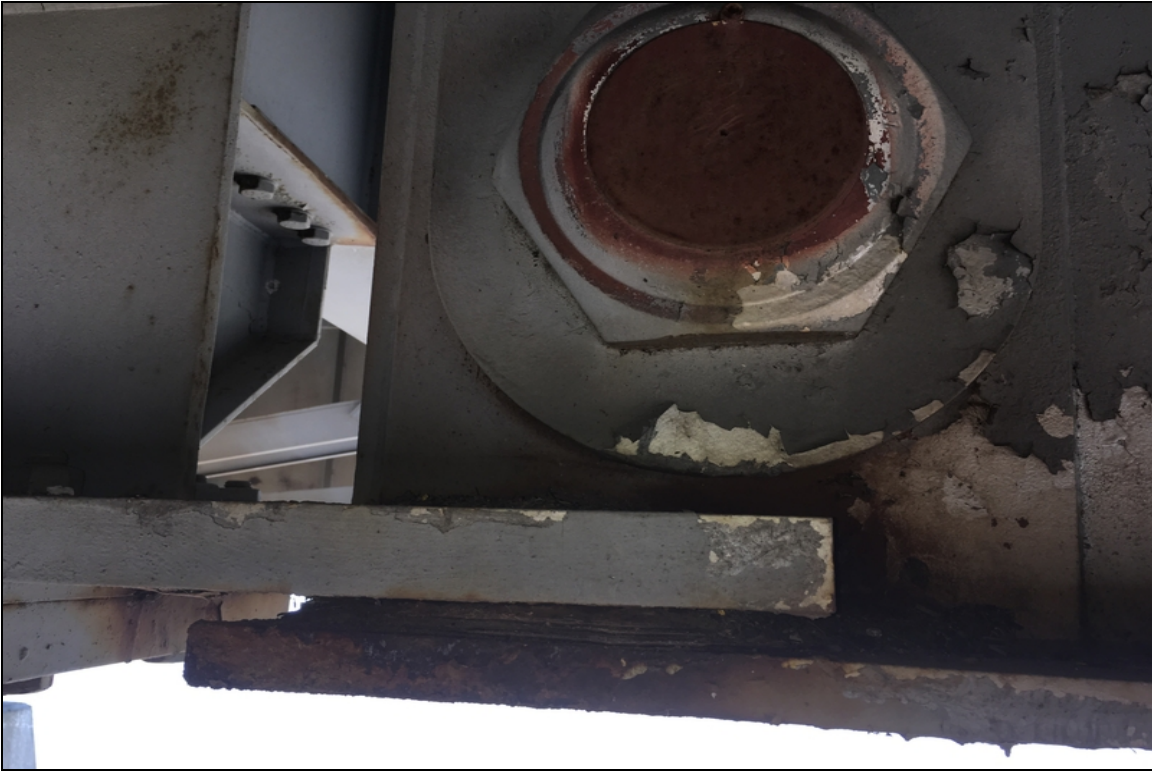
Joint 11 (Girder 3 wind-lock) has approximately 1" of pack rust accumulation between the bottom flange of girder 3 and the wind-lock.
