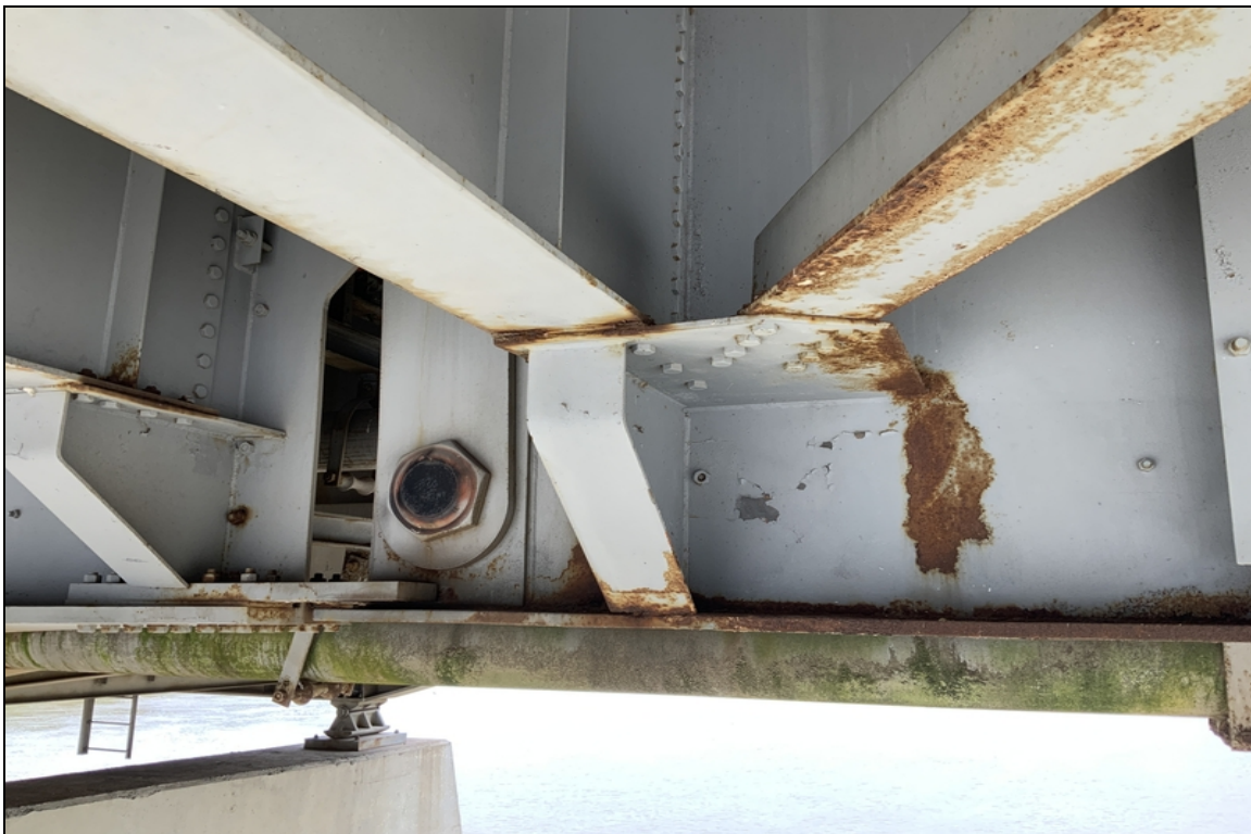
Span 11 Girder 2 Active corrosion
