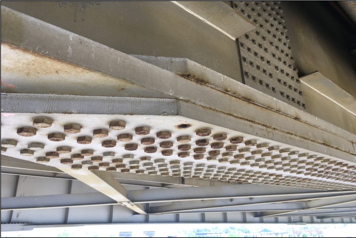
Span 12 (Girder 2 &ndash; 1st splice plate &ndash; AHD of Bent 12) has one missing bolt.
