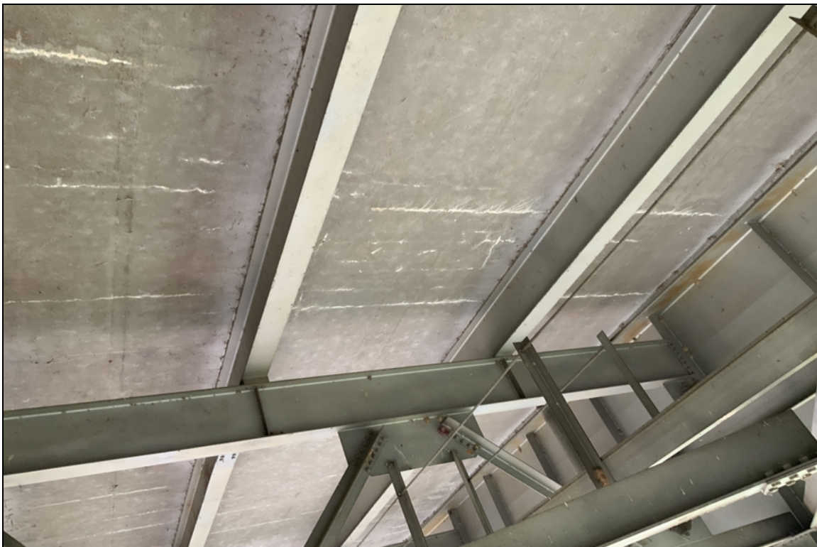
Typical undersurface efflorescence
