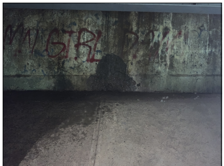
Abutment 1 left spall on the back wall
