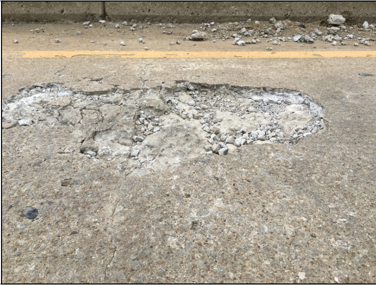
Span 3 (Westbound - Inside lane) has a deep spall with exposed reinforcing steel that is in the wheel path.
