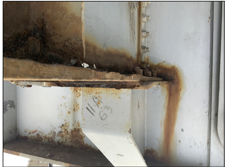
Span 11, Girder 3, Floor Beam Flange: Up to 5/16" section loss.
