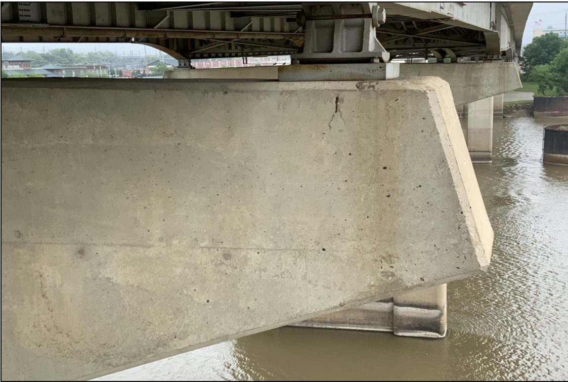
Bent 10 Right Spalling with exposed reinforcing steel
