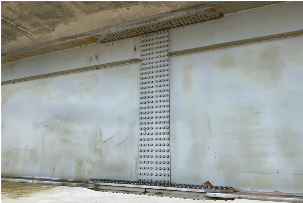
Span 11 Typical splice
