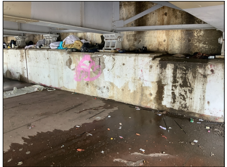
Abutment 2 spalling with exposed reinforcing steel.
