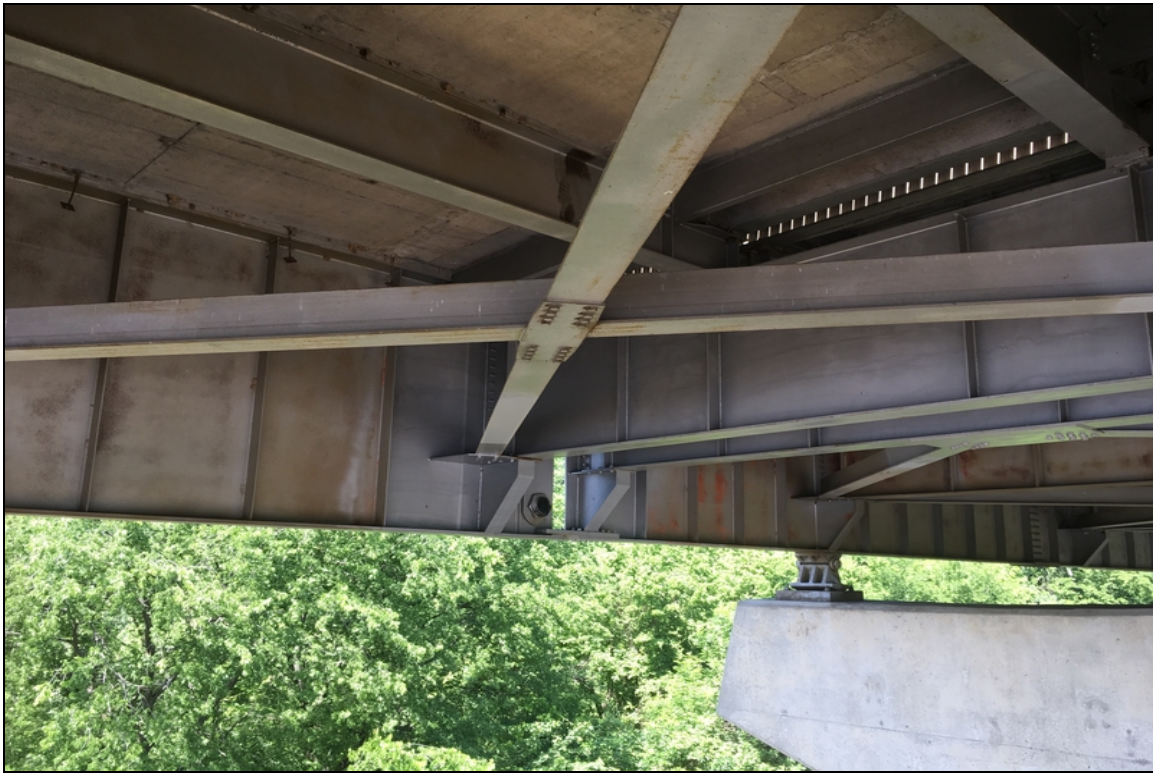
Joint 7 has recently been cleaned and painted.
