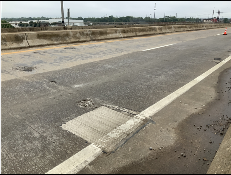
Span 13 eastbound spalling with asphalt repairs.
