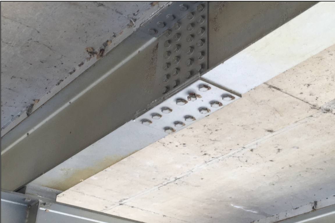
Span 9 (3rd Stringer) has one loose bolt.
