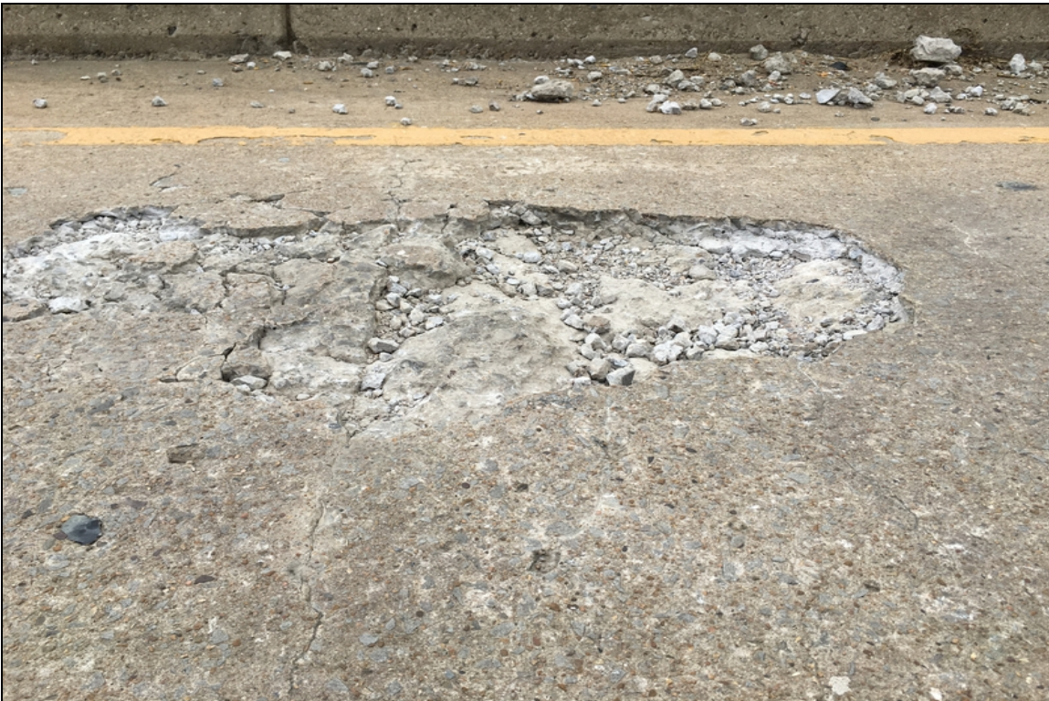
Span 3 (Westbound - Inside lane) has a deep spall with exposed reinforcing steel that is in the wheel path.
