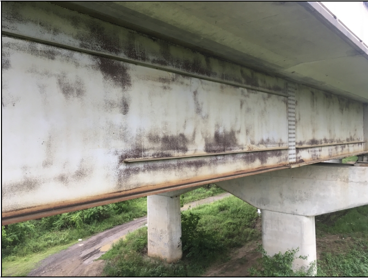
Span 4, Girder 1: Typical beam corrosion.
