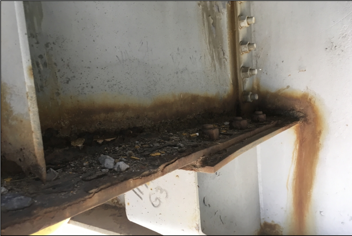
Joint 11 (Girder 3) floor-beam has active corrosion and holes rusted through the web. The bottom flange has approximately 1/8" section loss.
