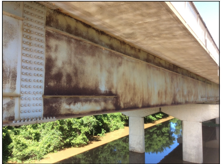
Span 5 girder 1: general paint condition.
