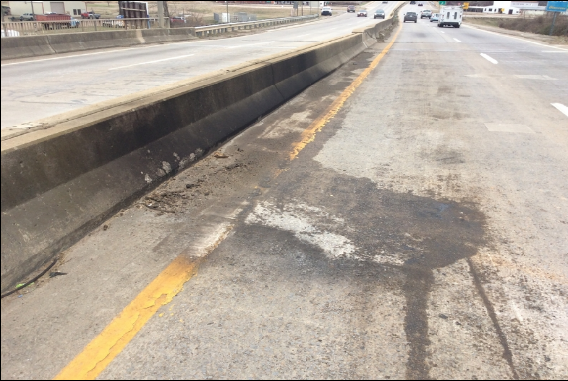
Generally observation of apparent vehicle fire on top of driving surface. No apparent delaminations or spalls at this inspection.
