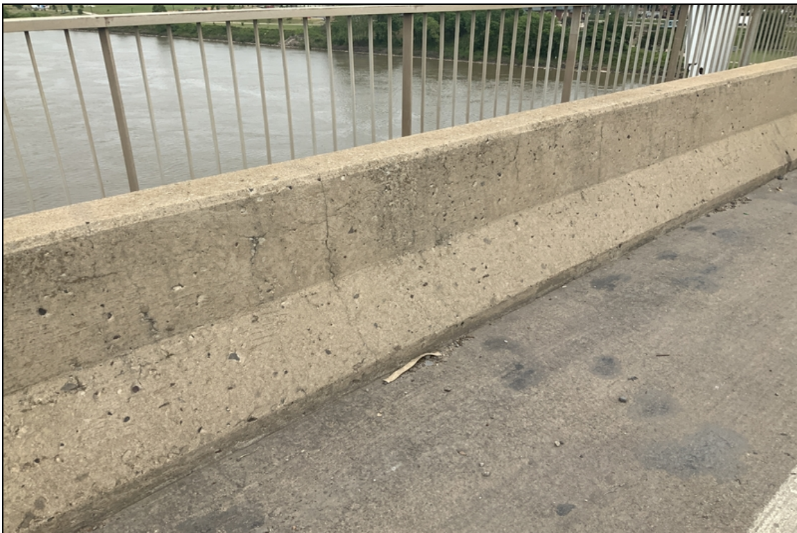
Vertical cracking in parapet wall.
