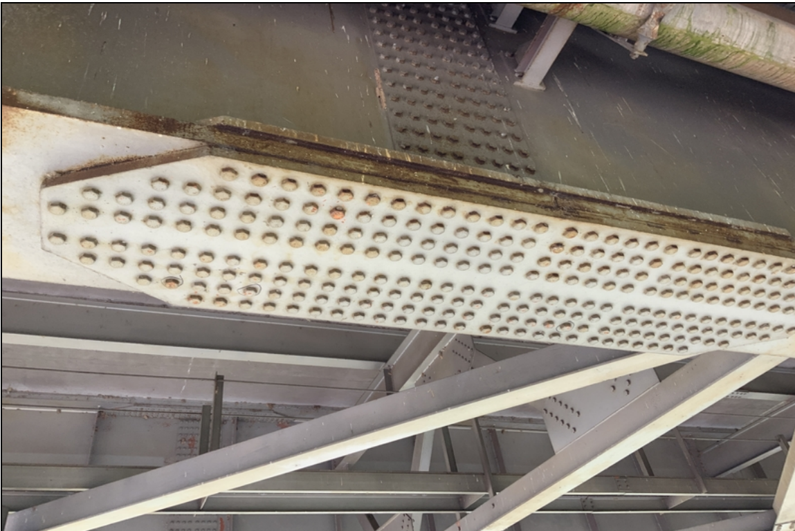
Span 3 Girder 2 Second splice plate loose bolts
