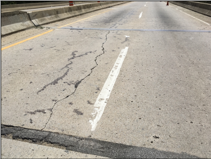
Bent 1, Approach Slab: Cracking with minor settlement.
