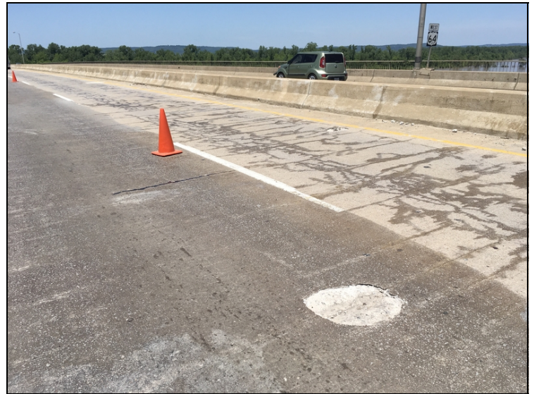
Span 12 (Eastbound) has 3 deep spalls with exposed reinforcing steel that is in the wheel path.
