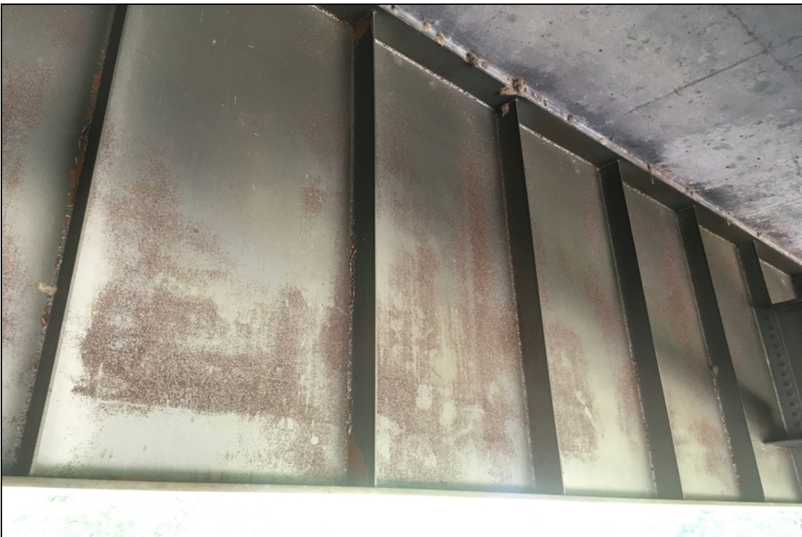
The primer is showing along all the girders throughout the structure (Typical at all locations).
