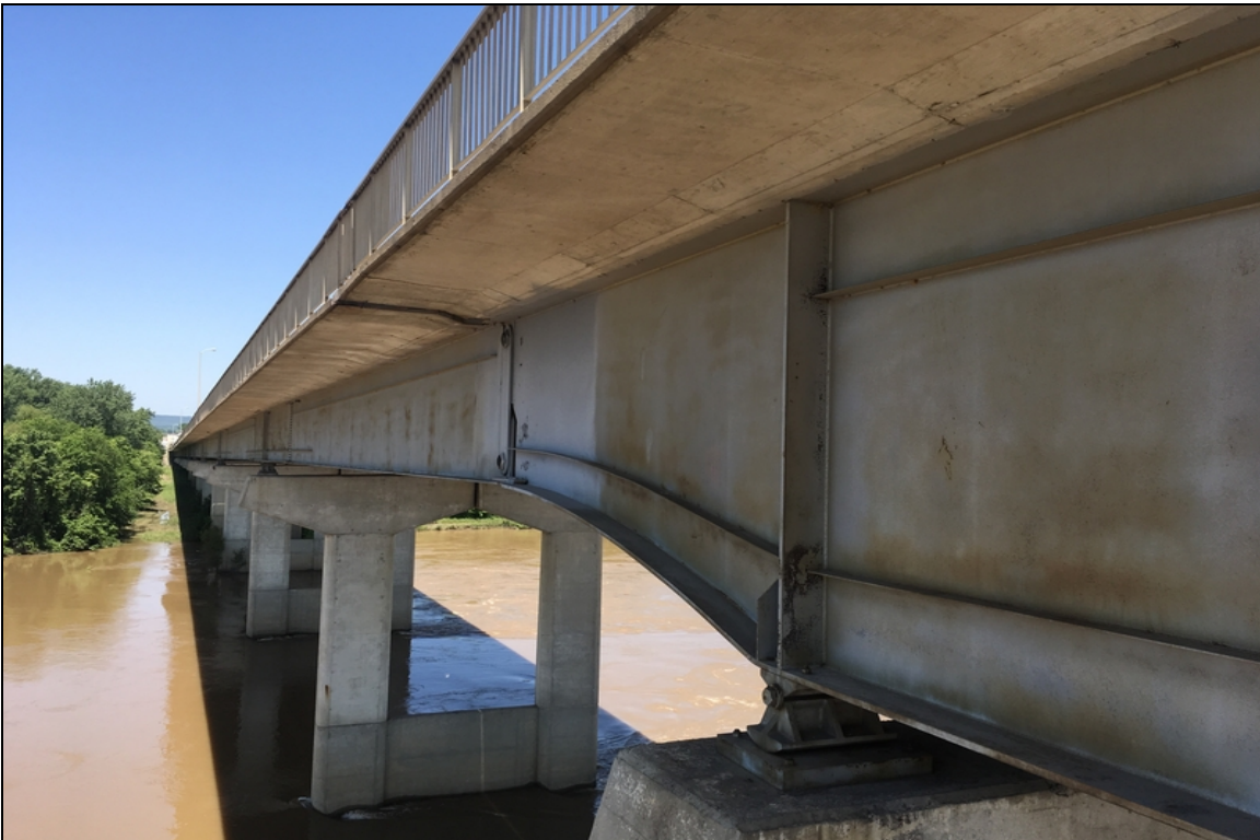
The exterior girders have a failing paint system that is dull, chalky, and has lost its primer along with light rust showing throughout the structure.
