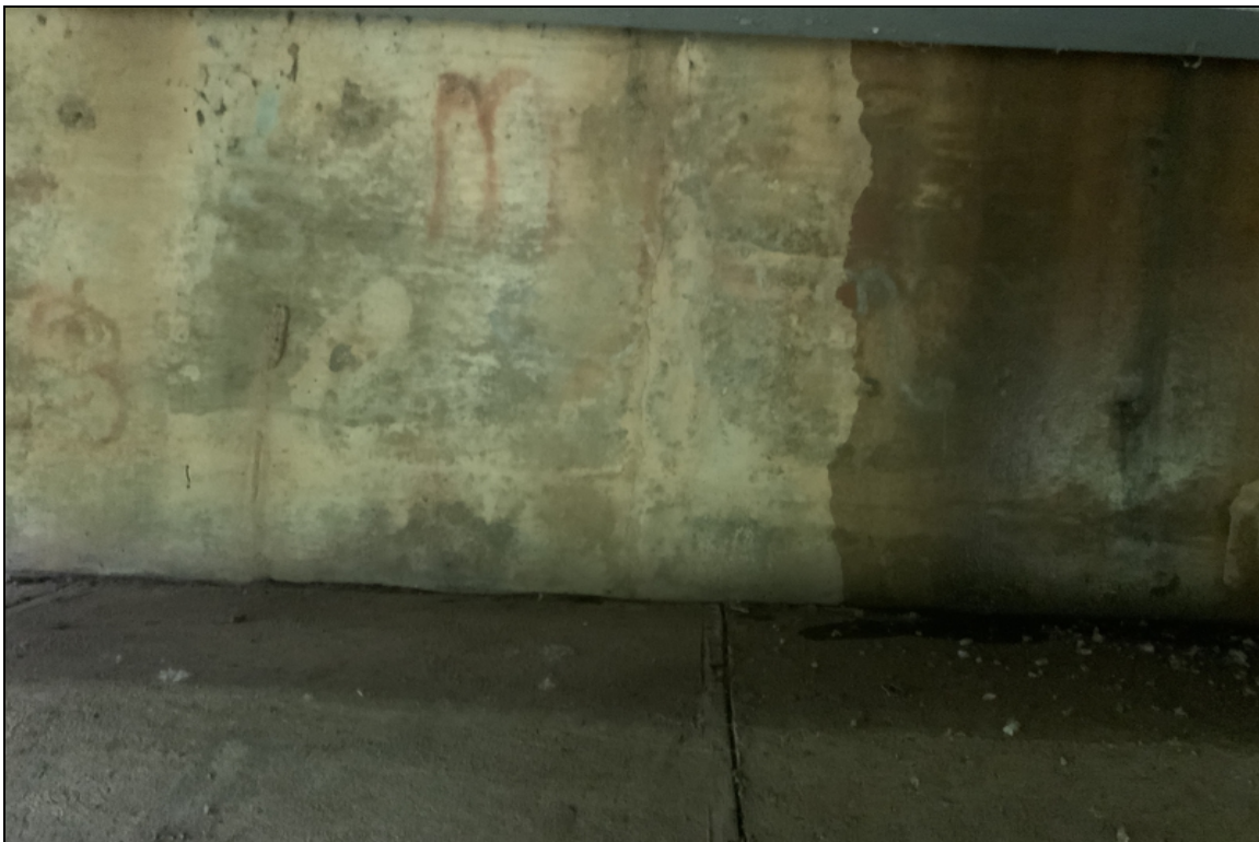
Abutment 1 right vertical crack in back wall
