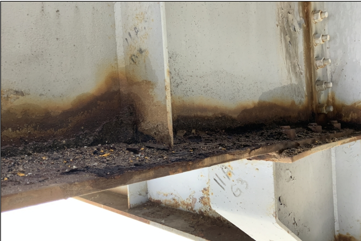
Span 11, Floor Beam back of Pin and Hanger: Active corrosion with holes rusted through.
