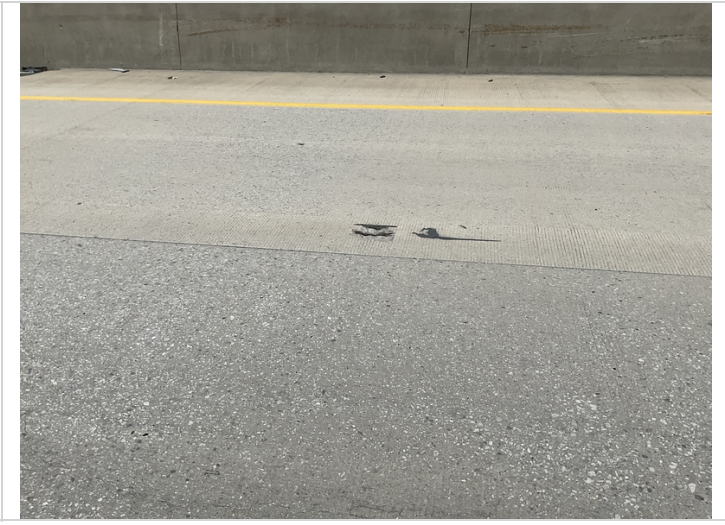
Span 7, missing plowable marker.
