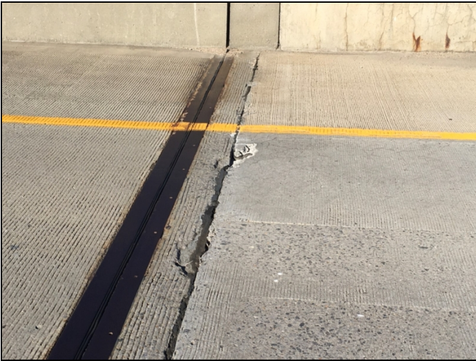
Approach 2: Spalling.
