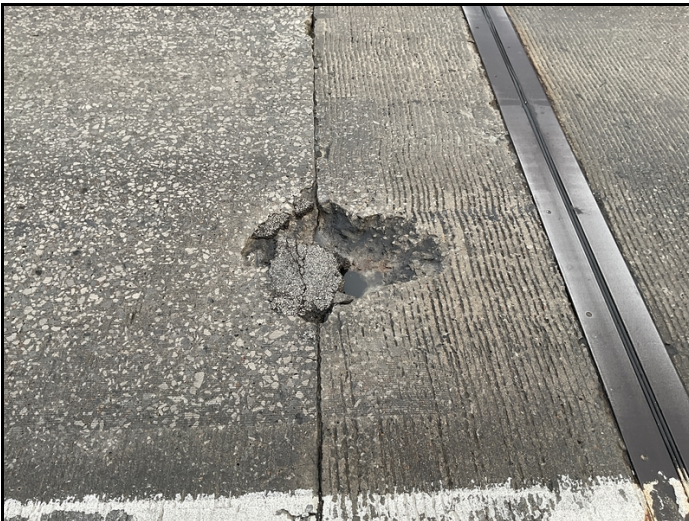
Large spall in the top of the backwall bent 1.
