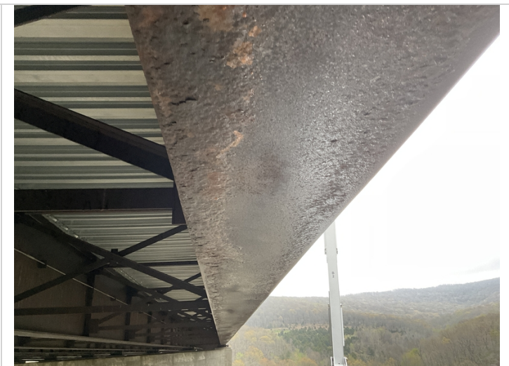
Span 3 girder 4, large flakes in the protective coating.
