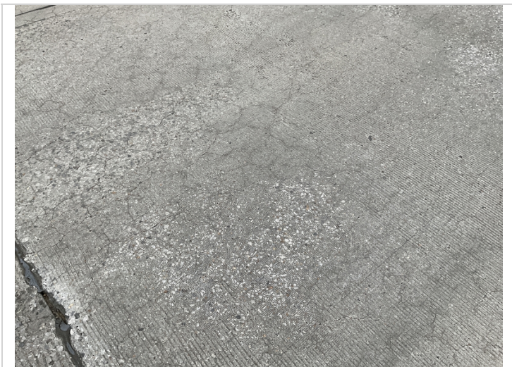
Map cracking in northern approach slab.
