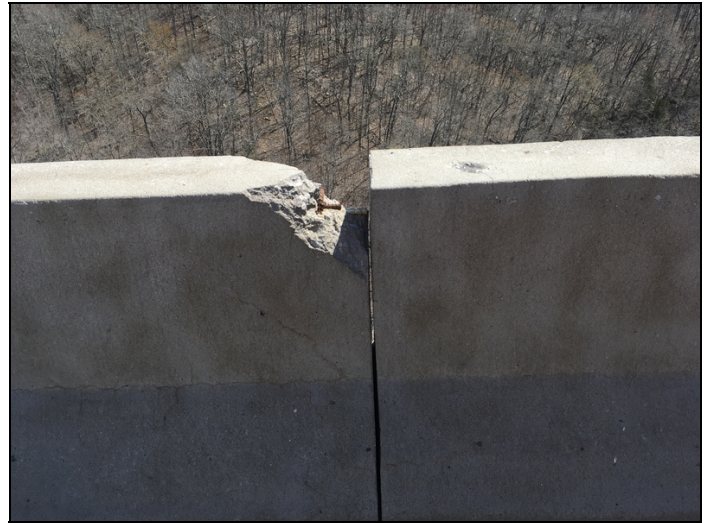
Span 5 Collision damage.
