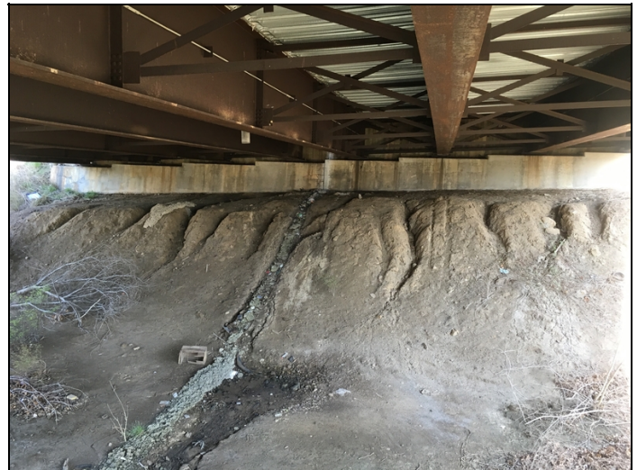
North Abutment embankment erosion.
