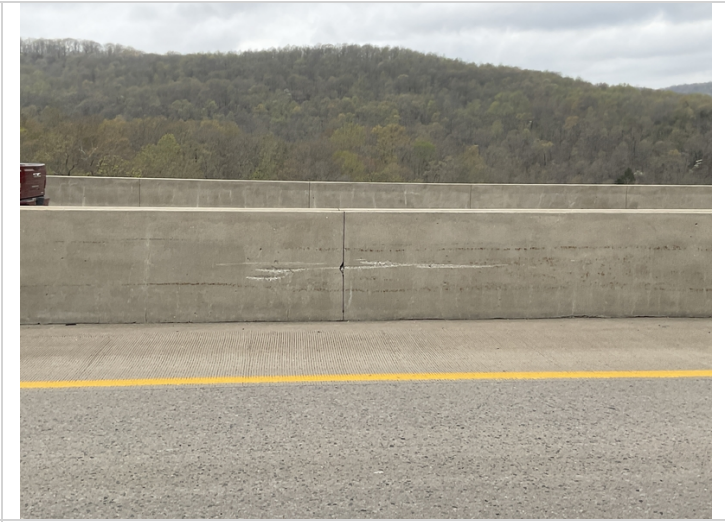
Minor collision damage on the left bridge rail in span 5.
