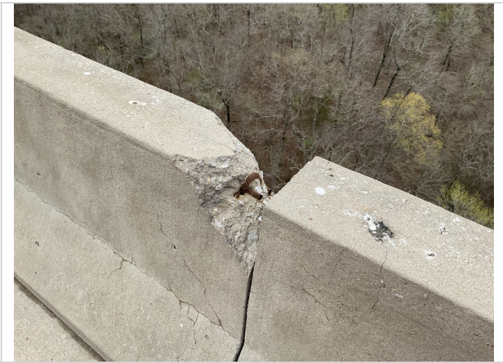
Span 6, right bridge rail, large spall with exposed rebar.
