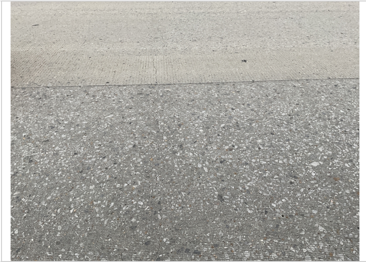
Span 10, large transverse cracks.
