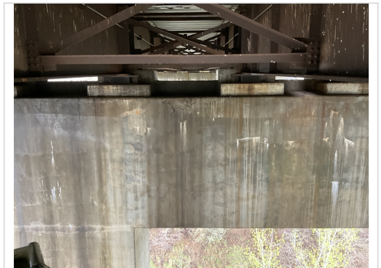
Bent 3 ahead side, large spall, horizontal cracking and efflorescence with build up.
