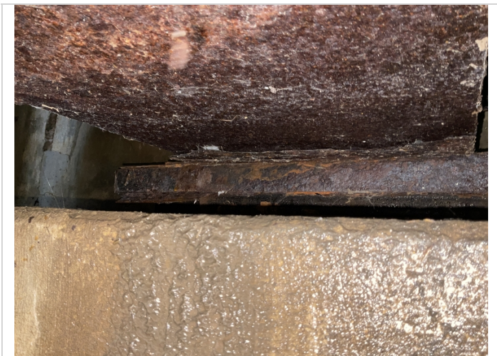
Bent 11 bearing 1, laminating rust
