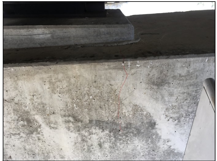
Bent 5 Hairline Cracking in face of cap.
