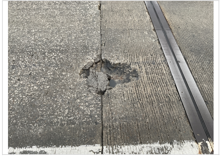
Large spall in the top of the backwall bent 1.
