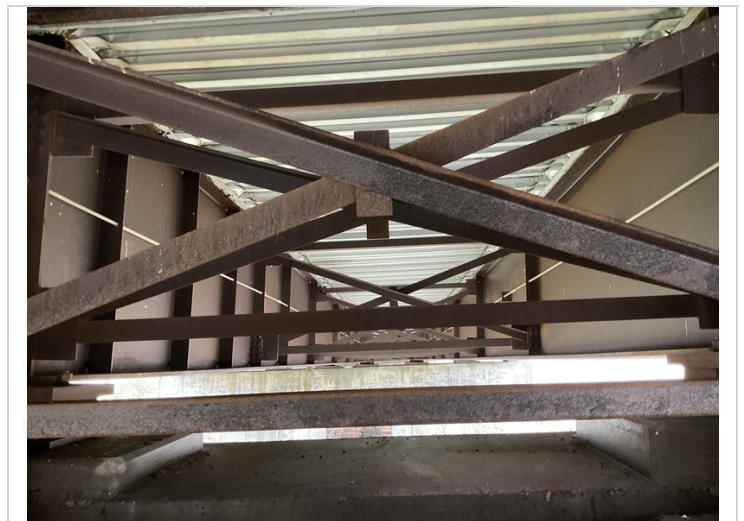
Span 7, bent 8, corrosion on diaphragm.
