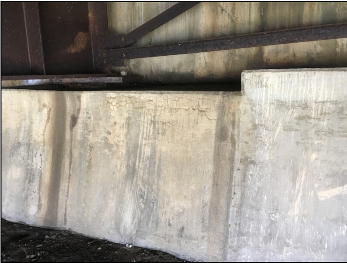
North Abutment map Cracking under Girders 1 and 2.
