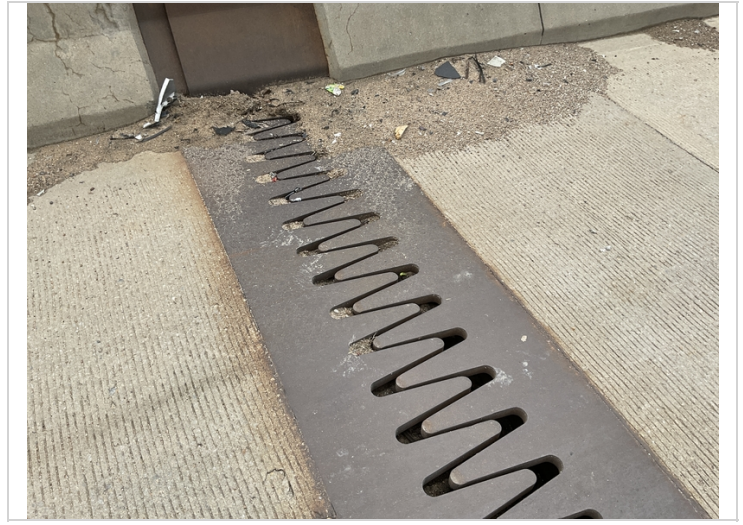
Bent 8, debris impact in assembly joint.
