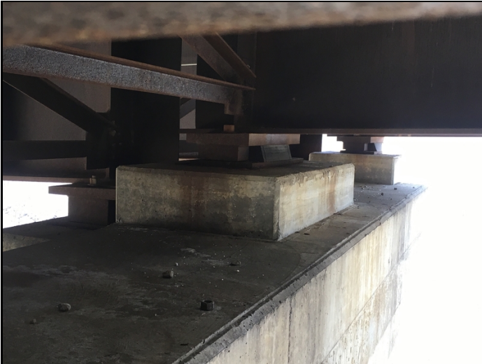
Bent 2 anchor bolt broken Bearing like 1" being fully extended.
