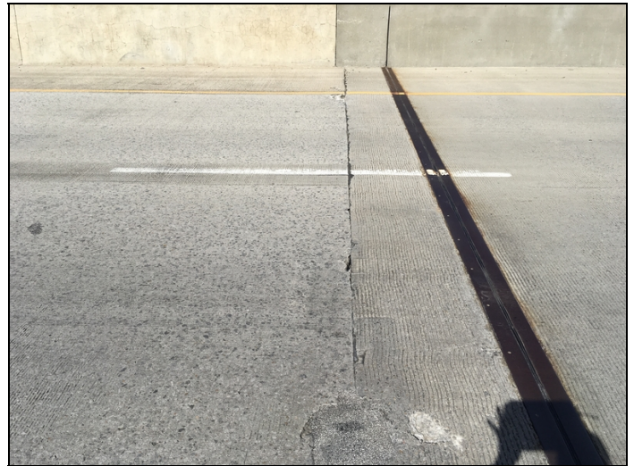
South Abutment Joint sealant has abraded.
