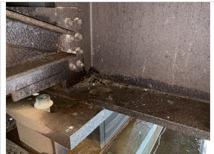
Span 7 girder 2, corrosion on bottom flange.
