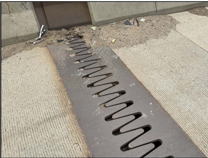
Bent 8, debris impaction in assembly joint.
