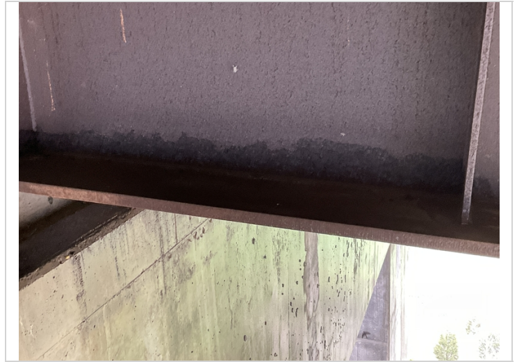
Span 8 girder 1, corrosion in lower web
