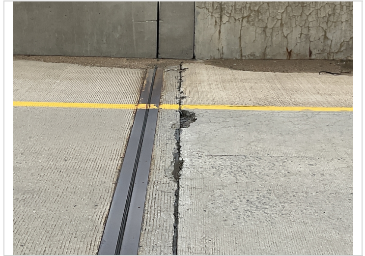
Large spall in northern approach slab.
