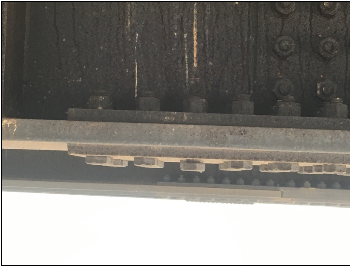
Span 4 Girder 1 first splice plate and loose bolt bottom flange.
