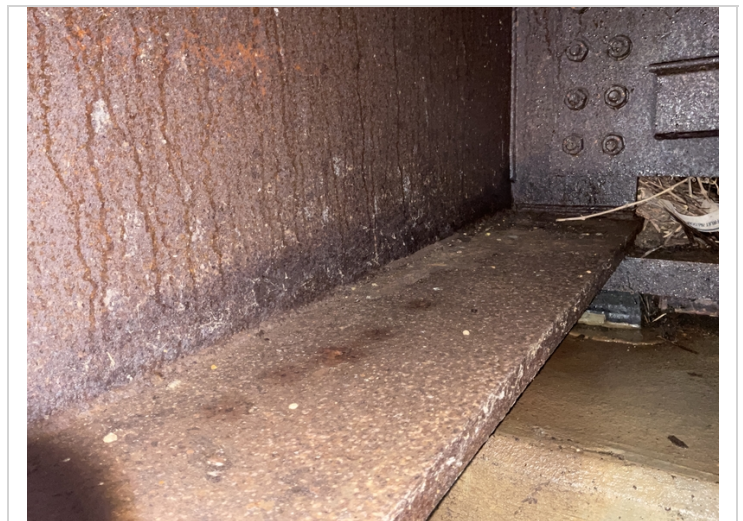
Bent 11 girder 3, protective coating is failing.
