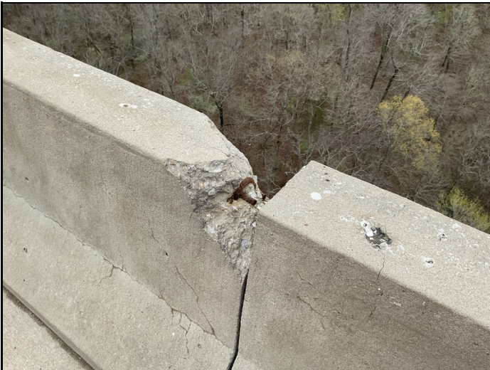
Span 6, right bridge rail, large spall with exposed rebar.
