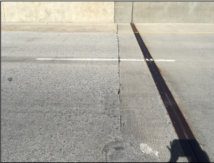
South Abutment Joint sealant has abraded.
