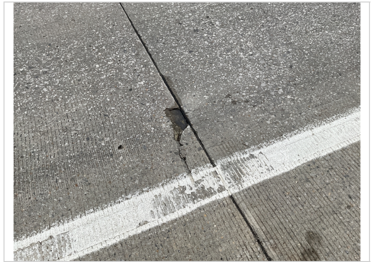
Span 7, deep spall in the right lane
