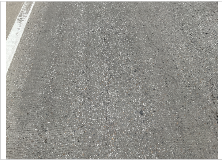
Span 9, longitudinal cracks.
