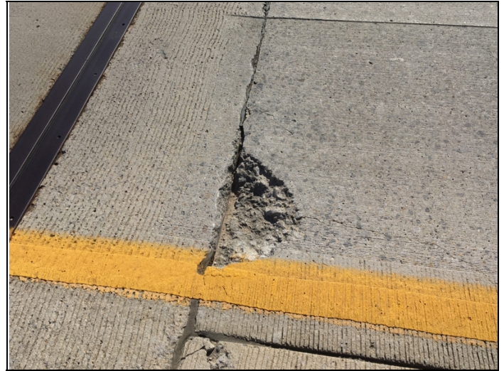
Approach 1: Spalling.
