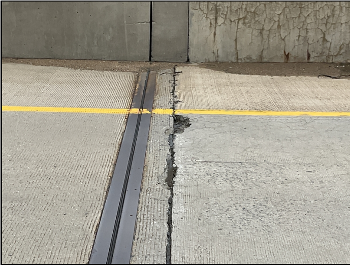
Large spall in northern approach slab.
