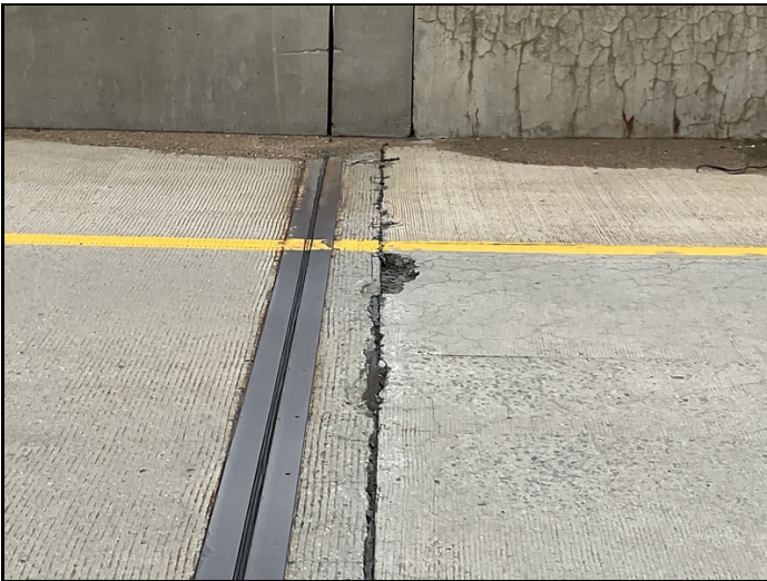
Large spall in northern approach slab.
