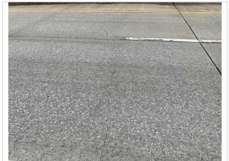
Large transverse cracks in northern approach slab.
