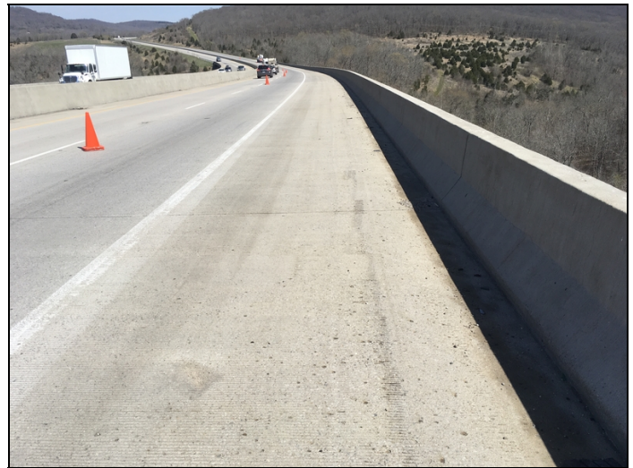
Minor dirt and debris in gutter areas.
