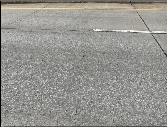
Large transverse cracks in northern approach slab.
