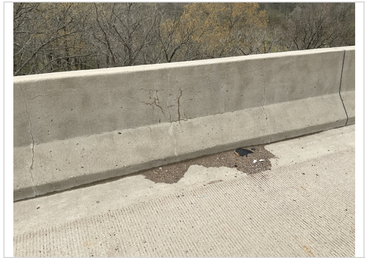
Typical cracks in concrete bridge rail
