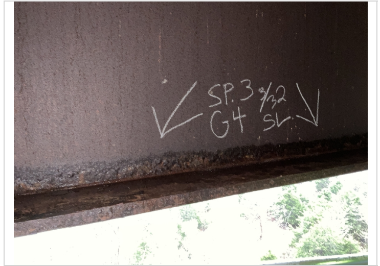
Span 3 girder 4, 3/32ths section loss to bottom flange. 1 3/8 is the thickness without section loss.
