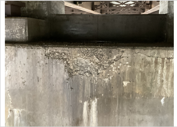
Bent 3, large spall on the ahead side.
