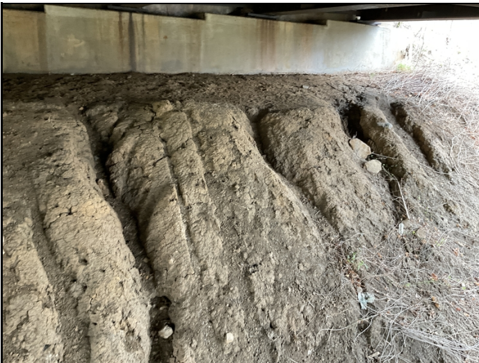
Erosion at bent 11,
