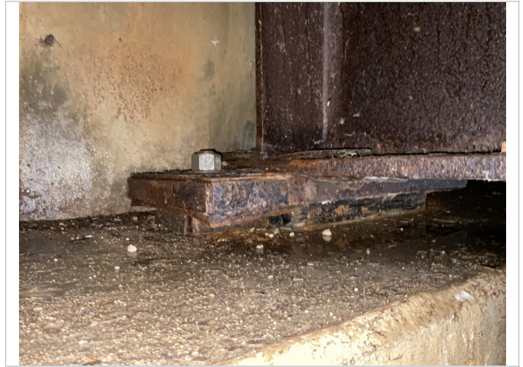
Bent 11 girder 1, laminating rust in girder and bearing.
