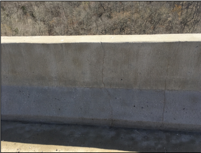
Vertical cracking in parapet wall typical throughout.
