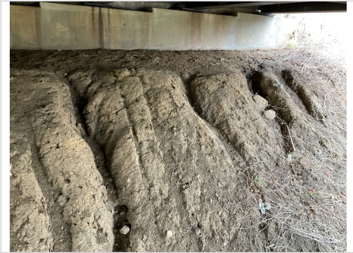
Erosion at bent 11,
