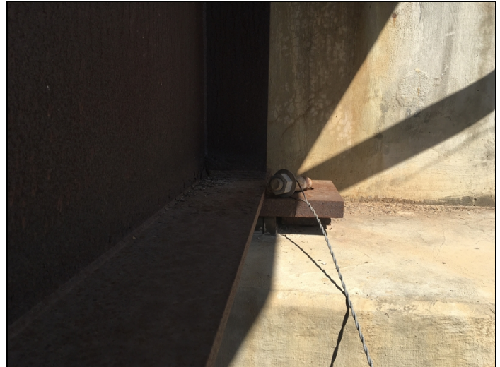
North Abutment Girder 4 broken anchor bolt.
