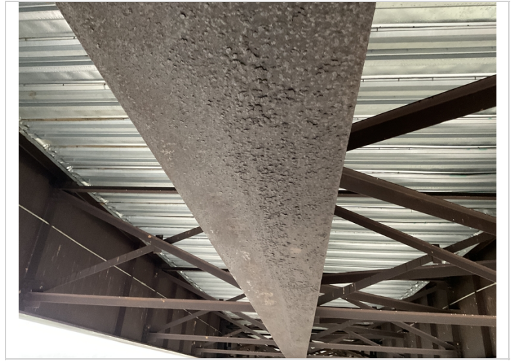
Span 3 girder 3, protective coating is failing.
