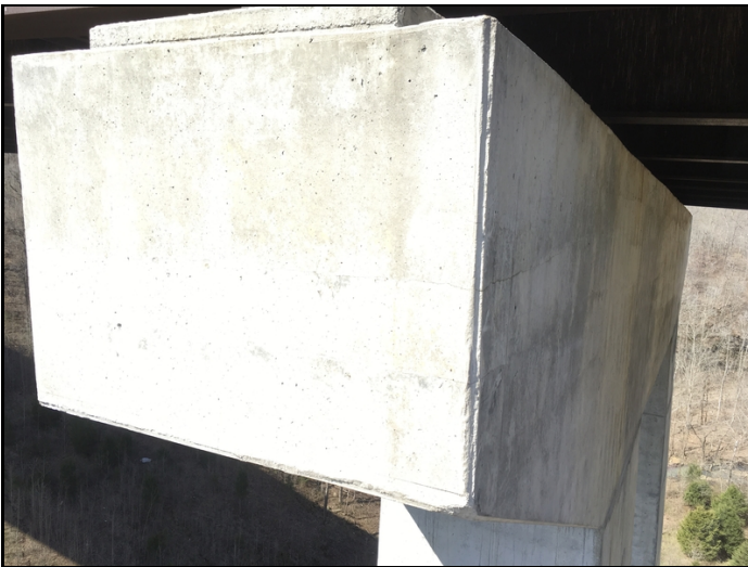
Bent 5 upstream end of cap map Cracking.
