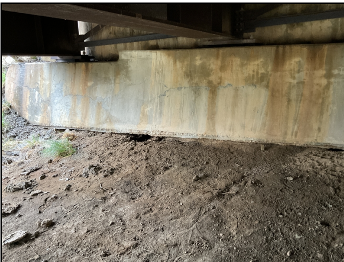
Bent 11, cracks and embankment settlement.
