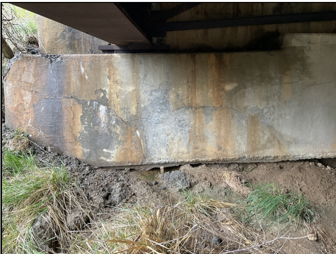
Bent 11 , large horizontal cracks in the face of the bridge seat.
