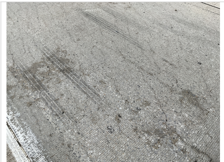
North side approach slab, cracking.
