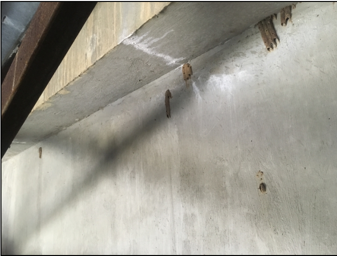
South Abutment Cracking in back wall with efflorescence.
