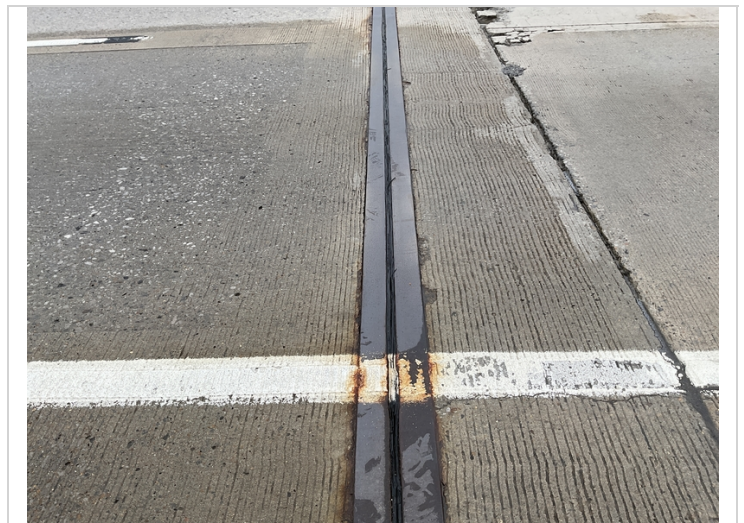
Bent 1 joint, damage.
