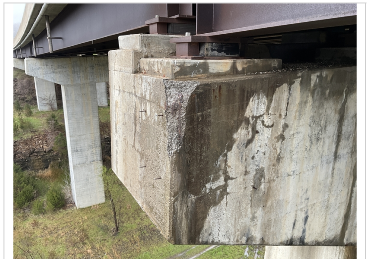
Bent 8 left side, large spall with exposed rebar with section loss.
