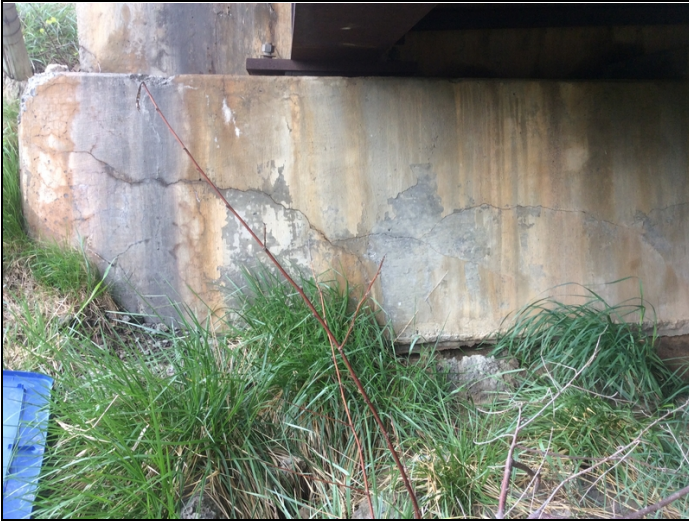
Bent 11 left side: horizontal and map cracking.
