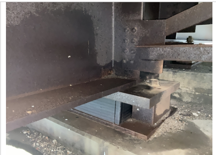
Span 7, bent 8 girder 3, protective coating has failed and there is minor section loss to the lower web.
