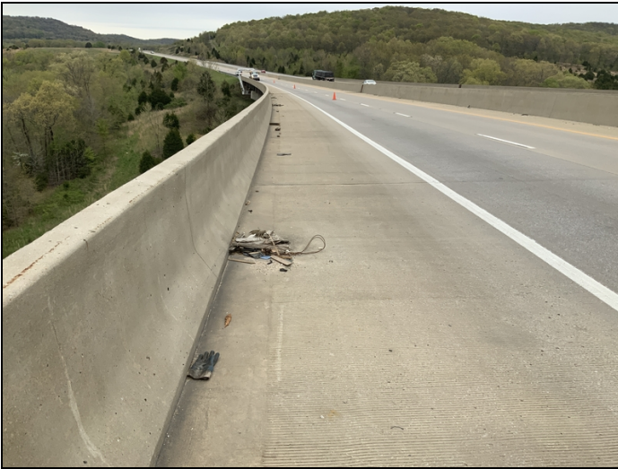
Deck drains full of debris typical throughout structure.
