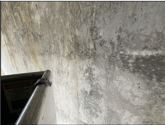
Bent 6 backside face of cap, long horizontal crack from left edge to middle of bay 3.
