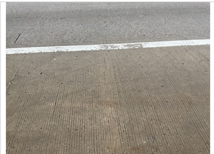
Span 4, large transverse crack.
