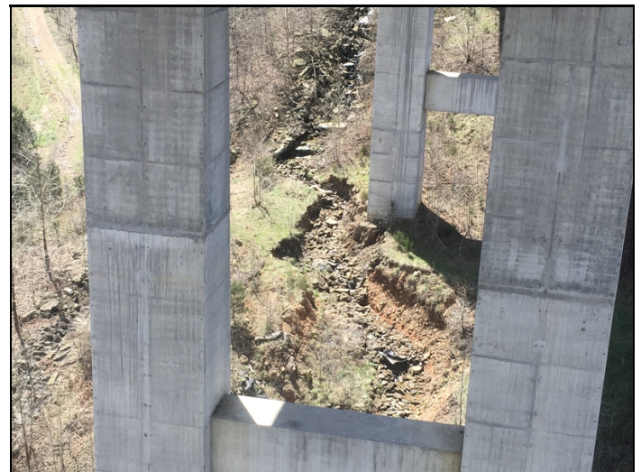
Bent 2 - 4 embankment erosion
