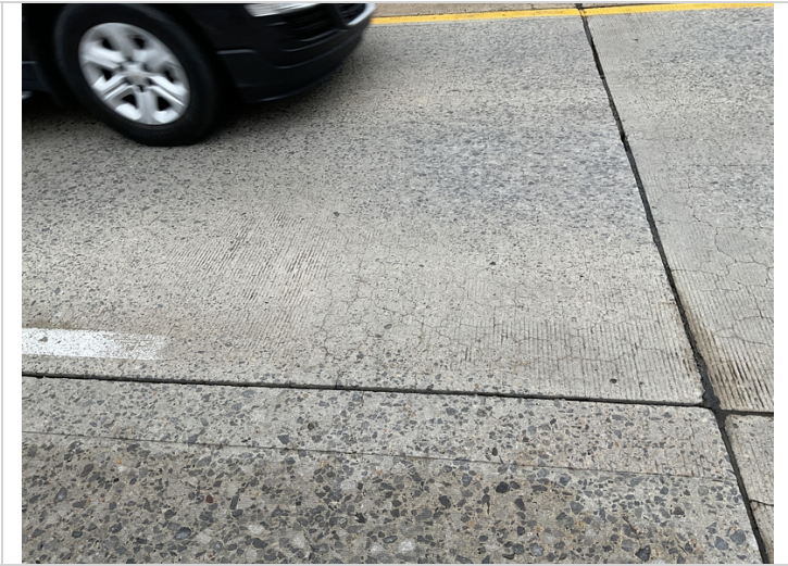
Map cracking southern approach slab.
