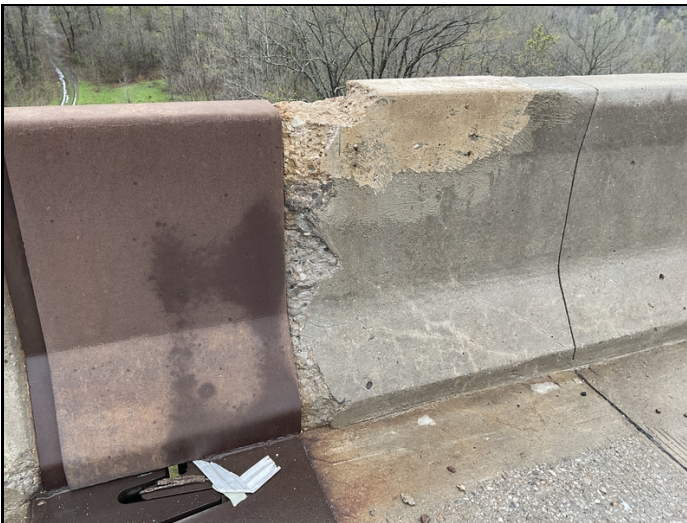
Bent 3, large spall in bridge rail.
