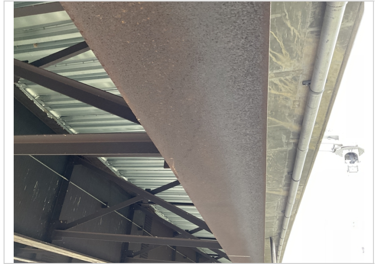
Span 6, typical condition of the protective coating on the bottom of the bottom flange.
