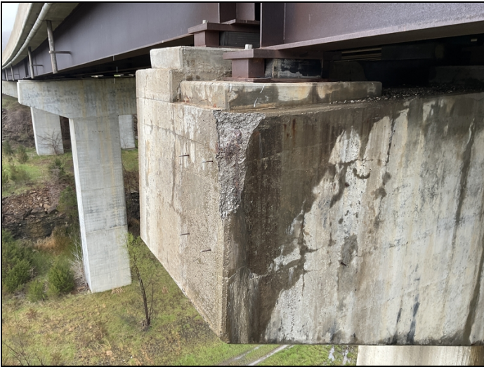
Bent 8 left side, large spall with exposed rebar with section loss.
