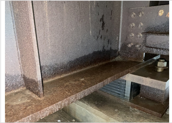
Bent 8 girder 3, corrosion.
