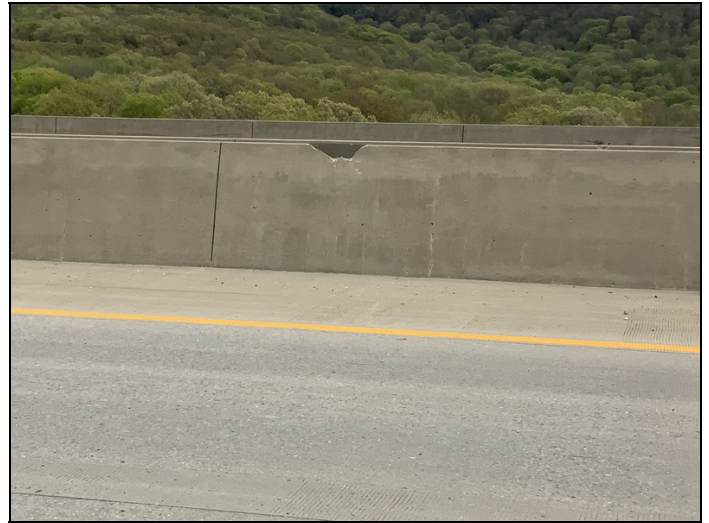
Span 6 center barrier wall collision damage.
