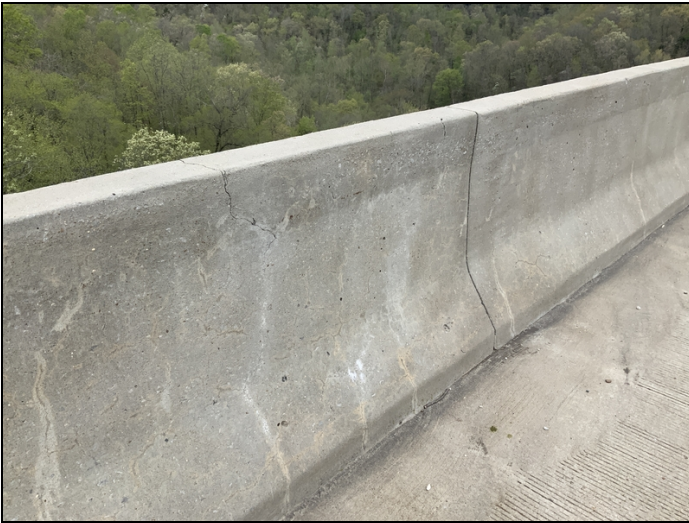
Typical cracking throughout barrier walls.
