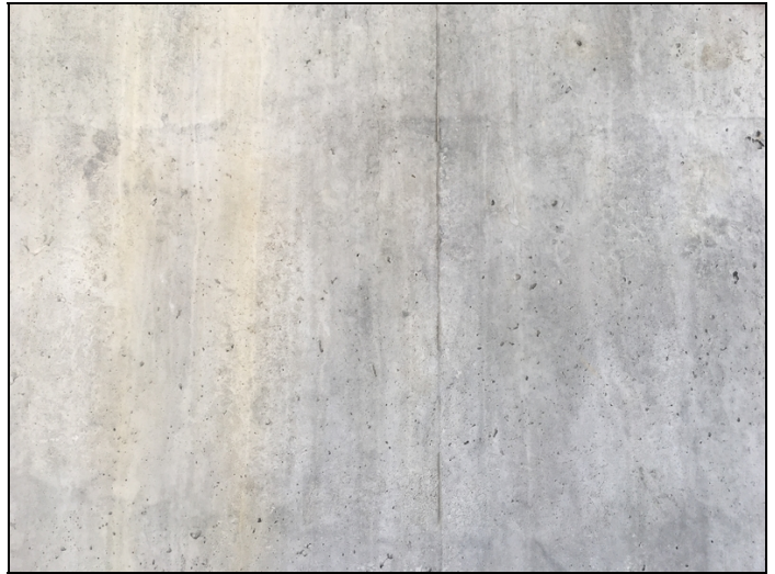
Bent 3 Hairline Cracking in face of cap.
