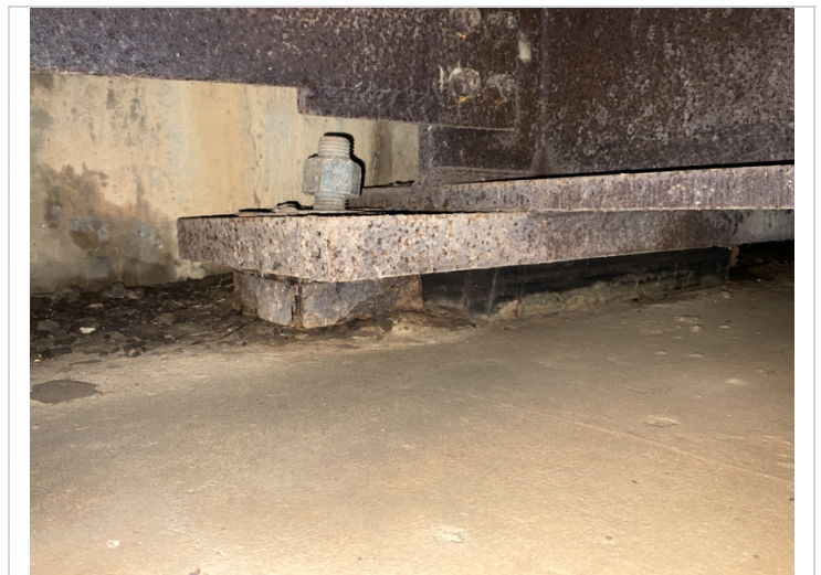
Bent 11 bearing 2, protective coating failing.
