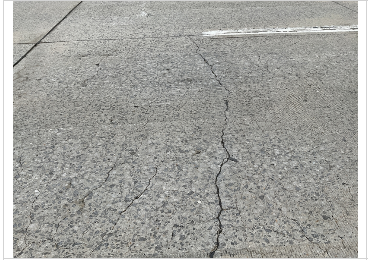
North side approach slab, large cracks.
