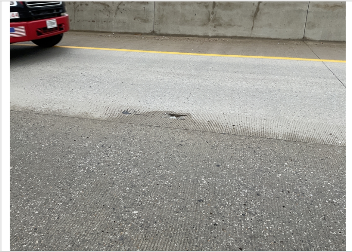
Span 5, missing plowable marker.
