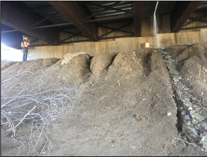
North Abutment embankment erosion.
