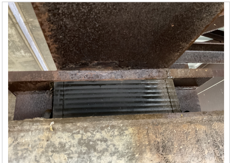
Bent 3 span 3 girder 4, failure of the protective coating.
