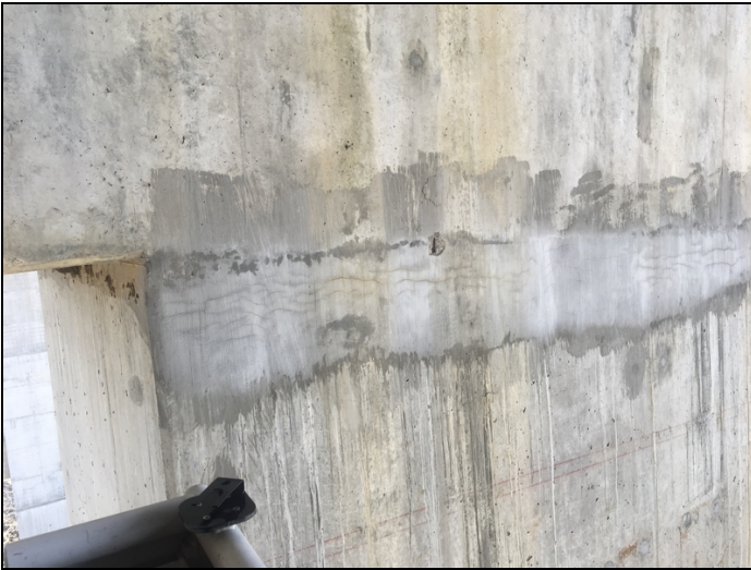
Bent 6 and left pier wall Spall with exposed reinforcing steel.
