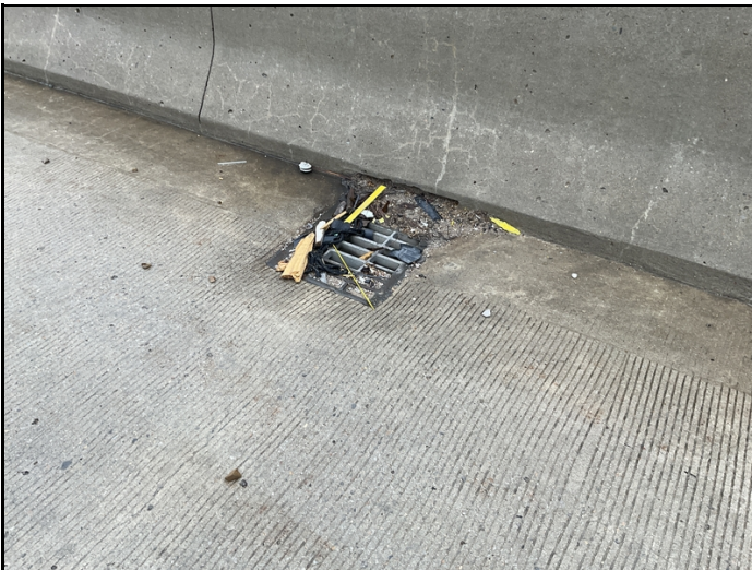
Span 5, typical debris in drains.
