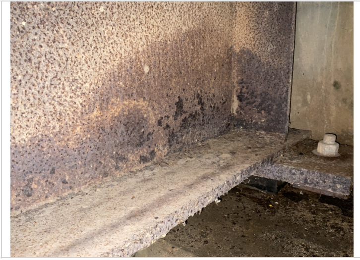
Bent 11 girder 4, the protective coating is failing and there is minor pitting in the lower web.
