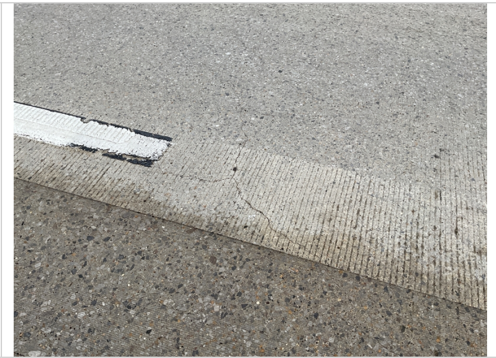
Span 6, large cracks at centerline.
