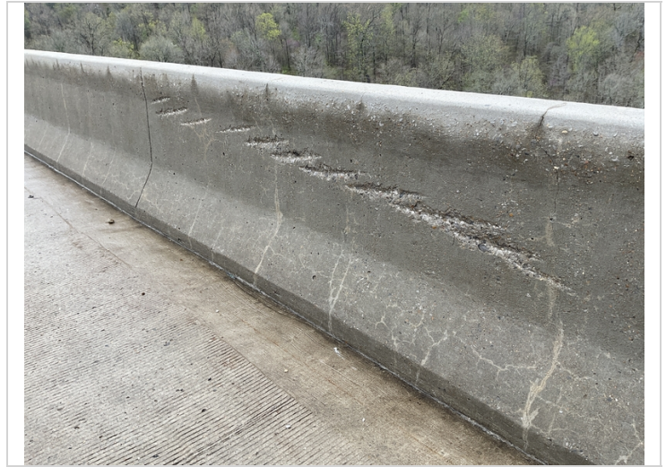
Left bridge rail span 4, 10' damage.
