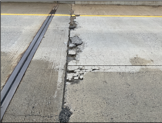
Left lane of southern approach slab, large spalls.
