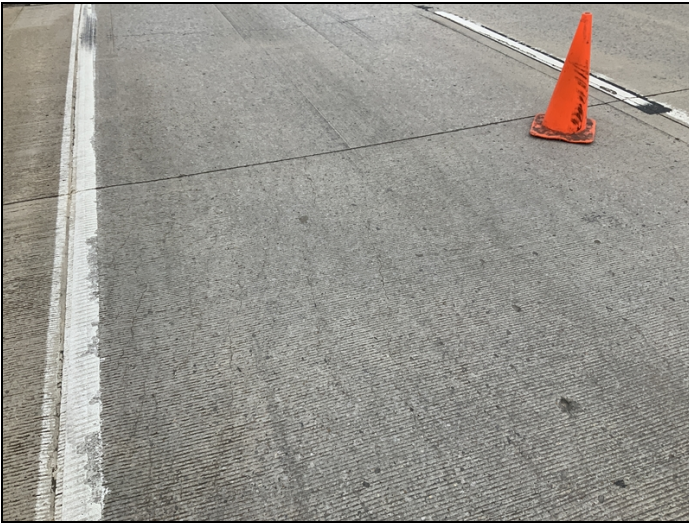
North approach sealable cracking.
