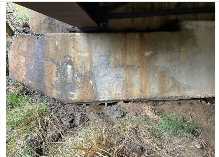
Bent 11 , large horizontal cracks in the face of the bridge seat.
