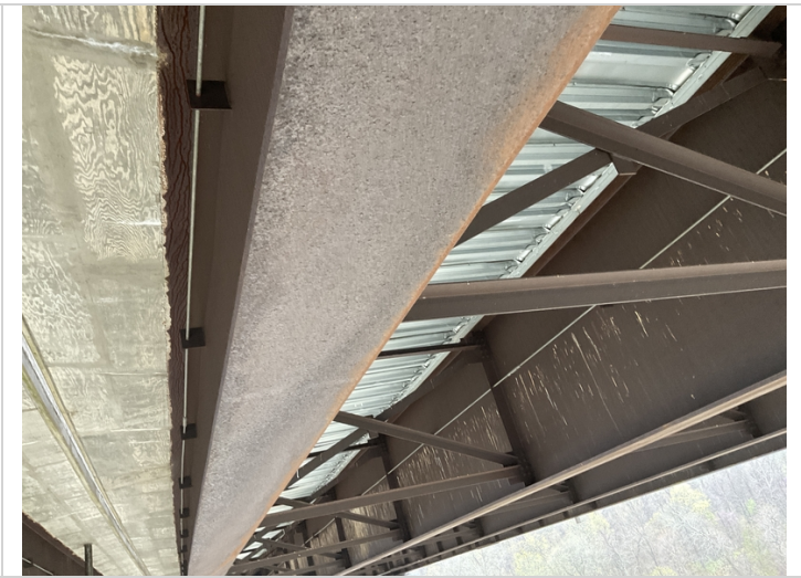
Span 6 girder 4, flaking in the protective coating.
