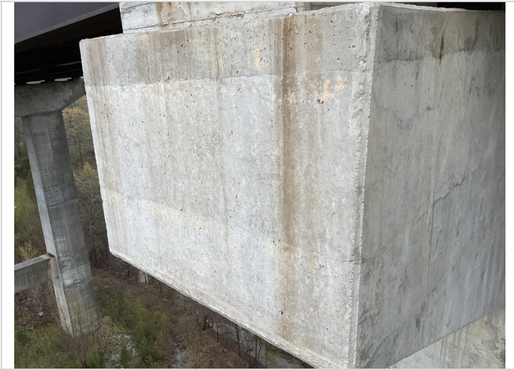
Left end of bent 6, cracking.
