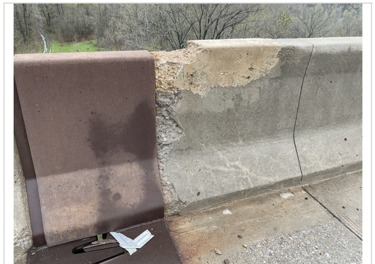
Bent 3, large spall in bridge rail.
