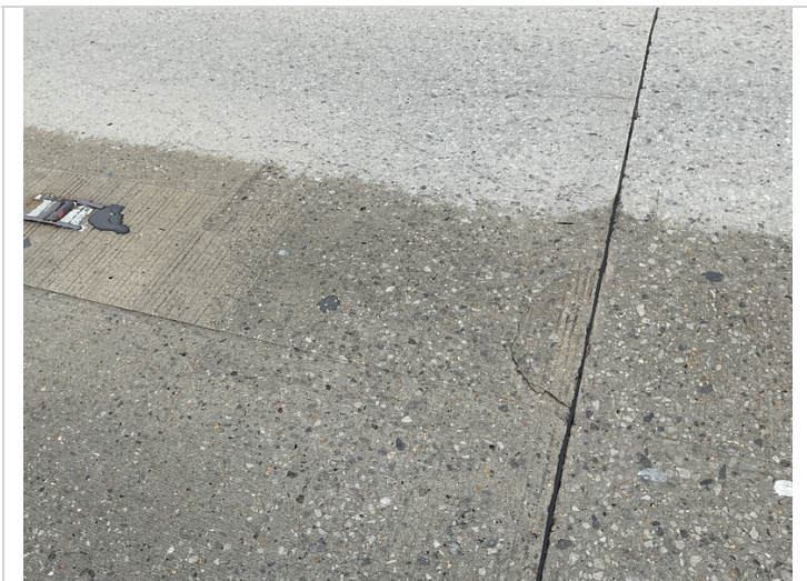
Span 3, delam at centerline.
