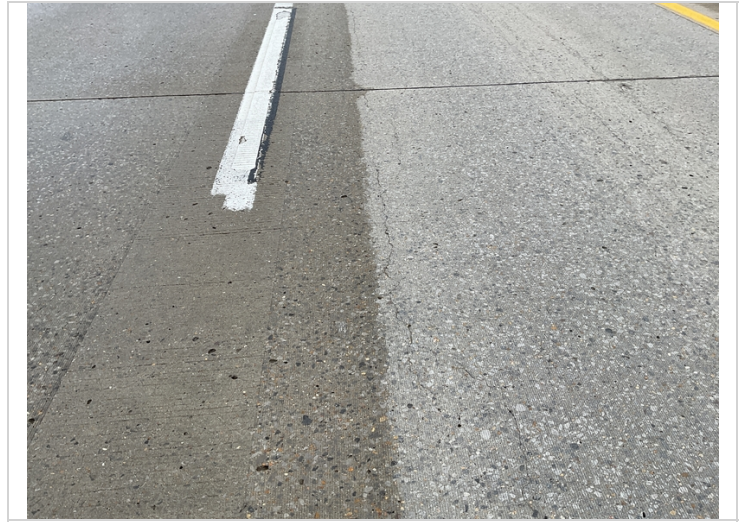
Span 2, large longitudinal crack.
