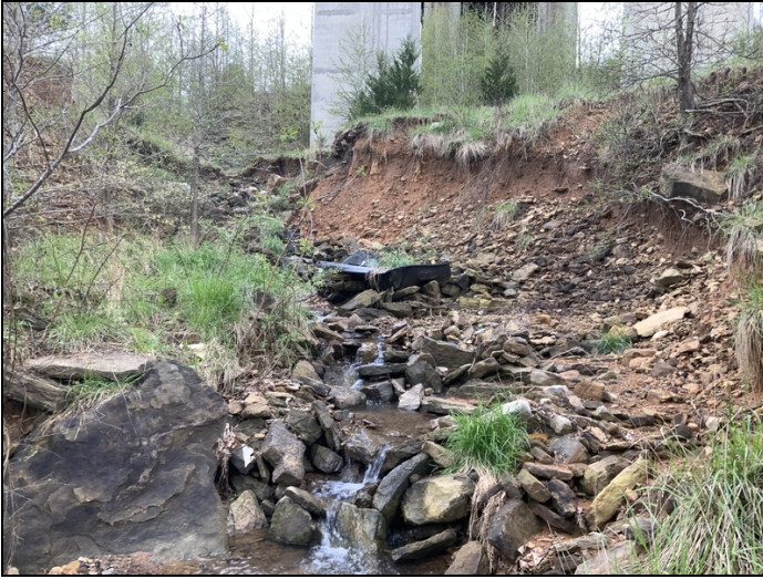
Bent 4 erosion.
