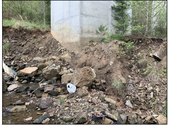
Bent 4 column 2 erosion .
