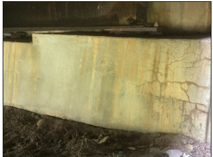
Bent 11 right side (abutment): map cracking and horizontal crack
