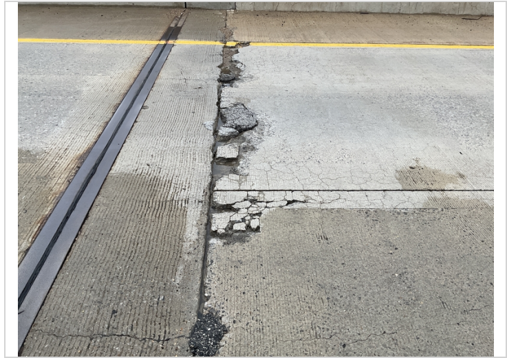
Left lane of southern approach slab, large spalls.
