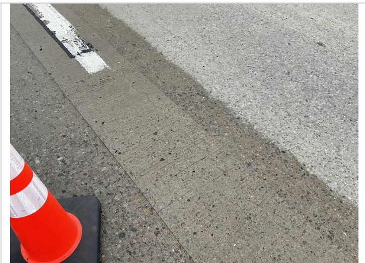
Span 1, cracking in the deck
