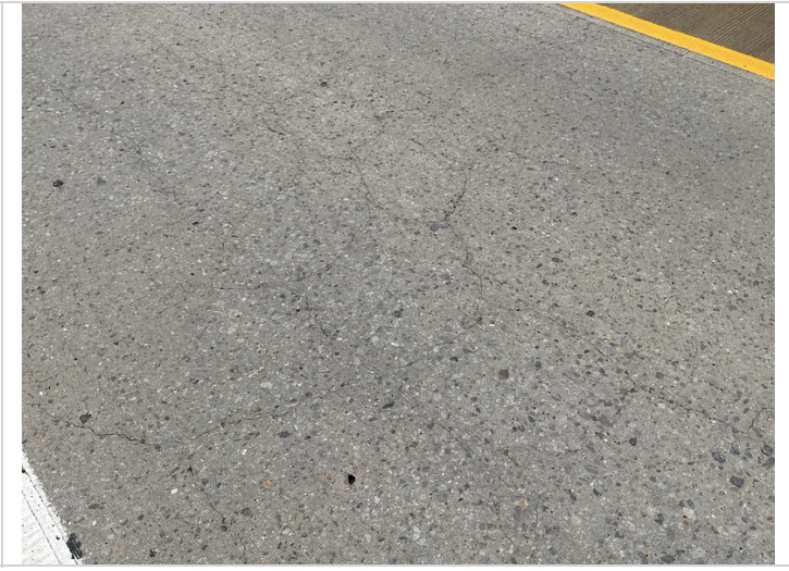
Span 6, large cracks.
