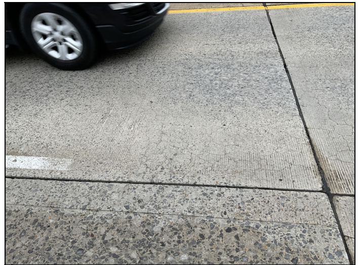
Map cracking southern approach slab.
