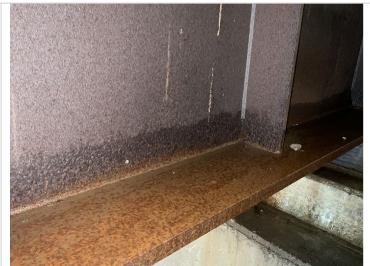
Span 3 girder 3 at bent 3, protective coating failing.
