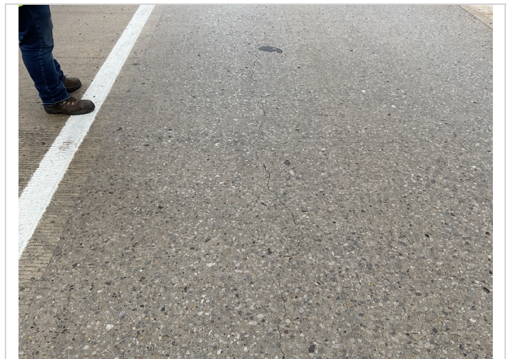
Span 8, large longitudinal crack.
