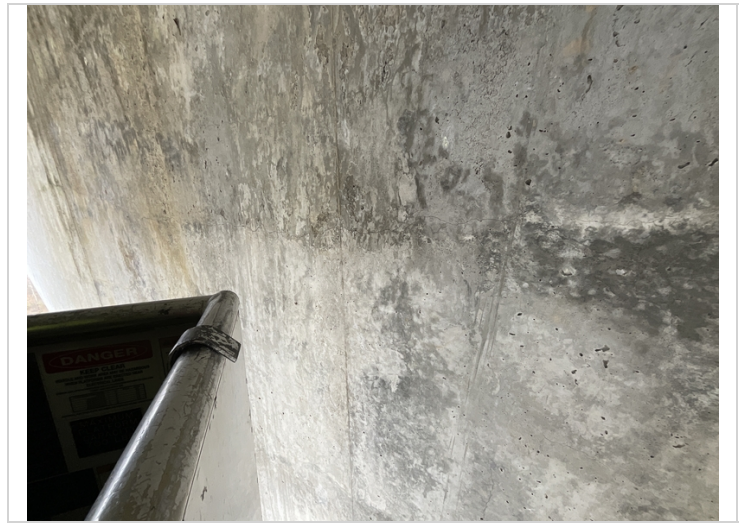
Bent 6 backside face of cap, long horizontal crack from left edge to middle of bay 3.
