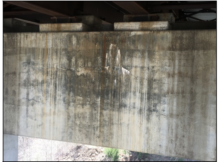
Bent 2 and map Cracking with efflorescence in face of cap.
