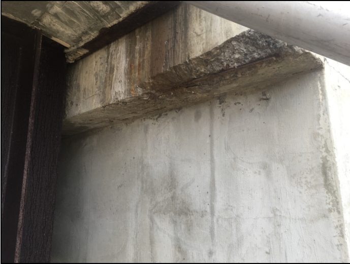
South Abutment left spall with exposed reinforcing steel.
