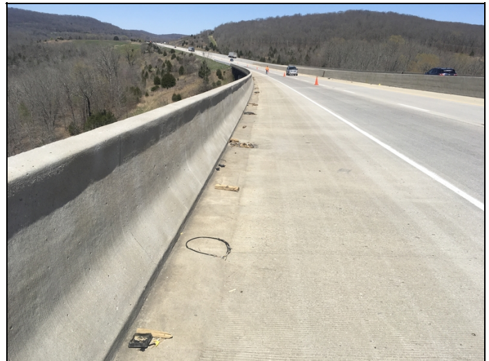
Dirt an debris in gutter.
