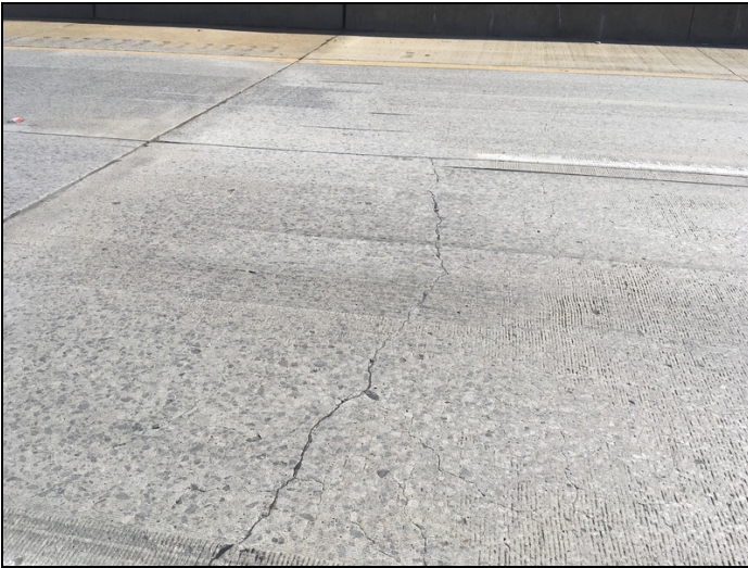
North approach slab sealed cracks.
