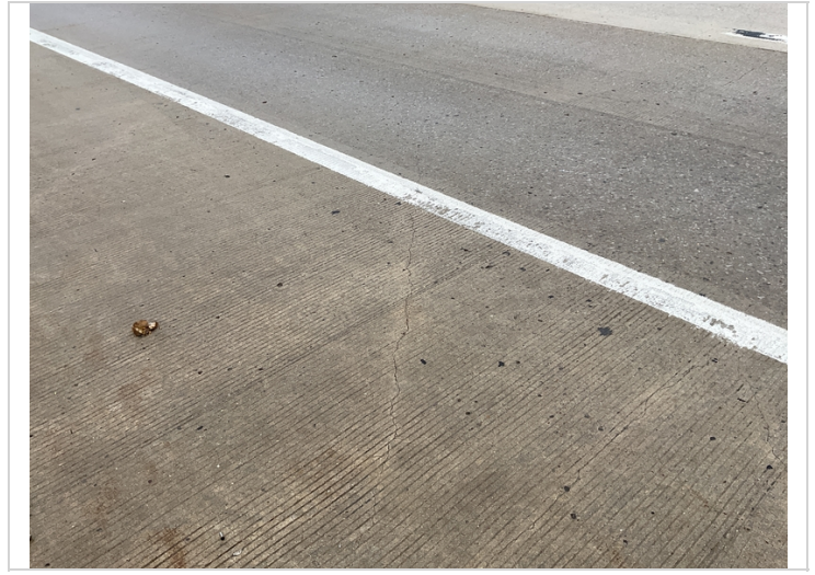
Span 6, large diagonal crack.
