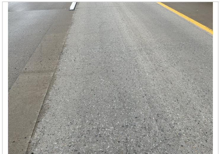
Span 3, large longitudinal crack
