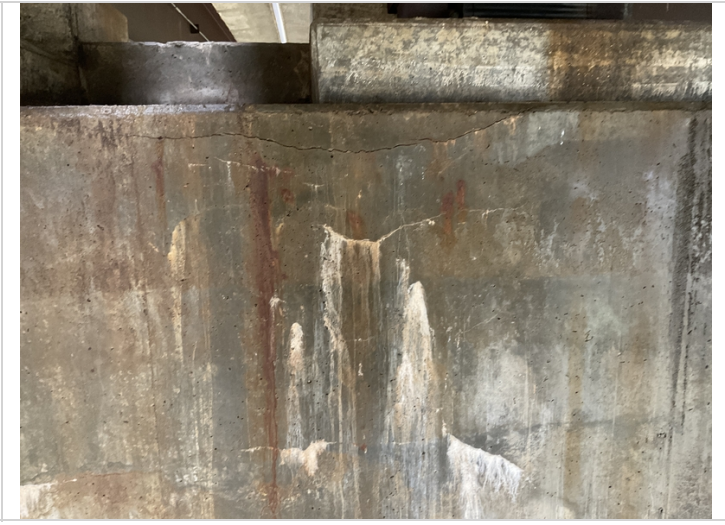
Bent 3 ahead side near girder 4, large horizontal cracks, rust staining and efflorescence.
