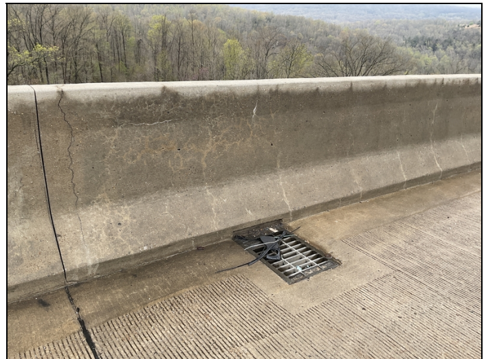
Typical concrete bridge rail.
