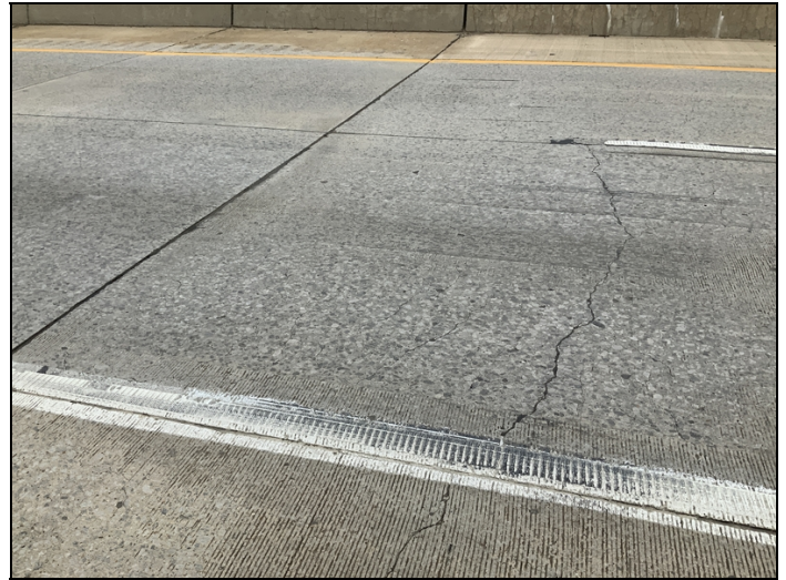
North approach right lane approximately 1" settlement with 20' CS-3 cracking.
