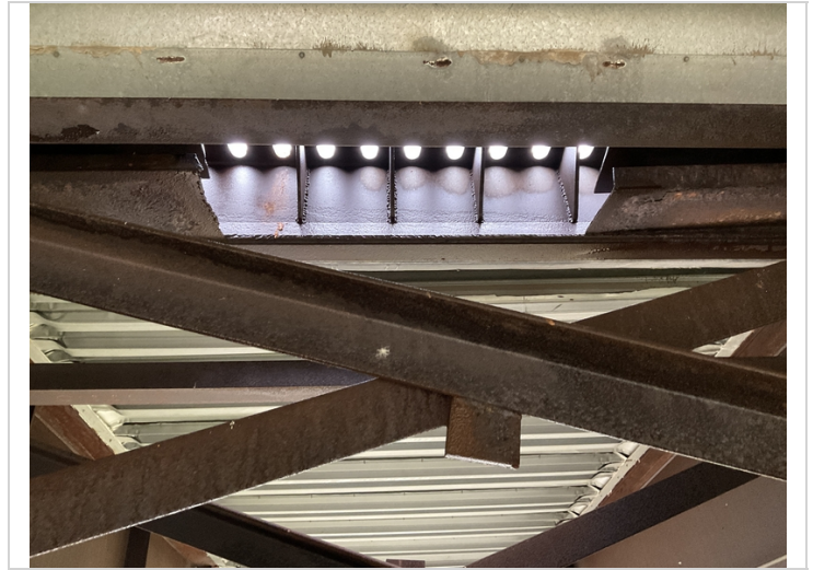
Bent 8 bay 3, 4' of the trough for the assembly joint has been removed by maintenance forces to reinforce the finger joint. Common.
