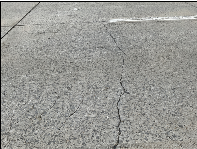
North side approach slab, large cracks.
