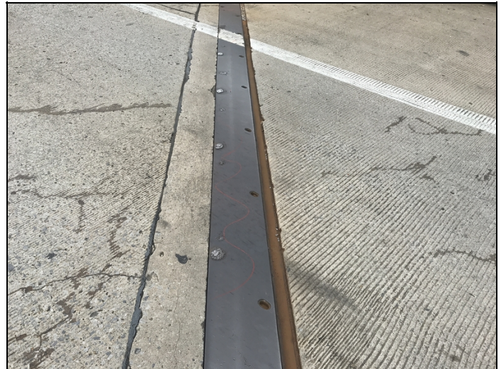
Abutment # 2 Sliding Plate Assembly is noisy in the right lane when impacted by traffic. Sounding indicates that approximately 15' of the assembly in the right lane is not securely anchored.
