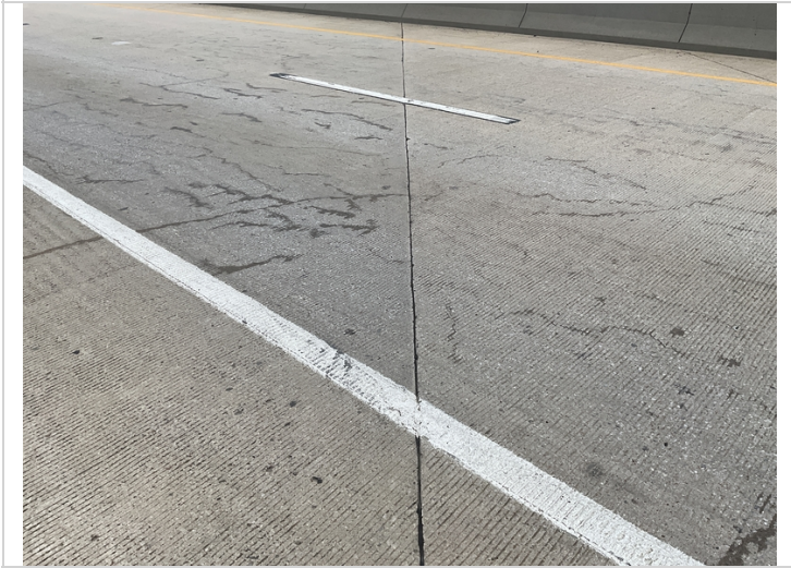
Failing saw joint sealant.
