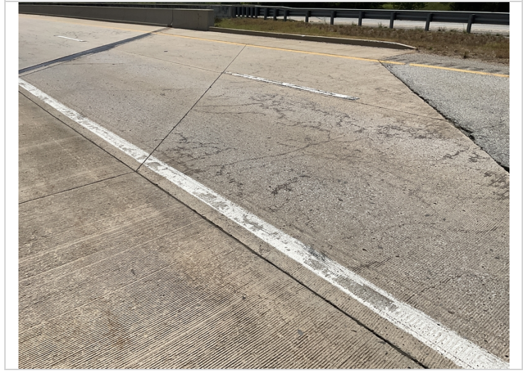
North approach slab cracking.
