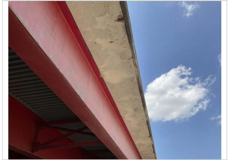
Span #3 Rt concrete delamination and spalling with exposed reinforcing steel.
