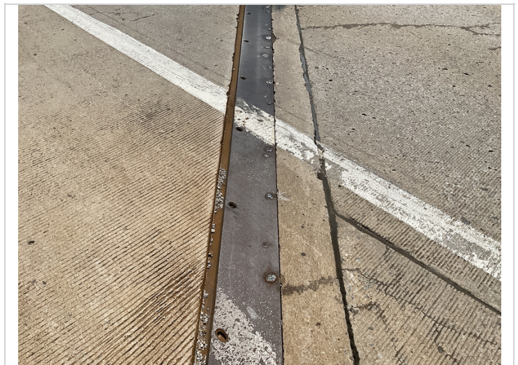
Abutment #2 new anchorage welds.
