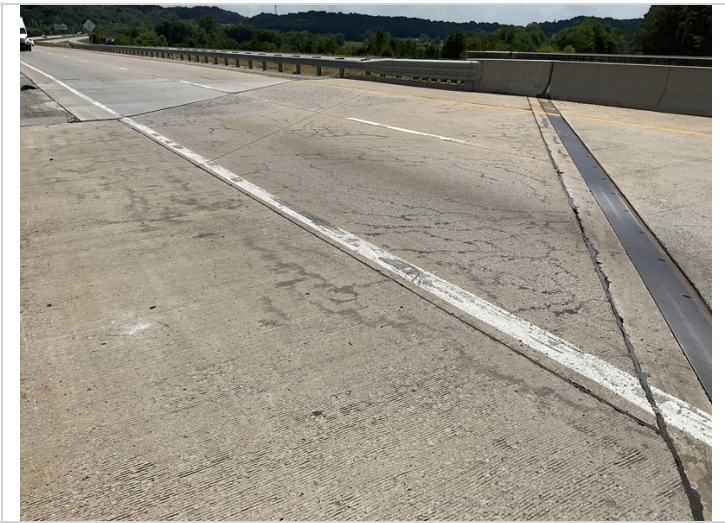
South approach slab cracking.
