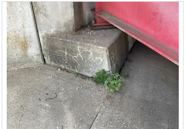
Abutment #1 Rt map cracking.
