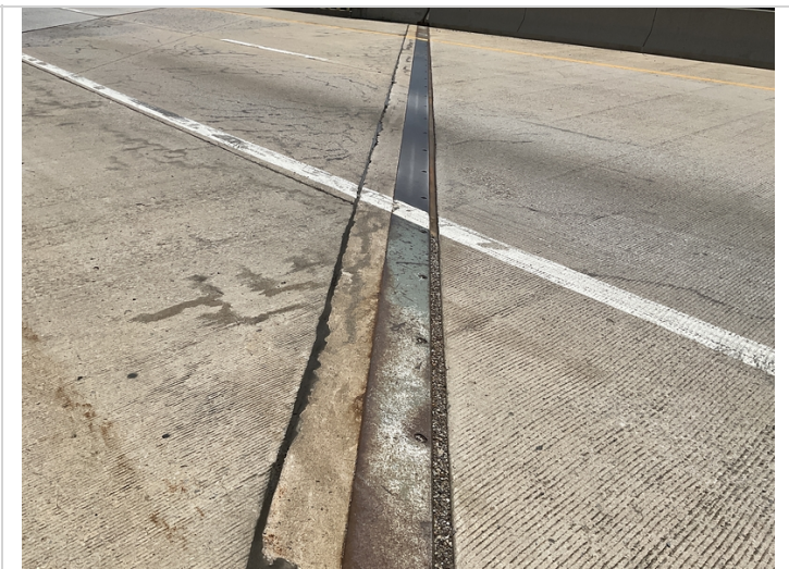
Abutment #1 sliding plate.
