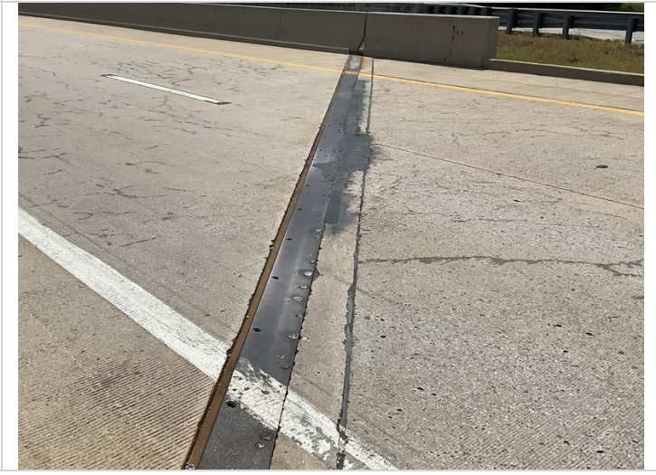
Abutment #2 top of backwall repair.
