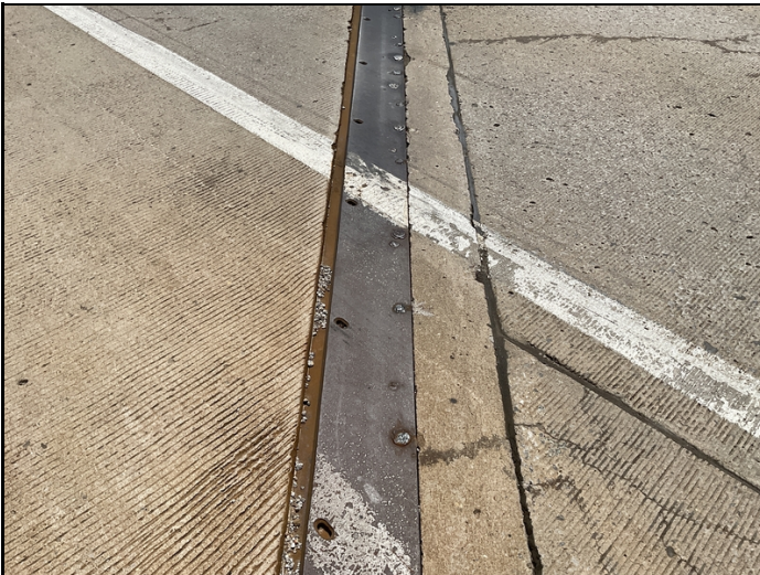
Abutment #2 new anchorage welds.
