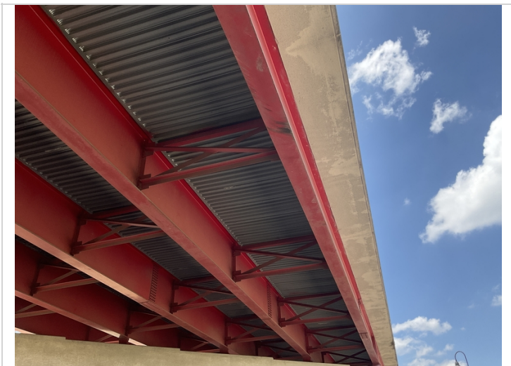
Span #2 beam #7 scrape marks.
