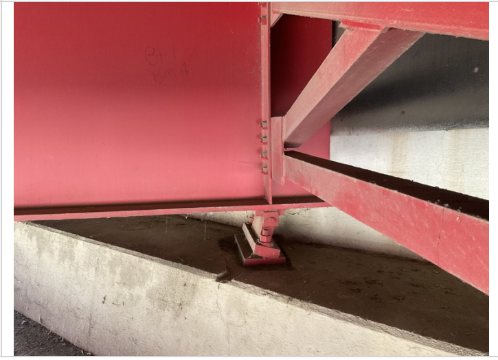
Abutment #1 bearings nearly fully expanded.
