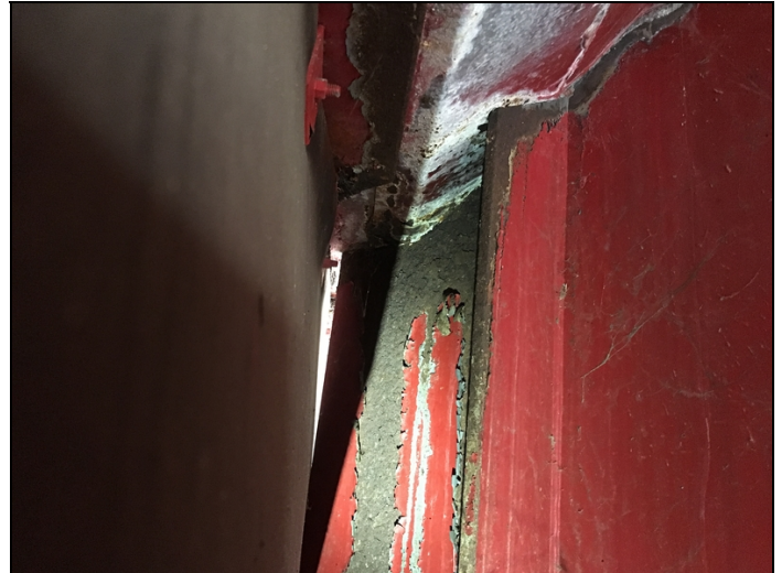
Span 1, Beam # 2 at abutment # 1 has corrosion with flaking rust to the upper portion of web behind bearing area.
