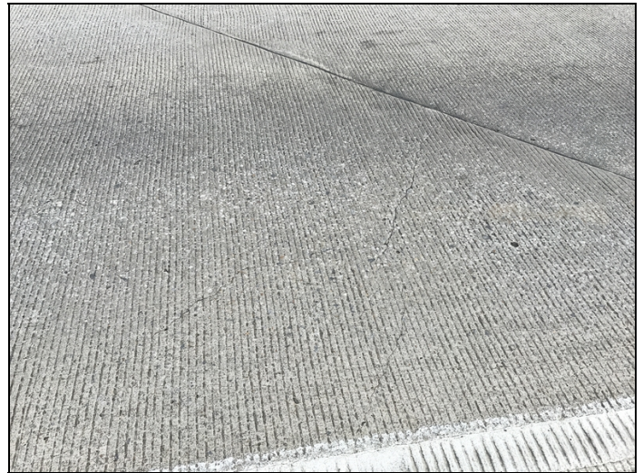
Span 1, left lane-Transverse cracking.
