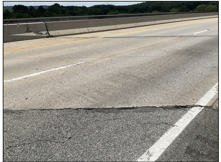
North approach slab cracking.
