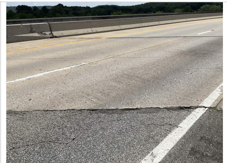
North approach slab cracking.
