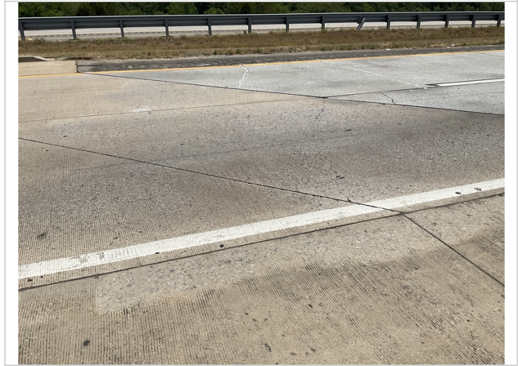
South approach slab wide transverse cracks.
