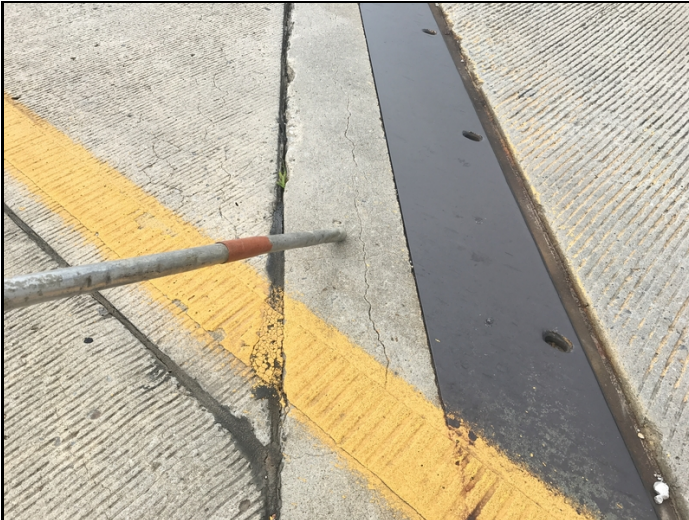
Abutment 1-Longitudinal cracking in top of backwall.
