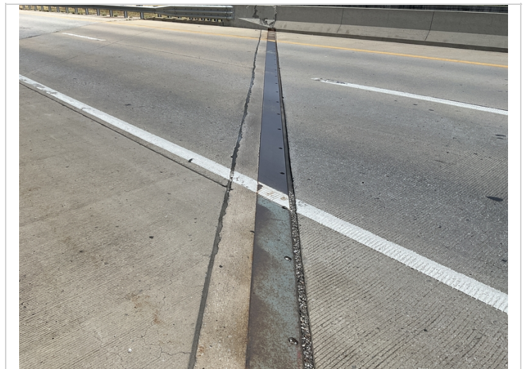
Abutment #2 sliding plate.
