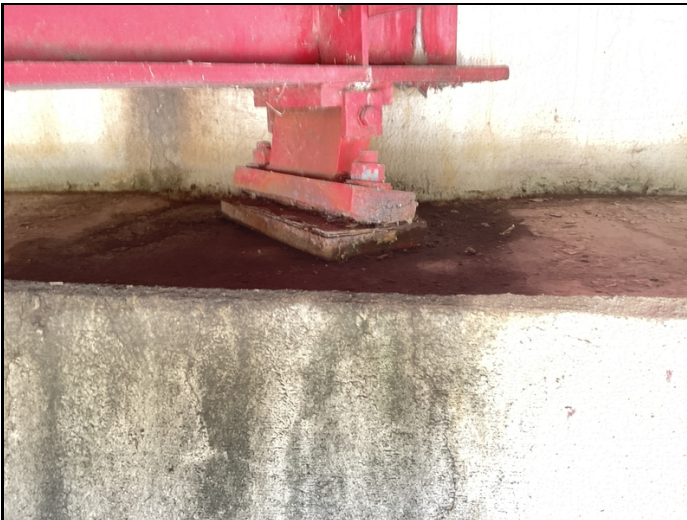
Abutment #1 bearing #2 active corrosion with pack rust.
