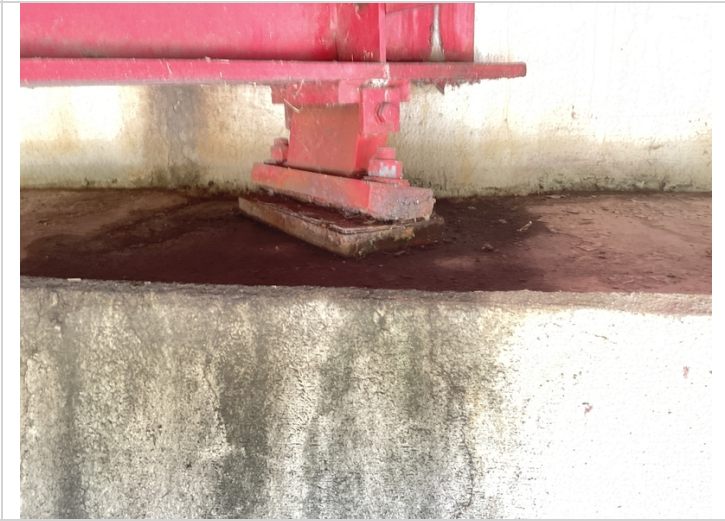
Abutment #1 bearing #2 active corrosion with pack rust.
