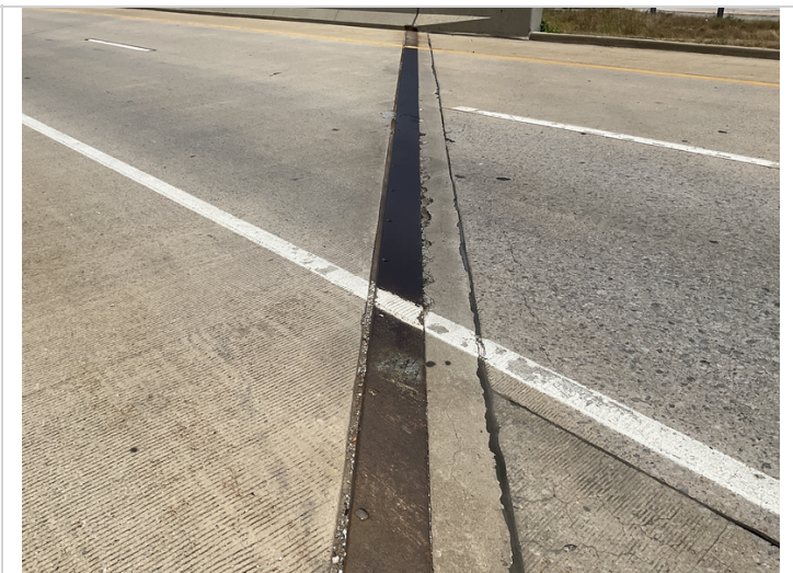
Abutment #1 sliding plate.
