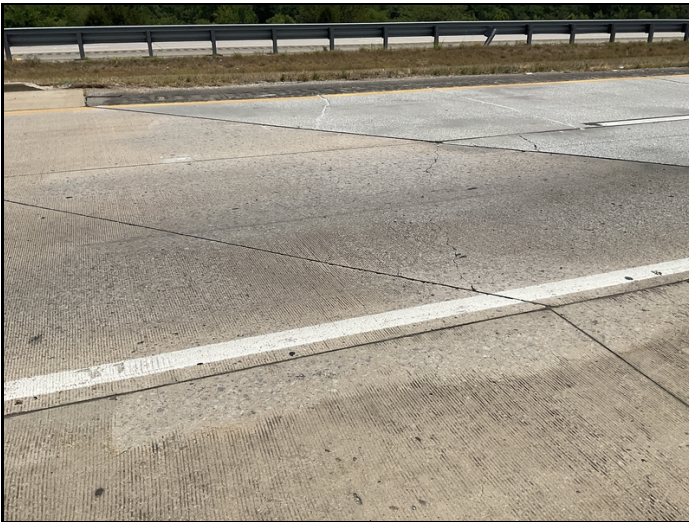
South approach slab wide transverse cracks.
