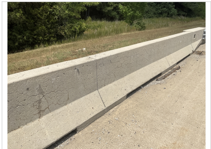
Typical bridge rail map cracking.
