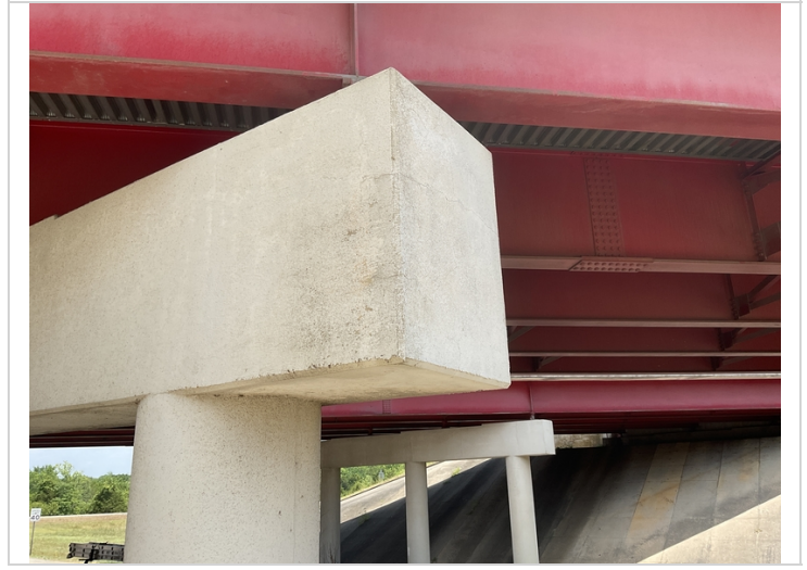
Bent #3 Lt cap map cracking.
