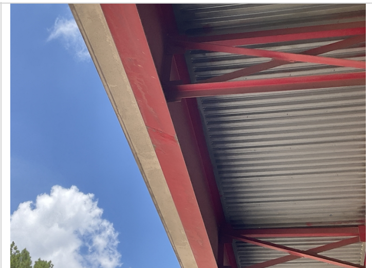
Span #2 beam #1 scrape marks on the undersurface of the bottom flange with no visible cracks.
