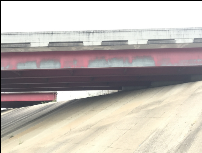
The paint system on the exterior beams is chalking in areas that expose the primer undercoat.
