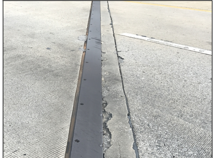
Abutment 1 backwall-Spalling with longitudinal cracking.
