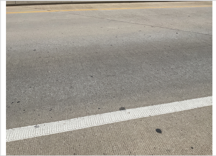
Sealable deck cracking.
