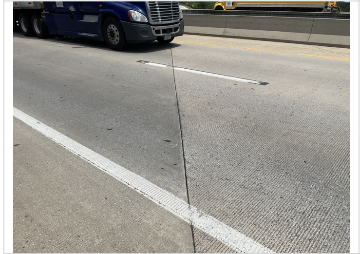
Failed saw joint sealant.
