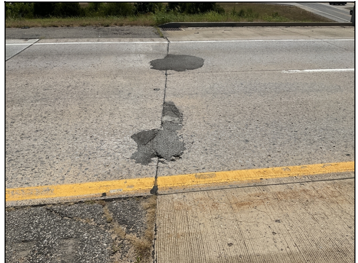
Abutment #2 approach slab spalling with temporary asphalt patches.
