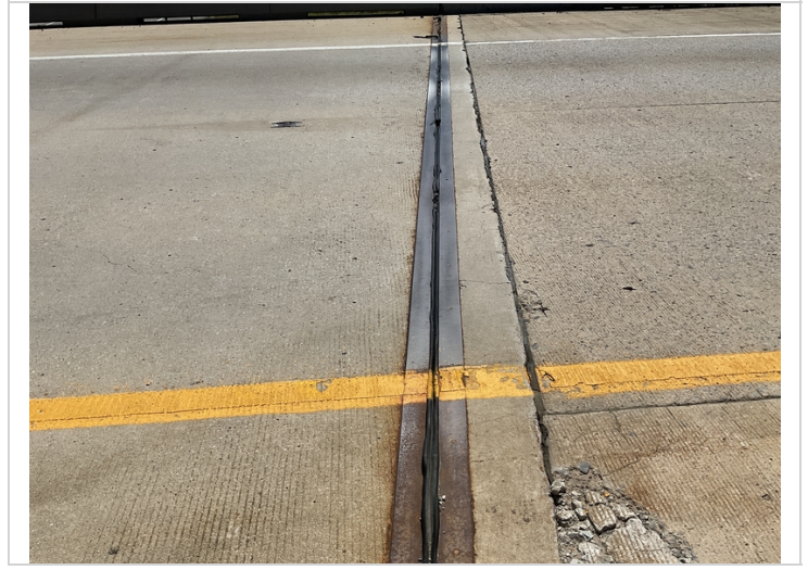
Abutment #1 compression joint seal.
