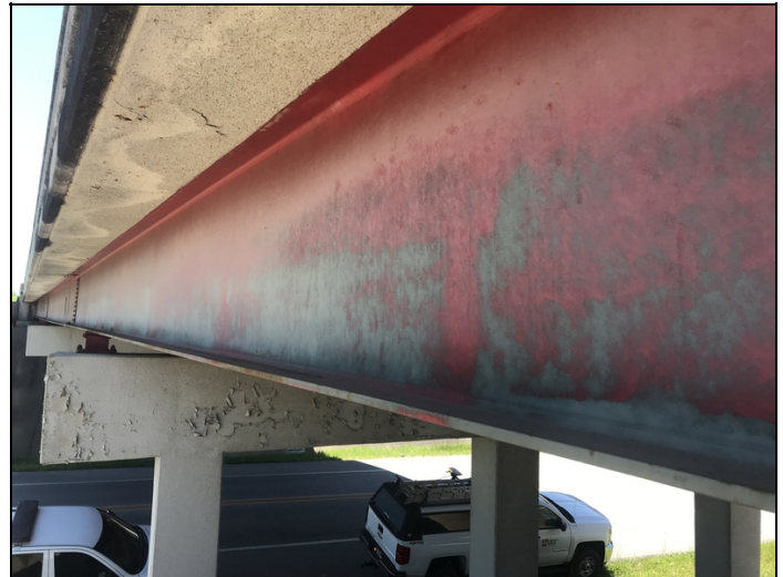
Paint system failing on exterior beams.
