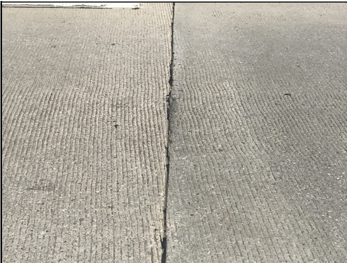
Sawn joint sealant missing.
