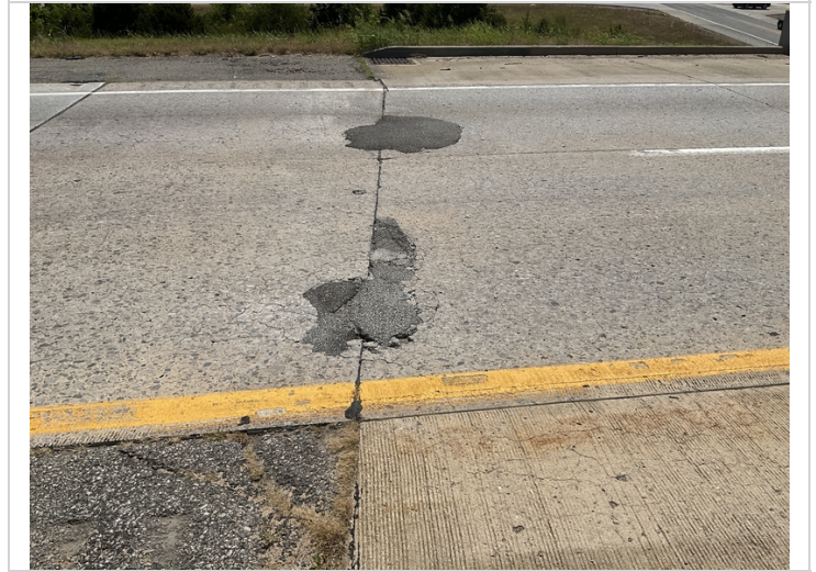
Abutment #2 approach slab spalling with temporary asphalt patches.
