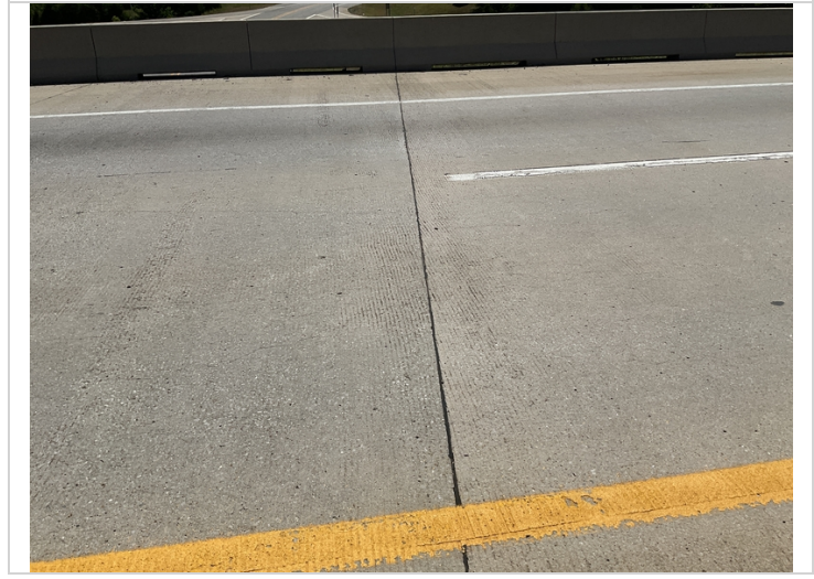
Failing saw joint sealant.
