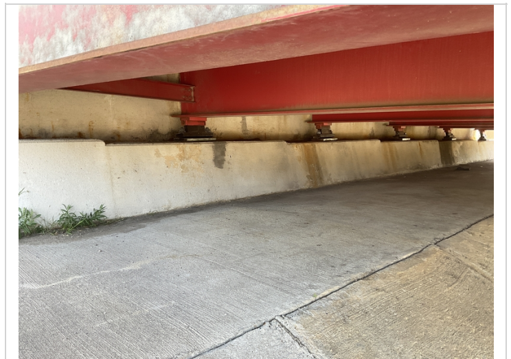
Abutment #2 bearings typical.
