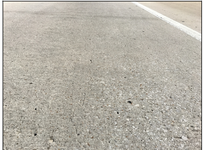
Span 1, right lane-Mapcracking.
