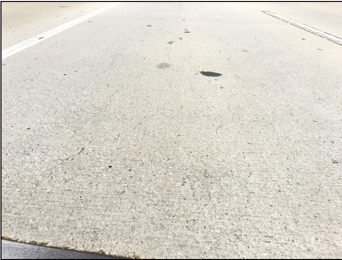
Span 3, right lane-Mapcracking.
