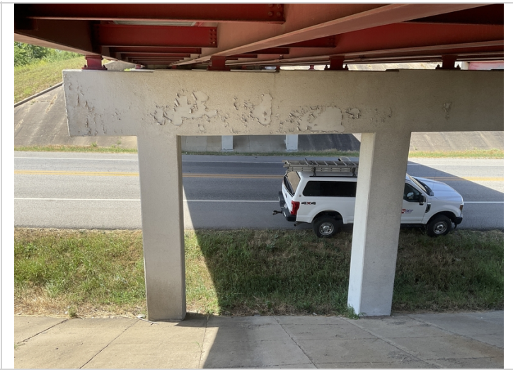
Bent #3 texicoat peeling.
