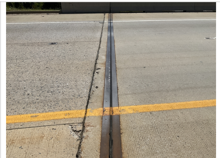
Abutment #2 typical joint seal.
