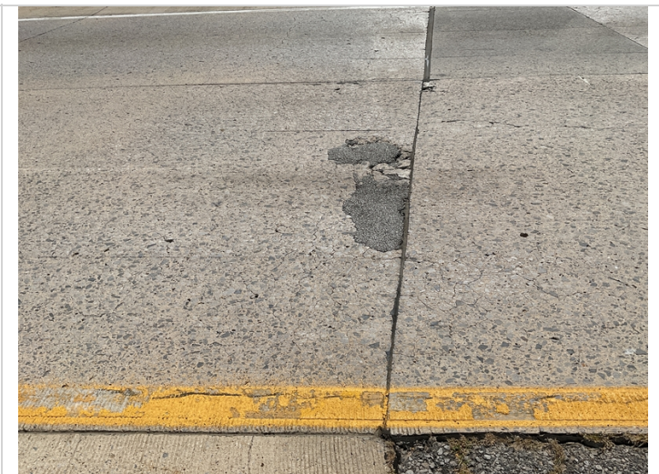
Abutment #1 approach slab spalling.
