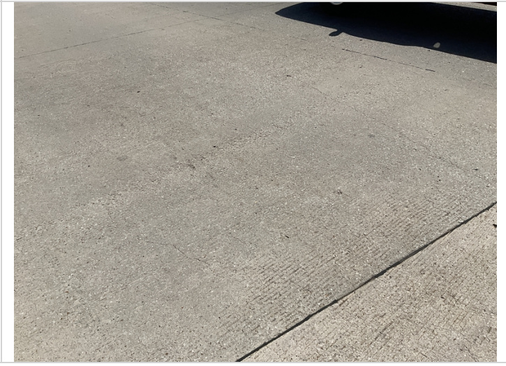
Sealable deck cracking.
