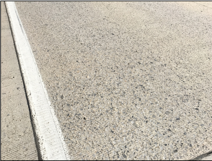
Approach slab-Mapcracking.
