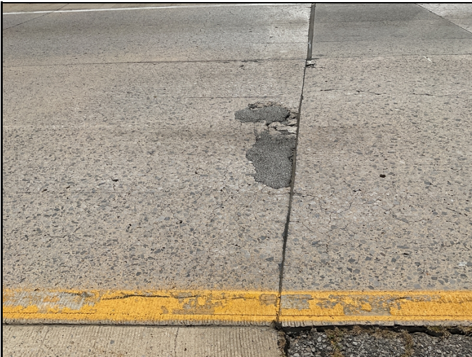
Abutment #1 approach slab spalling.
