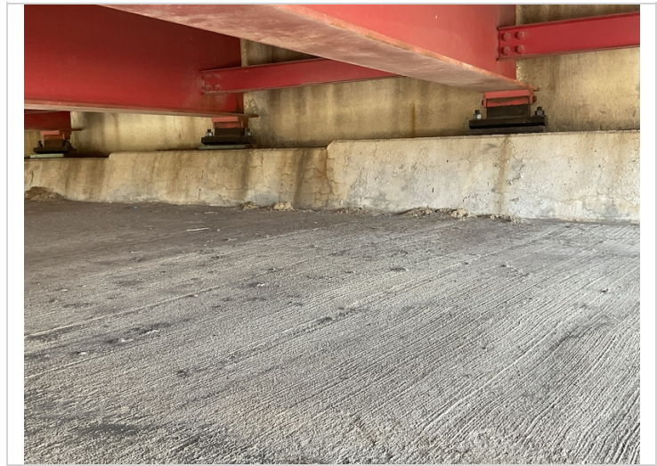
Abutment #1 typical map cracking.
