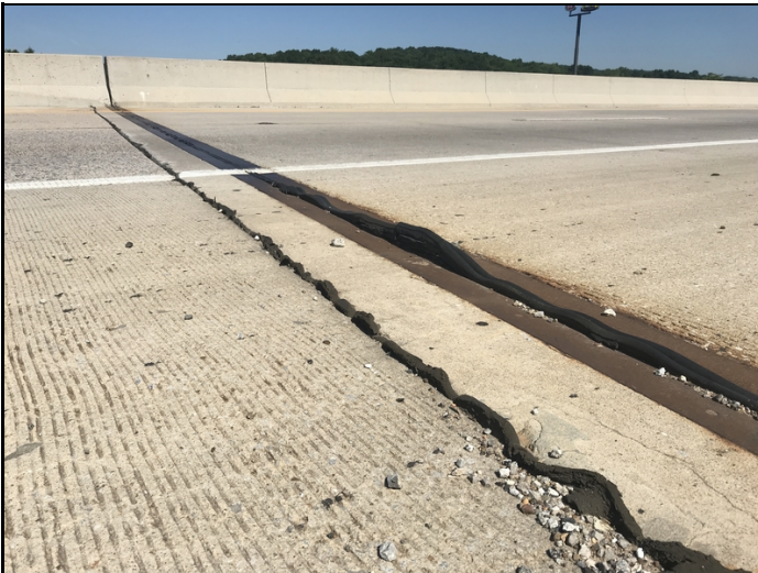
Abutment 1 expansion joint seal.
