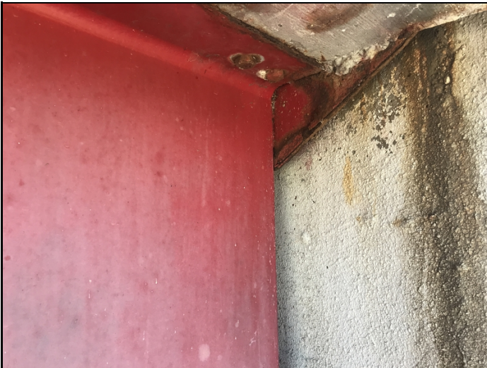
Beam # 6 has corrosion with initial section loss to the exterior side of the top flange over abutment # 2.
