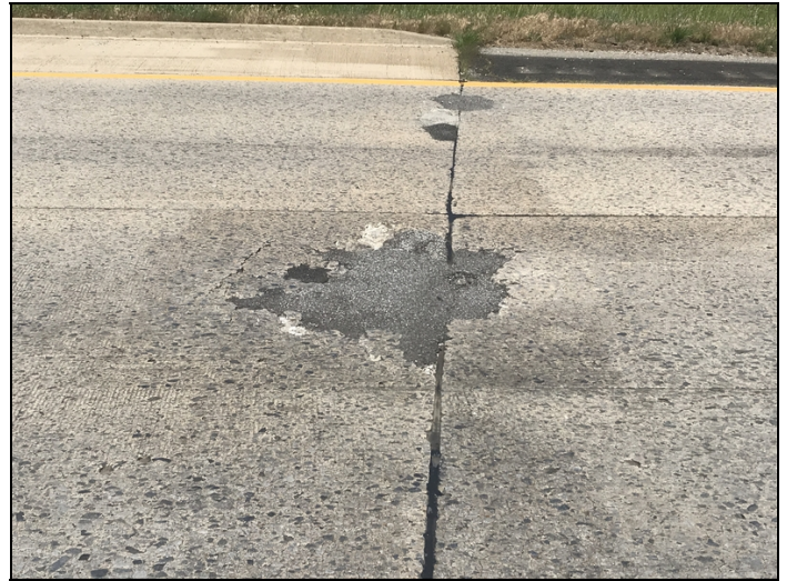
The North approach slab has a 4' x 4' area of settlement / spalling with failing asphalt repairs in the outside lane at the juncture of the approach roadway.
