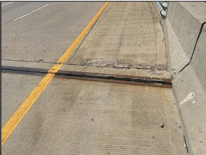
Abutment #1 Lt gutter spalling.
