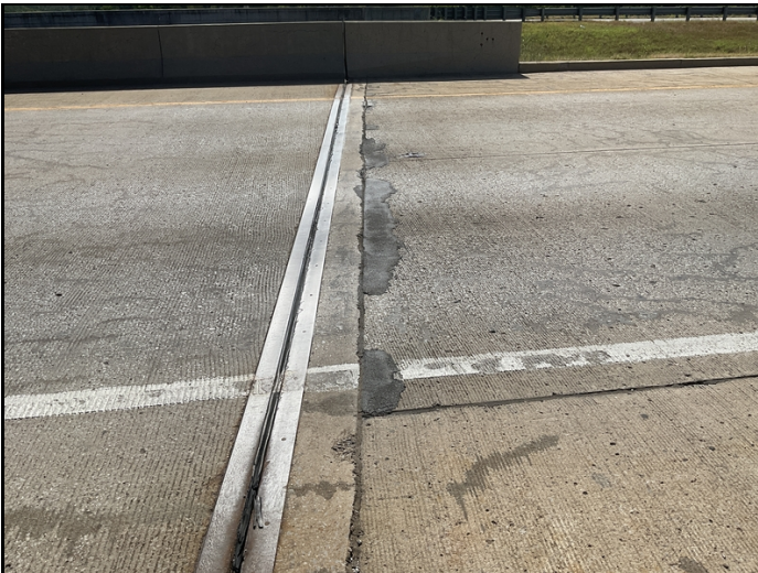
Abutment #1 approach slab repairs.
