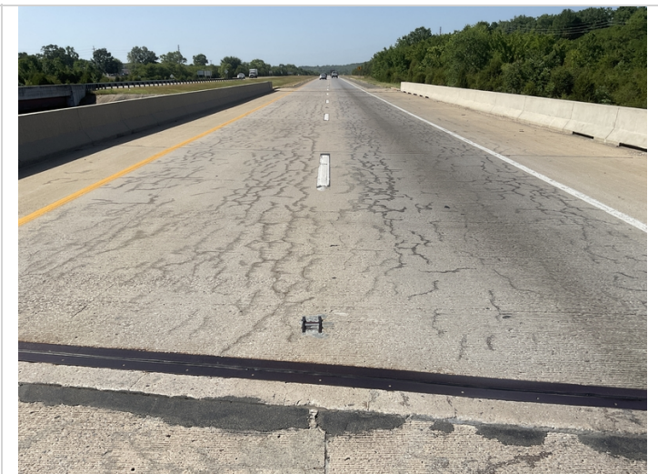
Typical driving surface of the deck.
