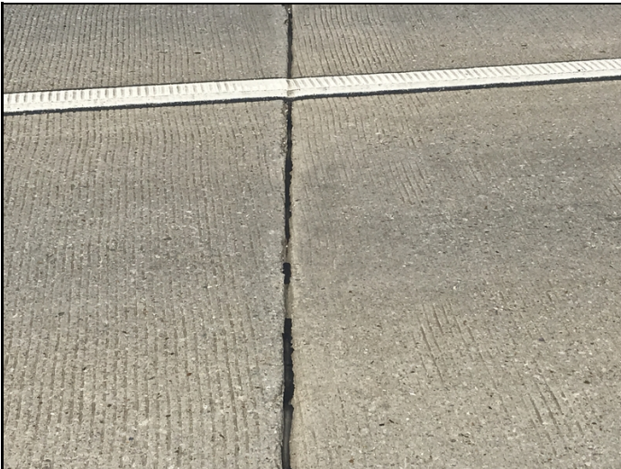
Sawn joint sealant missing.
