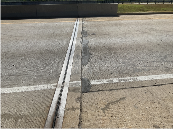
Abutment #1 top of back wall cracks sealed.
