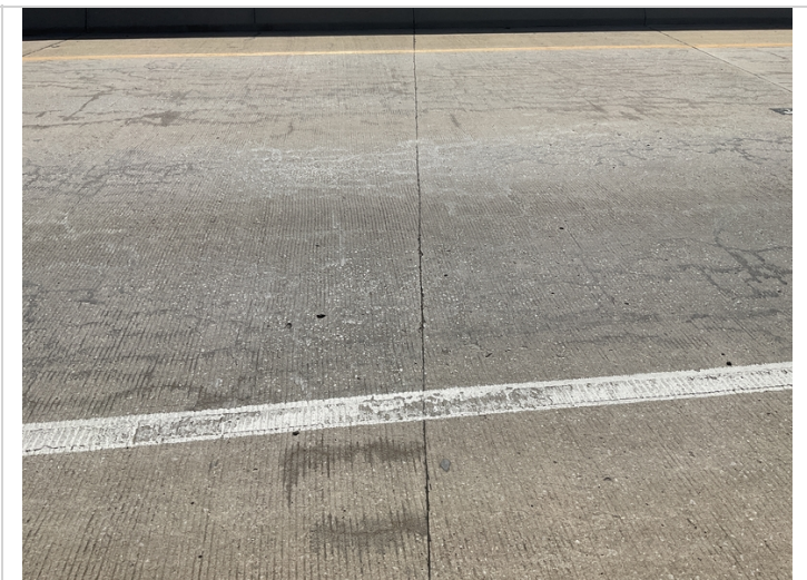
Failing saw joint sealant.
