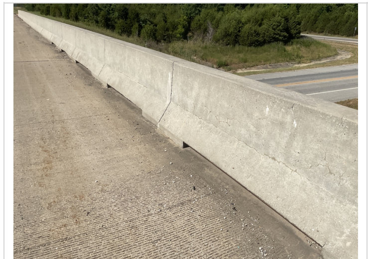
Typical concrete bridge rail.
