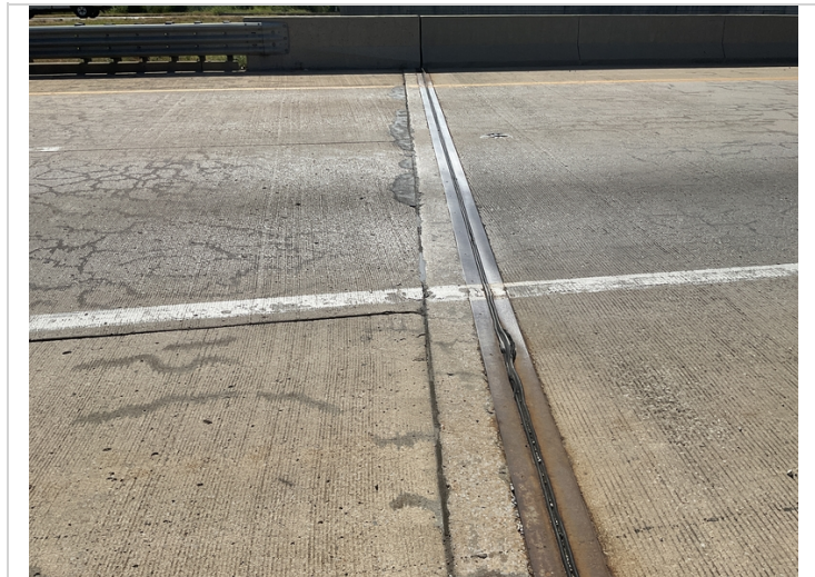
Abutment #2 compression joint seal.
