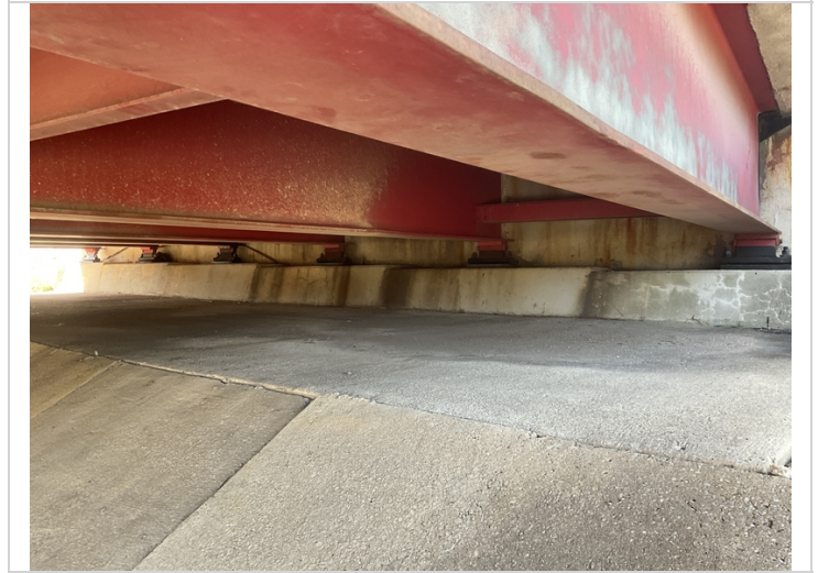
Abutment #1 bearings have been painted.
