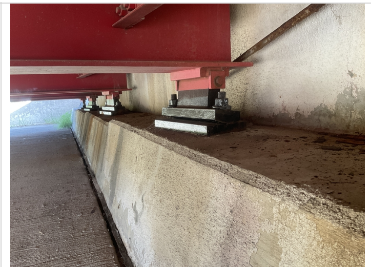
Abutment #2 bearings mostly painted
