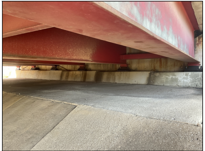
Abutment #1 bearings have been painted.
