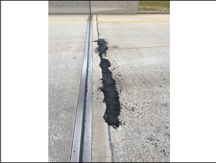
The South approach slab spall temporarily patched with HPM 7/1/20.
