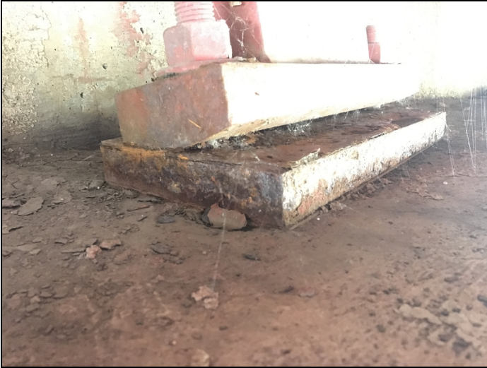
Some of the bearings at the abutments have active corrosion between the rocker and the masonry plate.
