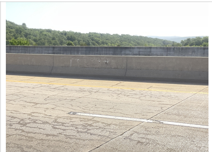
Rt bridge rail cracking with efflorescence buildup.
