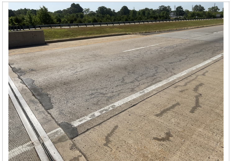
Abutment #1 approach slab cracks sealed.
