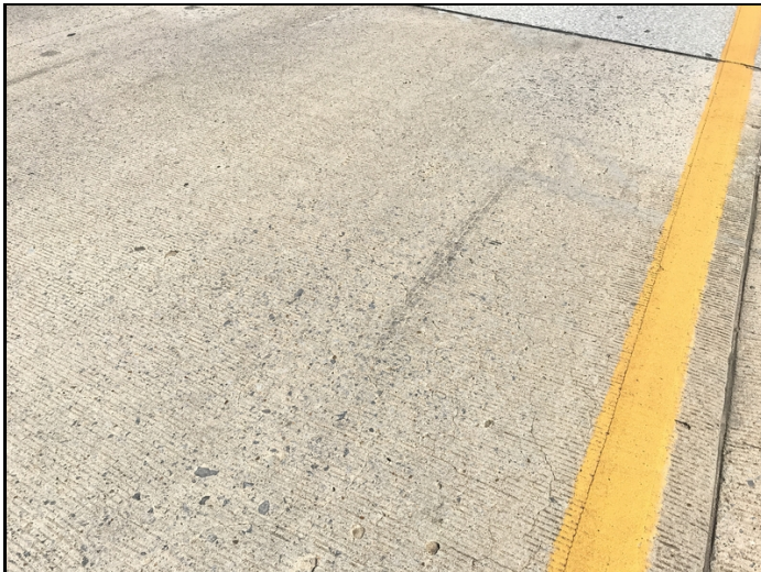
The approach slabs have sealable cracking .
