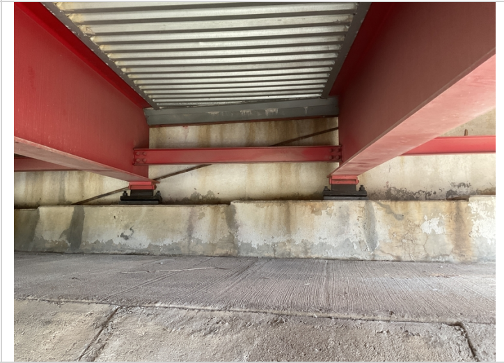
Abutment #2 road iron compression joint seal support fractured loose and dropped down out of position.
