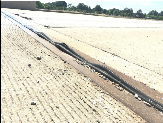
Abutment 1 expansion joint seal in left shoulder protruding above assembly.
