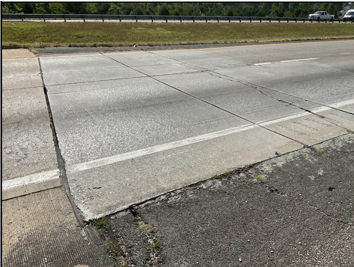
South approach roadway joint seal missing and fractured concrete slabs.
