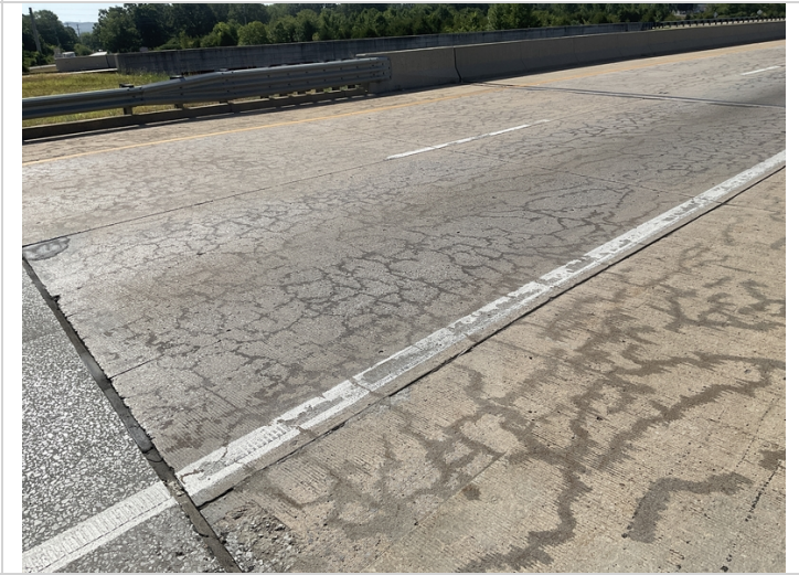
North approach slab cracking sealed.
