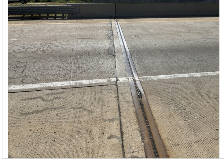
Abutment #2 top of back wall cracks sealed.
