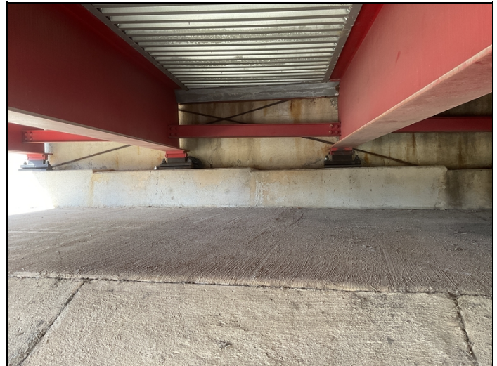
Abutment #1 road iron compression joint seal support fractured loose and dropped down out of position.
