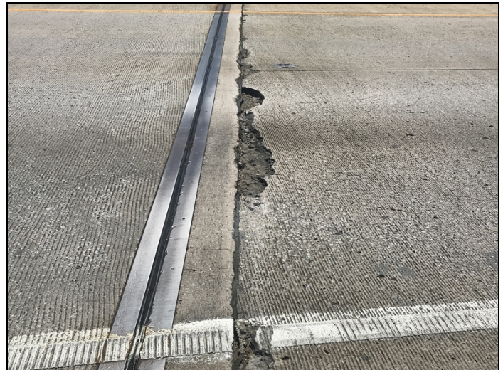
The South approach slab has several large spalls adjacent to the abutment backwall. The most extreme area is in the outside lane with a 7' long x 10" wide spall.
