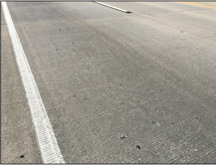
Span 3, left lane-Mapcracking.
