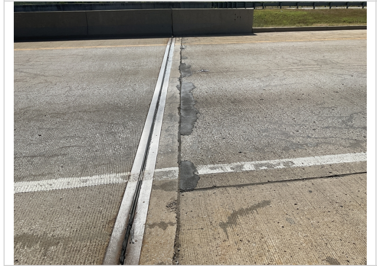
Abutment #1 approach slab repairs.
