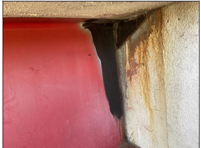
Abutment #1 beam #1 rust inhibitors applied to areas of active corrosion.
