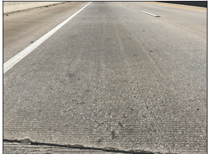
Span 1, left lane-Longitudinal cracking.
