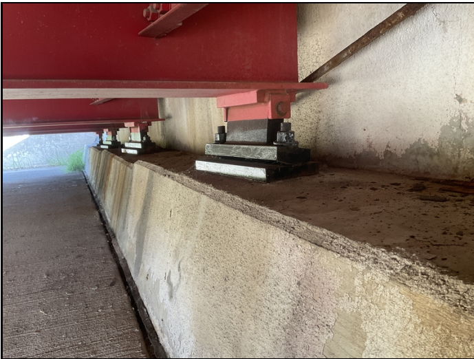
Abutment #2 bearings mostly painted
