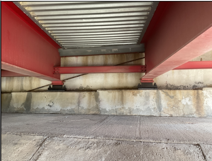
Abutment #2 road iron compression joint seal support fractured loose and dropped down out of position.
