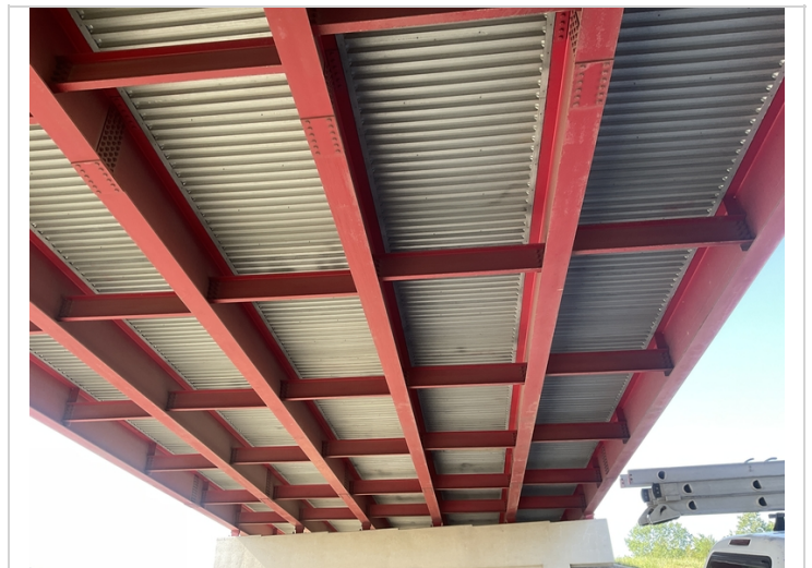
Span #2 typical undersurface of the deck.
