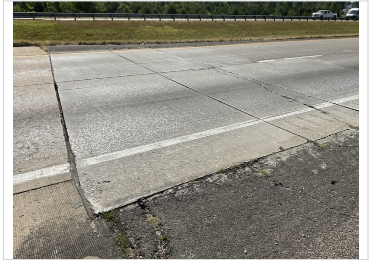
South approach roadway joint seal missing and fractured concrete slabs.
