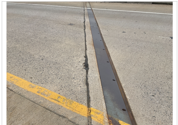
Abutment #2 top of the backwall transverse cracking with light wear.
