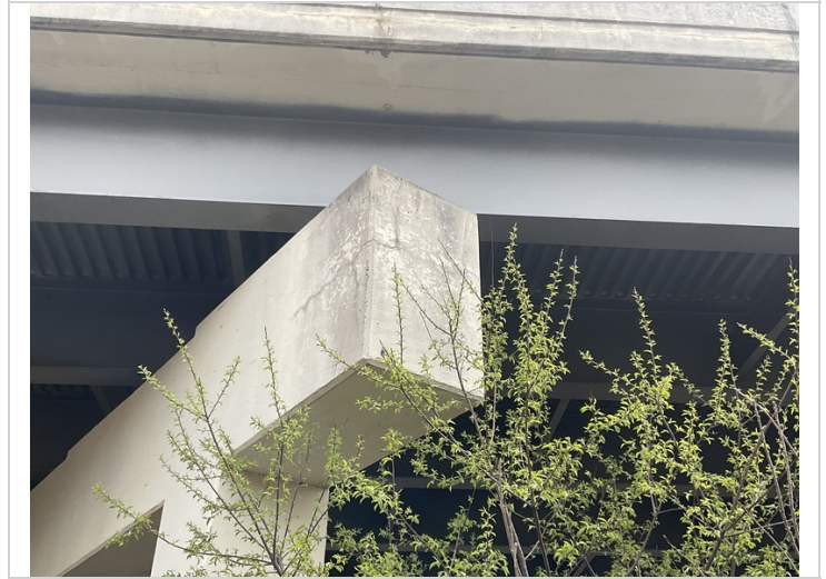
Bent #4 Lt map cracking.
