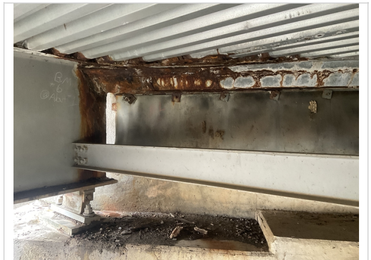
Abutment # 1 Beam # 6 active corrosion with up to 1/8" section loss at the base of the expansion dam.
