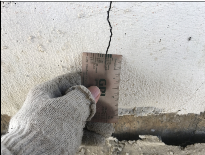
Bent # 2, column # 2 vertical cracks measure up to 0.060" in width during this inspection.
