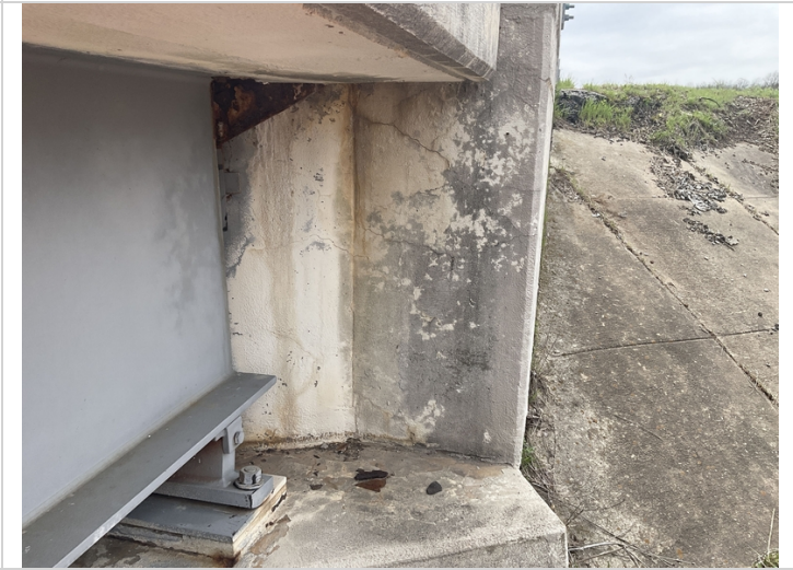
Abutment #1 Lt wing wall juncture map cracking.
