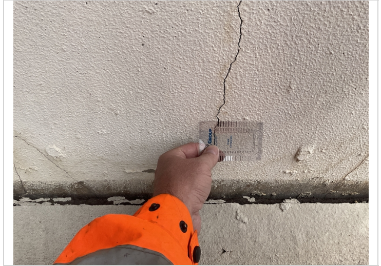
Bent # 2 column # 1 vertical cracking.
