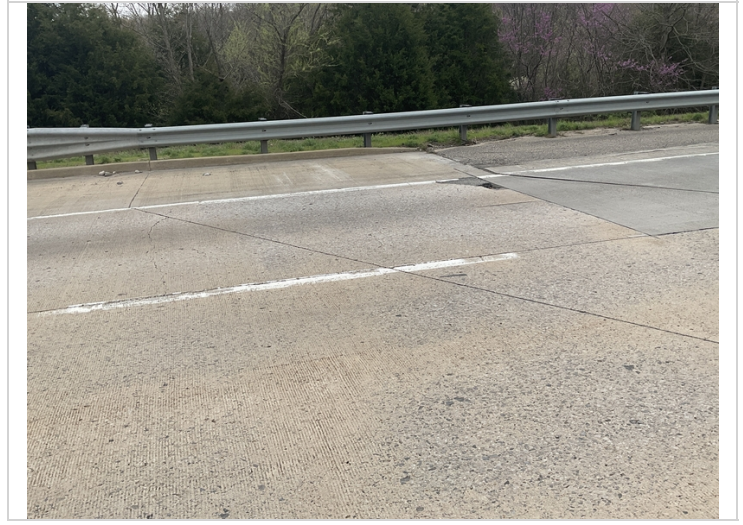
South approach slab concrete spalling and wide transverse cracking.
