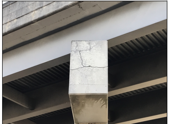
Left end of Bent # 3 cap.
