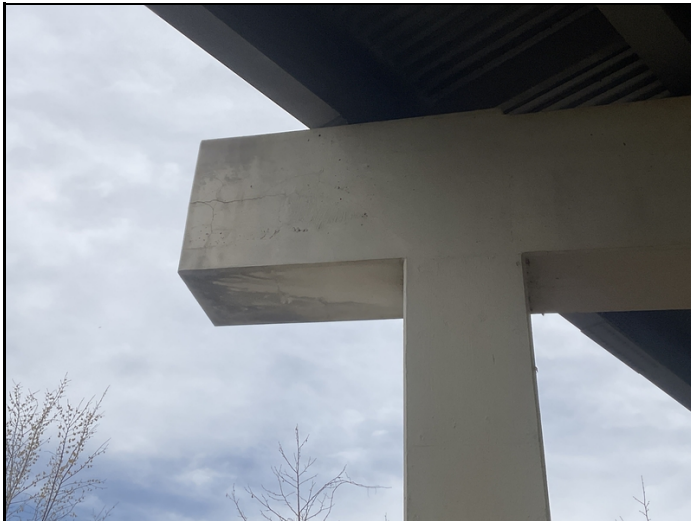
Bent 3 cap, left side-Wide cracking.
