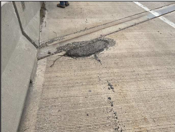
Span #1 Rt concrete deterioration with a failing temporary asphalt patch.
