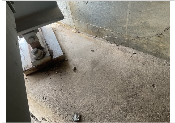
Abutment # 2 Lt map cracking at beam # 1.
