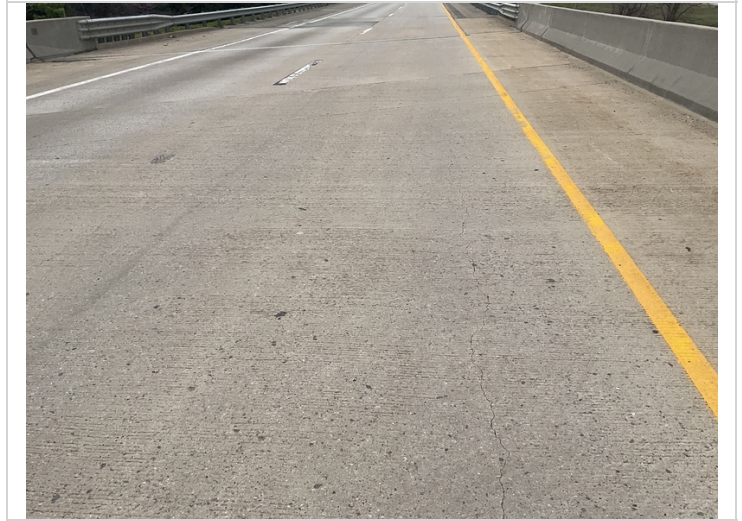
Span #1 sealable deck cracking.
