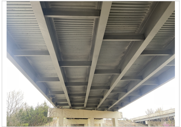
Typical undersurface of the deck.
