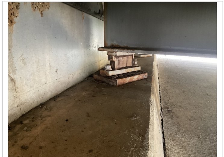
Abutment # 2 bearing # 3 active corrosion with pack rust.
