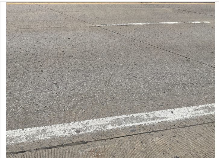
North approach slab cracking.
