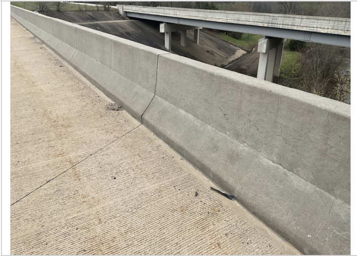
Typical bridge rail cracking.
