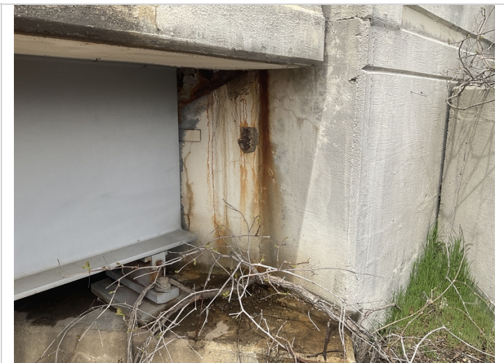
Abutment # 2 Rt concrete spalling with exposed reinforcing steel.
