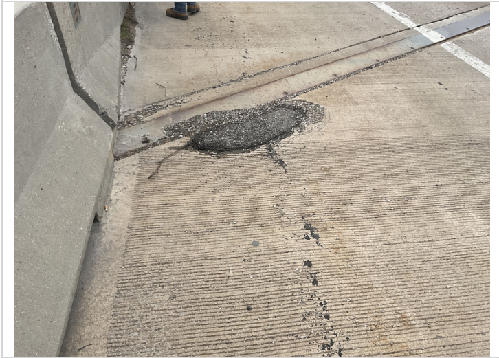
Span #1 Rt concrete deterioration with a failing temporary asphalt patch.
