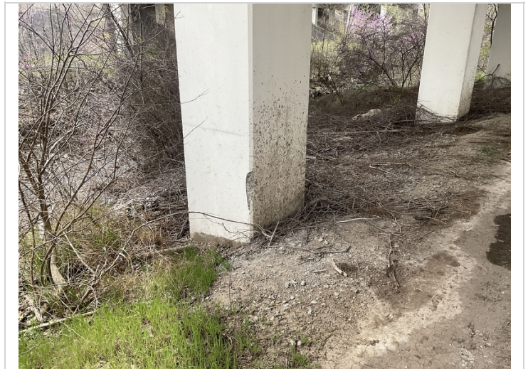
Bent # 4 column # 3 has a 5" spall in the corner of the column with no exposed reinforcing steel.
