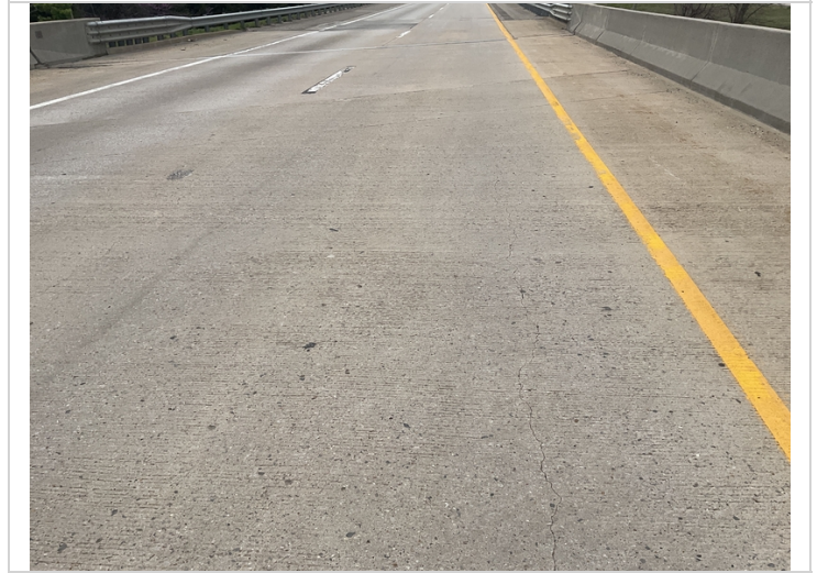
Span #1 sealable deck cracking.
