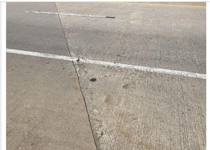
Span #3 Rt concrete deterioration and section loss.
