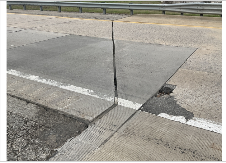
South approach slab joint seal missing.
