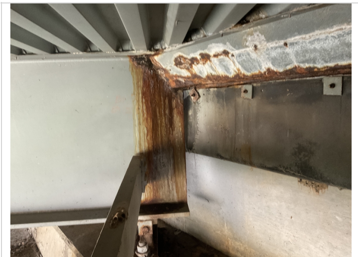
Abutment # 2 beam # 3 active corrosion with initial section loss at the expansion dam.
