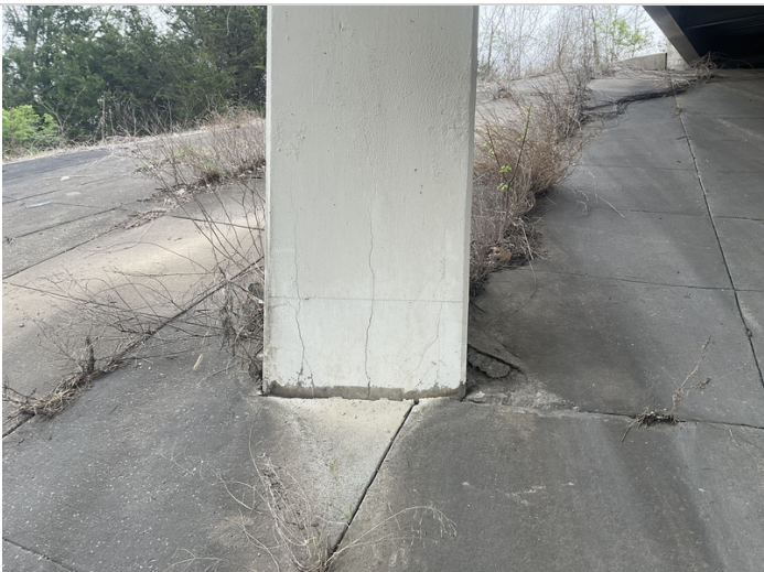
Bent # 2 Column #3 vertical cracks.
