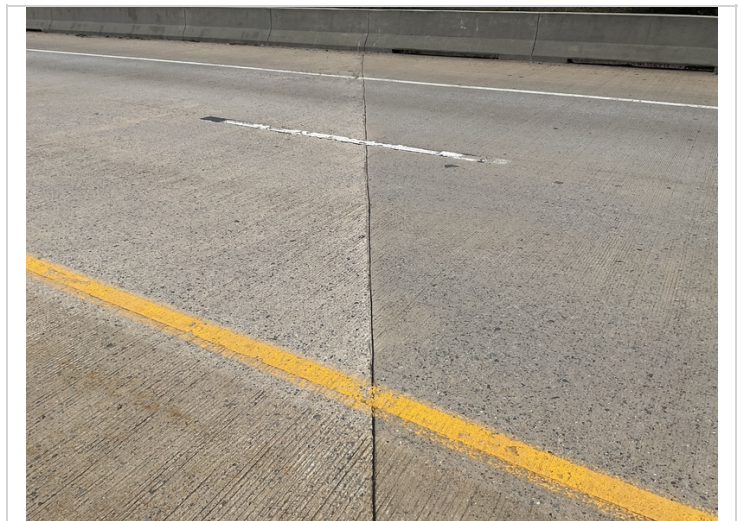
Failing saw joint sealant.
