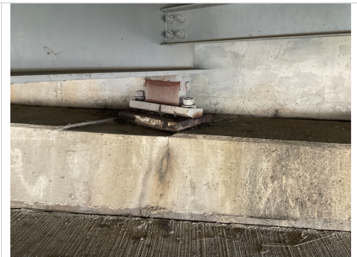
Abutment # 1 bearing #4 active corrosion with pack rust.
