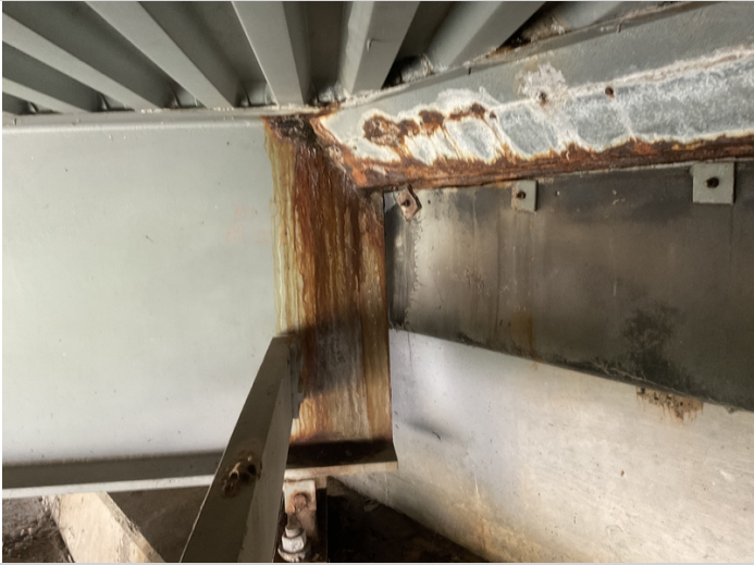
Abutment # 2 beam # 3 active corrosion with initial section loss at the expansion dam.
