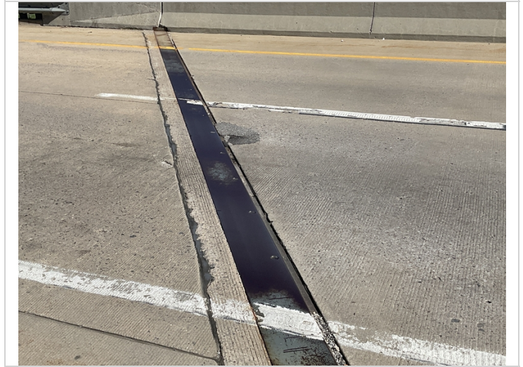
Span # 4 concrete spalling near the centerline at Abutment # 2.
