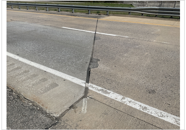
North approach slab spalling with temporary asphalt patches.
