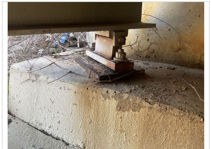
Abutment # 1 bearing # 6 active corrosion with flaking rust.
