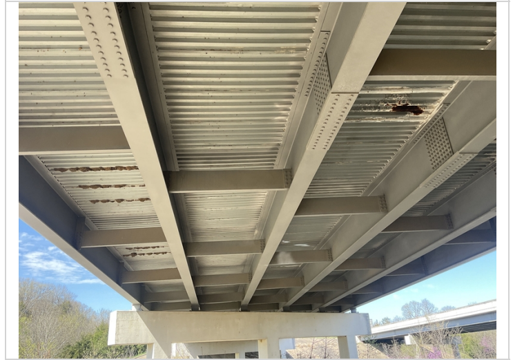
Span # 2 active corrosion in the deck pans.
