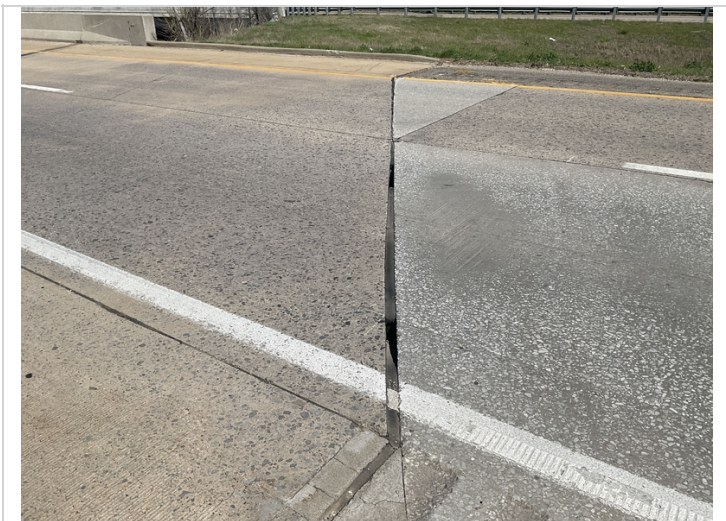
South approach slab missing joint seal.
