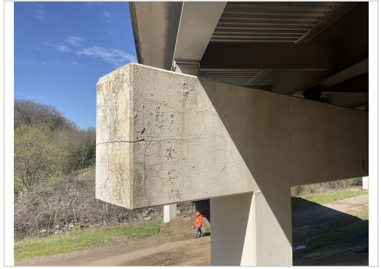
Bent # 2 Lt map cracking.
