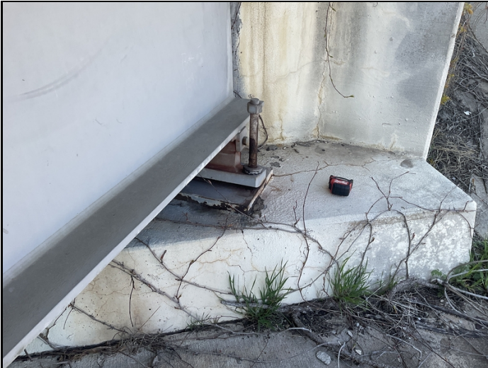
Abutment # 2 beam # 6 art anchor bolt working out of the cap.
