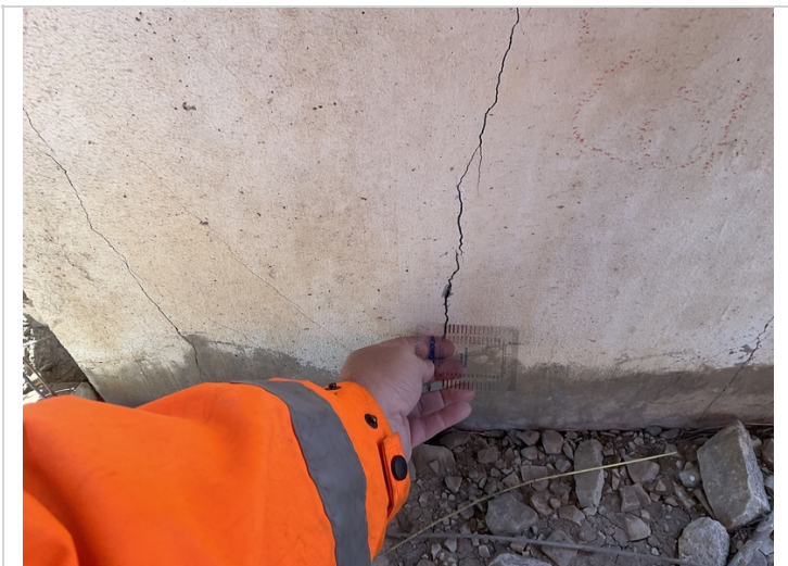
Bent # 4 column # 1 with 0.060" wide vertical cracking.
