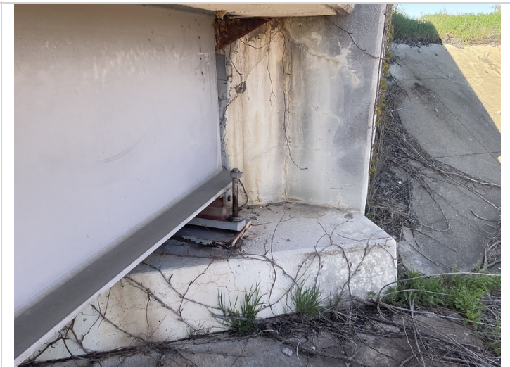
Abutment # 2 Rt end of the cap and back wall has map cracking with light efflorescence buildup.
