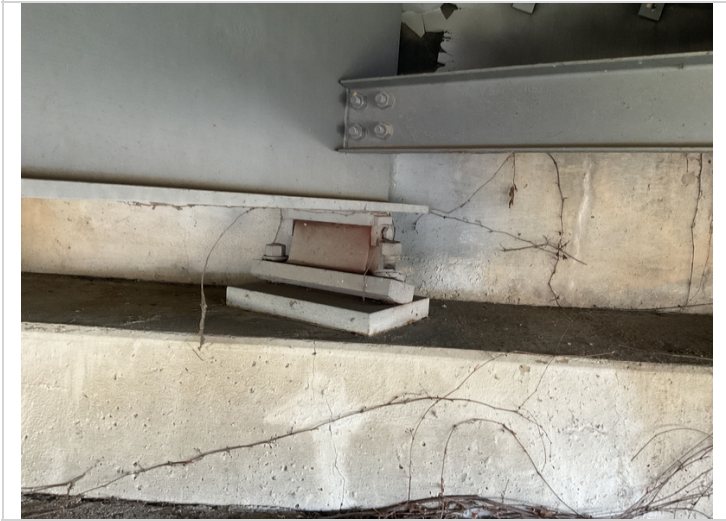
Abutment # 2 beam # 4 Rt bearing anchor bolt is working its way out of the cap.
