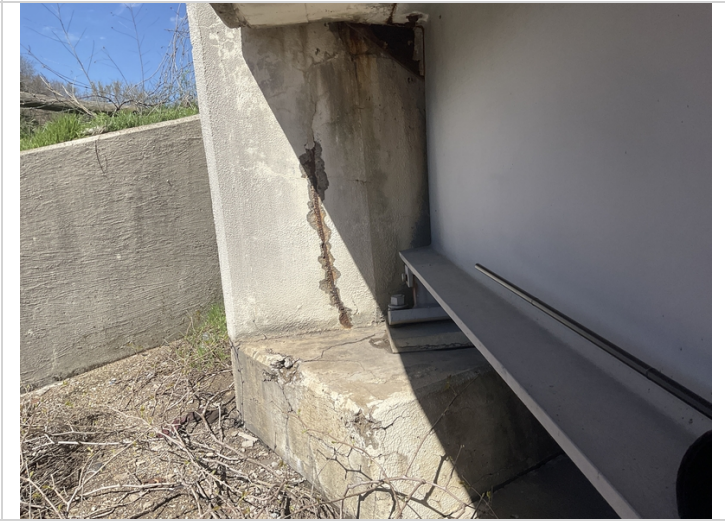
Abutment # 2 Lt back wall concrete spalling with exposed reinforcing steel.
