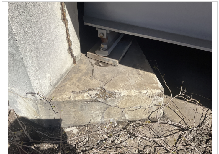
Abutment # 2 Lt end of the cap has concrete deterioration with up to 2" of section loss and map cracking in the bearing area.
