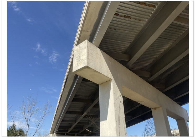
Bent # 3 Lt map cracking.
