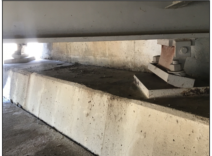
Bearings # 1 & 2 at abutment # 2. Temperature is 60 degrees Fahrenheit.
