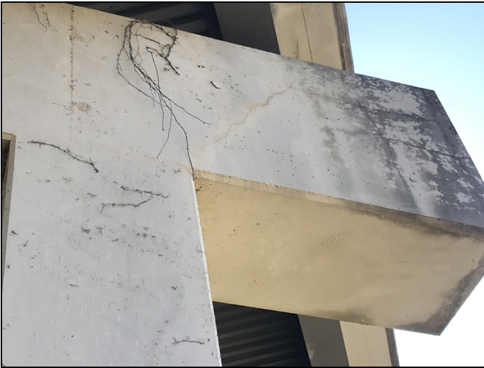
The ahead face of bent # 3 cap has a narrow diagonal shear type crack that propagates upward from exterior side of column # 1.
