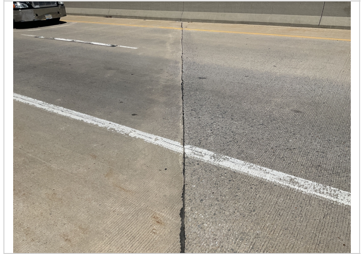
Span # 4 missing saw joint sealant.
