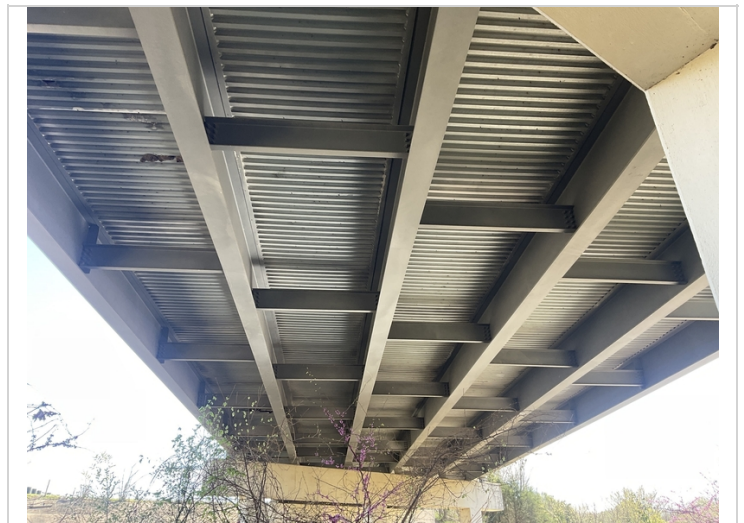
Typical undersurface of the deck.
