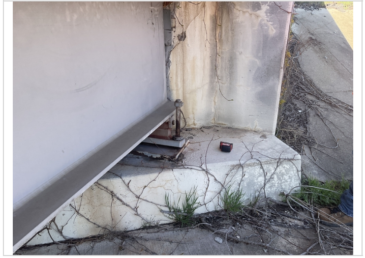
Abutment # 2 Lt map cracking at the end of the cap.
