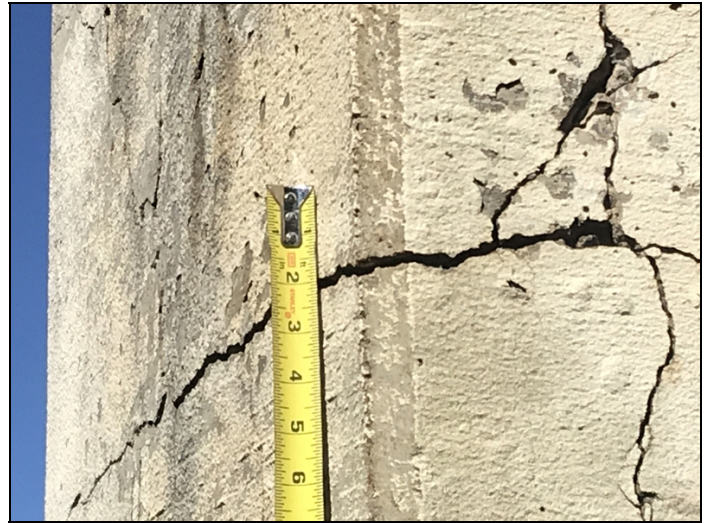
Bent 2 cap, left end-Wide mapcracking. Photo 1.
