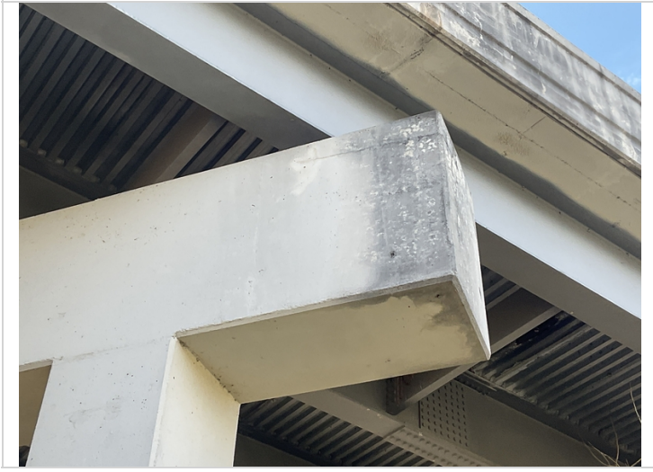
Bent # 3 Rt map cracking.
