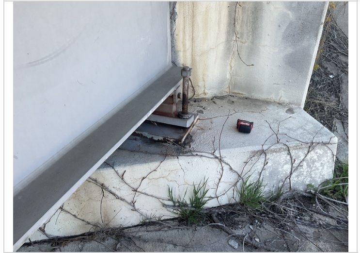
Abutment # 2 beam # 6 art anchor bolt working out of the cap.
