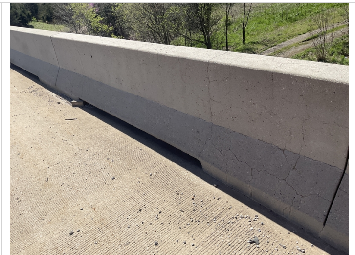
Bridge rail with wide vertical and map cracking.
