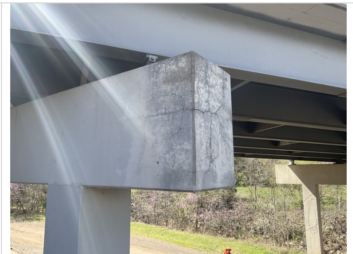
Bent # 2 Rt map cracking.
