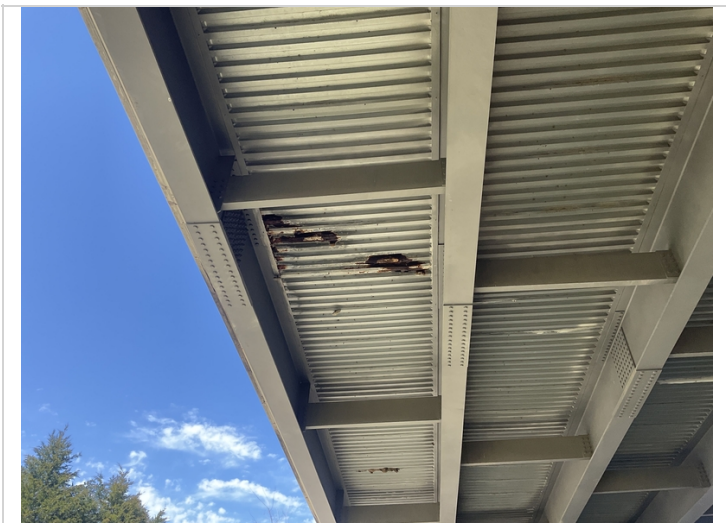
Span # 4 bay # 1 active corrosion in the deck pans.
