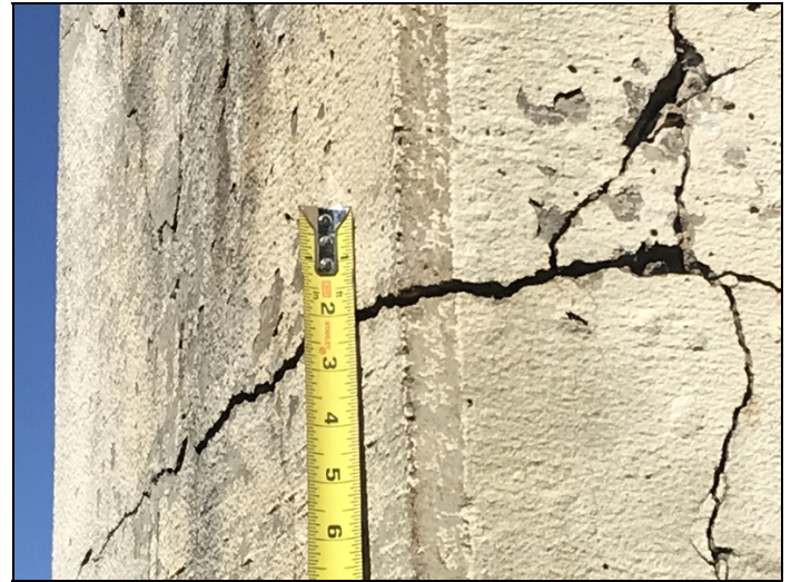
Bent 2 cap, left end-Wide mapcracking. Photo 1.
