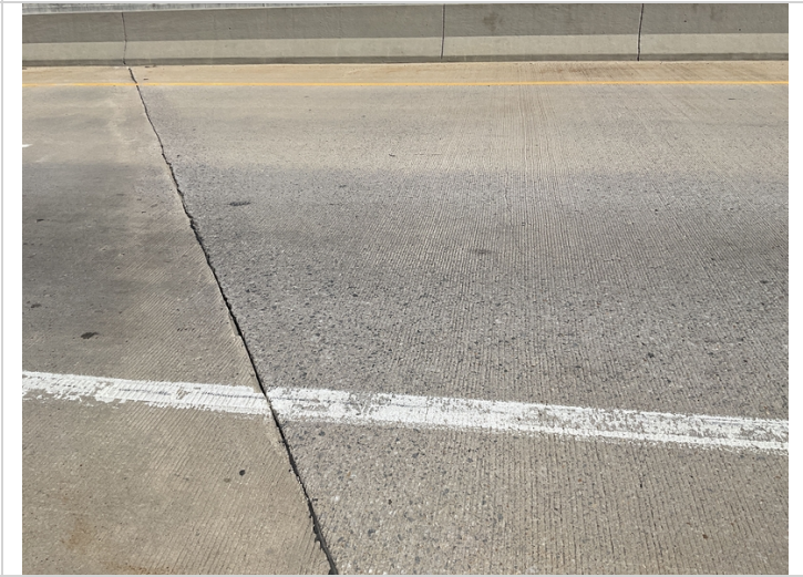
Sealable deck cracking.
