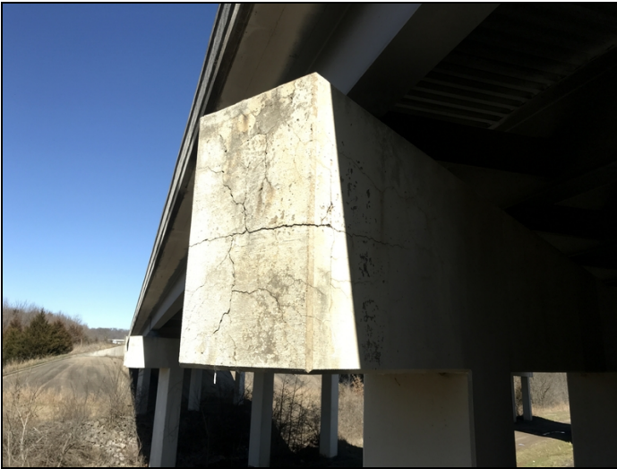
Bent 2 cap, left end-Wide mapcracking. Photo 2.
