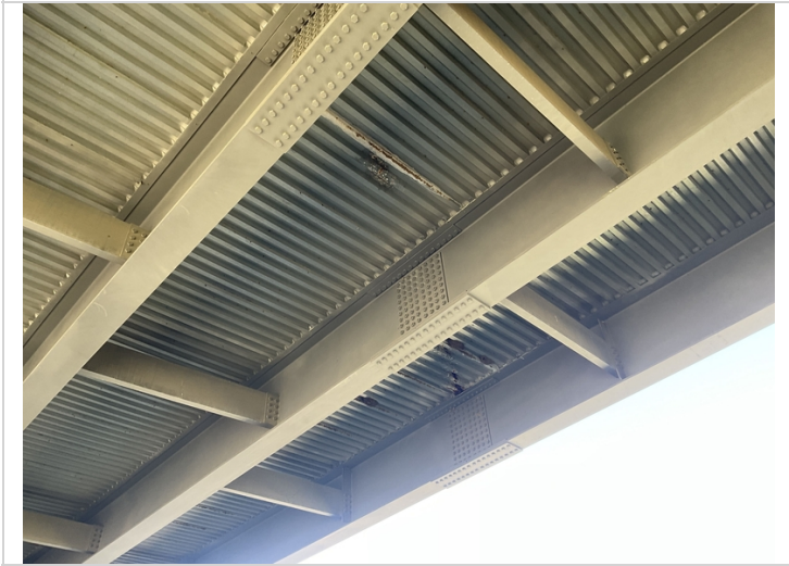
Span # 4 active corrosion in the deck pans.
