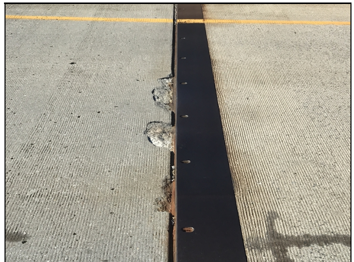
Span # 3 has areas of moderate sized spalling adjacent to bent # 4 sliding plate assembly.
