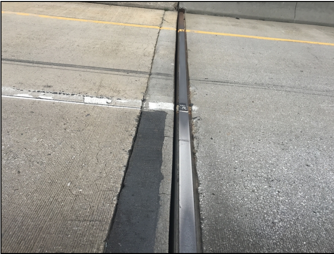
Missing expansion joint material at bent 1.
