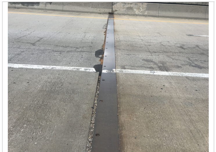
Bent # 4 sliding plate expansion joint typical.
