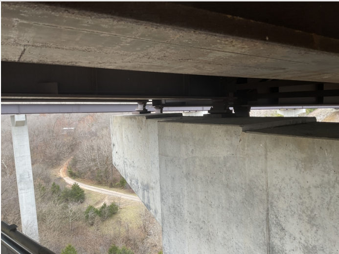
Bent # 4 bearings in the expanded position.
