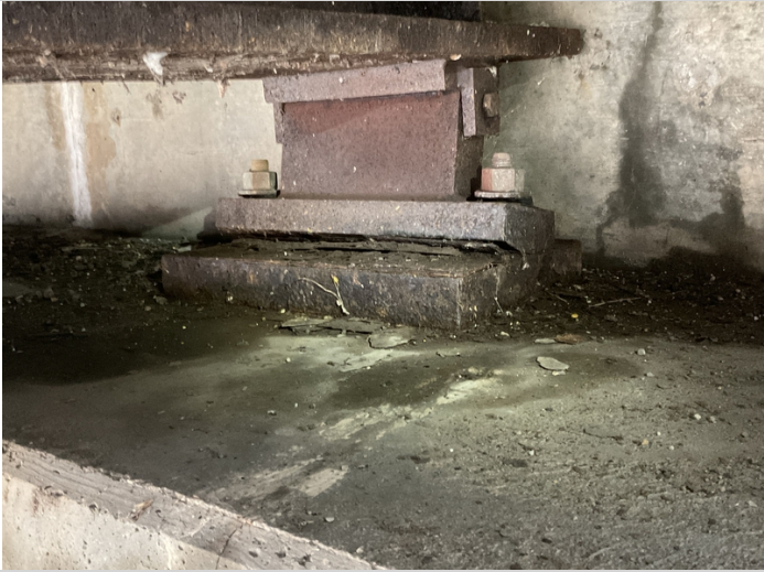
Abutment # 1 bearing #2 active corrosion with pack rust.
