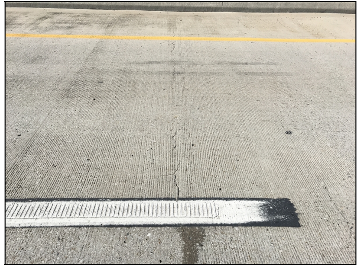
Transverse deck cracking.
