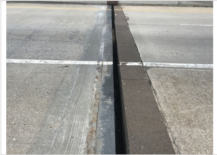
Abutment 2 open expansion joint.
