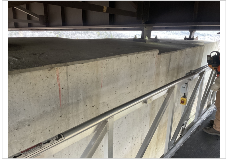
Bent #2 typical cracking.
