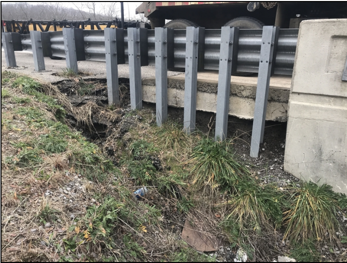
Right embankment at the south abutment has erosion with loss of cover to the approach railing and is beginning to undermine the approach gutter.
