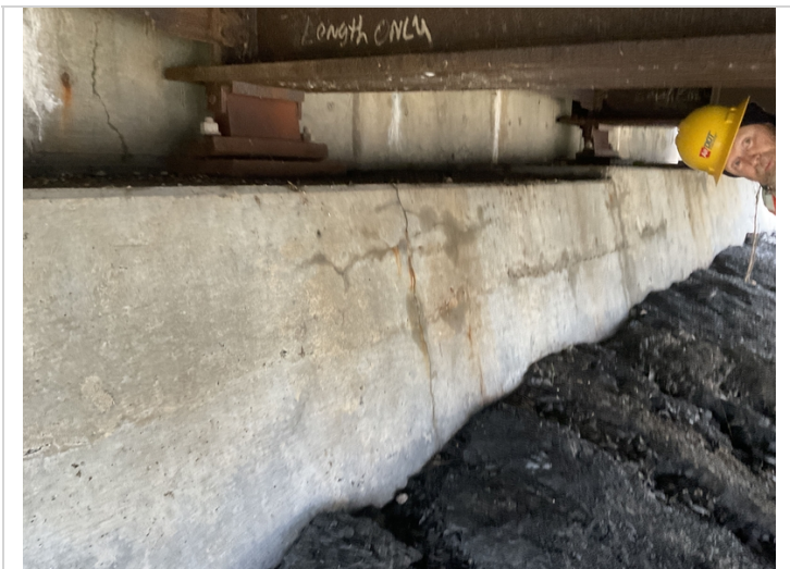
Abutment # 1 cap vertical and horizontal moderate width cracking.
