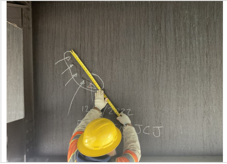
Span # 2 beam #3 laminar delamination in the web adjacent to diaphragm # 5 from bent #3.
