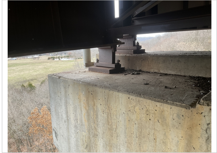
Bent # 4 Span #4 bearing #4 fractured anchor bolts.
