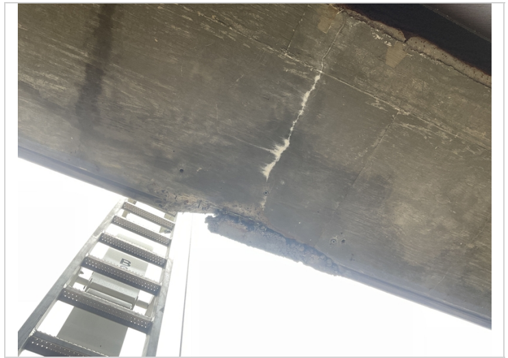
Span # 3 repair with honeycomb and exposed reinforcing steel.
