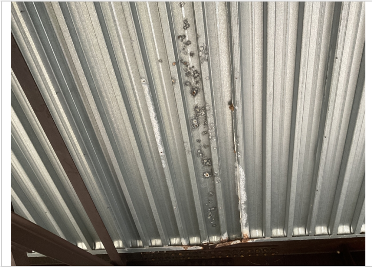
Span # 2 splice #1 bay# 2 active corrosion in the stay in place.
