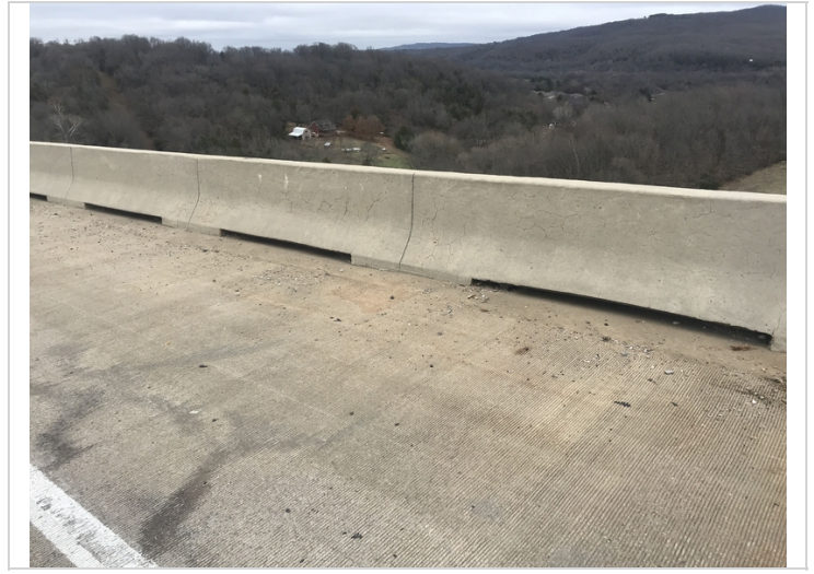
Heavy map cracking in the right parapet. Span 4.
