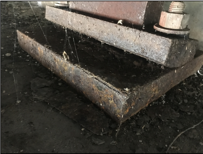
Abutment 1, bearing 3-Corrosion.
