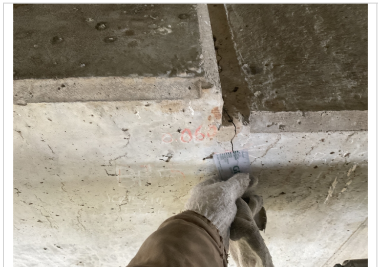
Bent # 5 vertical cracking at the centerline. 0.060" wide crack.
