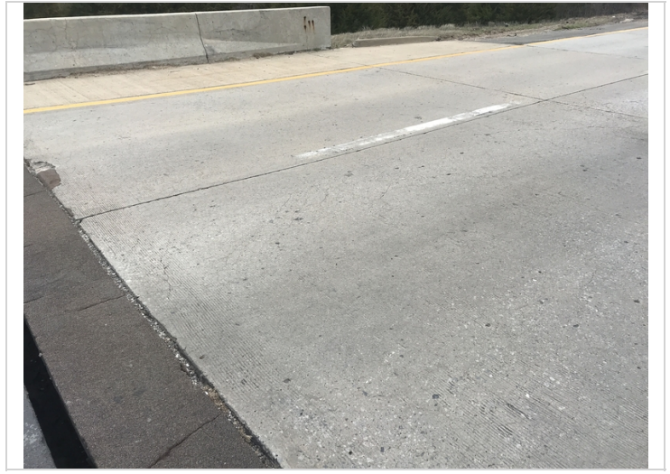
North approach slab. Sealable map cracking.
