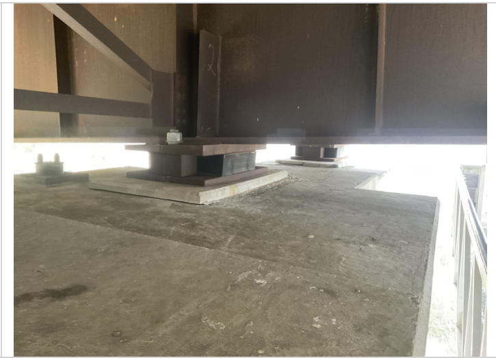
Bent # 7 bearing #3 elastomeric pad delaminated from the external load plate.
