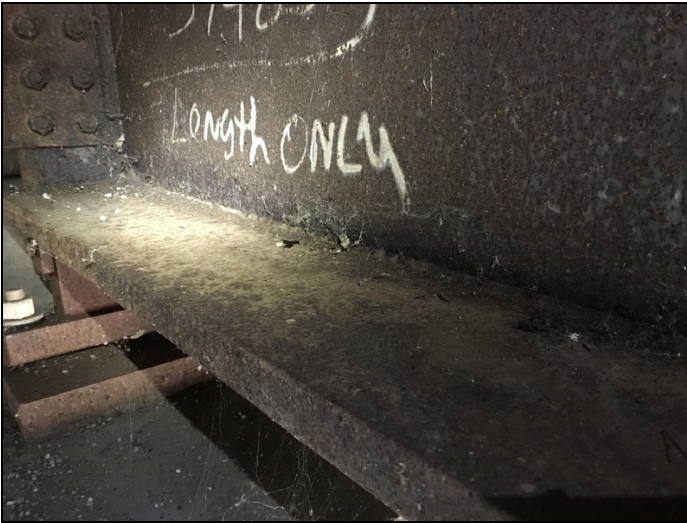
Span 1, girder # 3 at abutment # 1-Corrosion.
