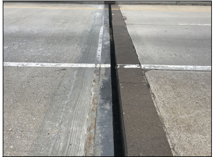
Open expansion joint at abutment 2.
