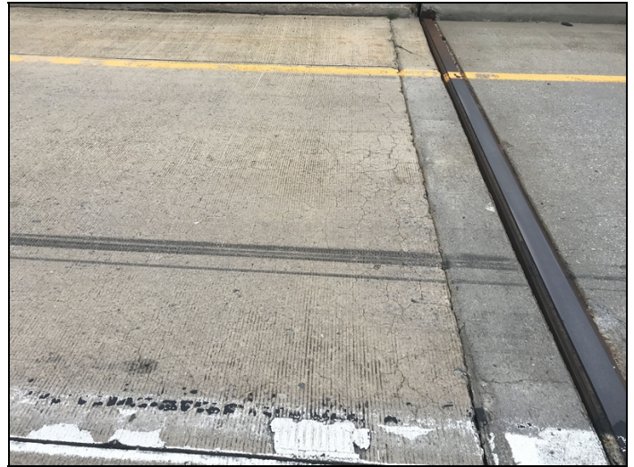
Sealable map cracking in the south approach slab.
