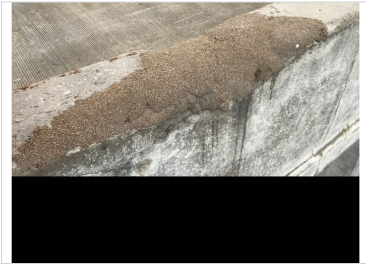
Epoxy and sand repair to a spall in span 5. Right.
