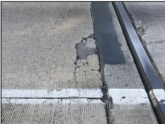
South approach slab, left lane-Spalling.
