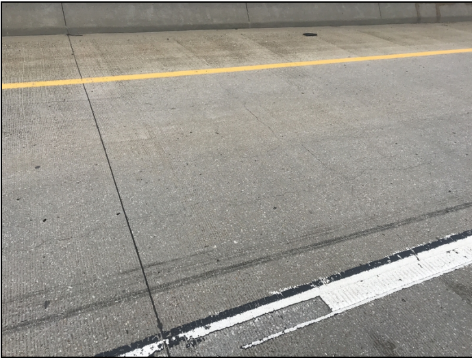
Sealable transverse cracking. Driving surface of the deck.
