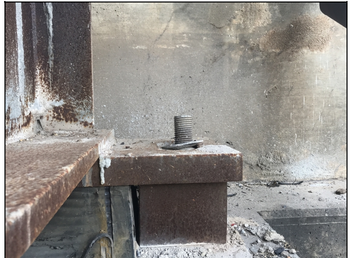
Abutment # 2, bearing # 4 has a missing anchor bolt nut.
