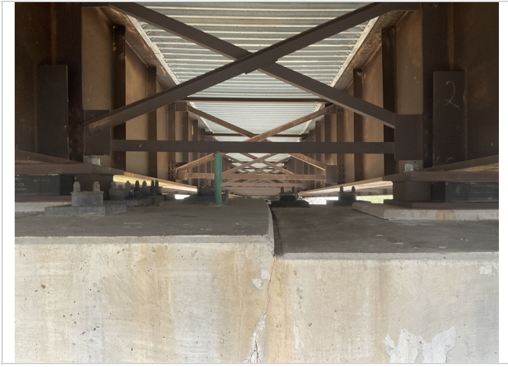
Bent # 7 repair appears to still be holding.
