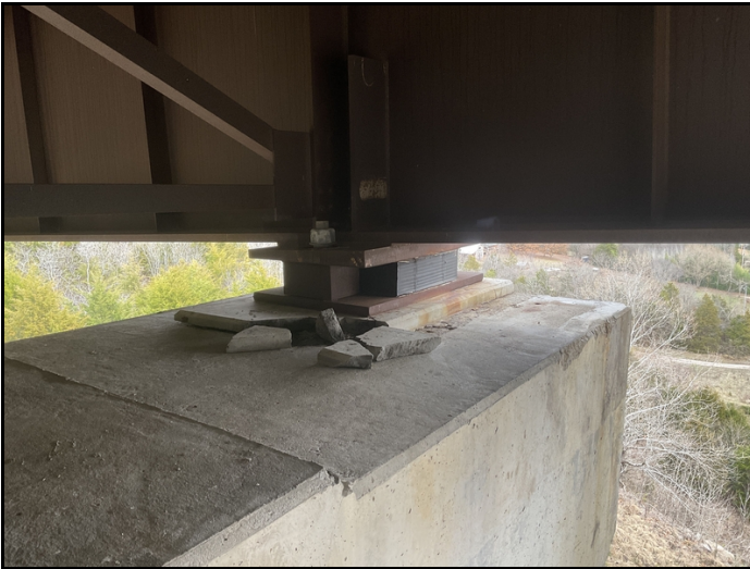
Bent # 7 bearing #4 fractured pedestal under the bearing.
