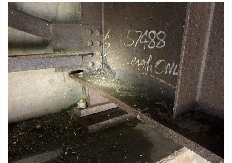
Abutment # 1 girder #2 active corrosion with pack rust over the bearing.
