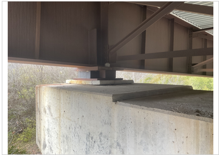
Bent # 7 beam #1 pedestal delaminated from the cap.
