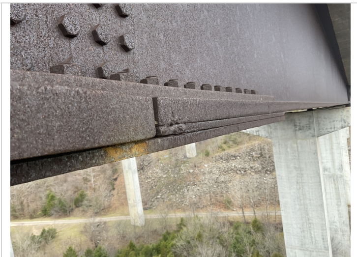
Span # 3 beam #4 tack weld on the splice spacer plate of the bottom flange.
