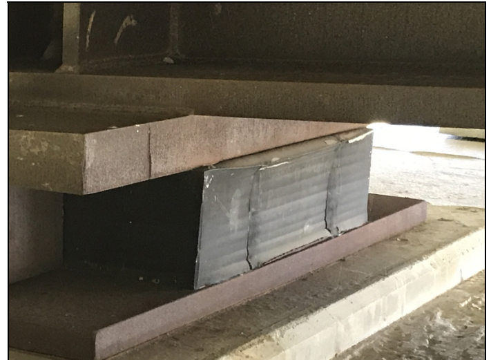
Bent # 7, Girder # 3 pad is de-bonded from the sole plate and protrudes 7/8" past the edge of the Sole plate.
