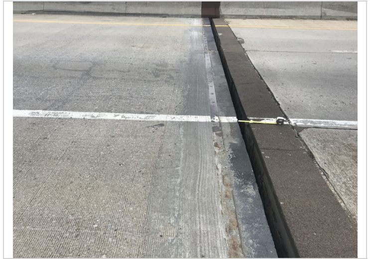
Grouted repairs adjacent to the north abutment.
