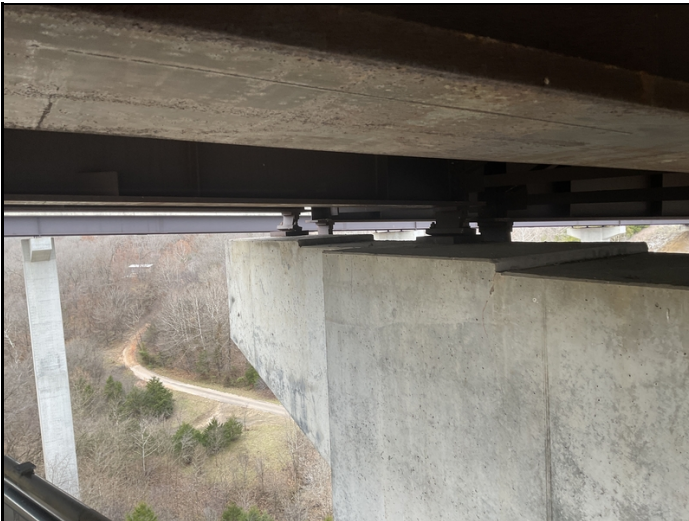
Bent # 4 bearings in the expanded position.
