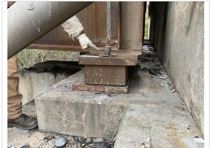
Abutment # 2 girder #4 missing anchor bolt nut.
