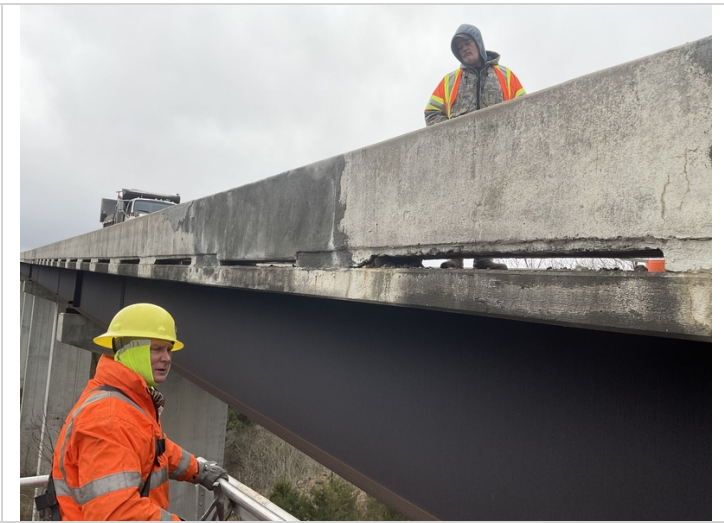
Span # 7 Rt exposed reinforcing steel in the base of the bridge rail.
