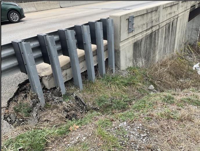
Abutment #1 Rt erosion.
