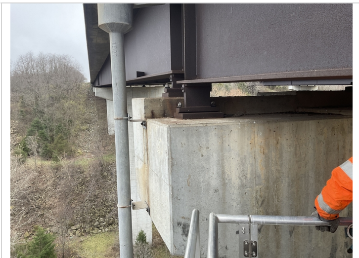
Bent # 4 Rt cap spalling with exposed reinforcing steel in the step of the cap.
