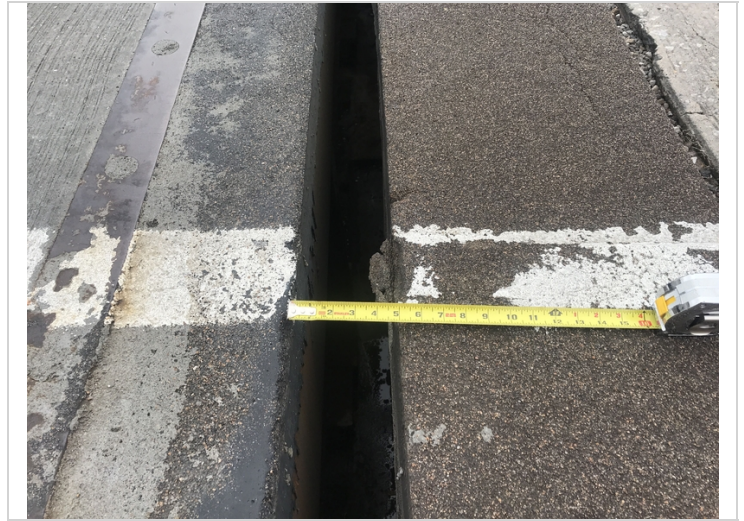
Abutment # 2 with a 5" wide open expansion joint measured at the white line.
