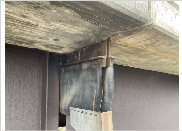
Bent # 4 expansion joint active corrosion with pack rust.
