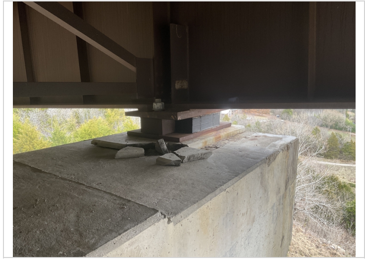
Bent # 7 bearing #4 fractured pedestal under the bearing.
