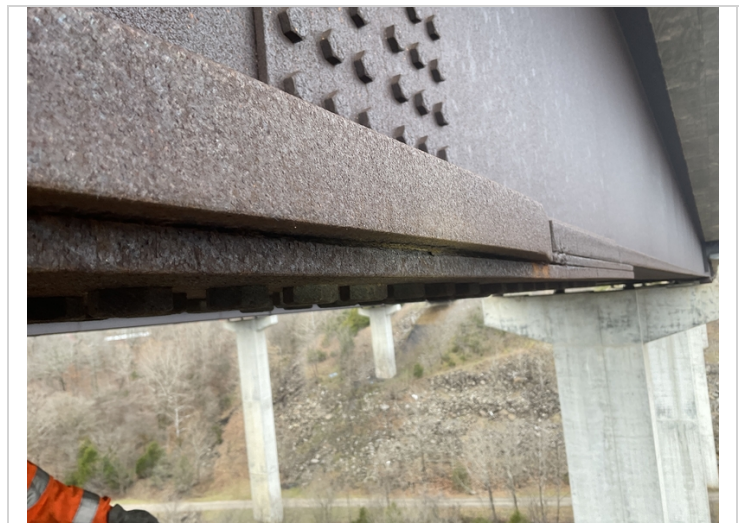
Span # 3 beam #4 pack rust between the splice plates.
