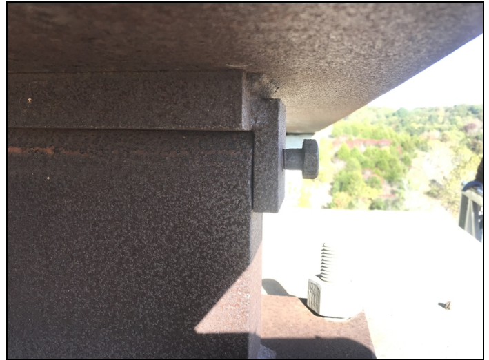
Fixed bearing # 5 at bent # 5 has one bolt that attaches the girder to the bearing device that is working out.
