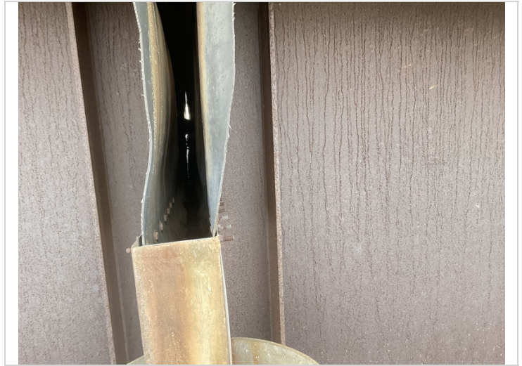
Bent # 4 minor debris accumulation in the trough.
