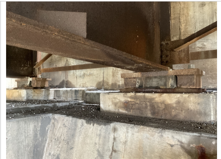
Abutment # 2 girders # 2 & 3 active corrosion with pack rust and section loss.
