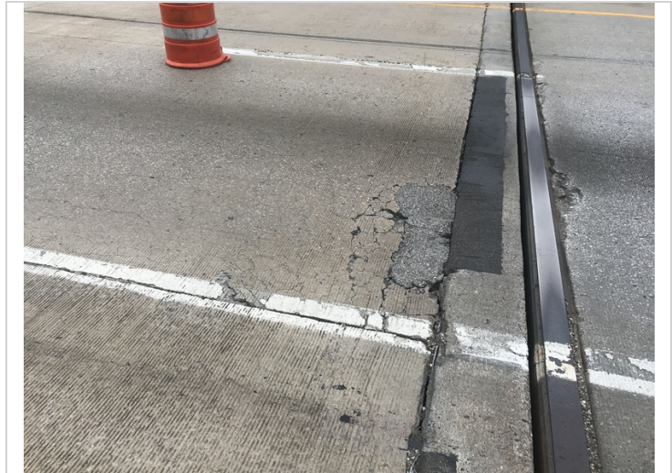
The south approach slab is breaking apart adjacent to the abutment # 1 backwall.
