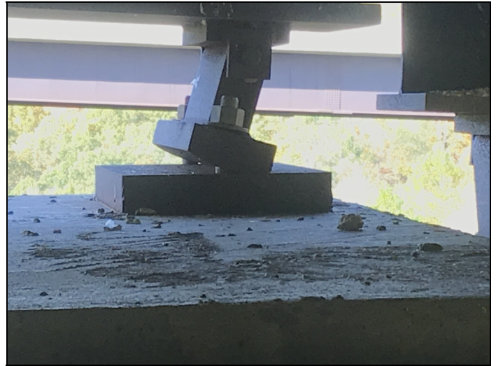
Span # 3, bearing 1 at bent # 4 appears to be fully expanded at this inspection. Ambient temperature at time of inspection is approximately 68 degrees Fahrenheit.
