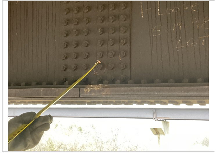
Span #3 girder #1 loose bolt in the splice.
