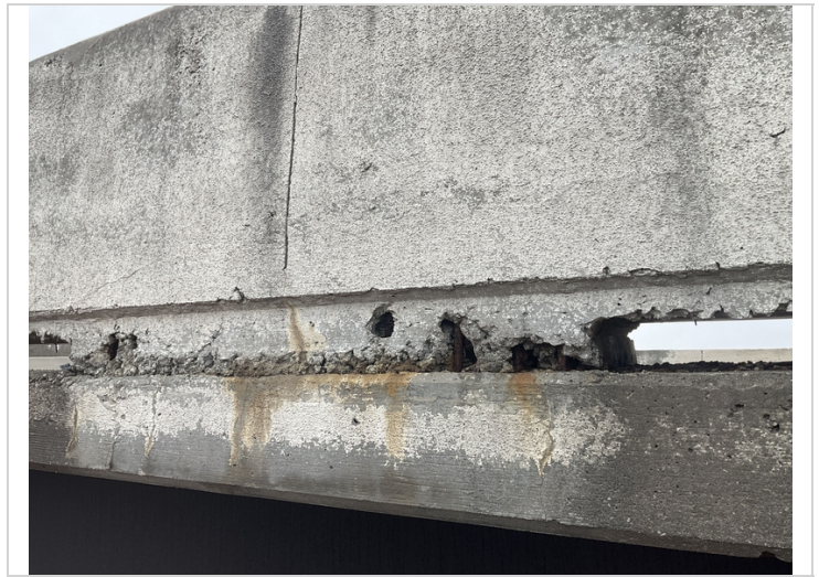
Span # 3 Rt bridge rail honeycomb with exposed reinforcing steel with active corrosion and pack rust.
