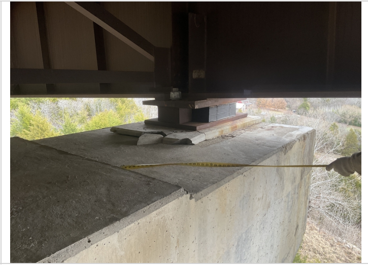
Bent # 7 bearing #4 fractured pedestal under the bearing.
