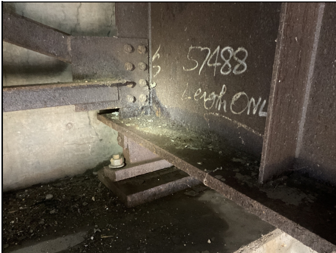
Abutment # 1 girder #2 active corrosion with pack rust over the bearing.
