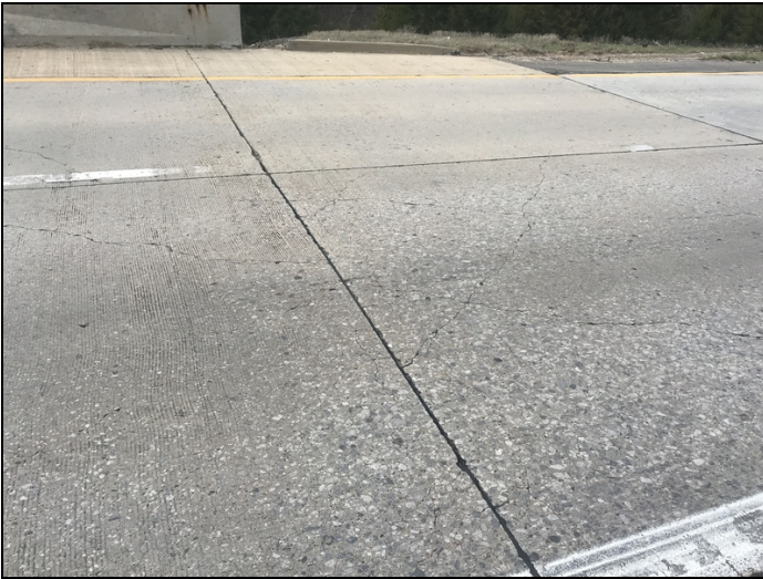
Wide diagonal cracks in the north approach slab.
