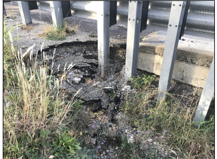
The slope on the right side of the South abutment has an area of erosion adjacent to the approach railing that has caused a loss of cover to the approach railing posts.
