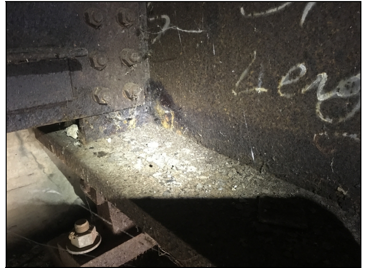
Span 1, girder # 2 at abutment # 1-Corrosion.
