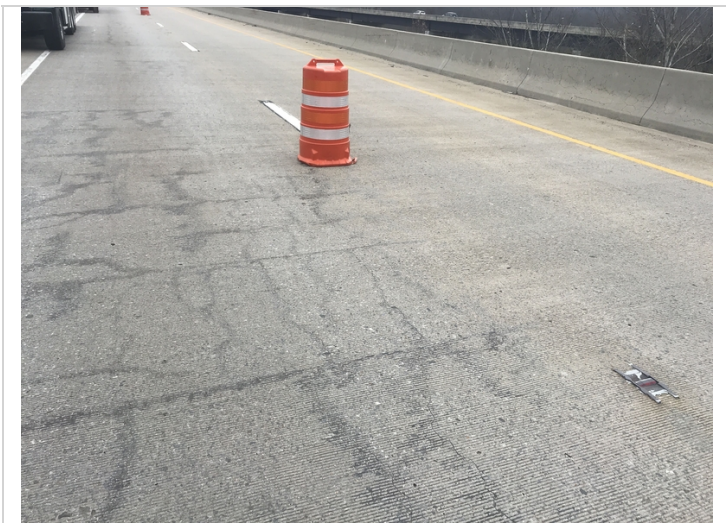
Span # 7 sealable cracking in the deck.
