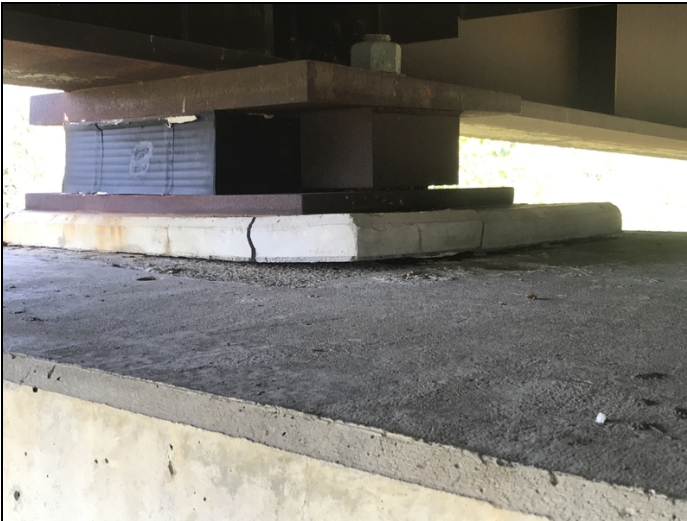
Southeast corner of the concrete pedestal for bearing # 1 is fractured in an area approximately 12" long x 8" wide with a portion of the fractured area that extends under the interior side of the masonry plate approximately 1-1/4".
