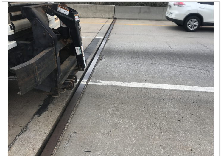
Abutment # 1 open expansion joint typical.
