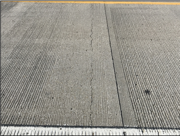
Span 3, left lane-Transverse crack.
