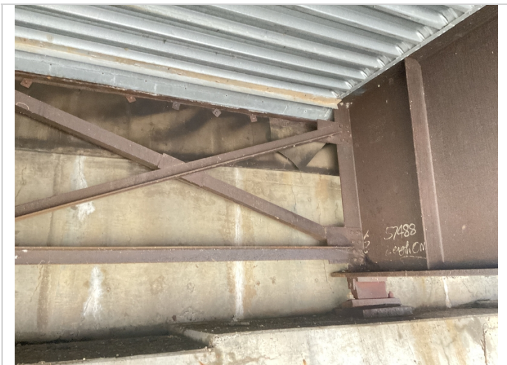
Abutment #1 trough tear adjacent to girder #2.
