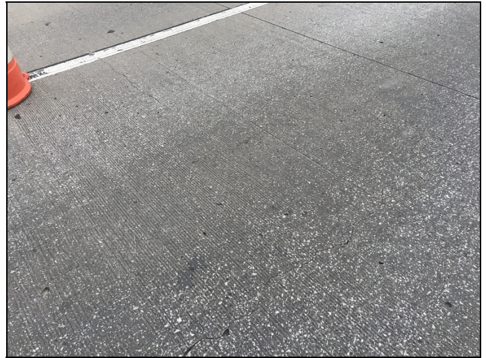
Span 1. Sealable longitudinal and transverse cracking in the driving surface of the deck.
