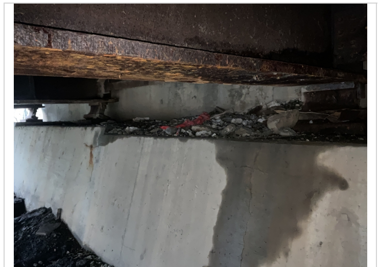
Abutment #1 bearings fully expanded.
