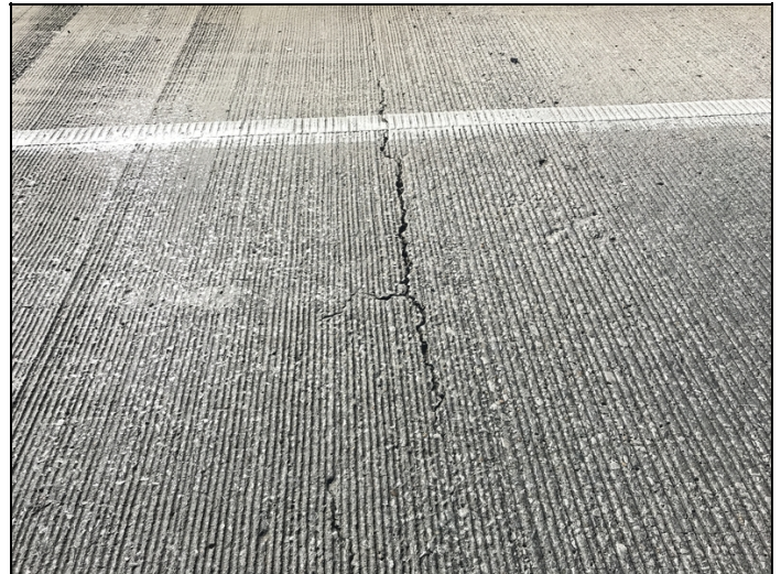
Span 3, left lane-Wide transverse cracking.
