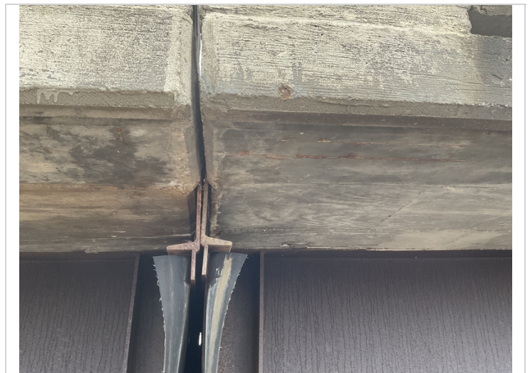
Bent #3 Lt expansion joint jammed together and touching.
