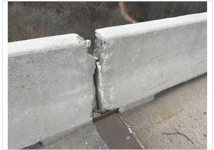
Spans 2 & 3. Spalling with exposed reinforcing in the left parapet over bent 3.
