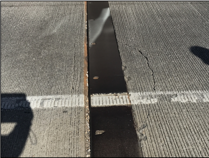
Bent 3, left lane-Wide cracking adjacent to sliding plate assembly.
