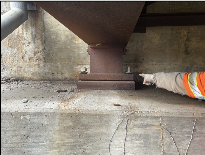
Abutment #2 girder #1 missing anchor bolt nut.
