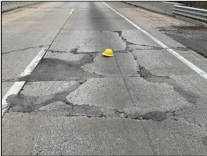
North approach roadway concrete breaking apart and settlement.
