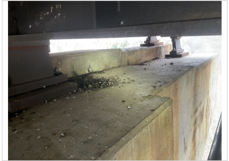
Span #3 bay #1 spalling with exposed reinforcing steel.
