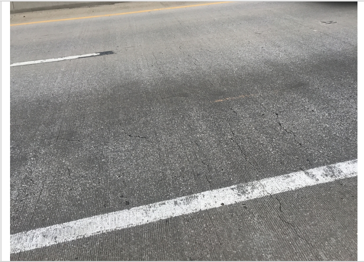
Span 1. Wide transverse and longitudinal cracks.
