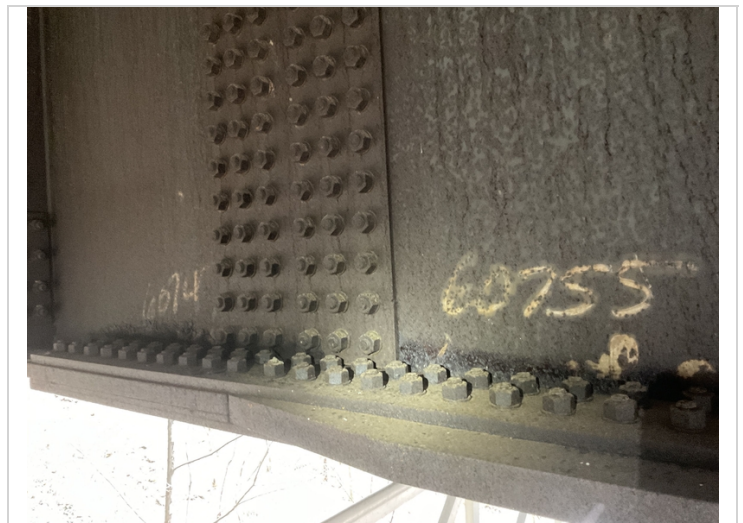
Span #1 girder #2 active corrosion with pack rust along the base of the web.
