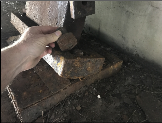
The bearings at abutment # 1 are fully expanded during this inspection with an approximate temperature of 80 degrees Fahrenheit. The left anchor bolts are sheared off at bearings # 2 and # 3 at abutment # 1. The remaining anchor bolts are leaning out of plumb.
