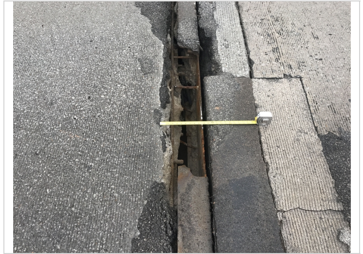
The expansion joint anchorage at bent 1 has fractured and is no longer supported by the deck for several feet.
