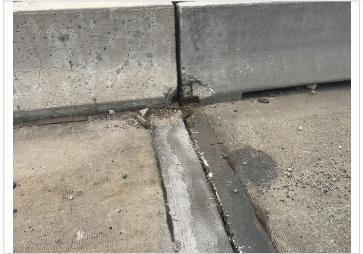
Spall with exposed reinforcing steel in the left parapet over bent 1.
