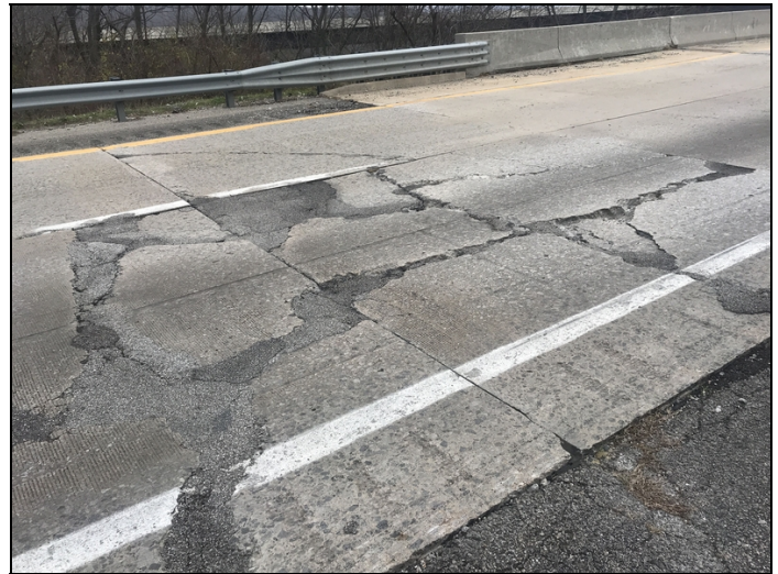
Approach roadway at the north end of structure is settling and breaking apart.
