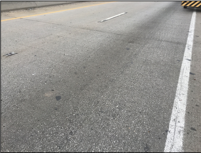
Sealable longitudinal cracking in the driving surface of span 5.
