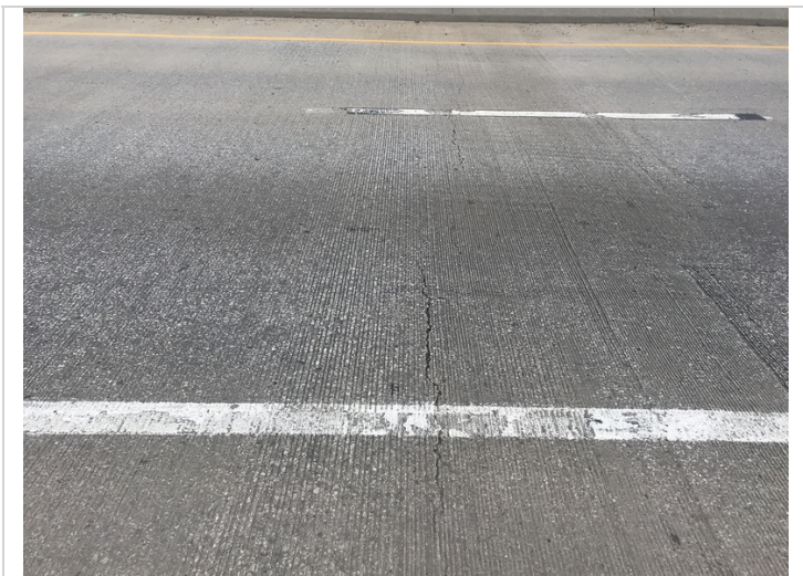
Wide transverse cracking in the driving surface of span 3.
