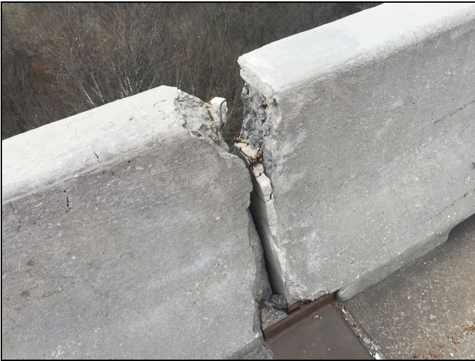
Spalls with exposed reinforcing steel in the left parapet over bent 3.
