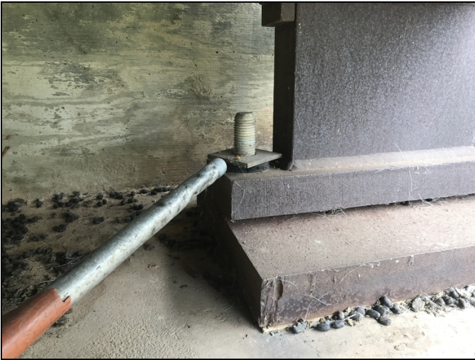
Bearings # 1, 3 and 4 at abutment # 2 are missing one anchor bolt nut.
