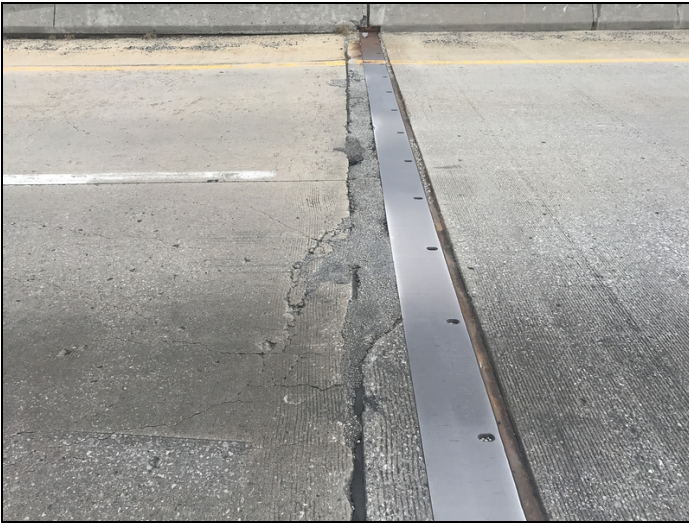
Spalls in the top of the backwall. Abutment 2.
