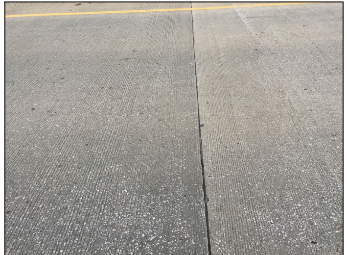
Saw joint sealant is deteriorated and missing in areas.
