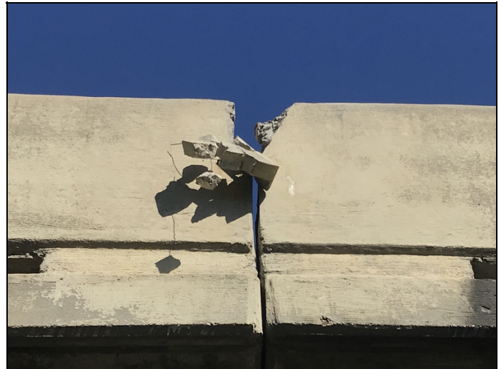
Left parapet over bent 3-Collision damage.
