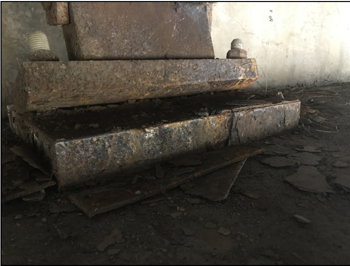
Abutment 1-Bearing 2-Corrosion.
