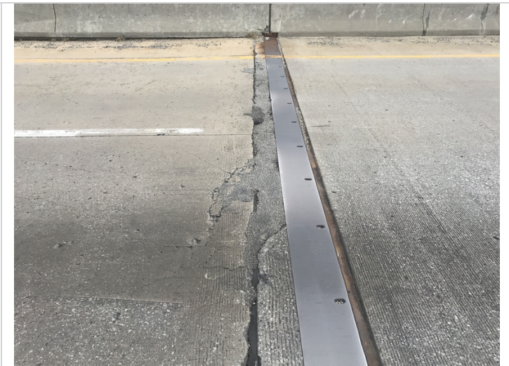
Abutment 2. Top of backwall. Spalling with temporary asphalt repairs.
