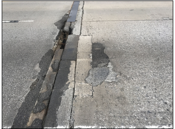
South approach slab. Deteriorating repairs.
