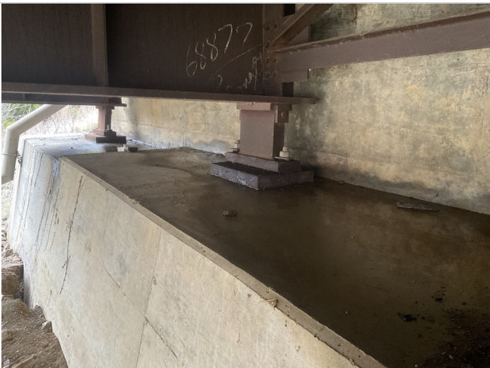
Abutment #2 active corrosion with pack rust.
