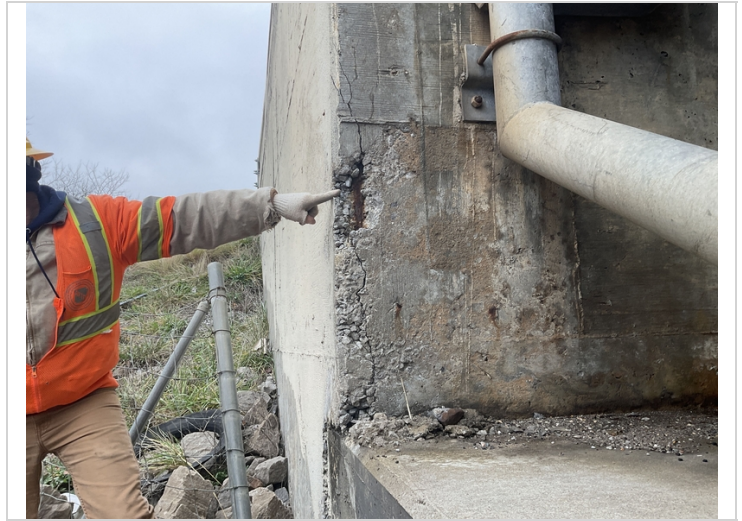
Abutment #2 Lt spalling with exposed reinforcing steel.
