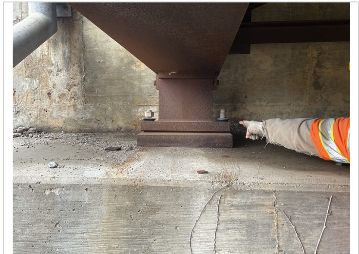
Abutment #2 girder #1 missing anchor bolt nut.
