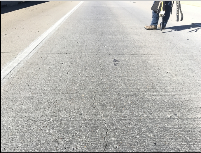
Span 4, left lane-Longitudinal cracking.
