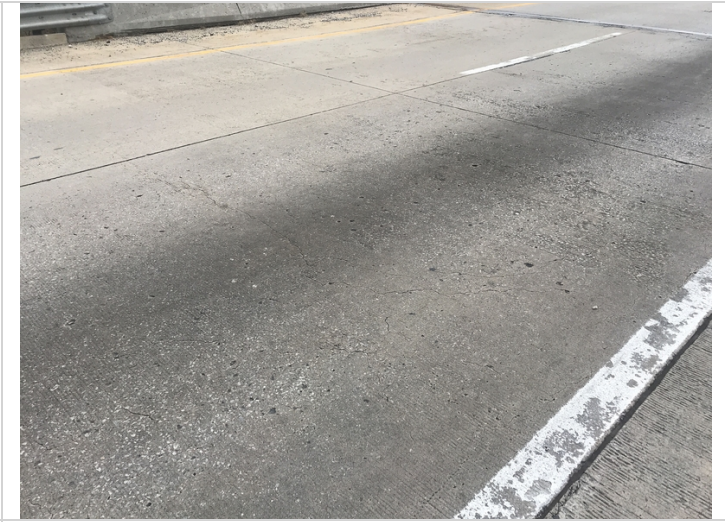
North approach slab. Sealable map cracking.
