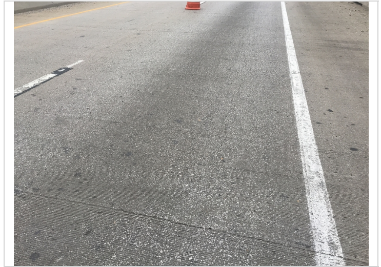
Sealable longitudinal cracking in driving surface of span 6.
