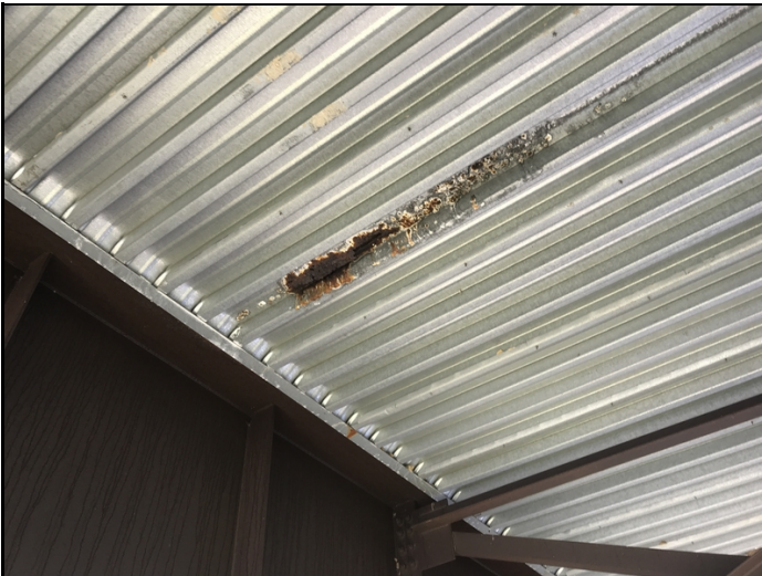
Span 2, bay 3-Corrosion in SIP forms.
