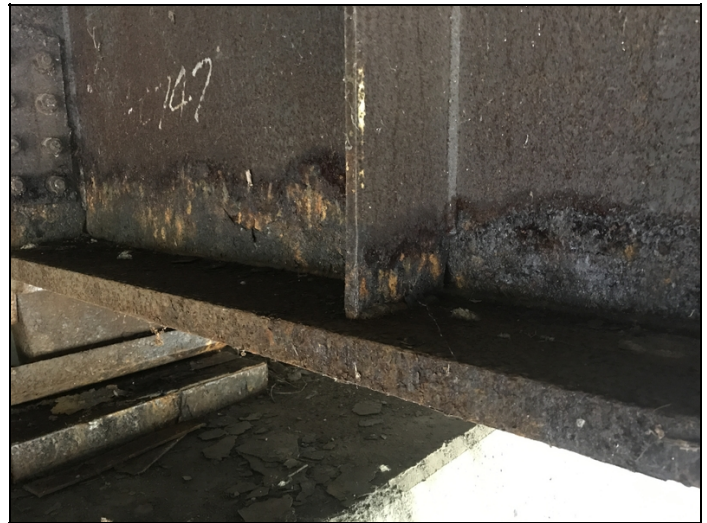
Span 1, girder # 2 at bent # 1-Corrosion with flaking rust.
