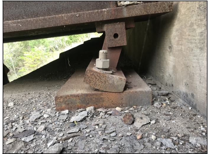
Abutment # 1, bearing 1-Fully expanded with sheared off bolt that attaches girder to bearing device.
