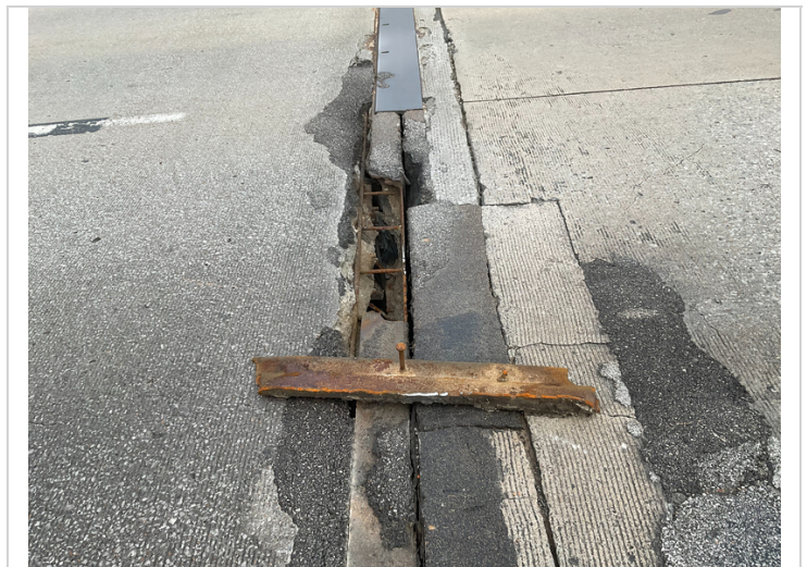
Abutment # 1 section of the road iron fractured.
