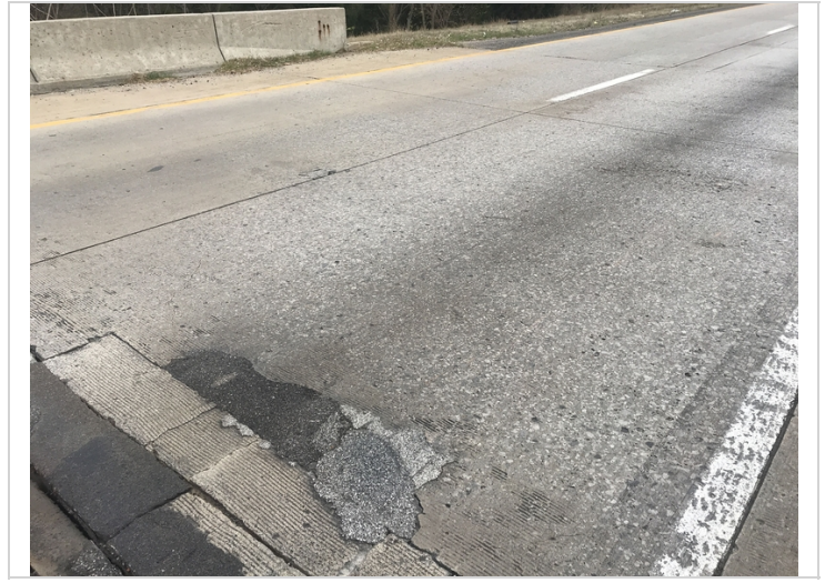
South approach slab. Temporary asphalt repairs.
