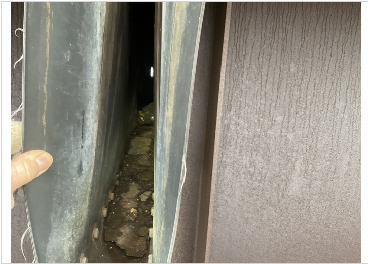
Bent #3 trough with debris accumulation.
