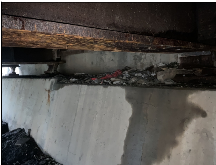
Abutment #1 bearings fully expanded.
