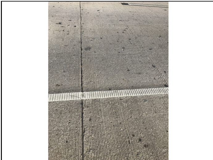
The sawn joint sealant is deteriorated and missing in locations.
