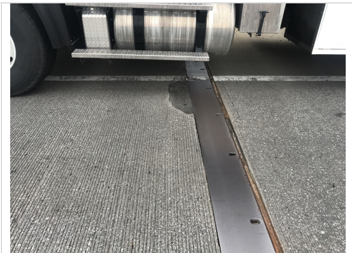
Bent 3. Circular cracking with spalling adjacent to the expansion joint assembly.
