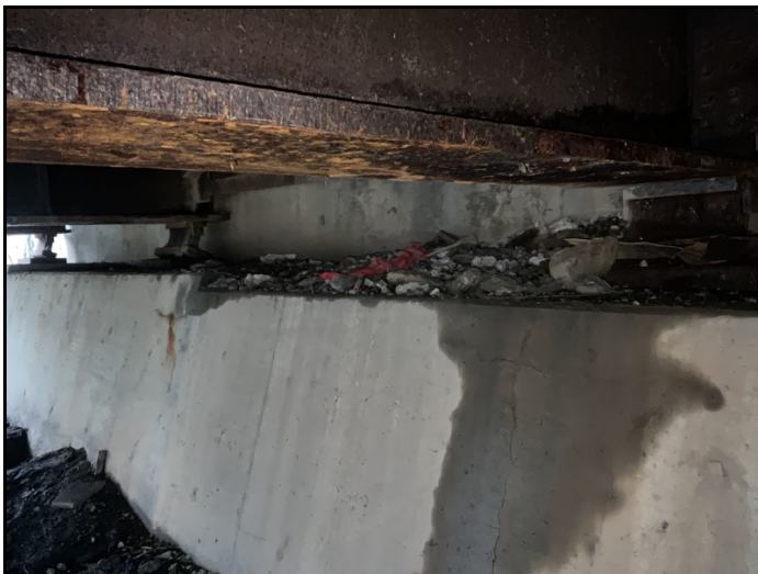
Abutment #1 bearings fully expanded.
