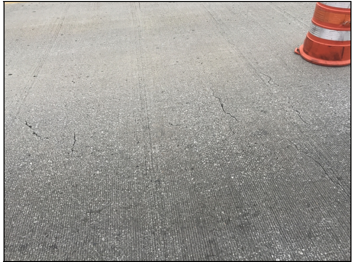
Sealable longitudinal and transverse cracks in the driving surface of the deck.
