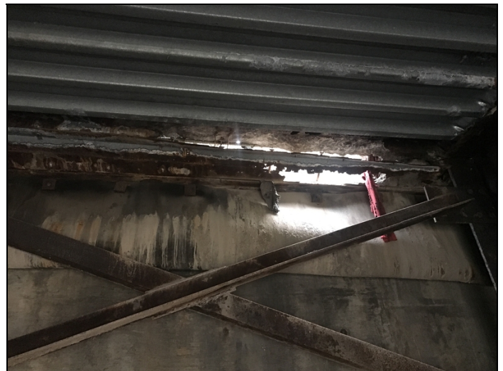
Undersurface of the full depth failure in span 1. Bay 2.
