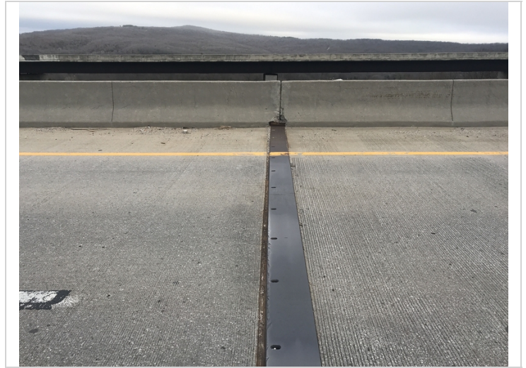
Bent 3. Right side of expansion joint is closed.
