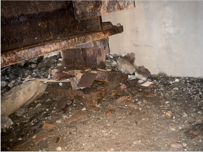
Abutment #1 bearing #2 missing anchor bolt.
