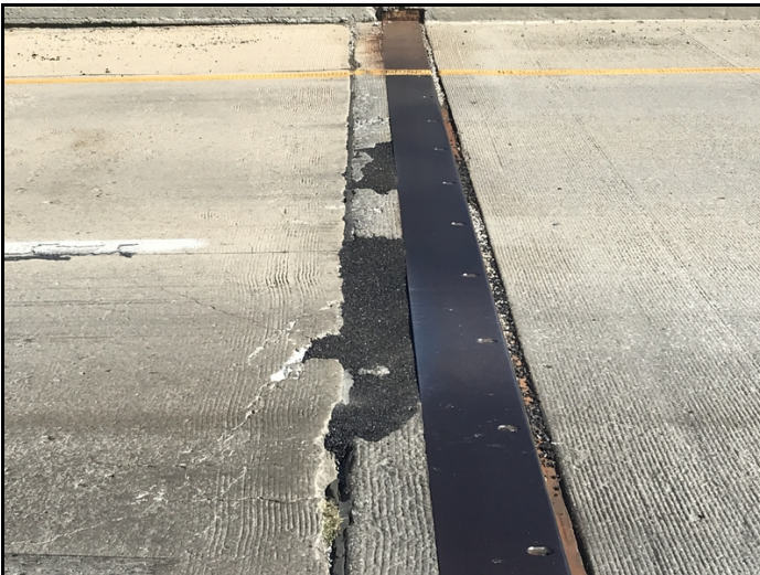
Abutment 2-Spalling in backwall with asphalt patches.
