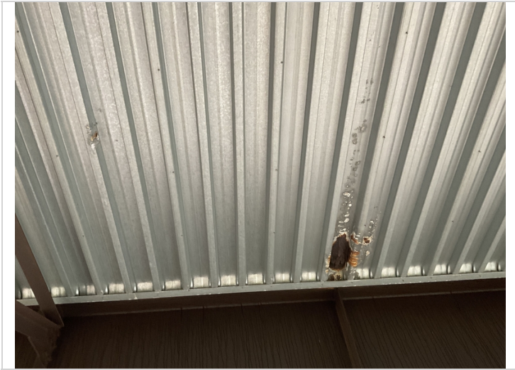
Span #3 bay #1 active corrosion in the stay in place forms.
