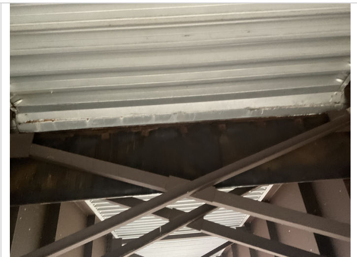
Bent #3 expansion dam with active corrosion and flaking rust.
