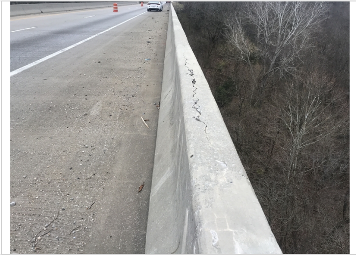
Wide longitudinal cracking in the top of the left parapet. Span 3.
