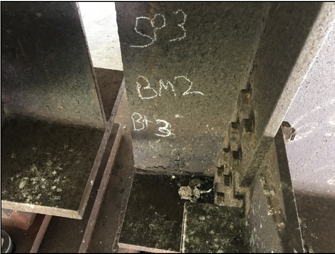
Span 2, Girder 2 at bent 3-Corrosion with flaking rust.
