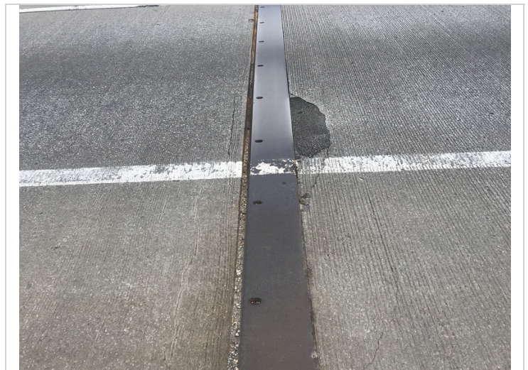
Expansion joint over Bent 3. Circular cracking adjacent to joint.
