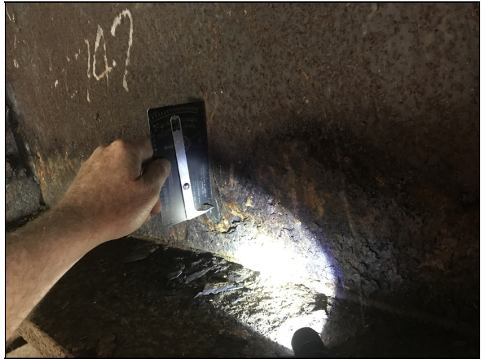
Span # 1, girder # 2 at bent # 1 has corrosion with flaking rust to base of web and bottom flange with up to approximately 1/16" section loss to base of web.
