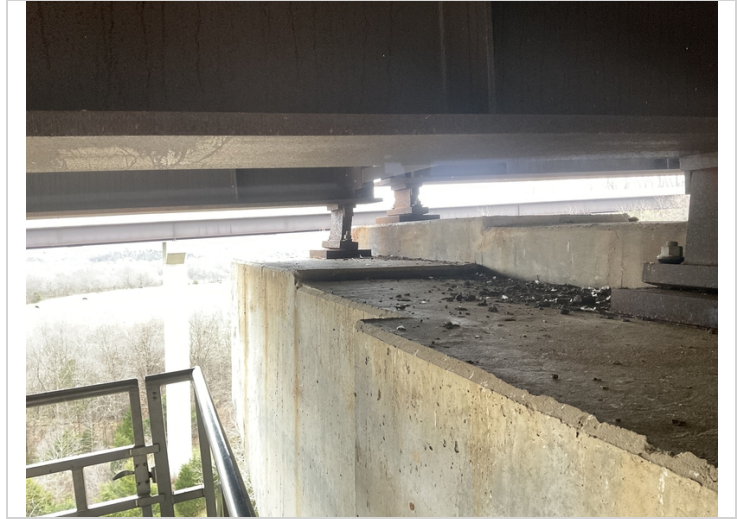
Bent #3 bearing #4 active corrosion with flaking rust.
