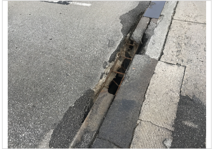
Spalling with exposed reinforcing steel adjacent to the south abutment.
