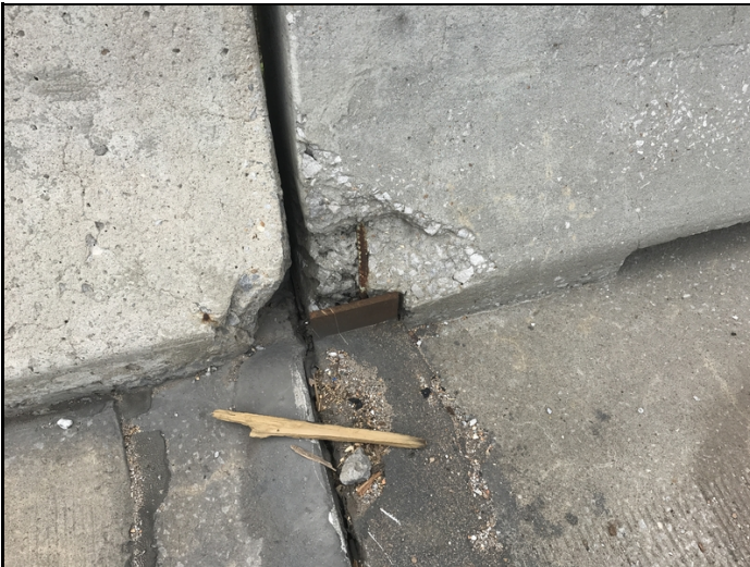
Left parapet at span 1-Spalling.
