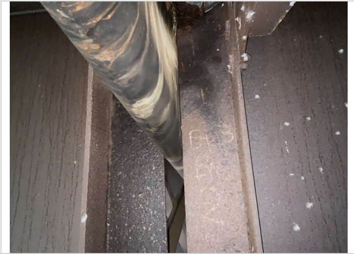
Bent #3 beam #2 active corrosion with flaking rust at the top of the web.
