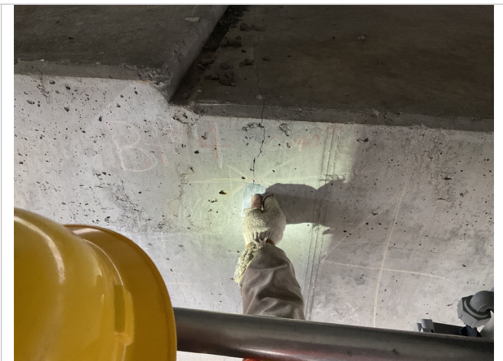
Bent #4 cap cracking.
