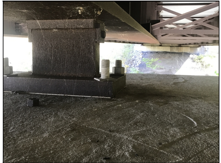
One anchor bolt nut is missing at bearings # 2 and # 3 over bent # 2.
