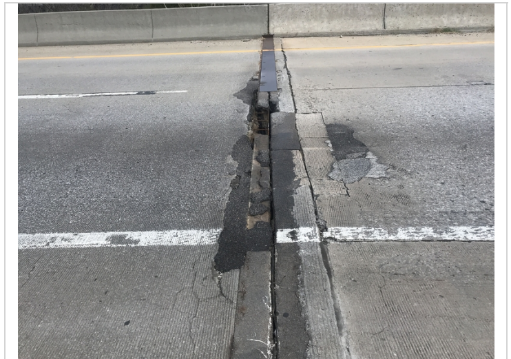
Bent 1. Top of backwall. Failing repairs.
