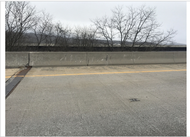
Right parapet. Map cracking with efflorescence adjacent to the north abutment.
