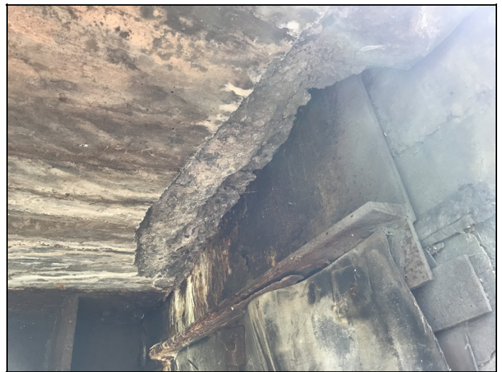
Span 1, left side at abutment 1-Spalling in deck undersurface.
