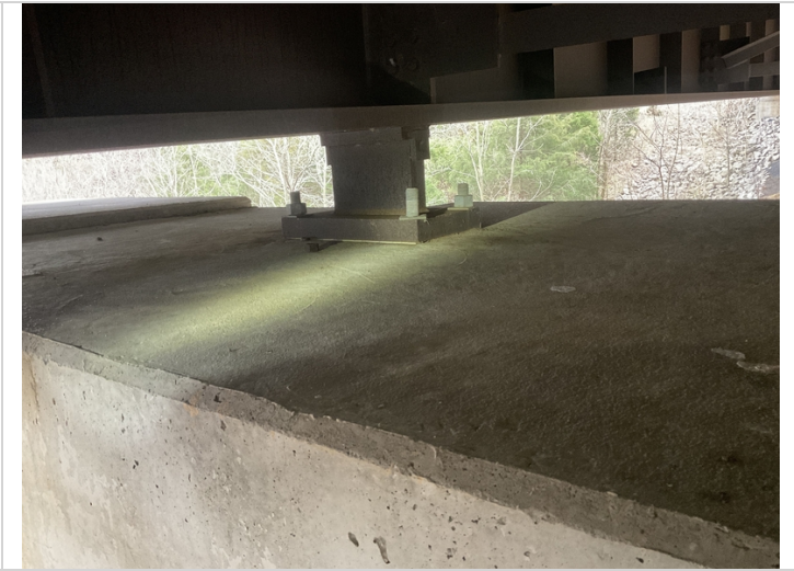
Bent #2 missing anchor bolt nuts.
