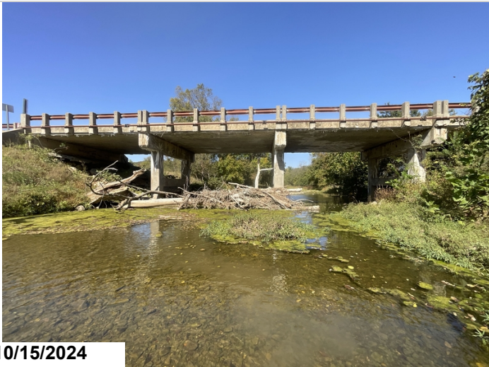
Drift accumulation under Spans 1, 2, & 3.
