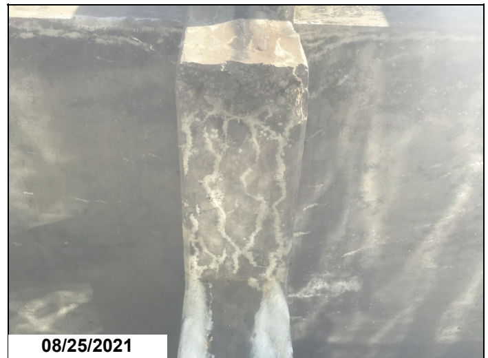
Bent 2 cap, right side-Spalling, concrete deterioration with mapcracking.
