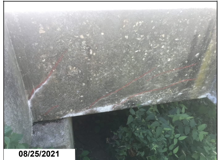
Span 4, left side-Shear type cracks.
