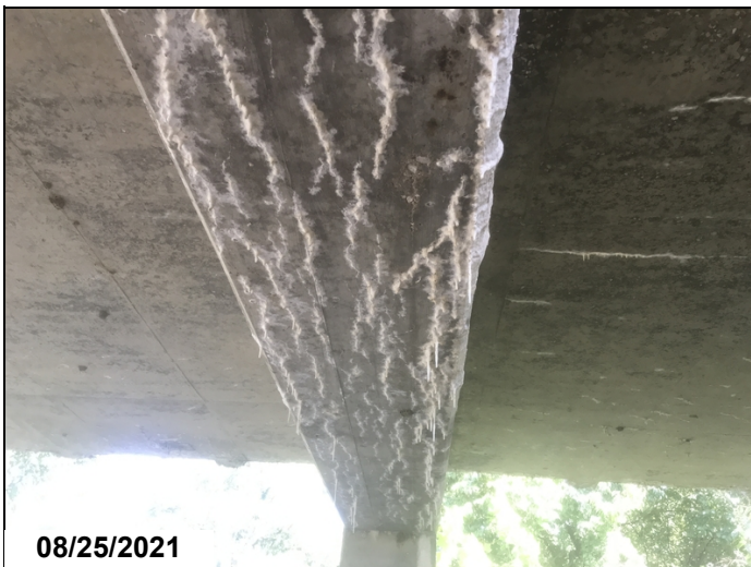
Undersurface of bent 4 cap-Concrete deterioration with heavy mapcracking.
