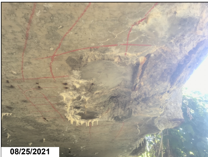
Span 4, right side-Spalling with exposed reinforcing steel and delaminated areas areas.
