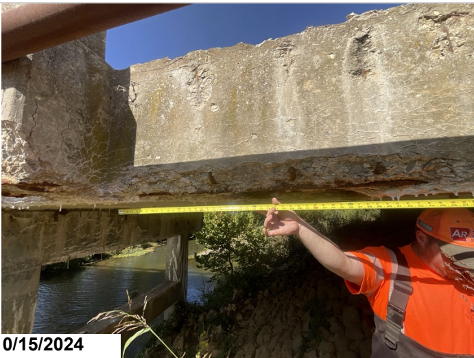
Span 4, Slab undersurface and exterior edge, Right side: 5' long spall with exposed reinforcing steel. 5SF CS3. Up to approximately 1/4" section loss
