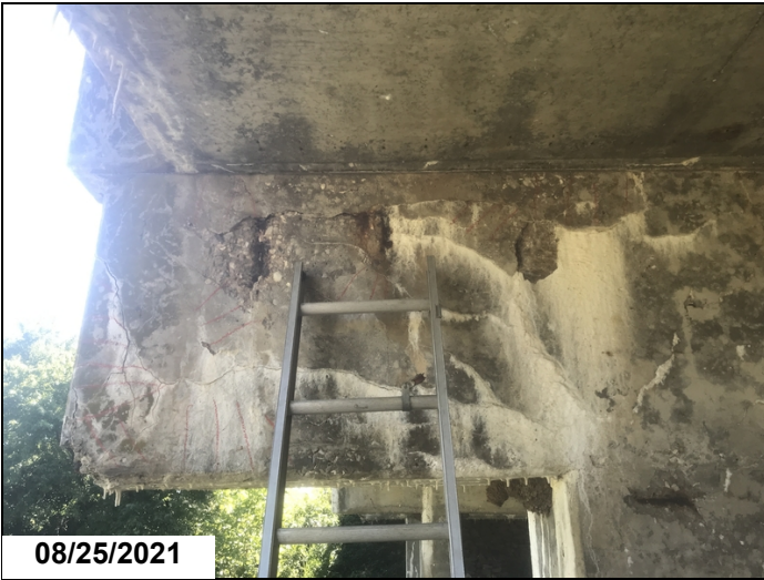
Bent 2 cap, left side-Delaminated areas in backface.
