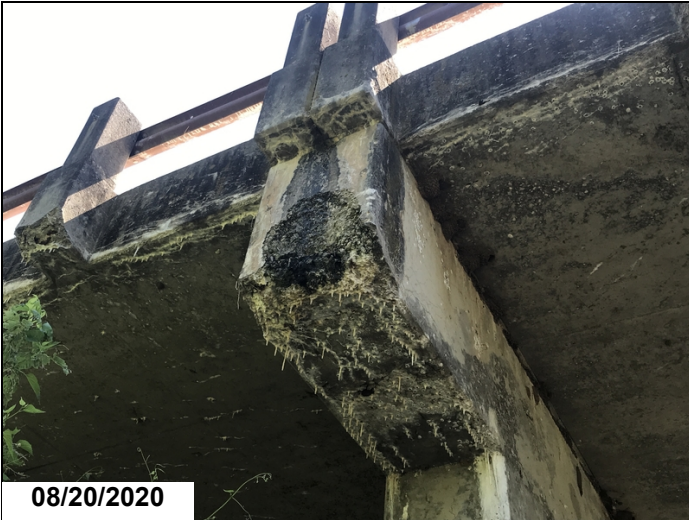
Bent 4 cap, left side-Concrete deterioration / spalling.
