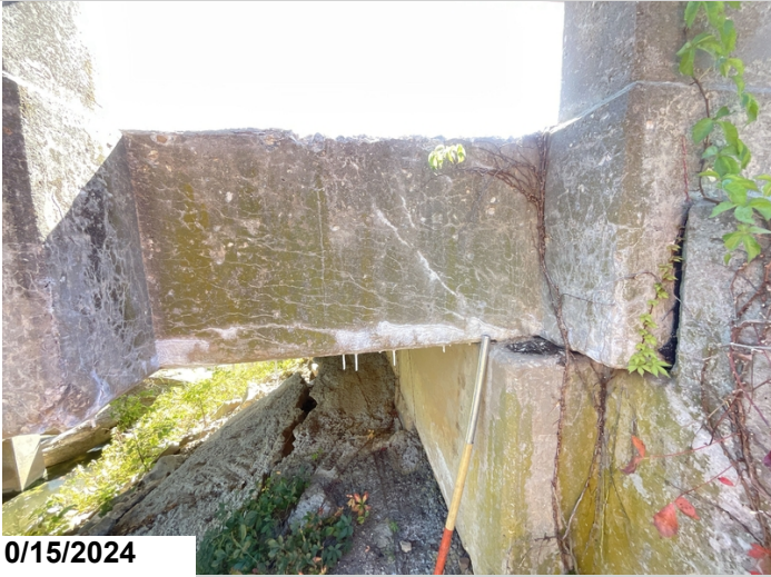
Span 1, Abutment 1, Left side: Diagonal cracks with efflorescence.
