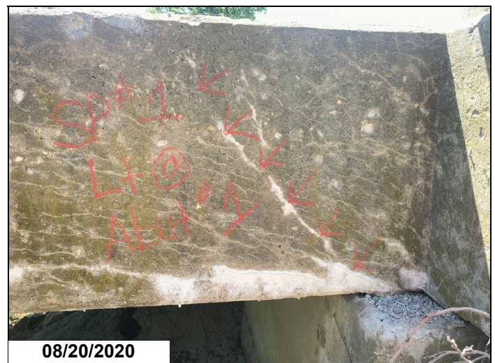
Span 1, right side-Shear crack.
