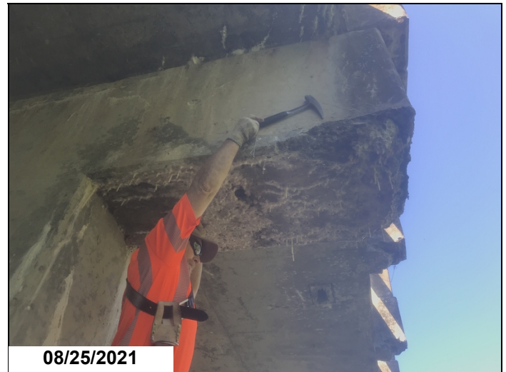
Bent 4 cap-Delaminated areas in left side of ahead face.
