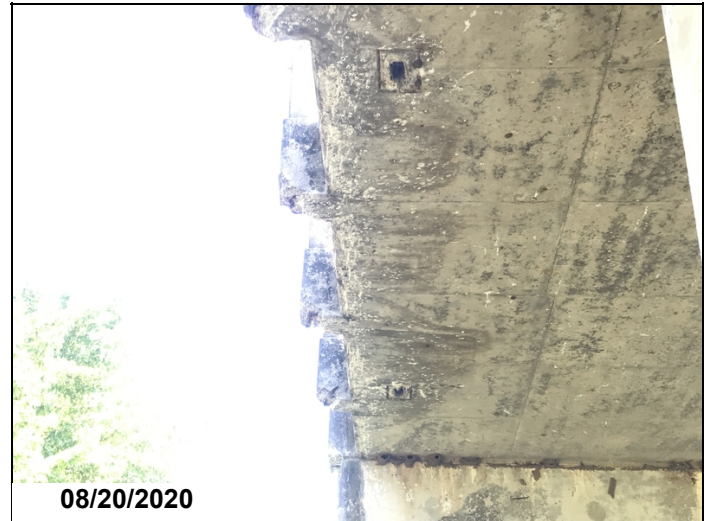
Span 2, left side-Spalling with exposed reinforcing steel to base of bridge railing posts.
