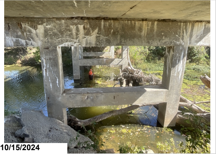
Probing substructure footings.
