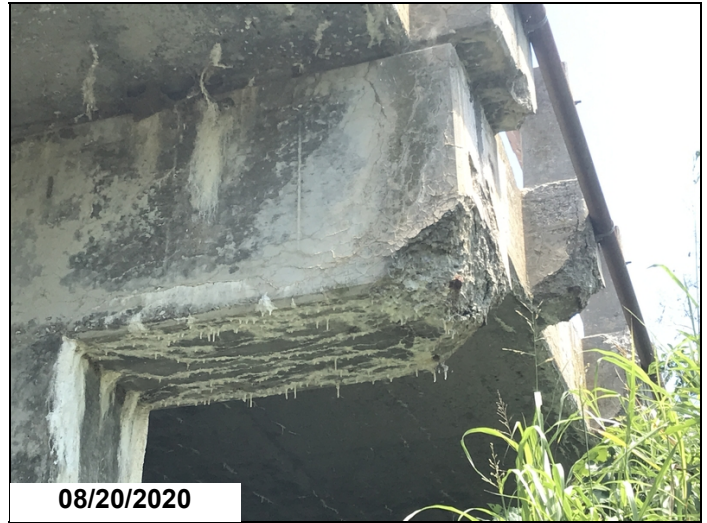
Bent 4 cap, right side-Concrete deterioration / spalling with exposed reinforcing steel.
