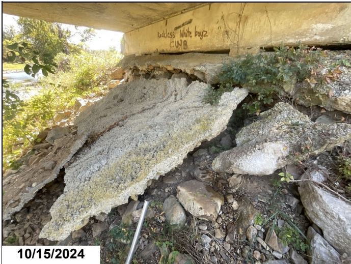
Abutment 1, settlement of grouted riprap.
