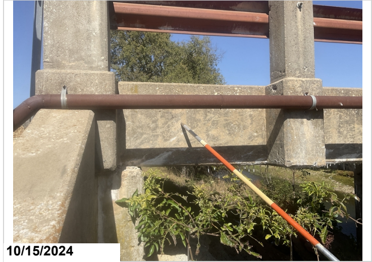
Span 1, Abutment 1, Right side: Diagonal cracks with efflorescence.
