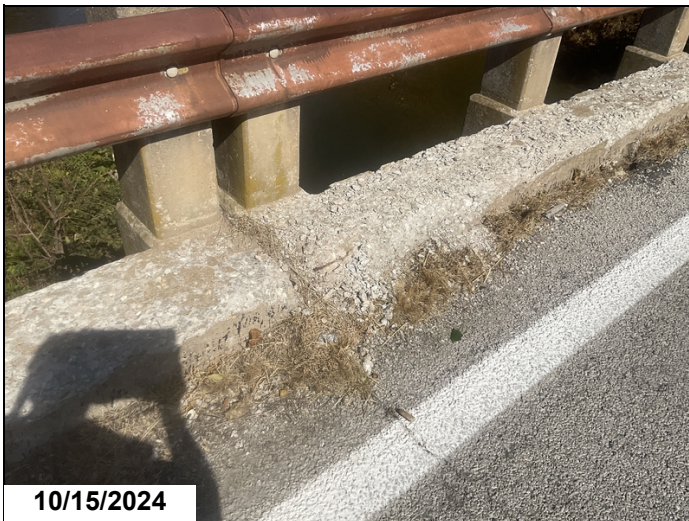
Span 1 curb, Left side: Rotten deteriorated concrete.
