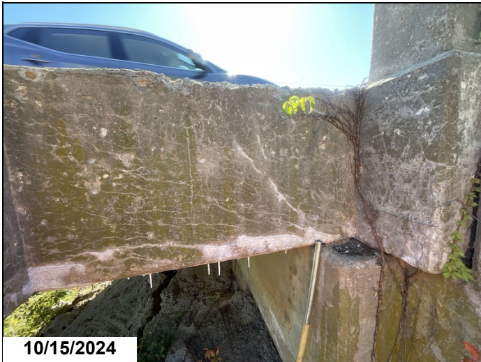
Span 1, Abutment 1, Left side: Shear type crack.
