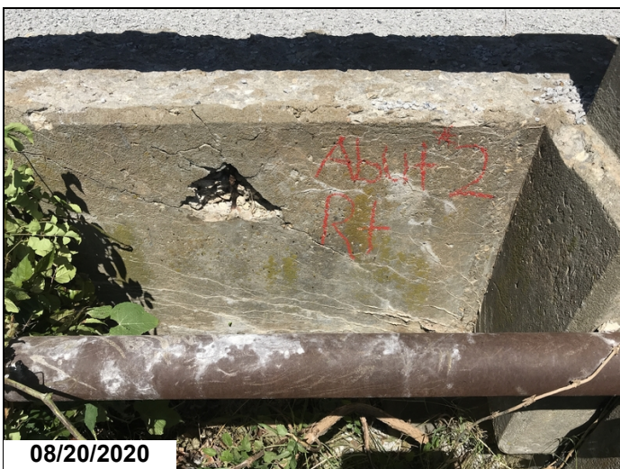
Abutment 2, right side-Shear type crack.
