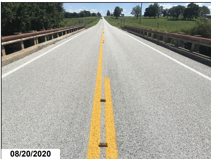
New chip and seal wearing surface.
