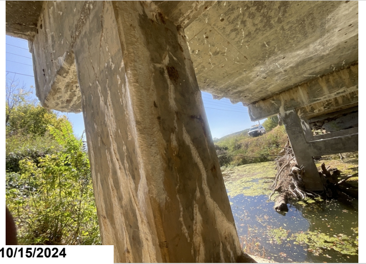
Bent 4, Right column. Spall with exposed reinforcing steel. 1EA CS3
