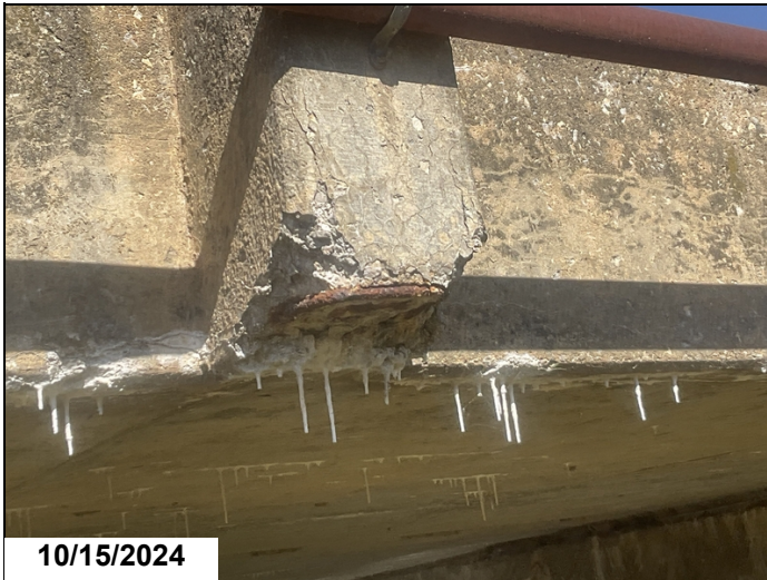
Span 1, Right bridge rail post: Soft deteriorated concrete with exposed reinforcing steel.
