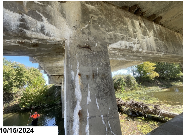
Bent 2, Left column, Back face, spall with exposed reinforcing steel.
