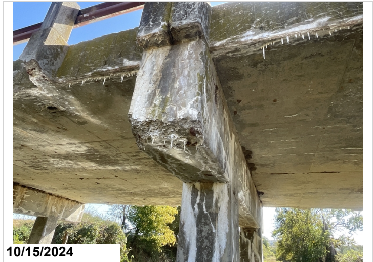
Left end of Bent 2 cap. Concrete deterioration with exposed reinforcing steel.
