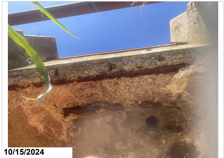
Span 4, undersurface of the slab, right side exposed reinforcing steel.
