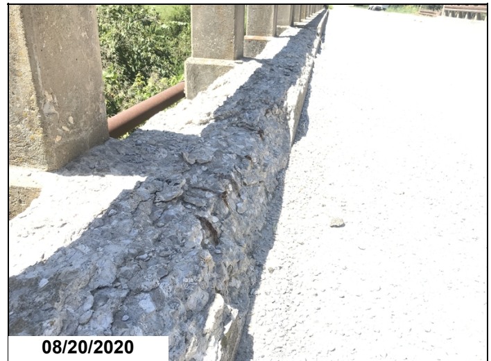
Span 4, right curb-Concrete deterioration.
