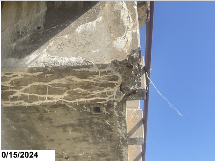
Bent 2 cap, Right end concrete deterioration with exposed reinforcing steel.
