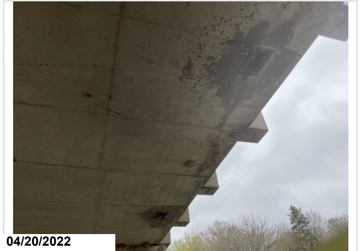
Span #5 Lt spalling with exposed reinforcing steel at the deck drains.
