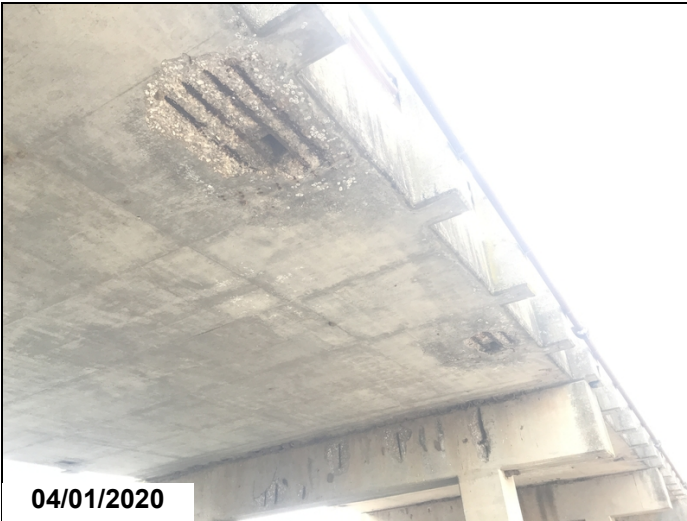
Span 4, right side-Spalling adjacent to deck drains.
