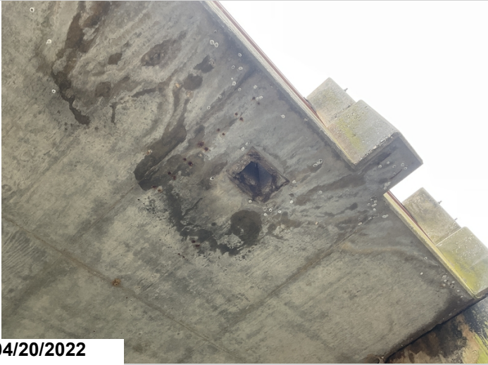
Span #4 Lt exposed reinforcing steel in the deck drain.
