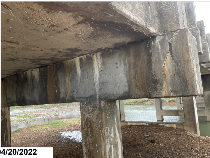
Bent #7 Lt vertical cracking in the Lt end of the cap.
