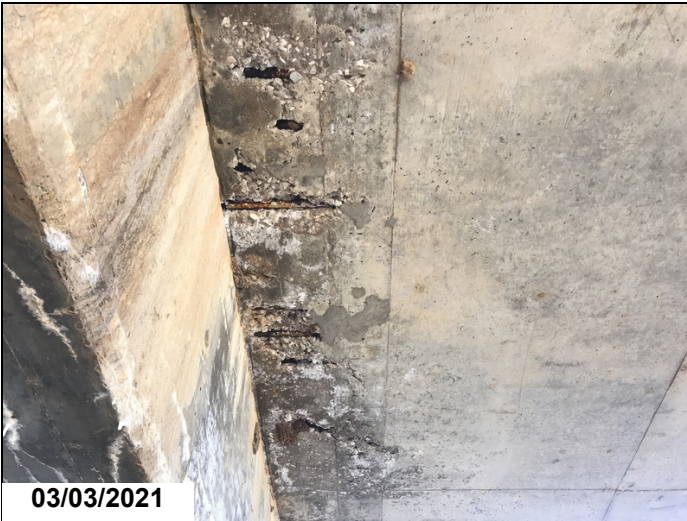
Span 6, at bent 7-Spalling / delaminated areas with exposed reinforcing steel.
