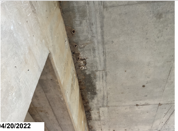
Span #5 bent #6 spalling with exposed reinforcing steel at the cap juncture.
