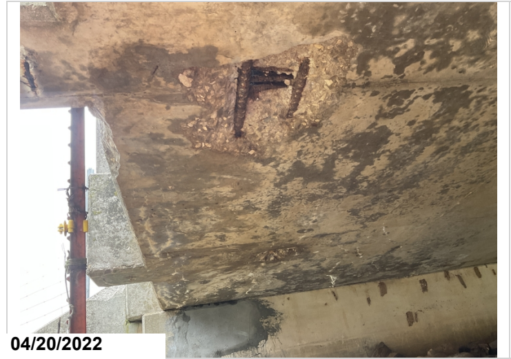
Span #7 Lt spalling with exposed reinforcing steel.
