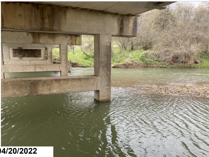
Bent #5 column #1 ahead face spalling with exposed reinforcing steel.
