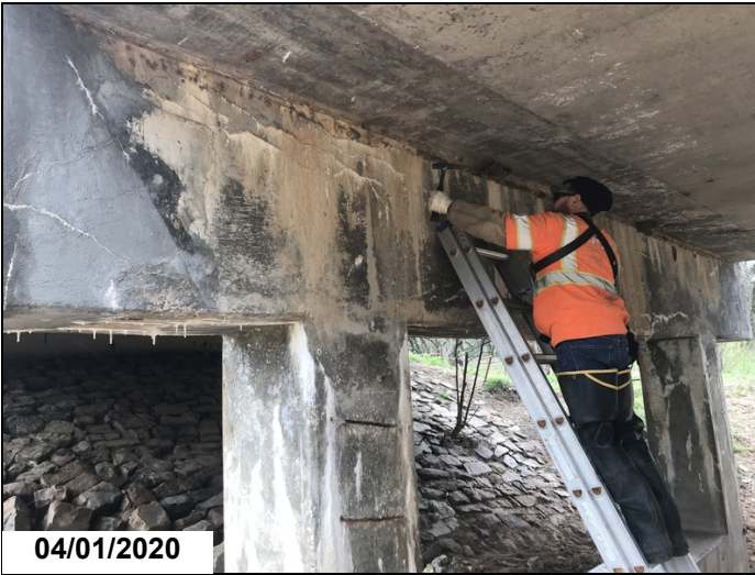
Bent # 7-Mapcracking / chloride contamination.
