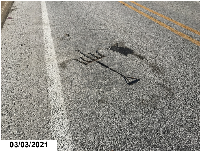
Span 5, right lane has a 12' x 6' delaminated area.
