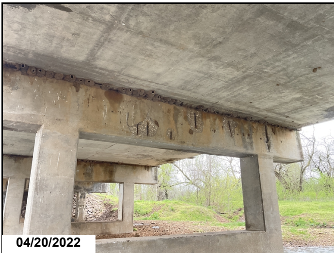
Bent #5 backface spalling with exposed reinforcing steel.
