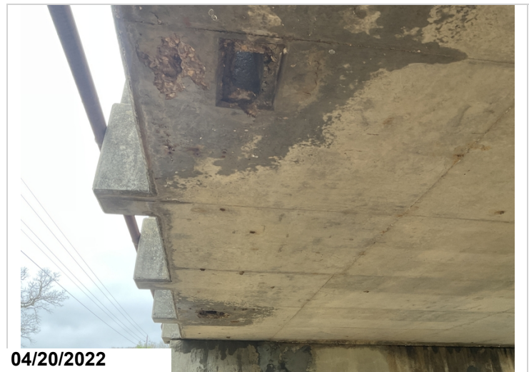
Span #6 Rt spalling with exposed reinforcing steel at the deck drains.
