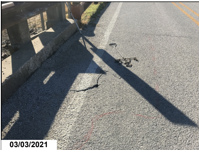
Span # 7, left lane at abutment # 2 has a 12' x 6' delaminated area with a portion failing repair beginning to spall.
