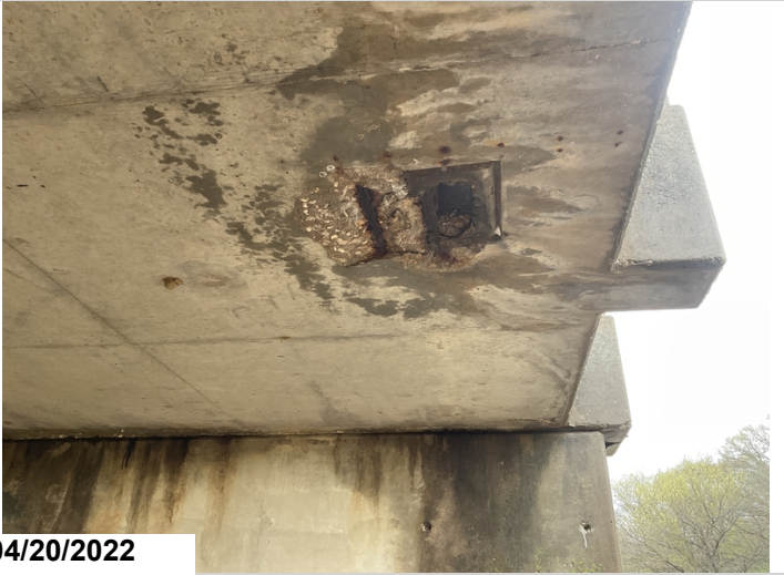
Span #6 Lt spalling with exposed reinforcing steel at the deck drain.
