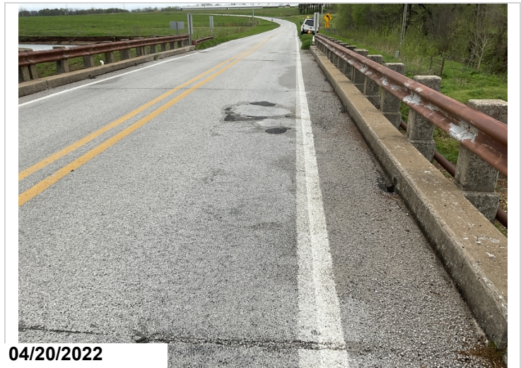
Span # 5, 6 & 7 Rt wearing surface delamination.
