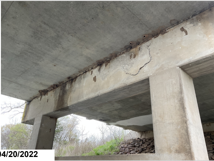
Bent #2 ahead face concrete delamination.
