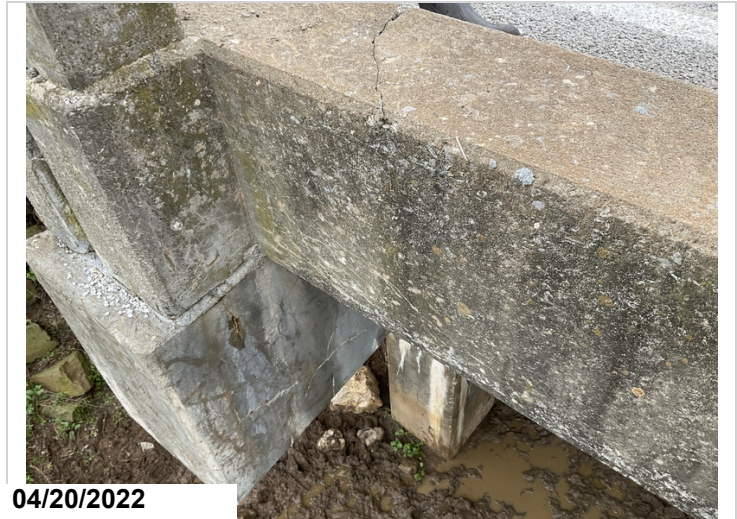
Span #6 Lt at Bent #7 shear type crack exterior edge of the slab.
