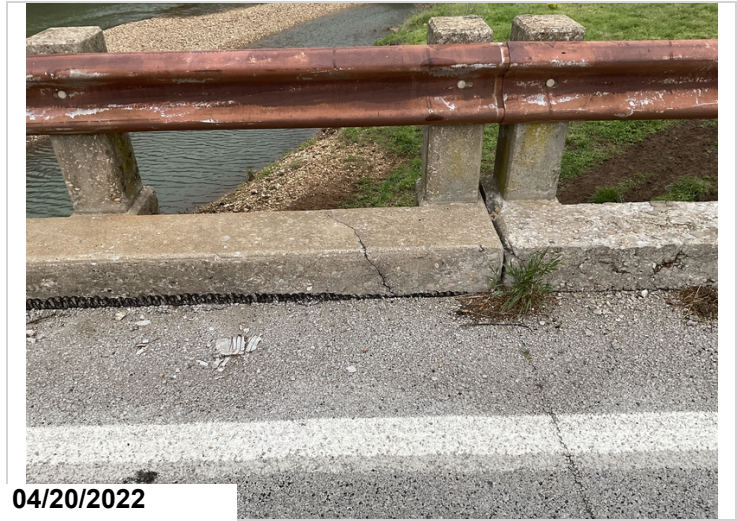
Span #6 Lt at Bent #7 shear type crack.
