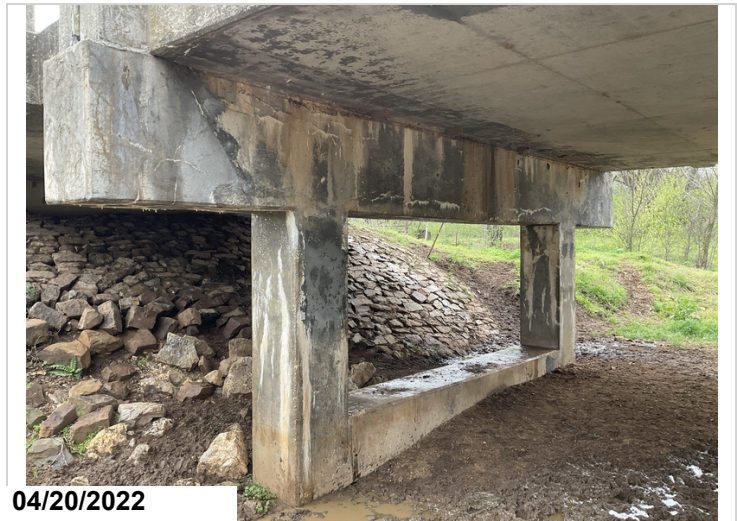
Bent #7 backface map cracking with efflorescence buildup.
