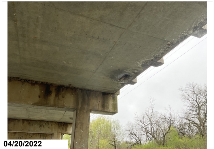
Span #2 Rt spalling with exposed reinforcing steel.
