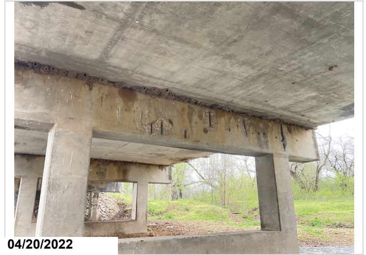
Bent #5 backface spalling with exposed reinforcing steel.
