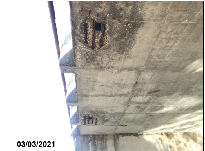
Span 4, right side-Spalling / delaminated areas with exposed reinforcing steel at deck drains.
