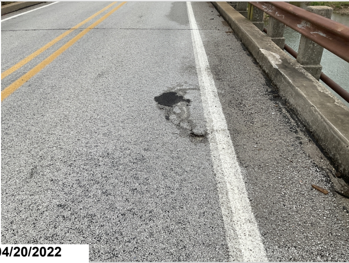
Span #1 Rt delamination of the wearing surface.
