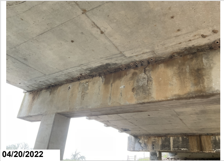
Bent #6 concrete delaminations and spalling with exposed reinforcing steel.
