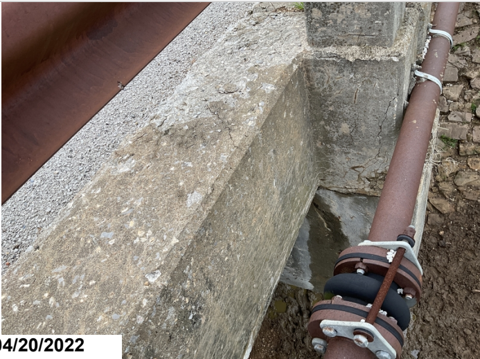
Span #6 Rt at Bent #7 shear type crack exterior edge of the slab.
