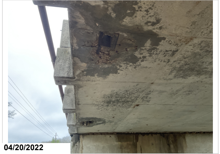
Span #5 Rt spalling with exposed reinforcing steel at the deck drains.
