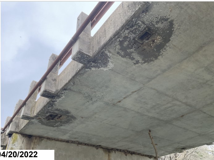
Span #3 Rt concrete spalling with exposed reinforcing steel.
