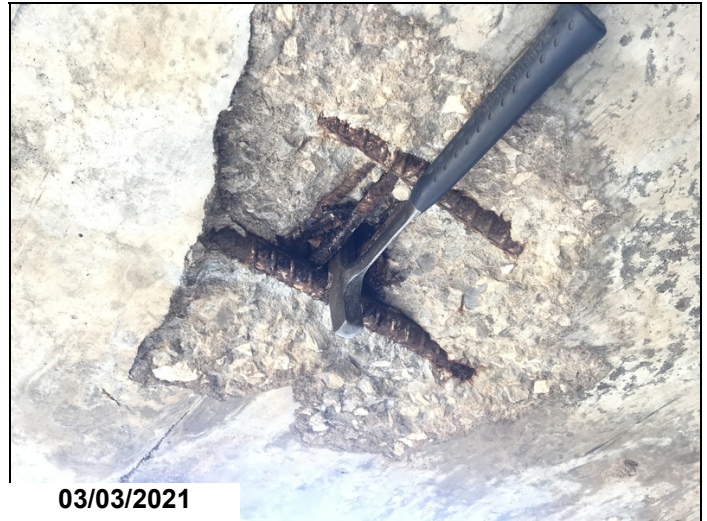
Span # 7, left side has a spall approximately 14" x 14" with two mats of exposed reinforcing steel and a 4" diameter area with up to approximately 5" of section loss that appears to be a possible full depth failure due to recent deck repairs. Photo 1.
