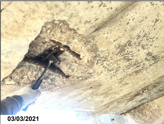
Span # 7, left side has a spall approximately 14" x 14" with two mats of exposed reinforcing steel and a 4" diameter area with up to approximately 5" of section loss that appears to be a possible full depth failure due to recent deck repairs. Photo 2.
