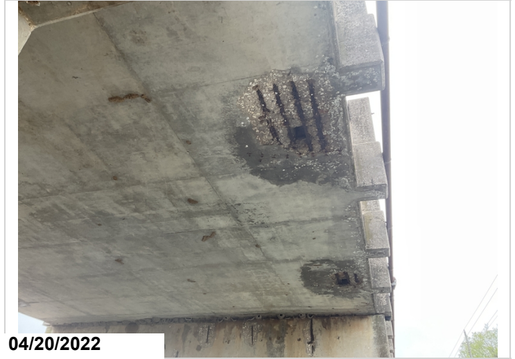
Span #4 Rt spalling with exposed reinforcing steel.
