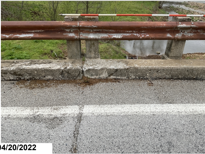
Span #6 Rt at Bent #7 shear type crack.
