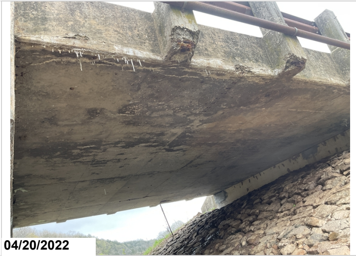
Span #7 has map cracking and efflorescence buildup visible from the undersurface of the slab.
