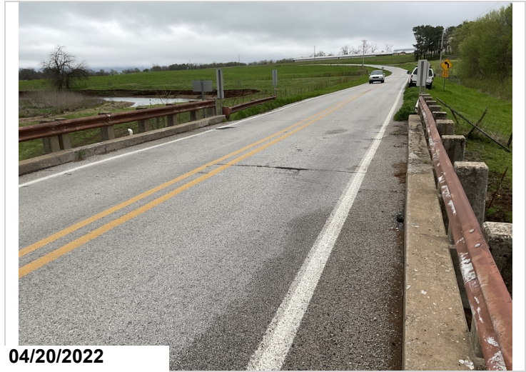
Span #7 curbs with concrete deterioration with section loss.
