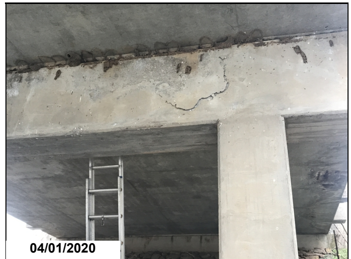
Bent 2 cap, ahead face on left side-Delaminated area.
