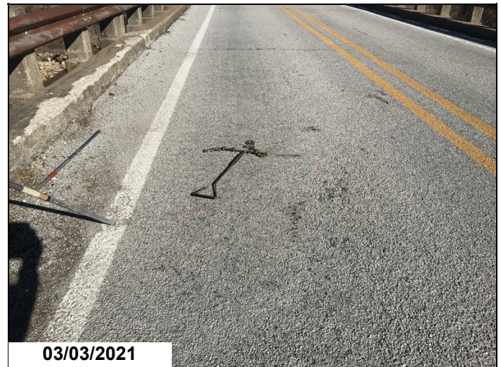
Span # 7, right lane near abutment # 2 has a delaminated area approximately 25' x 6' where previous repairs appear to have failed.
