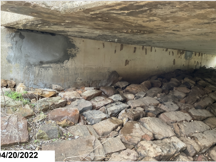
Abutment #2 grouted repairs.
