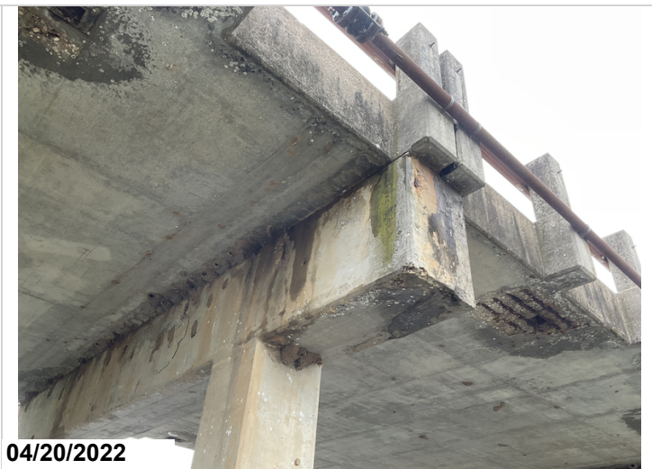
Bent #3 Rt cap with shallow spalling with exposed reinforcing steel.
