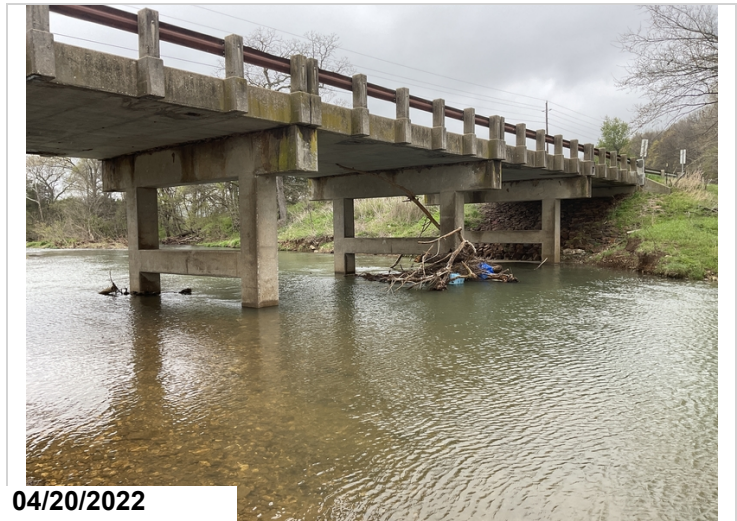
Bent # 2, 3 & 4 drift accumulation.
