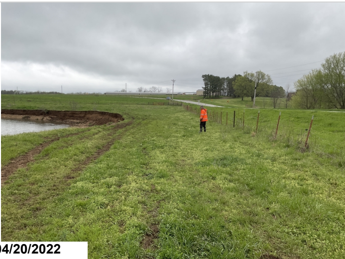
Channel migration has eroded the embankment and is currently 30' from the right of way fence.
