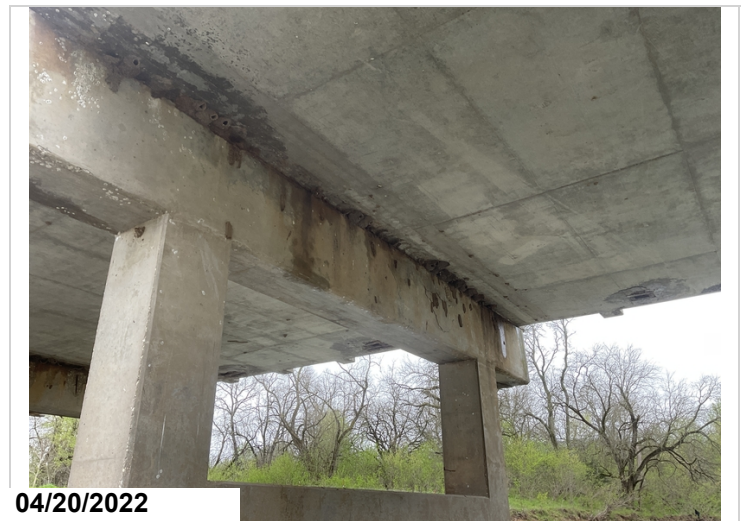
Bent #4 backface large concrete delamination.
