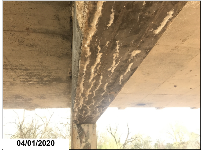
Bent 7 cap undersurface-Mapcracking with delaminated areas.
