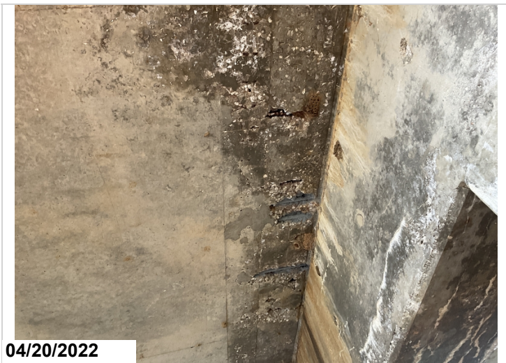
Span #6 adjacent to Bent #7 concrete deterioration with exposed reinforcing steel.
