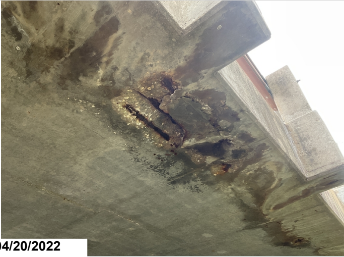
Span #1 Lt concrete spalling with exposed reinforcing steel at the deck drain.
