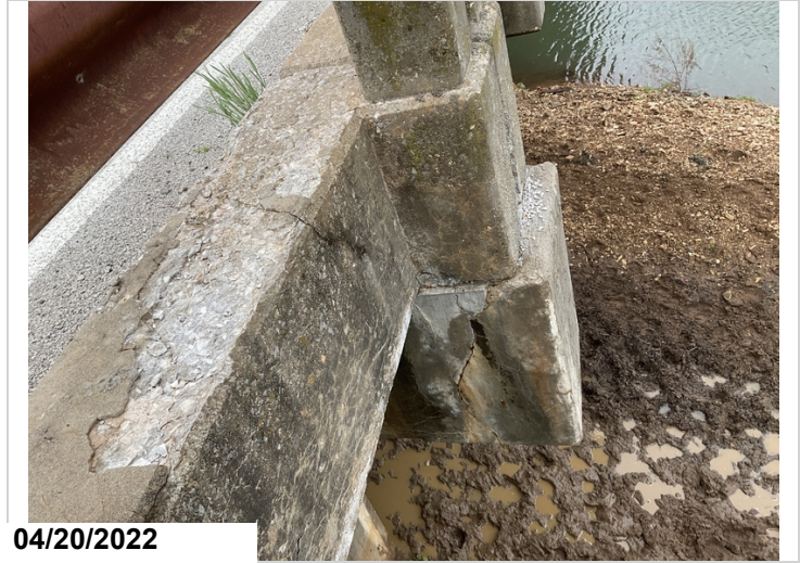
Span #7 Lt at Bent #7 shear type crack exterior edge of the slab.
