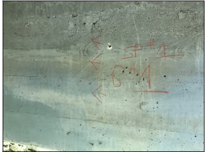
Span # 1, girder # 1-Hairline vertical cracking.
