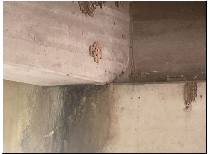
There is a moderate width diagonal crack (Not shear) in the end of girders # 1 and 2 of span # 1 over bent # 2. Photo taken of Span # 1, Girder # 1 at Bent # 2.
