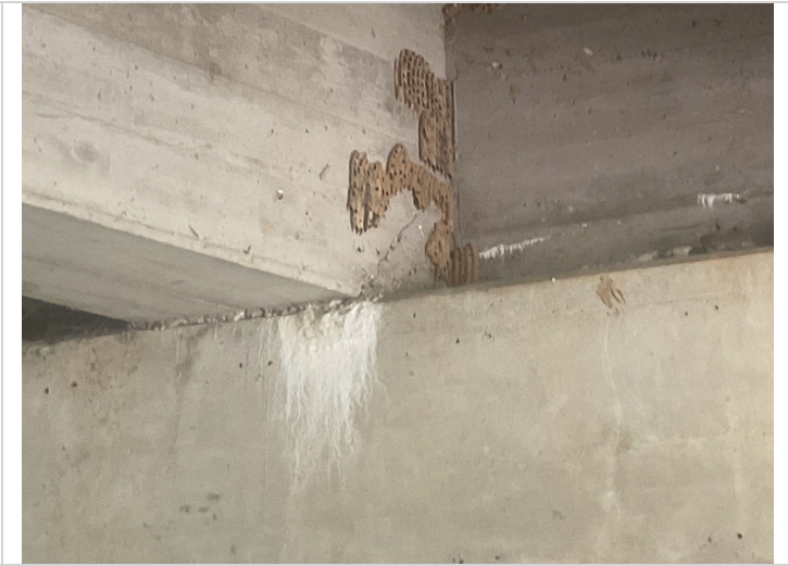
There is a moderate width diagonal crack in the end of Girders # 1 and 2 in Span # 1 at Bent # 2. Diagonal cracks are located at the base of girders and are approximately 14" long. (Not shear type cracks). Photo taken at Girder # 2.
