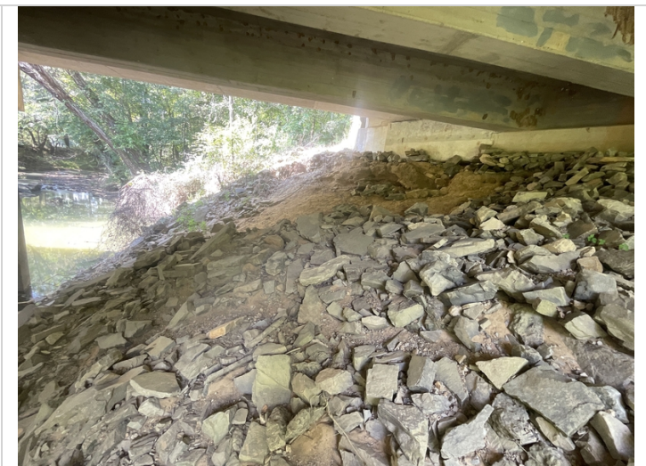
Abutment # 1 has riprap displacement with embankment erosion at the inlet end of the abutment.
