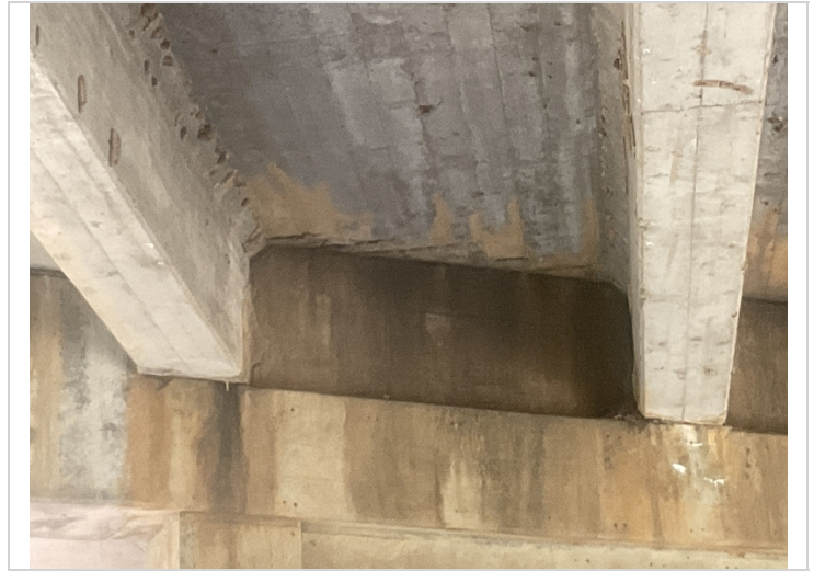
Span # 2. Bay # 2 deck soffit. Spalls with exposed reinforcing steel.
