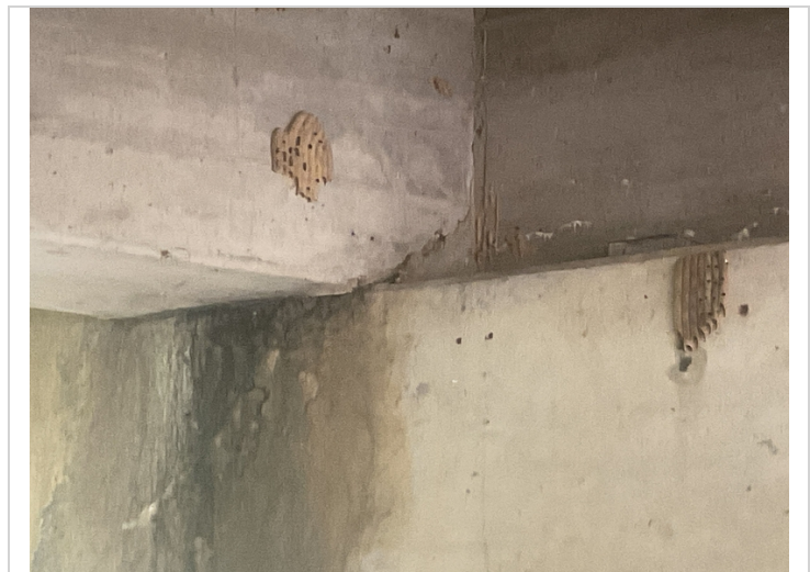
There is a moderate width diagonal crack in the end of Girders # 1 and 2 in Span # 1 at Bent # 2. Diagonal cracks are located at the base of girders and are approximately 14" long. (Not shear type cracks). Photo taken at Girder # 1.
