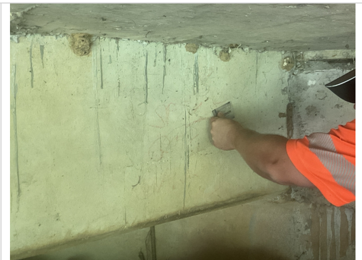
The exterior edge of Girder # 1 has a shear type crack at Abutment # 1 that measures 0.008" during this inspection.
