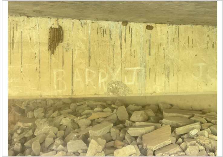
Span # 1, Girder # 1 has a shallow 6" spall with no exposed reinforcing steel in the base of girder located approximately 10' from Abutment # 1.
