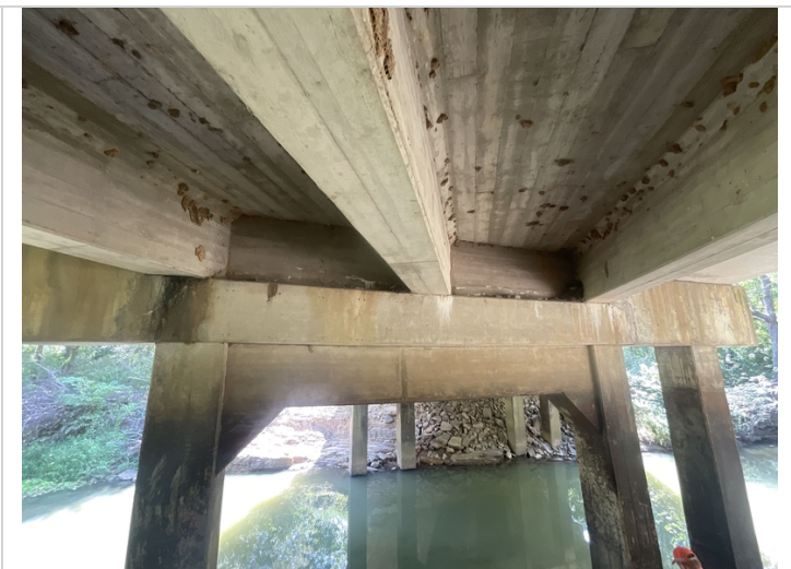
There is map cracking with efflorescence in the end diaphragms between the girders over Bent # 2.
