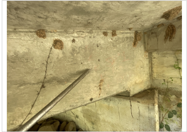
The Left edge of the slab at Abutment # 1 has a hairline shear type crack that measures 0.010" during this inspection.
