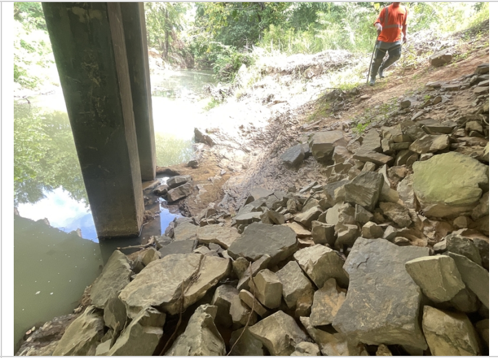
Shale is exposed along the East embankment.
