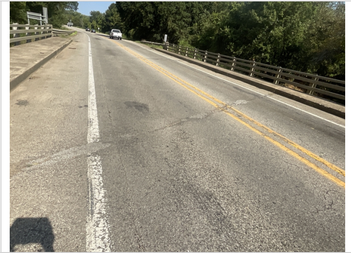
Asphalt has numerous patches over the expansion joint. Photo of Bent # 3 expansion joint.
