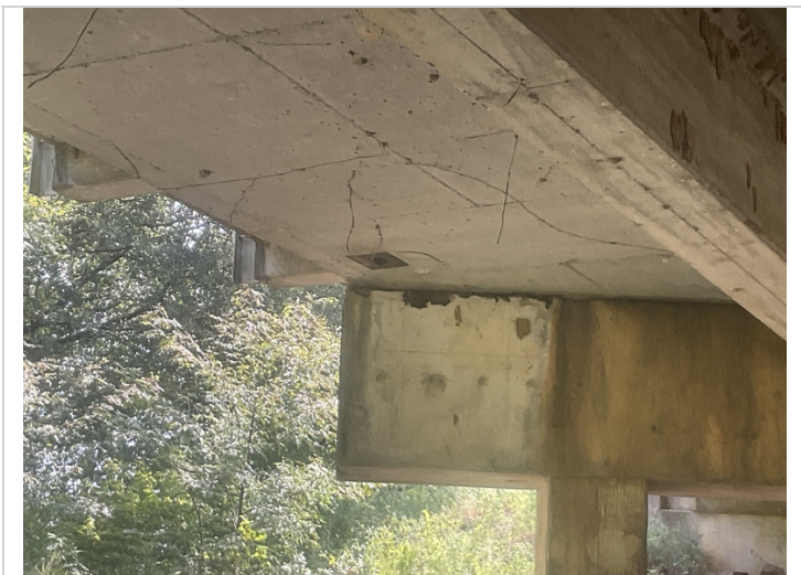
Span # 2 deck soffit: Photo of an 18" delaminated area adjacent to the Span # 2 deck drain located near the Left end of Bent # 3 cap.
