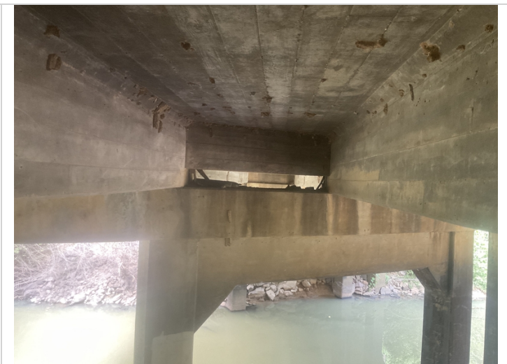
Debris accumulation on Bent # 3 cap.
