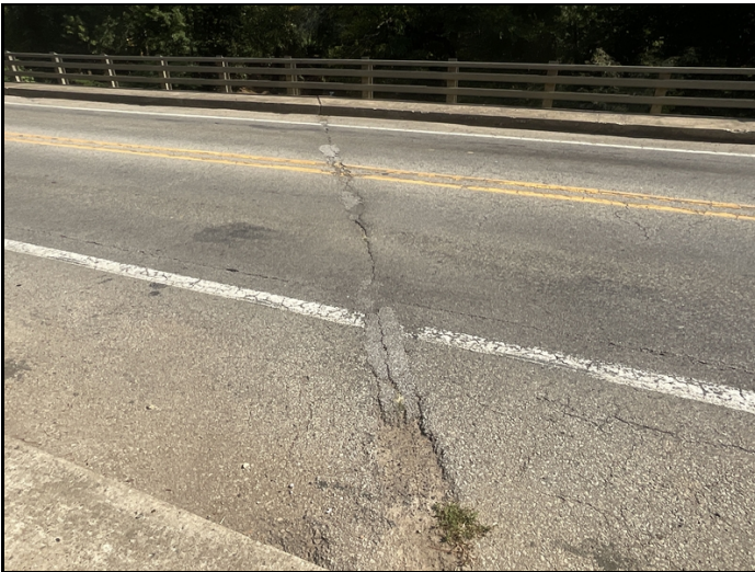
08/31/2023 - JCJ & TJL - The asphalt driving surface has numerous patched areas over the expansion joints.
