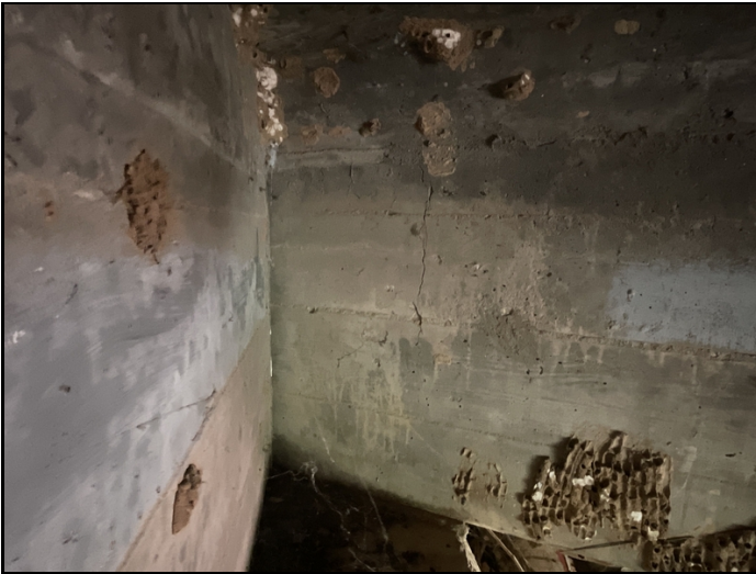
Span # 3, girder # 3 at abutment # 2 Left face has a vertical crack approximately 1/16" wide located approximately 1' from the face of the abutment backwall.
