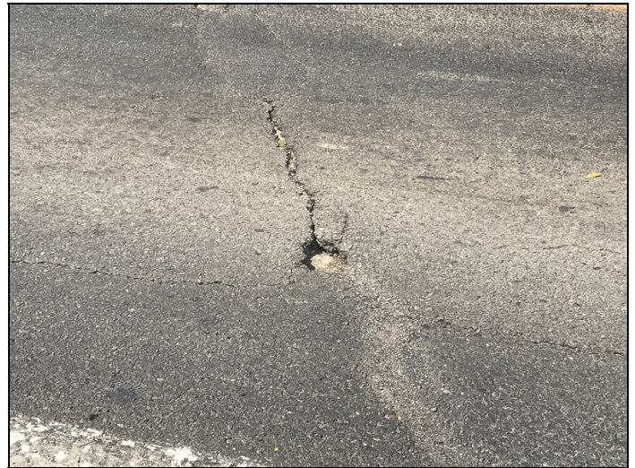
Pothole forming in wearing surface of left lane over bent # 3.
