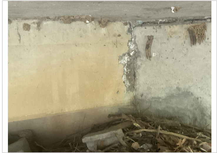
Span # 3, Girder # 3 at Abutment # 2 has a vertical crack and shallow spalling at the abutment interface.
