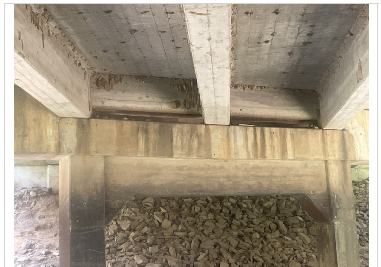
Staining due to joint leakage. Photo of Bent # 3. Cap.
