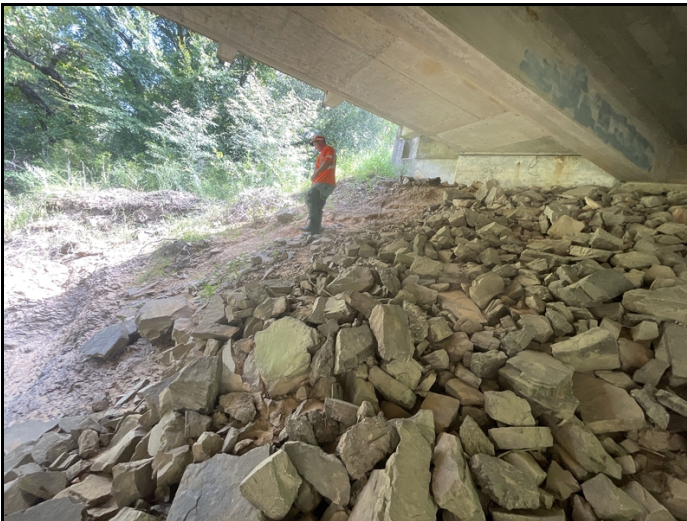
Abutment # 2 has riprap displacement with embankment erosion at the outlet end of the abutment.
