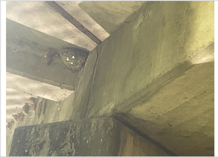
Span # 1, Left vertical face of slab over Bent # 2 has a delaminated area that is up to approximately 2" wide and 22" tall.
