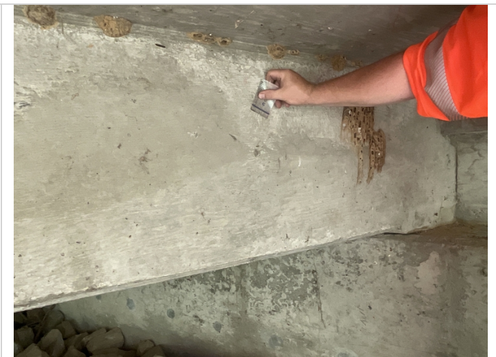
Span # 3, Right side of slab portion of structure has a diagonal crack in undersurface and a shear type crack near abutment # 2 that measures 0.006".
