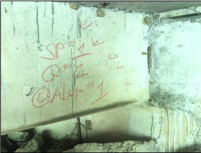
Span # 1, girder # 1 at abutment # 1-Hairline shear type crack.
