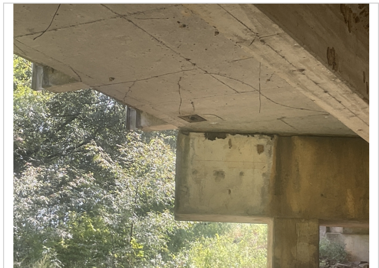
Span # 2 has an 18" delaminated area adjacent to the Span # 2 deck drain located near the Left end of Bent # 3 cap.
