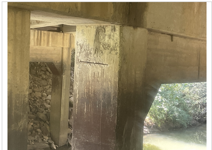
Bent # 2, Column # 2 has shallow spalling with exposed reinforcing steel in the upper portion of the column that has very little concrete cover from the construction process. Exposed reinforcing steel has up to initial section loss and appears to be a hoop around the primary vertical reinforcing steel in the column.
