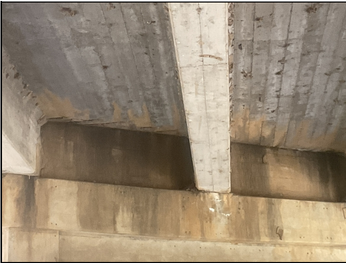
Span # 2-Spalling with exposed reinforcing steel between Girders # 2 and 3 at Bent # 2.
