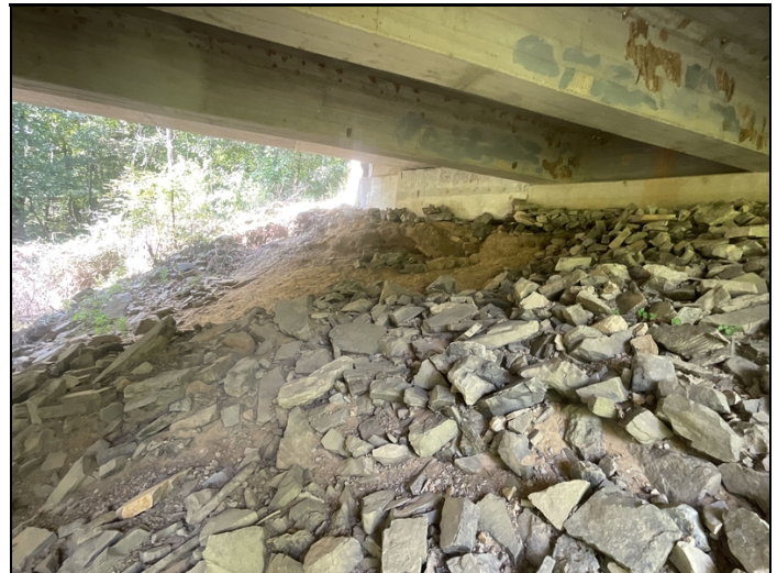
Abutment # 1 has riprap displacement with embankment erosion at the inlet end of the abutment.
