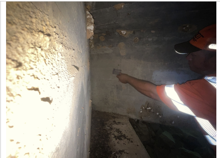
-Span # 3, Girder #3 at Abutment # 2 Left face has a vertical crack approximately 1/16" wide located approximately 1' from the face of the abutment backwall.
