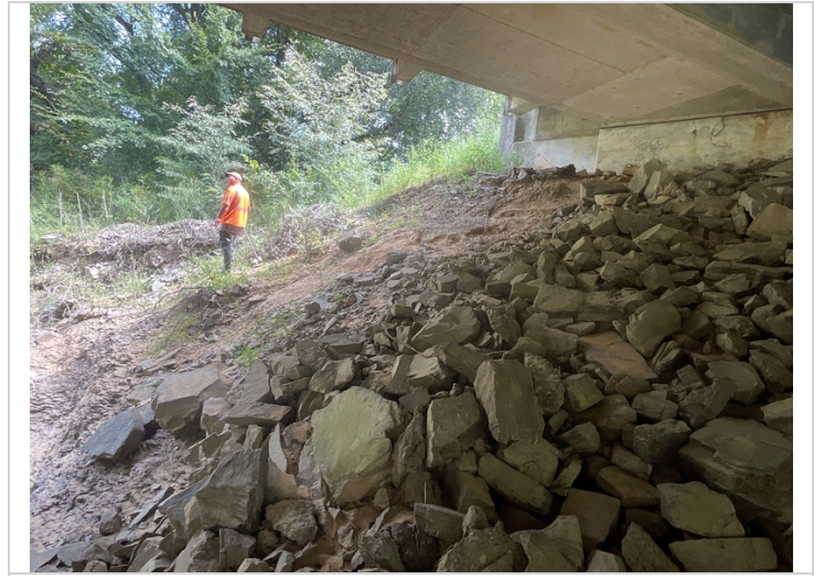
Abutment # 2 has riprap displacement with embankment erosion at the outlet end of the abutment.
