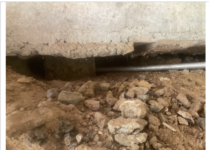
Abutment # 1. Right side has earth settlement with 1 steel pile exposed in the widened portion of the abutment located approximately 4' from Girder # 3.
