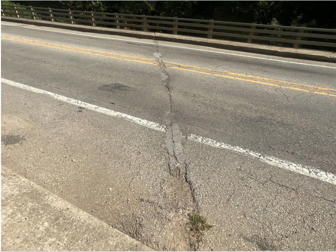
The asphalt driving surface has numerous patched areas over the expansion joints. Photo taken over Bent # 3.
