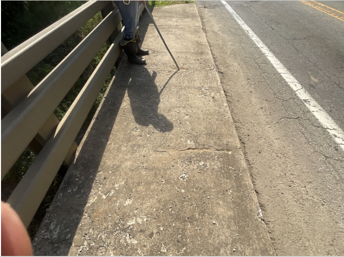
Sidewalk: The Left sidewalk on Spans # 1 and 3 have shallow spalls with exposed reinforcing steel. Exposed reinforcing steel has very little concrete cover from the construction process. Exposed reinforcing steel has up to initial section loss.
