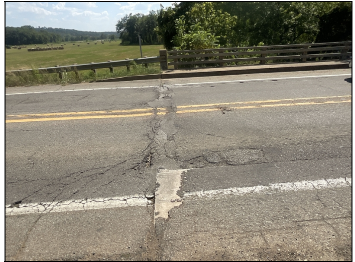
Asphalt driving surface breaking apart over Abutment # 2.
