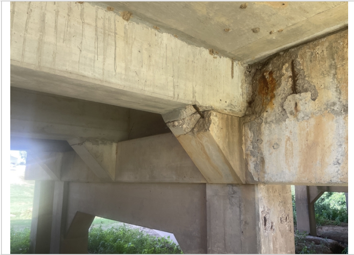
Span # 1. Girder # 3. Fixed end. Spall with exposed reinforcing steel.
