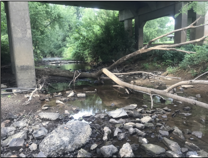
The channel has drift accumulation at bent #5.
