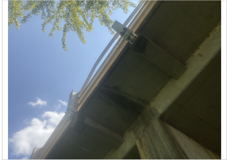
Left side of Span # 5 & 6. Metal rail posts are split from apparent impact damage.
