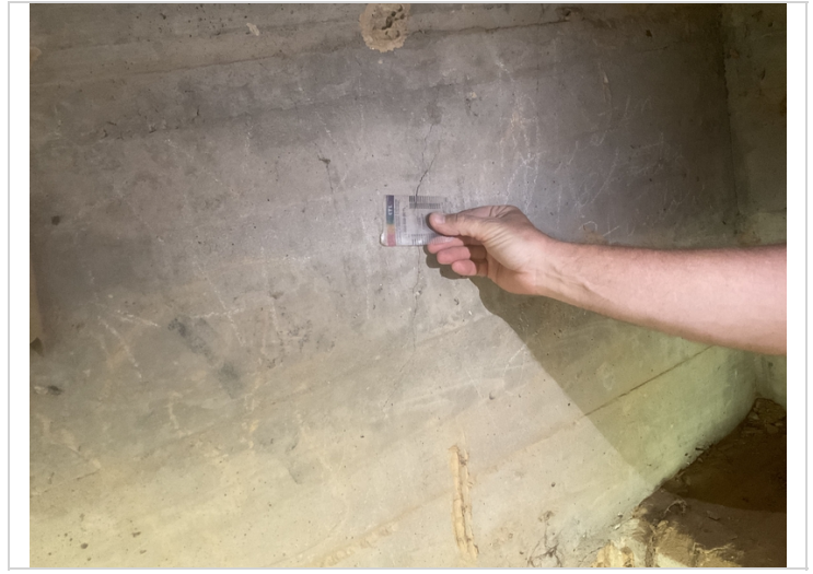
Girder # 3. Bent # 1. Vertical crack measured 0.030".
