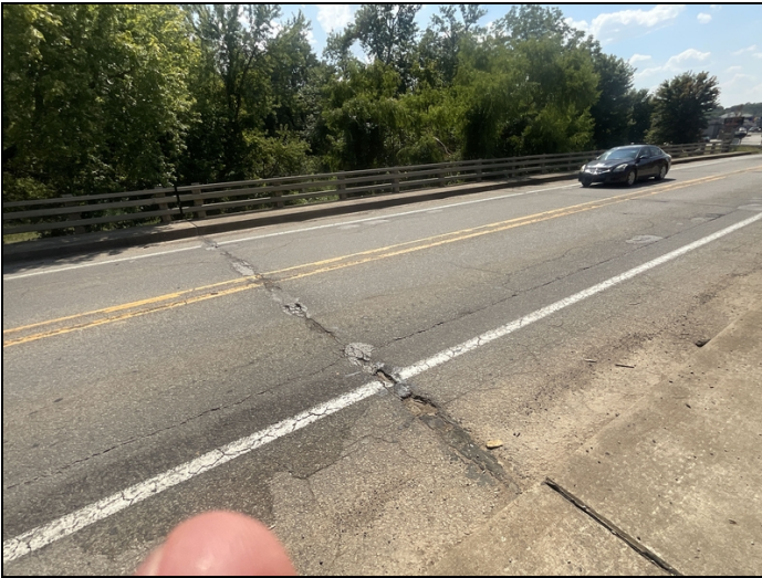
Asphalt driving surface breaking apart over Bent # 5.
