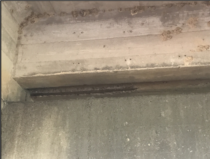
Span # 3 deck haunch over bent # 3-Spalling with exposed reinforcing steel.
