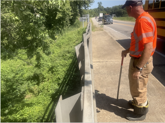
Approximately 15' of collision damage to bridge railing in Spans # 5 & 6 Left.
