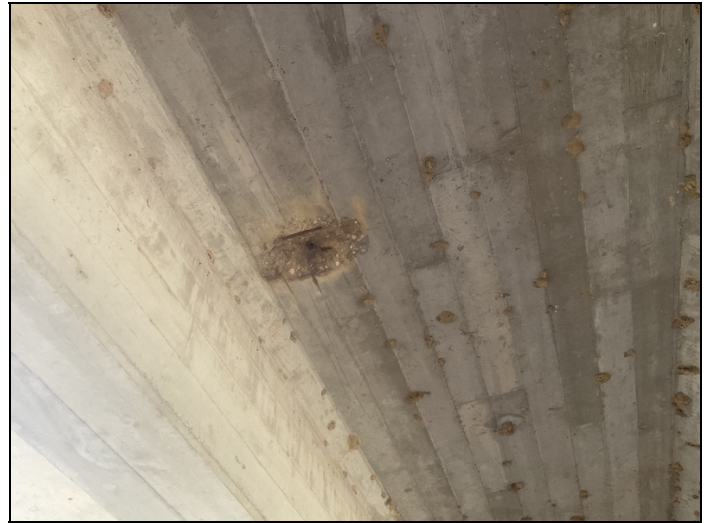
Span # 2. Bay # 1. Spall with exposed reinforcing steel.
