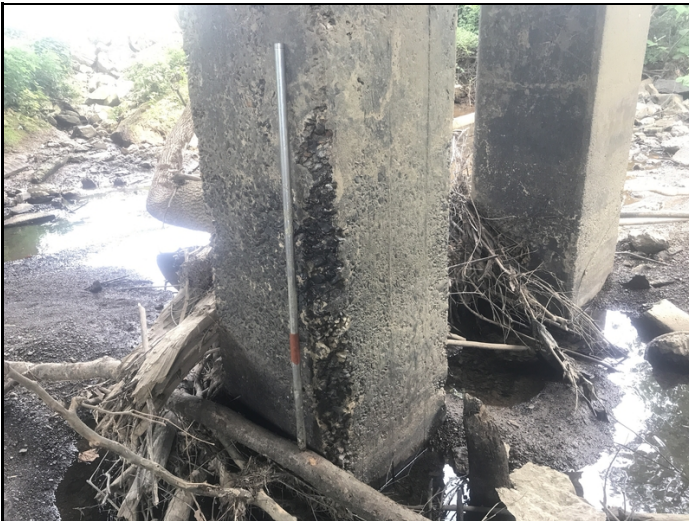
Bent # 5, column # 2-Heavy abrasion / concrete deterioration.
