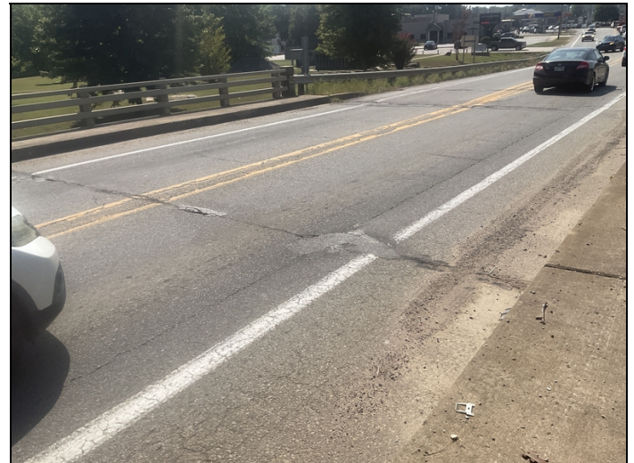
Asphalt driving surface breaking apart over Bent # 2.
