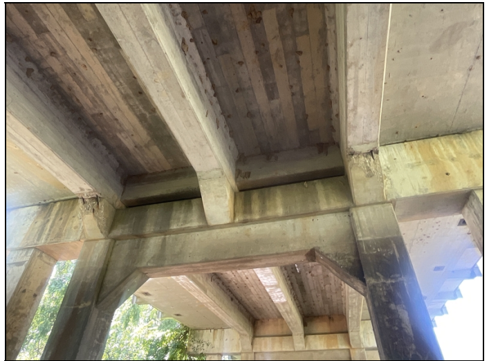
Bent # 5. Spalls with exposed reinforcing steel in the cap haunches.
