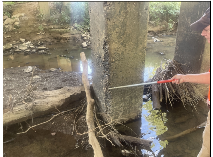
Bent # 5, Column # 2 has concrete deterioration and section loss with no exposed reinforcing steel.
