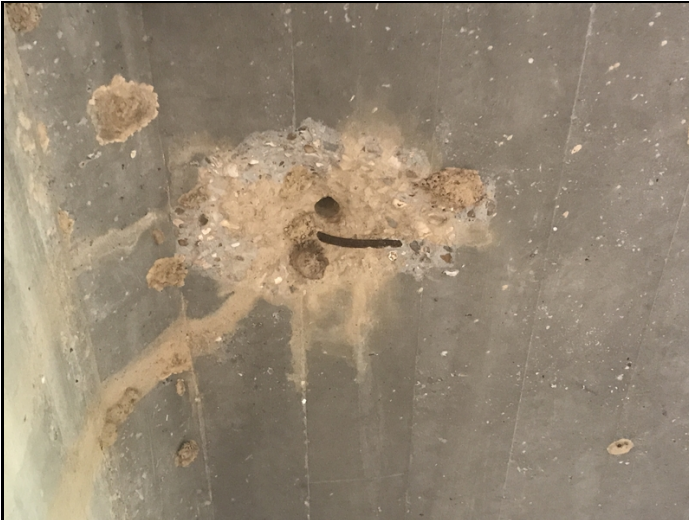
Span # 1, bay # 2-Spall with exposed reinforcing steel.
