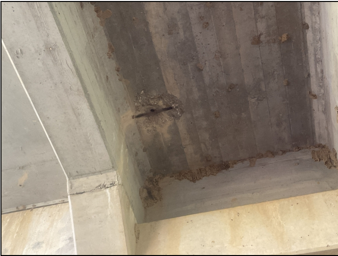
Span # 5. Bay # 1. Spall with exposed reinforcing steel.
