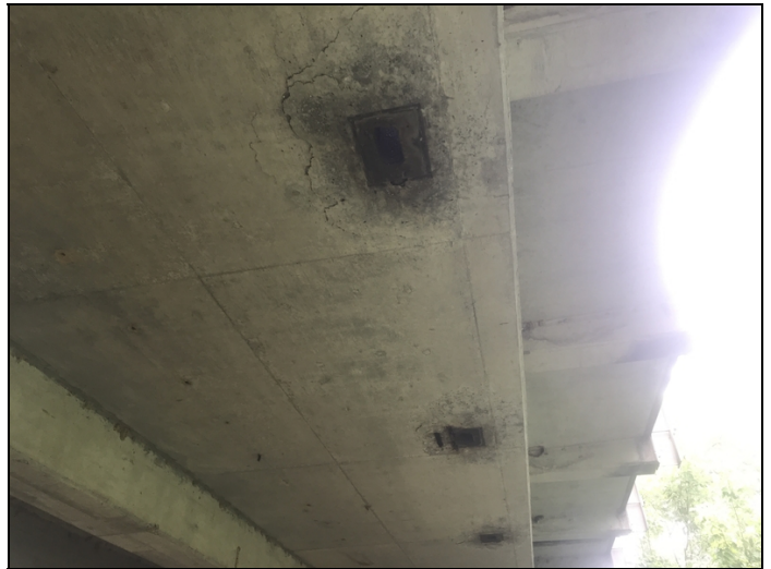
Span # 3, right side-Delaminated and spalled areas with exposed steel adjacent to deck drains.
