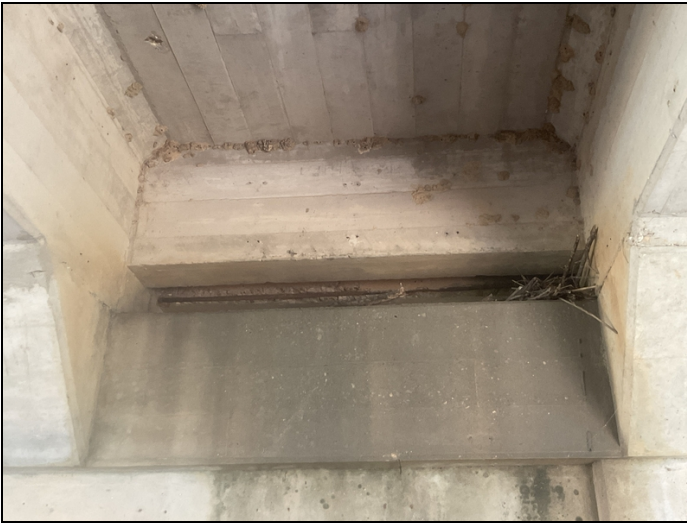
Span # 3. Bent # 3. Spalling with exposed reinforcing steel in the diaphragms.
