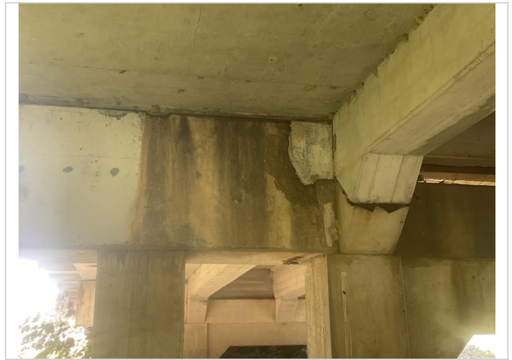
Bent # 3. Ahead face. Spall adjacent to Girder # 3.
