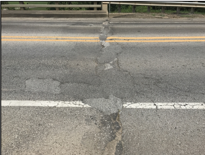
Abutment # 2 expansion joint.
