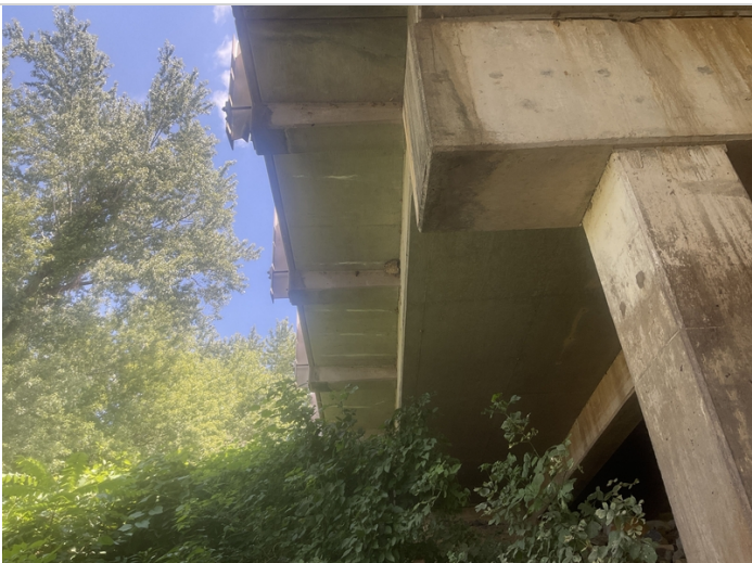
Span # 6. Transverse cracks with efflorescence in the sidewalk portion of structure.
