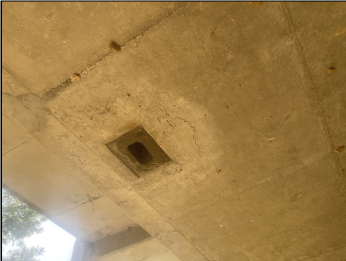
Span # 2. Right. Delaminated areas adjacent to the deck drains over the pedestrian walkway.
