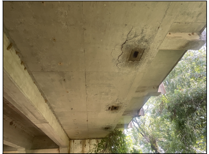
Span # 3. Slab soffit. Spalls with exposed reinforcing steel and delaminated areas.
