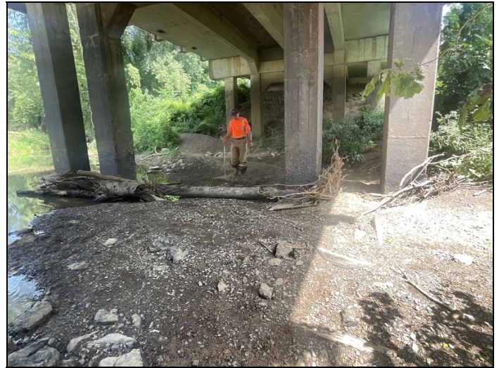
Bent 5. Drift accumulation.
