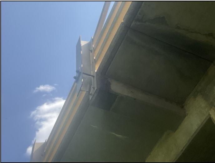
Left side of Span # 5 & 6. Metal rail posts are split from apparent impact damage.
