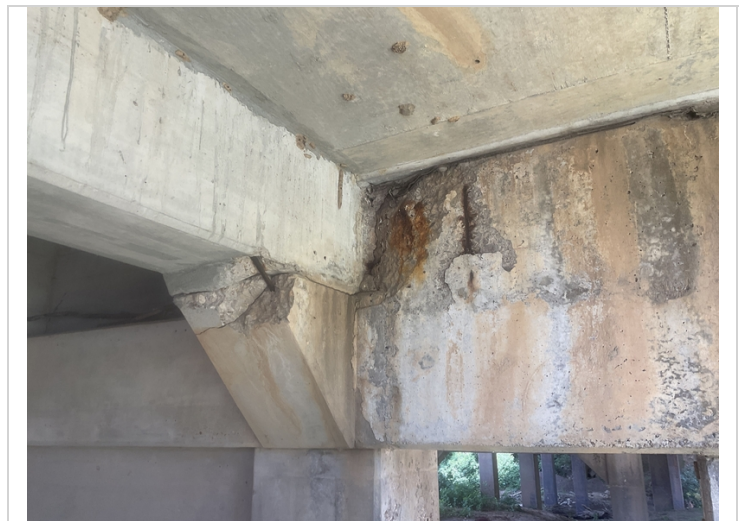
Bent # 2. Spalling with exposed reinforcing under and adjacent to Girder # 3.
