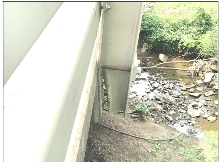
Span # 5, left-Collision damage to railing and post.
