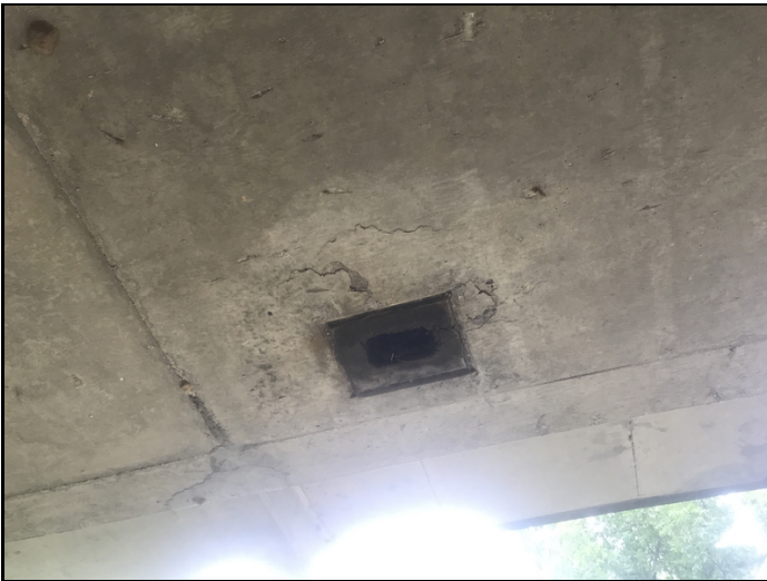
Span # 2, right side-Delaminated area adjacent to deck drain.
