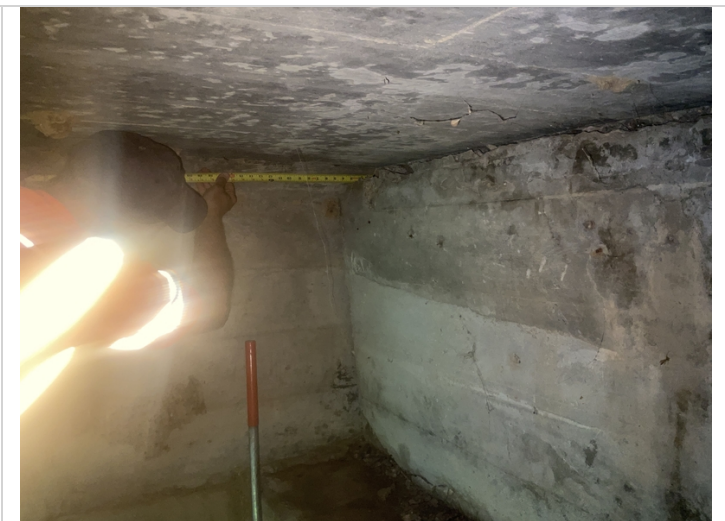
The end diaphragm in Bay # 2 over Abutment # 2 - Top of end diaphragm appears to be rotated towards the channel approximately 3.25" during this inspection.
