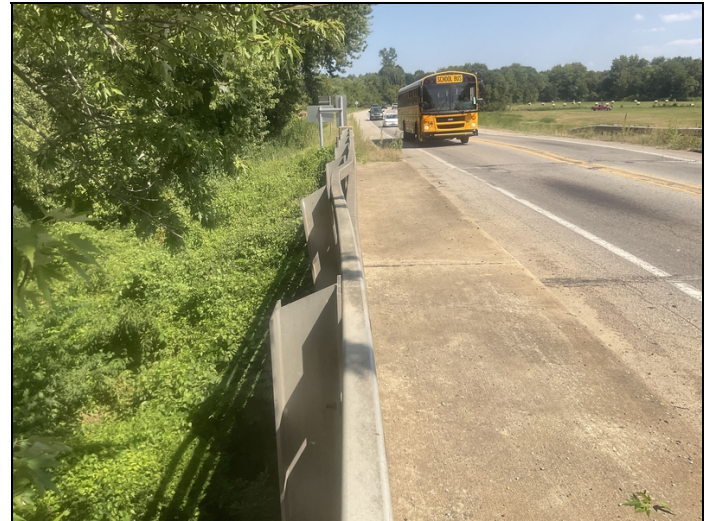
Approximately 15' of collision damage to the bridge railing on the Left side of Span # 5 & 6.
