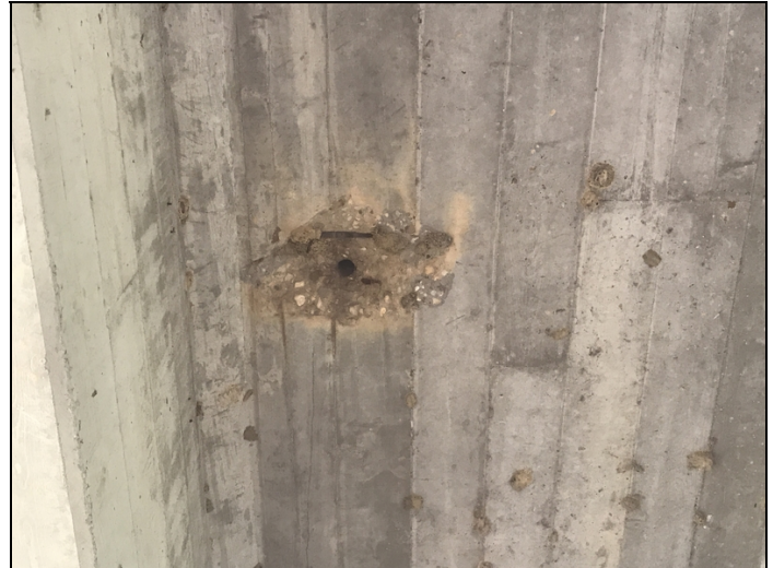
Span # 2, bay # 1-Spalling with exposed reinforcing steel in undersurface of deck.
