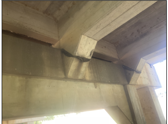
Span # 3. Girder # 2. Spalling with exposed reinforcing steel.
