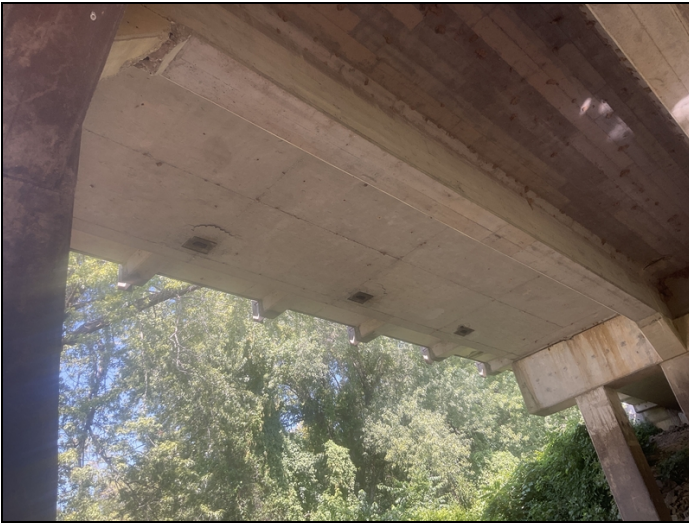
Span # 5. Slab soffit. Delaminated areas adjacent to the deck drains.
