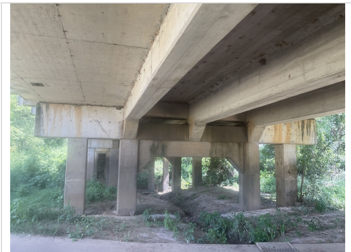
Compression Joint Seals - Staining on the substructure indicates that the compression joint seals leak water.
