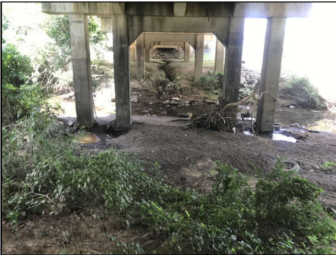
Bent #5 light drift accumulation.
