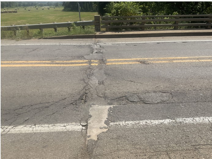
Asphalt driving surface breaking apart over Abutment # 2.
