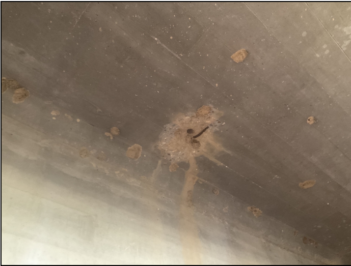
Span # 1. Bay # 2. Spall with exposed reinforcing steel.
