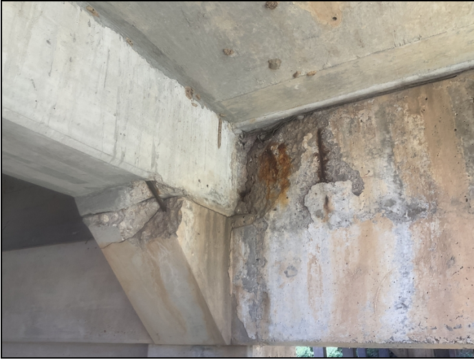
Bent # 2. Spalling with exposed reinforcing steel.
