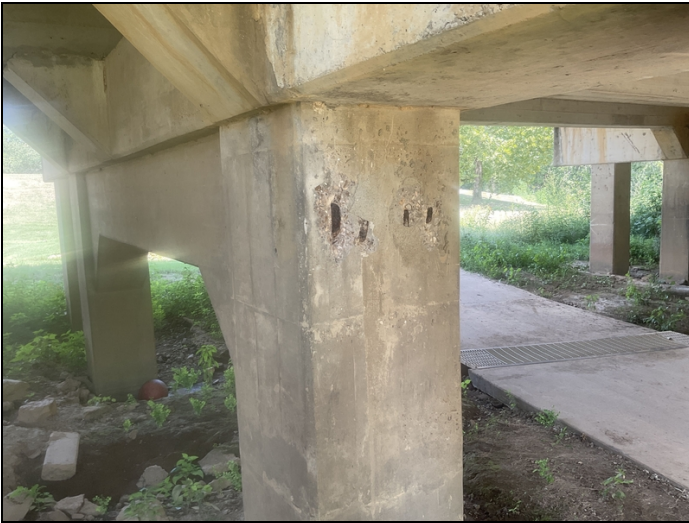
Bent # 2. Column # 2. Spalls with exposed reinforcing steel.
