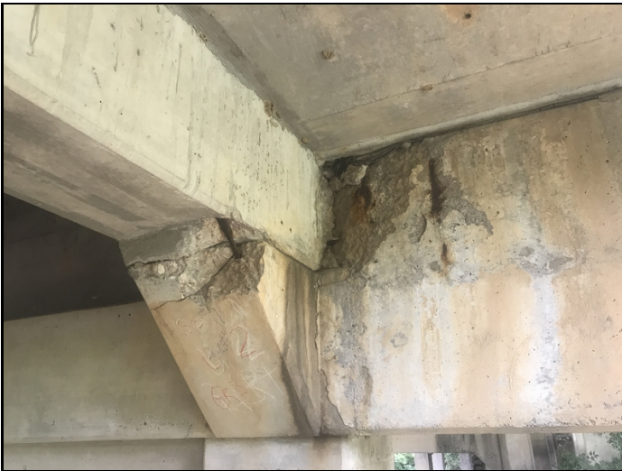
Bent # 2-Spalling with exposed reinforcing steel at girder # 3.
