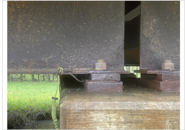
Beam 1. Bent 2. Span 2. There is 1/2" remaining section in the bottom flange thickness.
