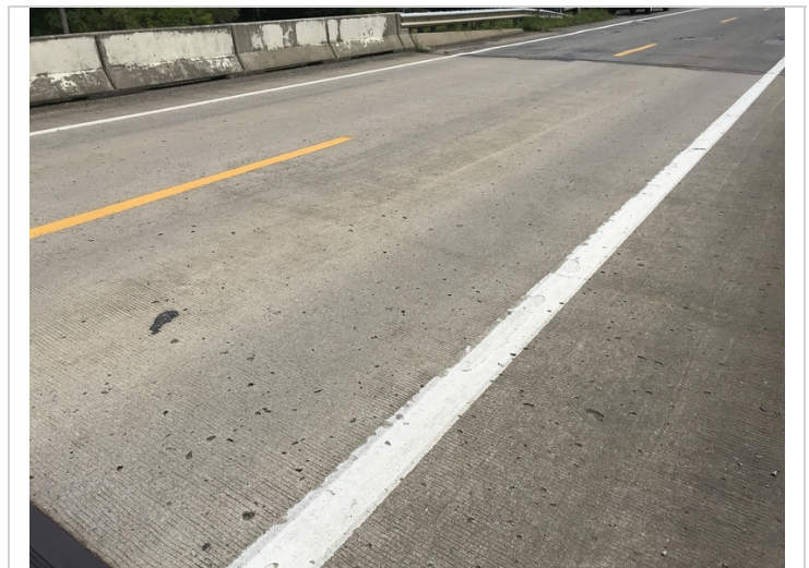
Span # 7 pop outs on the driving surface of the deck.
