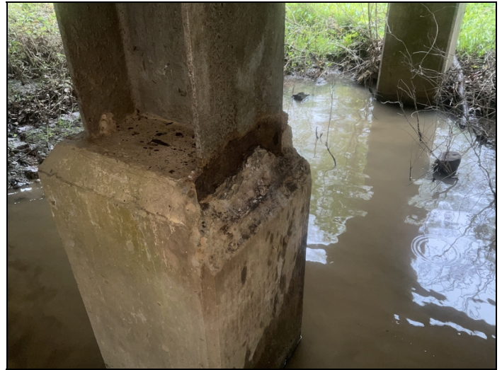
Active corrosion with pack rust. Bent # 3. Pile # 3.
