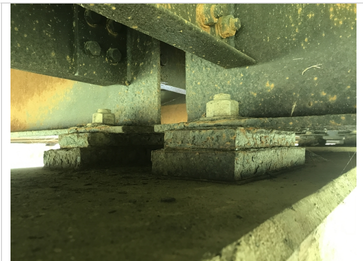
Fixed bearings with active corrosion and layers of flaking rust.
