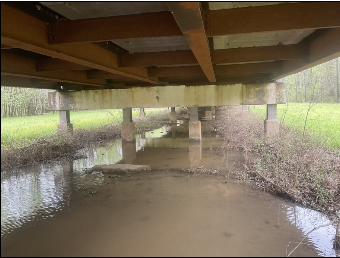
Staining in the bent caps from apparent joint leakage.
