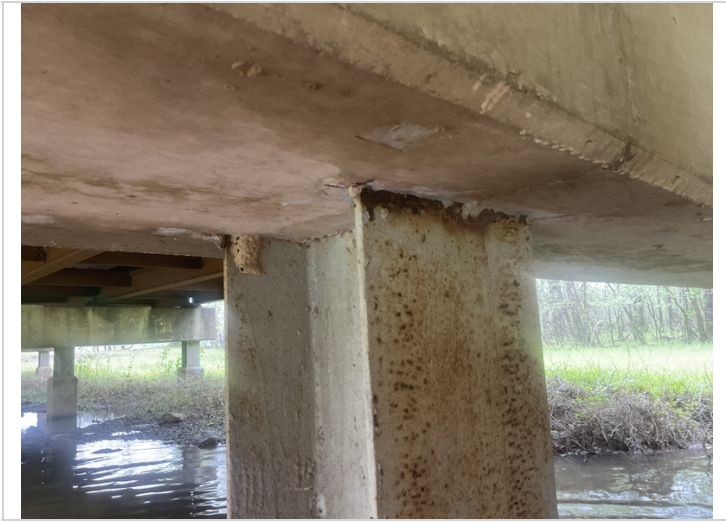
Active corrosion in the steel piles at the cap juncture. Pile # 4. Bent # 2.
