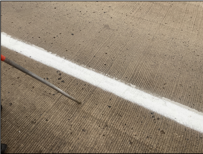
Transverse cracks in the driving surface of the deck.
