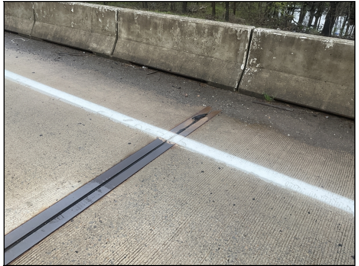
Damaged compression joint seal over bent # 3. Left.
