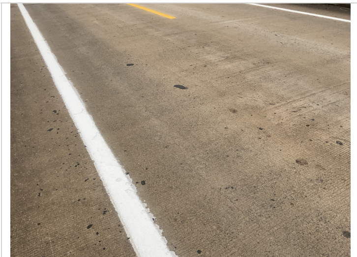
Longitudinal and transverse cracking in Span # 2. Driving surface.
