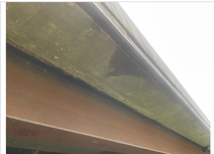
Transverse cracks with efflorescence in the overhang of the deck.
