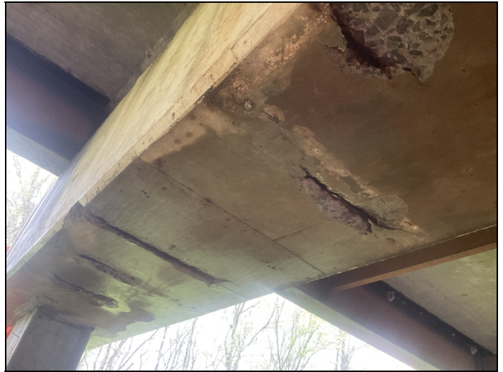
Undersurface of bent # 4. Several spalls with exposed reinforcing.
