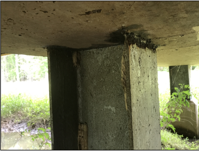
Typical active corrosion along the cap / steel pile interface.
