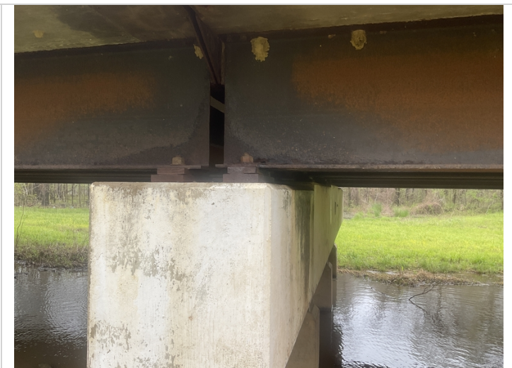
Beam 5. Bent 5. Active corrosion in the beam ends.
