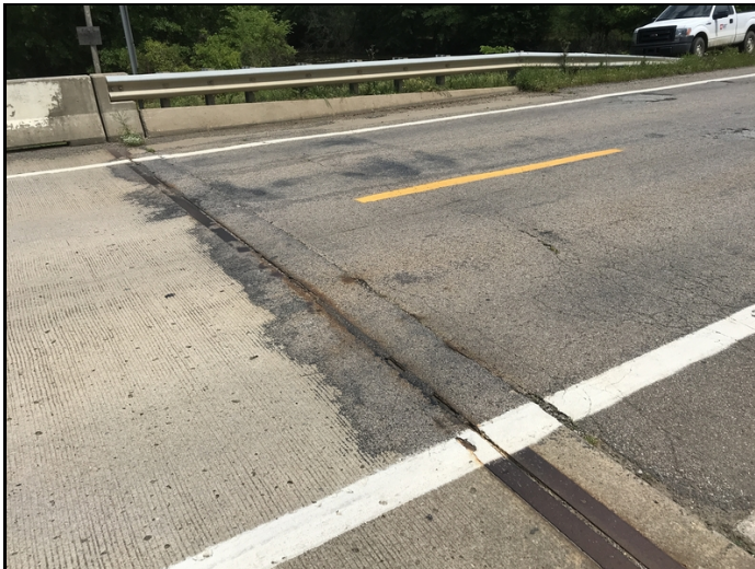
Bent # 8 minor asphalt settlement.
