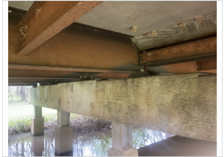
Active corrosion in the bearings.
