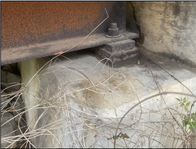
Beam # 5. Bent # 8. Active corrosion in the bearings.
