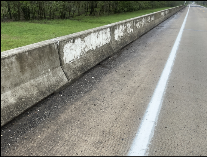
Right gutter. Debris accumulation.
