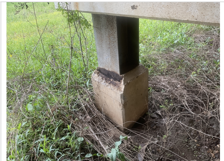
Active corrosion with flaking rust in the steel pile. Spalling with exposed reinforcing steel in the concrete collar. Bent # 7. Pile # 4.
