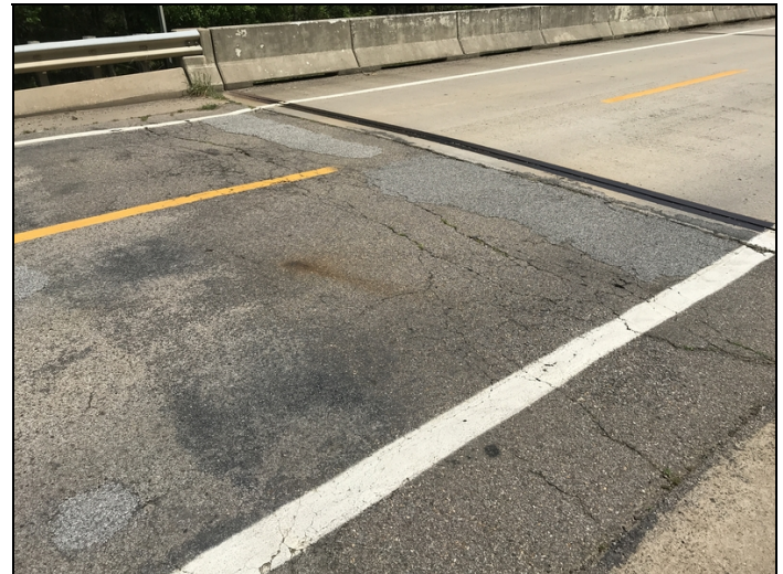
Bent # 1 approach roadway asphalt breaking apart and minor settlement.
