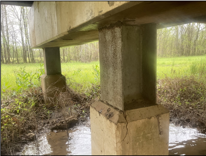
Bent # 6. Pile # 3. Active corrosion with section and delaminated concrete collar.
