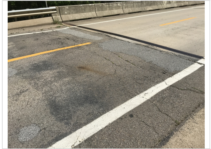
Bent # 1 approach roadway asphalt breaking apart and minor settlement.
