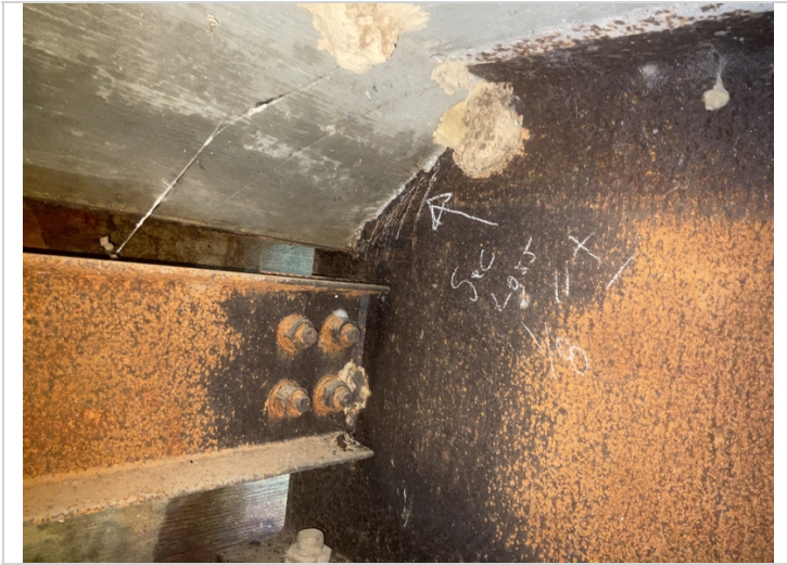
Beam 1. Bent 1. Active corrosion with section loss that measured 1/8" deep during this inspection.
