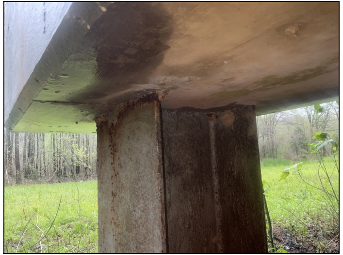
Active corrosion with section loss in the steel piles at the cap juncture. Bent # 2. Pile # 1.
