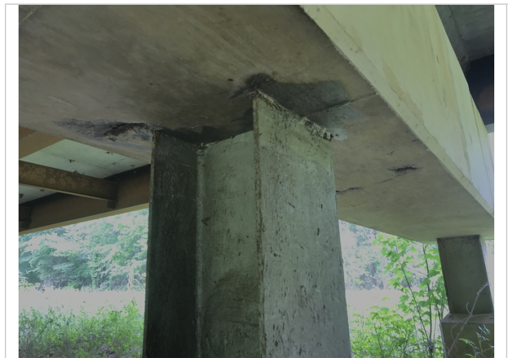
Bent # 3 spalling with exposed reinforcing steel on the undersurface of the cap.
