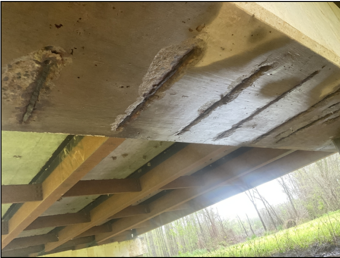
Undersurface of bent # 7. Spalls with exposed reinforcing steel.
