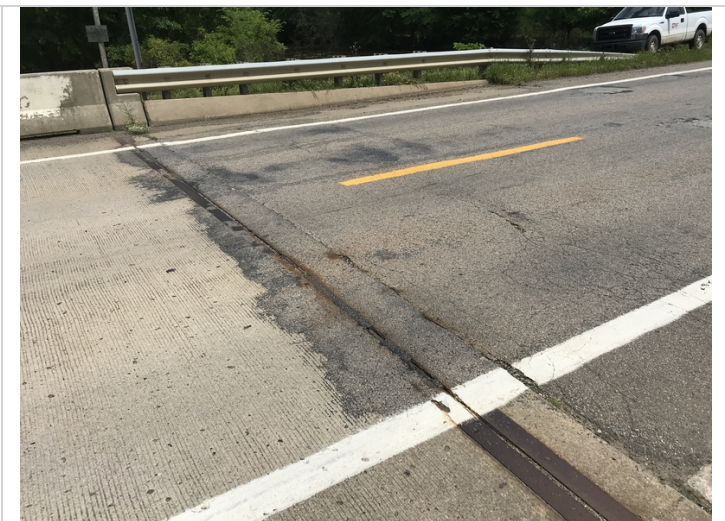
Bent # 8 minor asphalt settlement.
