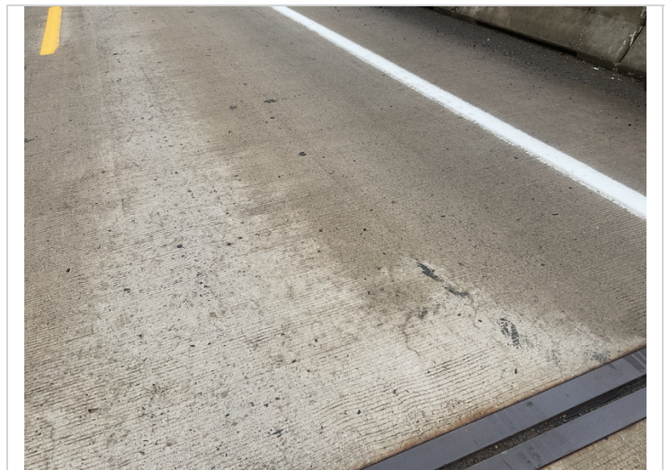
Longitudinal cracking in driving of Span # 1.
