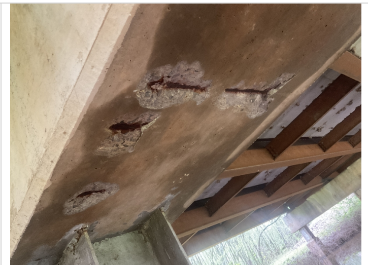
Undersurface of bent # 3. Spalls with exposed reinforcing steel.
