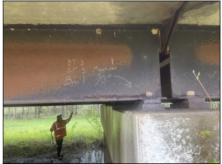
Span # 3. Beam # 1. Bent # 3. Has been reduced down to 3/8" thickness.
