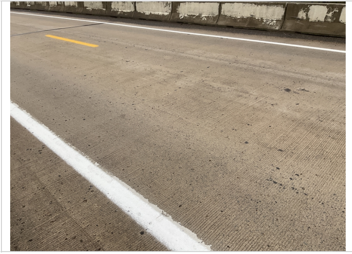
Driving surface of Span # 7. Several pop outs.
