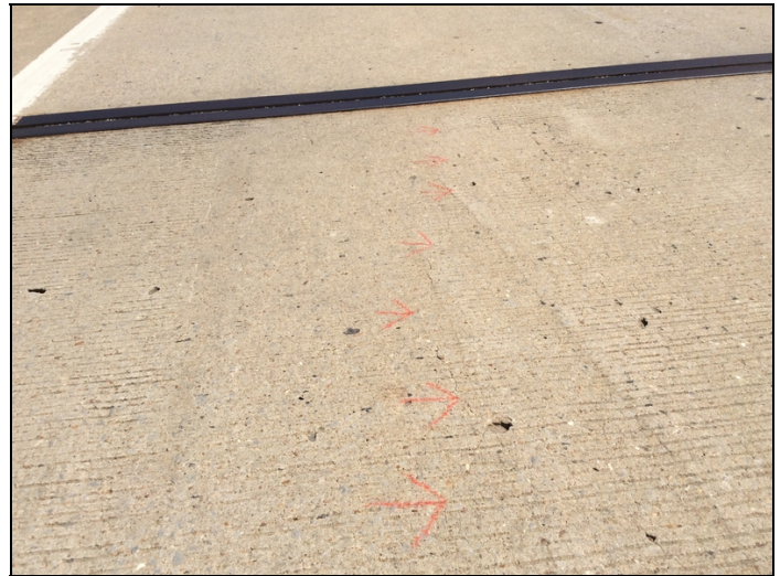
Span # 1, left lane-Longitudinal cracking.
