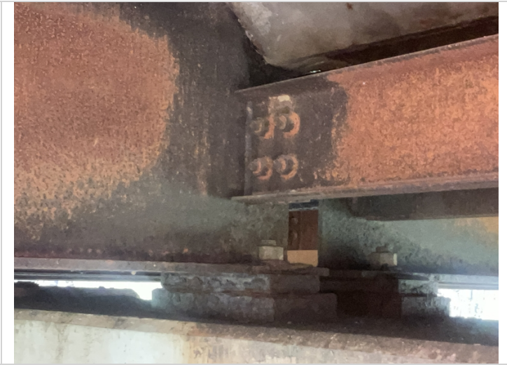
Active corrosion. Beam 2. Over Bent 4.
