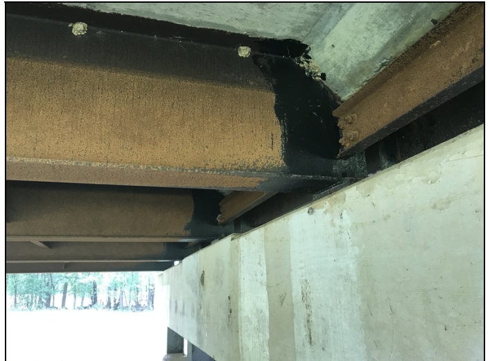
Bridge mate applied to the beam ends in some locations.
