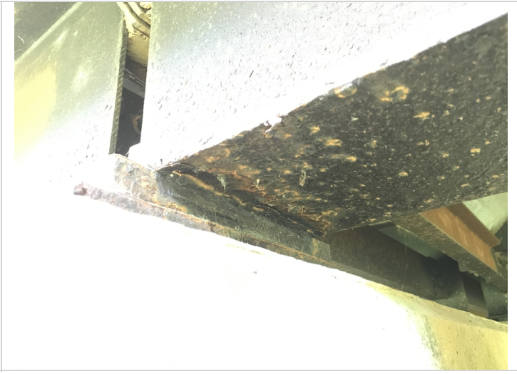
Bent # 3 Beam # 1 with initial section loss along the edge of the sole plate and the bottom surface of the bottom flange.
