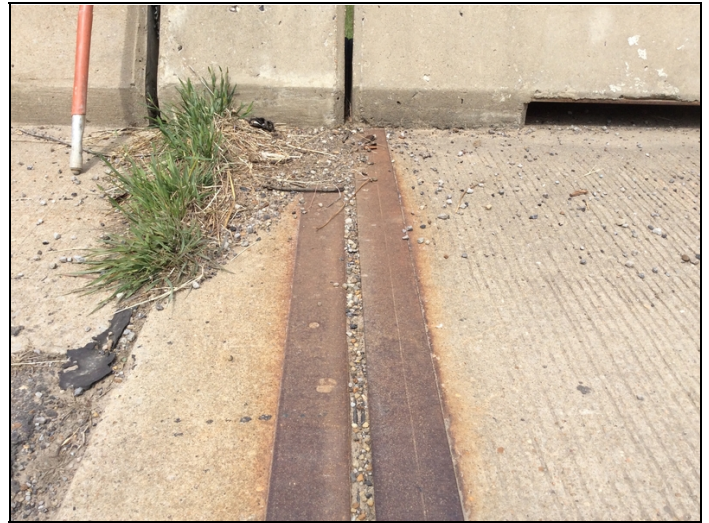
Expansion joints have dirt and debris impaction in the gutters.
