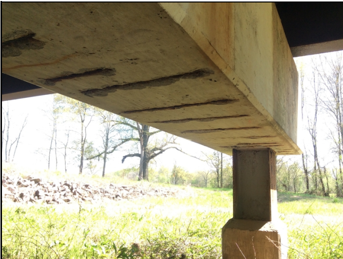
Bent # 7 undersurface of cap exposed reinforcing steel.
