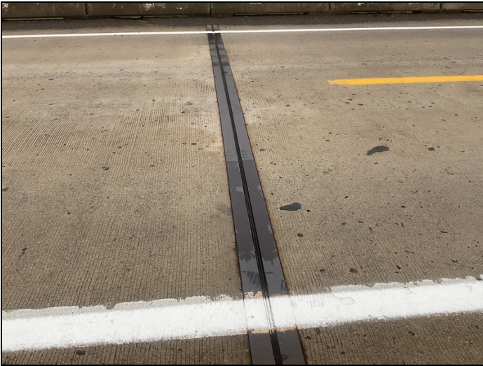
Deteriorated expansion joint seal over bent # 7.
