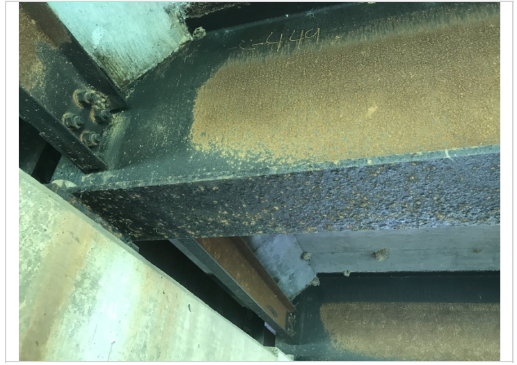
Typical flaking rust at the beam ends.
