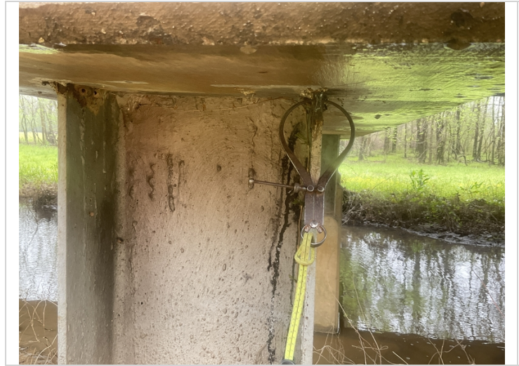
Bent # 4. Pile # 1. Flange edge has been reduced down to 1/8" thickness.
