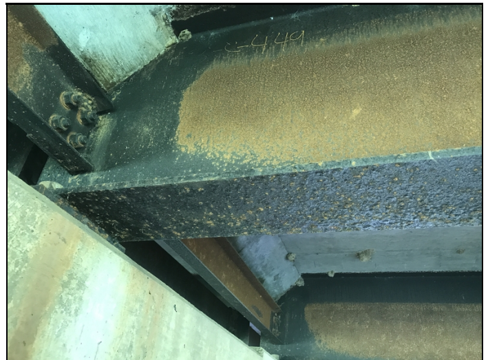
Typical flaking rust at the beam ends.
