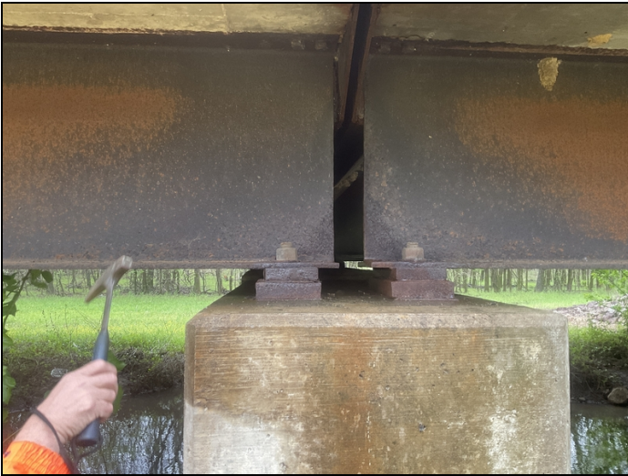
Active corrosion with flaking rust in the beam ends and bearings.
