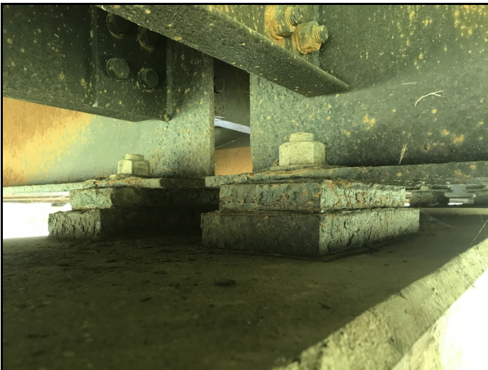
Fixed bearings with active corrosion and layers of flaking rust.
