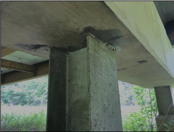
Bent # 3 spalling with exposed reinforcing steel on the undersurface of the cap.
