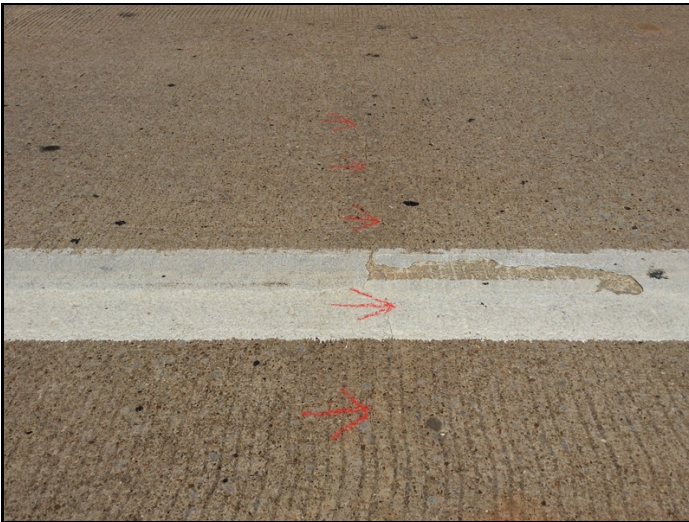
Span # 5, Right lane-Transverse cracking.
