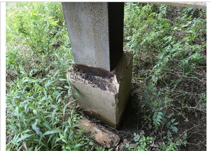
Active corrosion between concrete collar and the steel pile column.
