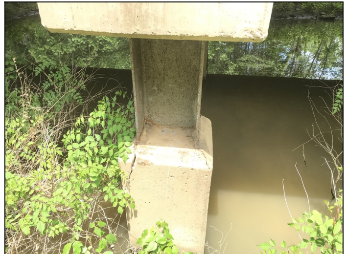
Bent # 2 Column # 4 active corrosion that is cracking the concrete collar at the base of the steel pile.
