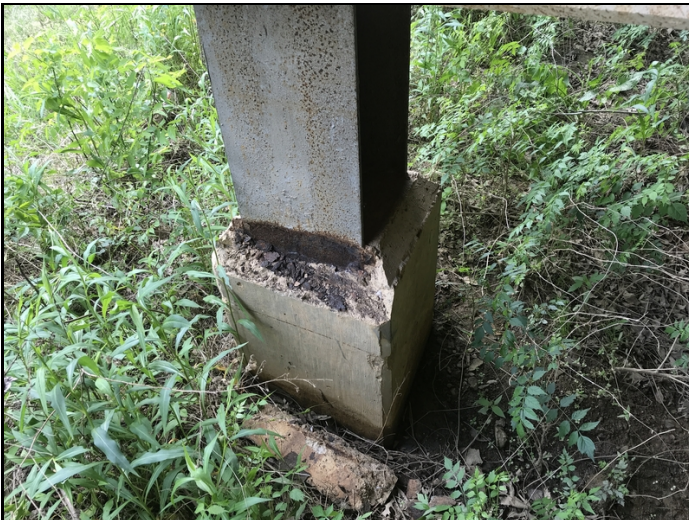
Active corrosion between concrete collar and the steel pile column.
