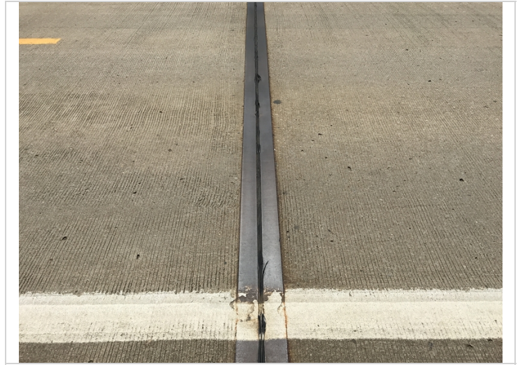
Bent # 4 failing compression joint seal.
