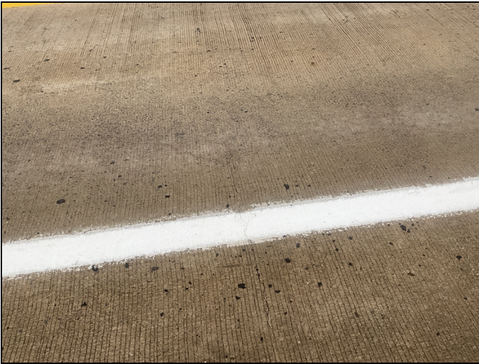
Sealable transverse cracks in the driving surface of the deck.
