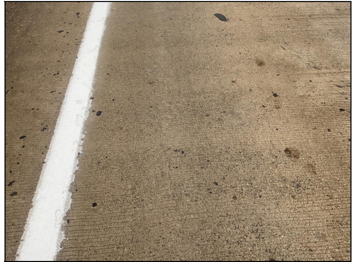
Sealable Longitudinal cracking in span # 2.
