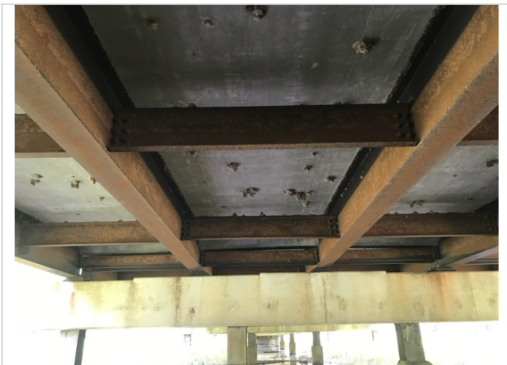
Typical undersurface of the deck.
