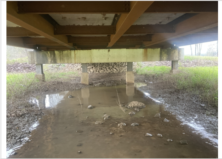
Bent # 7. Stains from apparent joint leakage.
