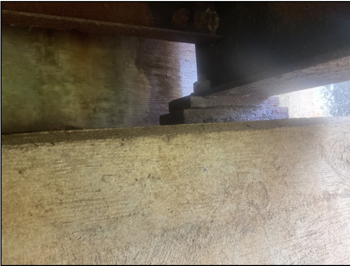
Active corrosion in the bottom flange adjacent to the bearings. Beam # 1. Bent # 1.
