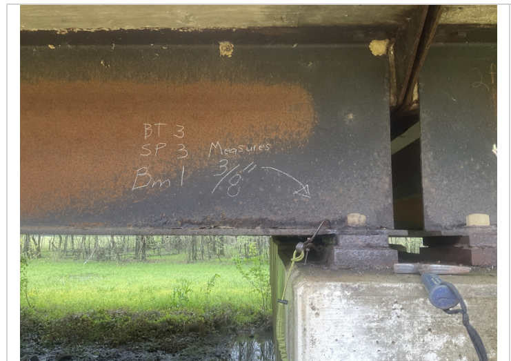
Span 3. Bent 3. Beam 1. Bottom flange has been reduced down to 3/8" thickness.
