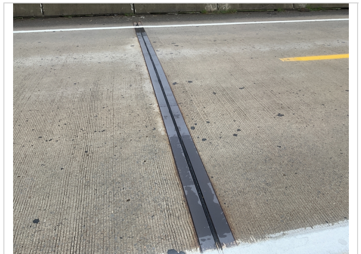
Compression joint seal over bent # 5.
