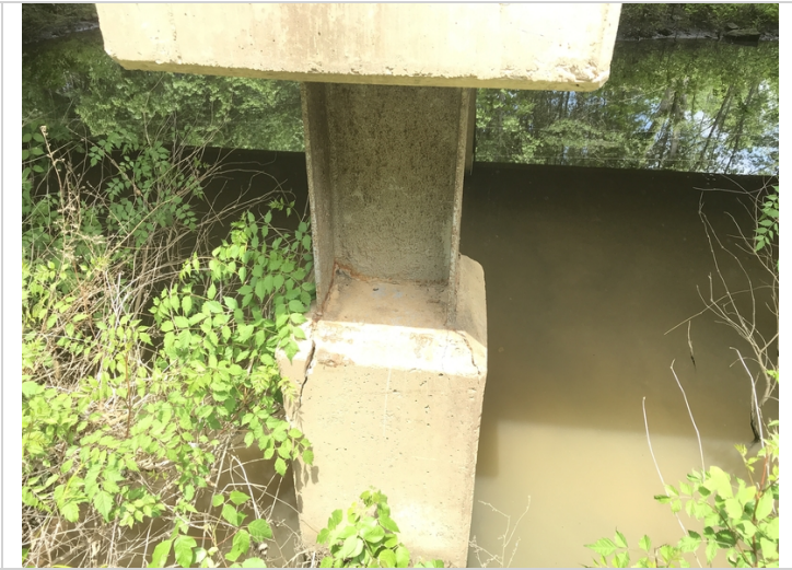
Bent # 2 Column # 4 active corrosion that is cracking the concrete collar at the base of the steel pile.
