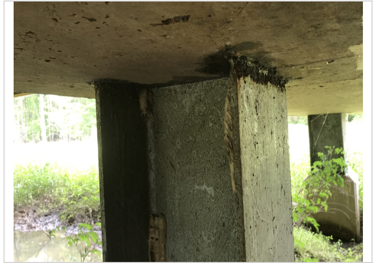
Typical active corrosion along to cap / steel pile interface.
