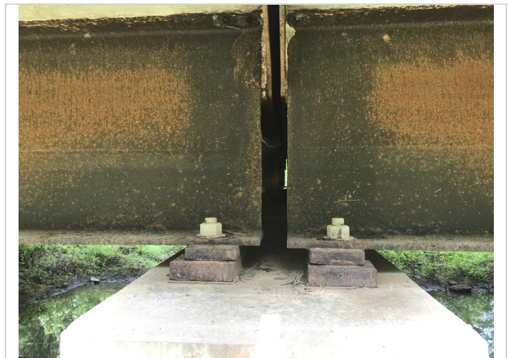
Bent # 2 Beam # 5 active corrosion along the bottom flange and base of the web.
