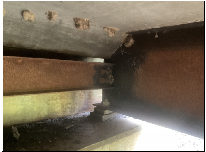
Active corrosion with section loss adjacent to the expansion dam.
