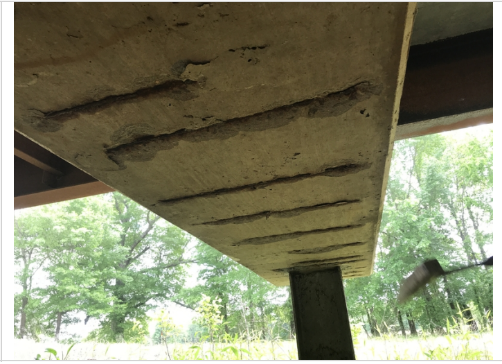
Bent # 7 cap undersurface spalling with exposed reinforcing steel.
