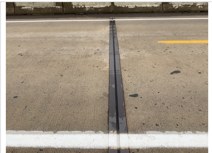
Compression joint seal over bent # 7.
