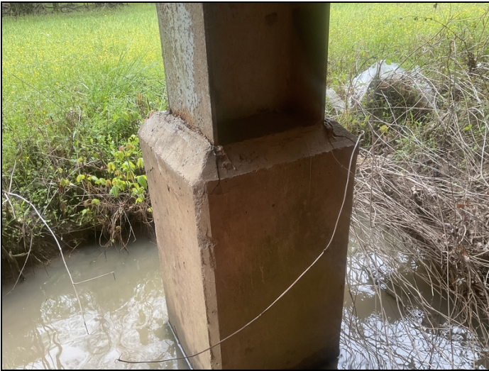
Bent # 2. Pile # 4. Delaminated areas in the top of the concrete collars.
