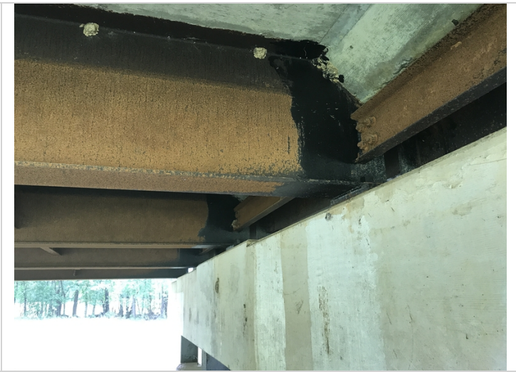
Bridge mate applied to the beam ends in some locations.
