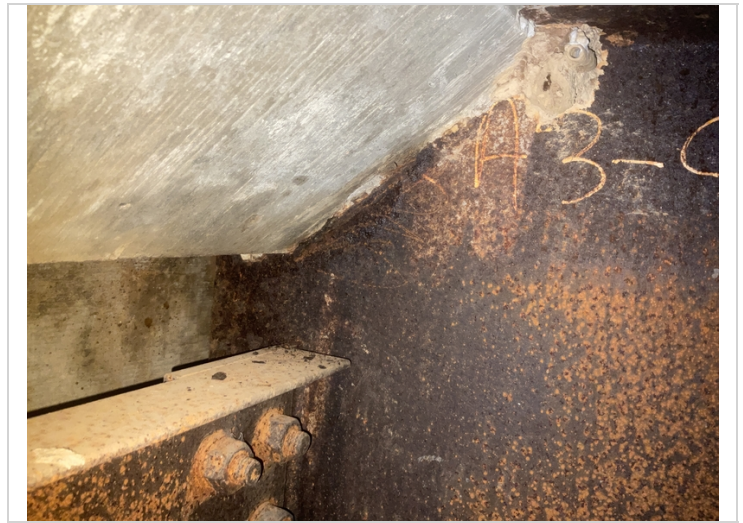
Active corrosion with section loss adjacent to the expansion dam. Beam 4. Bent.
