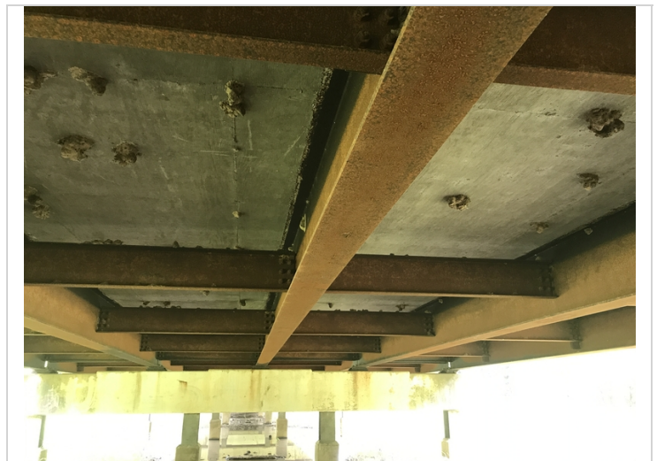
The protective coating has a light orange patina forming on the lower 3/4 of the beams and diaphragms from being inundated by the recent flooding events.
