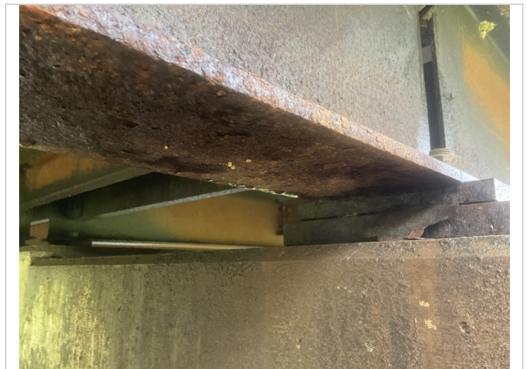
Active corrosion in the bearings.
