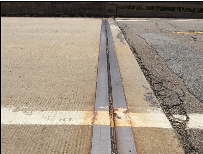
Expansion joint seals deteriorated.
