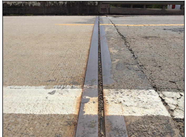
Deteriorated expansion joint seals.
