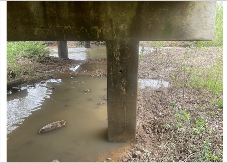
Left column of Bent # 4. No apparent change since the last inspection.
