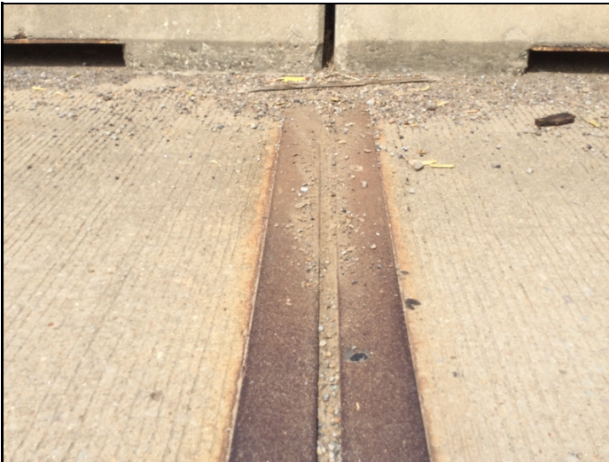
Dirt and debris impaction in assemblies.
