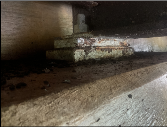
Bent # 1. Beam # 3 bearing corrosion.
