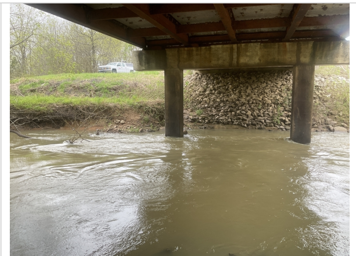
There is embankment erosion with some displacement of rip rap at the West embankment.
