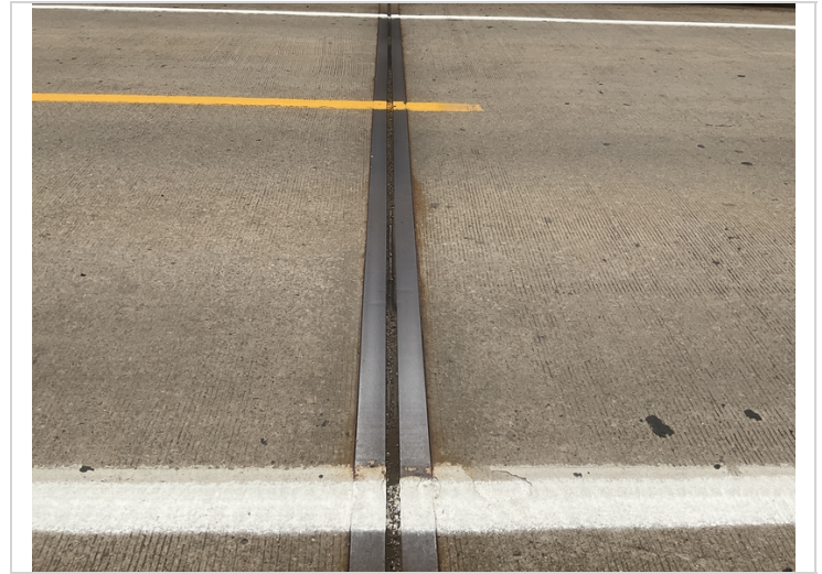
Expansion joint seal over Bent # 4.
