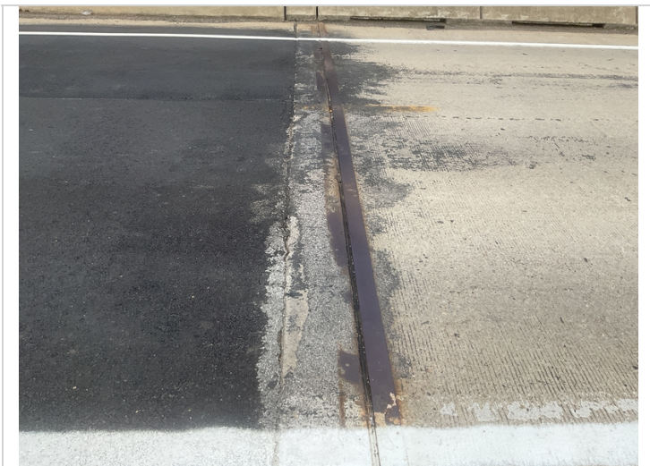
Top of Bent # 1 back wall. Partially covered with asphalt.
