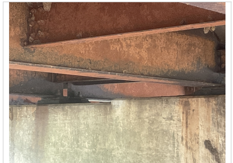
Bearing corrosion. Typical.
