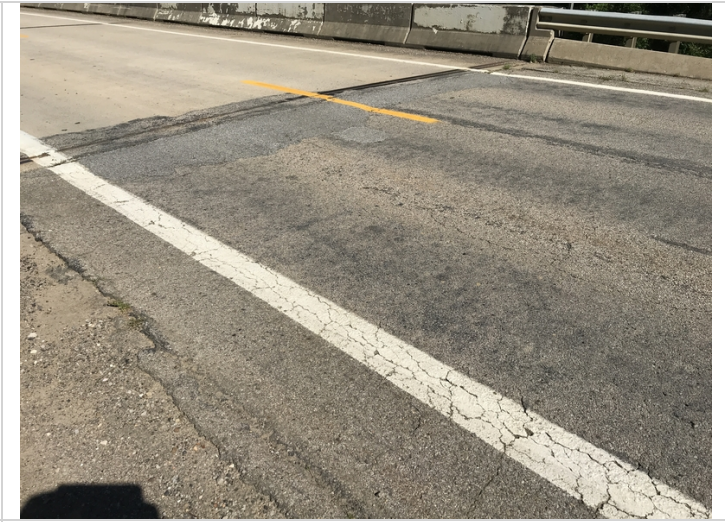
East approach asphalt settlement.
