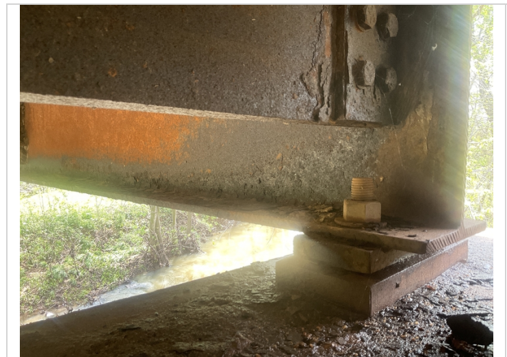
Span # 2. Beam # 5 beam corrosion.
