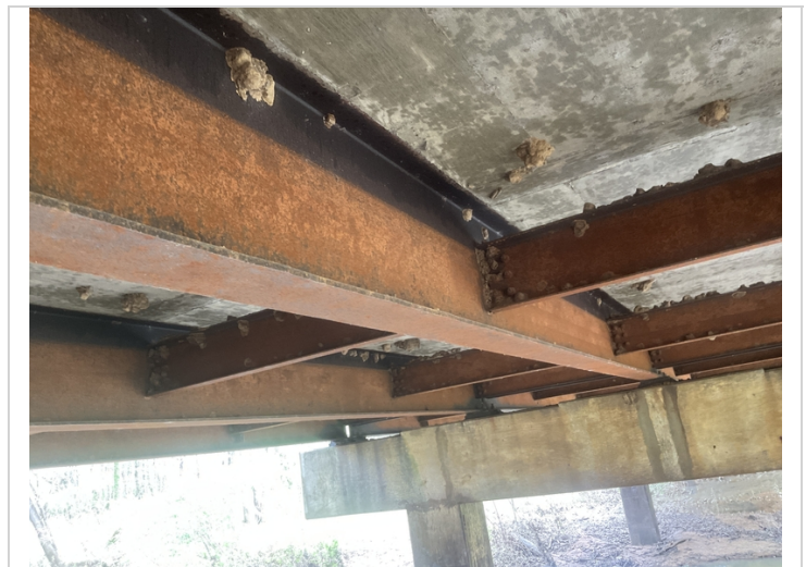
Superstructure has light rust nodes at the base of the beams. High Water elevation marks on the beams indicate that the water has reached the superstructure in the past.
