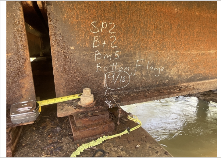
Span # 2. Bent # 2. Beam # 5 bottom flange measures 9/16" remaining section adjacent to the bearing.
