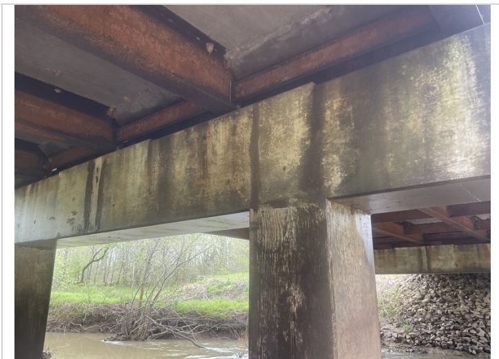
Wet substructure caps due to leaking expansion joint seals. Photo of Bent # 3. Typical.
