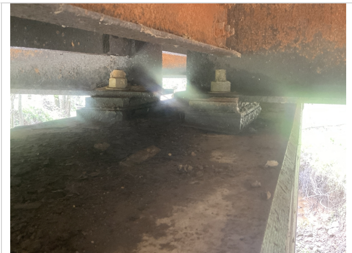
Bent # 2. Beam # 3 bearing corrosion.
