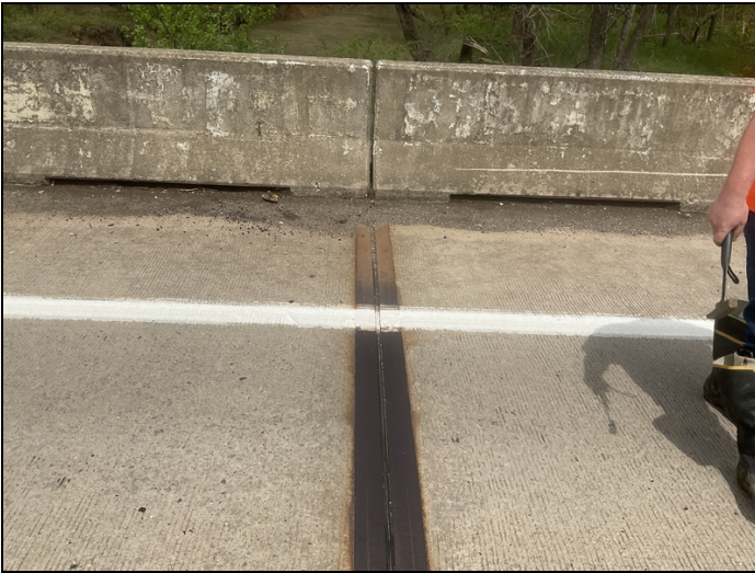
Expansion joint seal over Bent # 3. Typical.
