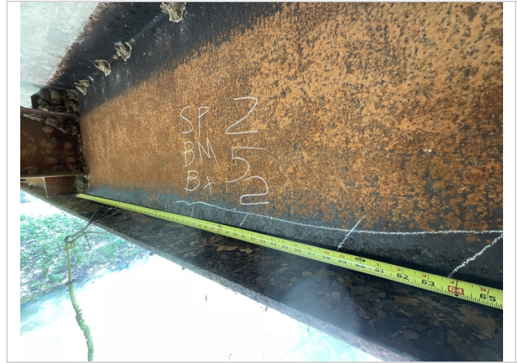
Span # 2. Bent # 2. Beam # 5 bottom flange measures 9/16" remaining section adjacent to the bearing. The remaining base of web and bottom flange has active corrosion with initial section loss.
