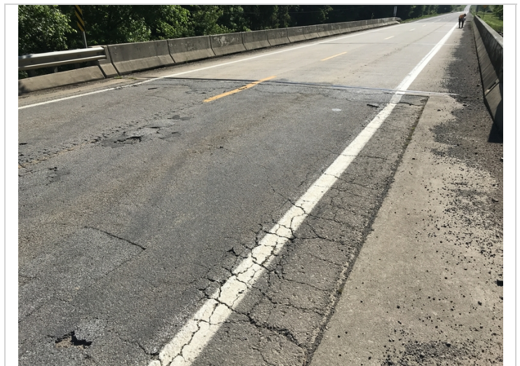
West approach roadway with asphalt deterioration and settlement.
