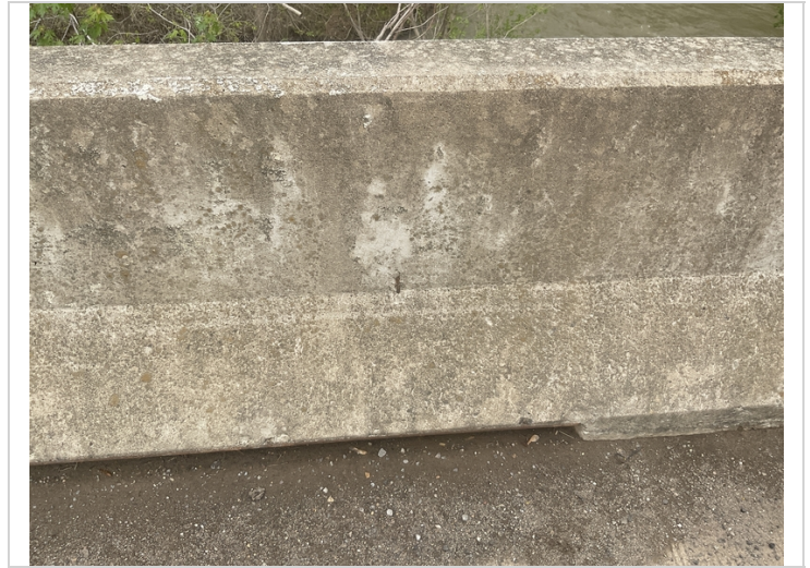
2" spall with exposed reinforcing steel in the face of the Left parapet wall.
