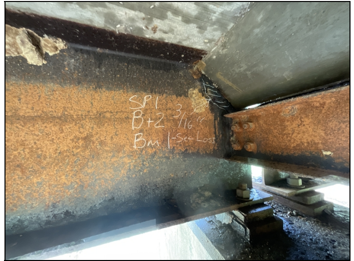
Span # 1. Bent # 2. Beam # 1 has 3/16" section loss to the web at the expansion dam juncture.
