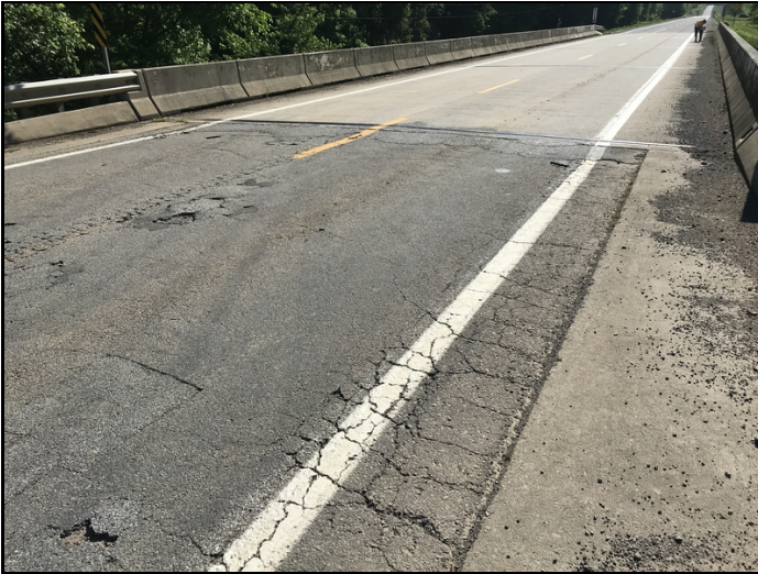
West approach roadway with asphalt deterioration and settlement.
