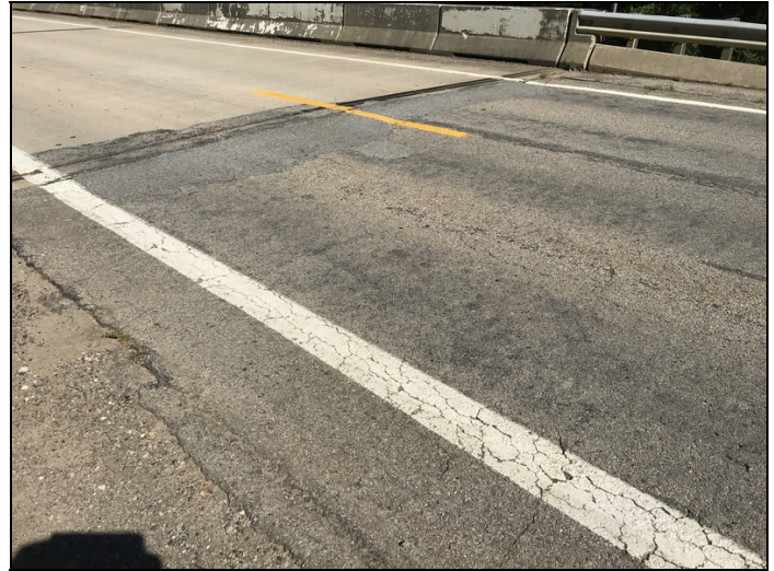
East approach asphalt settlement.
