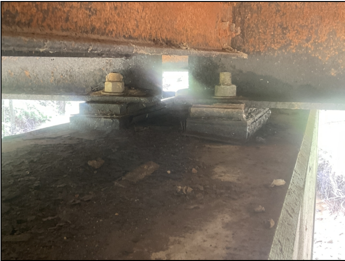
Bent # 2. Beam # 3 Bearing corrosion.
