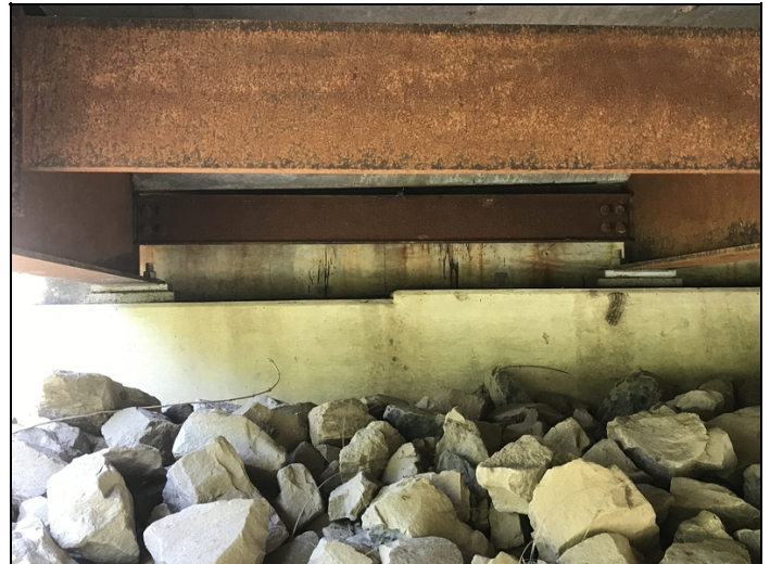
Bent # 1 bearings have been painted in the past with active corrosion under the paint.
