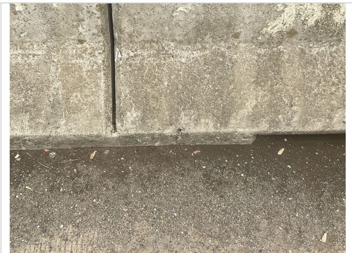
Minor spall in the base of the Left parapet.
