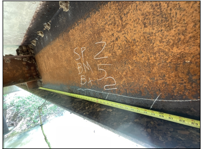
-Span # 2. Bent # 2. Beam # 5 bottom flange measures 9/16" remaining section adjacent to the bearing. The remaining base of web and bottom flange has active corrosion with initial section loss.
