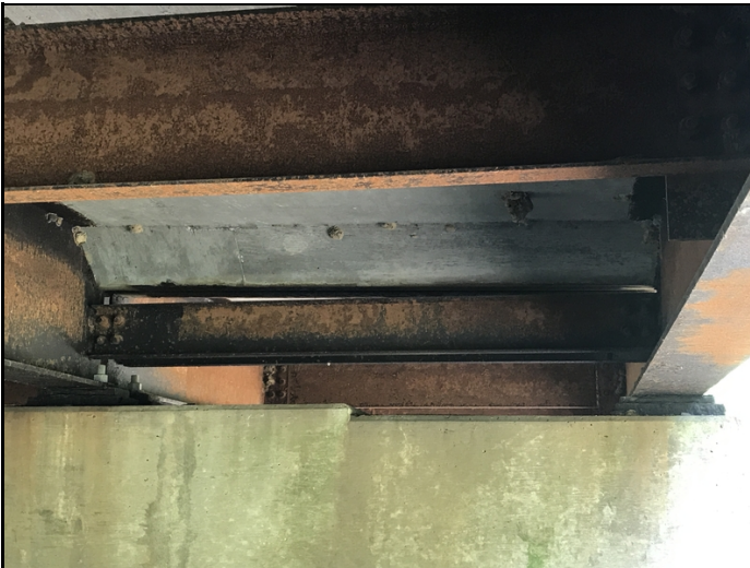
Bearings have layers of flaking rust that is causing section loss.
