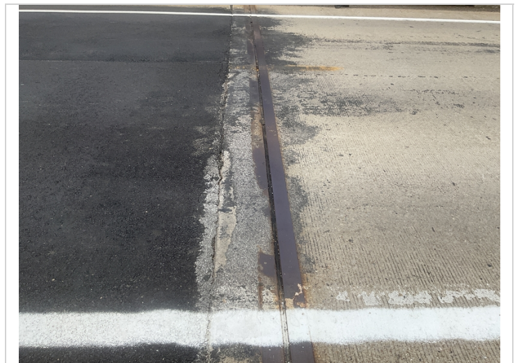
Bent # 1 expansion joint seal.
