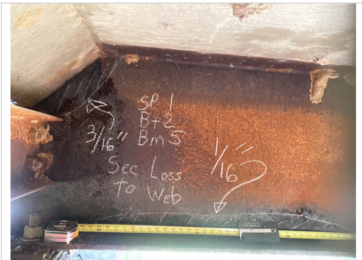
Span # 1. Bent # 2. Beam 5 has 3/16" section loss to the web at the expansion dam juncture. There is a 3' x 4" tall area with up to 1/16" section loss at the base of the web.
