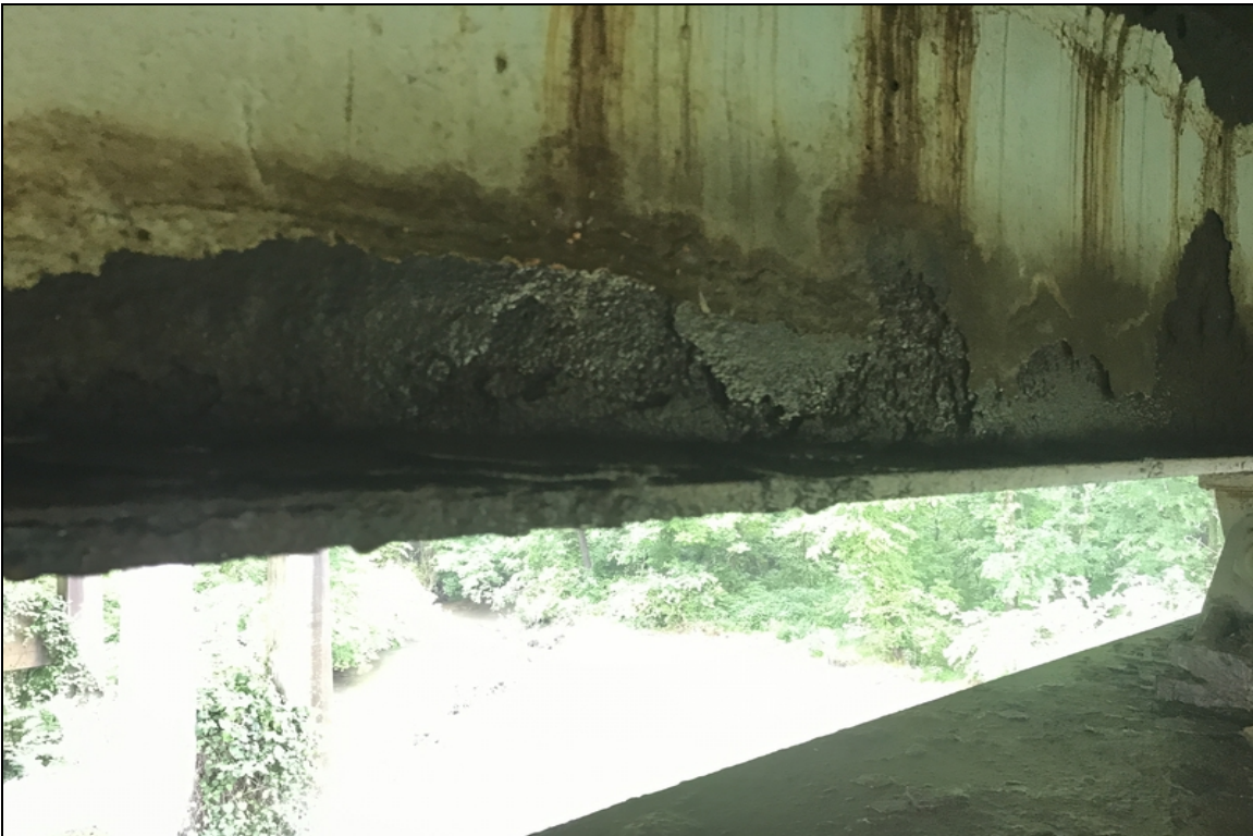
Span 1, bay 1 at bent 2-Corrosion to diaphragm.
