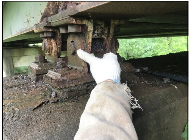
Bearing # 1 of span # 3 over bent # 4 is missing the bearing pin retaining nut.
