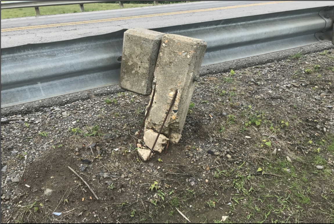
Post # 3 of the Southwest approach railing is broken at the base.
