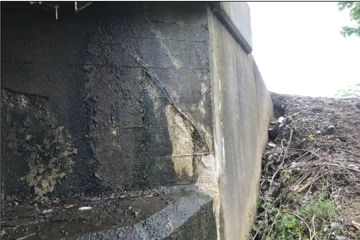
Abutment # 1, left side-Diagonal cracking with efflorescence.
