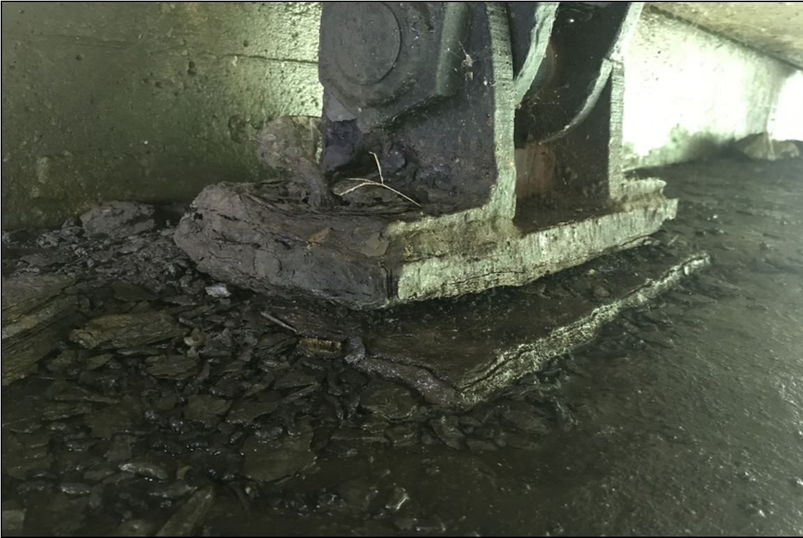
Abutment 1, bearing # 4-Heavy corrosion.
