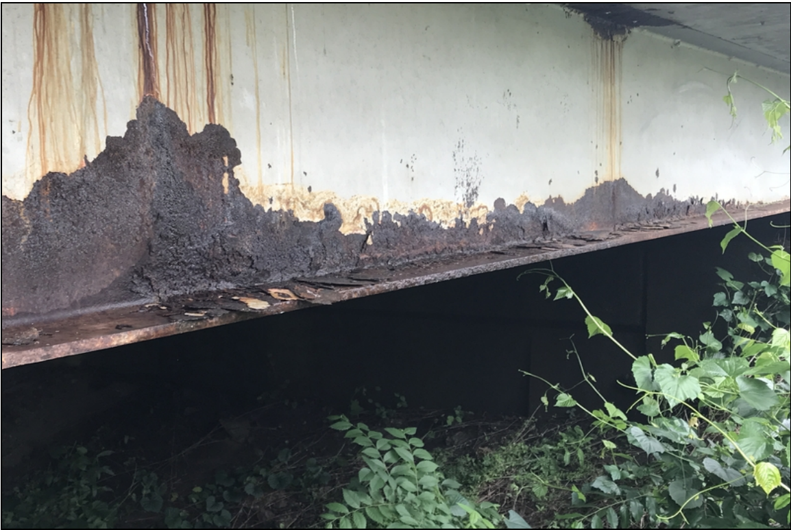
Span # 6, beam # 5-Corroaion.
