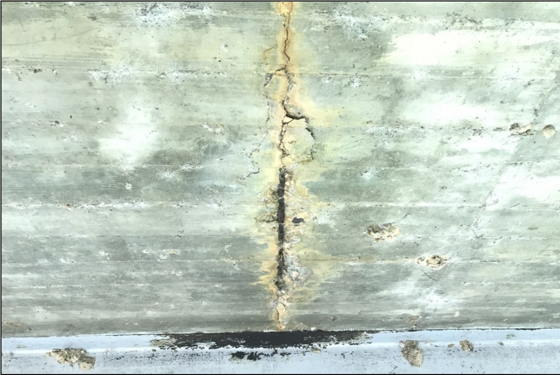
Span # 3, bay # 1-Spalling with exposed reinforcing steel.
