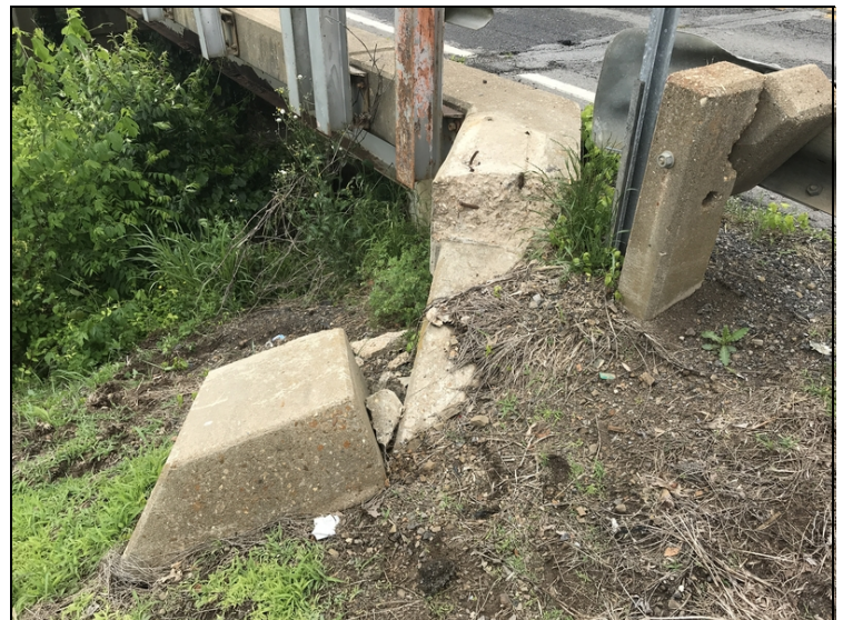
Collision damage has displaced the Southeast end post. The end post is lying on the embankment.
