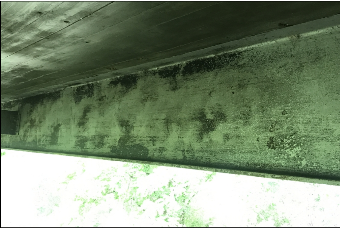
Paint system peeling.
