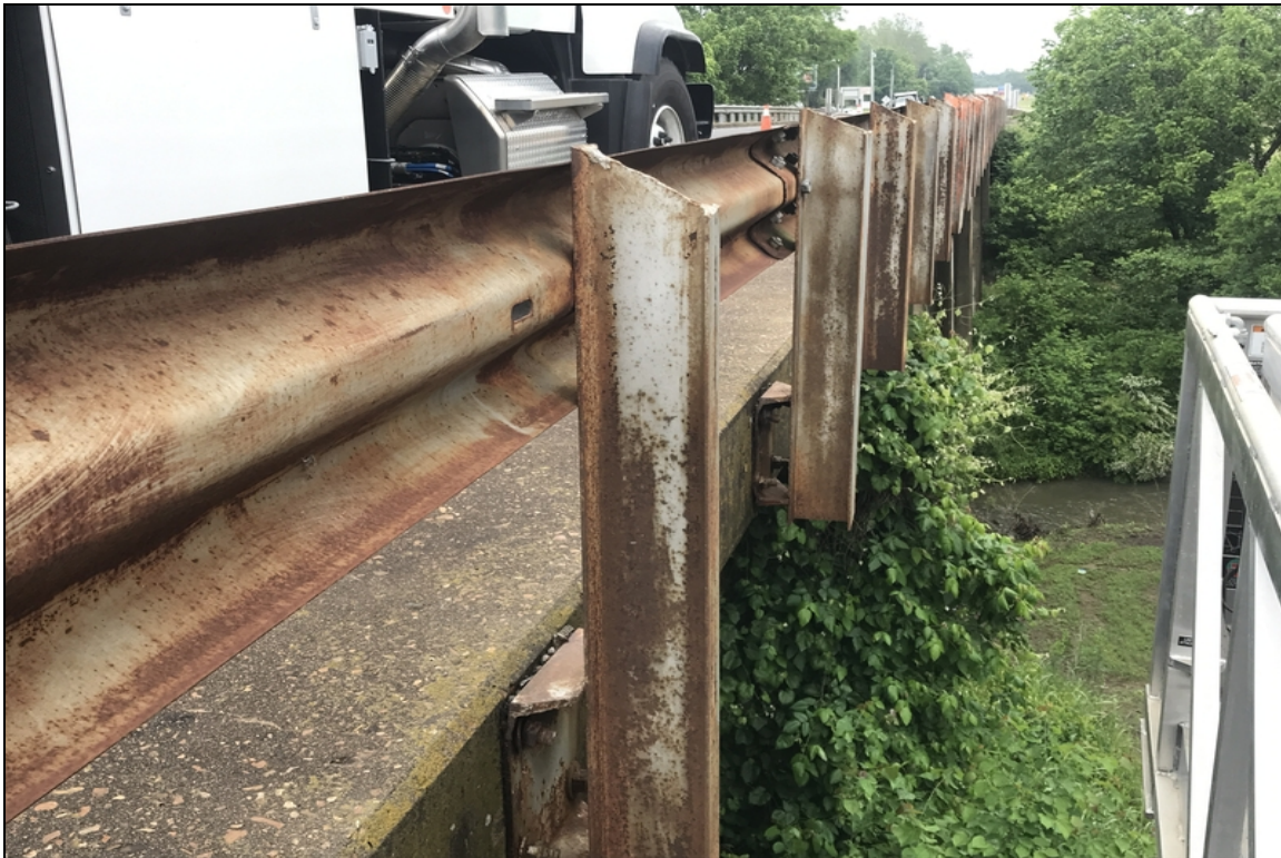
Bridge railing has rust coating.
