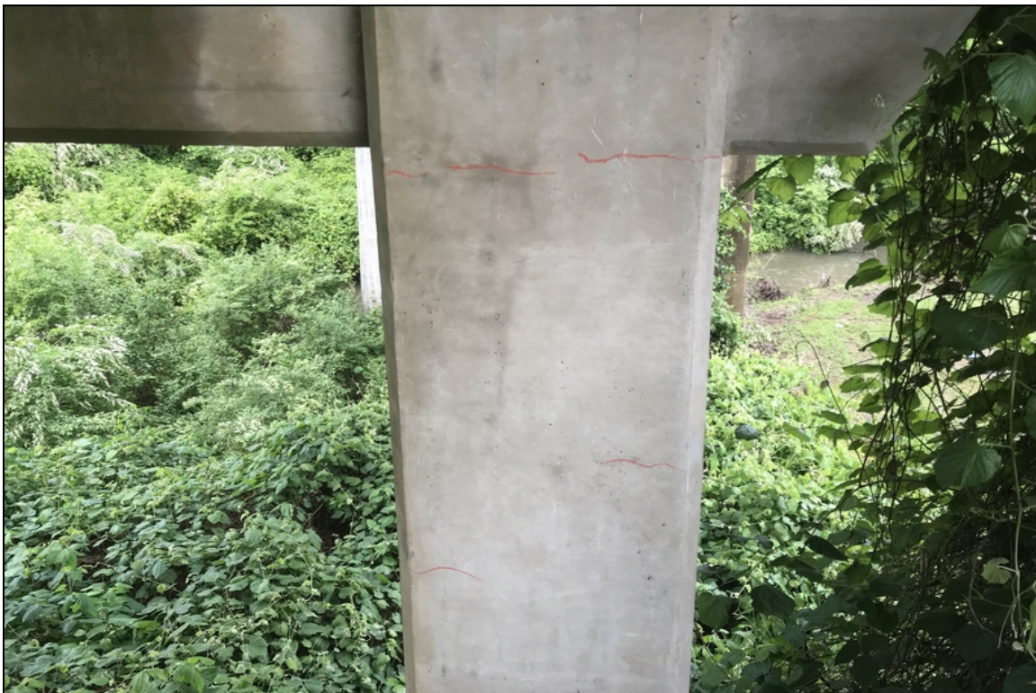
Bent 2, column 2-Hairline horizontal cracks.
