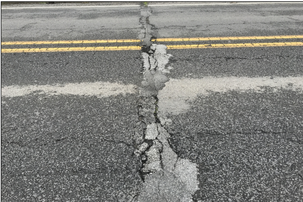
Asphalt breaking apart over intermediate bents.
