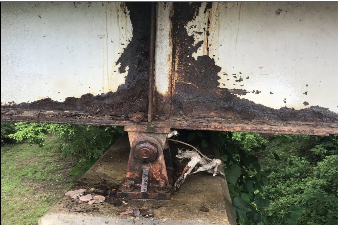
Beam 5 over bent 6-Corrosion.
