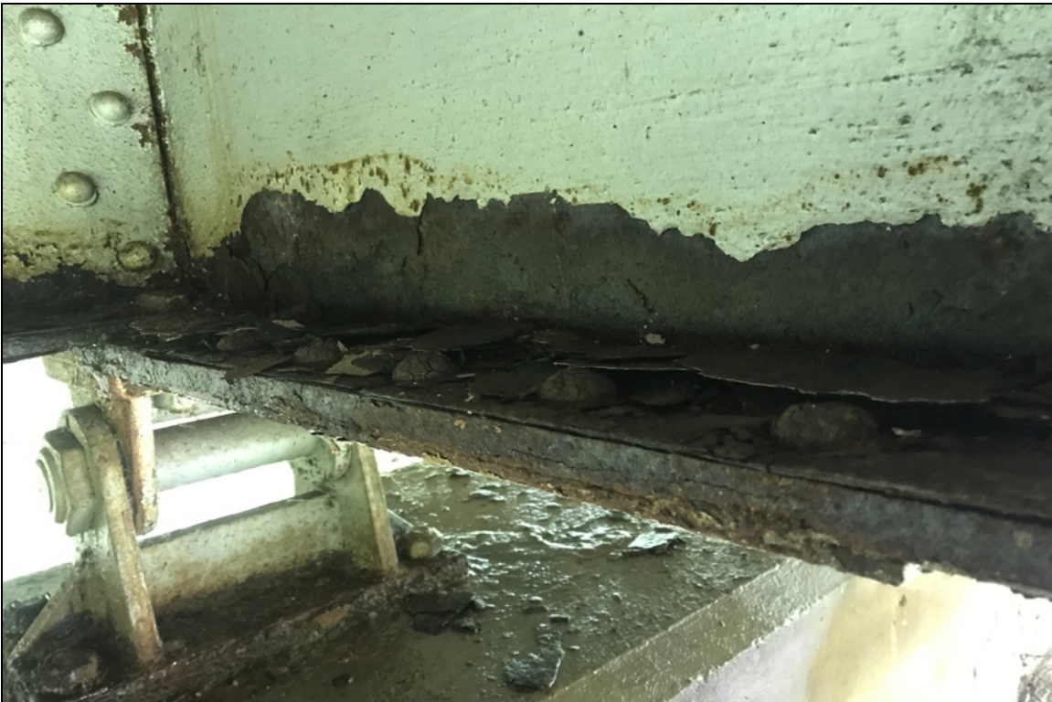
Span 5, beam 3-Corrosion.
