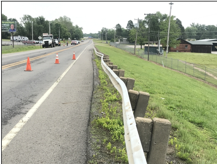
Collision damage to Southeast approach railing.
