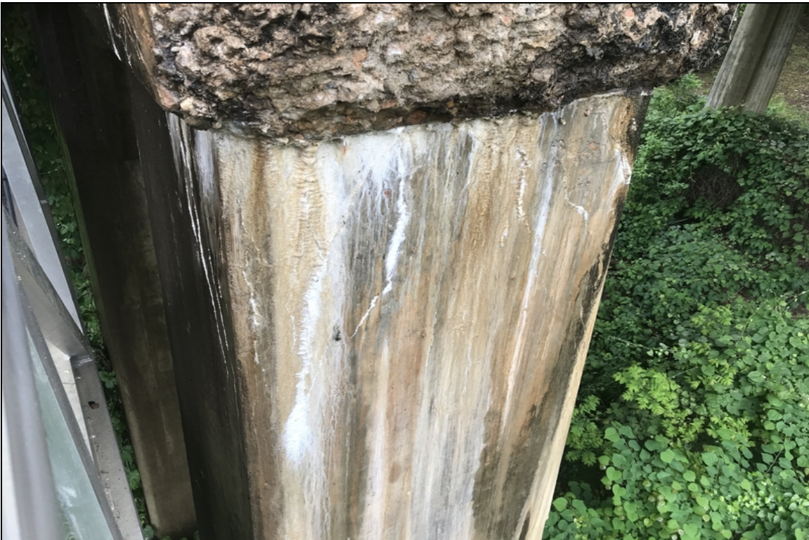
The upper portion of column # 3 of bent # 4 has mapcracking with efflorescence.
