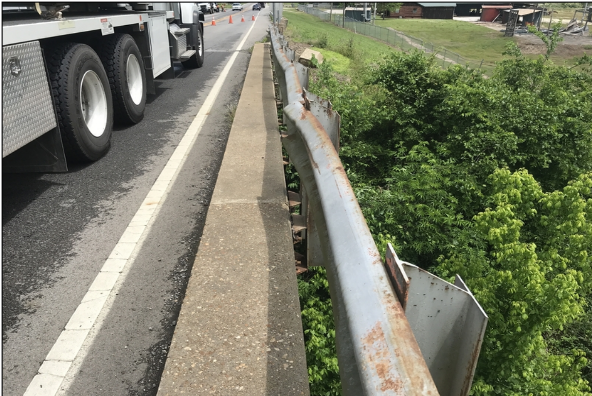
Right bridge railing-Minor collision damage to railing.
