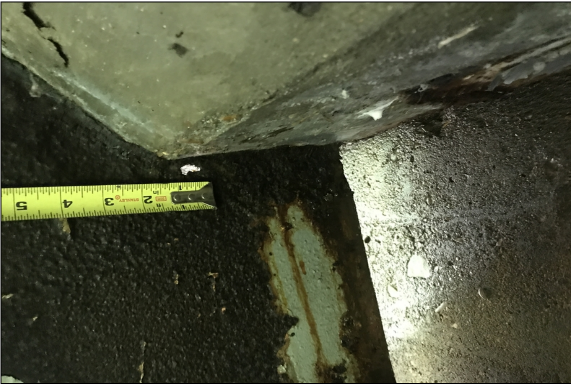
Span # 6, beam # 1 over abutment # 2-Hole rusted through web at expansion dam.
