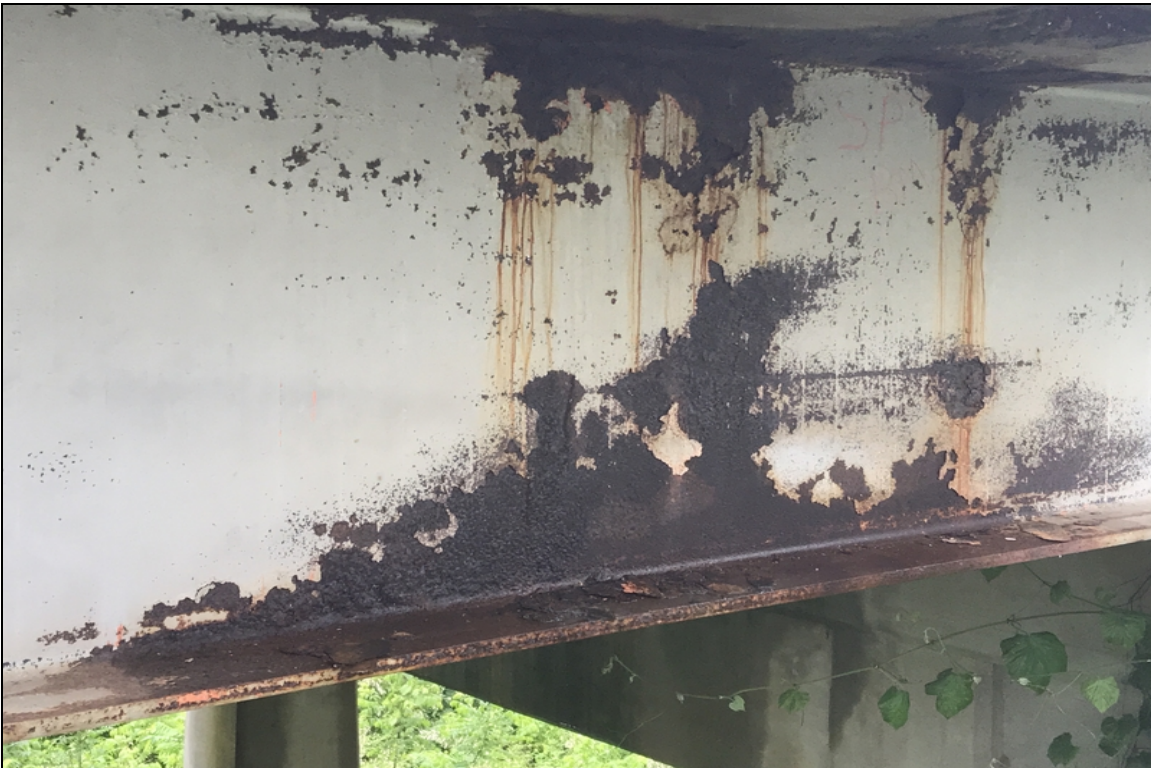
Span 1, beam 5-Corrosion where deck drain discharges water on beam.
