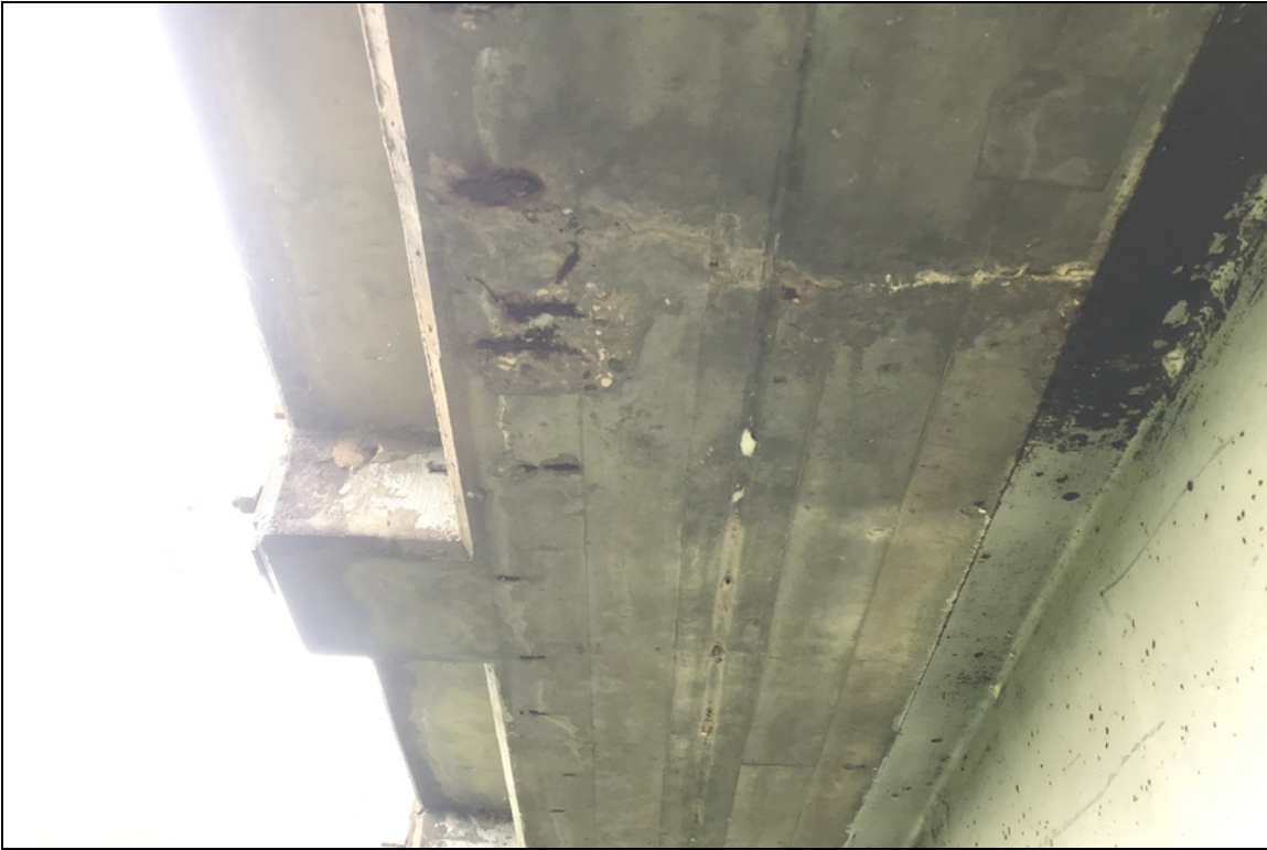
Span 2, left side-Spalling with exposed reinforcing steel in deck overhang.
