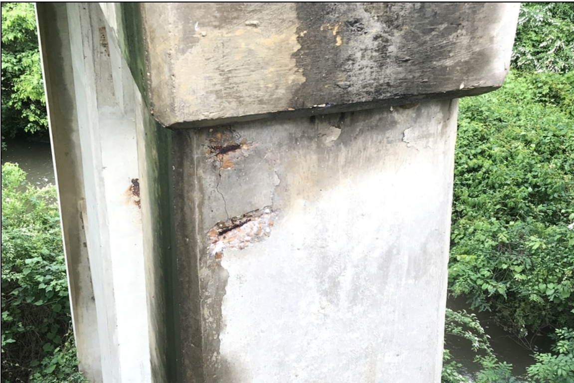
Bent # 3, column # 3 has two 4" spalls with exposed reinforcing steel near cap juncture.
