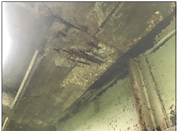
Left deck overhang, span 5 over bent 5-Spalling with exposed reinforcing steel.
