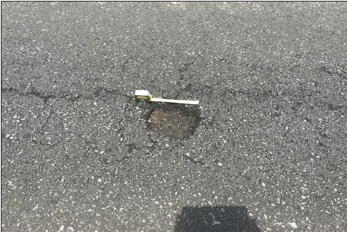
The right lane of span # 2 has an 8" spall in the asphalt driving surface.
