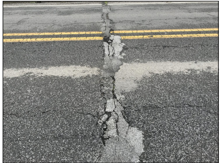
Asphalt breaking apart at expansion joints.
