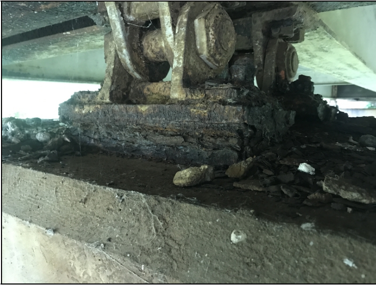
Typical of movable bearings over bent 4.
