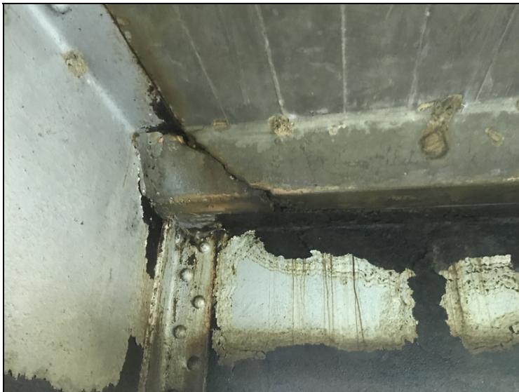
The expansion dams have delaminated and spalled areas with wide cracking adjacent to the beams.
