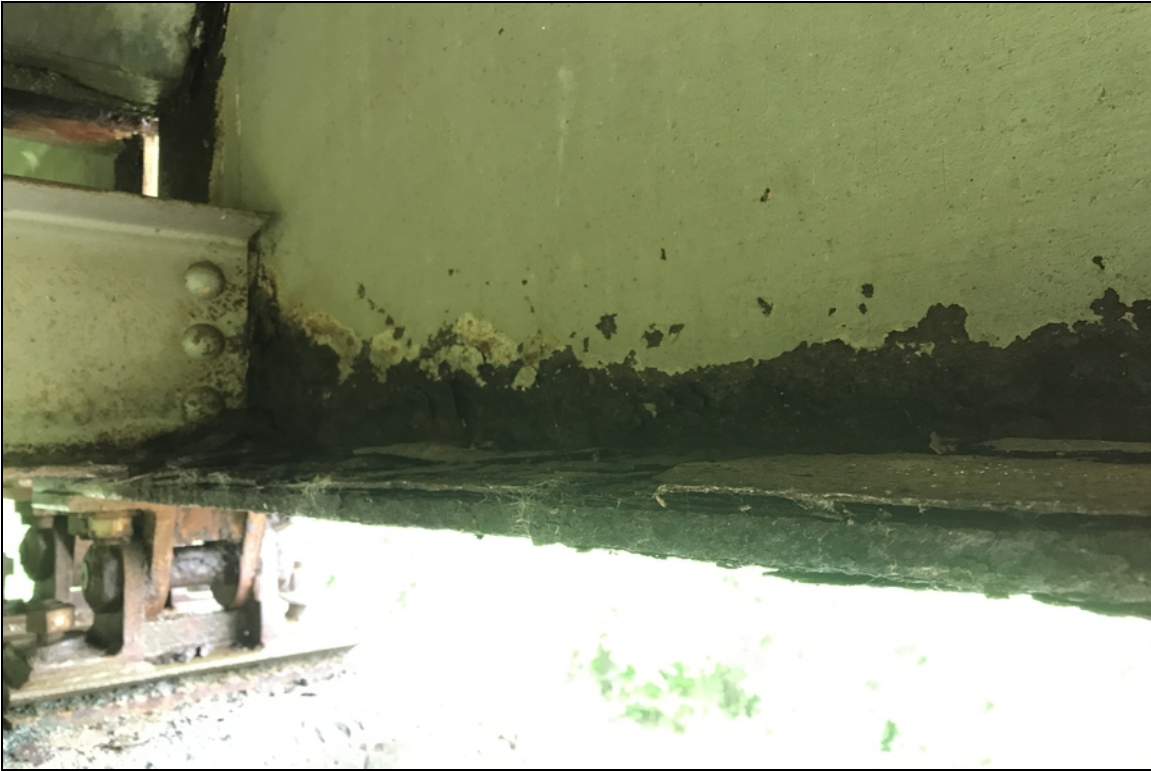
Span 3, beam 5 at bent 4-Corrosion.
