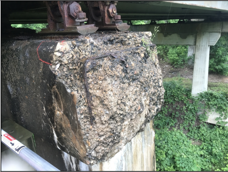
Bent # 4 cap-Concrete deterioration / spalling.
