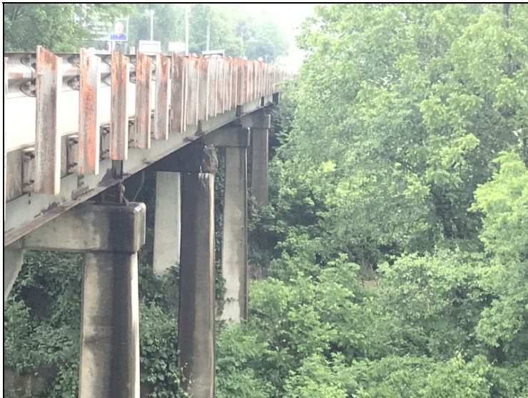
The bridge railing posts have active corrosion in the lower connections to the deck.
