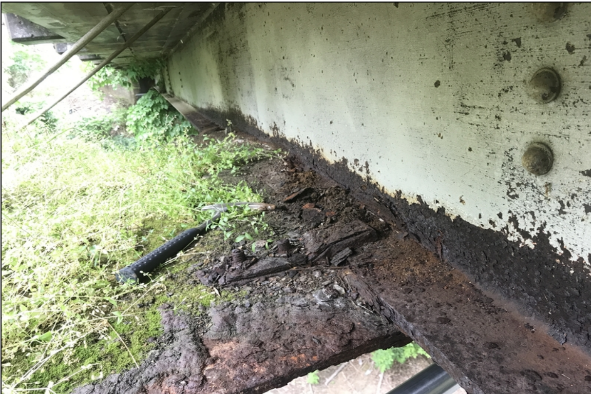
Span 5, beam 1-Heavy corrosion where steel plate is attached To bottom of beams.
