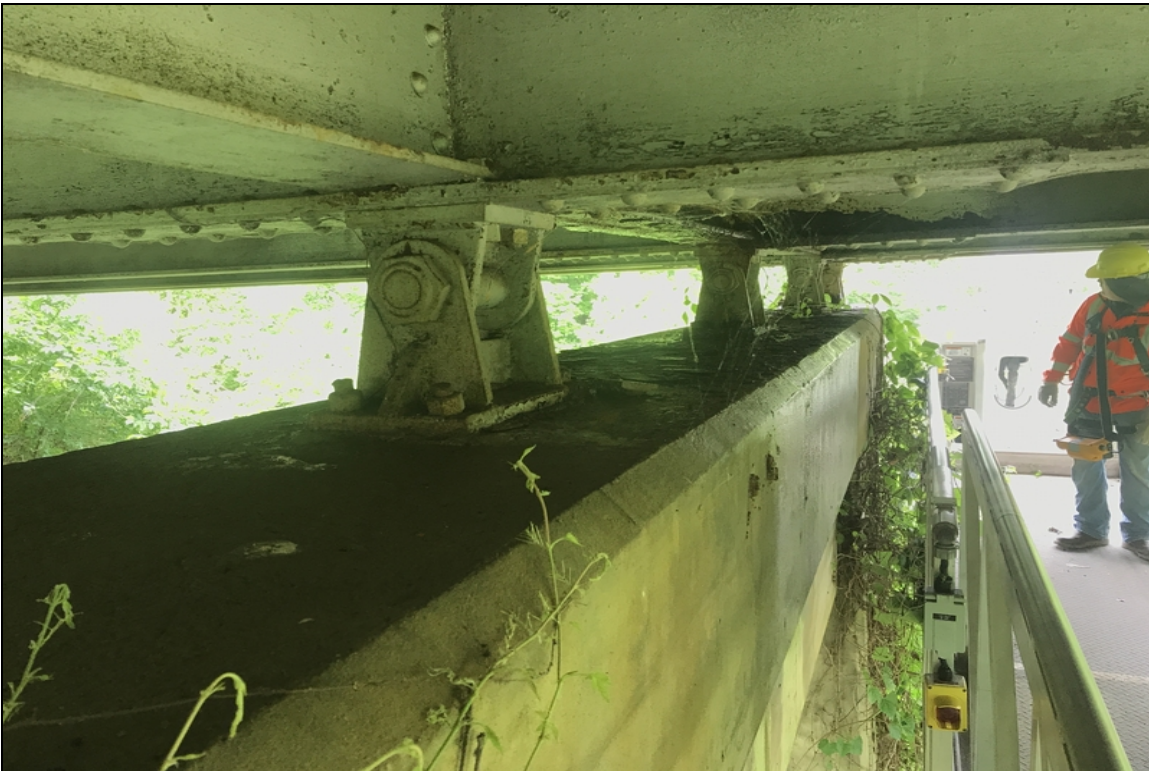
Bent 6 bearing area.
