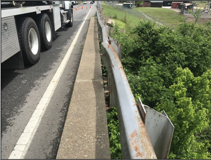
Right bridge railing-Minor collision damage to railing.
