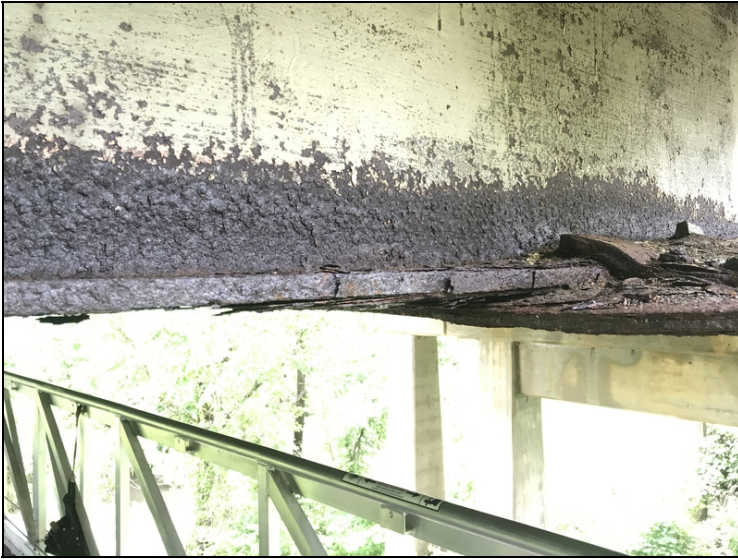
Span 5, beam 1-Corrosion to bottom flange where steel plate is attached.
