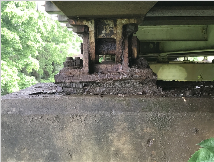
Span 3, bearing 1 over bent 4-Corrosion.
