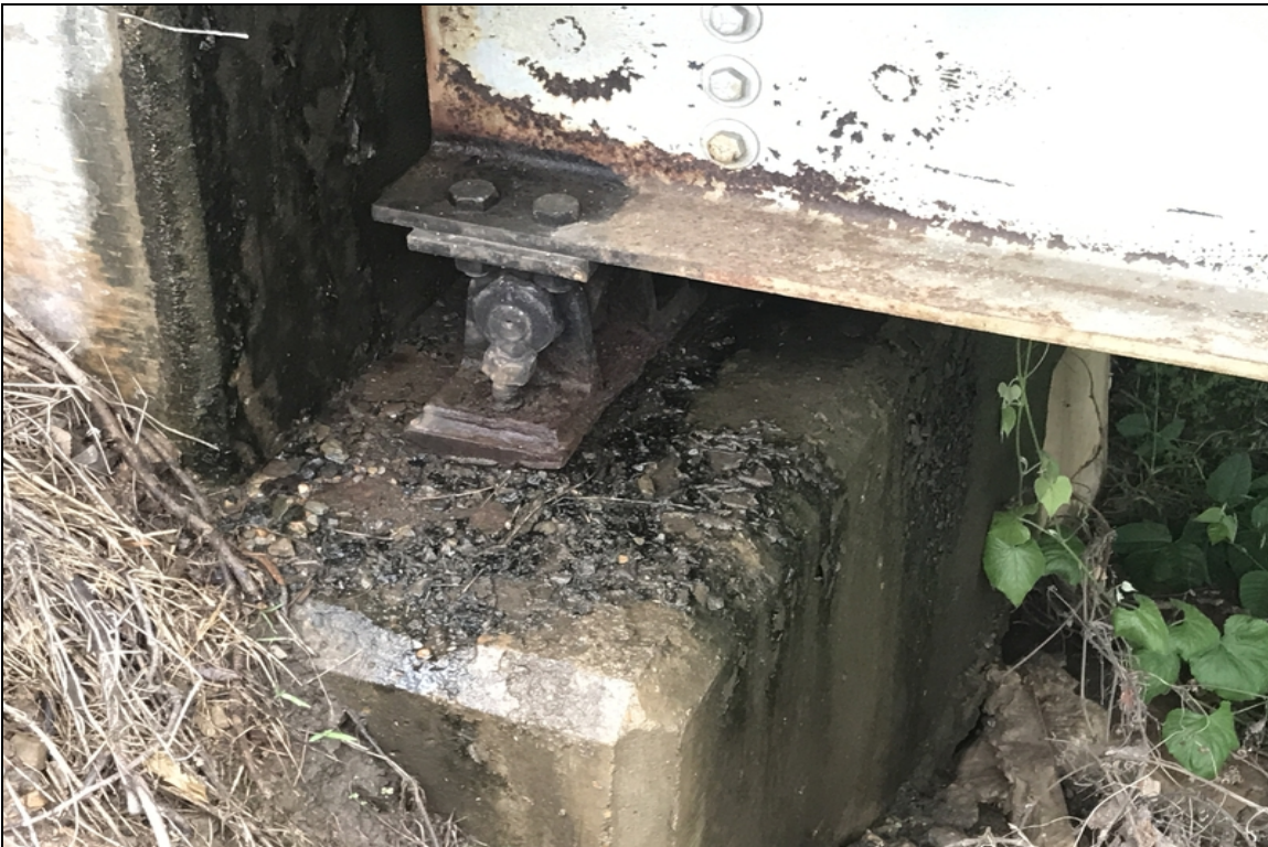
Abutment 1, bearing 5-Corrosion.
