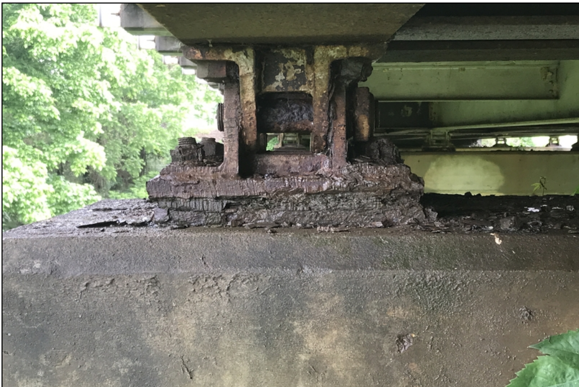
Span 3, bearing 1 over bent 4-Corrosion.
