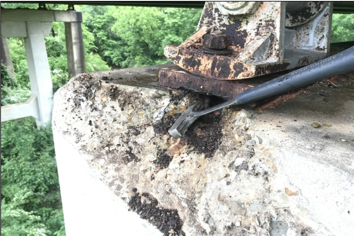
The left end of bent # 2 cap has a 20" x 8" spall that has caused approximately 3" of bearing area loss under the exterior bearing. The bearing anchor bolt is exposed and has approximately 60% section loss.
