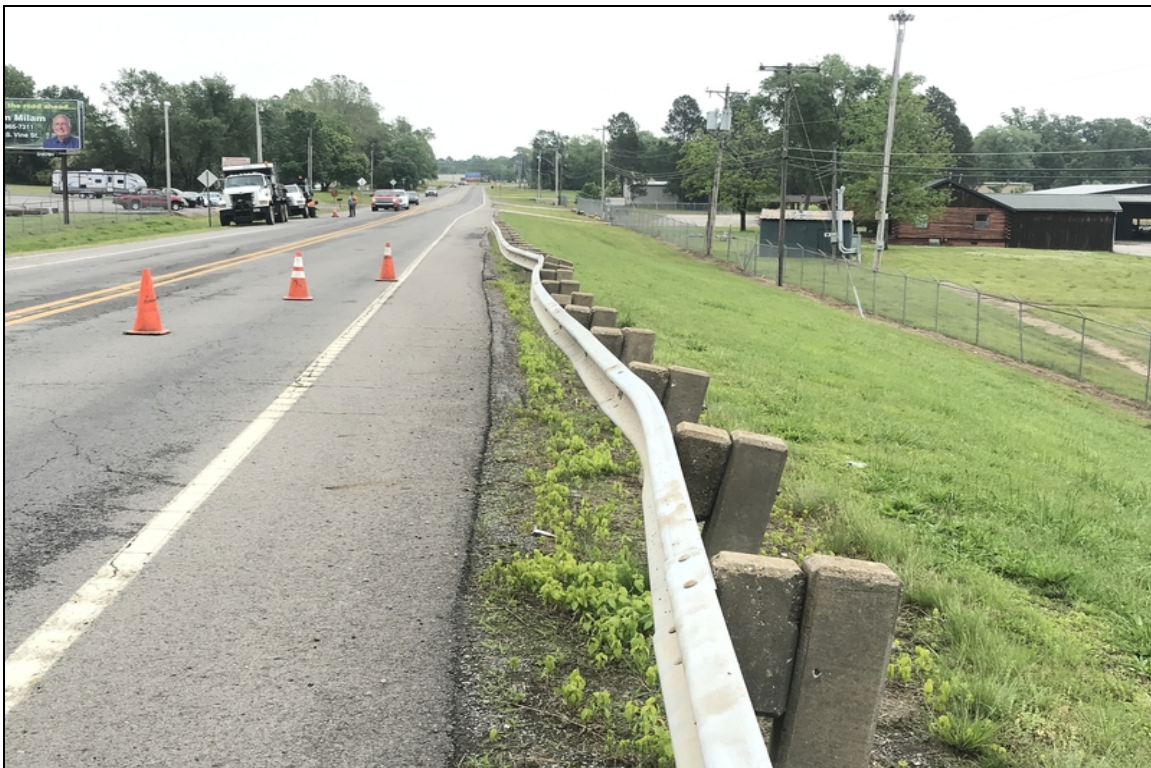
Collision damage to Southeast approach railing.
