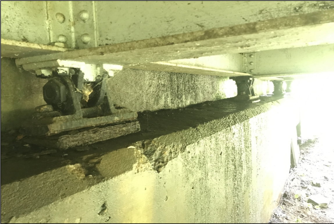
Abutment 2 bearing area.
