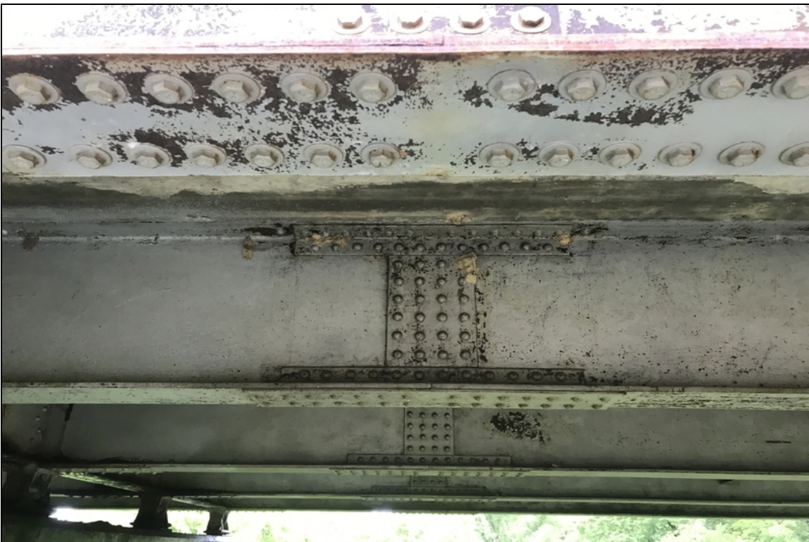
Span 2-General view of splice plate connections.
