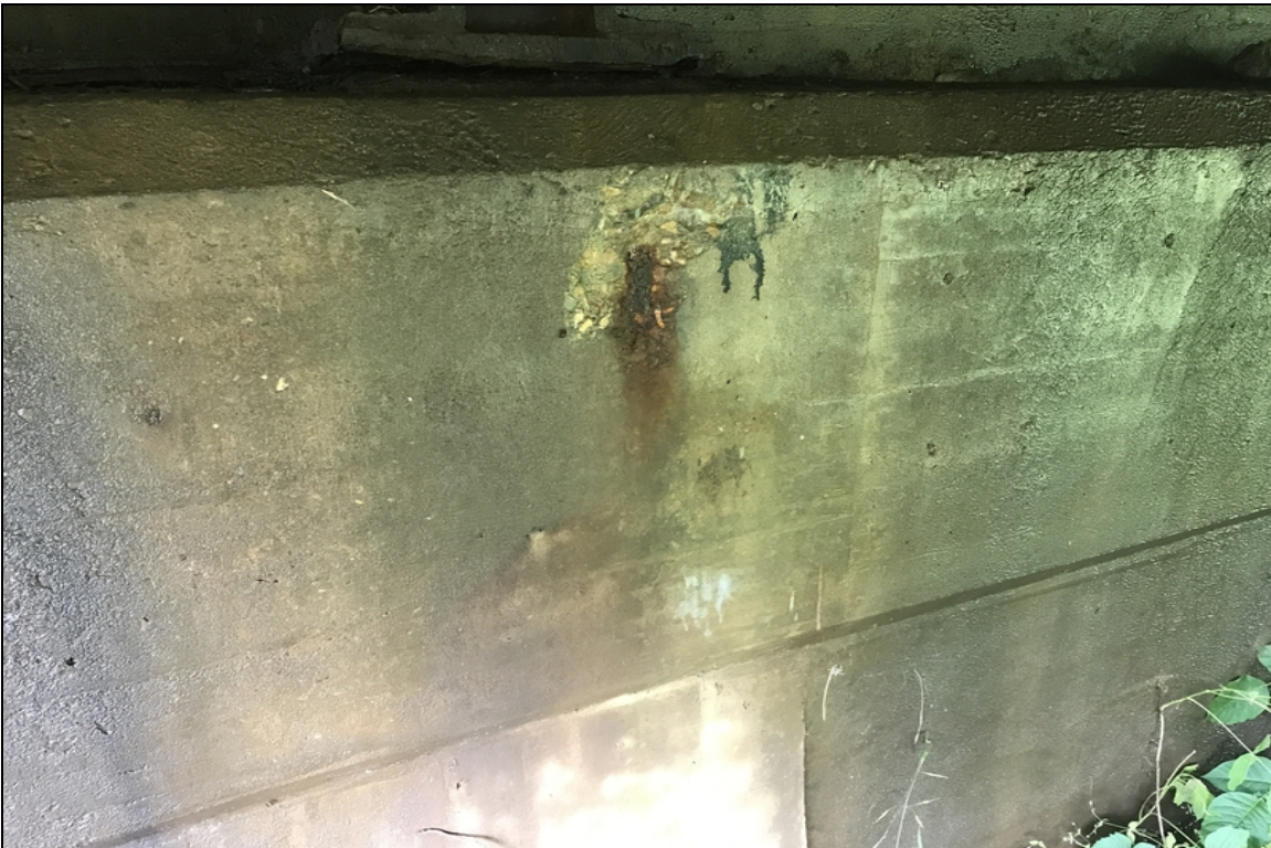
Abutment # 2-Spall with exposed reinforcing steel.
