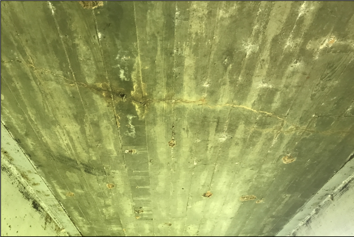
Span 4-Transverse cracking with light efflorescence.
