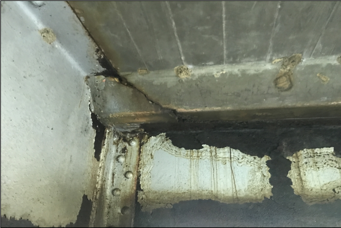
The expansion dams have delaminated areas with wide cracking adjacent to the beams.
