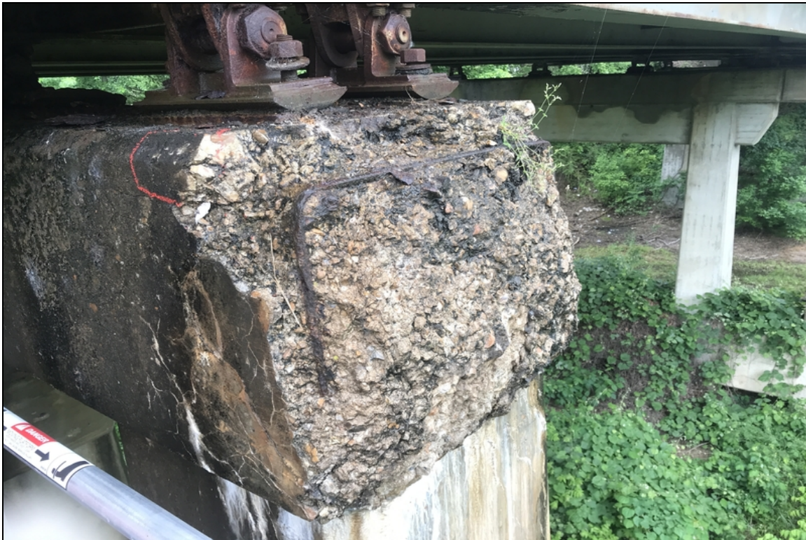
Bent # 4 cap-Concrete deterioration / spalling.
