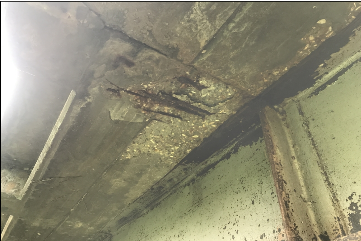
Left deck overhang, span 5 over bent 5-Spalling with exposed reinforcing steel.
