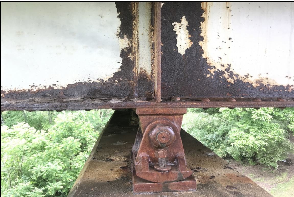
Beam 5 over bent 5-Corrosion.
