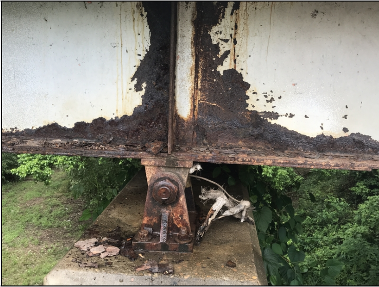
Beam 5 over bent 6-Corrosion.
