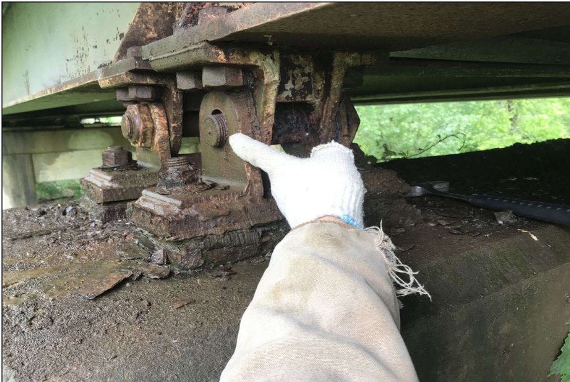
Bearing # 1 of span # 3 over bent # 4 is missing the bearing pin retaining nut.
