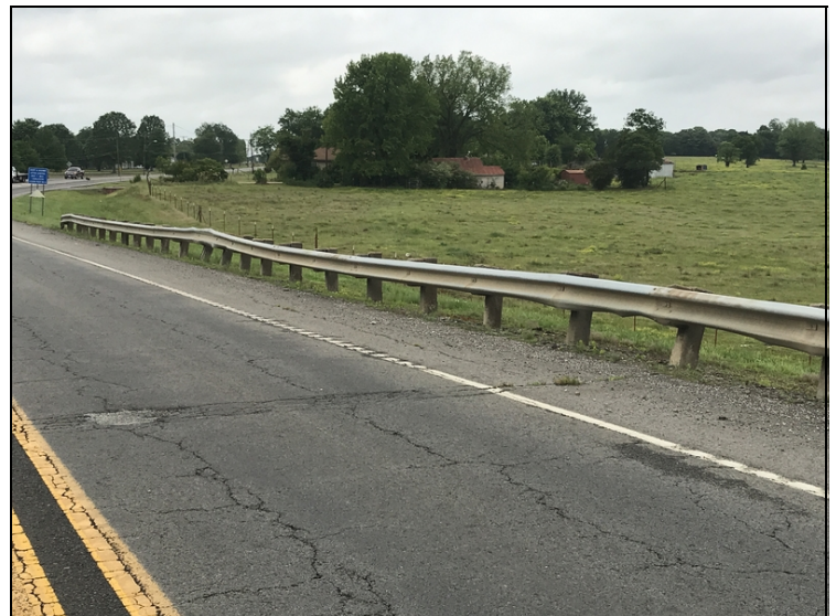
Collision damage to the Northwest approach railing.
