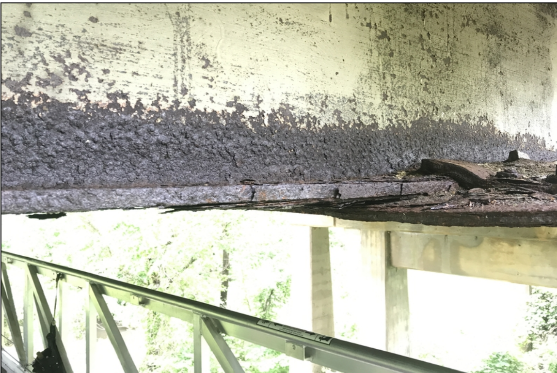
Span 5, beam 1-Corrosion to bottom flange where steel plate is attached.
