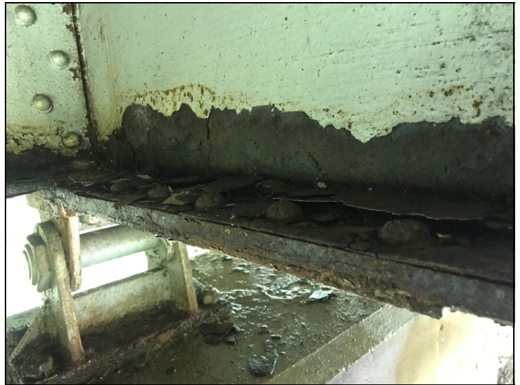
Span 5, beam 3-Corrosion.
