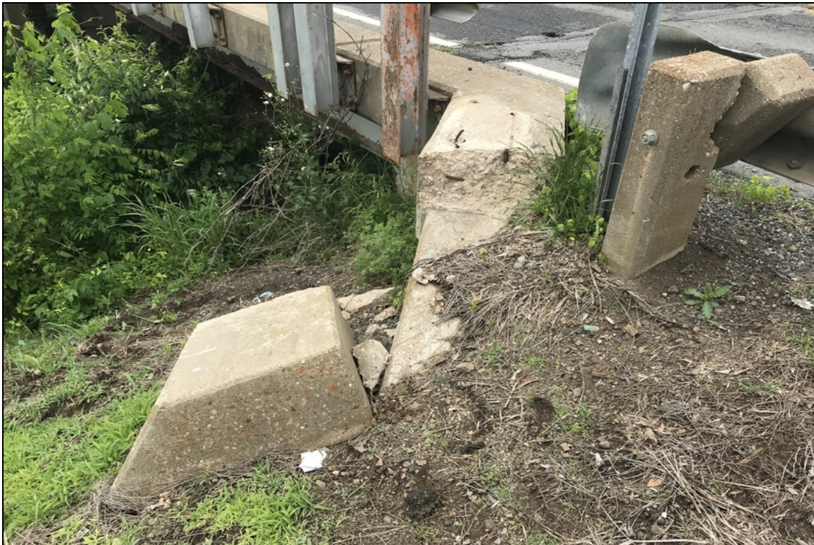
Southeast end post has been displaced.
