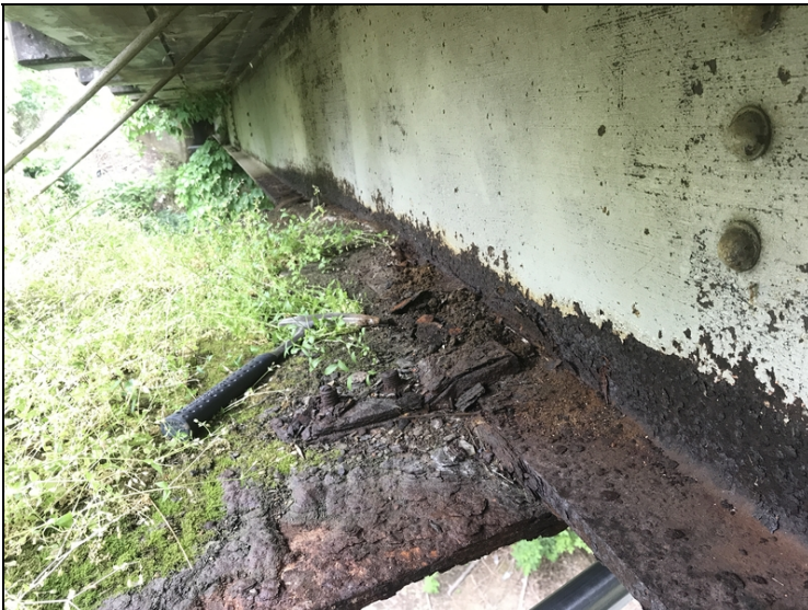
Span 5, beam 1-Heavy corrosion where steel plate is attached To bottom of beams.
