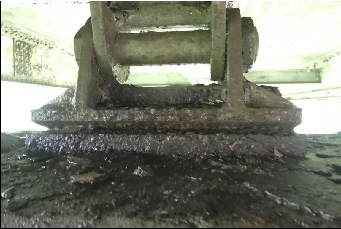
Bent 2, bearing 2-Corrosion.
