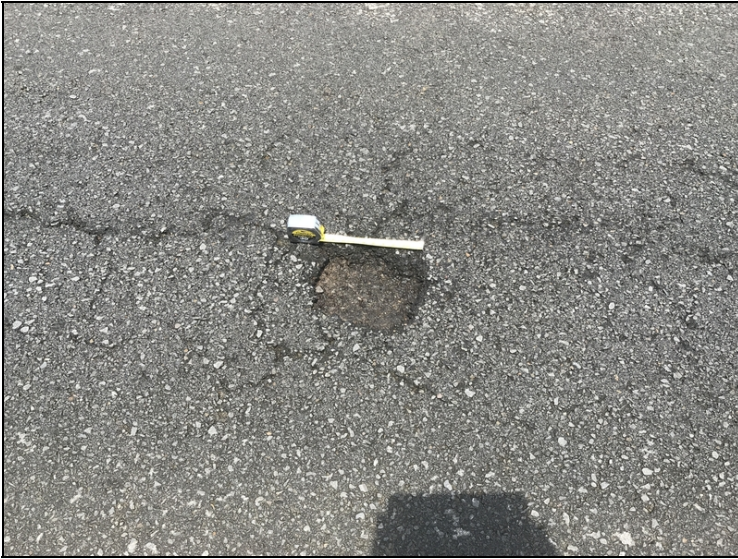
The right lane of span # 2 has an 8" spall in the asphalt driving surface.
