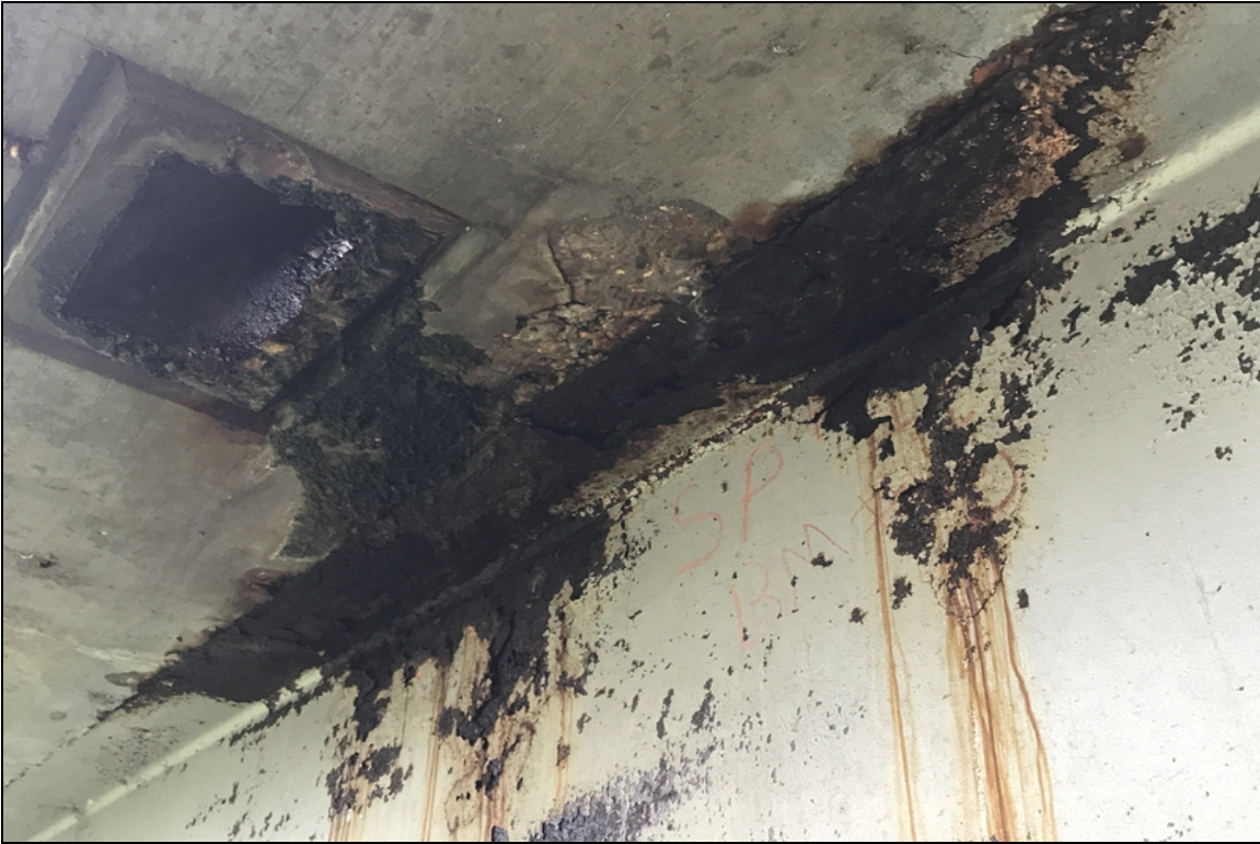
Span 1, beam 5-Corrosion section loss where deck drain discharges water.
