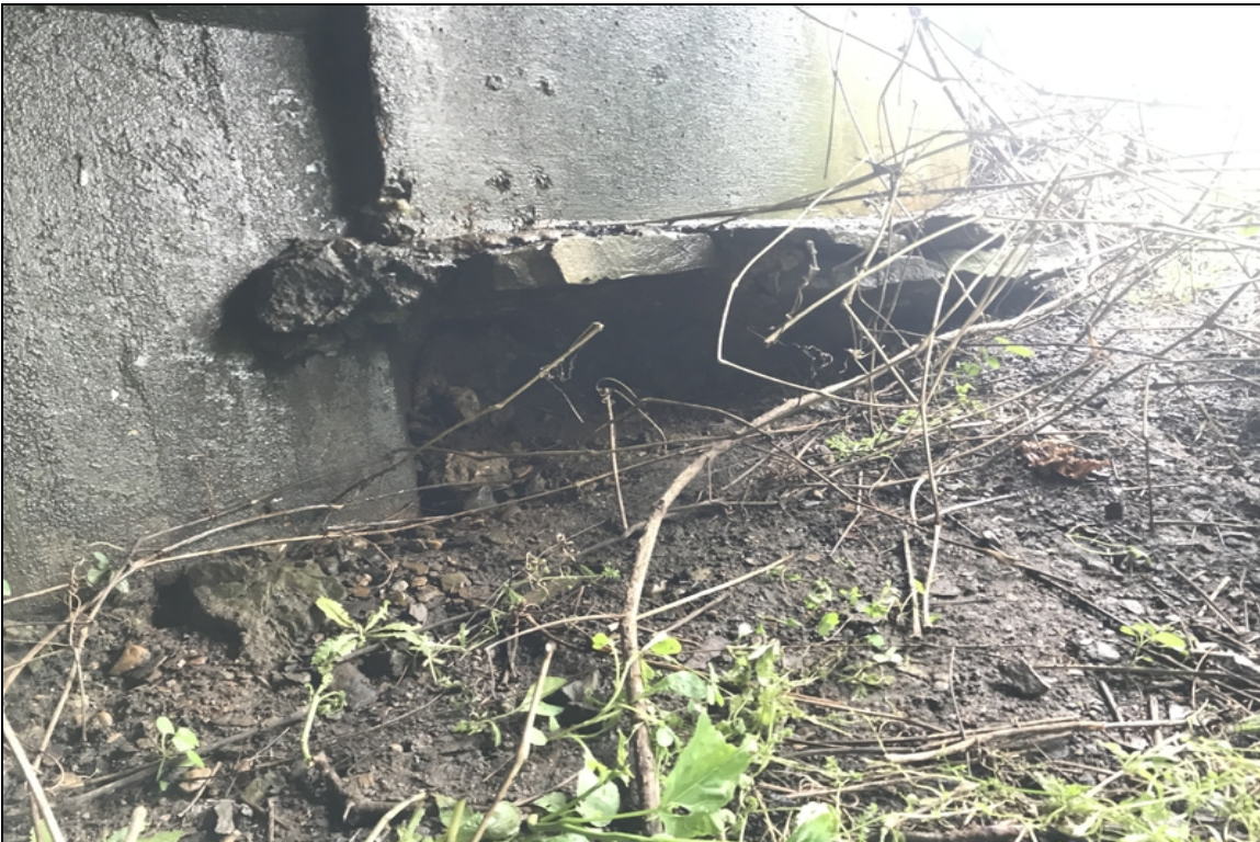
Abutment 2, right side-Minor earth settlement.
