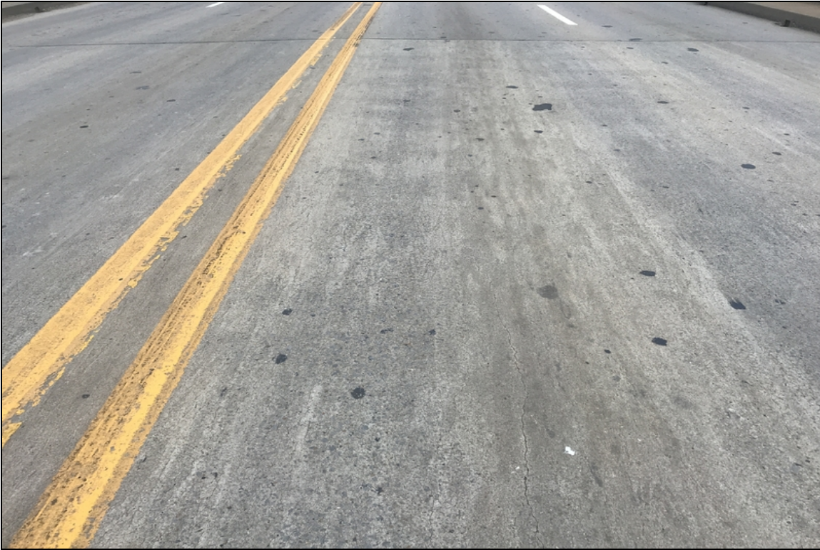
Longitudinal cracking on the driving surface of the slab.
