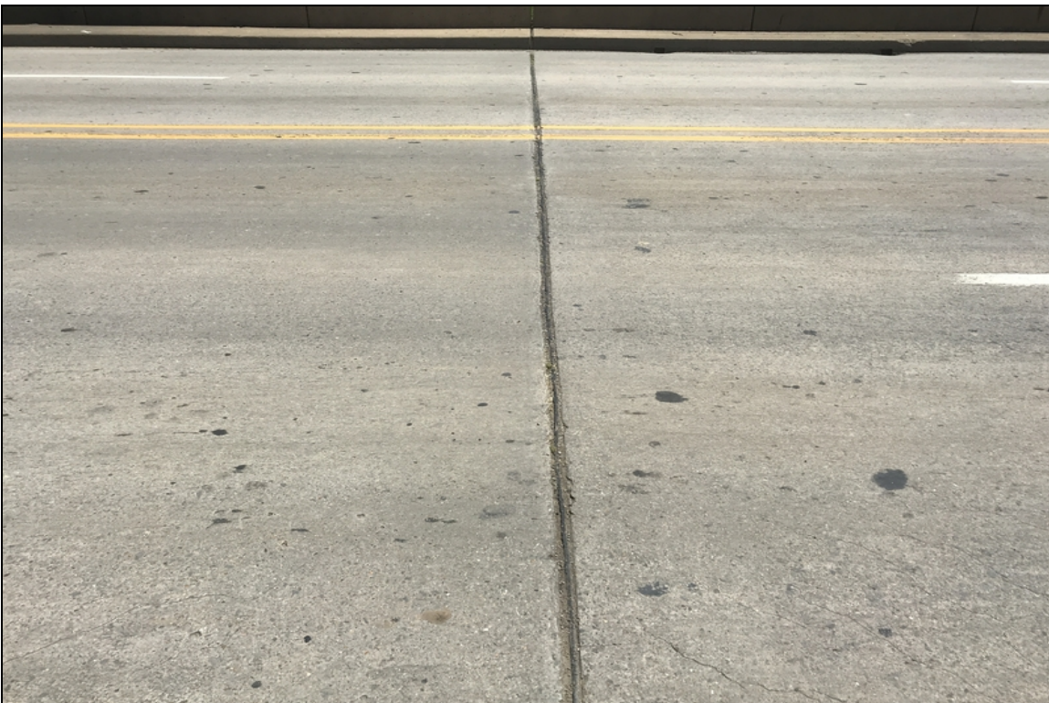
Bent # 3 joint seal deterioration with debris impaction.
