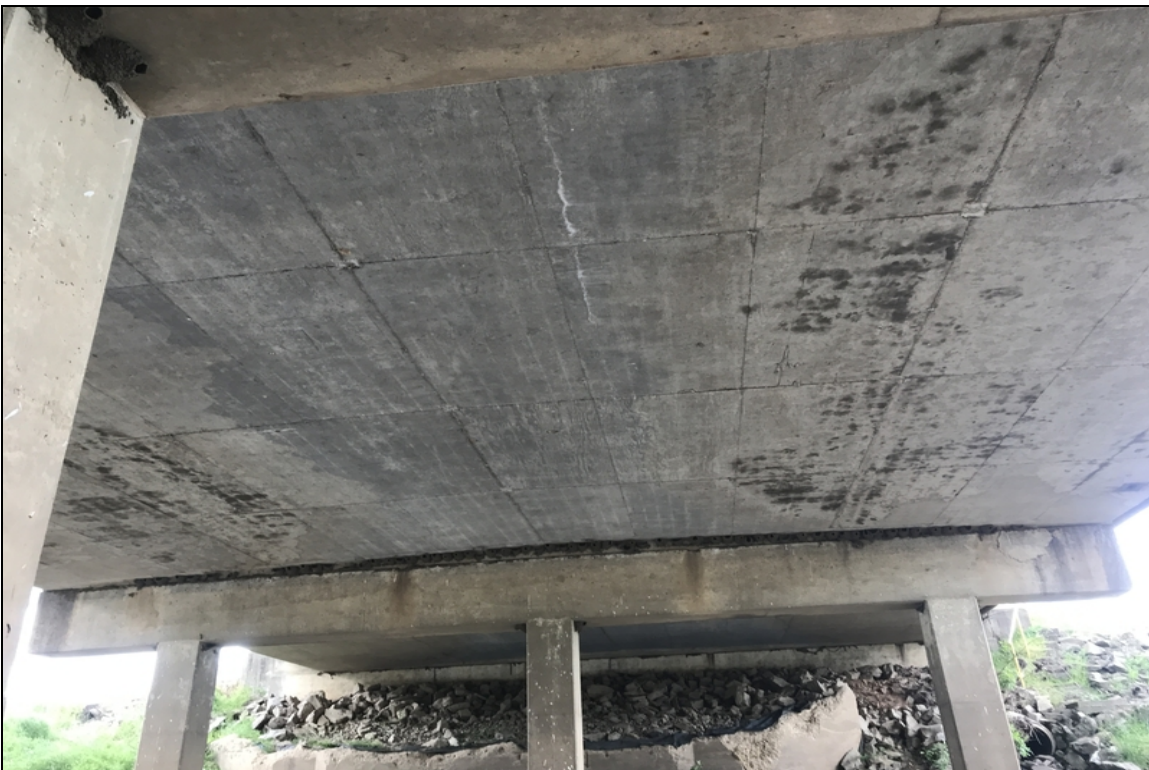
Typical undersurface of the slab.
