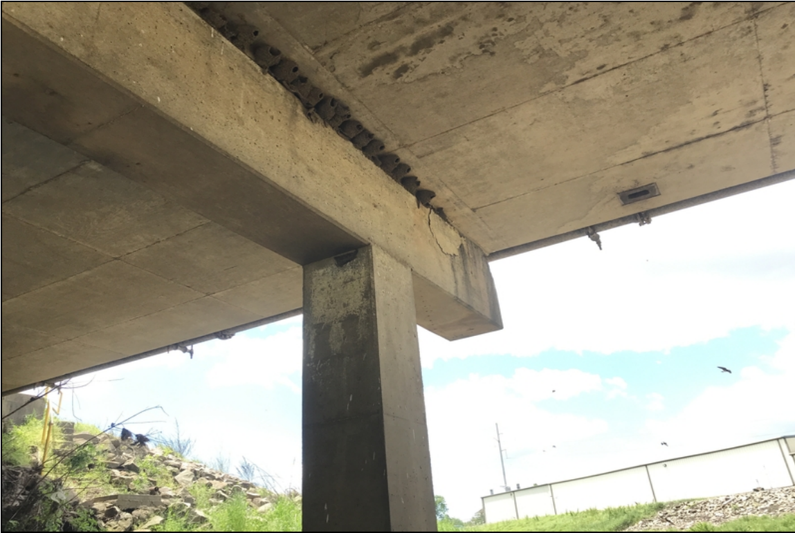
Bent # 2 Lt cap large delamination
