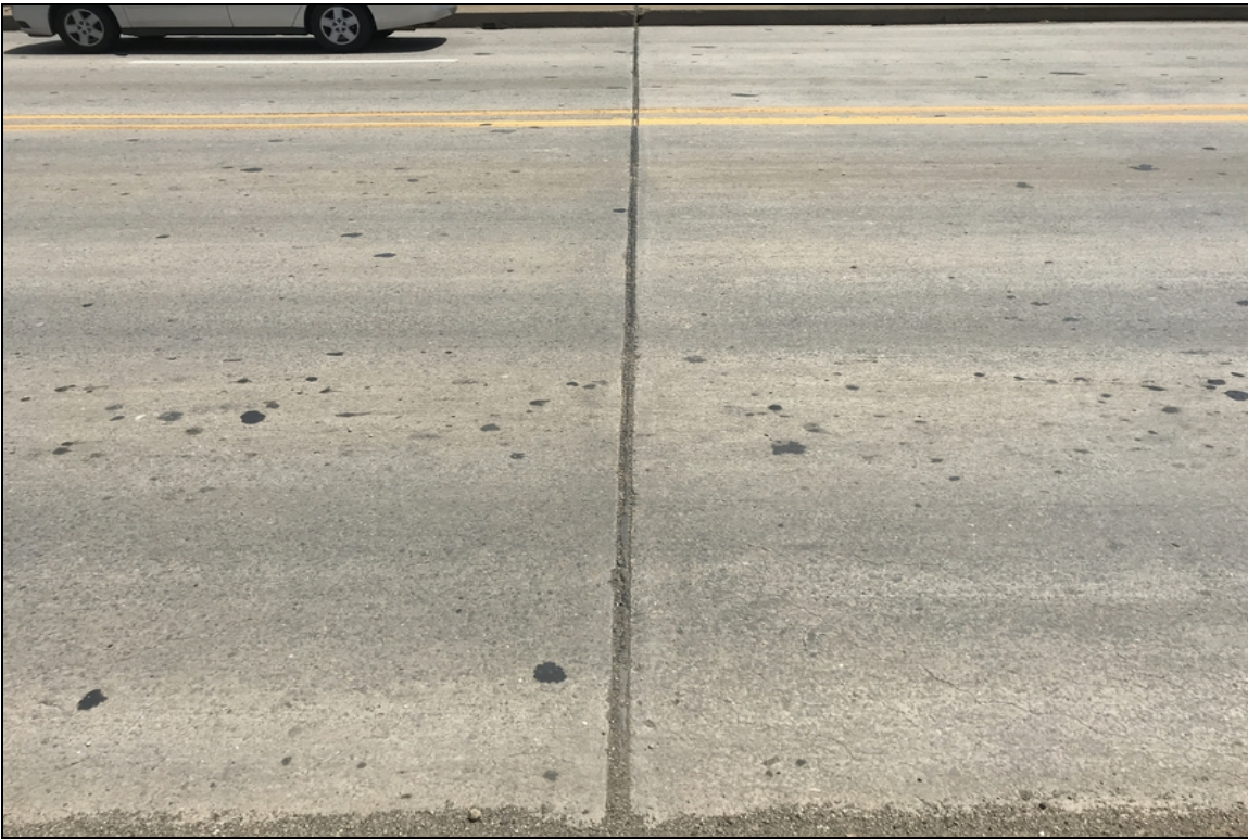
Bent # 2 joint seal with debris impaction.
