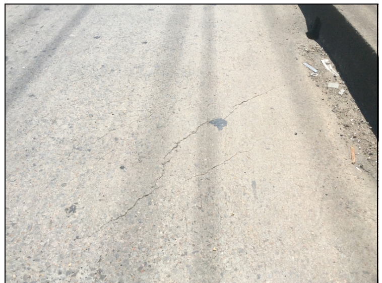
Span #2, left lane-Diagonal cracking.
