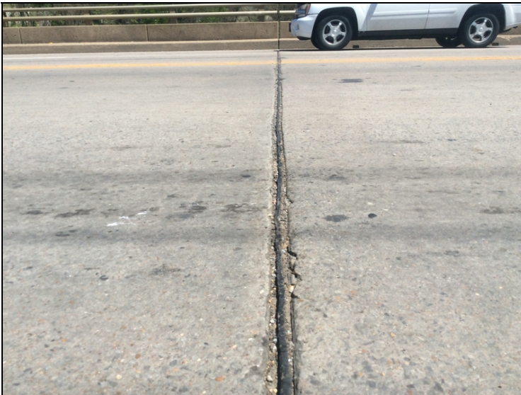
Bent #3 expansion joint-Debris impaction.
