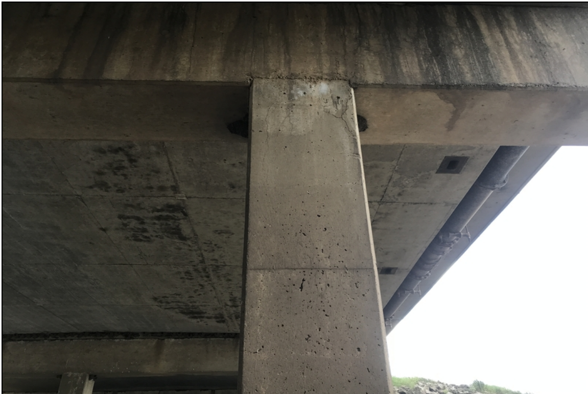
Bent # 3 Column # 1 vertical cracking at the cap juncture.
