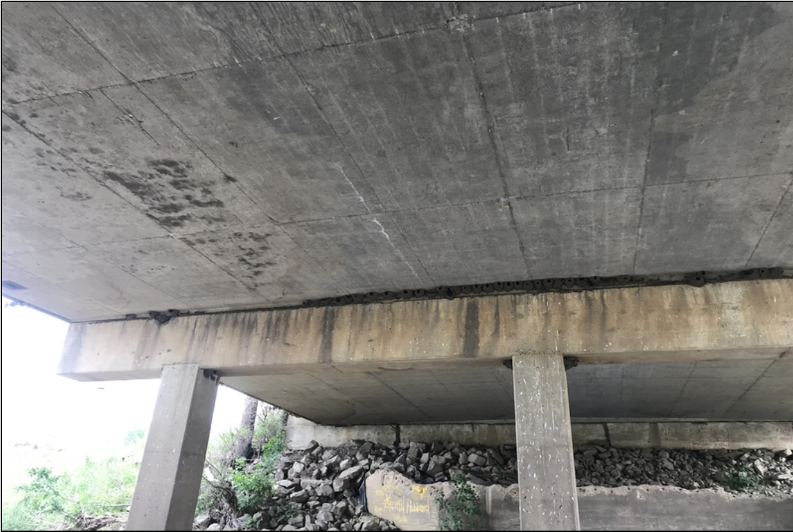
Span # 2 longitudinal cracking with light efflorescence buildup.
