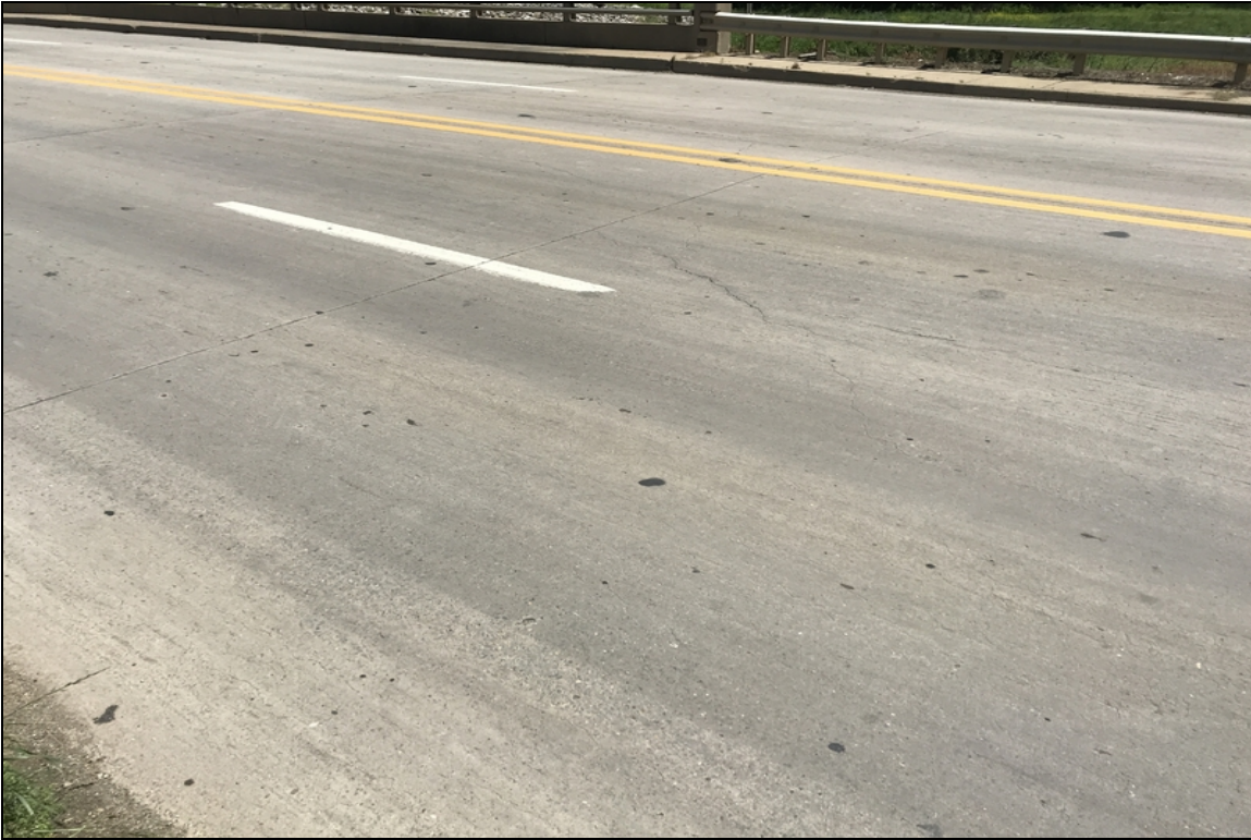
South approach slab cracking.
