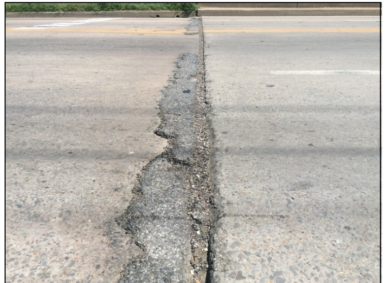
North approach slab settlement.
