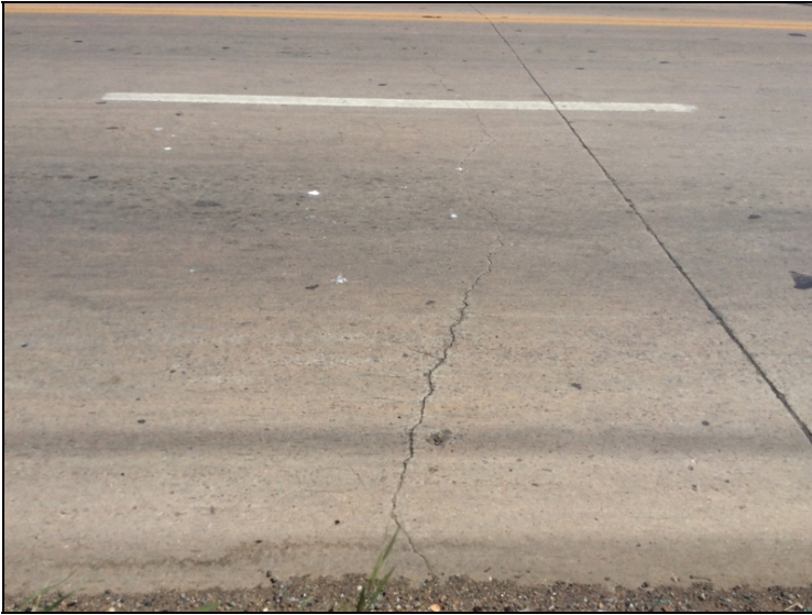
South approach slab-Transverse cracking
