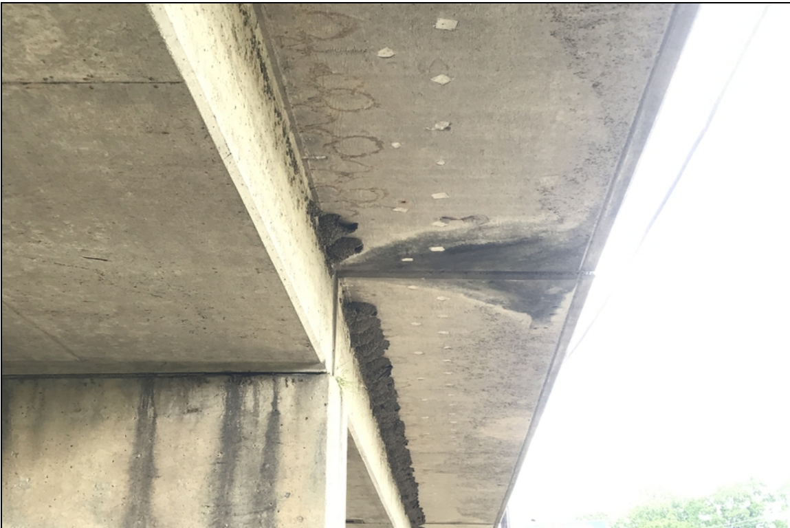
Span # 1 Rt shallow spalling with exposed reinforcing steel on the undersurface of the overhang.
