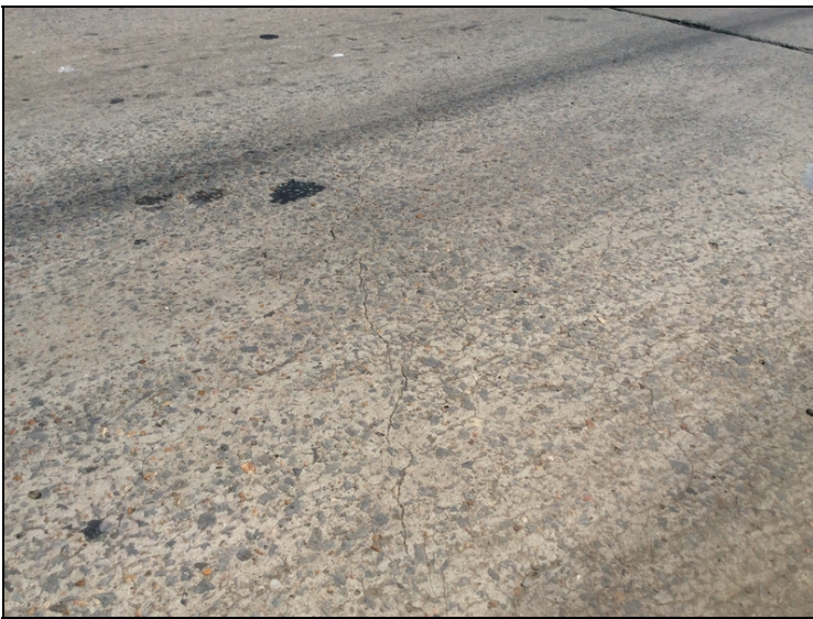
Span #1, left lane-Cracking.
