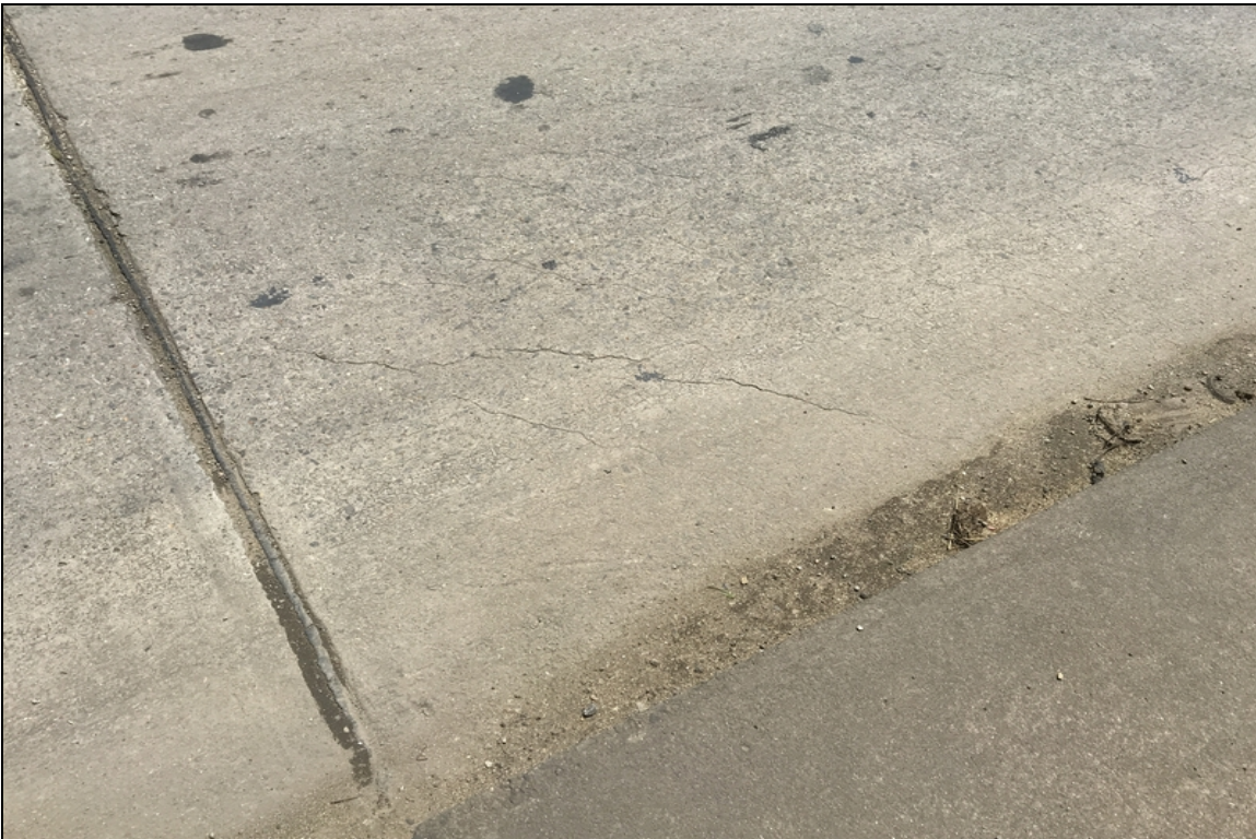
Sealable deck cracking.
