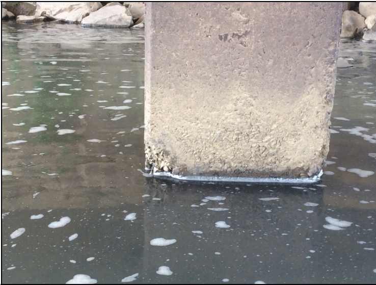
Bent #3, column #2-Concrete deterioration with section loss.
