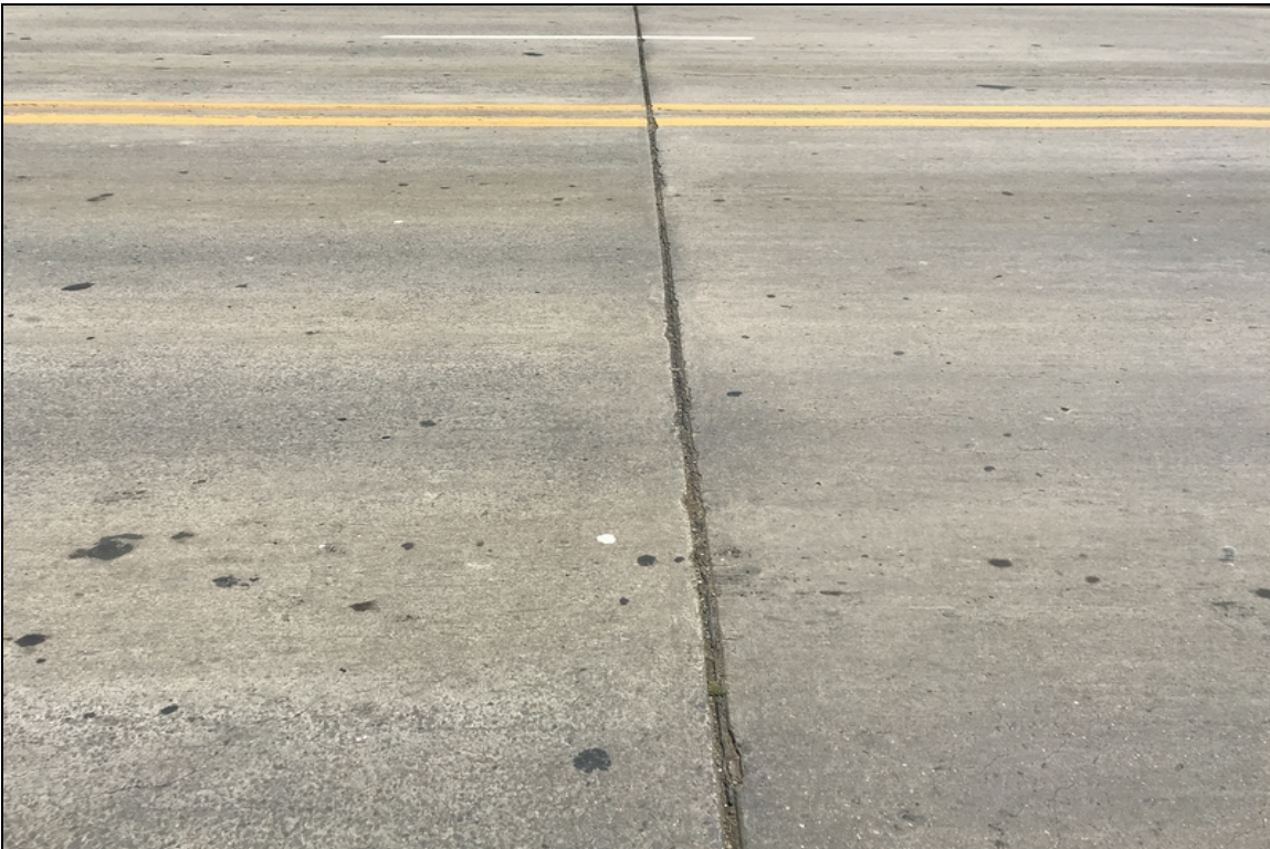
Bent # 1 joint seal with debris accumulation/ impaction.
