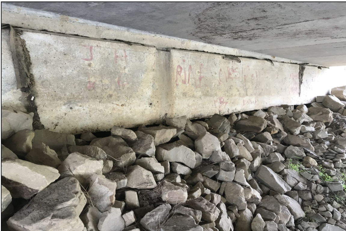
Bent # 4 earth settlement under the abutment cap.
