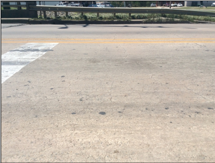
North approach slab-Cracking.
