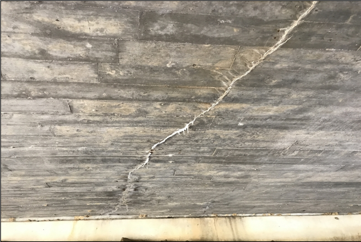
Span #1 concrete cracking with efflorescence buildup.
