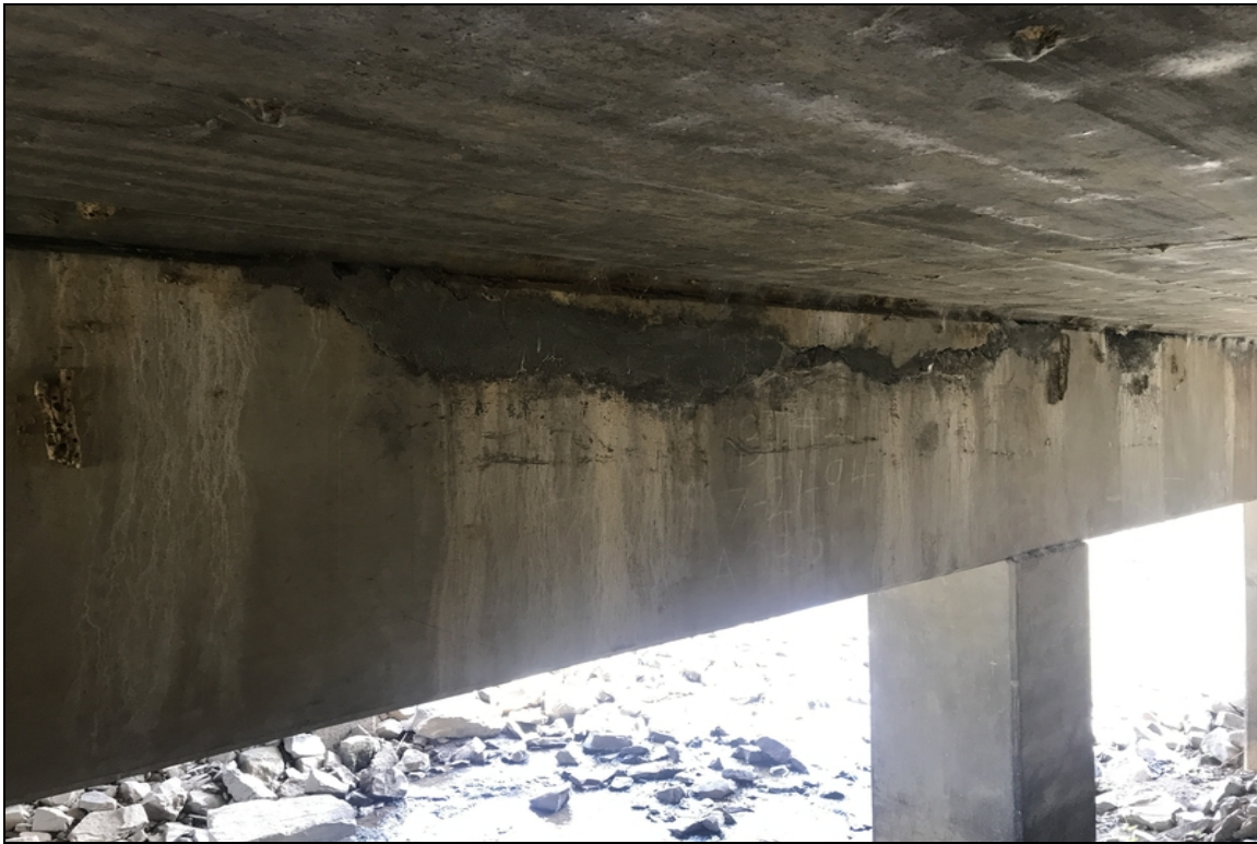
Bent #2 concrete delamination's and spalling over column #3.
