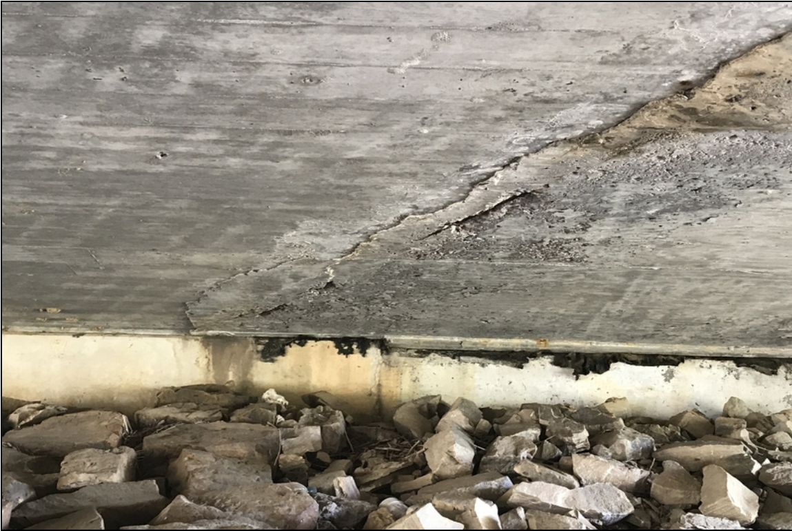
Span #3 Rt spalling with exposed reinforcing steel on the undersurface of the slab.
