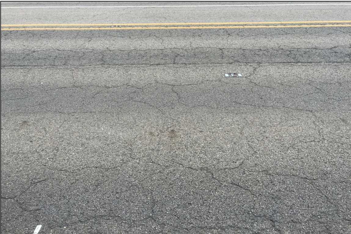
Typical cracking on the driving surface of the slab.
