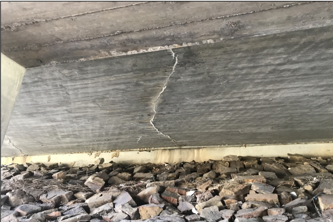
Span # 3 cracking with efflorescence buildup.
