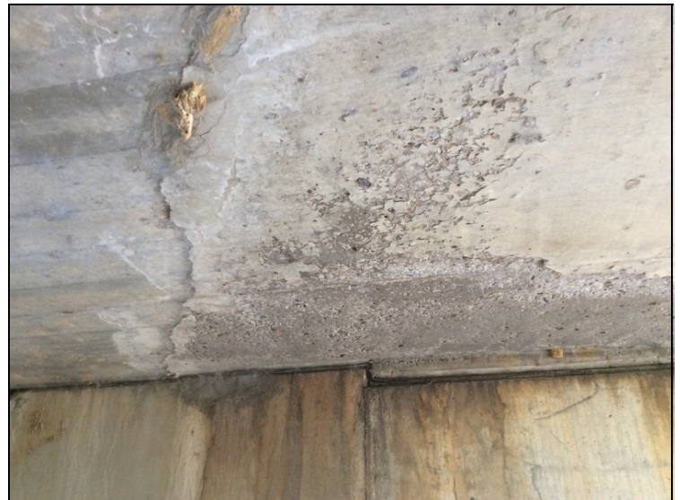
Span #1 undersurface-Scaling adjacent to bent #2.
