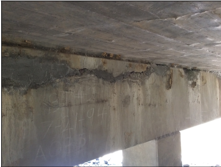
Bent #2 cap-Spalling / delaminated area in back face.
