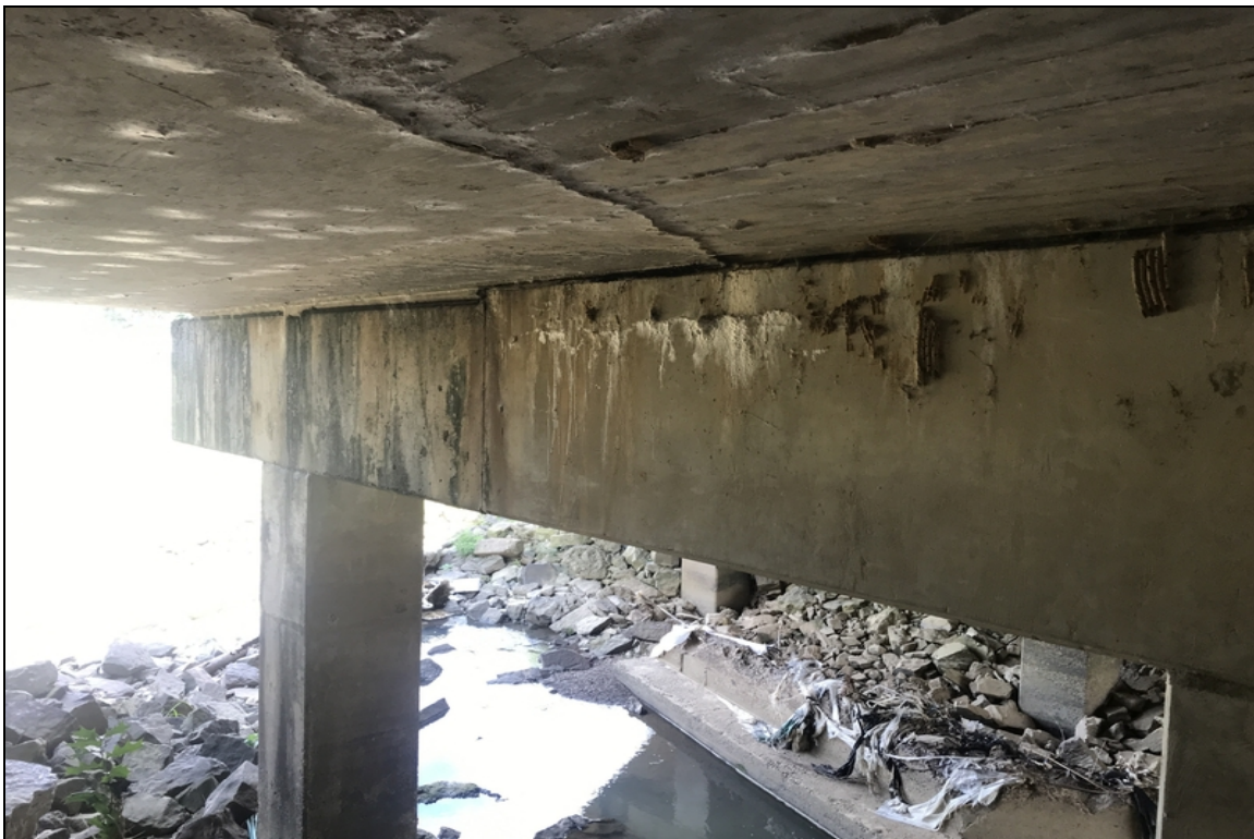
Bent #2 Lt concrete cracking with efflorescence buildup.
