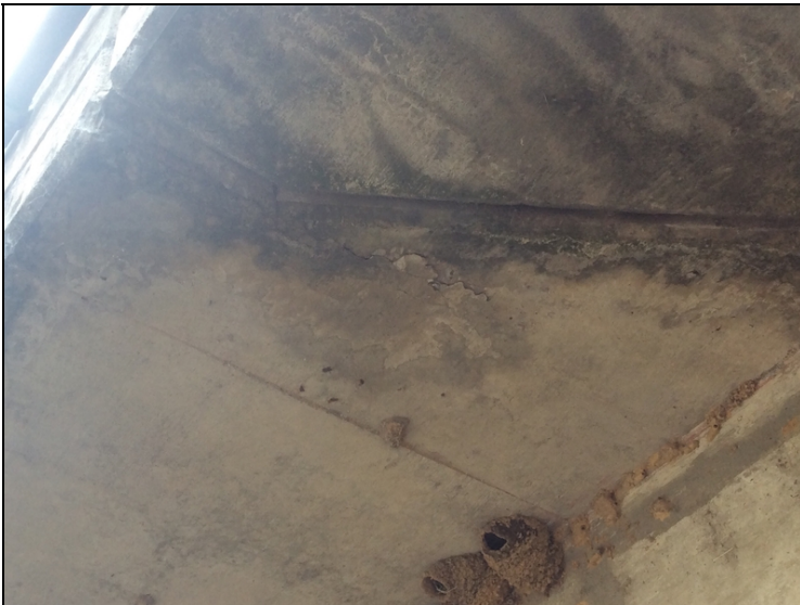
The undersurface of the right pedestrian sidewalk has a 24" delaminated area with spalling that exposes reinforcing steel over bent #3.
