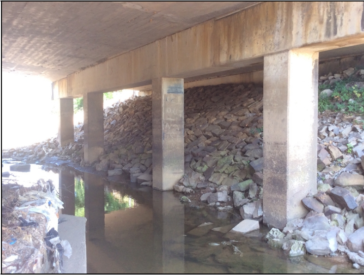
Staining due to leaking deck joints.
