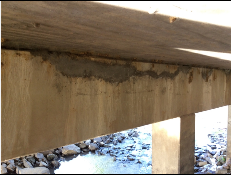
Bent 2 cap repair
