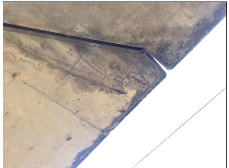
Span #2, left pedestrian sidewalk-Exposed reinforcing steel in undersurface.
