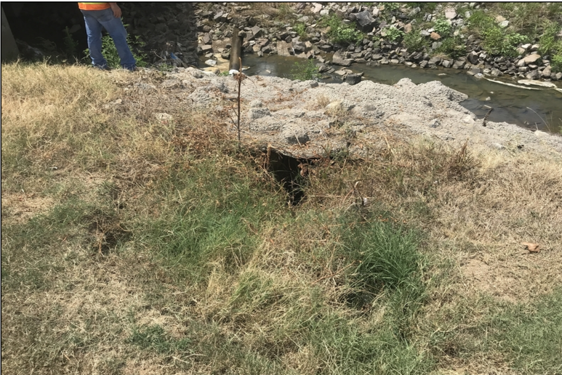
Northeast embankment with erosion under the grouted rip rap.
