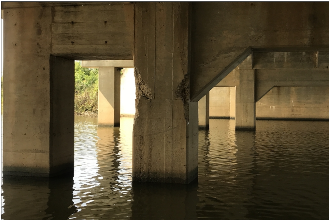
Bent #3 column #5 spalling with exposed reinforcing steel.
