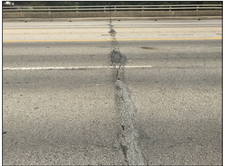
Asphalt breaking up over bent #3.
