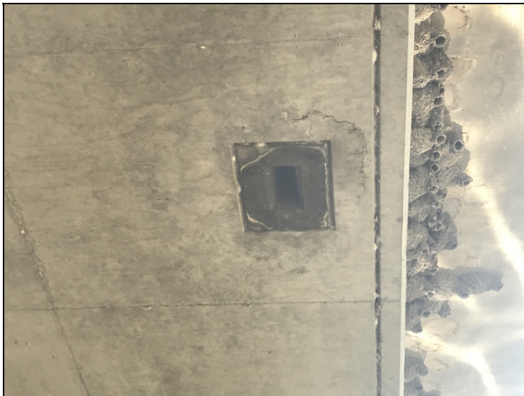
Span #2, right side-Delaminated area at deck drain.
