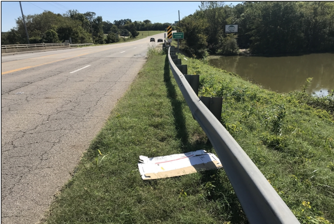
Southwest approach rail collision damage.
