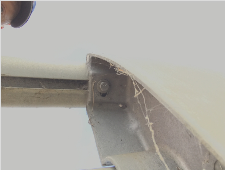
Span #3, right bridge railing at post #1-Loose connection.
