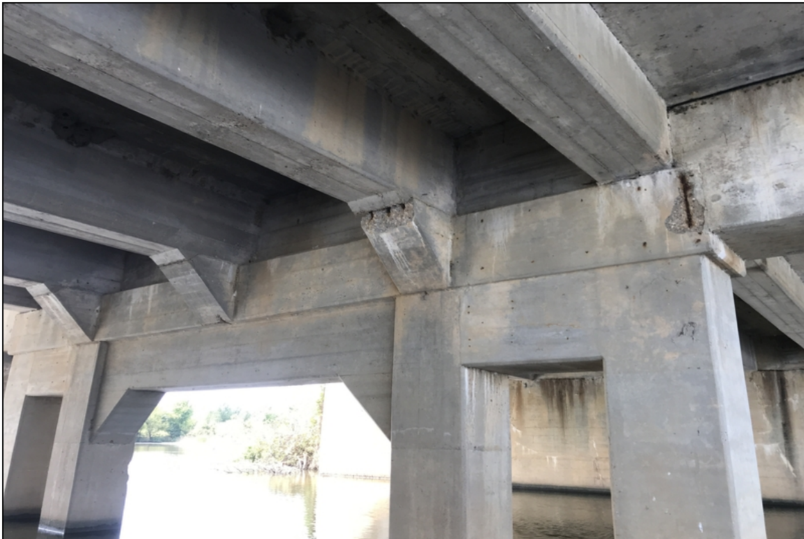
Bent #2 Span #2 girders # 1,2 & 3 spalling with exposed reinforcing steel.
