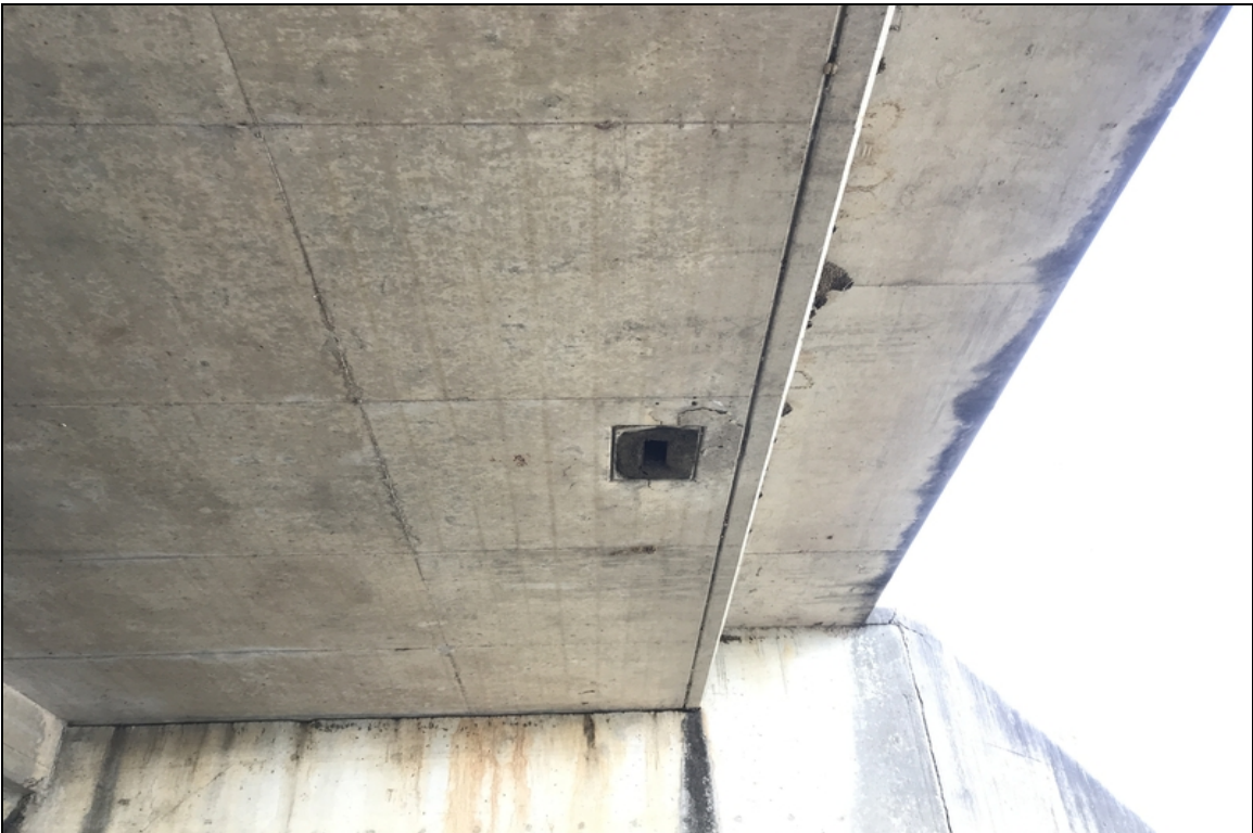
Span #1 Lt concrete delamination's at the deck drain.
