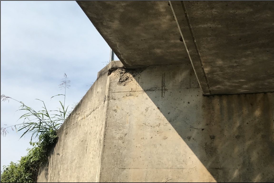
Abutment #1 Rt spalling in the abutment at the wingwall juncture.
