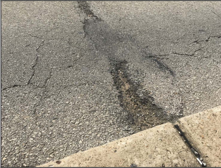
Asphalt breaking up over bent #3, left side.
