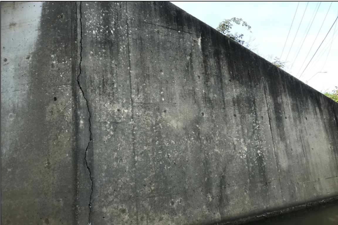
Abutment #1 Lt wing wall cracking.
