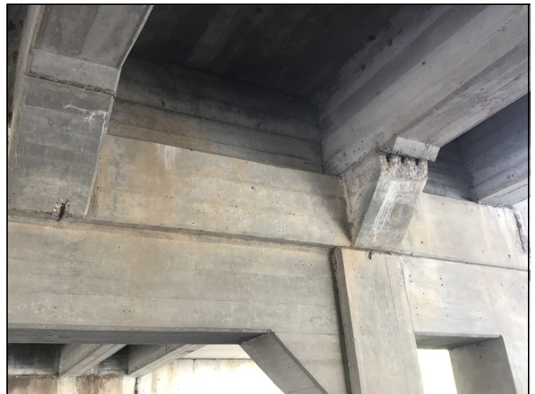
Bent #2 cap-Spalling with exposed reinforcing steel.
