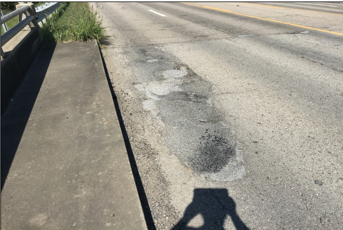
Span #1 Rt with failing asphalt patches.
