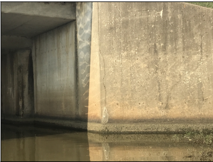
Northwest wing wall-Wide vertical cracking.
