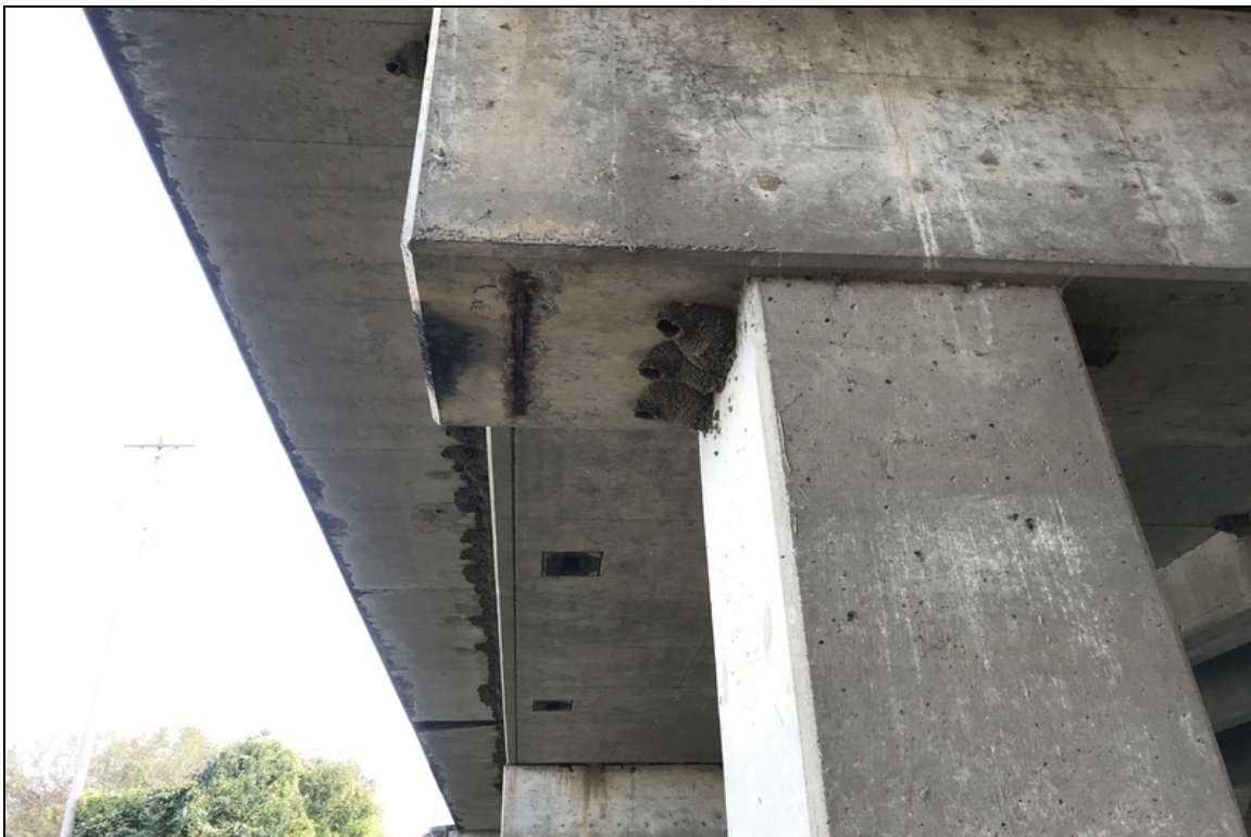
Bent #2 Lt shallow spalling with exposed reinforcing steel.
