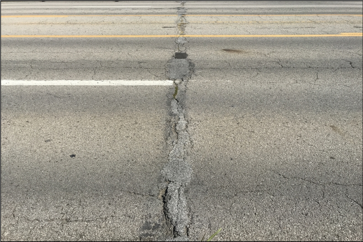
Bent #3 asphalt breaking apart over the deck joint.
