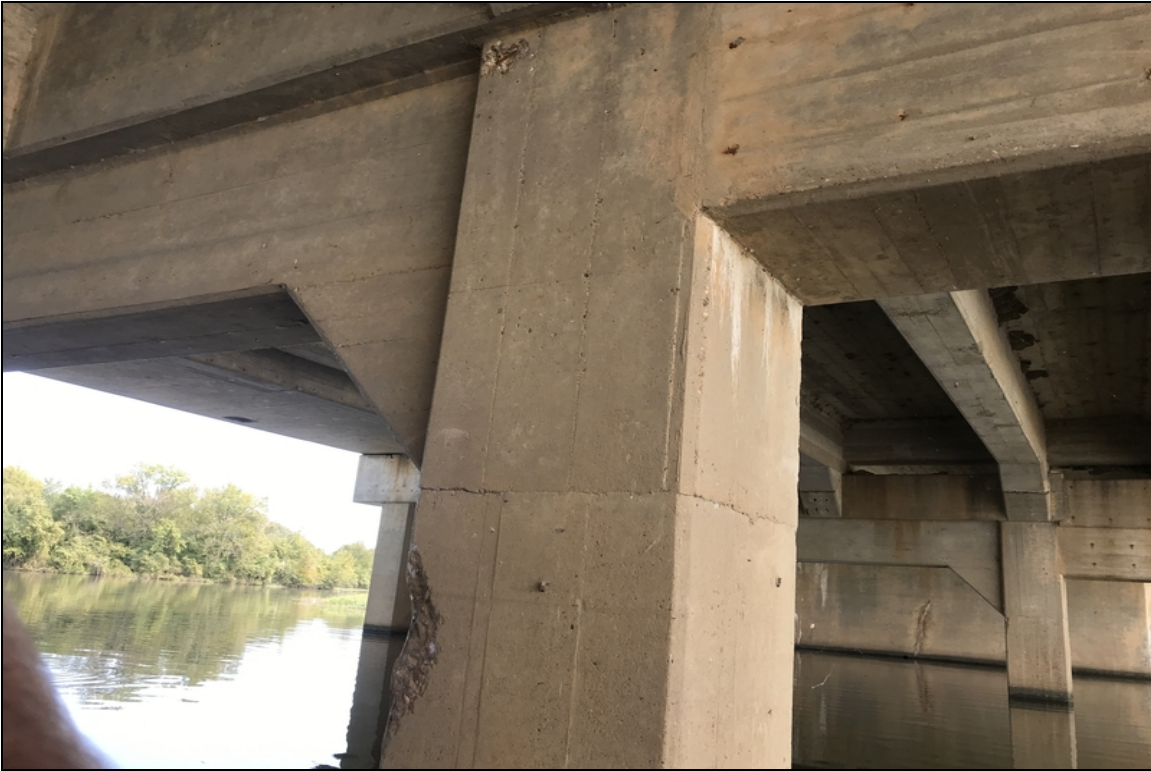
Bent #2 column #5 spalling with exposed reinforcing steel and a concrete spall near the water elevation.
