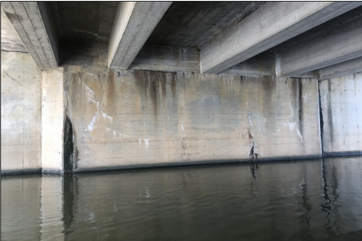
Abutment #1 cracking in the original portion of the abutment stem.
