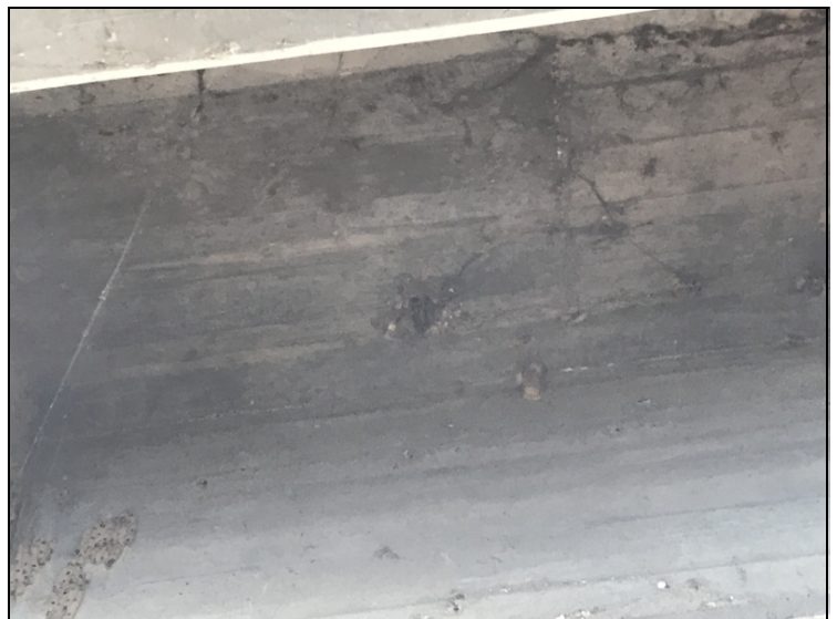
Span #3, bay #4-Spall with exposed reinforcing steel near abutment #2.
