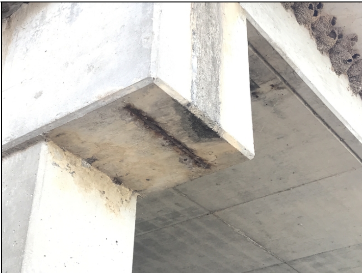
Bent #2 cap, left side-Spalling with exposed reinforcing steel.
