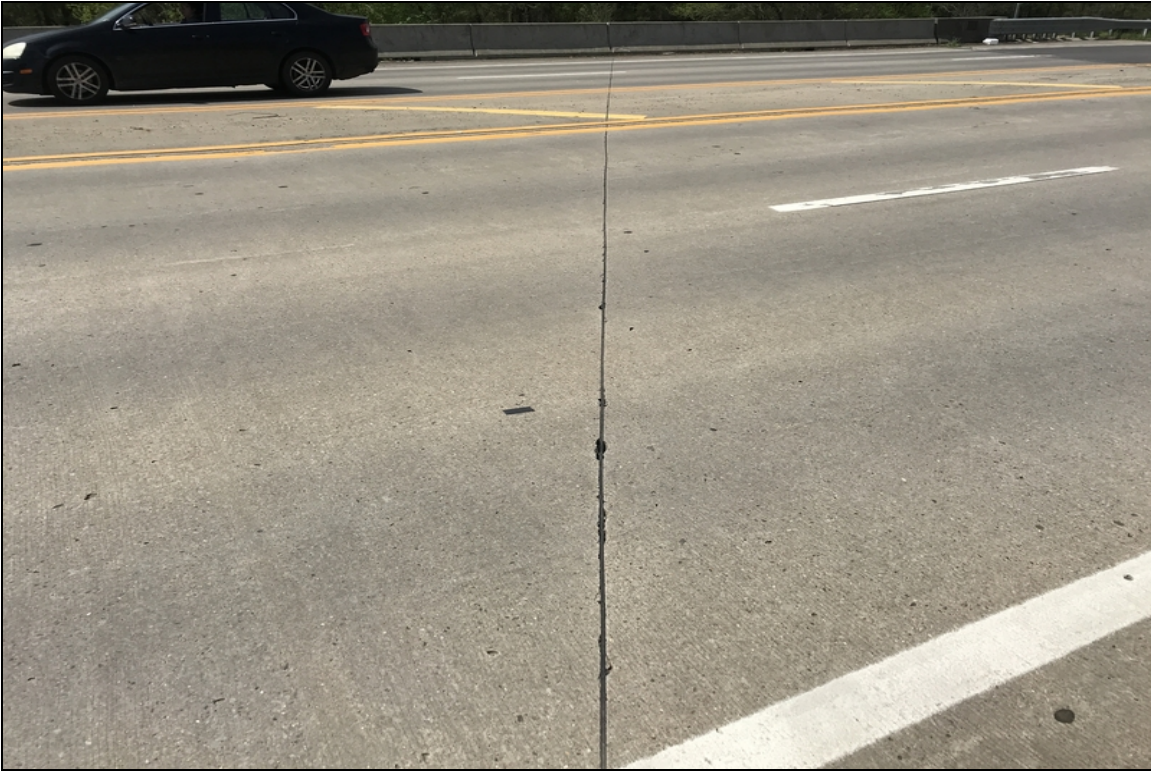
Deteriorating poured joint sealant.
