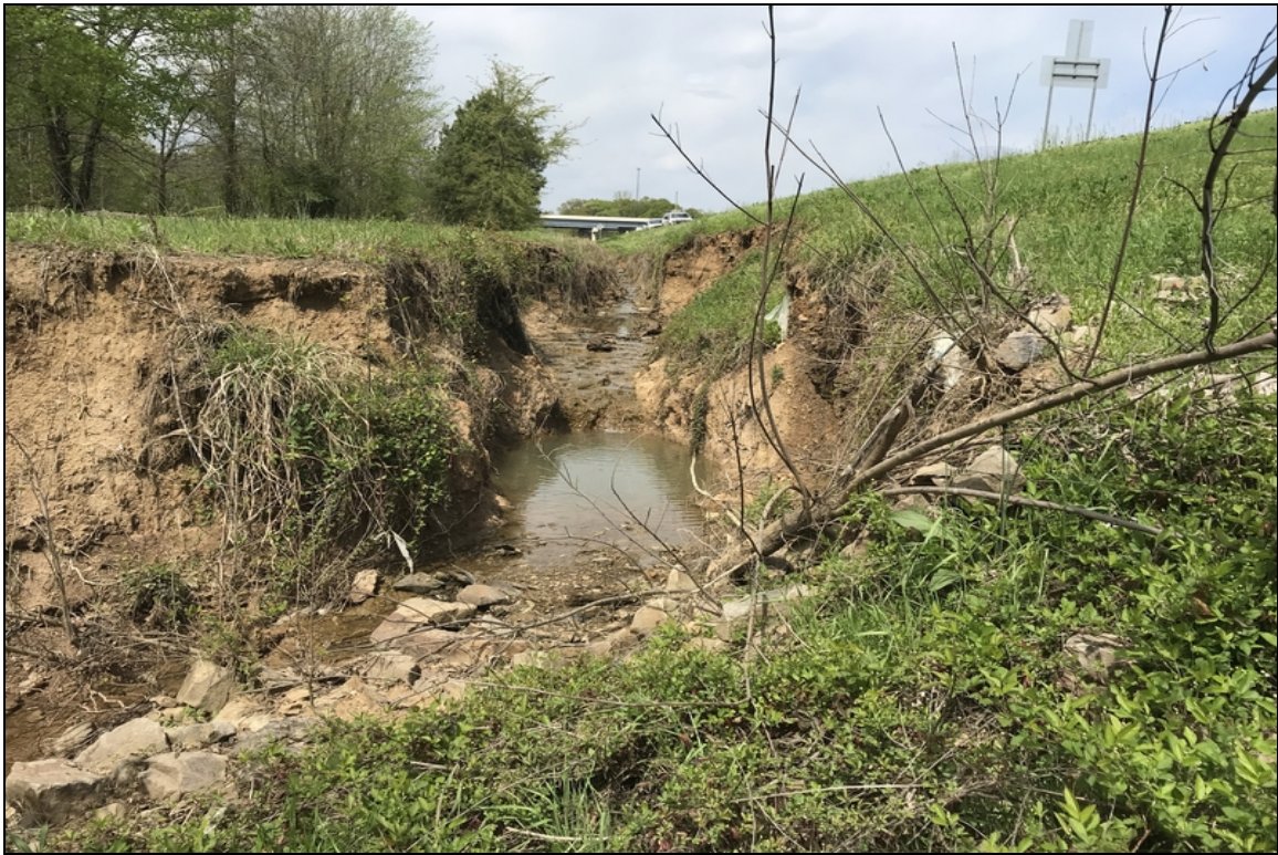
Southwest bridge end with approximately 7' of head cut scour.
