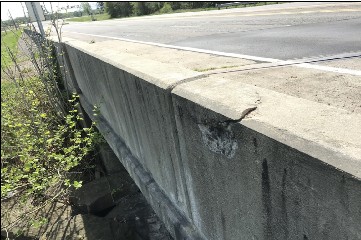
Span # 3 Lt concrete spalling/ delamination.
