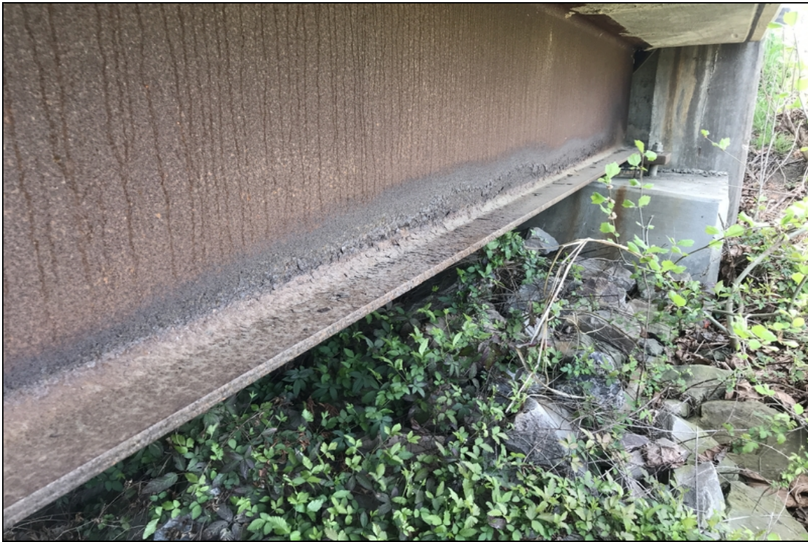
Bent # 1 Beam # 1 exterior base of web and bottom flange with flaking rust
