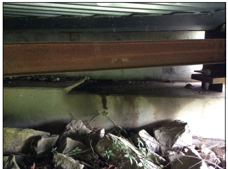
Debris on bent 1 seat.
