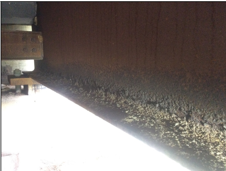
Span #1, beam #1-Corrosion with flaking rust on bottom flange and base of web at abutment #1.
