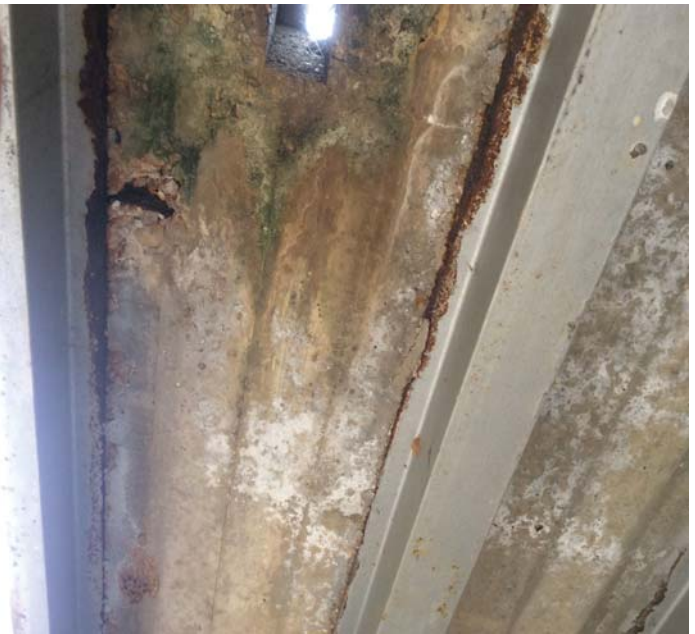
PHOTO 2 Description Bay 1 has 1 shallow baseball size spall with exposed reinforcing steel on the undersurface of the deck.
