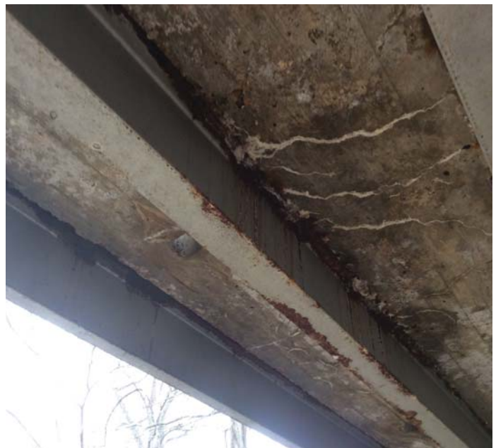
PHOTO 2 Description Beam 9 has active corrosion with initial section loss adjacent to the deck drain near mid-span.
