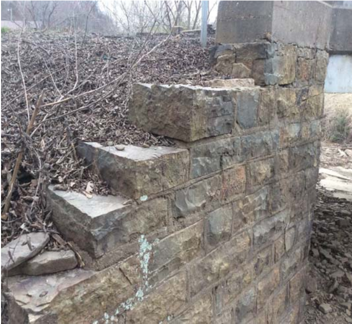
PHOTO 3 Description A few of the stones have been displaced in the top of the Southeast wing wall.
