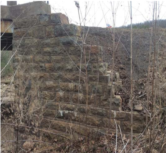
PHOTO 4 Description A few of the stones have been displaced in the top of the Northeast wing wall.
