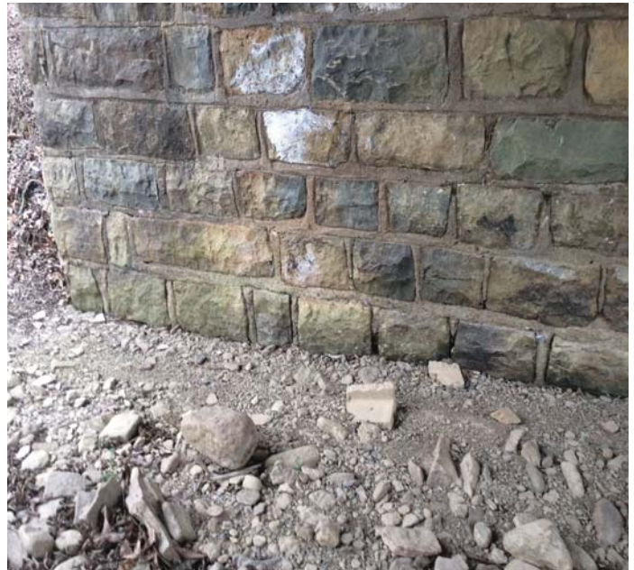
PHOTO 2 Description Grout deterioration between the stones at the base of the walls is typical in both abutments.
