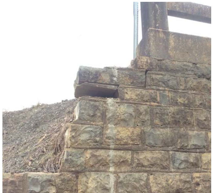
PHOTO 2 Description A few of the stones have been displaced in the top of the Northwest wing wall.
