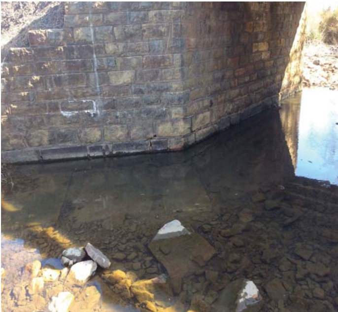
PHOTO 1 Description Concrete slabs placed at the base of Bent 2 to control scour are in place and functioning as intended. No apparent scour or scour problems at this inspection.
