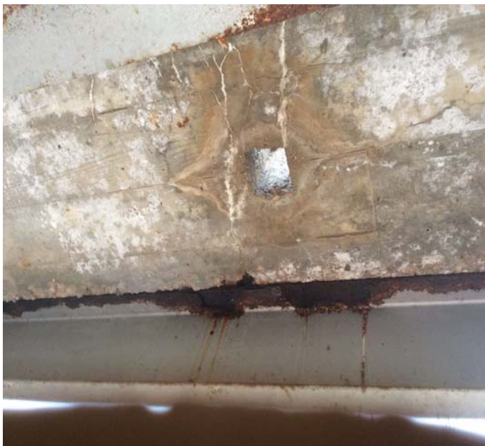
PHOTO 3 Description Bay 9 has 3 shallow baseball size spalls. Spalls have exposed reinforcing steel that has active corrosion with initial section loss.
