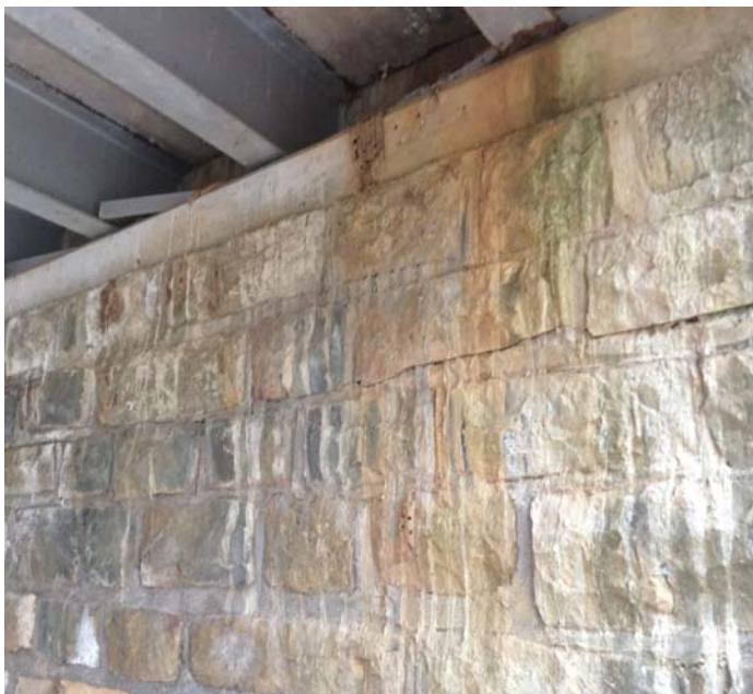
PHOTO 3 Description Rock masonry substructure with a horizontal hairline crack in grout approx. 18" below cap at Bent 2.
