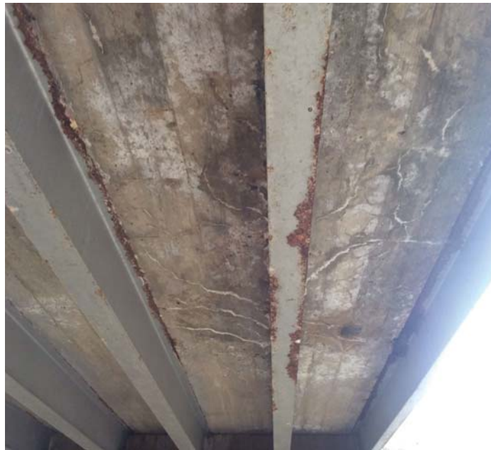
PHOTO 1 Description Map cracking with light efflorescence visible from the undersurface of the deck in Bays 8 & 9.
