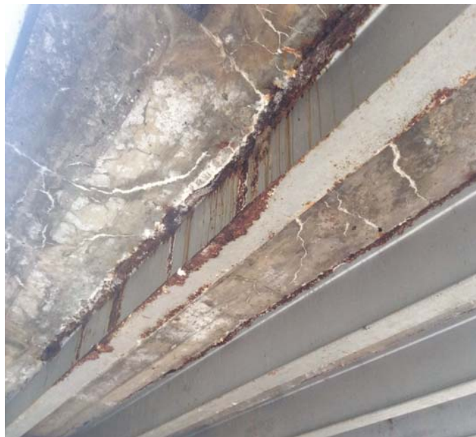
PHOTO 1 Description Beams 1,2,3, 8,9, & 10 have areas of active corrosion along the top flanges of the beams.
