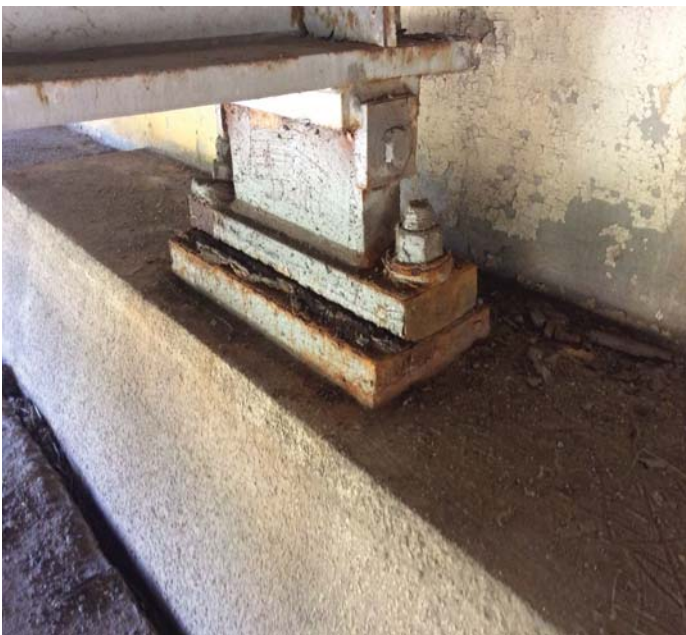
PHOTO 1 Description Bearings have active corrosion with layers of rust on the masonry plates.
