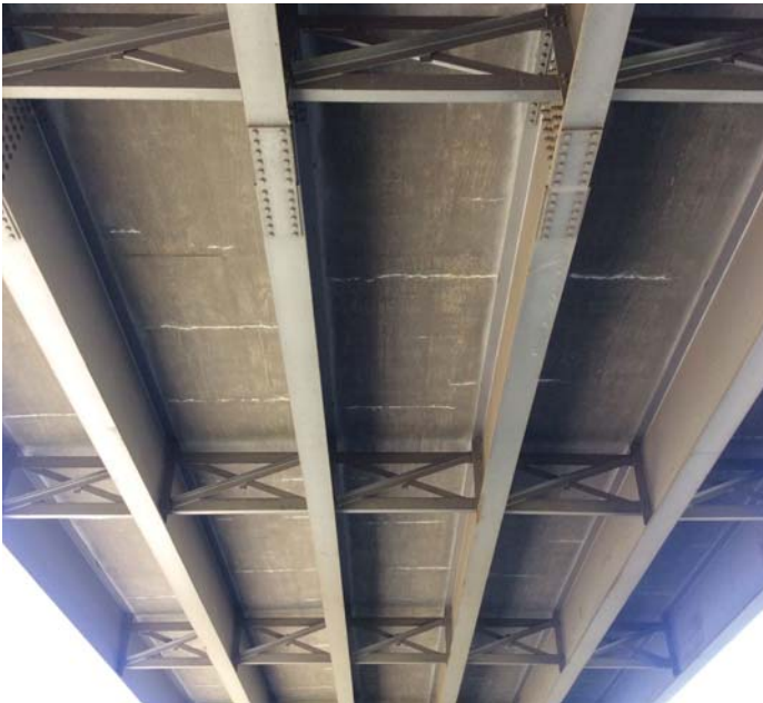
PHOTO 1 Description Light / medium efflorescence visible in undersurface of all Spans.
