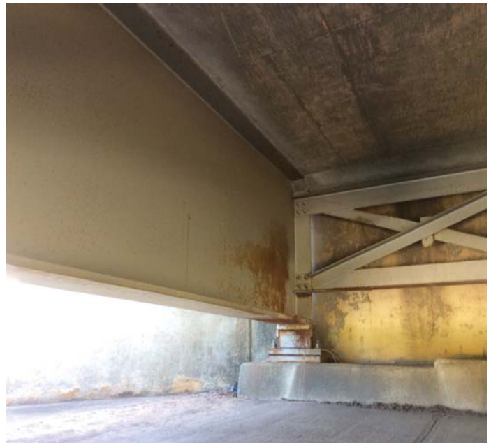
PHOTO 2 Description Superstructure has a failing paint system with freckled rust and active corrosion in the top flanges of the beams and diaphragms with isolated area of flaking rust.
