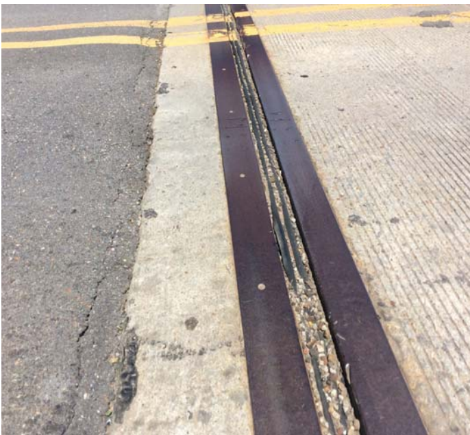
PHOTO 1 Description The joint seal at Bent 1 has cracks and appears to be deteriorating from weathering.
