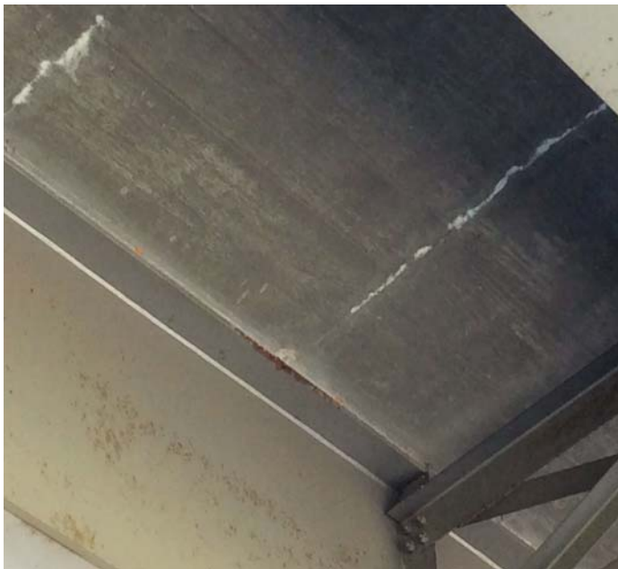
PHOTO 1 Description Transverse cracks appear to be full depth with leakage contributing to the active corrosion on the top flanges of the beams.
