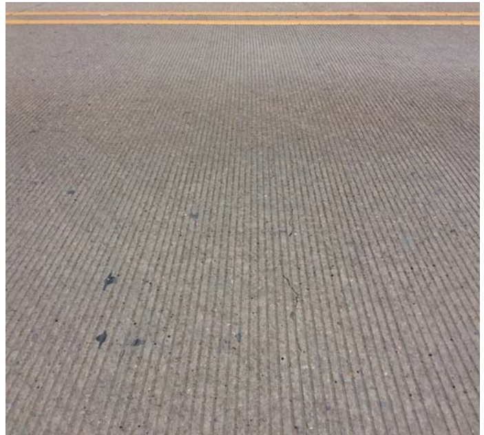
PHOTO 2 Description The driving surface of the deck has sealable transverse deck cracks with light efflorescence.
