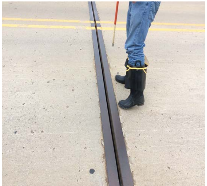
PHOTO 2 Description Bent 4 deck joint seal missing
