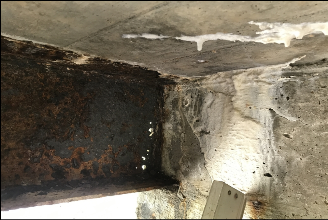
Span # 4- Beam # 1, Bent # 5 face- 2" x 5" area that is paper thin with multiple holes and perforations.
