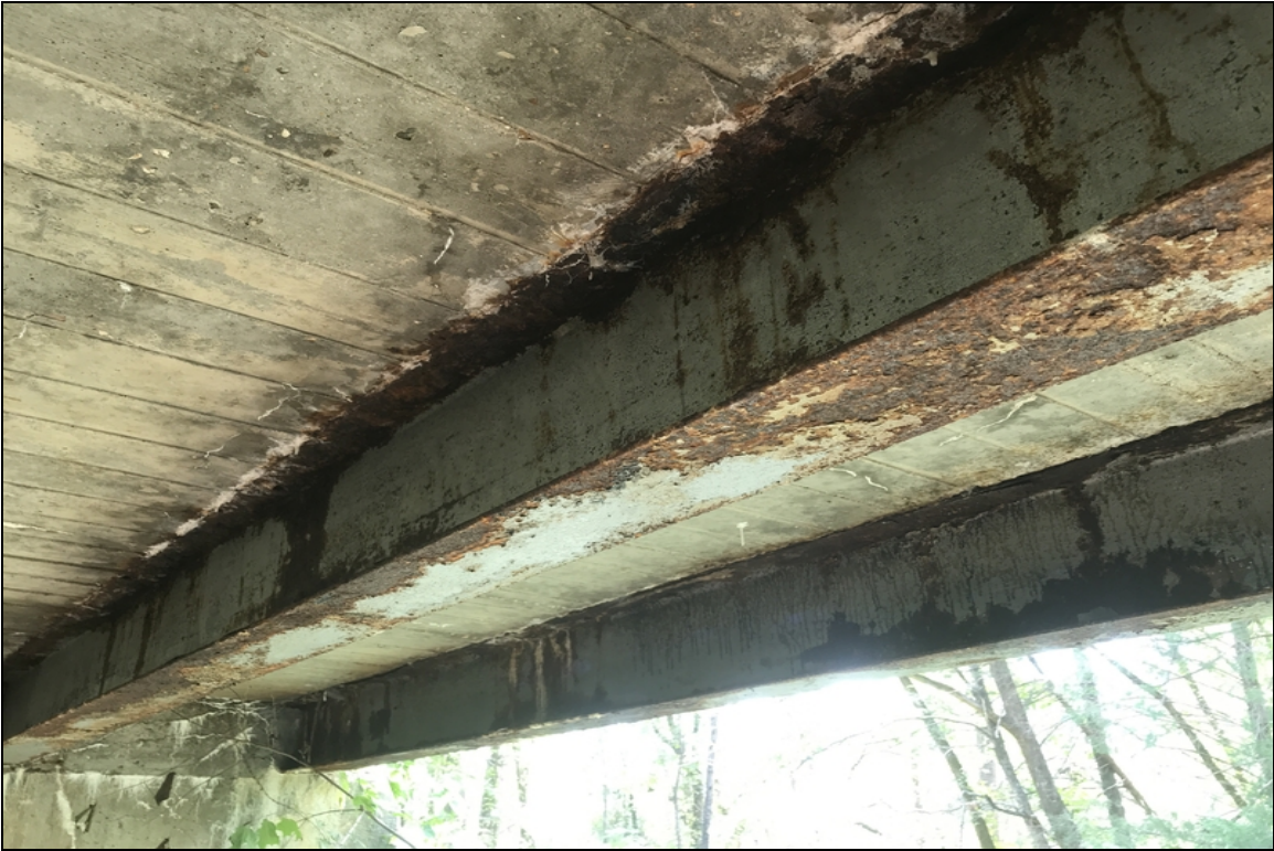
Span 1 Beams 8 & 9 active corrosion.
