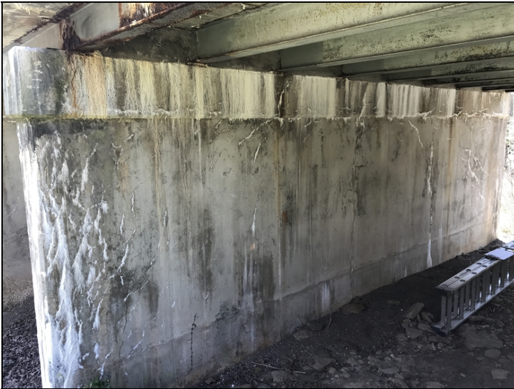
Bent # 2 cracking with efflorescence buildup.
