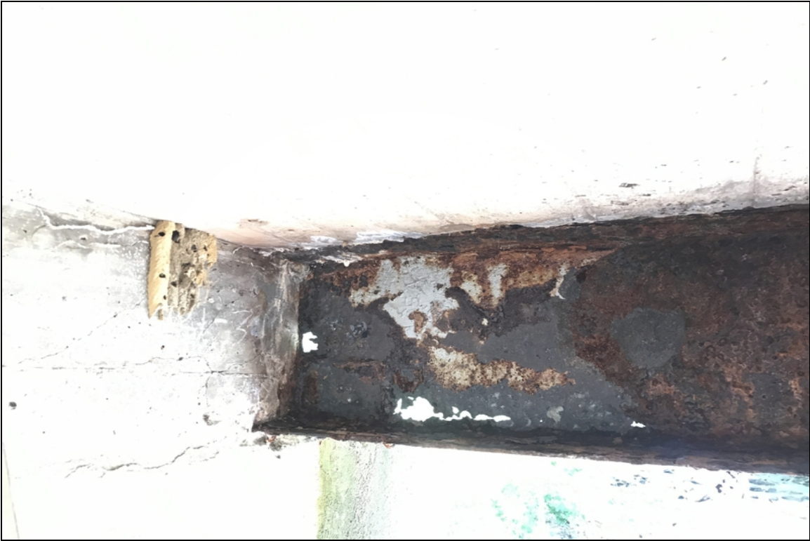
Span # 3- Beam # 1 Bent # 3 face- multiple holes rusted through base of web.
