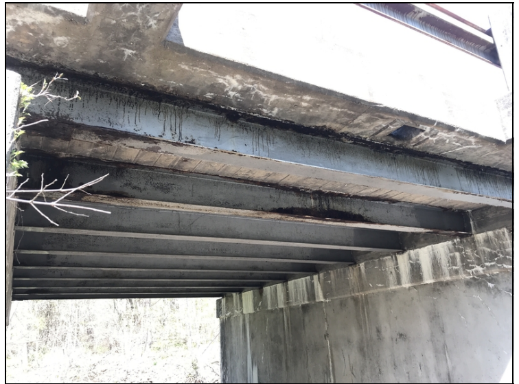
Span # 2 active corrosion with soft deteriorating concrete and efflorescence buildup.
