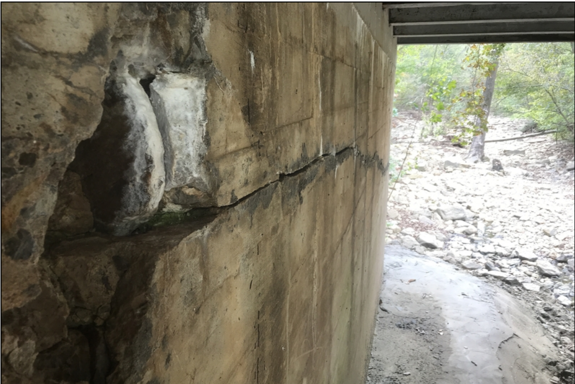
South abutment horizontal cracking.
