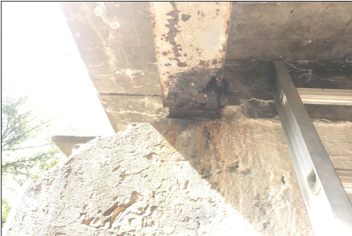
Span 4 Bent 4 Beam 9 hole in the bottom flange.
