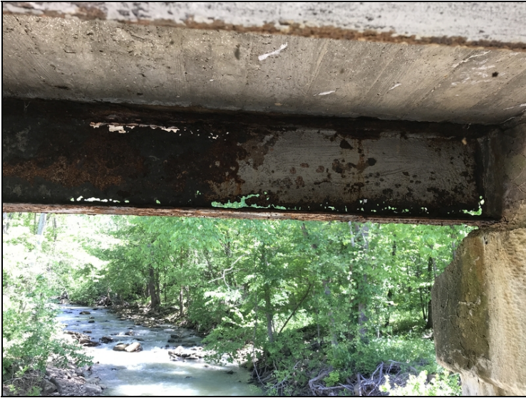
Span # 3 Beam # 1 Bent # 3- multiple holes within 4' of Bent # 3.
