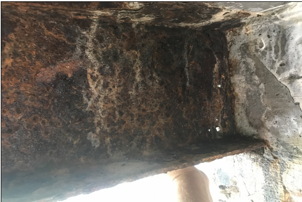
Span 4 Bent 5 Beam 1 holes in the web.
