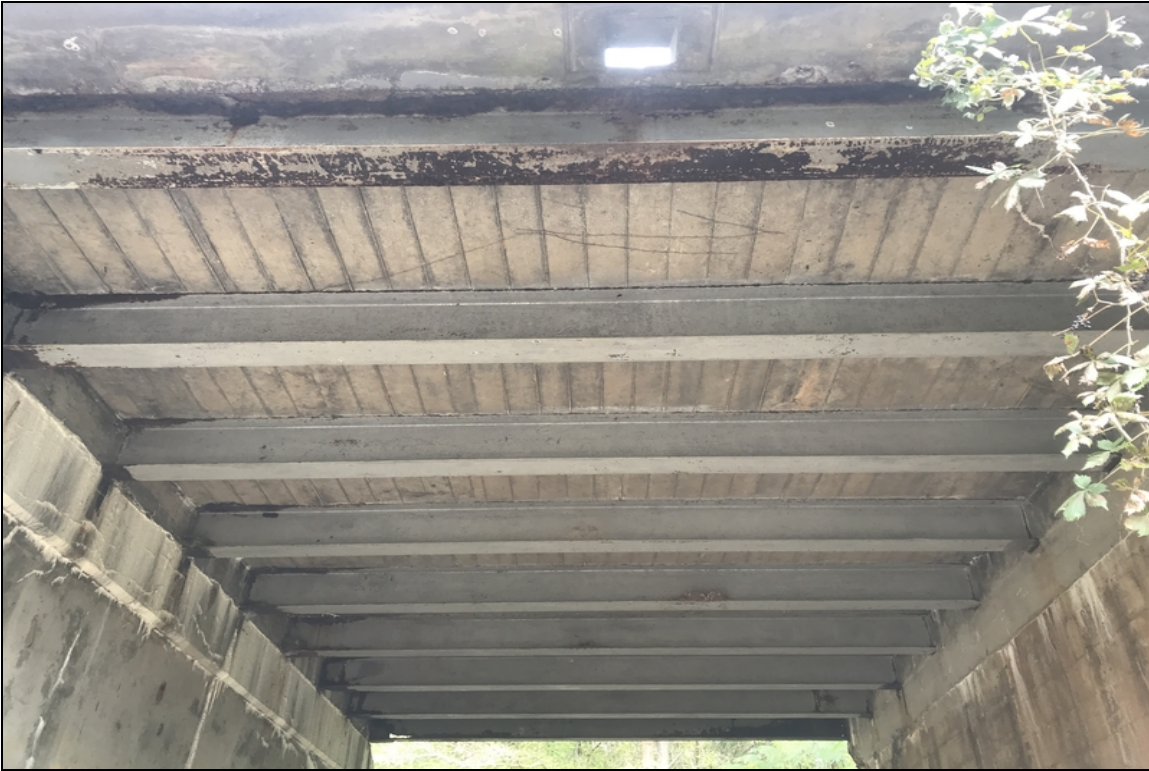
Span 4 typical active corrosion in the superstructure.
