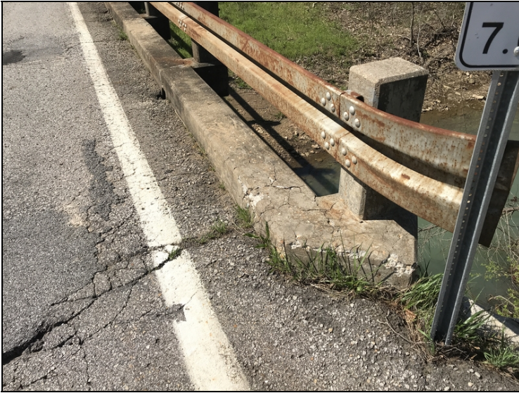
Cracking in the curbs.
