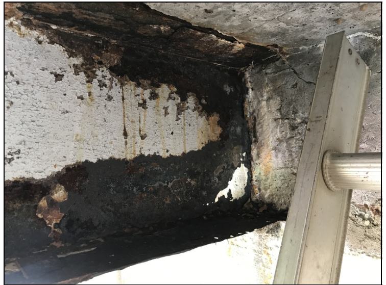
Span # 3 Beam # 2 Bent # 3 - a 4" hole in the web at Bent # 3 face.
