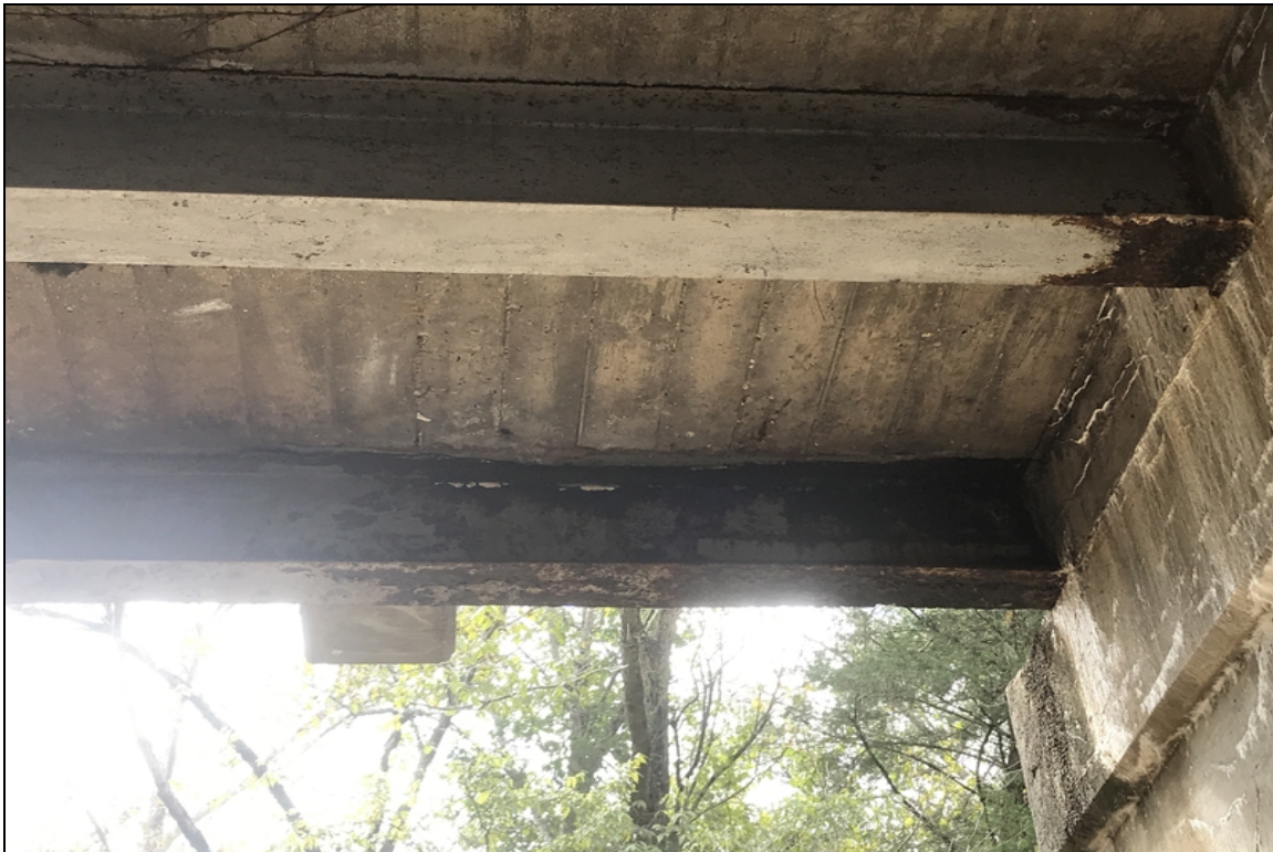
Span 3 Beam 9 @ Bent 3 holes in the web.
