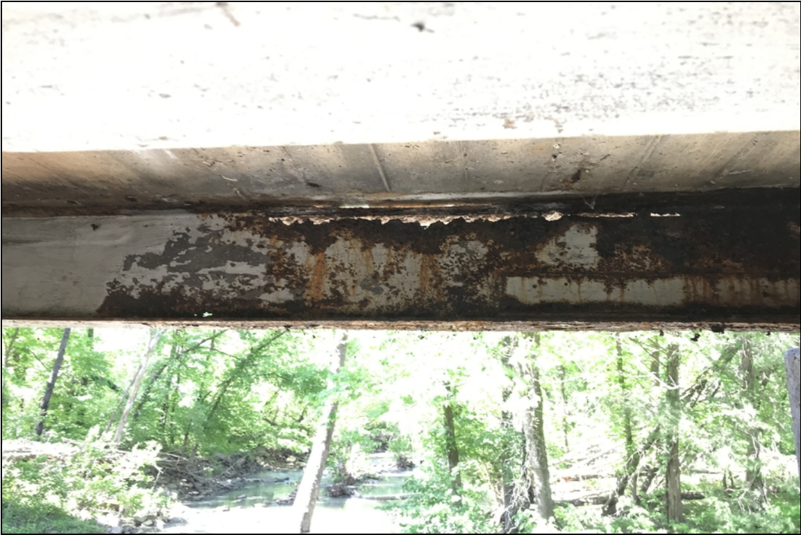
Span # 3, Beam # 9. 3' section of web missing.
