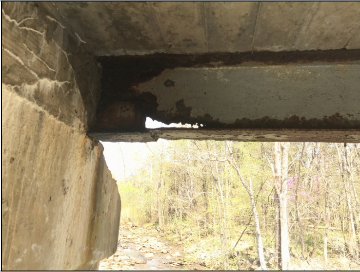
Span # 4, Bent # 4, Beam # 1 has a 3" x 8" hole in the web.
