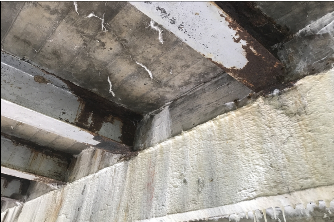
Bent 4 Span 4 Beams 2 & 3 holes in the bottom flanges.
