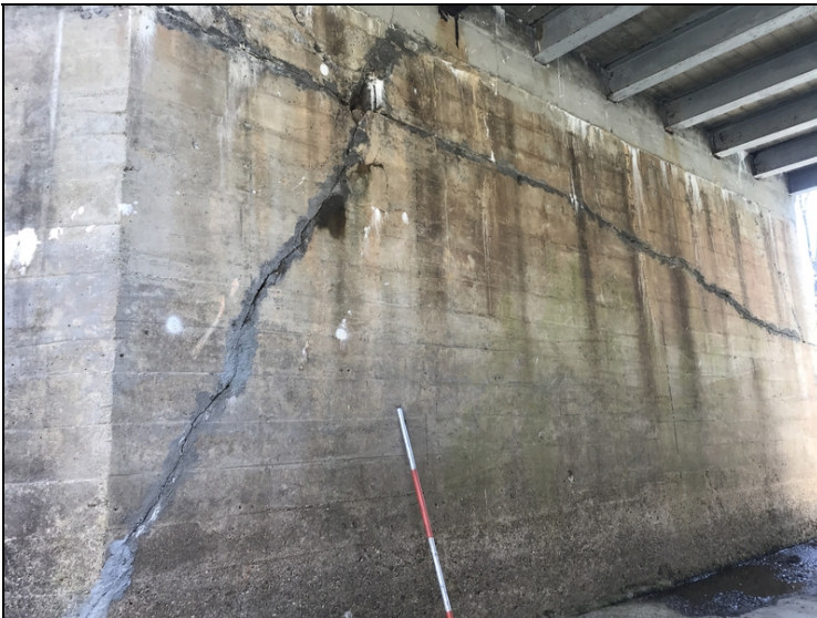
Bent # 5 cracking in the abutment stem.
