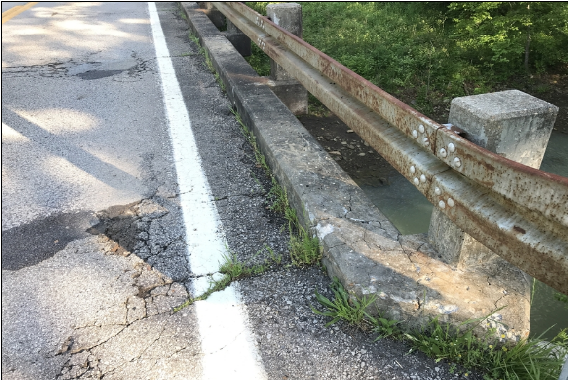
Left curb. Span # 4. Map cracking.
