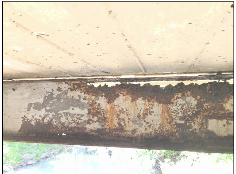
Span # 3. Beam # 9 section loss with 1/2" space between the top of the beam and the undersurface of the deck.
