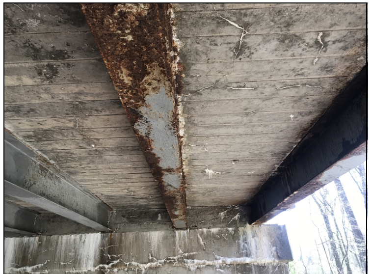
Span # 1 cracking with efflorescence on the undersurface of the deck.
