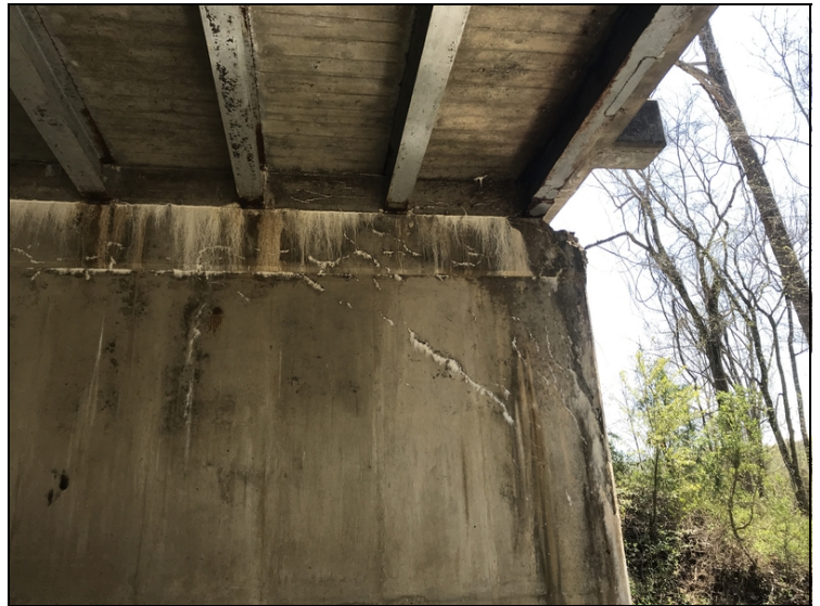
Bent # 4 Rt concrete deterioration and section loss with exposed reinforcing steel.
