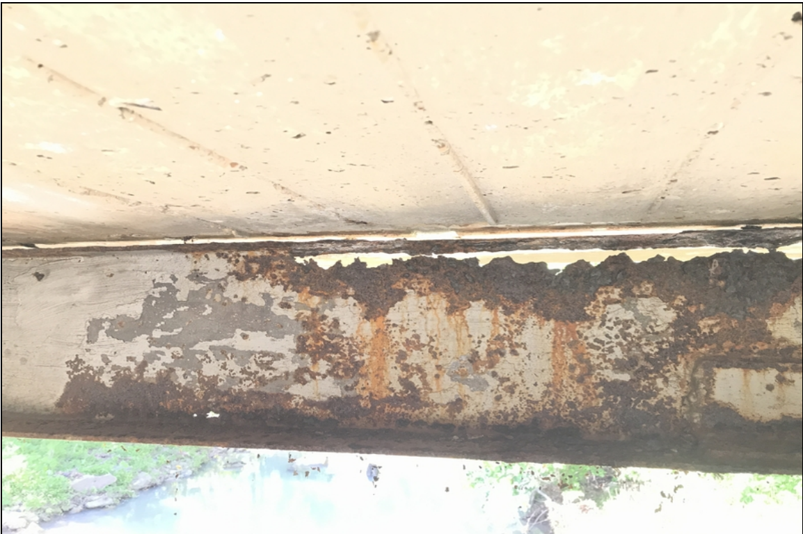
Span # 3. Beam # 9 section loss with 1/2" space between the top of the beam and the undersurface of the deck.
