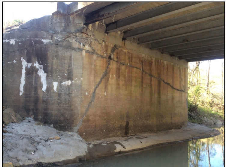
Bent # 5 cracking and concrete deterioration.
