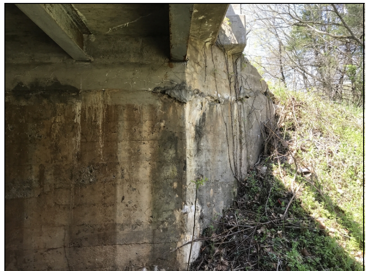
Bent # 1 Lt wing wall deterioration.
