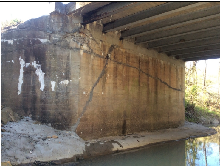
Bent # 5 cracking and concrete deterioration.
