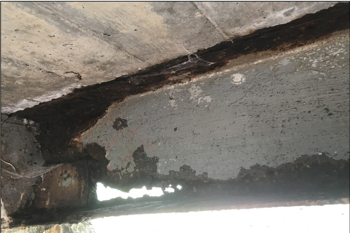
Span 4 Bent 4 Beam 1 large hole through the web.
