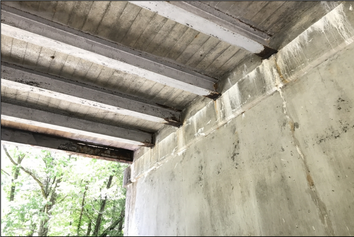
Span # 3 superstructure at Bent # 3. Typical of Beam corrosion.
