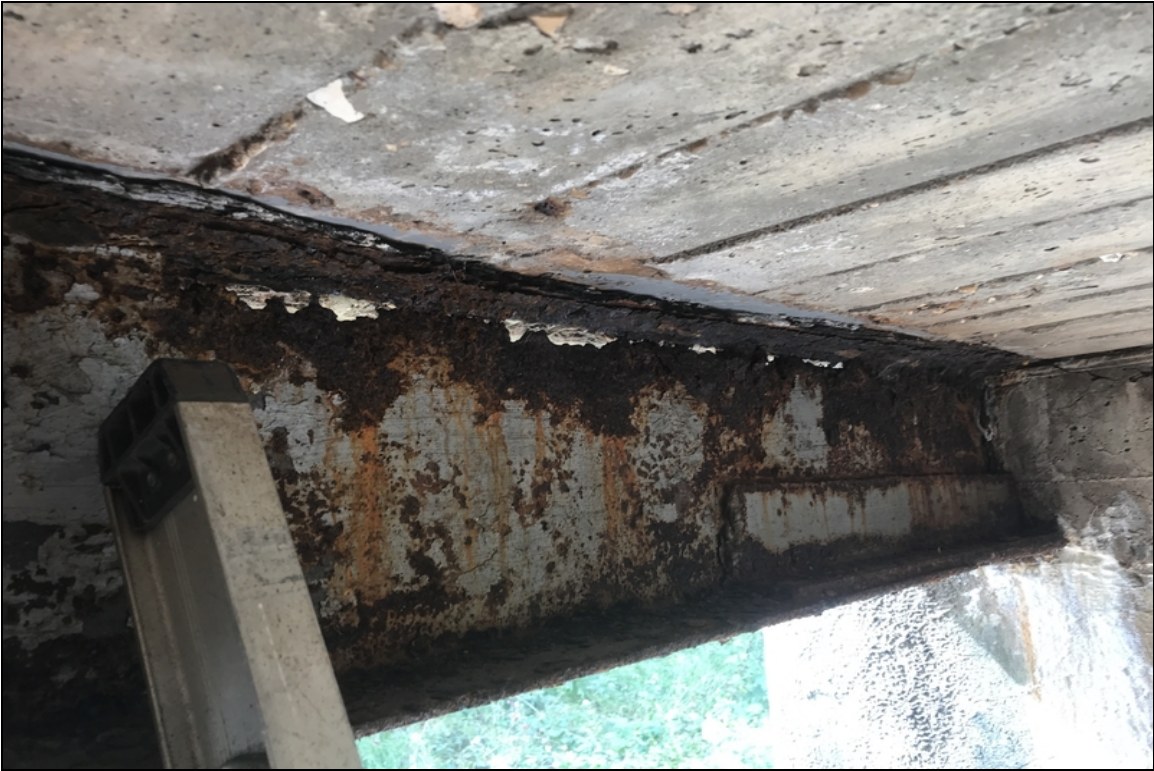
Span 3 Beam 9 Numerous holes in the web.
