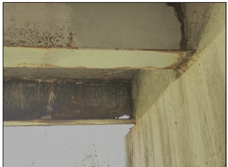
Span # 1 Beam # 1 @ Bent # 2 with a hole rusted through the base of the web.
