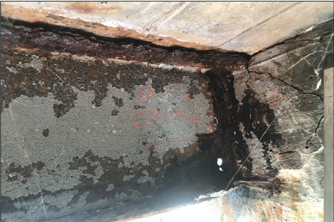
Bent 4 Span 4 Beam 9 holes through the web.
