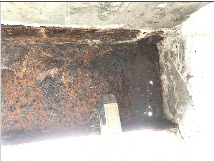
Bent # 5 Beam # 1 with holes rusted through the web adjacent to the bent cap.
