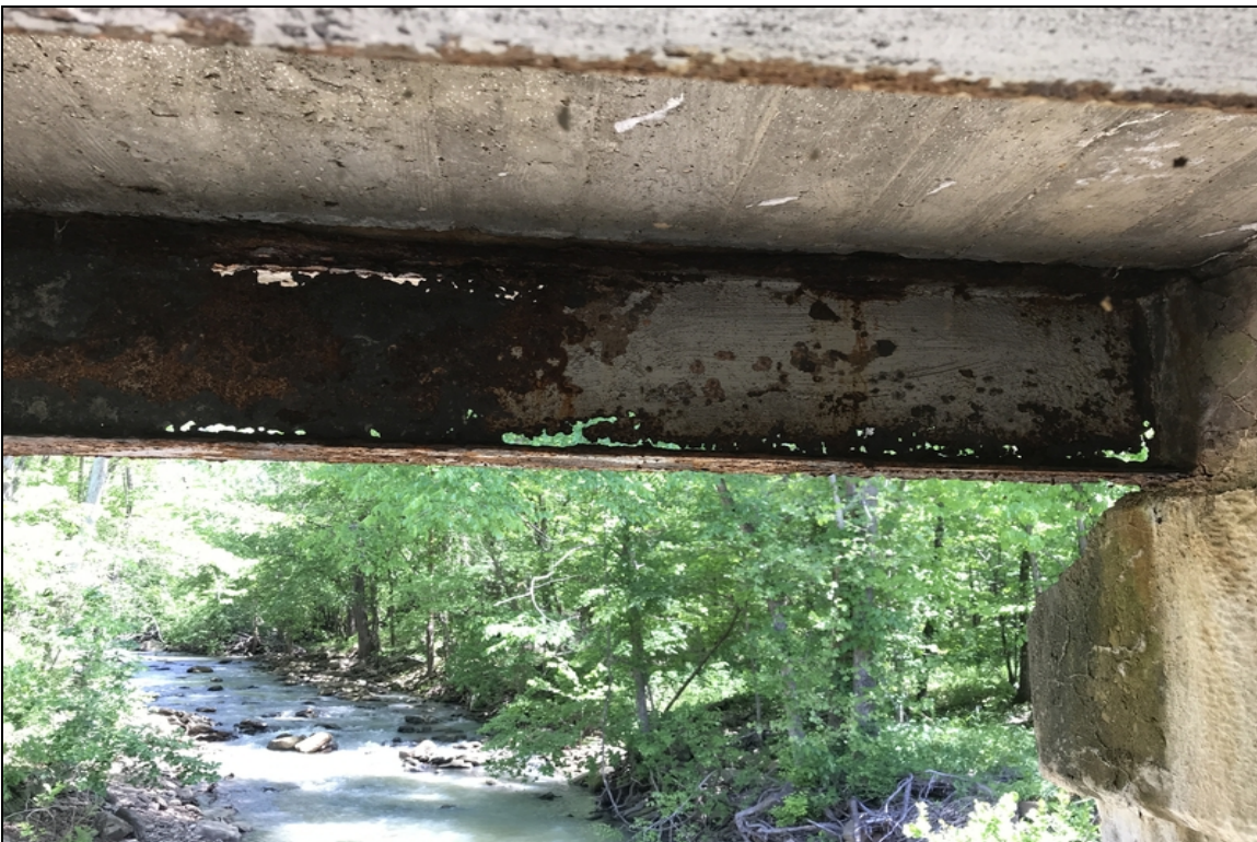
Span # 3 Beam # 1 Bent # 3- multiple holes within 4' of Bent # 3.
