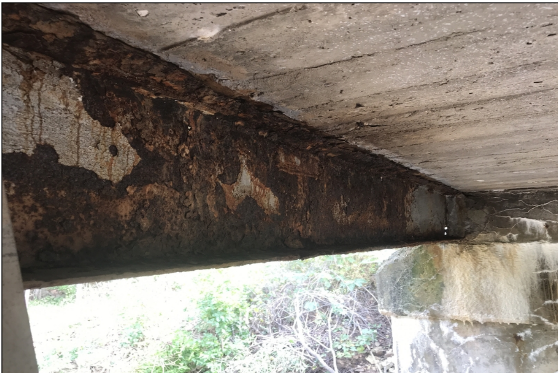
Span 3 Beam 1 Numerous holes in the web.
