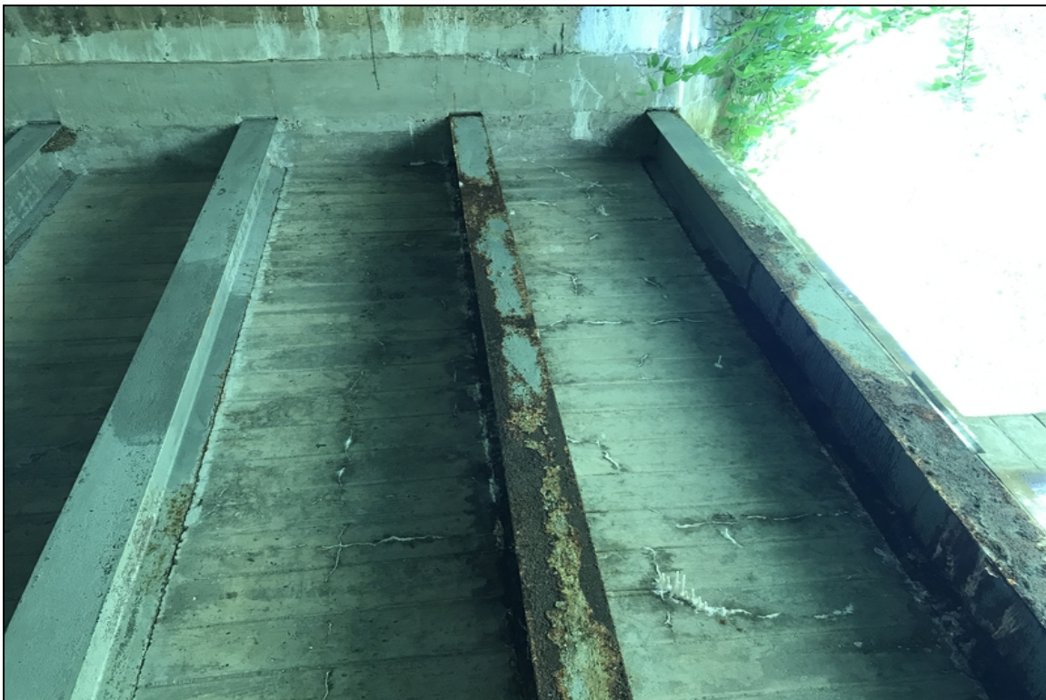
Undersurface of Span # 1. Efflorescence.
