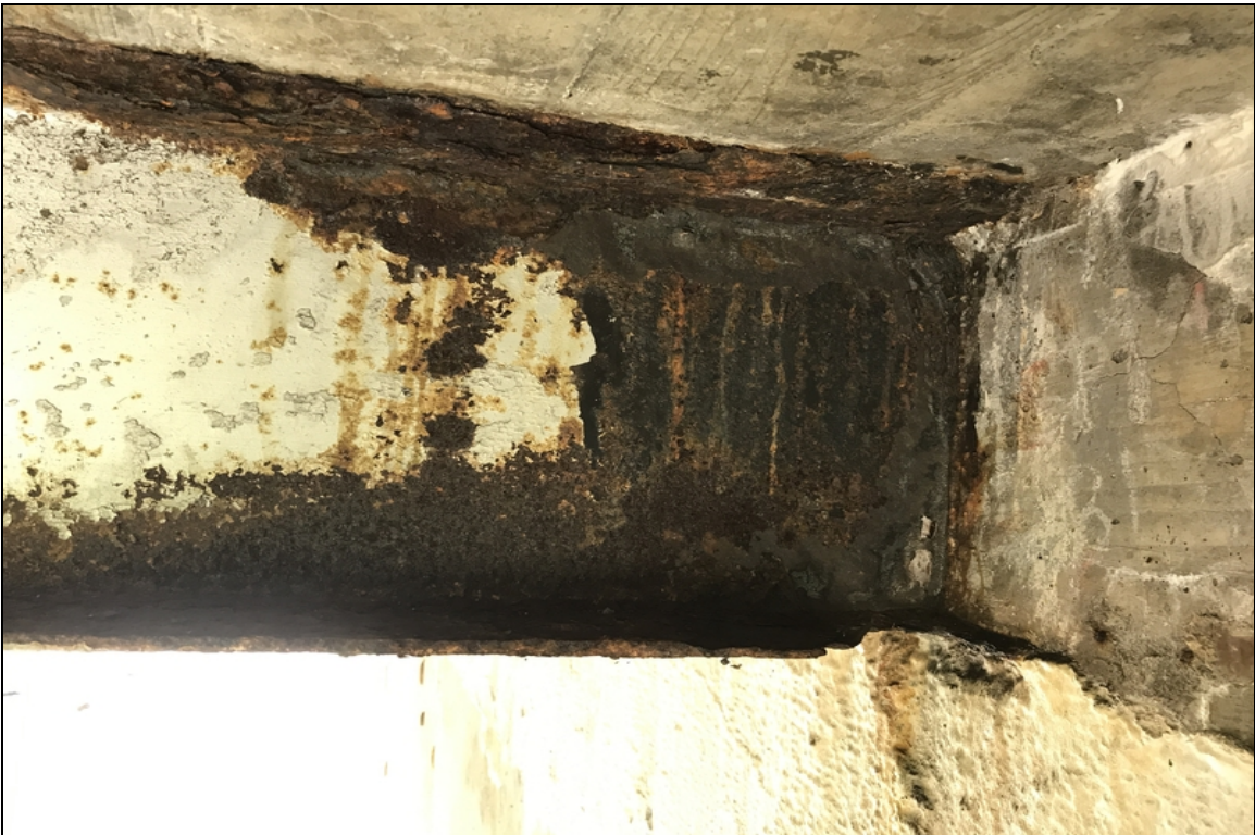
Span # 4 Beam # 2 Bent # 4 face- 2" hole, bottom flange reduced to 2" in width.
