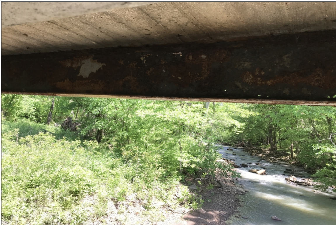
Span # 3 mid-span Beam # 1 - multiple holes in web near mid-span.
