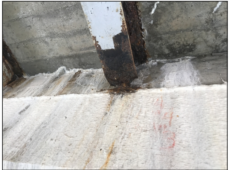
Span # 4, Bent # 4, Beam # 3 has significant section loss to the bottom flange.
