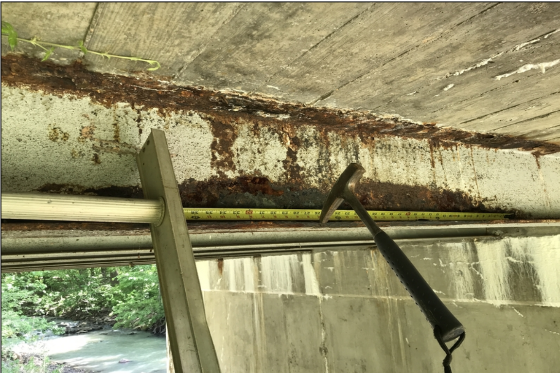
Span # 2, Beam # 8 located near mid-span- bottom flange is paper thin with perforations. Web is reduced to approximately 1/16". 3" tall x 3' long area.
