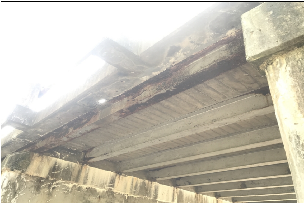
Span 3 Beam 1 active corrosion.
