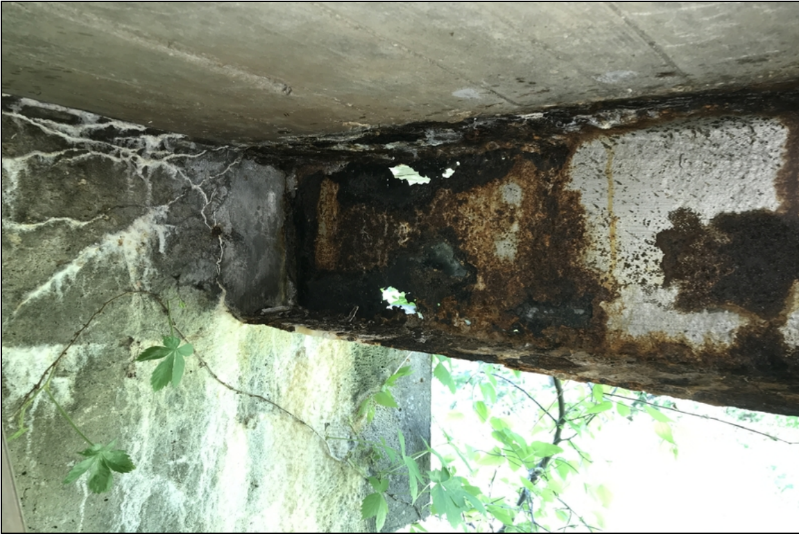
Span # 1. Beam # 9 at Bent # 2. 12" area that is paper thin with multiple holes rusted through the web. Top and Bottom flanges are paper thin and reduced in width to 5".
