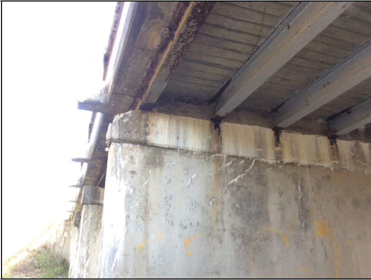
Typical concrete deterioration in the cap of Bent # 4.
