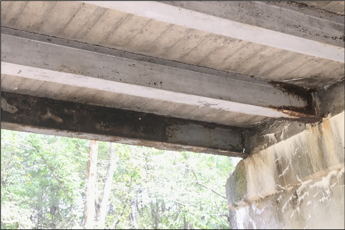
Span 3 Bent 4 active corrosion with holes through the web.
