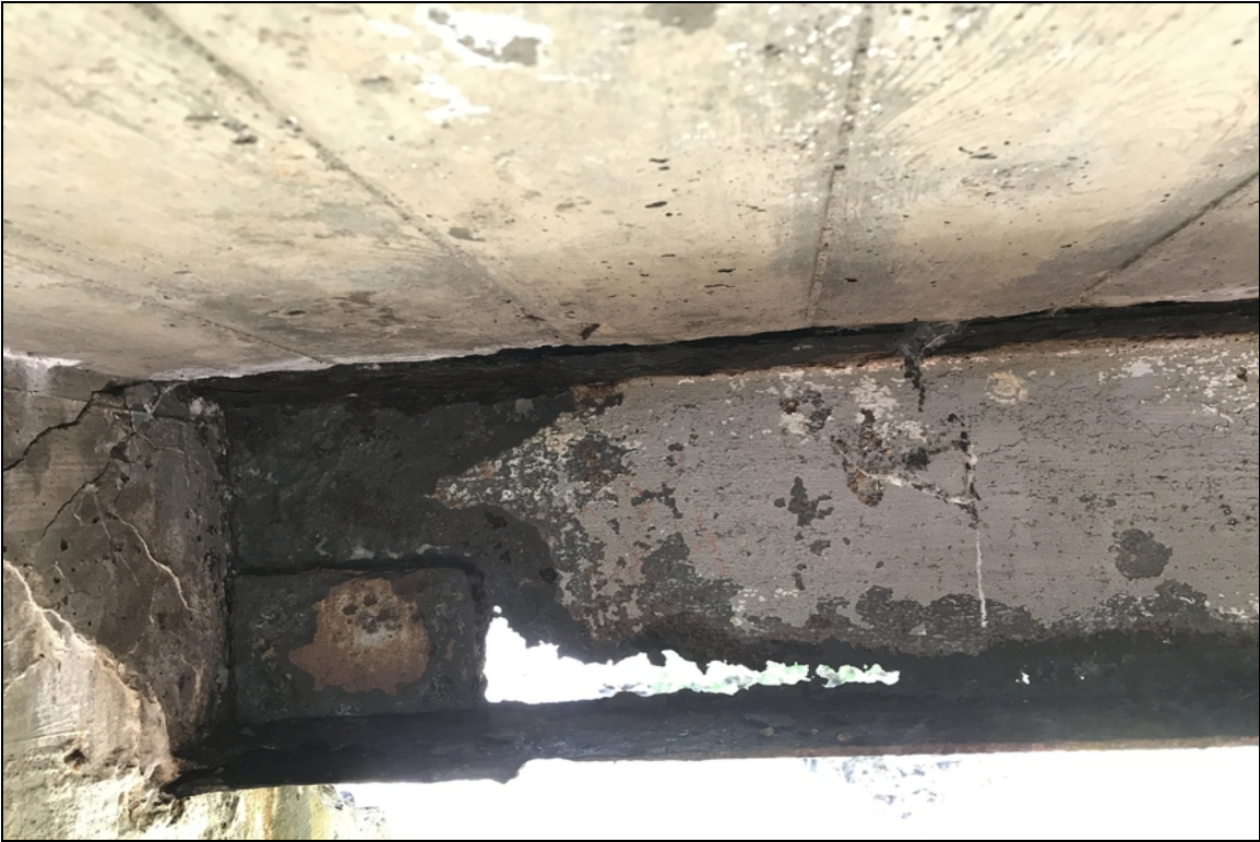
Span # 4- Beam # 1 Bent # 4- 10" x 3" hole adjacent to fish plate repair.
