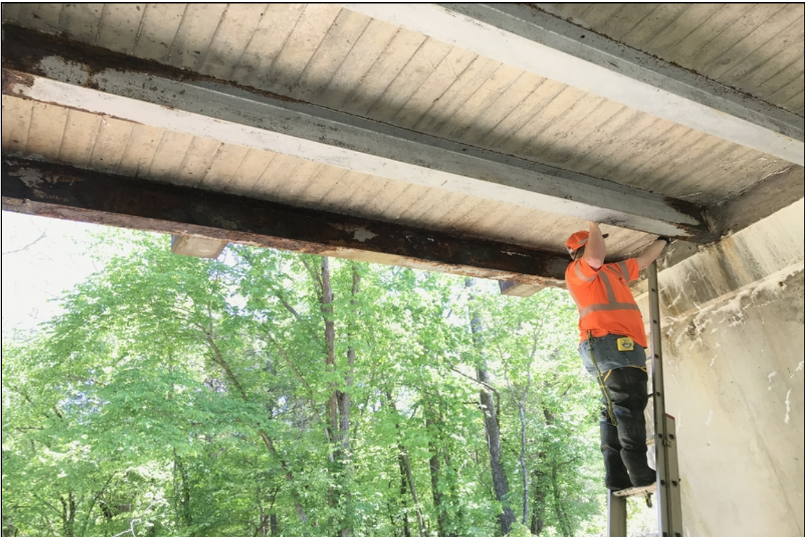
Span # 3. Beam # 1. Active corrosion with multiple holes rusted in the web.
