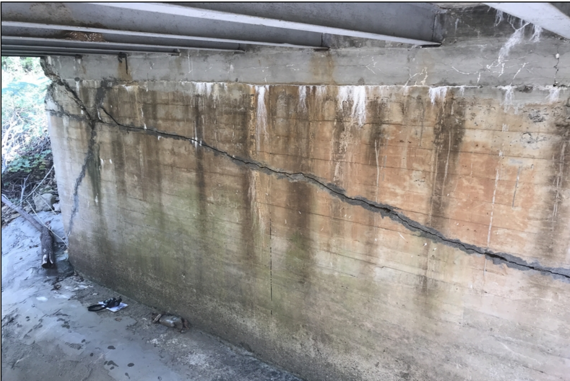
Bent 5 cracking.
