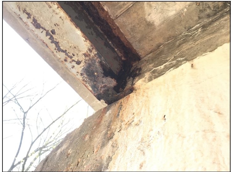
Span # 4, Bent # 4, Beam # 9 has significant section loss to the bottom flange.
