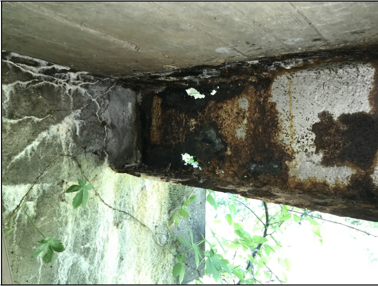
Span # 1. Beam # 9 at Bent # 2. 12" area that is paper thin with multiple holes rusted through the web. Top and Bottom flanges are paper thin and reduced in width to 5".
