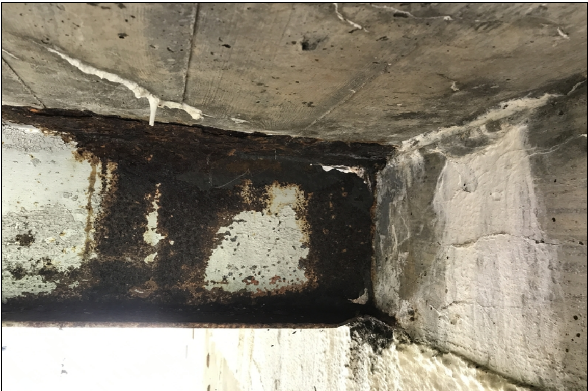
Span 4- Beam 3 Bent 4 face- 4" hole and 1.75" hole, bottom flange is reduced to 2" in width.
