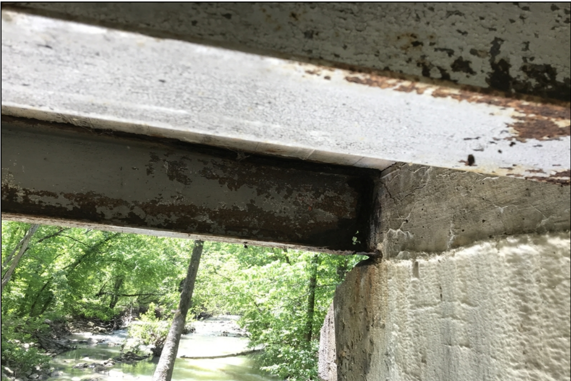
Span # 4 - Beam # 9 Bent # 4 face - Bottom flange has knife edge section loss and is reduced to 2 3/4" in width. The base of web has a 2" hole. Top flange is reduced to 3" in width.
