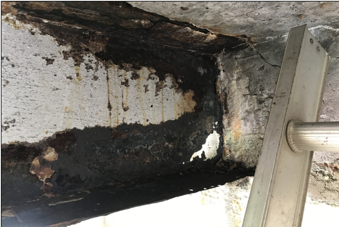
Span # 3 Beam # 2 Bent # 3 - 4" hole in the web at Bent # 3 face.
