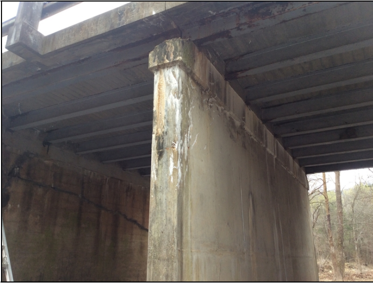
The exterior edges of the intermediate bents have vertical and map cracking with efflorescence.
