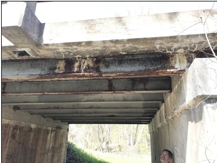
Span # 1 Rt active corrosion in the Beams with soft deteriorated concrete with heavy efflorescence buildup.
