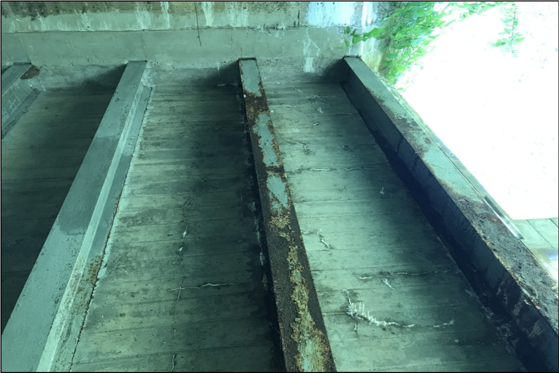
Undersurface of Span # 1. Efflorescence.
