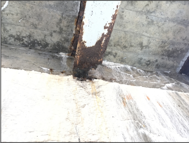
Span # 4, Bent # 4, Beam # 2 has significant section loss to the bottom flange.
