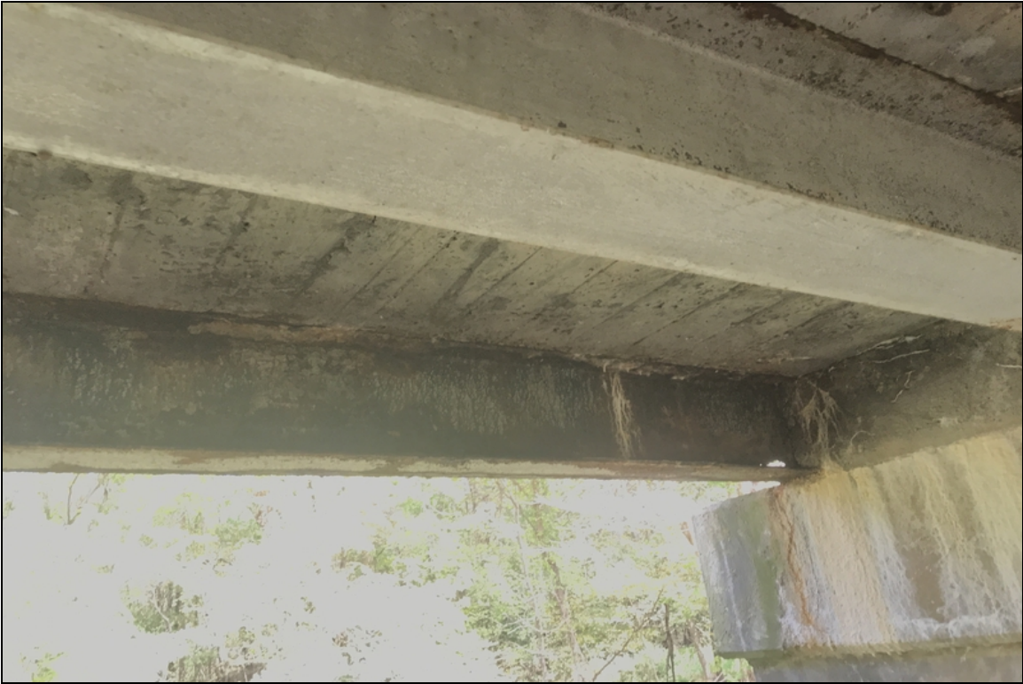
Span 1 Bent 2 holes rusted through the web.
