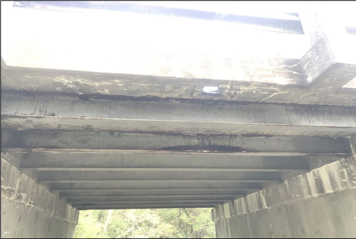
Span 2 Beams 8 & 9 active corrosion.
