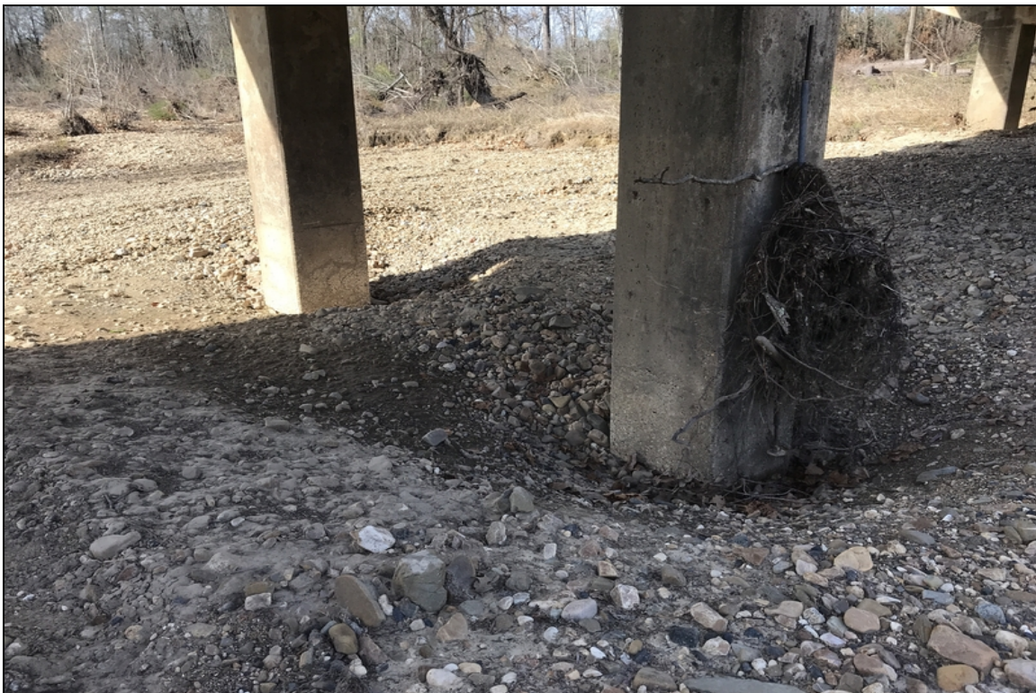
Bent #5 scour around columns
