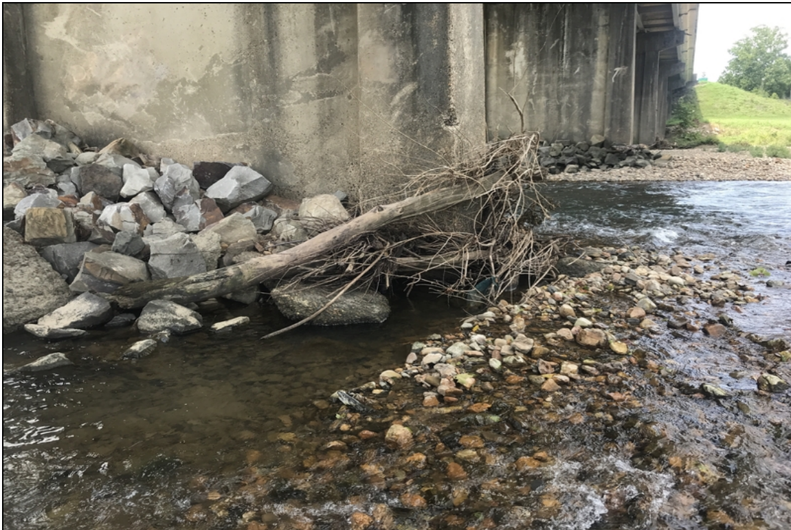
Drift at bent 6
