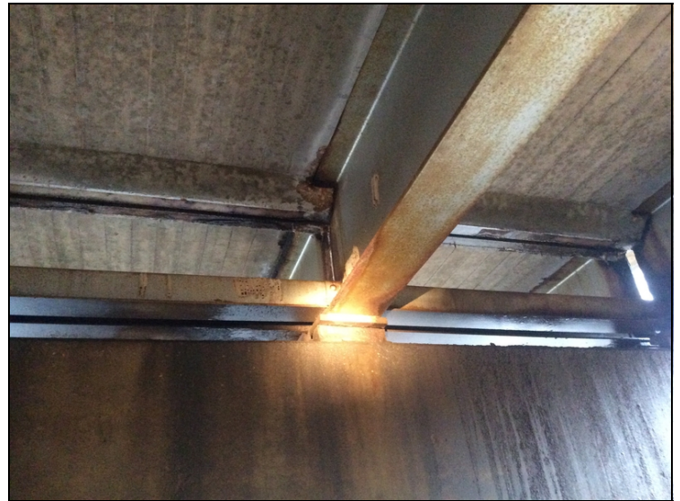
Beam rust typical
