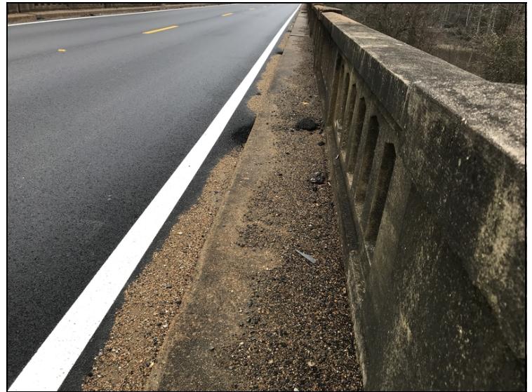
RT side curb and sidewalk has loose asphalt and debris.
