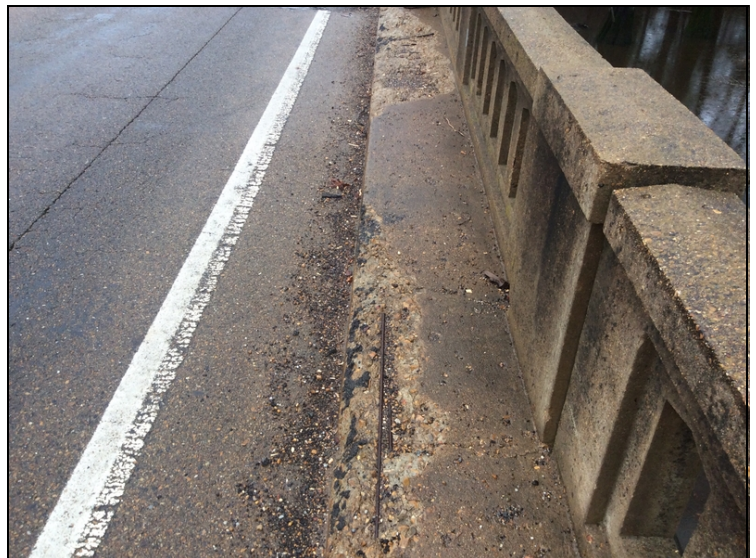
Spalls with rebar exposed curb left side various locations
