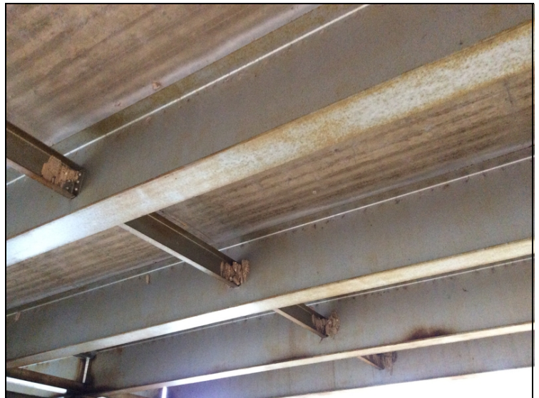
Rust on beams all spans typical
