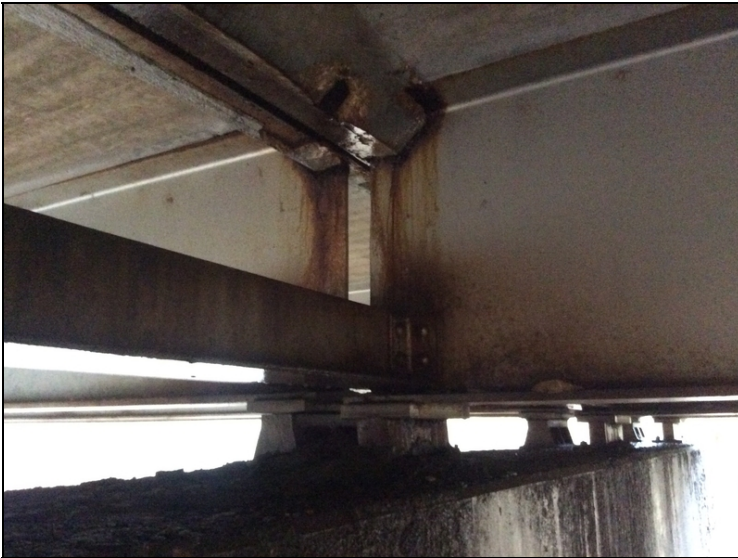
Rust at beam ends
