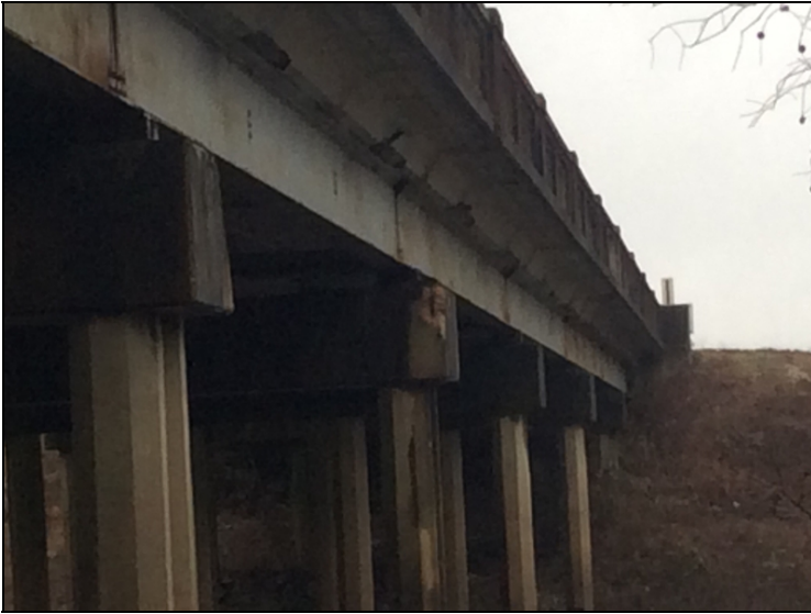
Rebar exposed and spall right end of bent 5 cap
