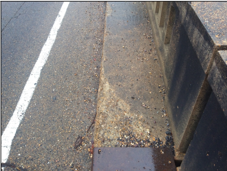
Curb left side various locations spalls
