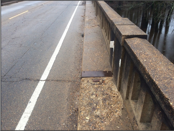
Curb left side spalls various locations
