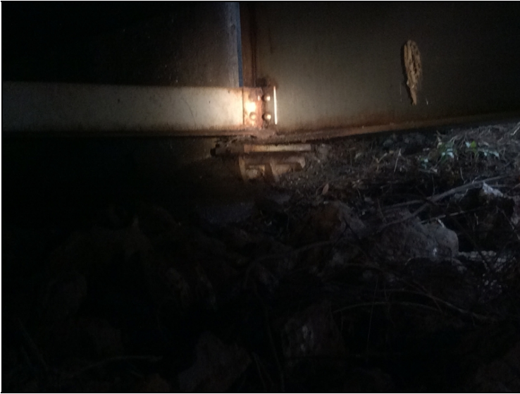
Corrosion end of beam 5 bent 8 pack rust and section loss
