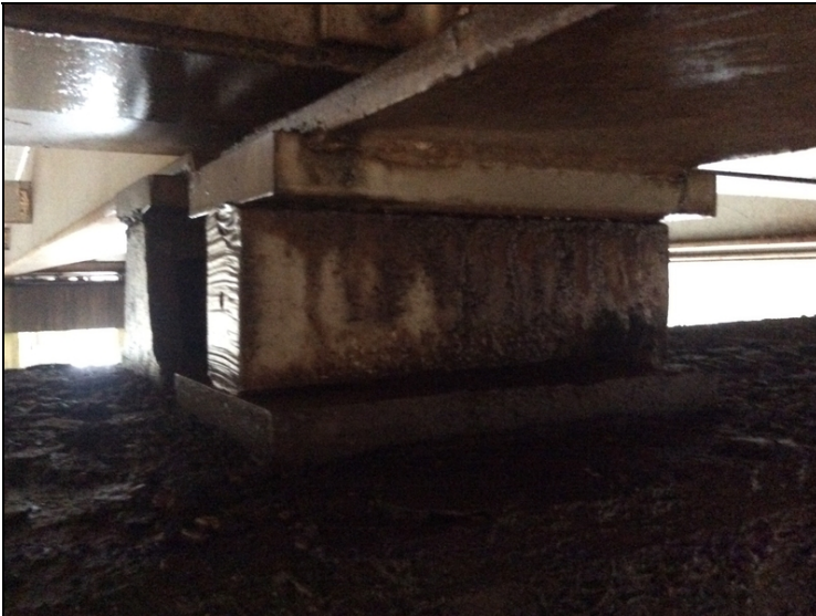
Bearings rust and section loss Bents 1-9
