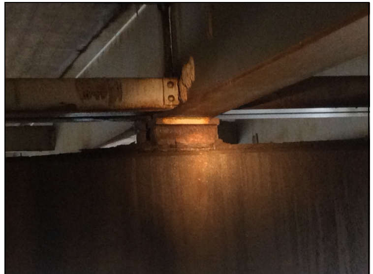
Section loss to bearings
