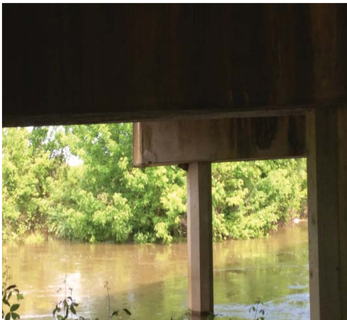
PHOTO 1 Description Delam bent 4 cap left end west face
