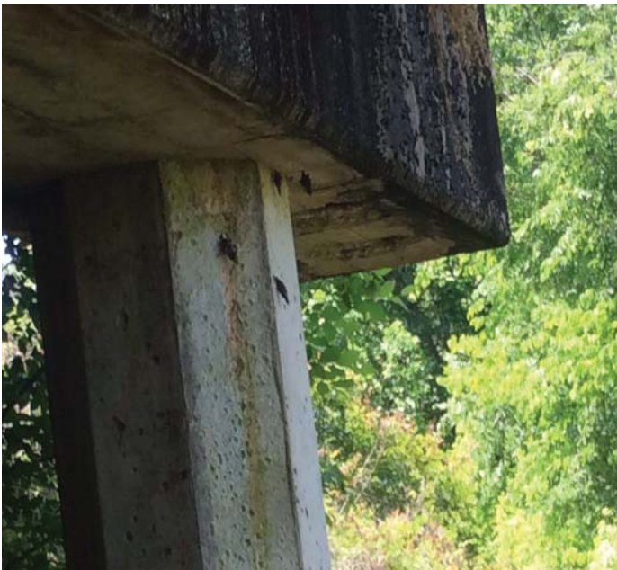
PHOTO 1 Description SPALLS on the left end of cap at bent 2
