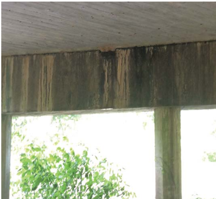
PHOTO 1 Description Delam between pile 1 and 2 west face of bent 3 cap.
