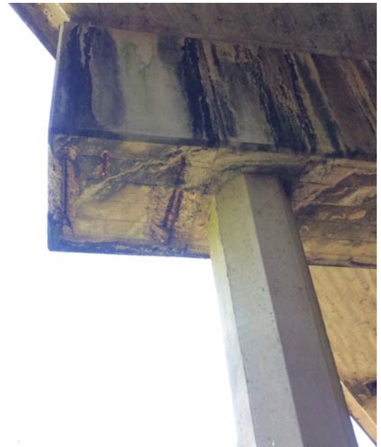
PHOTO 2 Description Spalls at the left end of cap at bent 3
