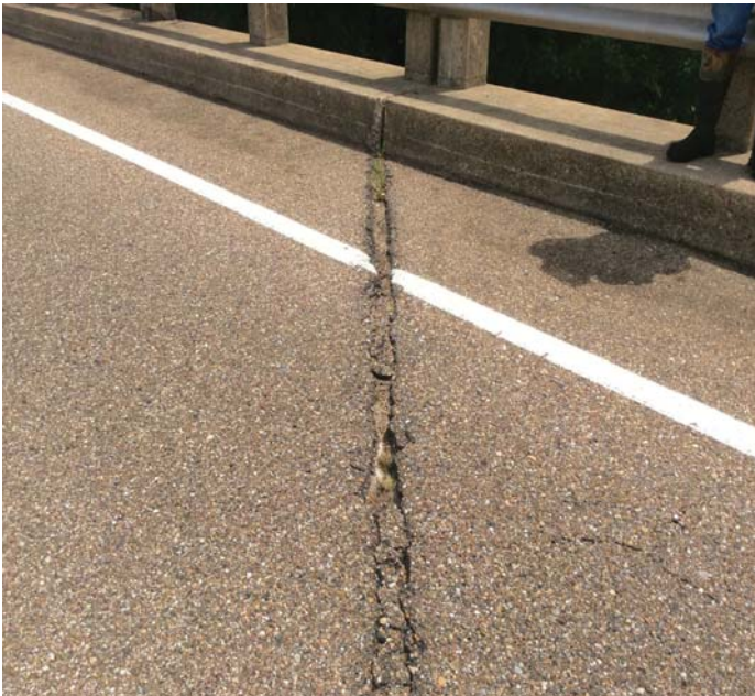
PHOTO 1 Description Joints need cleaning some have grass growing
