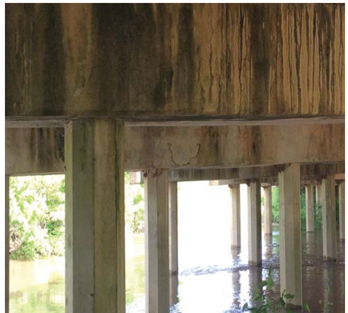
PHOTO 2 Description Delam bent 4 cap between pile 2 and 3 west face
