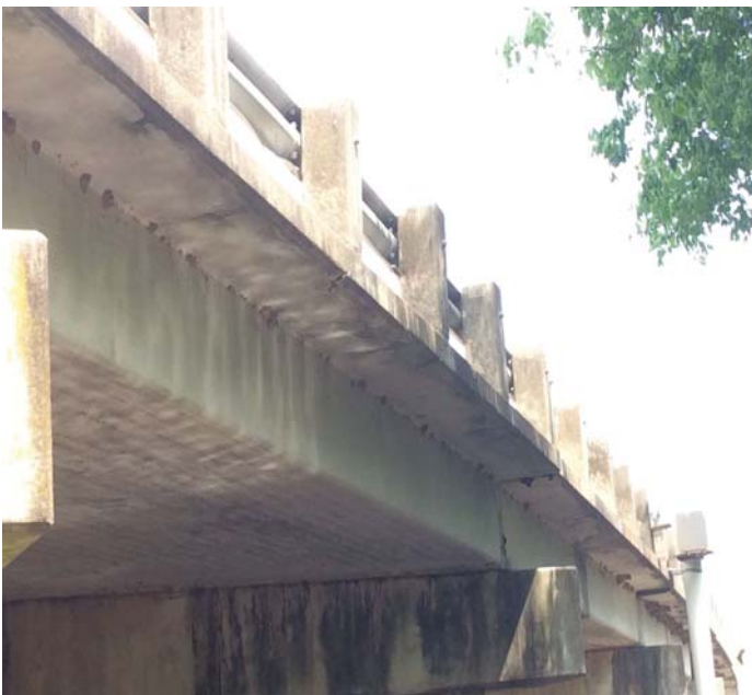
PHOTO 1 Description Span 3 overhang right side delams under guard rail posts
