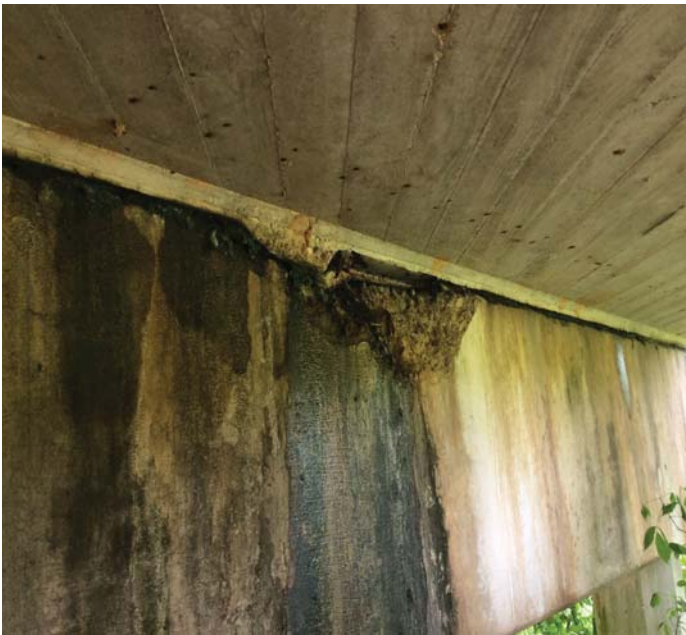
PHOTO 1 Description Bent 9 east face top of cap between piles 1 and 2. 2' x 18" spall
