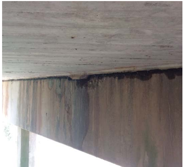
PHOTO 2 Description Bent 9 east face top of cap between piles 4 and 5. 1' x 6" spall
