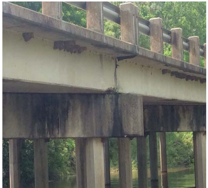
PHOTO 2 Description Spall bent 7 corner of slab left side rebar exposed
