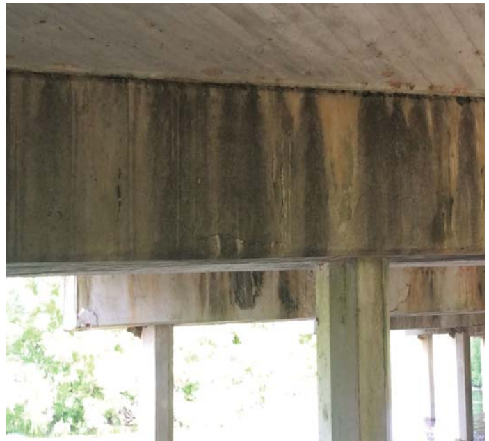
PHOTO 2 Description Delam between pile 2 and 3 west face of bent 3 cap.
