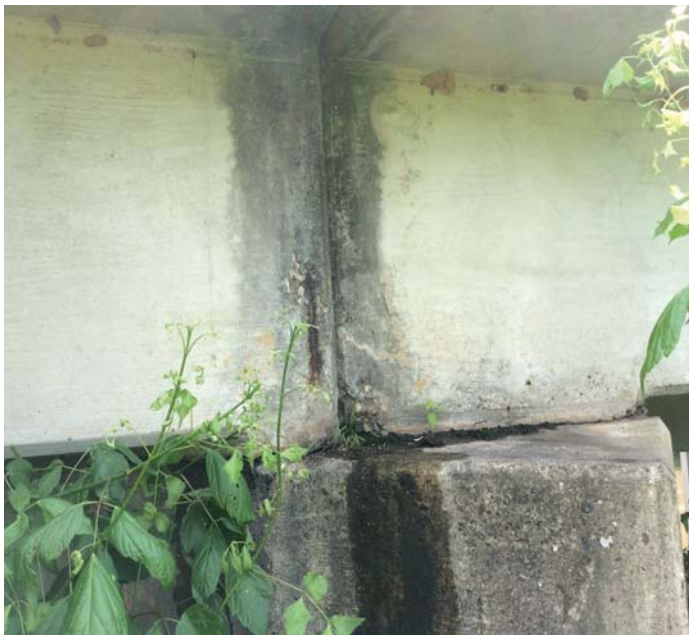
PHOTO 1 Description Spall bent 9 left side corner of slab
